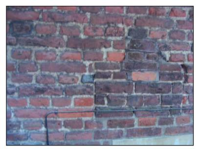
Plate 4: Type I Wren bricks used on infill patch face 1
