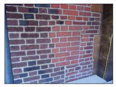
Plate 5: Type I Wren bricks beside north facing elevation ground floor window
