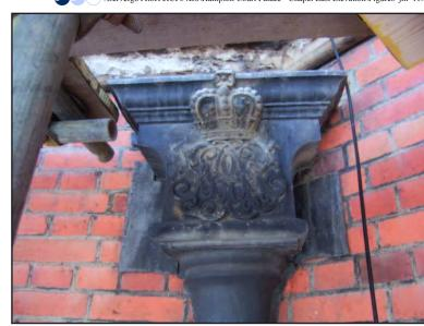
Plate 18: George IV lead hodder and 19th century brickwork
