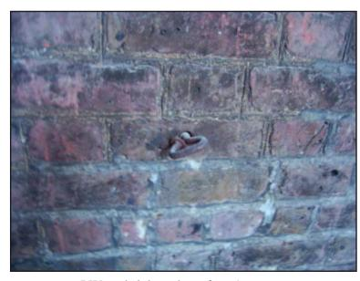
Plate 3: Type I Wren brickwork on face 1
