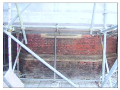
Plate 8: Type T brickwork on plinth
