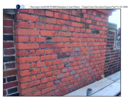
Plate 14: Victorian diaperwork on north elevation chimney type T bricks
