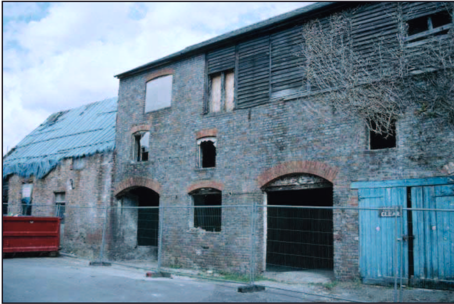
Plate 1: West elevation, showing two and three storey ranges
