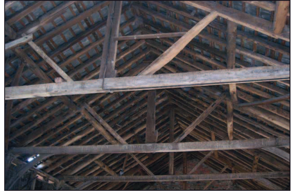
Plate 15: Roof of 3-storey range from north end
