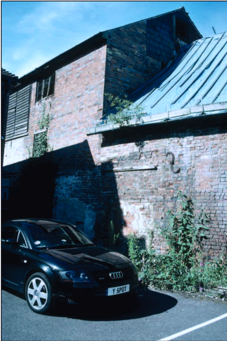
Plate 10: East elevation, three storey range
