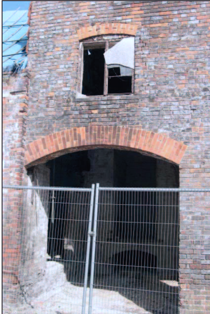
Plate 5: West elevation, three storey range, south door and window
