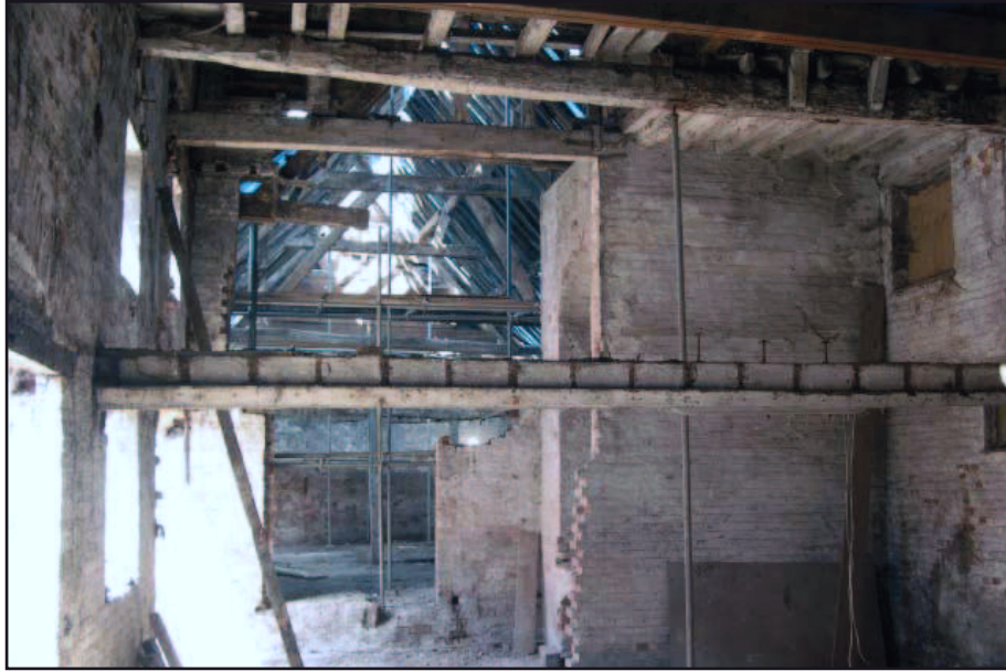
Plate 14: General internal view of 3-storey range from south end
