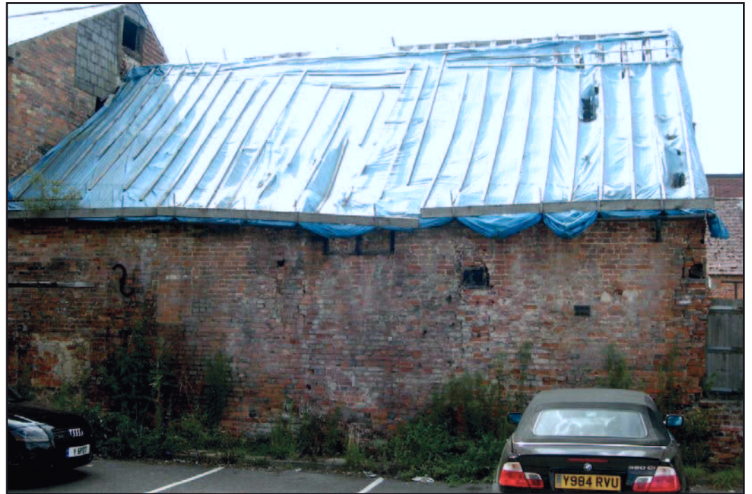
Plate 11: East elevation, two storey range
