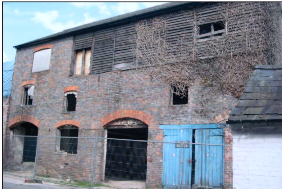
Plate 3: West elevation, three storey range, north door
