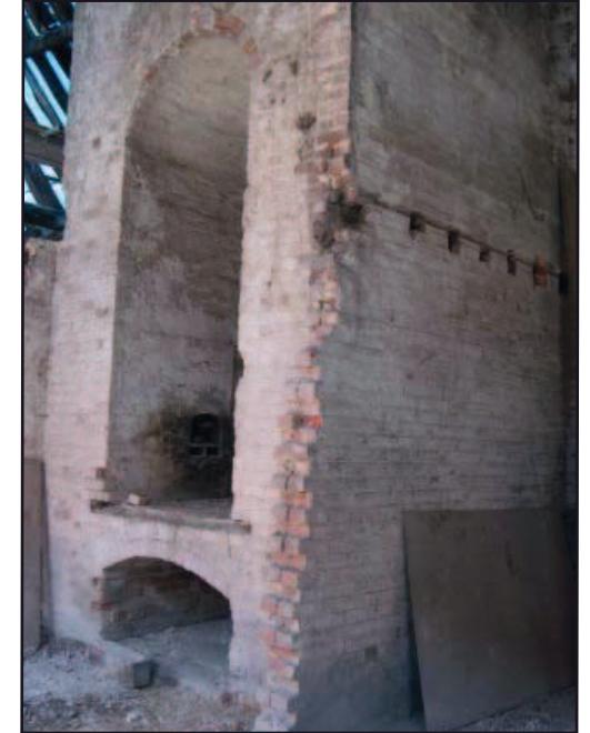
Plate 17: Brick structure which supported brewhouse furnace at top
