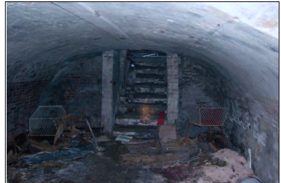
Plate 25: Southernmost cellar with access steps to off-license
