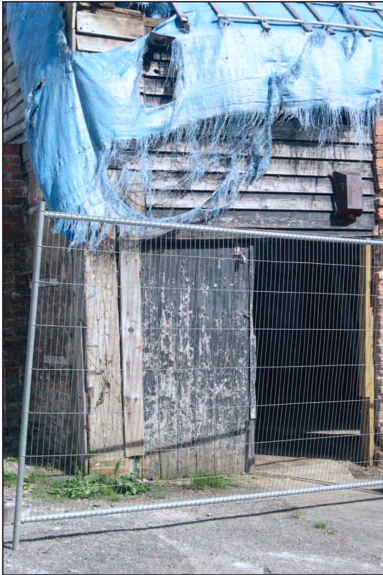
Plate 8: West elevation, two storey range, south door
