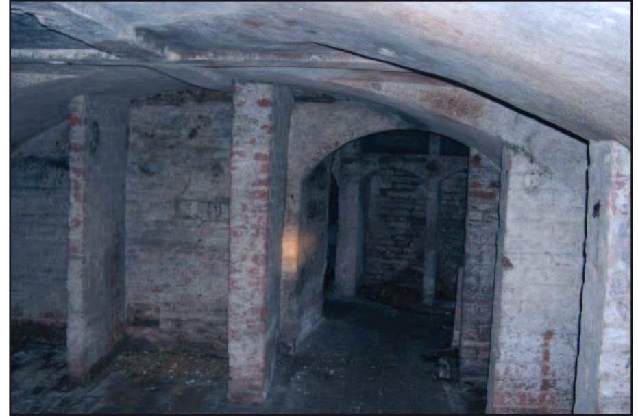
Plate 23: Cellar beneath 2-storey range
