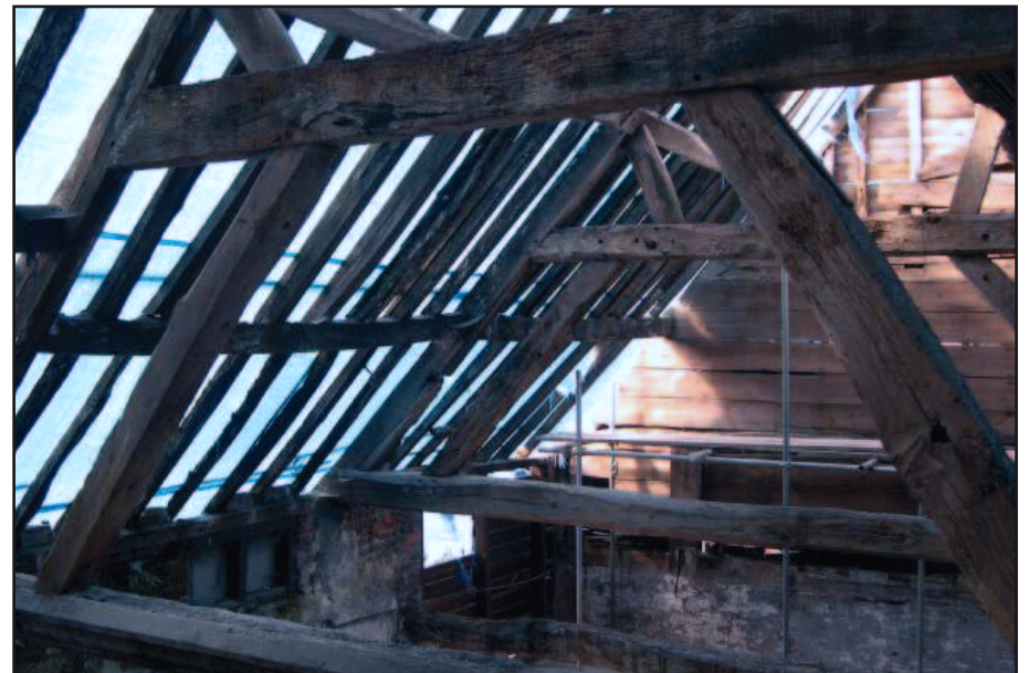
Plate 21: Roof structure in 2-storey range from south end
