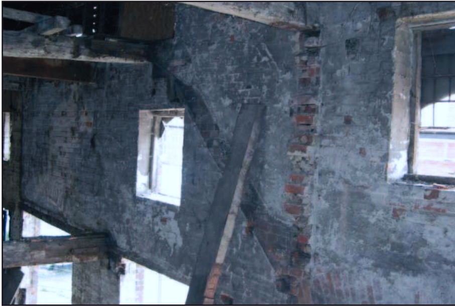
Plate 18: Imprint of former stairs at north-west corner of 3-storey range
