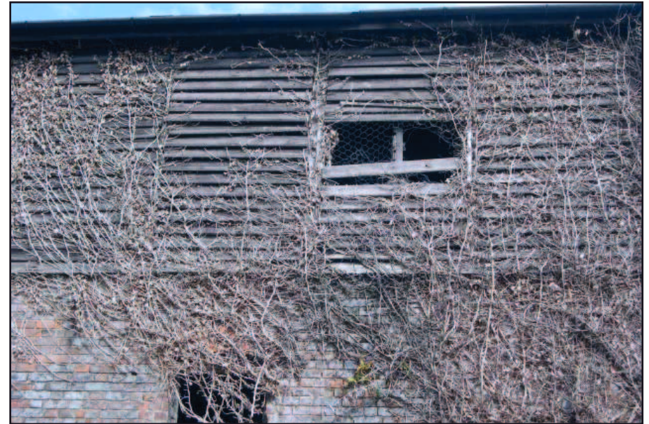
Plate 6: West elevation, wood louvres
