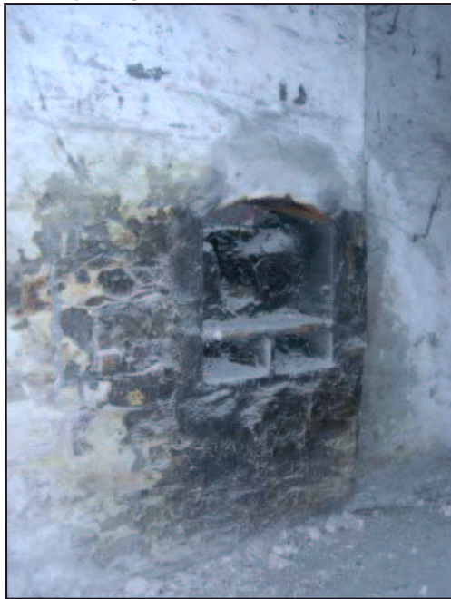
Plate 16: Shaft bearing box at north end of 3-storey range
