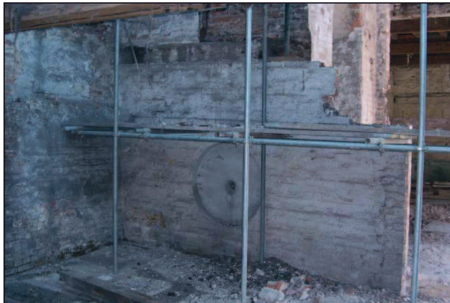
Plate 20: South end of 2-storey range with imprint from former drive wheel
