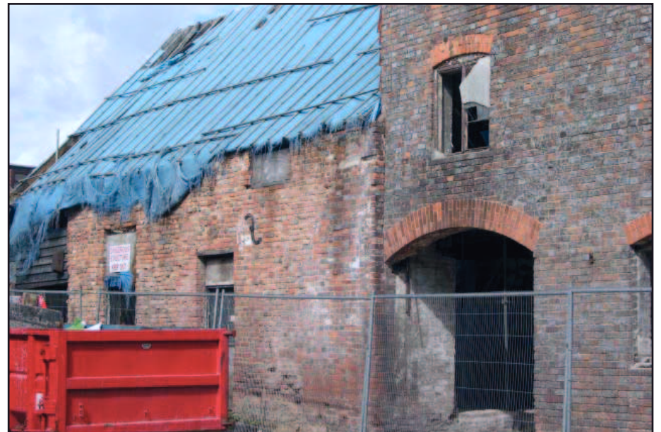
Plate 7: West elevation, two storey range
