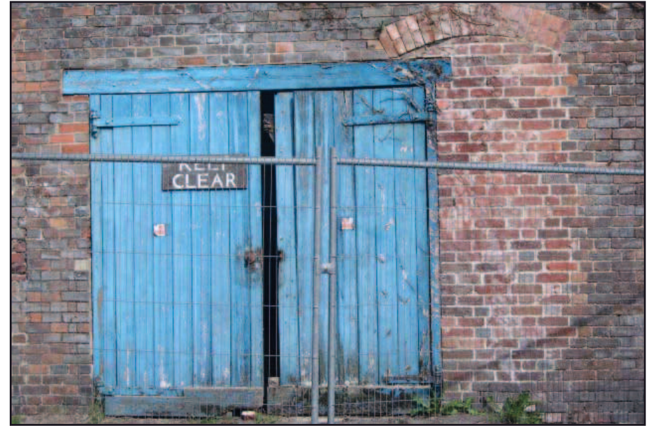
Plate 2: West elevation, three storey range
