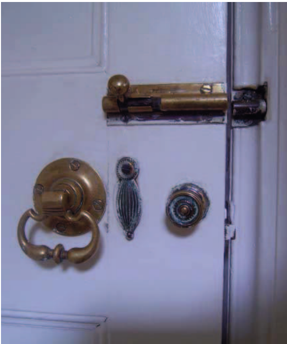
Plate 77: Second floor bathroom door fittings
