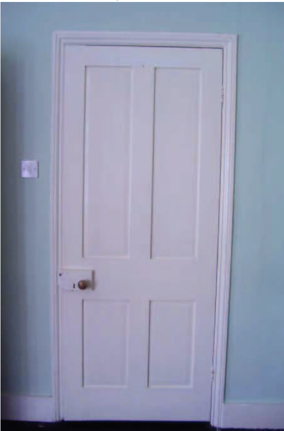
Plate 83: Northend door, north-west bedroom facing east
