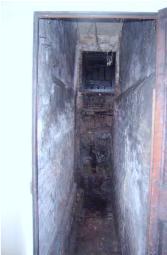
Plate 43: Coal cellar, facing west
