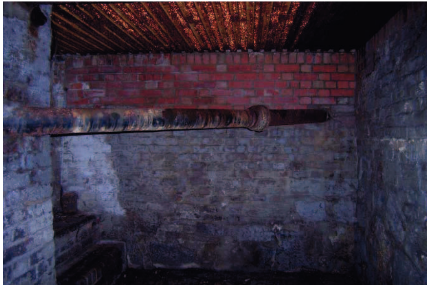
Plate 95: South wall of underground cellar
