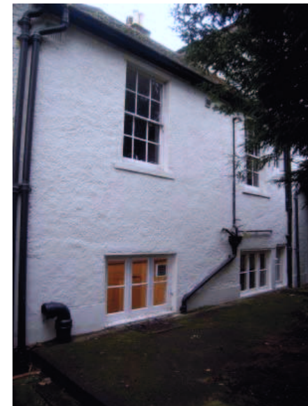
Plate 8: West elevation, Victorian extension
