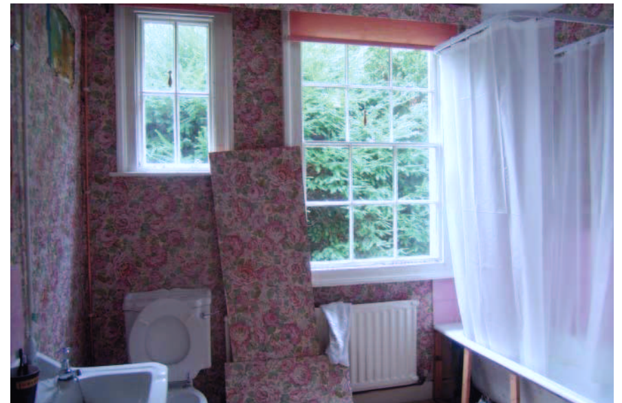
Plate 64: First floor bathroom windows, facing west
