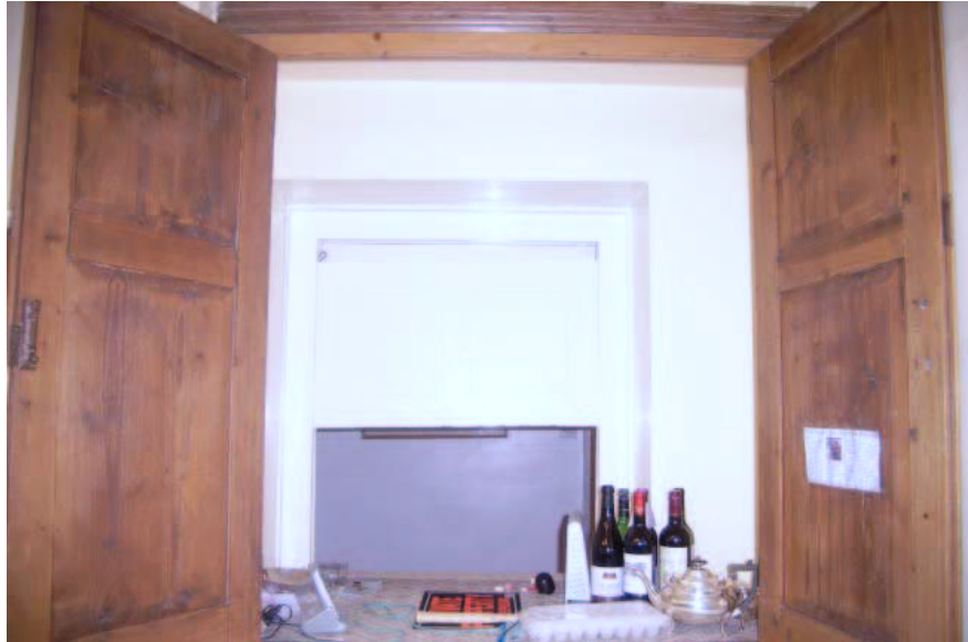
Plate 29: Serving hatch, facing south
