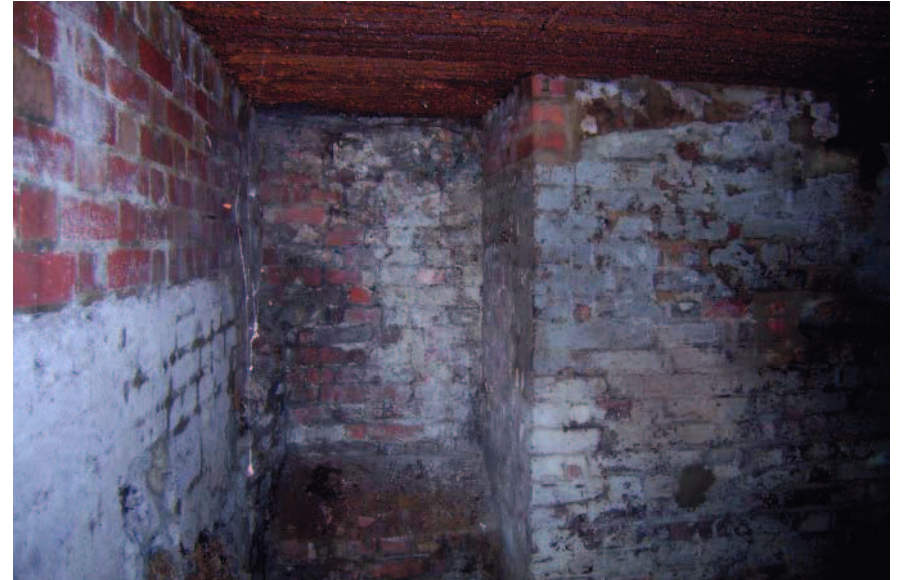
Plate 94: East wall of underground cellar
