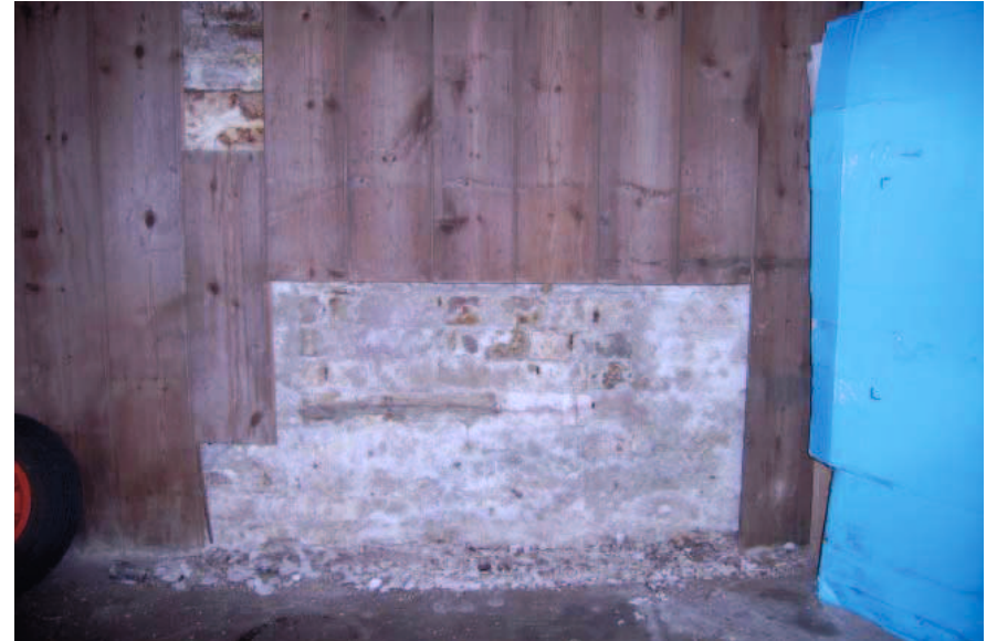
Plate 90: Interior of coach house, visible brickwork in west wall
