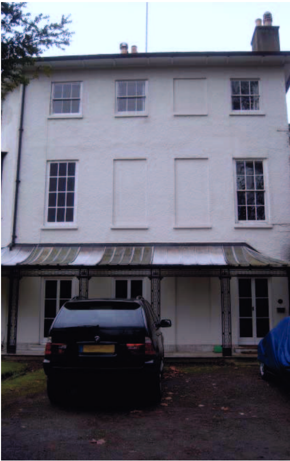
Plate 1: East elevation of Original House
