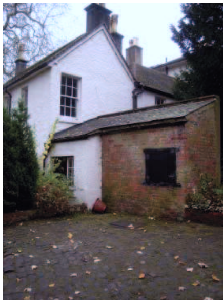
Plate 7: West elevation, Victorian extension
