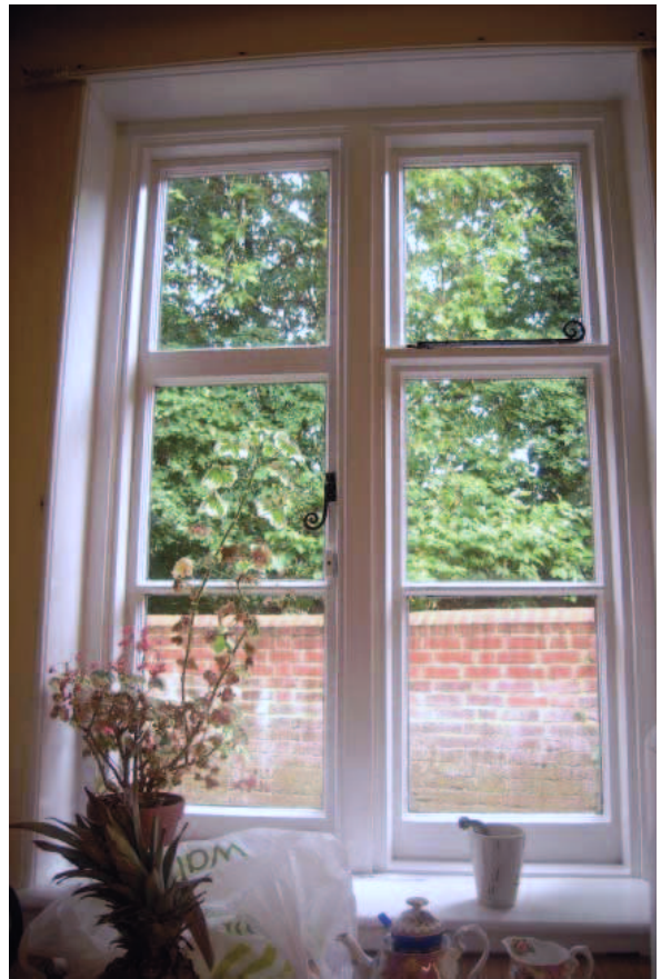
Plate 34: Kitchen window, facing east
