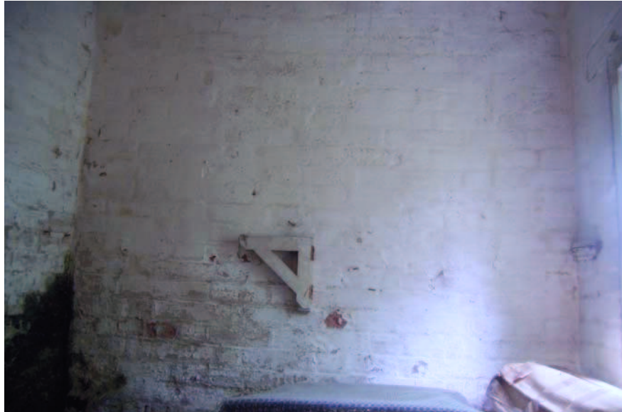
Plate 93: Interior of storeroom, facing west
