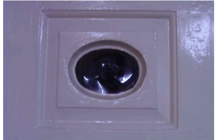
Plate 32: Window in kitchen door
