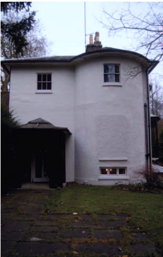
Plate 3: West elevation of Original House
