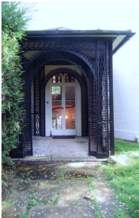
Plate 4: Main entrance, west elevation
