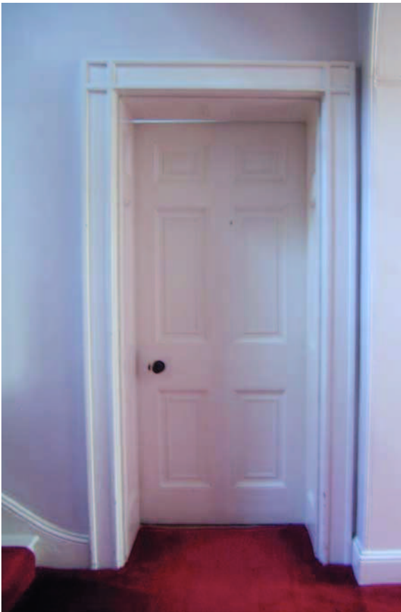
Plate 51: Bathroom door, facing north
