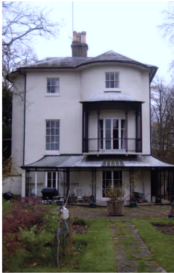
Plate 2: South elevation of Original House
