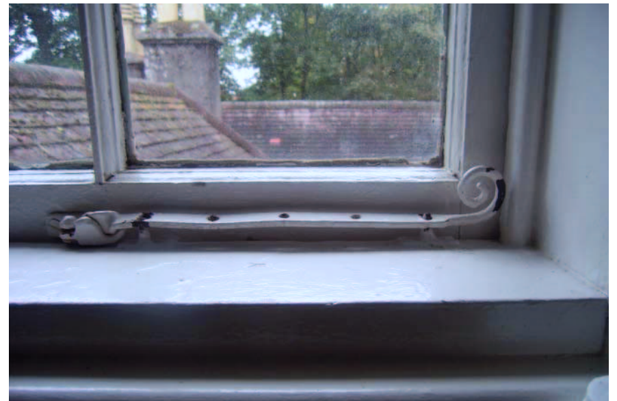
Plate 76: Second floor bathroom window, facing north
