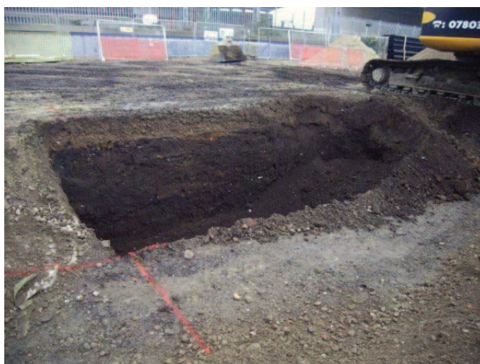
Plate 3: General view of SWINT 3, looking south
