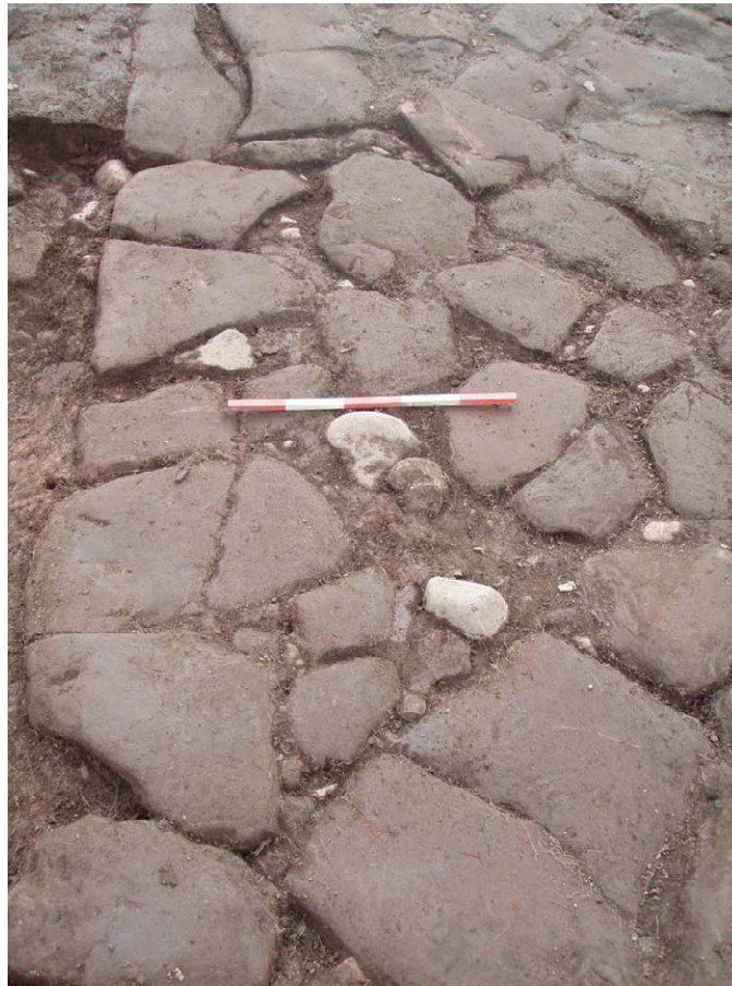
Plate 23: Sandstone surface 10681, in the external area between the central and southern building plots, looking west
