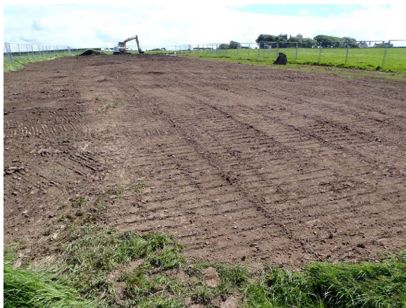
Plate 6: Trench 5 backfilled at the end of the 2014 season, prior to reseeding, looking east
