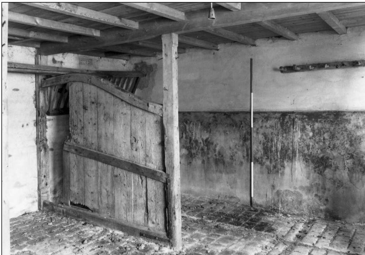
Photo 56: Stable in brick building to south of aisled barn
