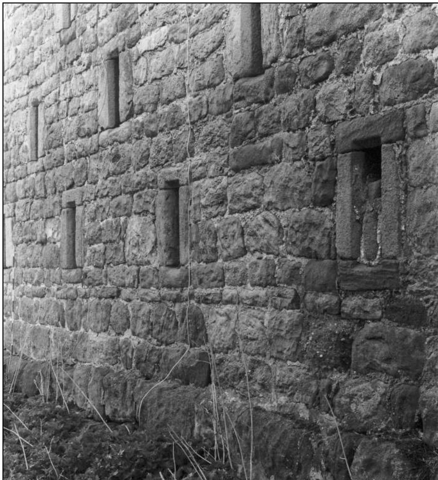
Photo 18: North gable: detail of breathers and footings
