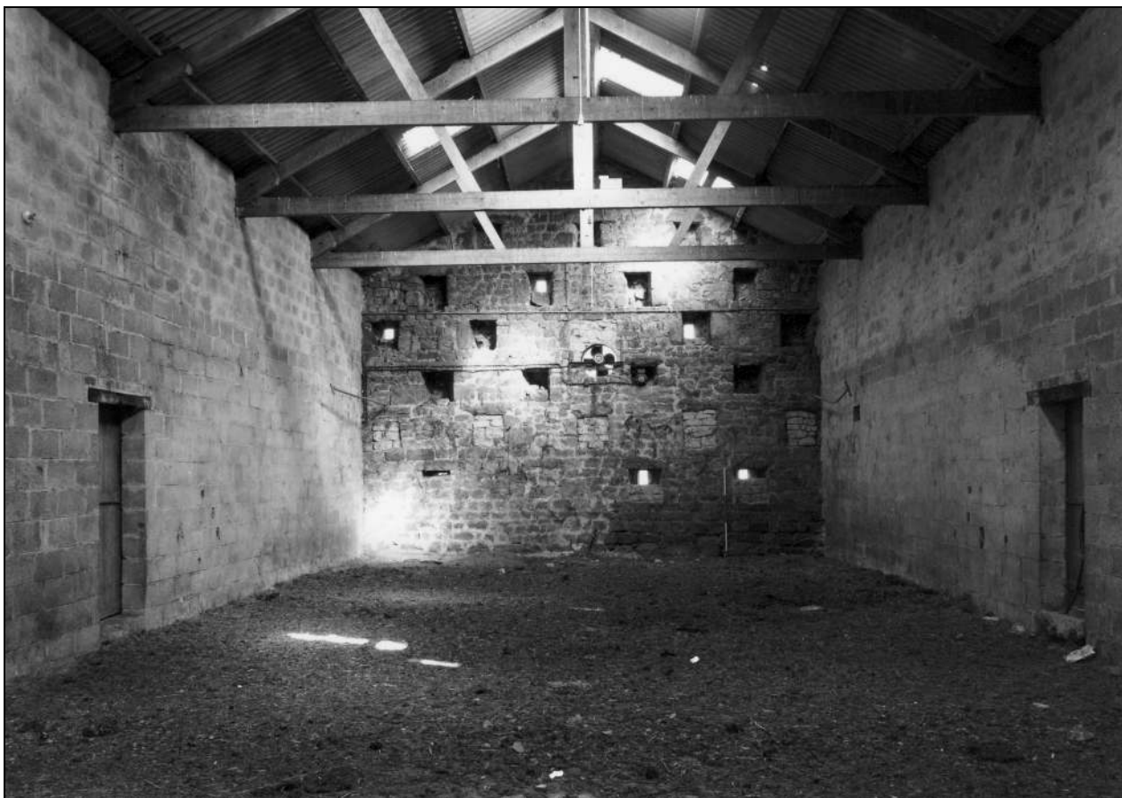
Photo 39: Interior of north end of aisled barn, from the south
