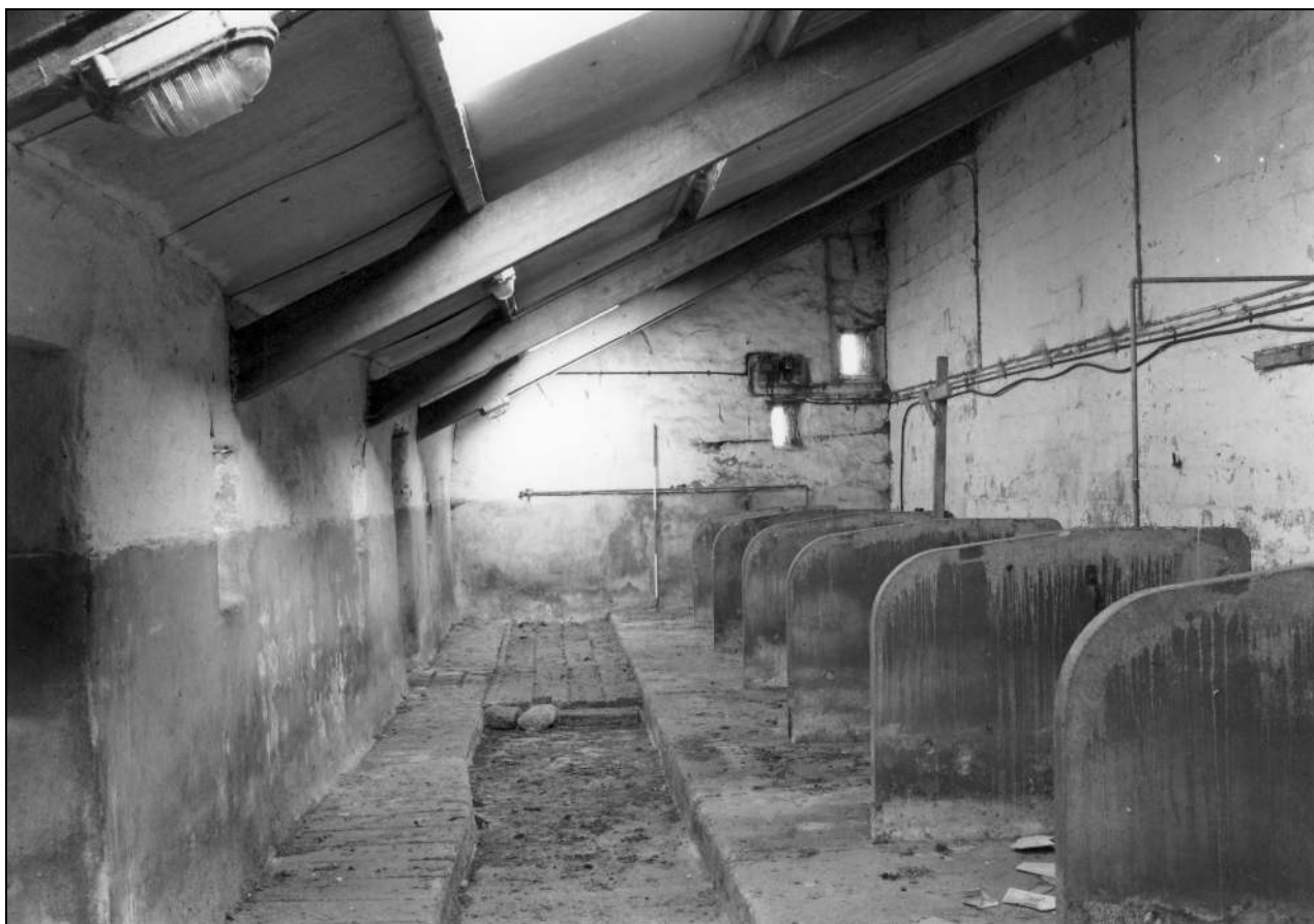
Photo 41: North-west shippon: interior, from the south
