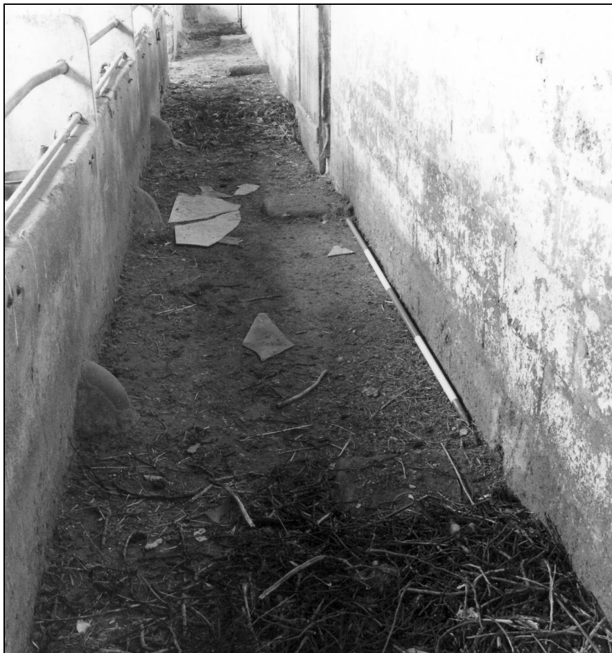
Photo 38: Padstones in feeding passage of north-west shippon, from the south
