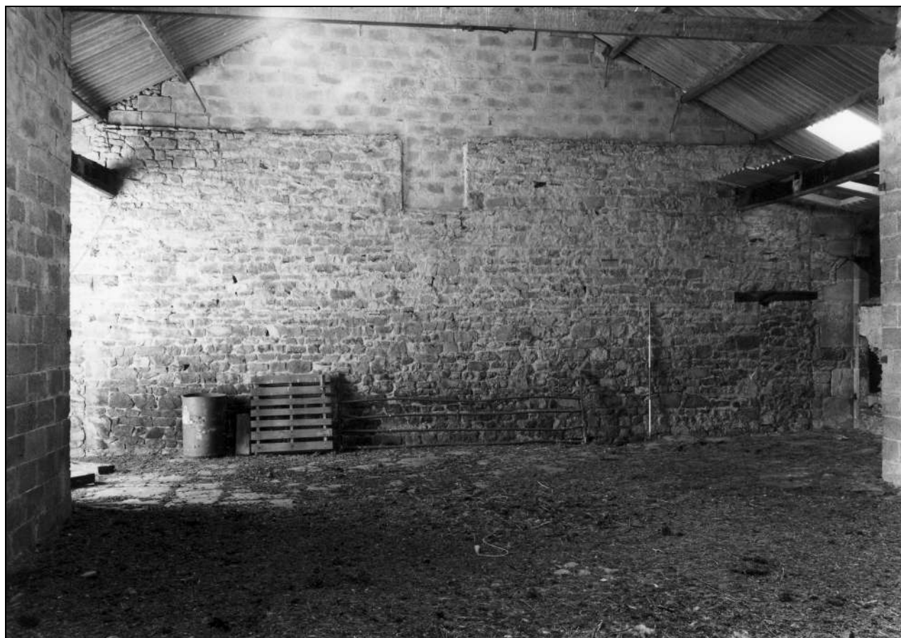
Photo 25: Inserted cross wall in aisled barn, from the north
