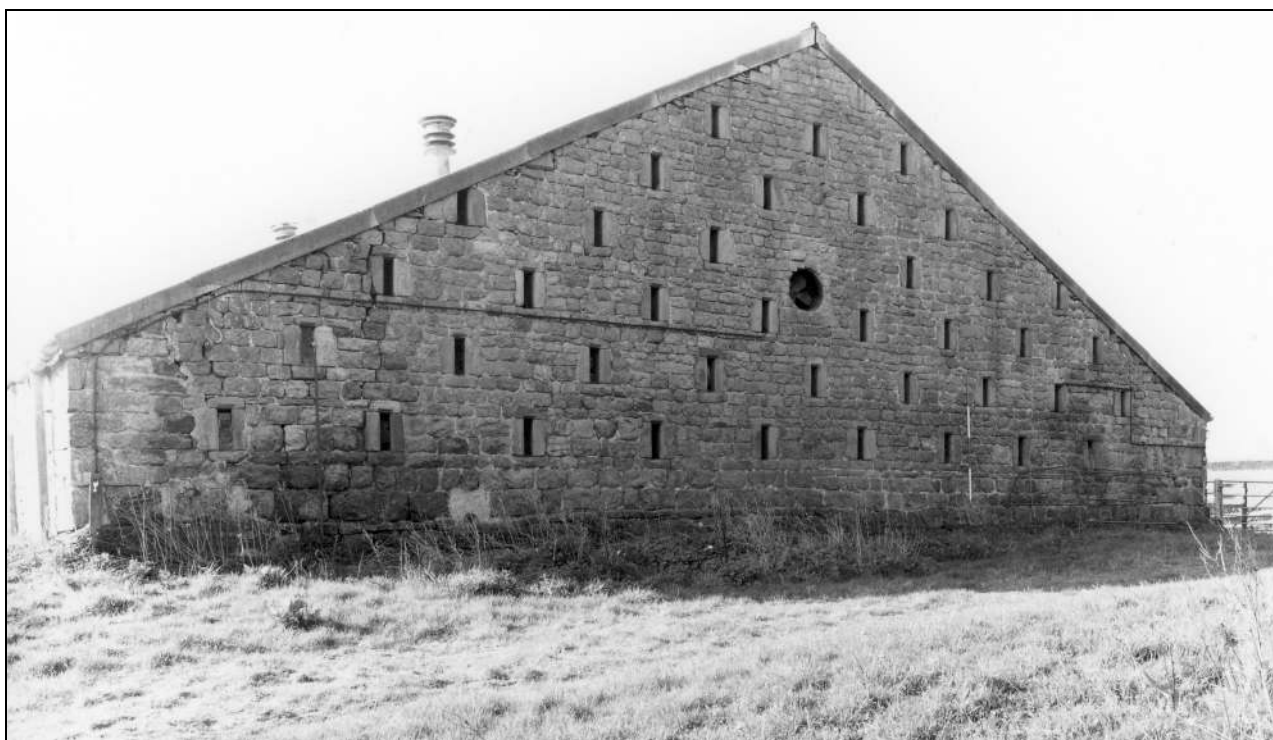
Photo 17: The north gable
