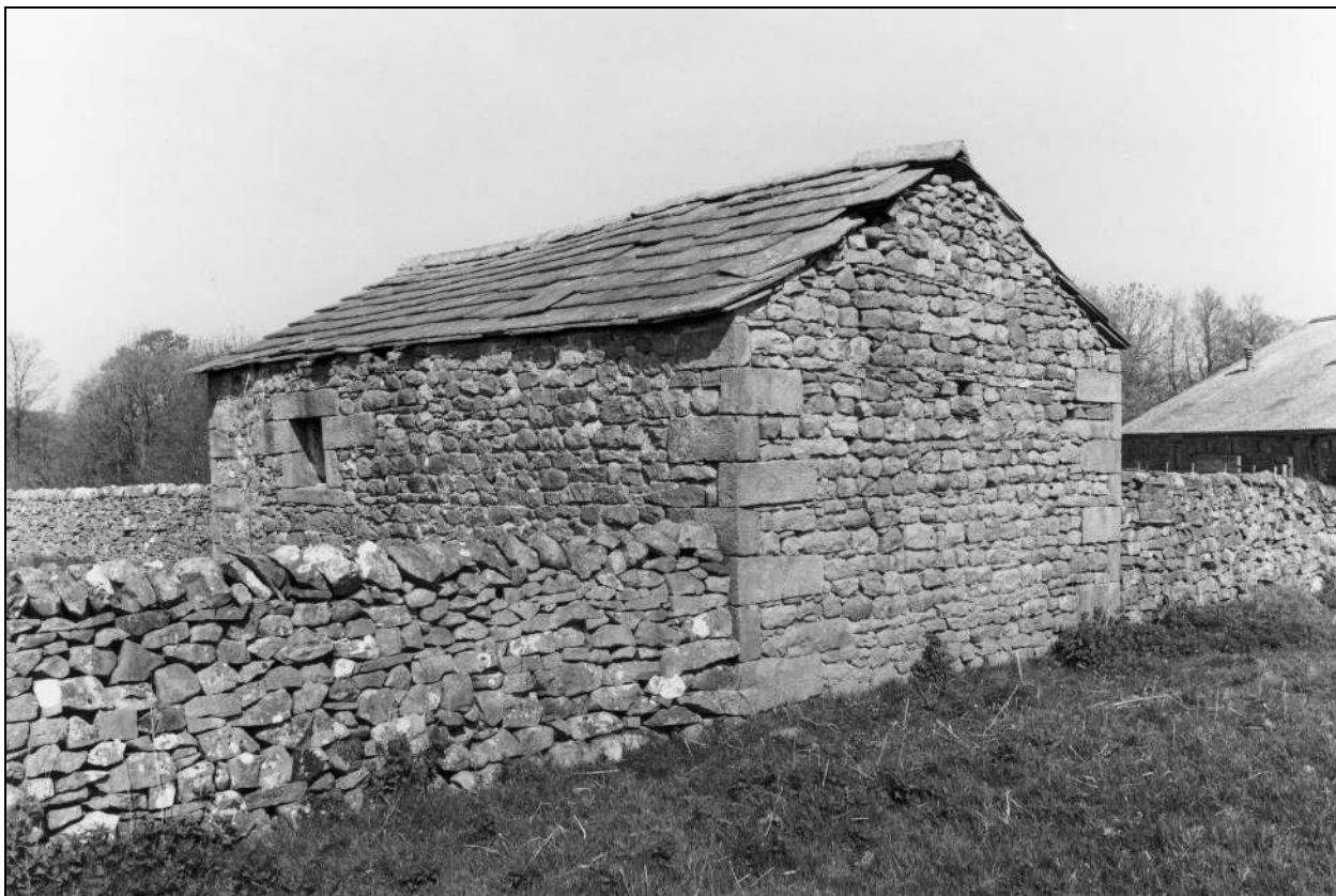
Photo 53: Detached building to west of barn, from the south-east
