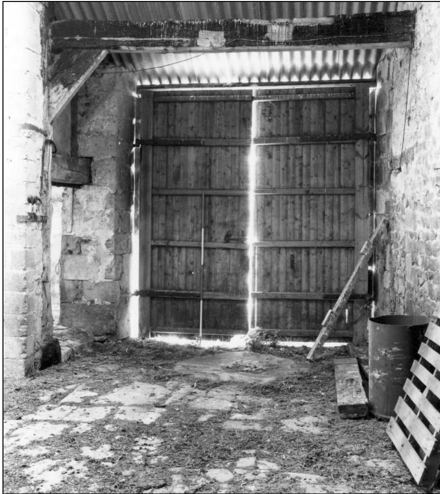
Photo 20: Interior view of east cart entry to aisled barn
