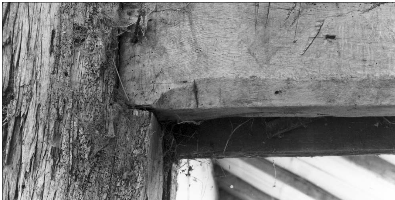
Photo 32: Detail of chamfer and stop on east aisle tie (south side)
