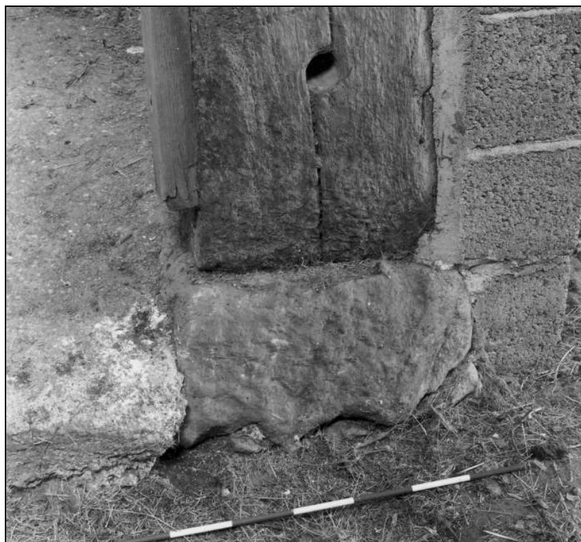
Photo 31: Detail of foot of west arcade post, and padstone, from the south
