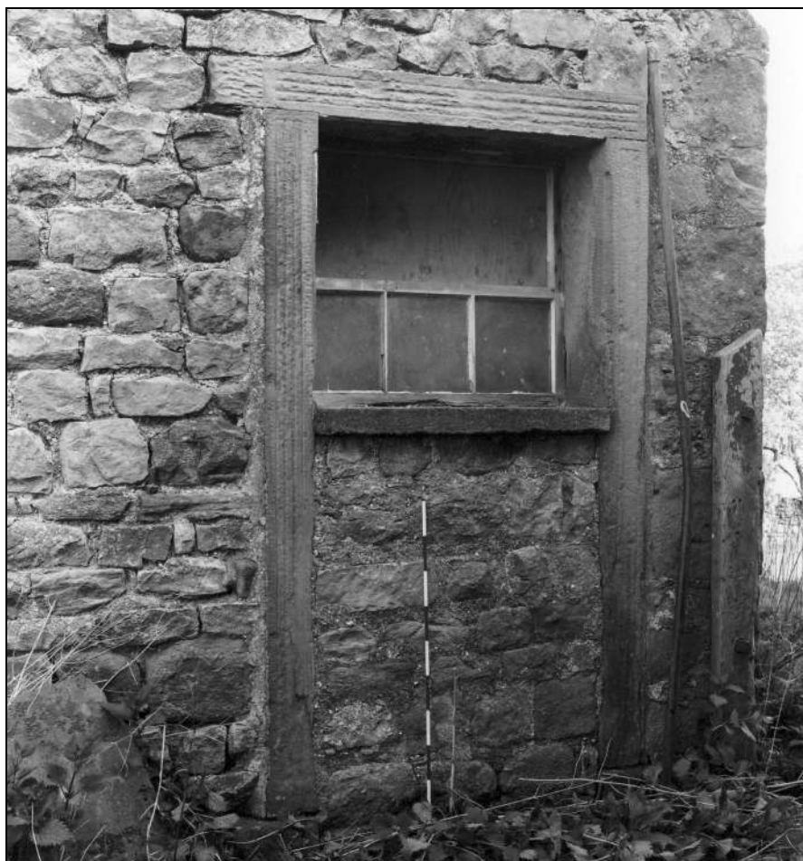
Photo 48: South extension: detail of doorway in south gable
