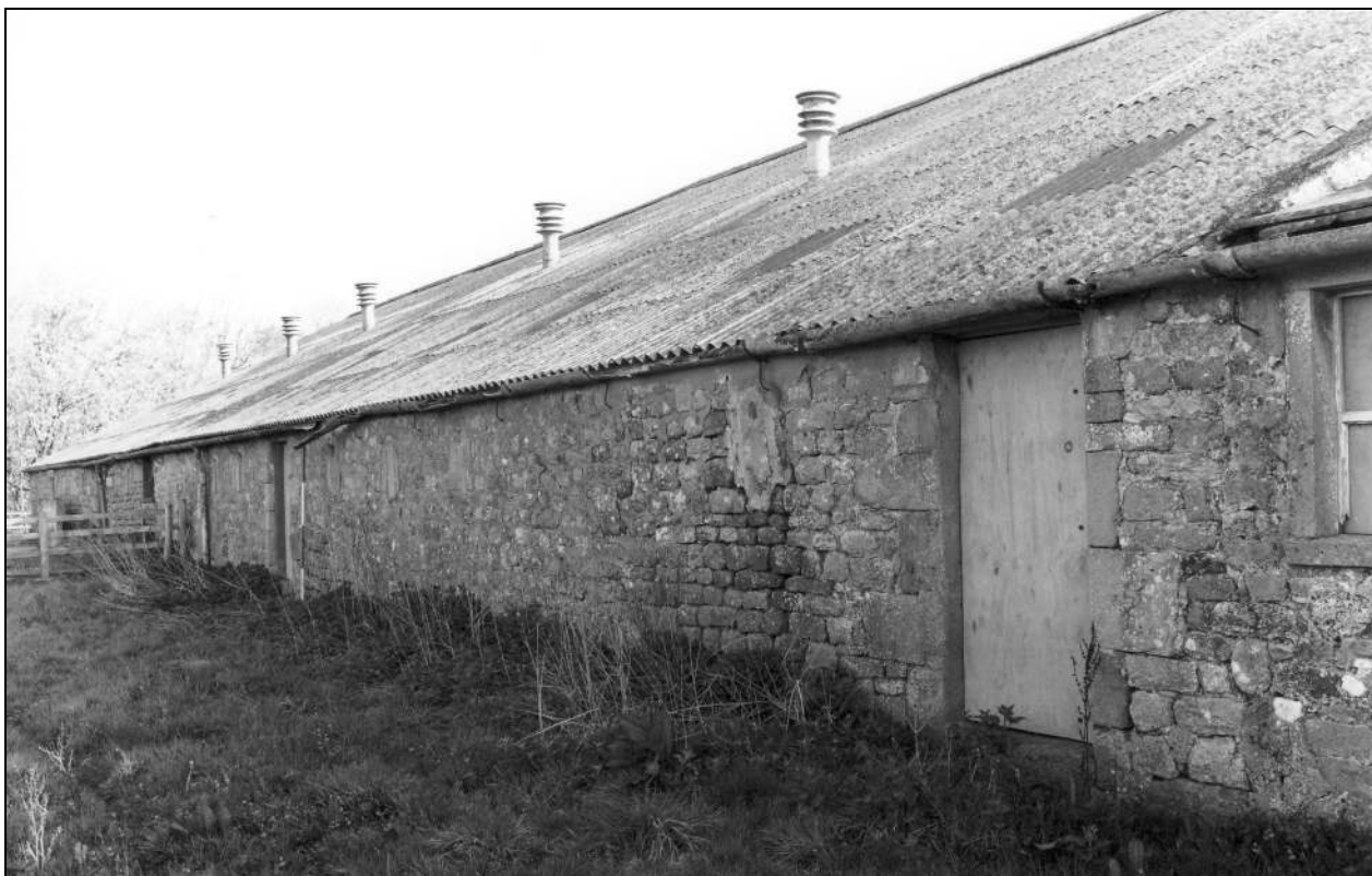
Photo 16: West elevation of original barn, from the south-west
