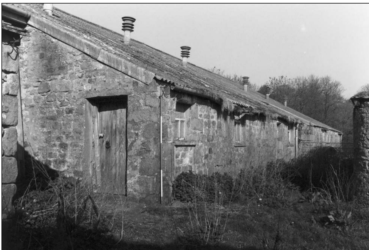
Photo 12: South-east shippon, from the south-east: truncated, and with inserted openings
