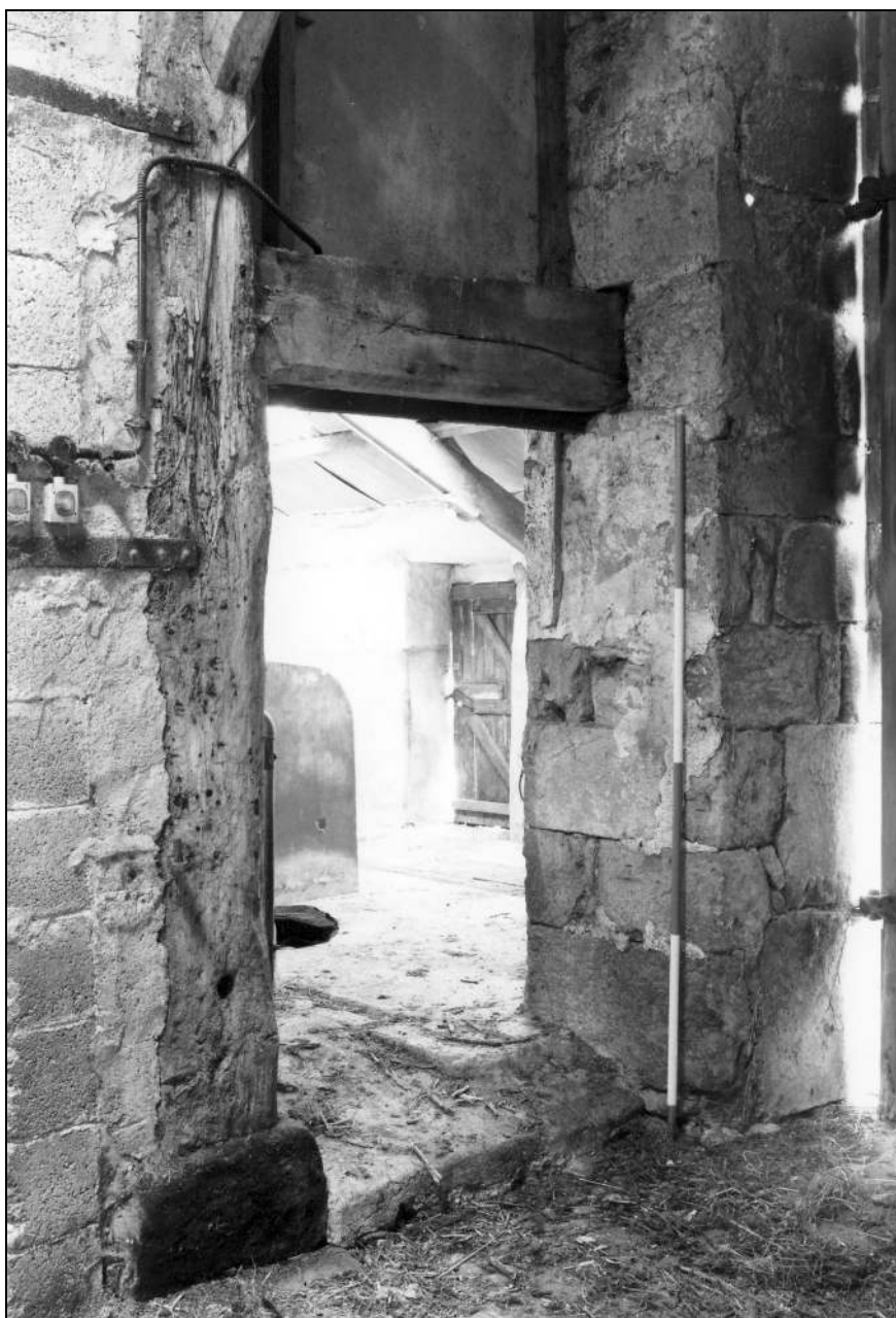
Photo 28: Lower part of arcade post and end of aisle tie, by east cart entry
