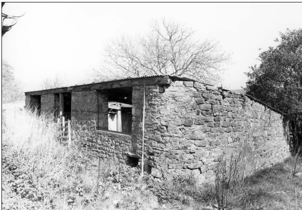
Photo 54: Detached building to east of barn (covered middenstead), from the south-west
