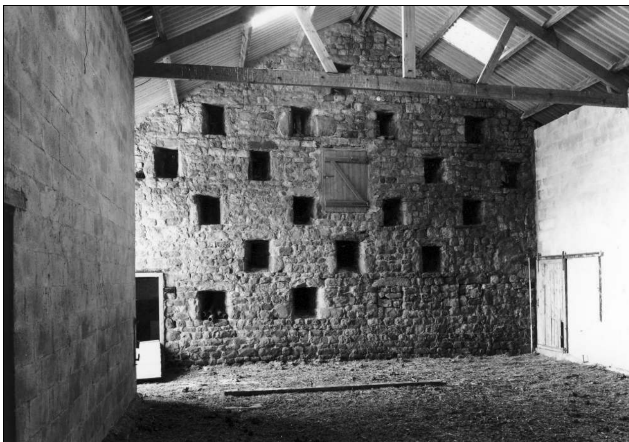
Photo 43: Interior face of south gable of aisled barn
