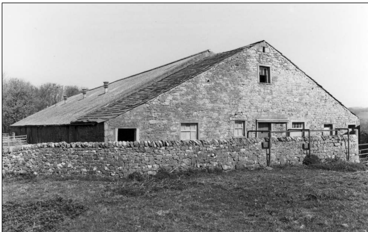
Photo 2: The barn from the south-west, showing extension with stone slate roof
