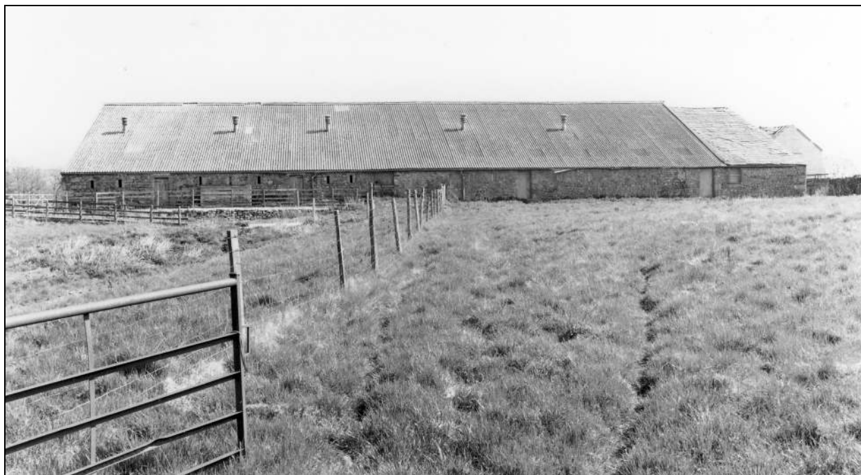
Photo 1: The barn from the west, showing extension with stone slate roof
