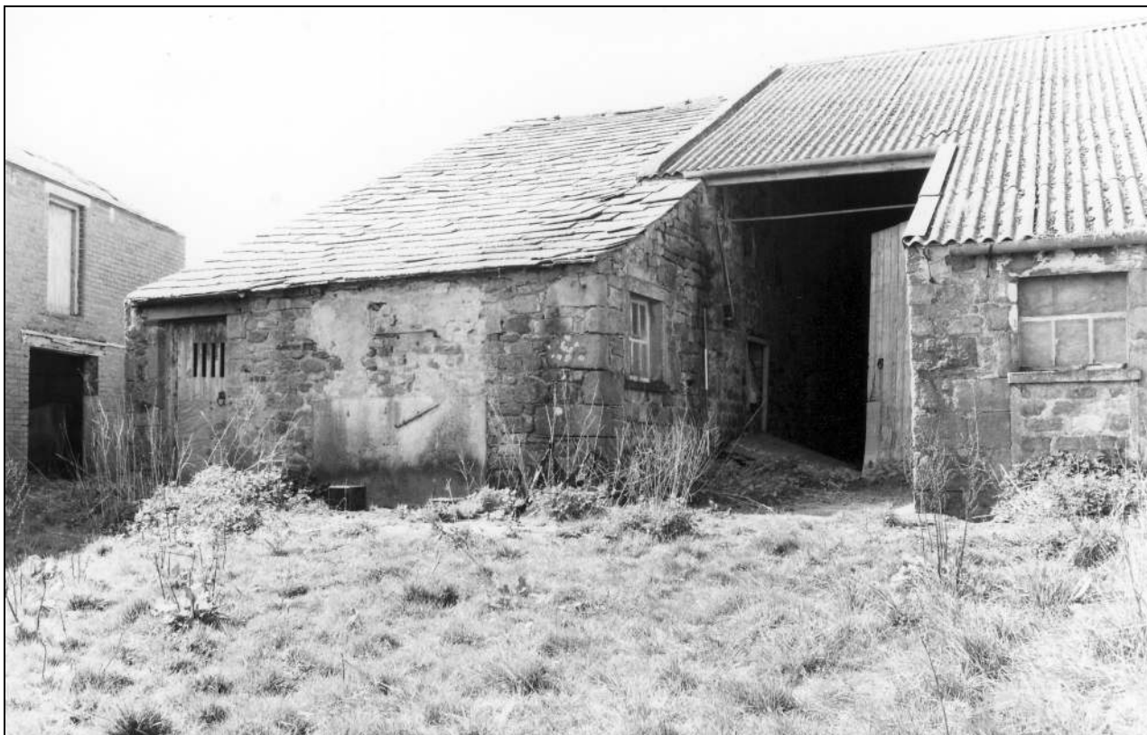
Photo 11: South extension, and new cart entry to south-east corner of aisled barn
