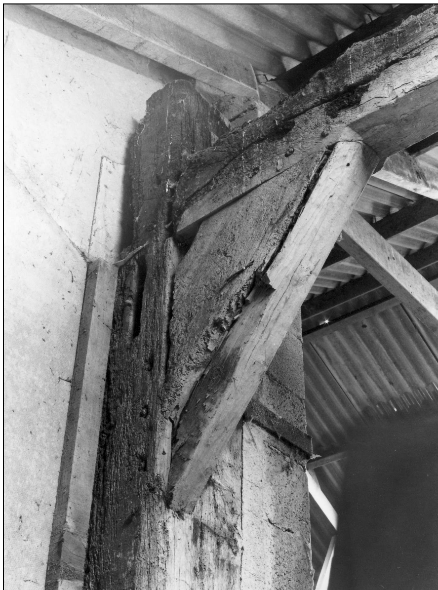
Photo 34: Top part of outer face of west arcade post (arcade plate lowered?)
