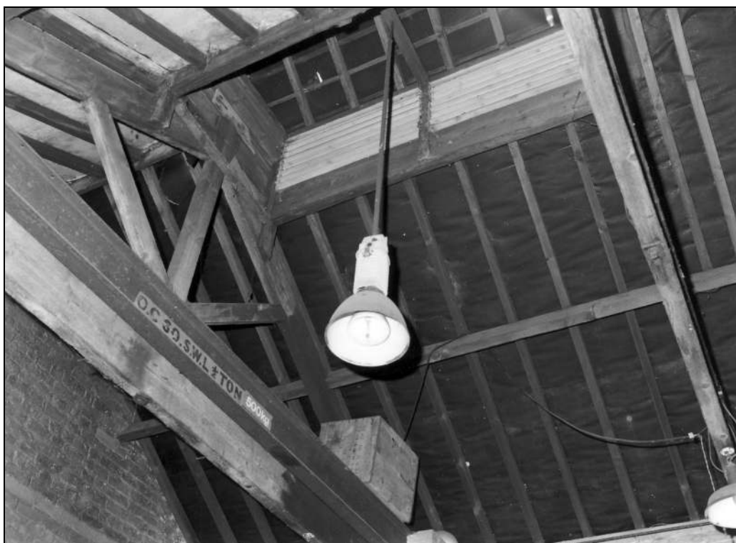
Photo 24: The retort house: roof truss and ridge vent, from the west (film 2, frame 12)
