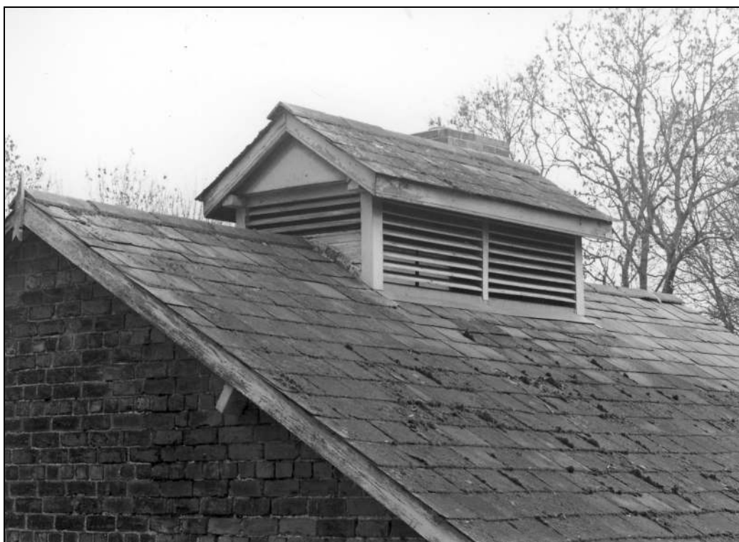
Photo 7: Detail of ridge ventilator to retort house, from the south (film 1, frame 13)
