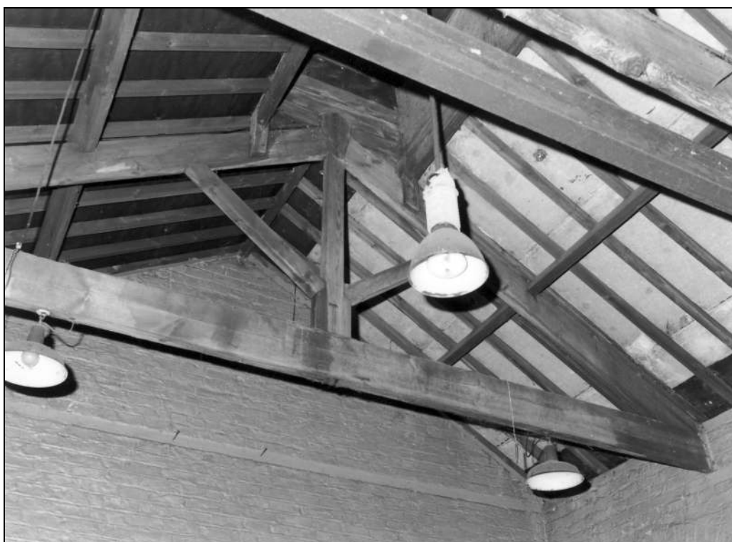
Photo 23: The retort house: roof truss, from the east (film 2, frame 11)
