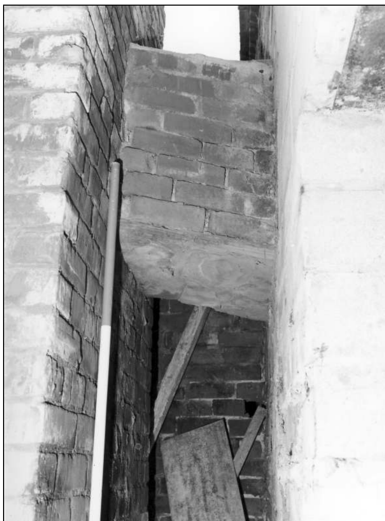
Photo 35: Detail of flue from retort house to chimney (film 2, frame 17)
