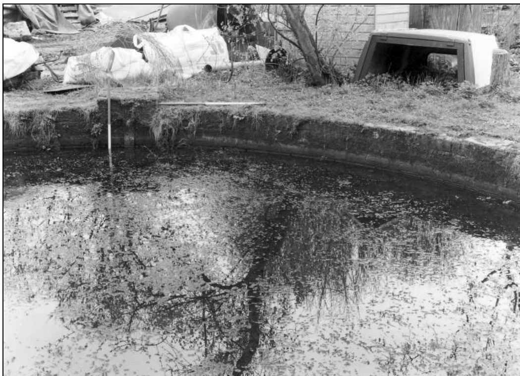
Photo 38: Gasholder pit: detail of brick lining with stone block, from the south (film 1, frame 17)
