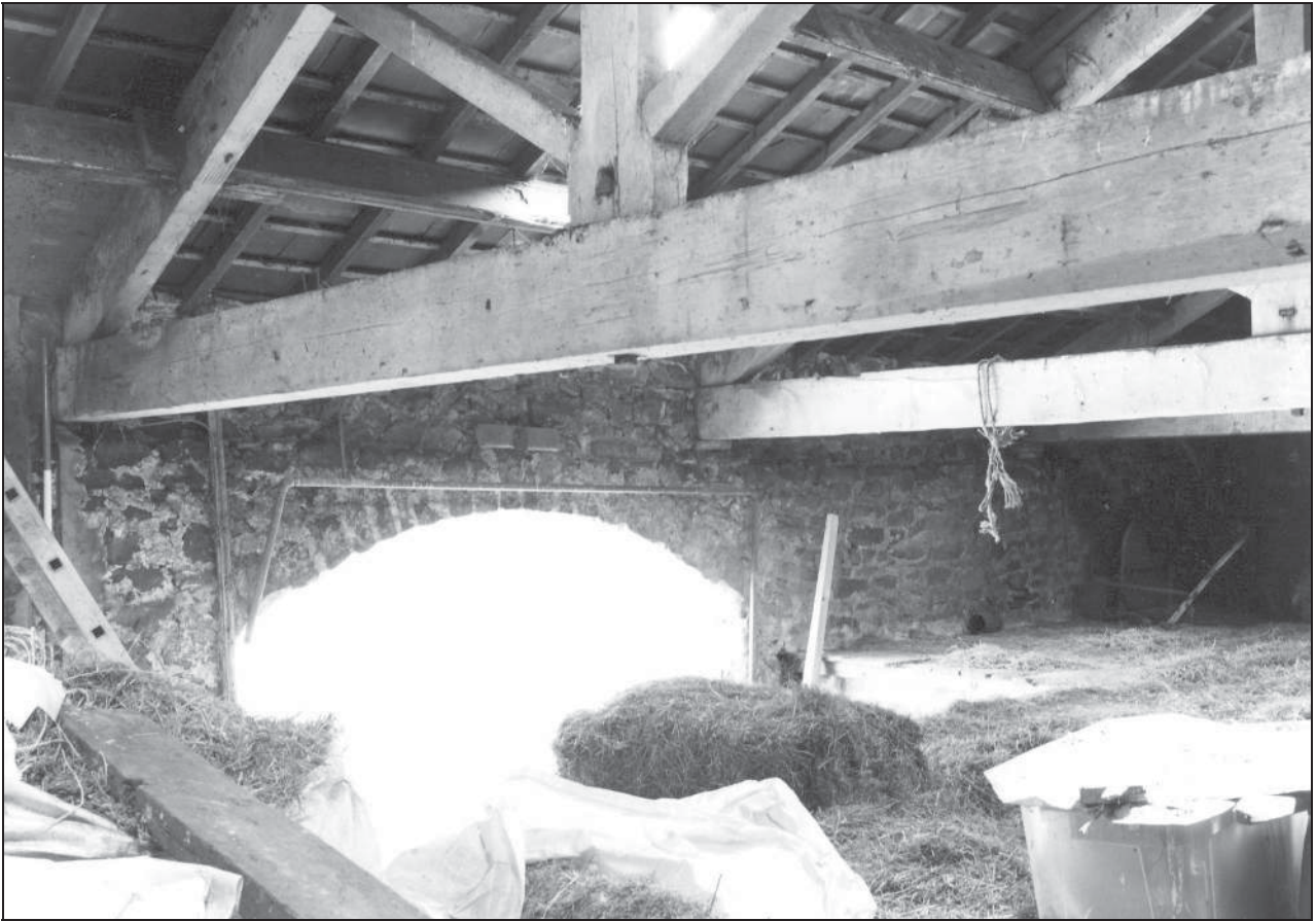
Photo 5: Hay loft, from the west
