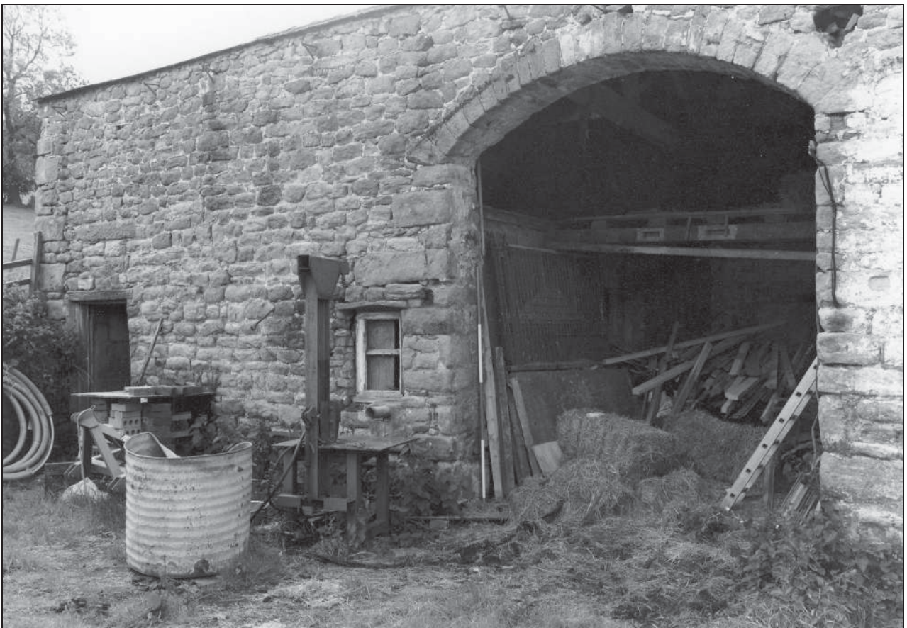
Photo 6: Detail of arched cart entrance, north-east elevation
