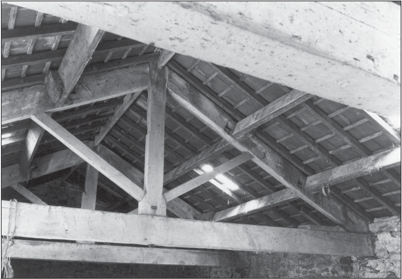
Photo 15: Typical roof truss, from the north
