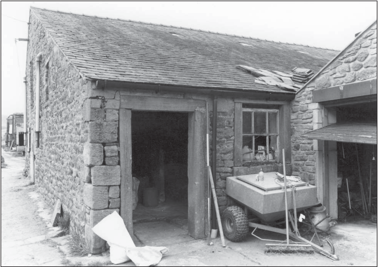
Photo 19: Detail of doorway to stable in south-west shippon
