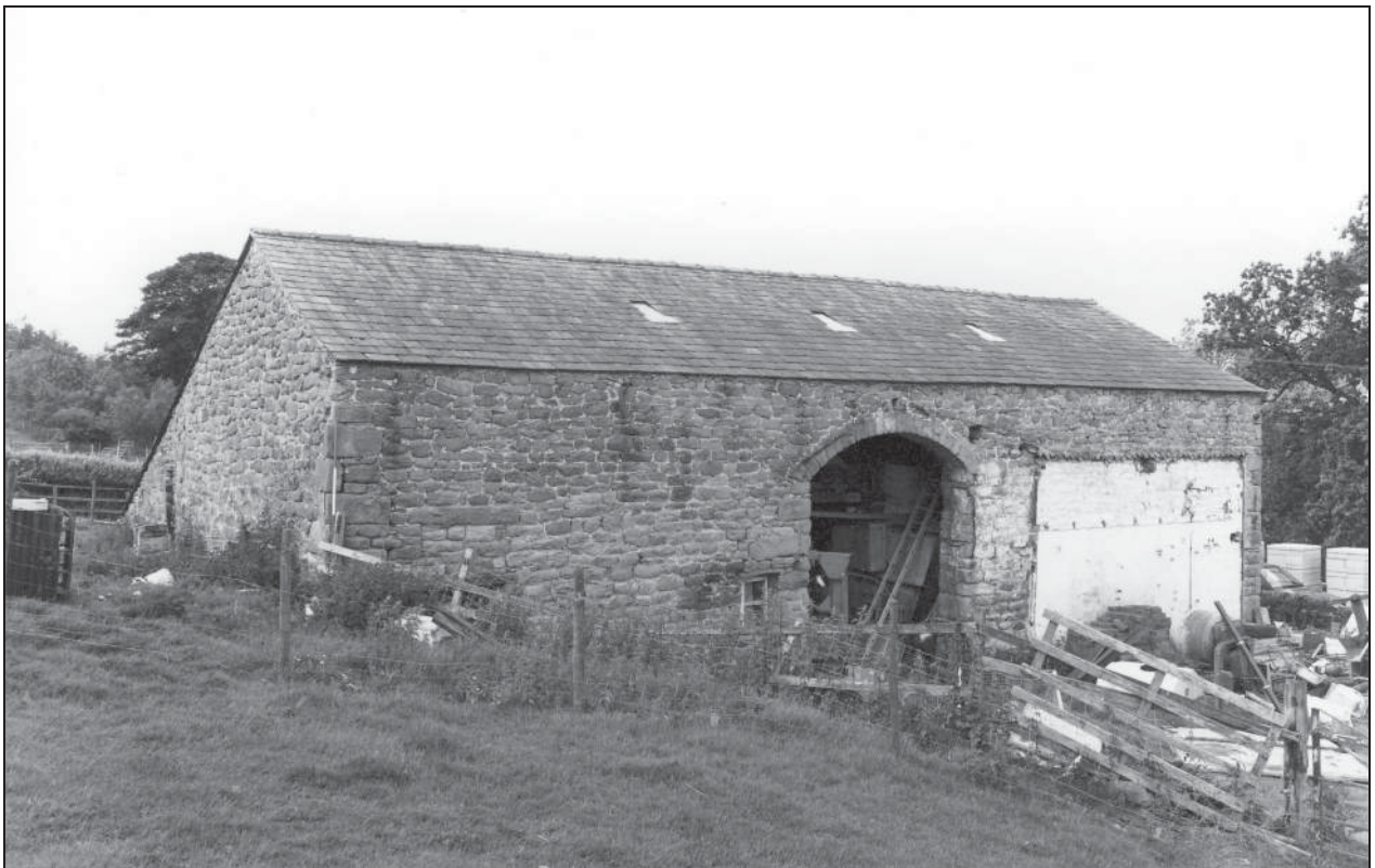
Photo 4: The barn, from the east
