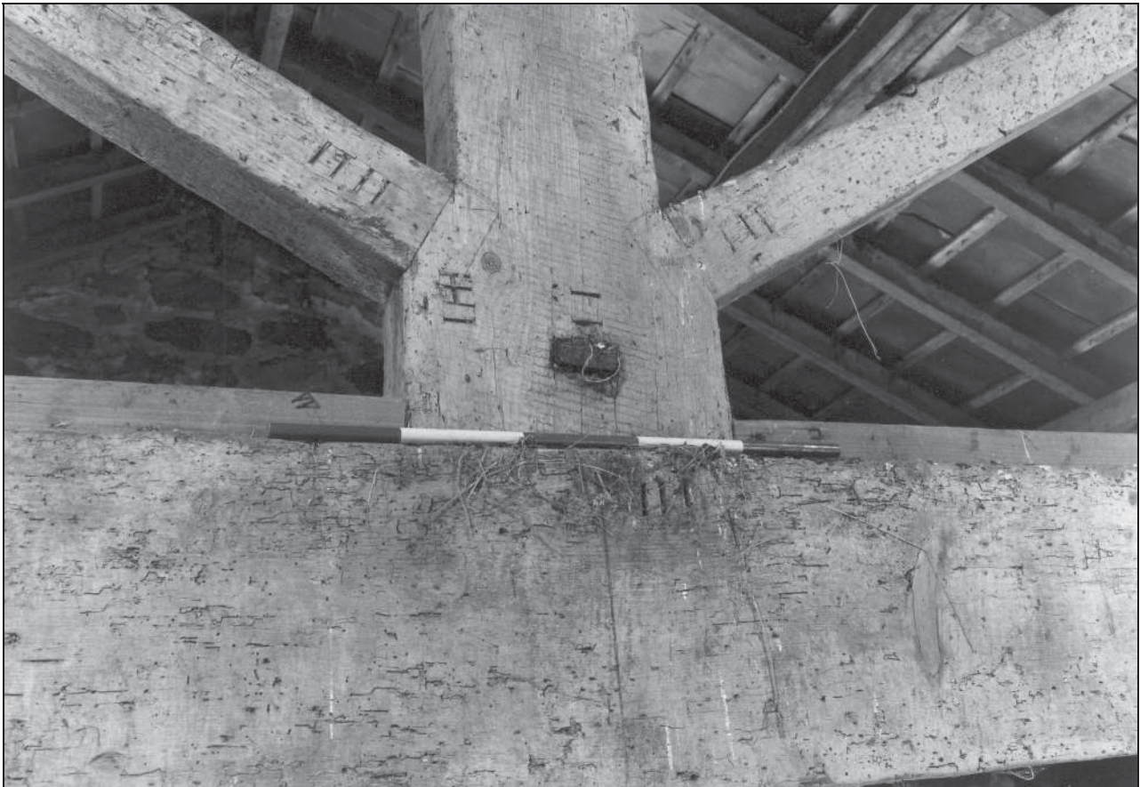
Photo 16: Detail of joint numbering on roof truss
