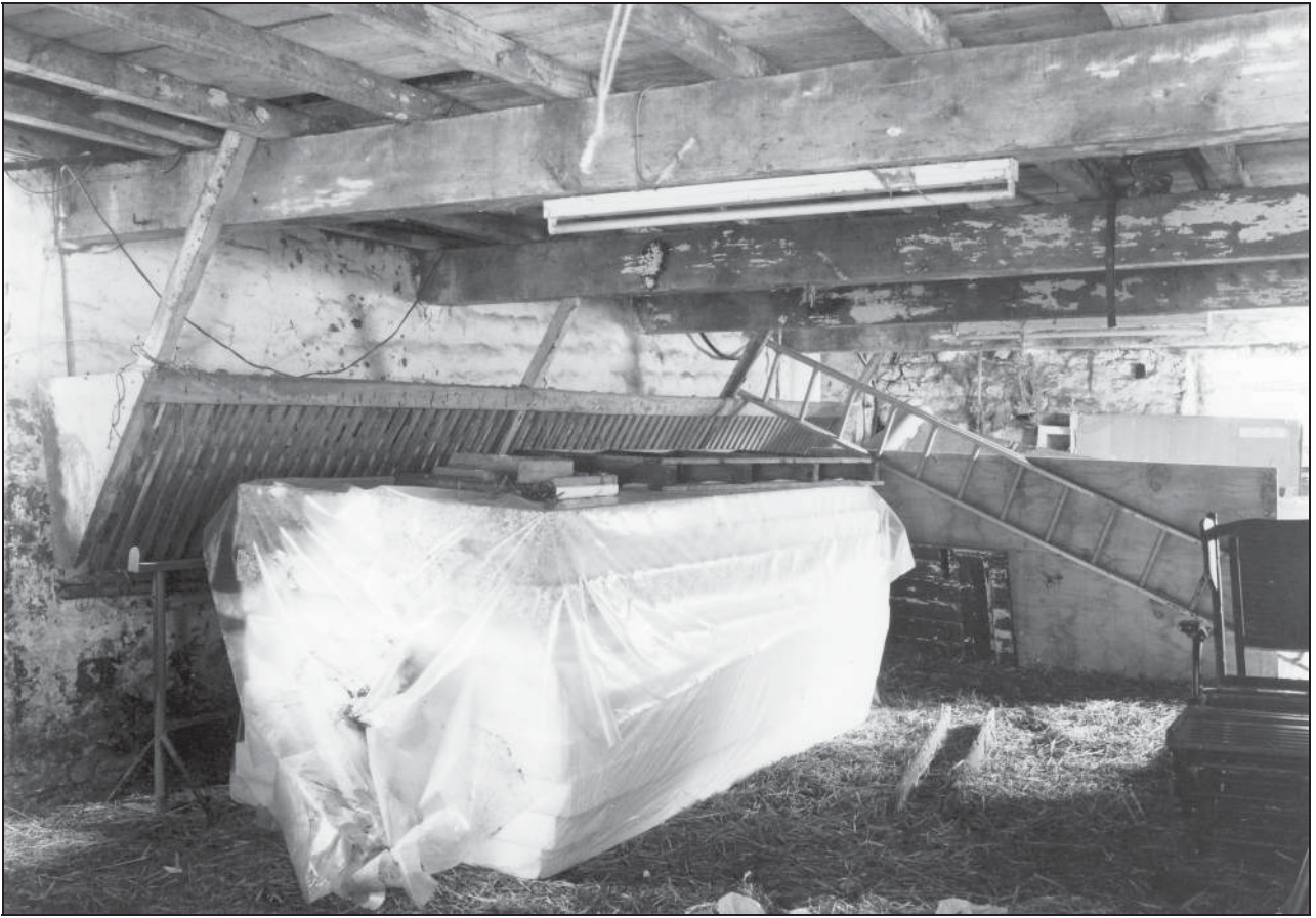
Photo 21: Interior of lean-to shippon
