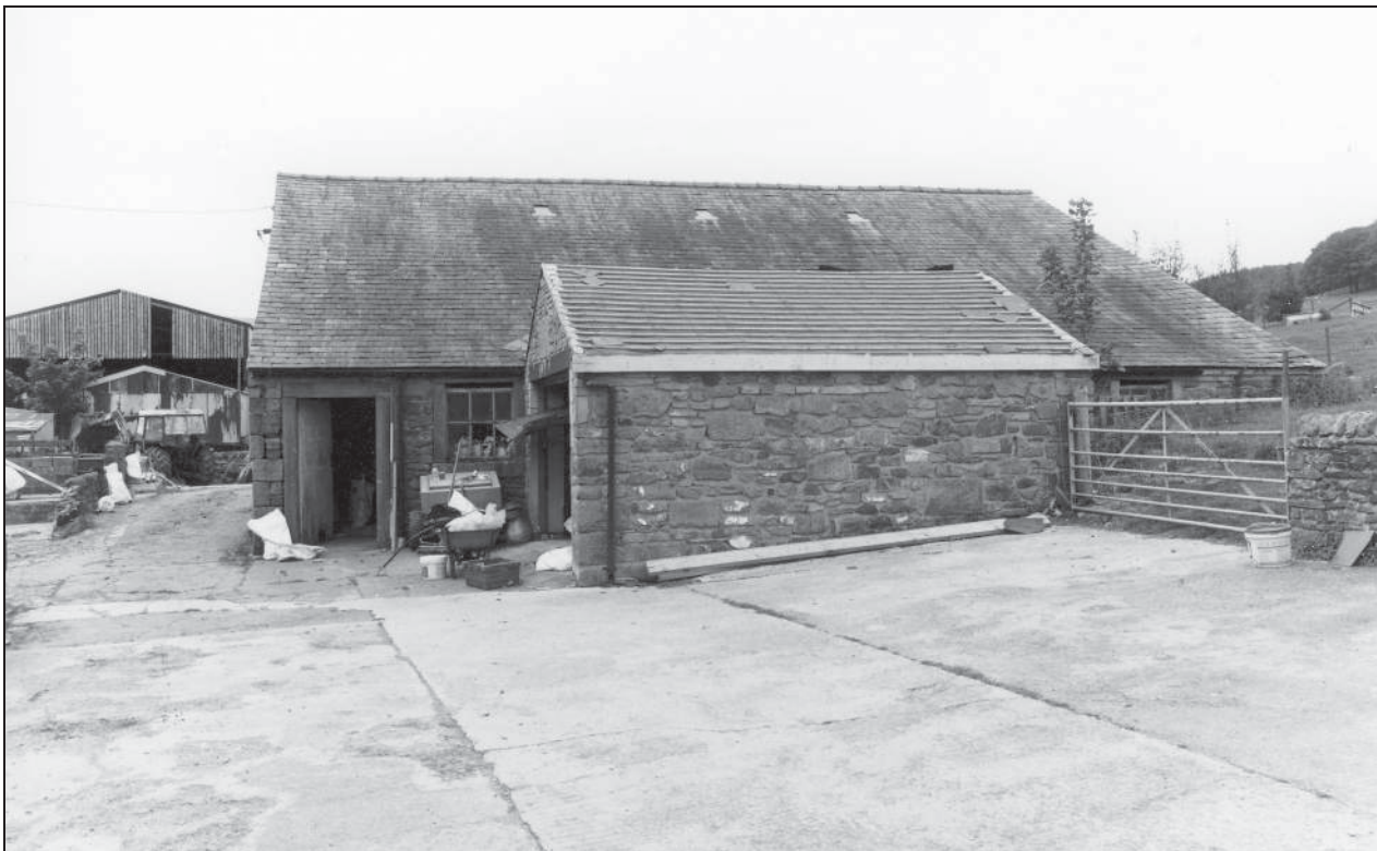
Photo 18: The barn, from the south-west
