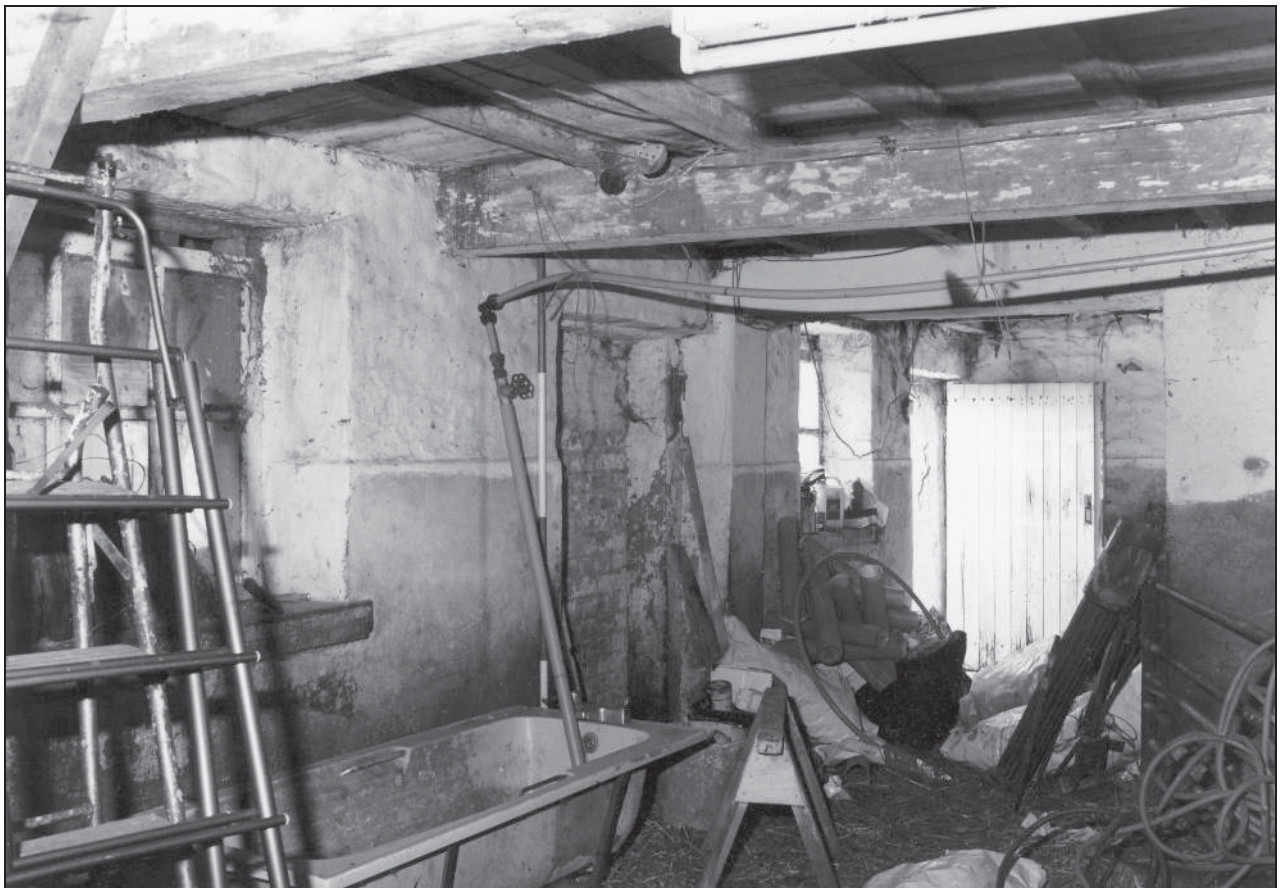
Photo 22: Interior of lean-to shippon
