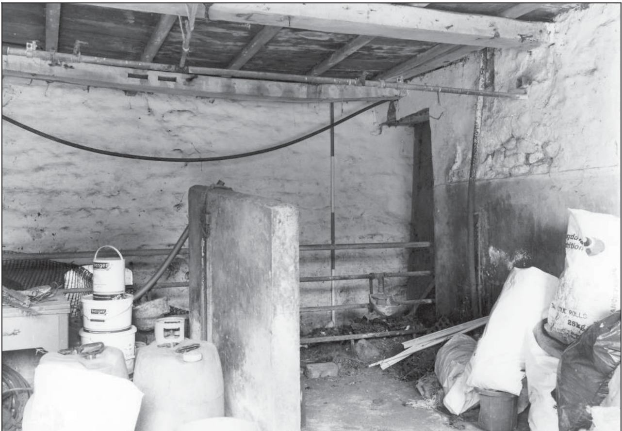
Photo 20: Interior of lean-to shippon, north-west end (former stable)
