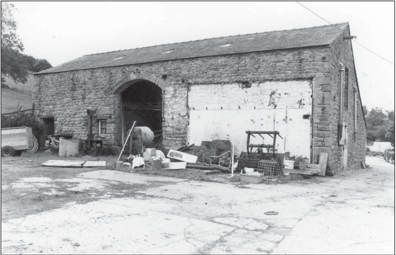
Photo 3: The barn, from the north
