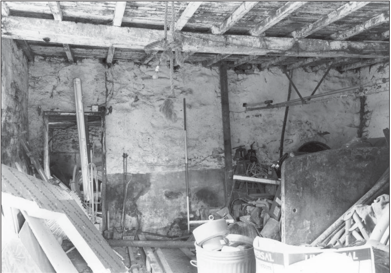
Photo 13: Shippon in south-east end of barn
