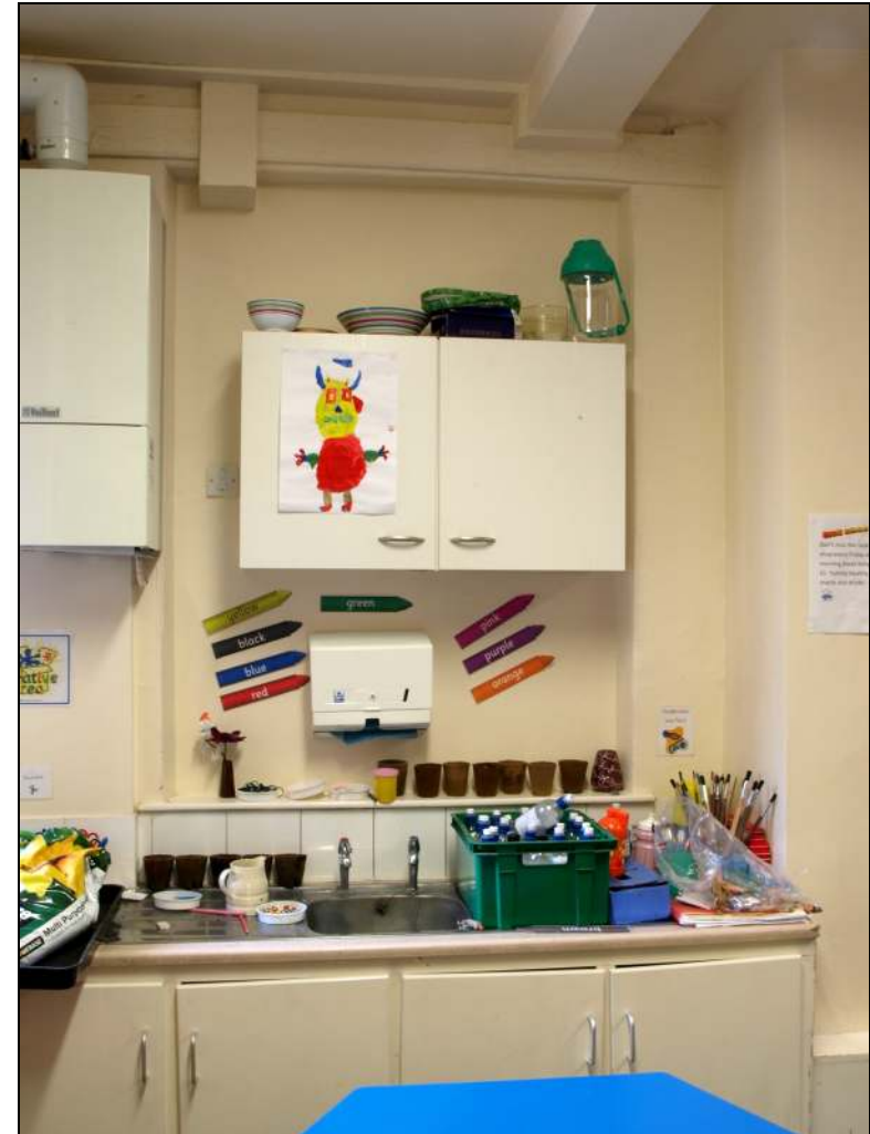
Photo 16: Blocked window, north side of rear south room
