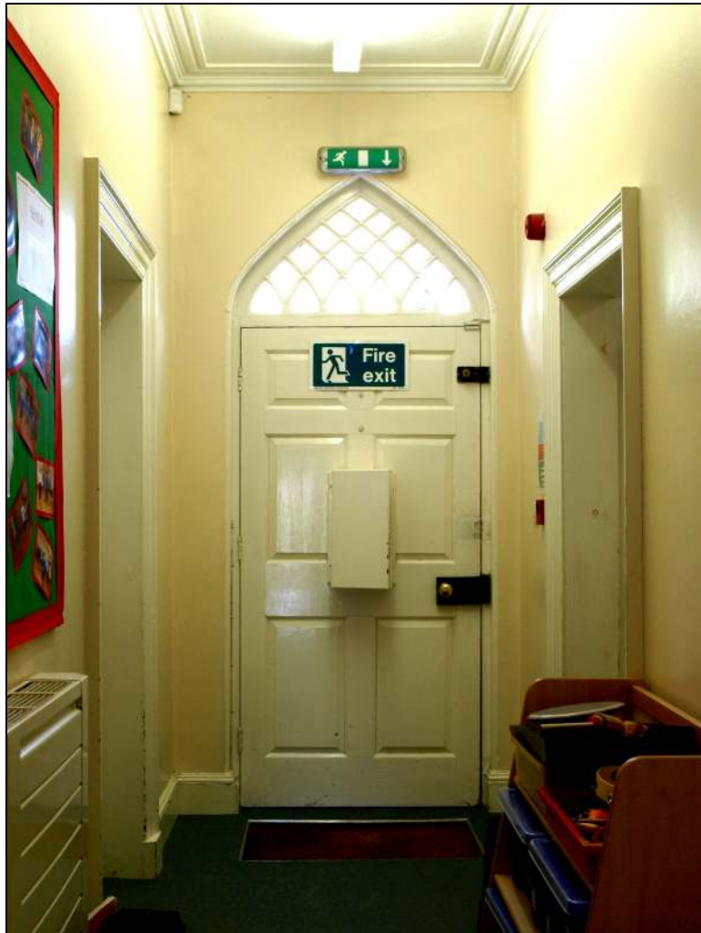
Photo 5: Entrance hall, looking towards the front
