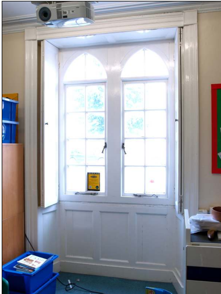
Photo 13: Front window, north front room
