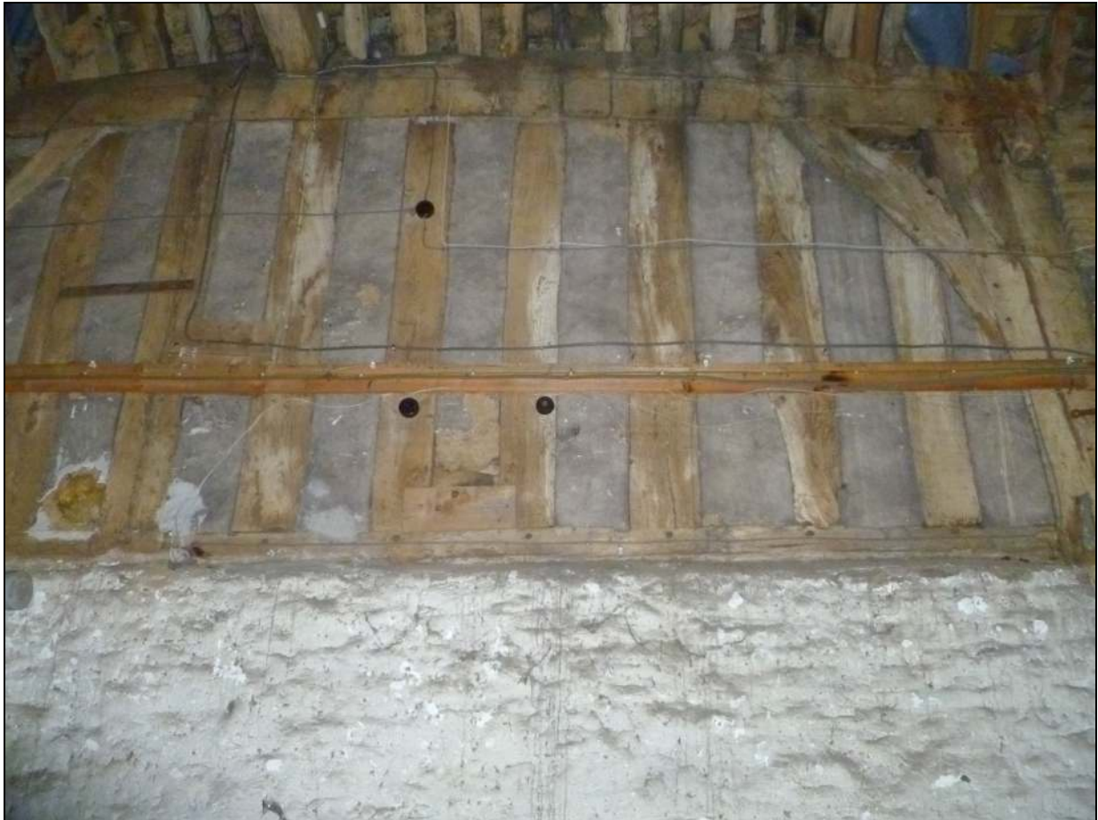
Photo JCM11: Close studding at upper level, adjoining house
