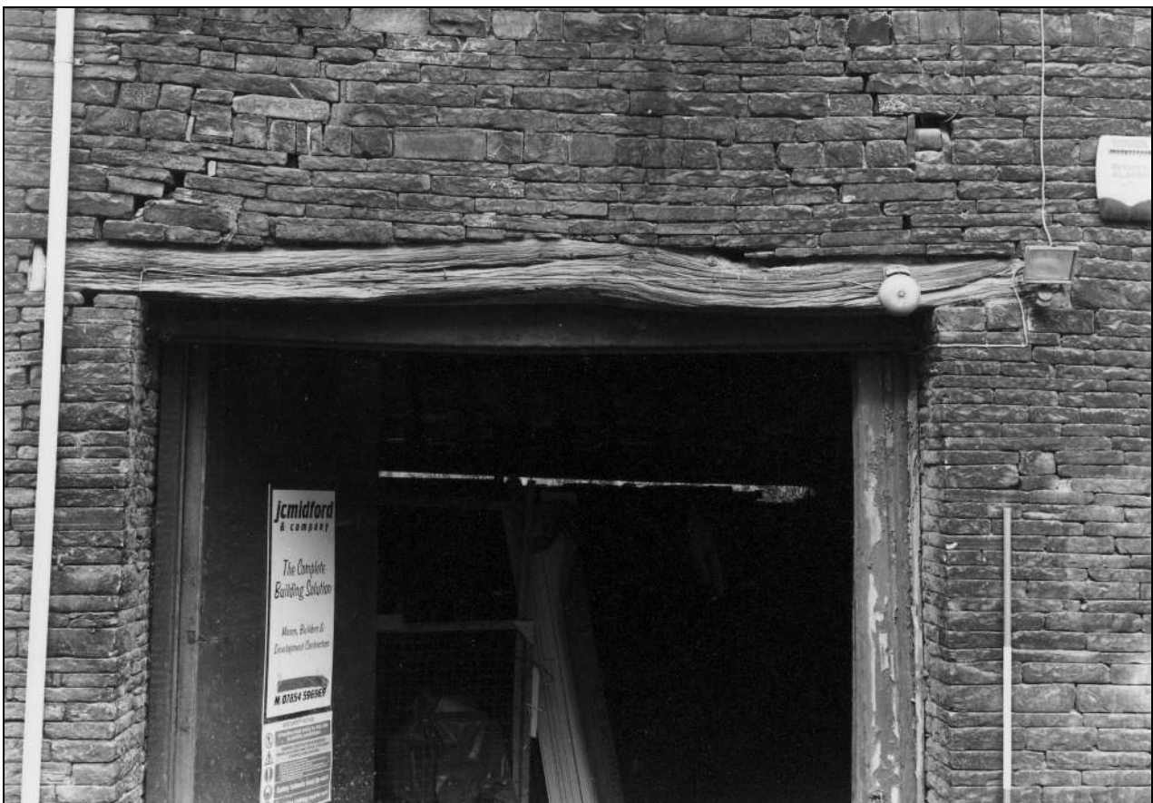
Photo 6: Detail of lintel over doorway, east elevation (film 1, frame 6)
