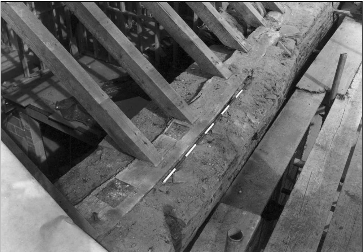
Photo 50: Wall plate on east wall, during watching brief (film 5, frame 17)
