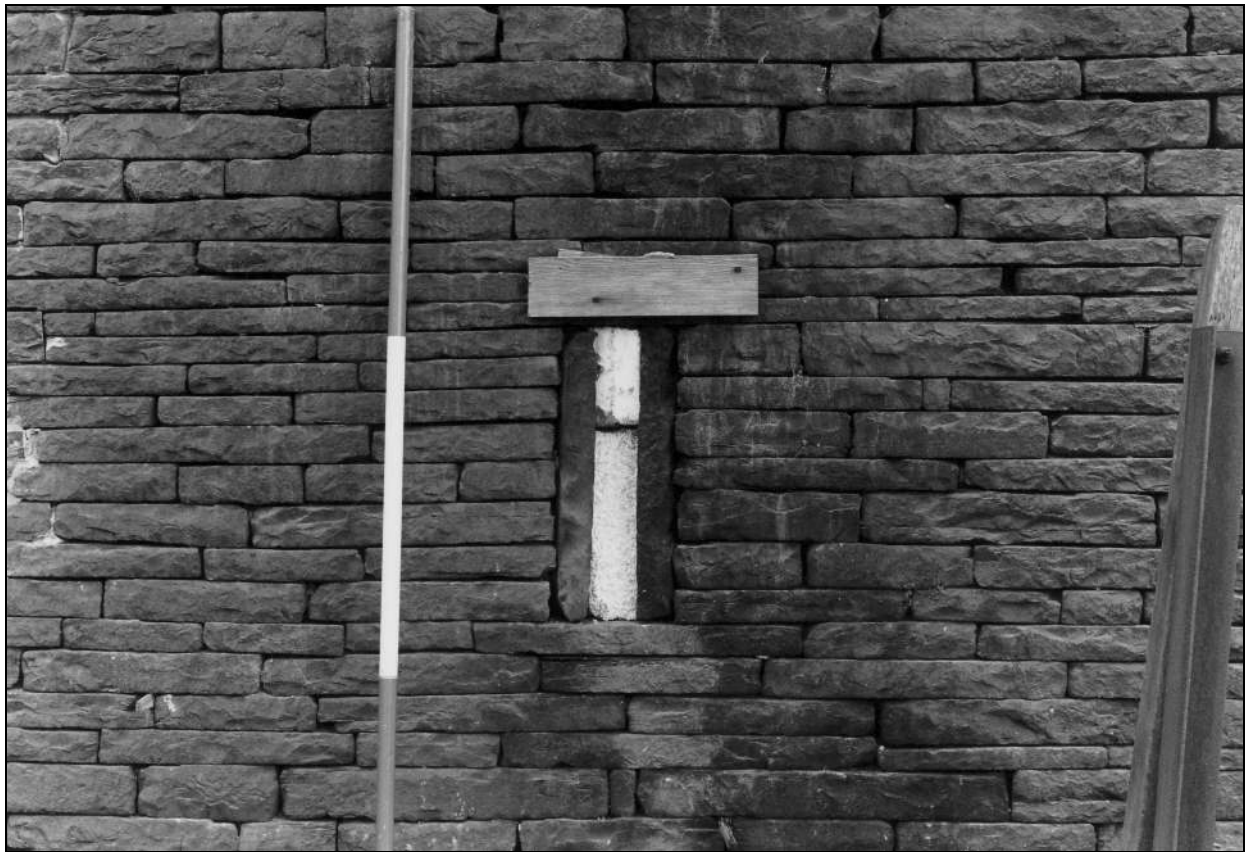
Photo 13: Detail of breather, west elevation (film 1, frame 12)
