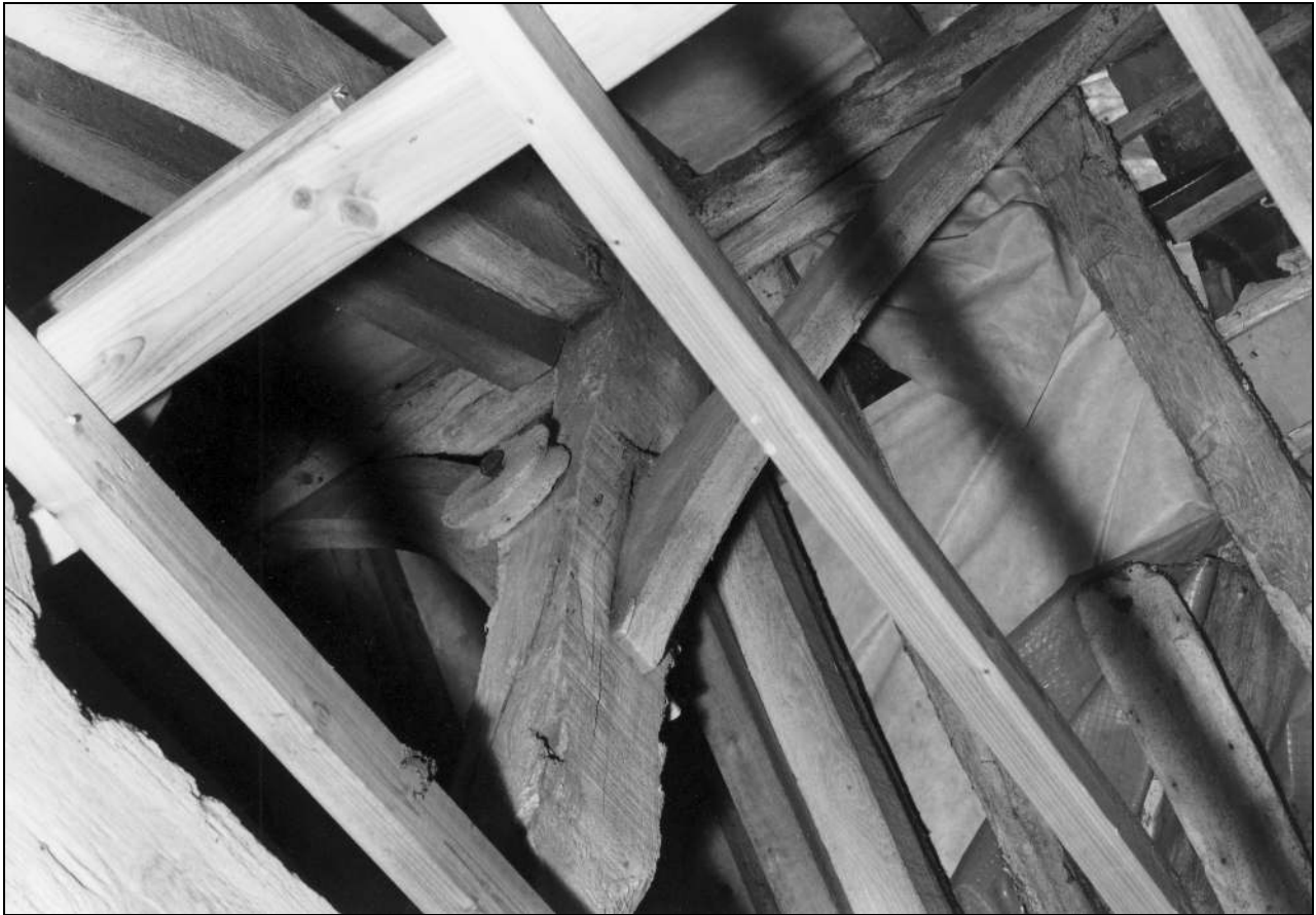
Photo 41: North truss, showing pulley attached to west side of king post (film 2, frame 11)
