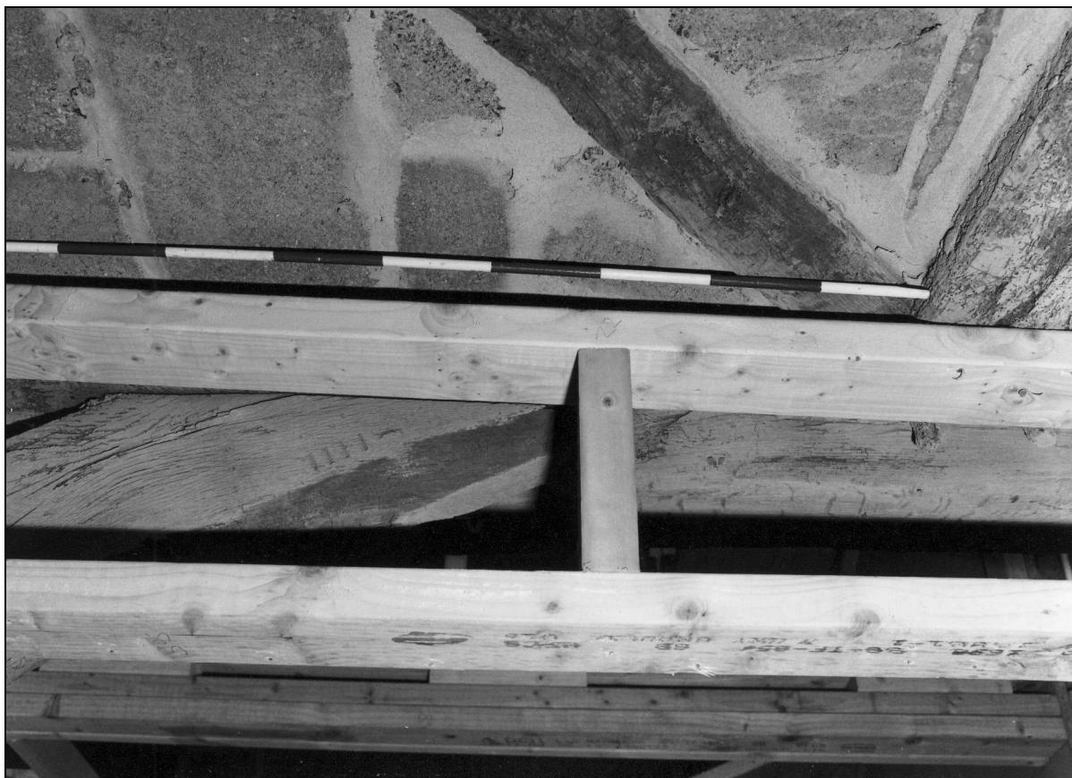
Photo 47: Detail of south arcade post, from the west, showing numbering "II" and "I" (film 2, frame 18)
