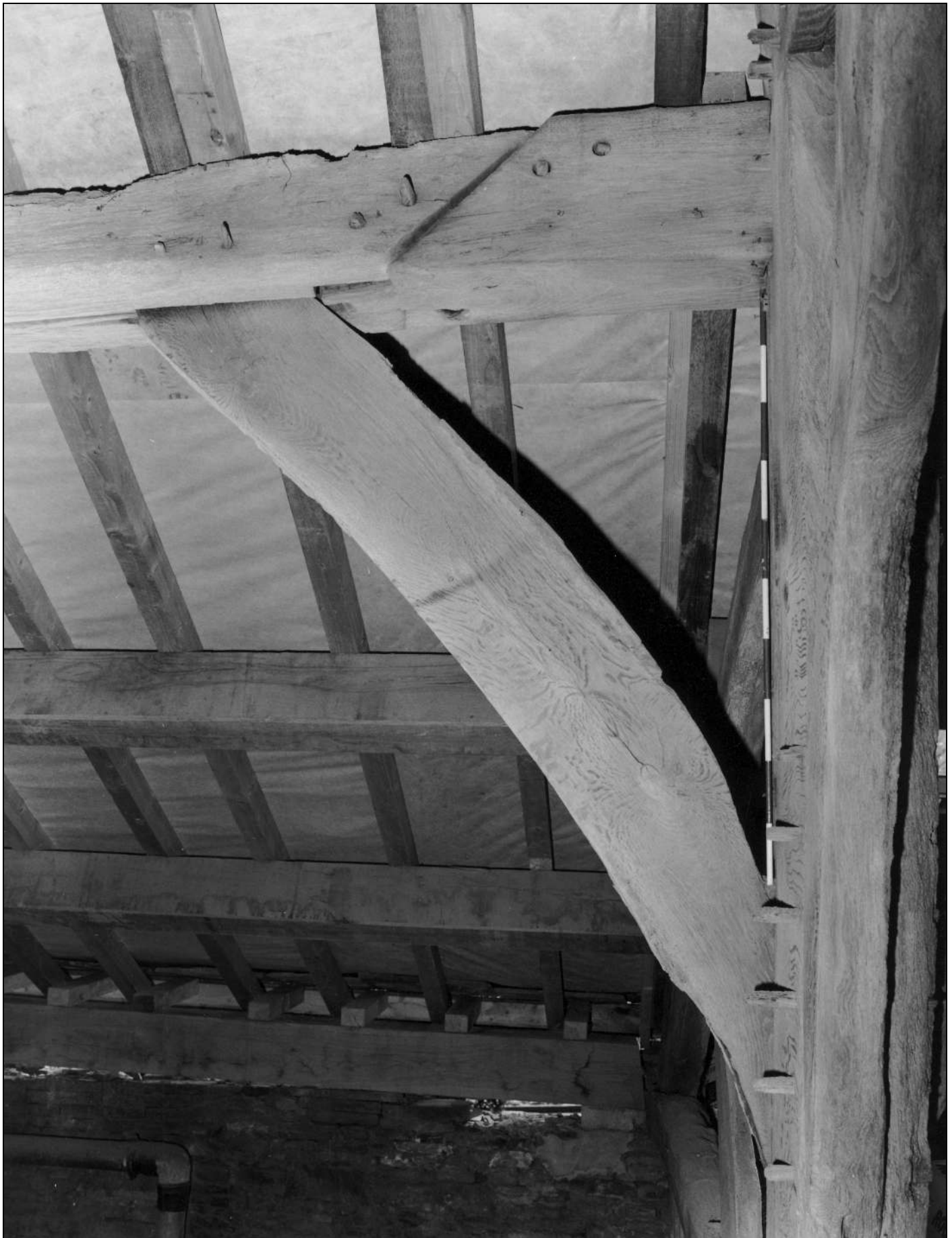
Photo 36: South arcade post, arch brace and scarf joint, from the east (film 3, frame 13)
