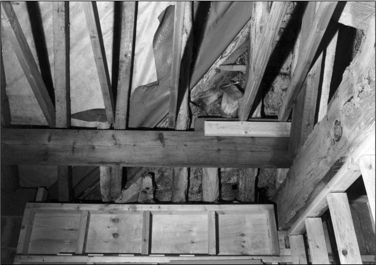
Photo 27: Lath and daub in roof, between house and barn (north part) (film 2, frame 7)
