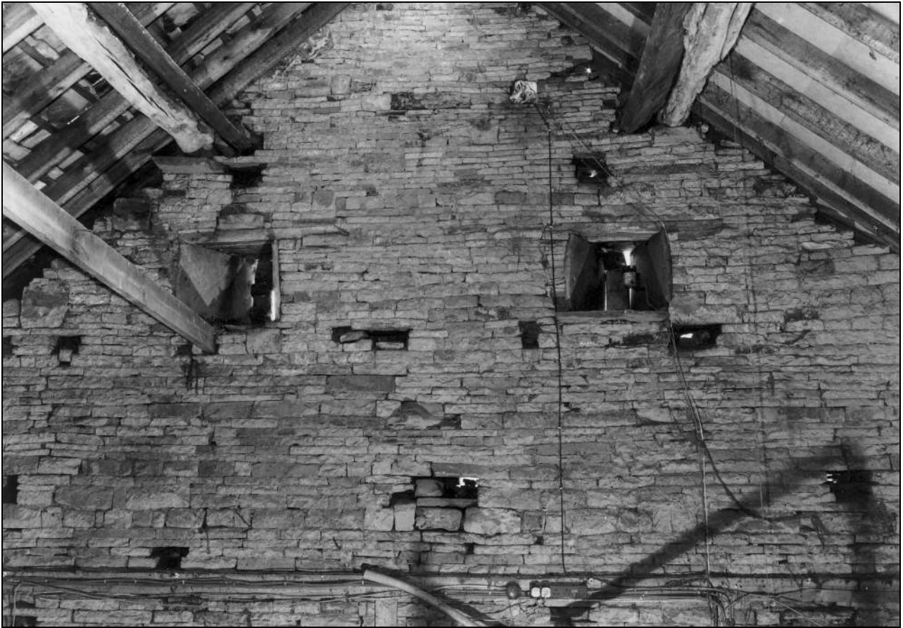
Photo 23: South gable: interior face with breathers (film 3, frame 10)
