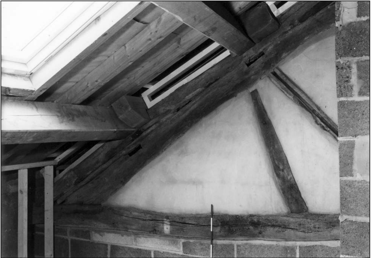
Photo 45: Roof structure over aisle, north truss, from the south (film 2, frame 15)
