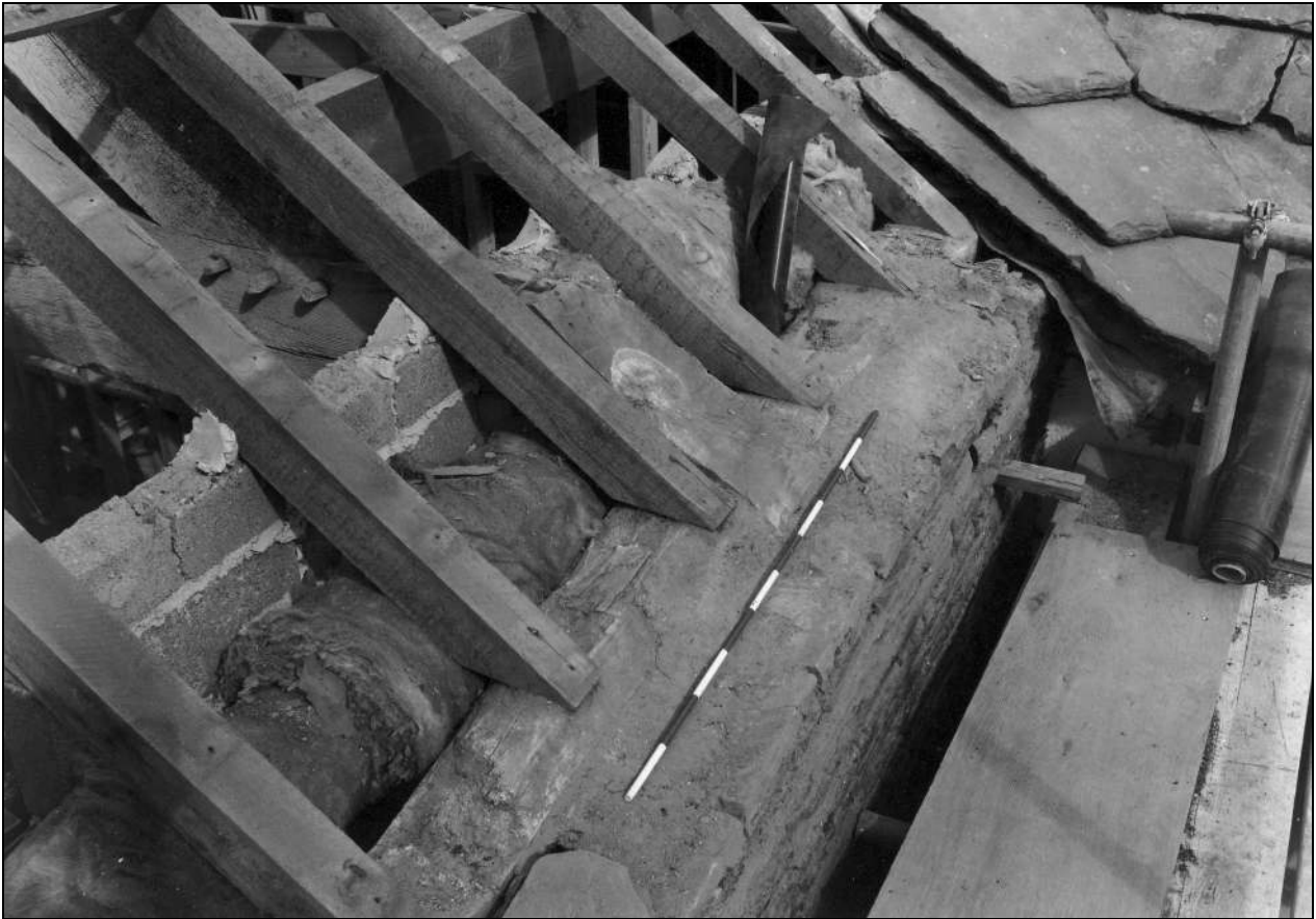
Photo 51: Wall plate on east wall, with end of south tie beam, during watching brief (film 5, frame 16)
