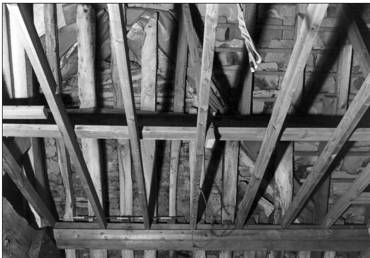
Photo 26: Lath and daub in roof, between house and barn (south part) (film 2, frame 9)
