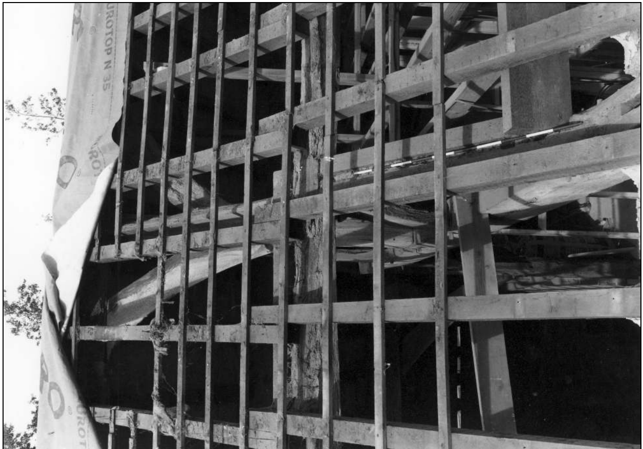
Photo 51: Wall plate on east wall, with end of south tie beam, during watching brief (film 5, frame 16)
