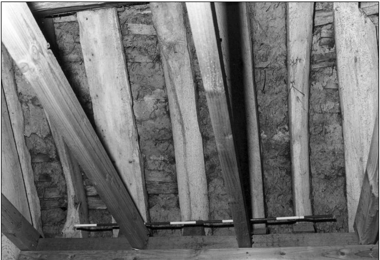
Photo 28: Detail of daub in roof, between house and barn (film 2, frame 10)
