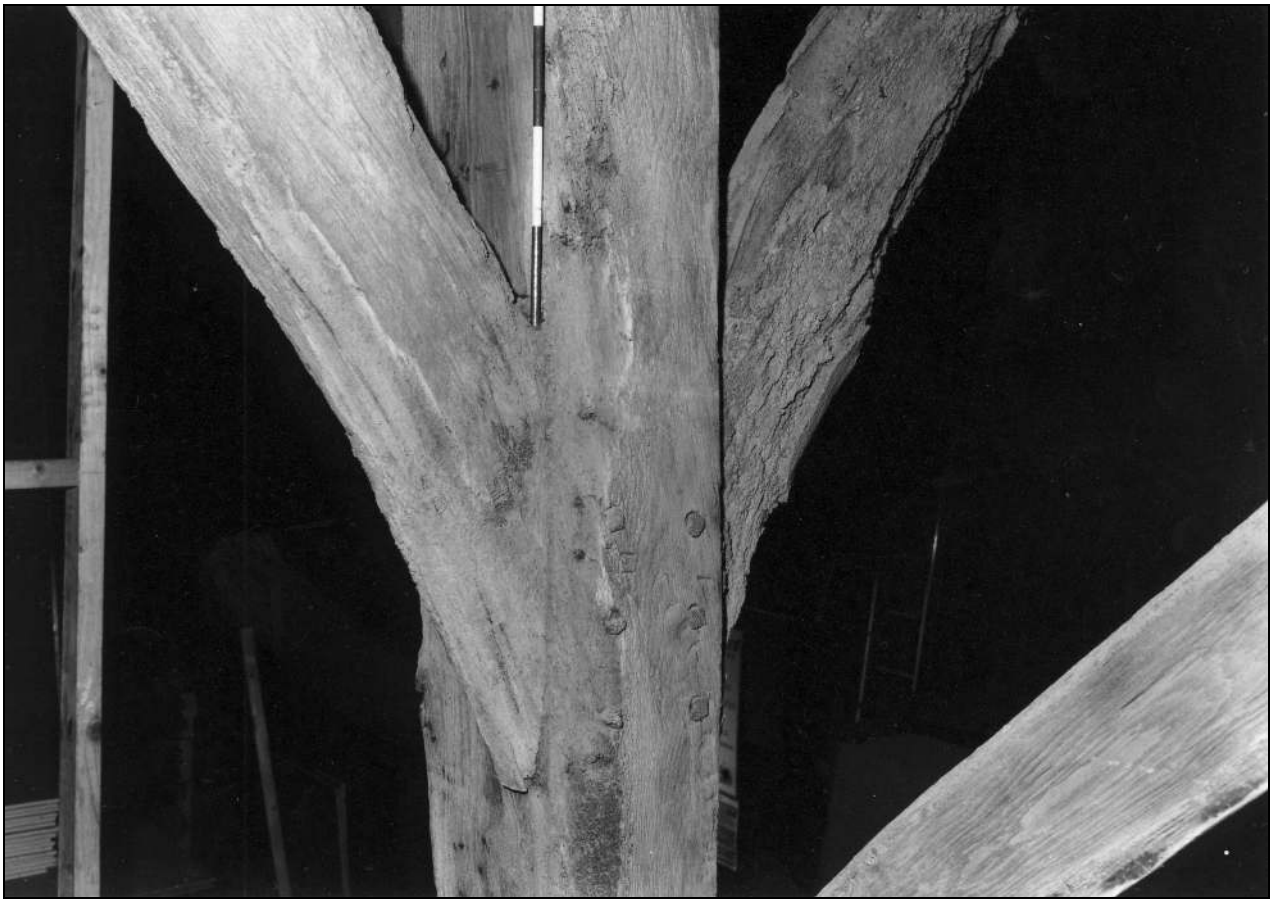
Photo 47: Detail of south arcade post, from the west, showing numbering "II" and "I" (film 2, frame 18)
