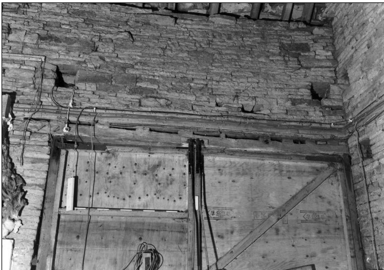
Photo 25: Detail of internal lintel over doorway in east side of south bay (film 3, frame 9)
