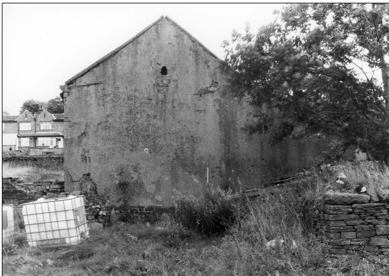
Photo 6: The barn: west gable (film 1, frame 5)
