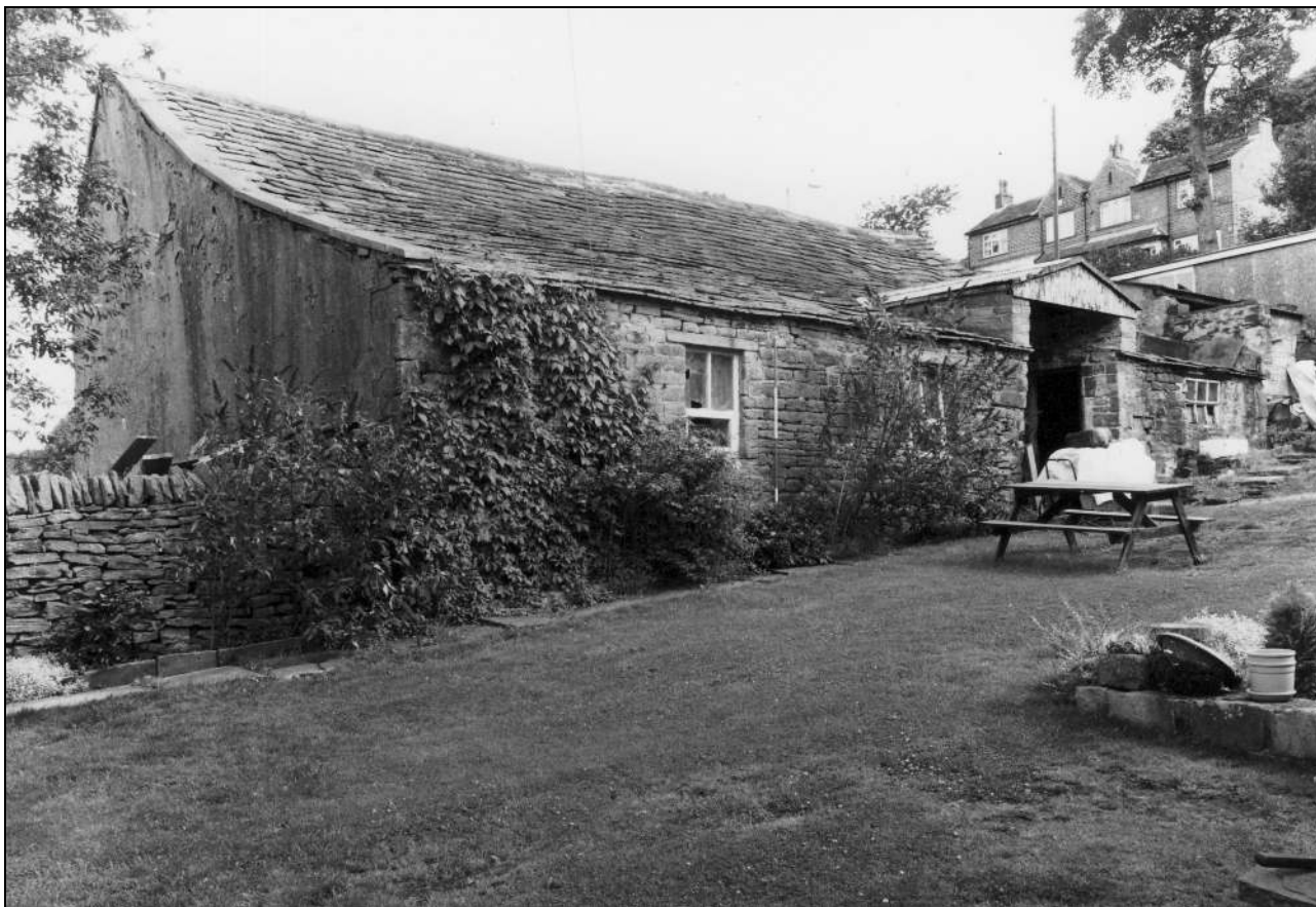
Photo 5: The barn, from the south-west (film 1, frame 4)
