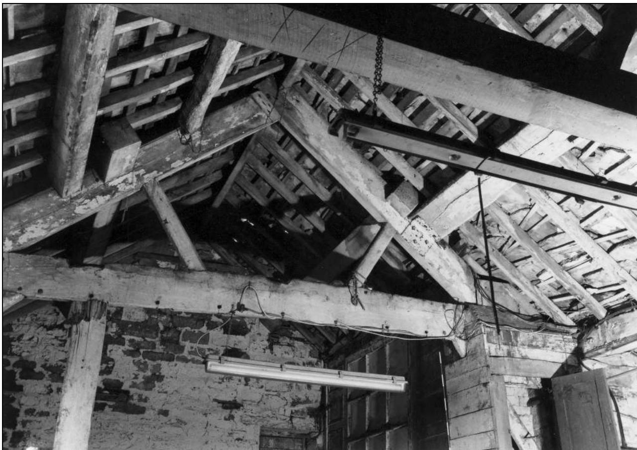
Photo 50: East roof truss, from the west (film 3, frame 17)
