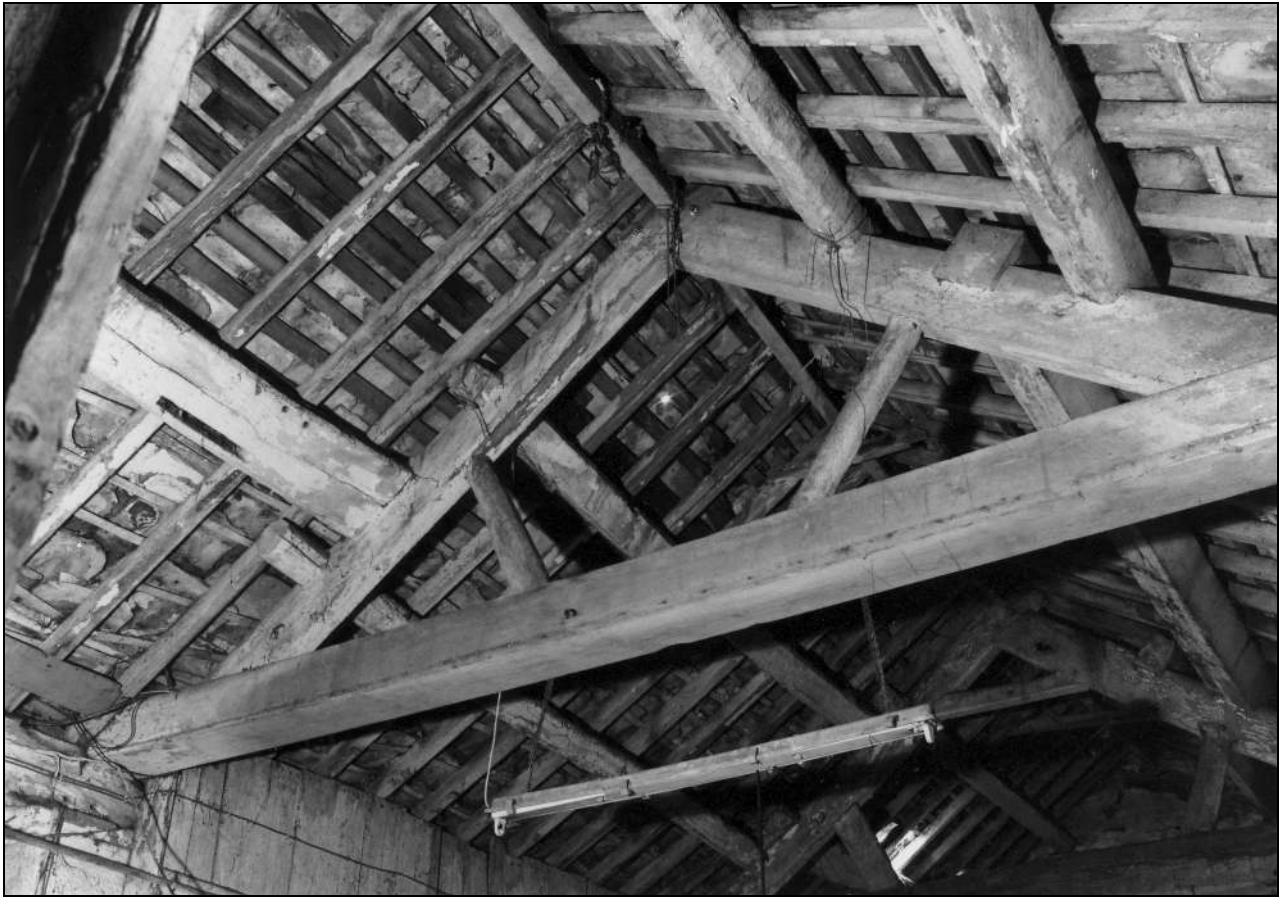
Photo 48: Central roof truss, from the north-east (film 4, frame 5)
