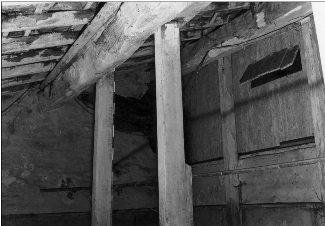
Photo 54: Purlin in south-west outshut (west end), from the east (film 3, frame 9)
