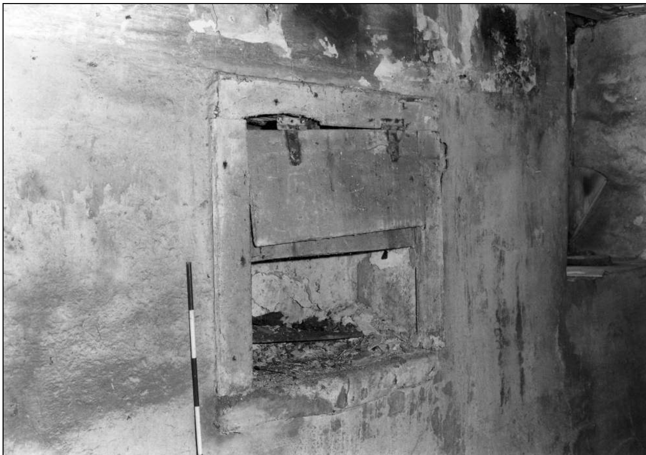
Photo 29: Recess/cupboard in south side of south-west outshut (film 4, frame 13)
