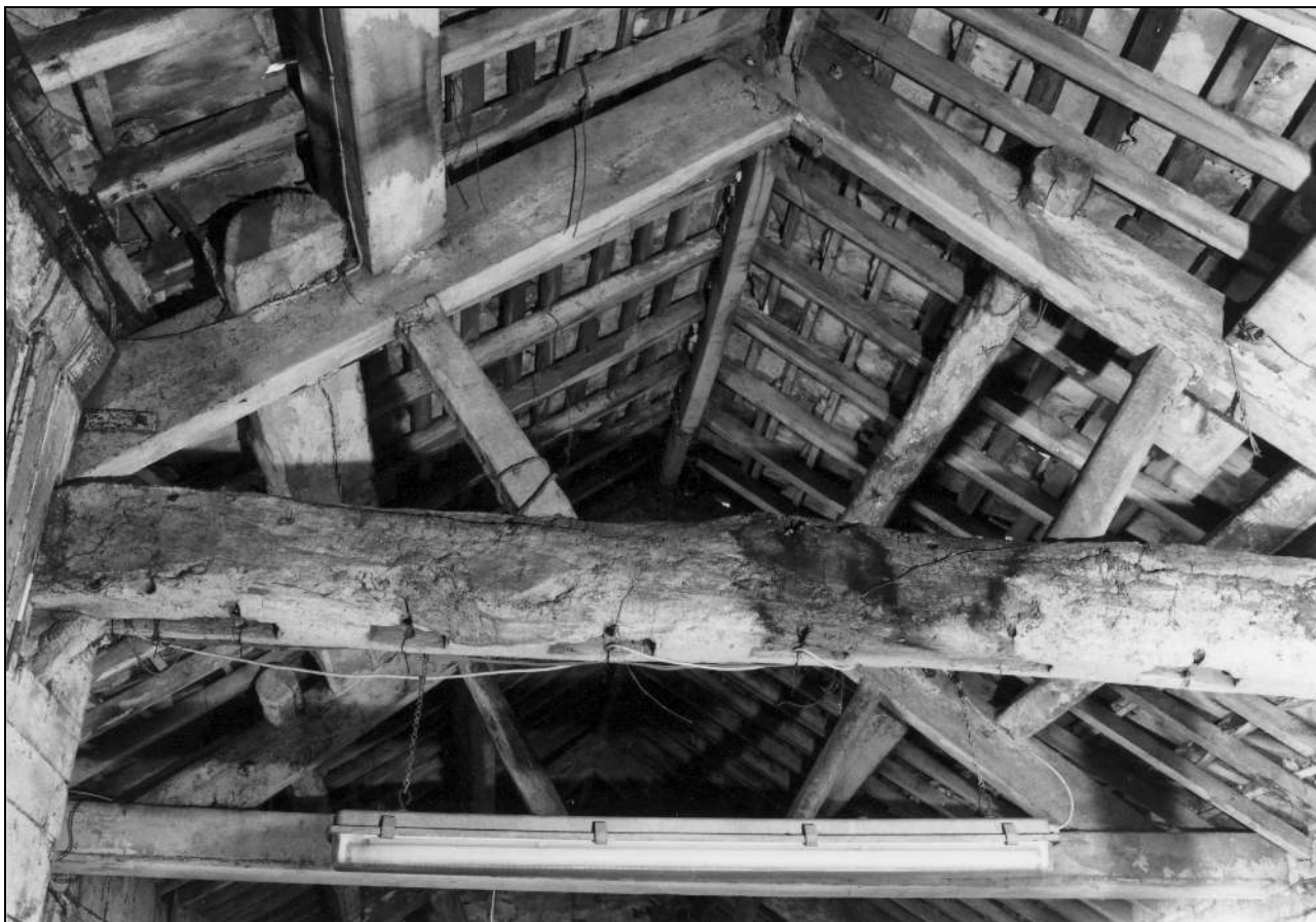
Photo 52: East roof truss, from the east (film 3, frame 18)
