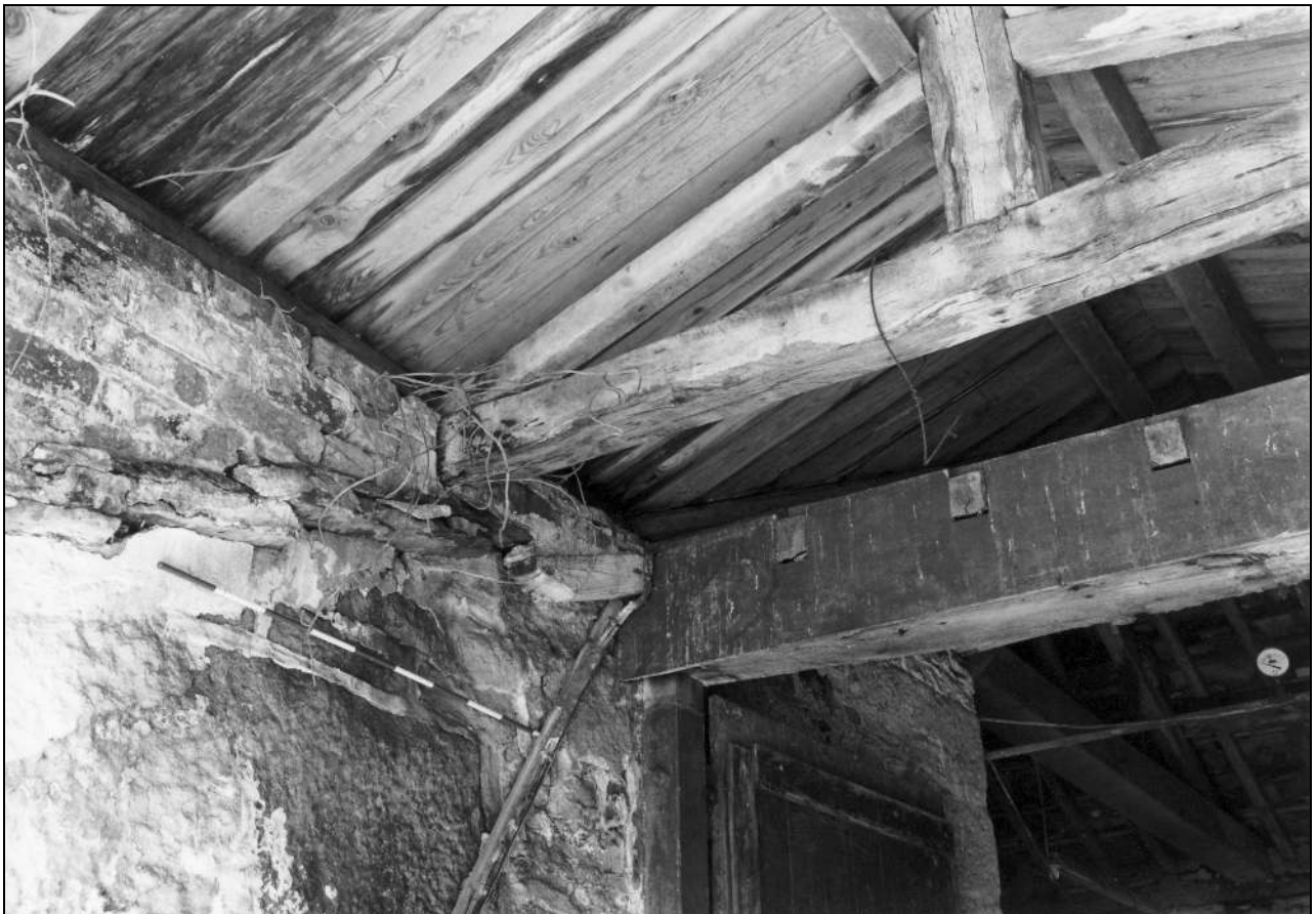
Photo 16: Modern roof over entrance and position of doorway (film 2, frame 7)
