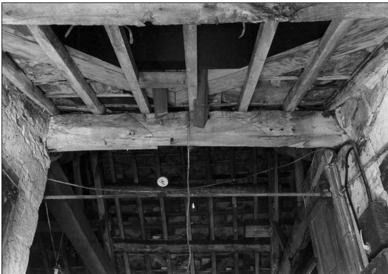
Photo 46: Arcade plate over barn entrance, from the south (film 2, frame 6)
