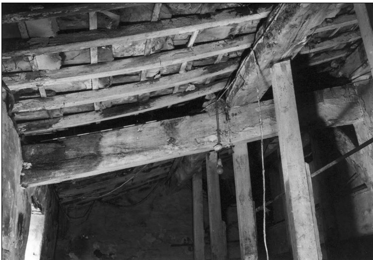
Photo 43: Aisle rafter (re-used post), from the east (film 2, frame 16)
