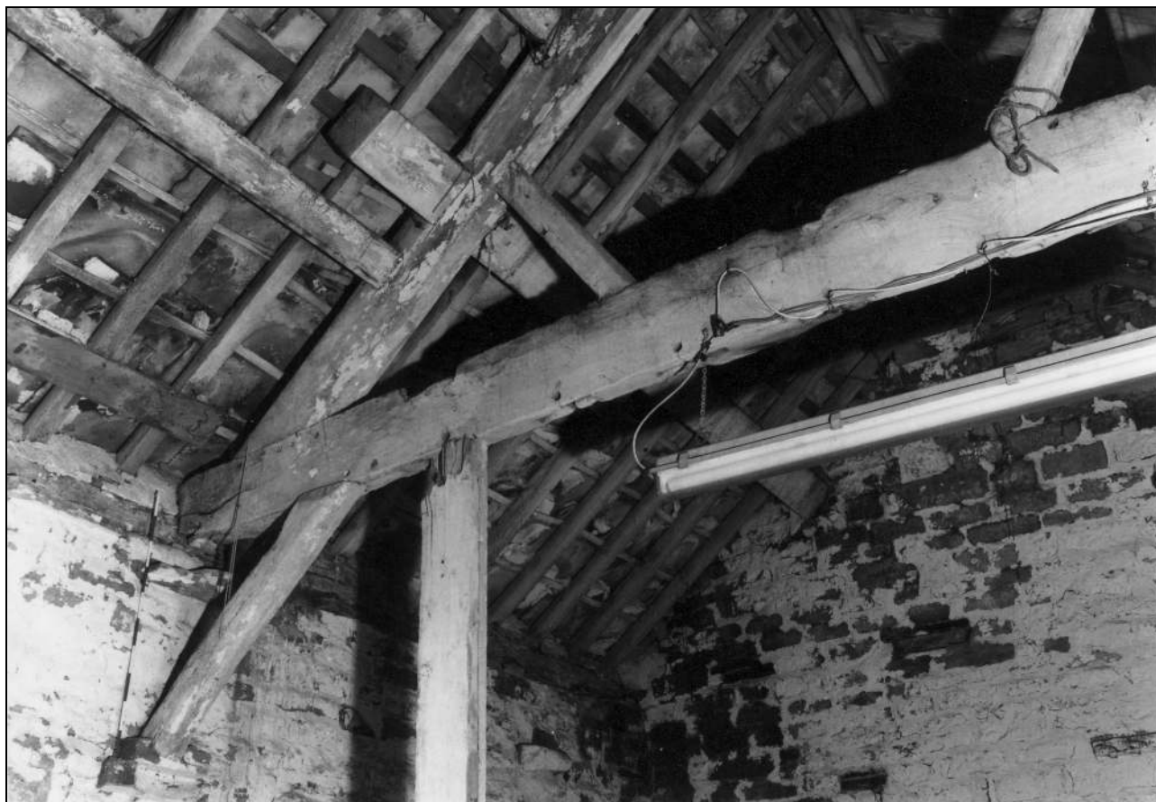
Photo 51: North end of east roof truss, from the south-west (film 3, frame 16)
