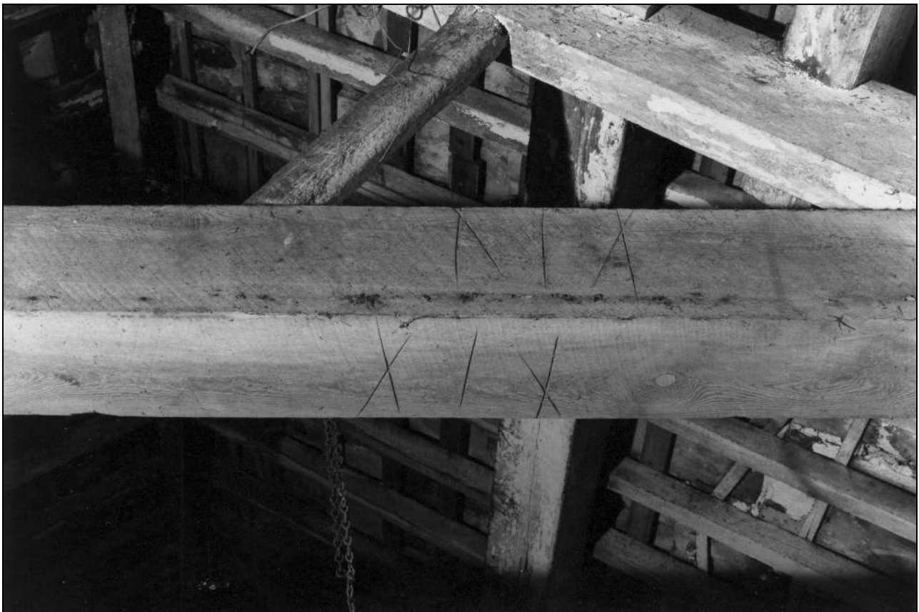
Photo 49: Detail of merchant's mark on central tie beam, from the east (film 4, frame 7)
