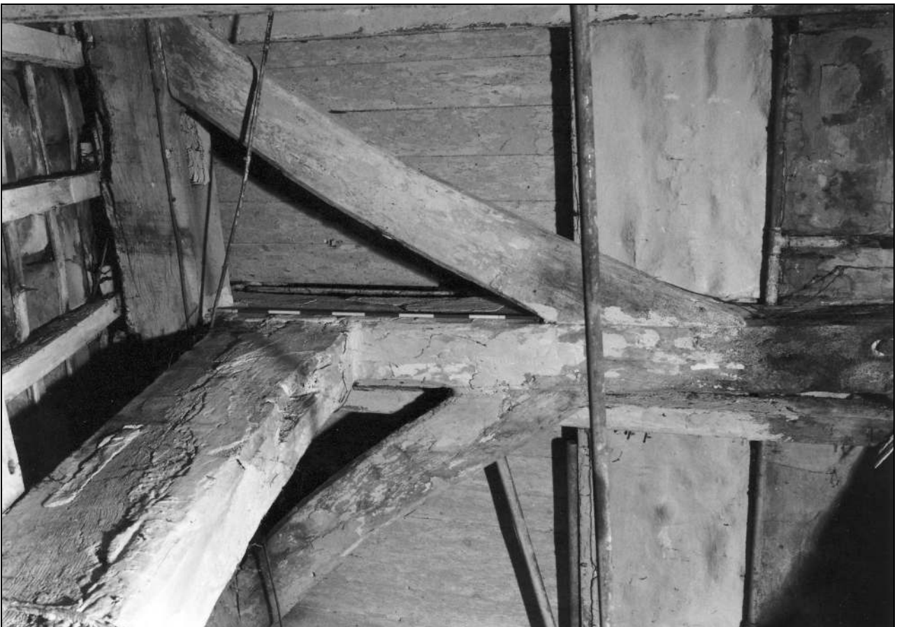
Photo 41: Arcade post, from the south (film 3, frame 1)
