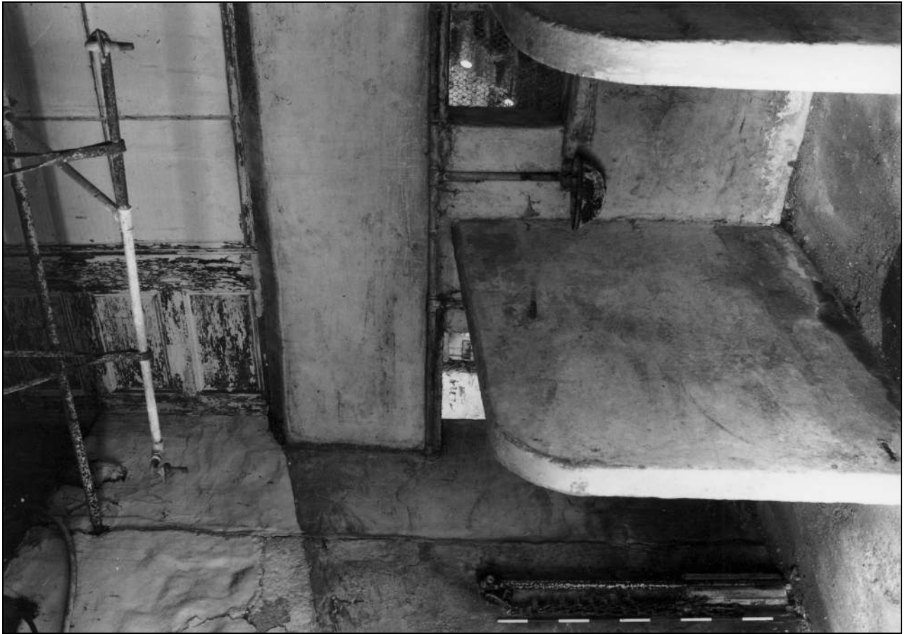
Photo 32: Shippon within south-east outshut, from the south-east (film 2, frame 1)
