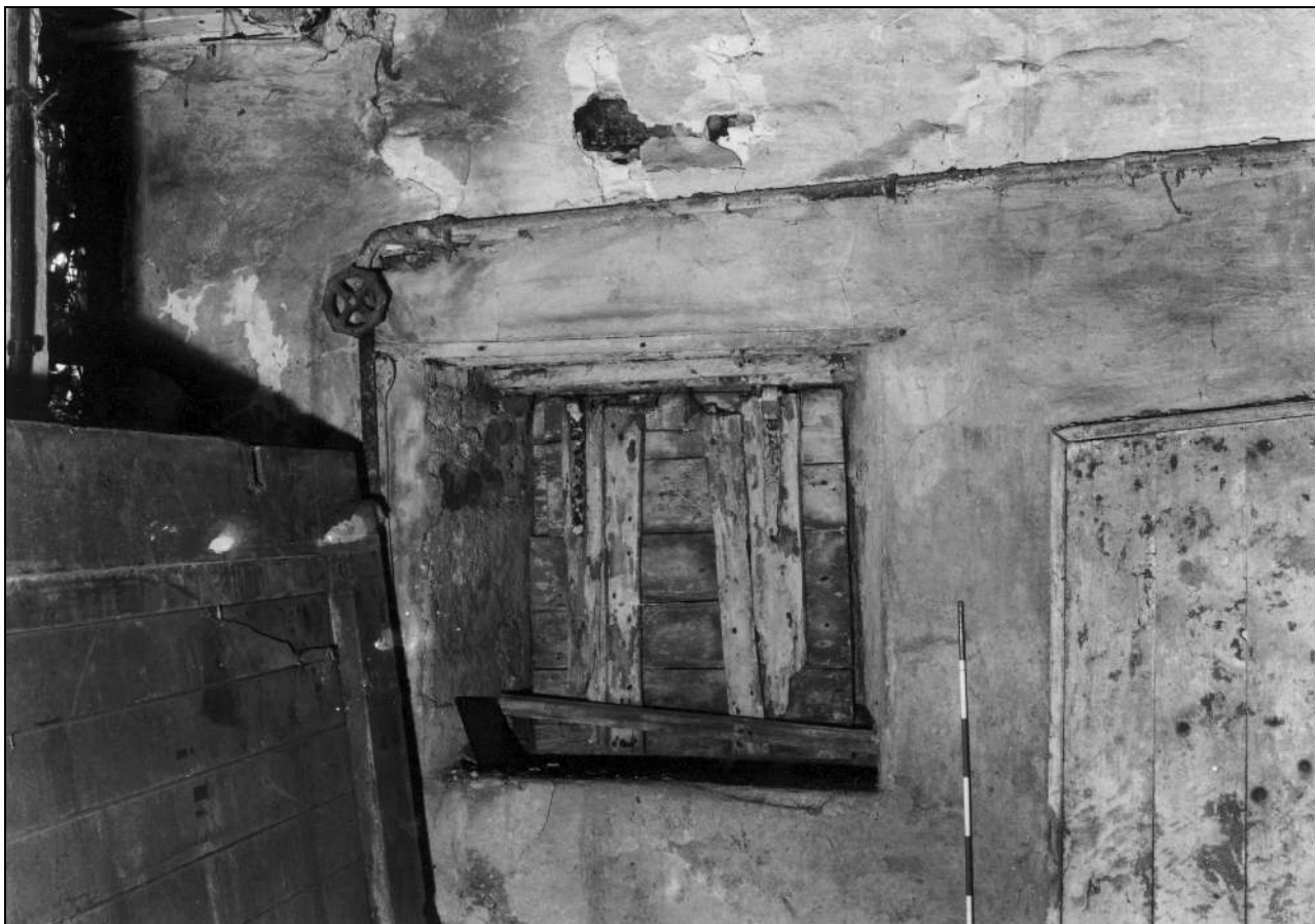
Photo 30: Mucking-out hole in west end of south-west outshut (film 2, frame 15)
