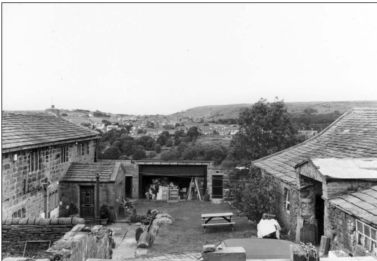
Photo 3: General view of the barn and farmhouse, from the east (film 1, frame 16)
