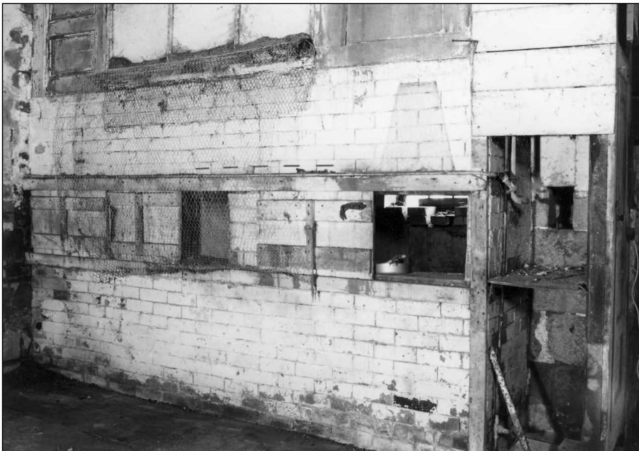
Photo 24: Brick wall to south-east outshut, from the north (film 3, frame 13)
