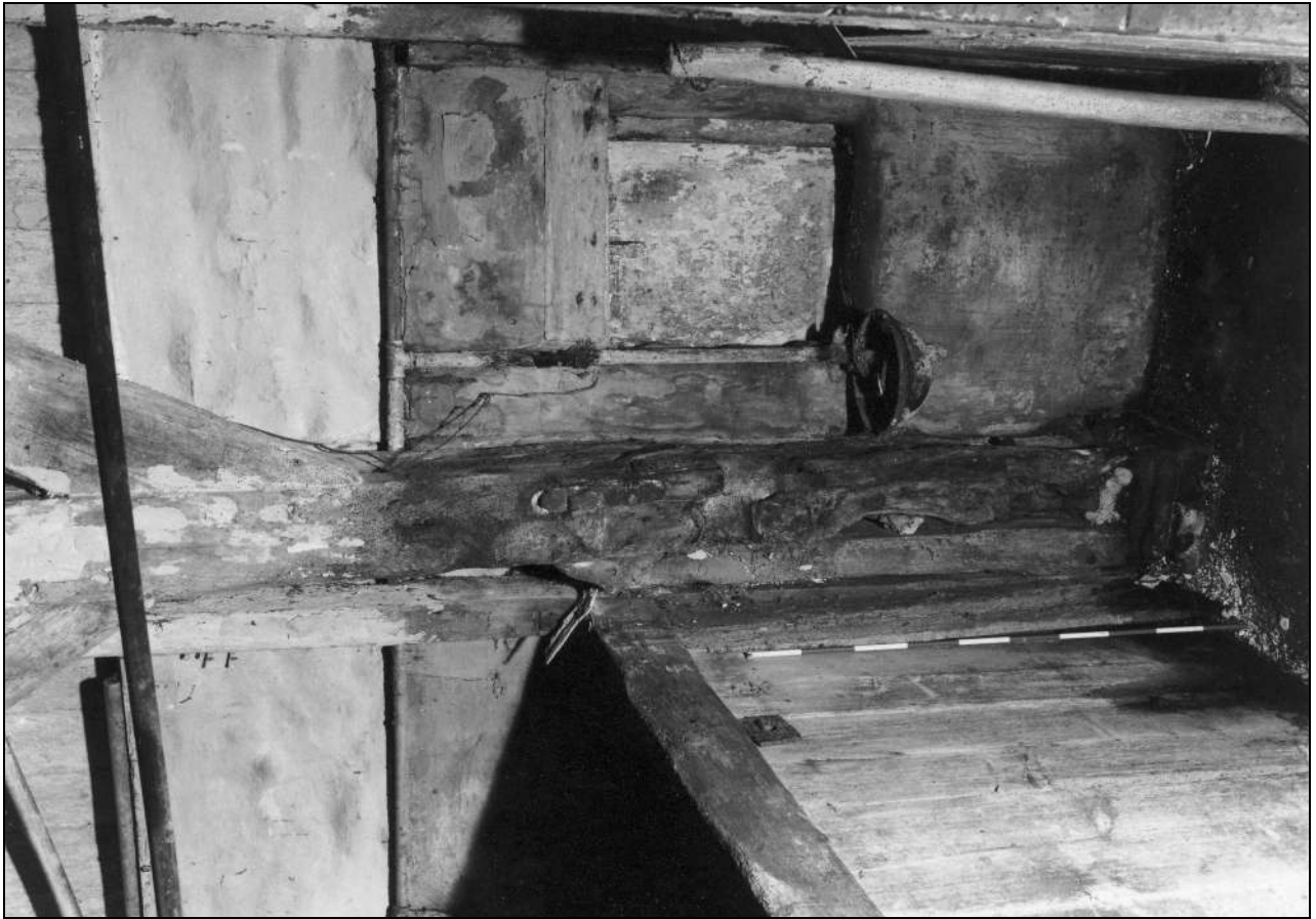
Photo 40: Foot of arcade post, from the south-east (film 3, frame 3)
