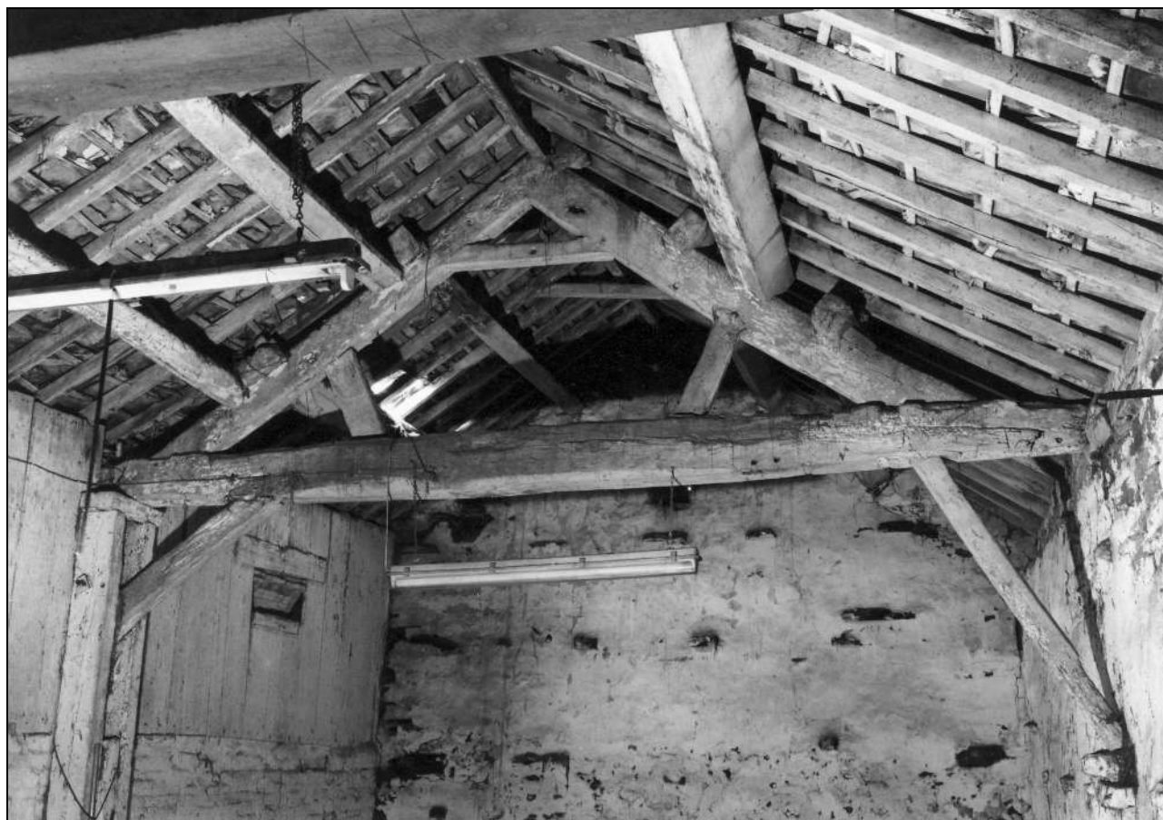
Photo 37: West roof truss, from the east (film 4, frame 9)
