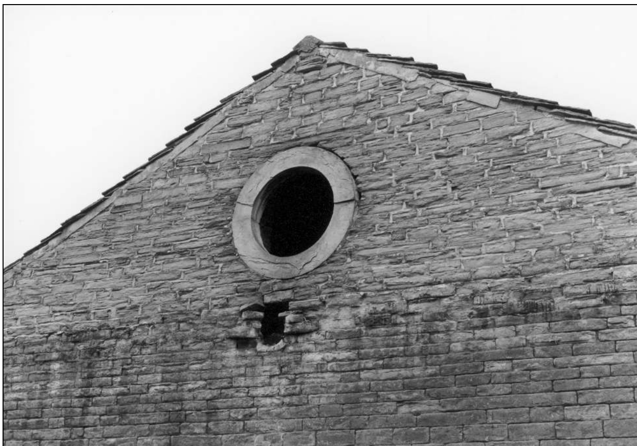
Photo 17: Detail of pitching eye in south gable (film 2, frame 4)
