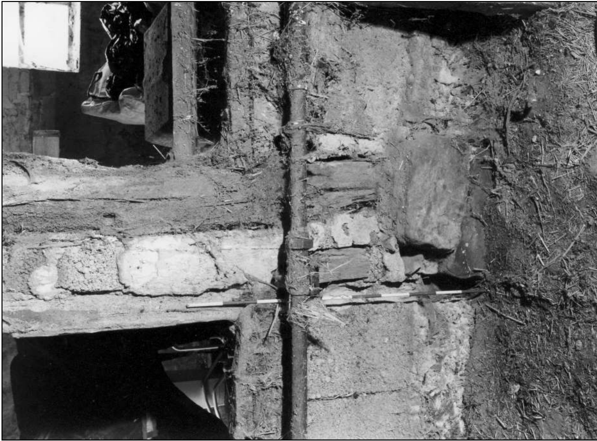
Photo 57: Truss 1: foot of arcade post and pad-stone, from the east (film 3, frame 17)
