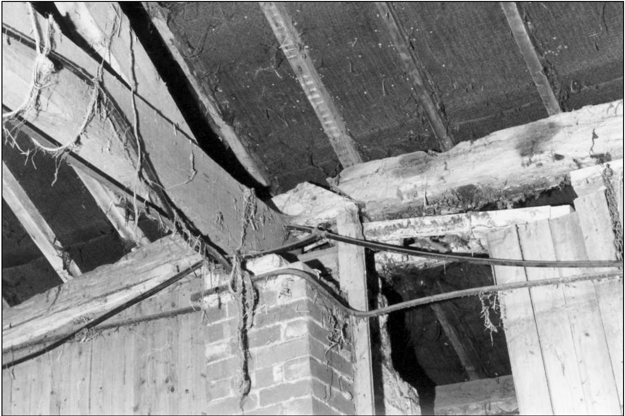
Photo 89: Scarf joint in arcade plate, north side of truss 5, from the east (film 6, frame 1)
