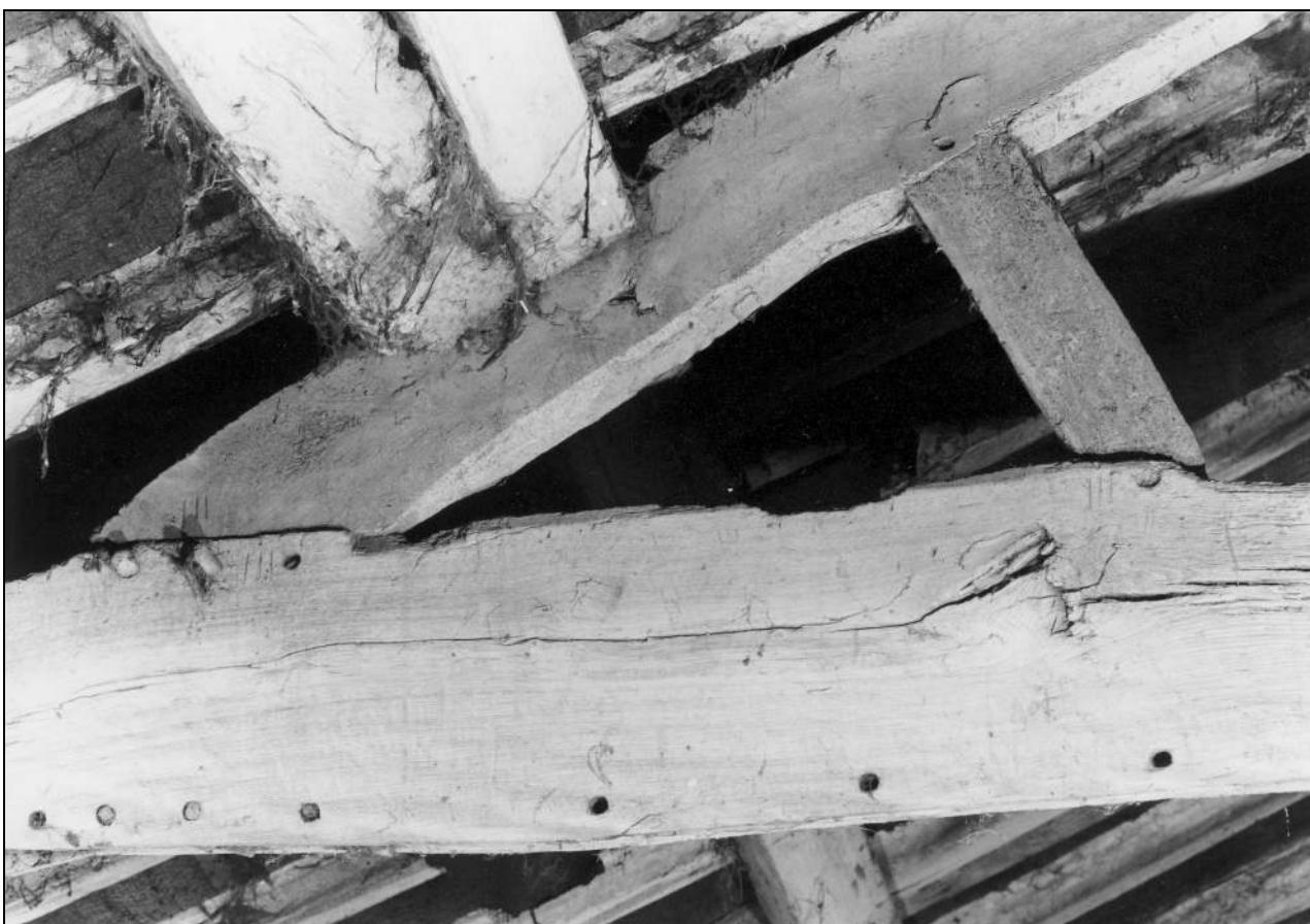
Photo 65: Truss 2: east end of tie beam, from the north, showing joint numbering "III" (film 4, frame 15)
