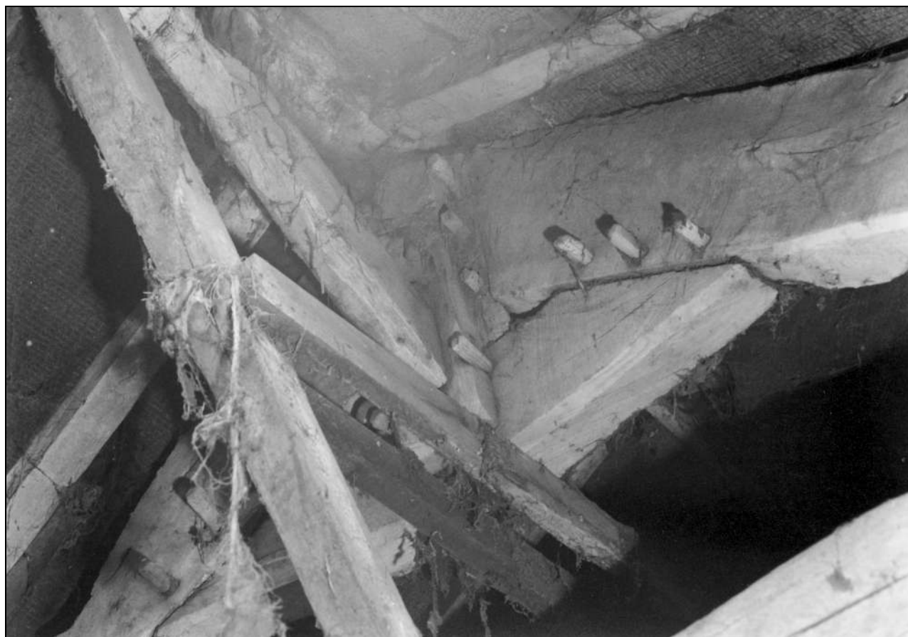
Photo 84: Truss 4: detail of king post and collar, from the south-east (film 5, frame 16)
