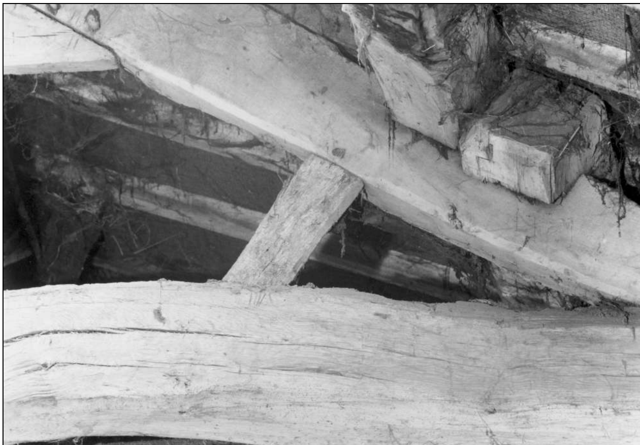
Photo 79: Truss 4: east strut above tie beam, from the south, showing joint numbering "IIIV" (film 5, frame 15)
