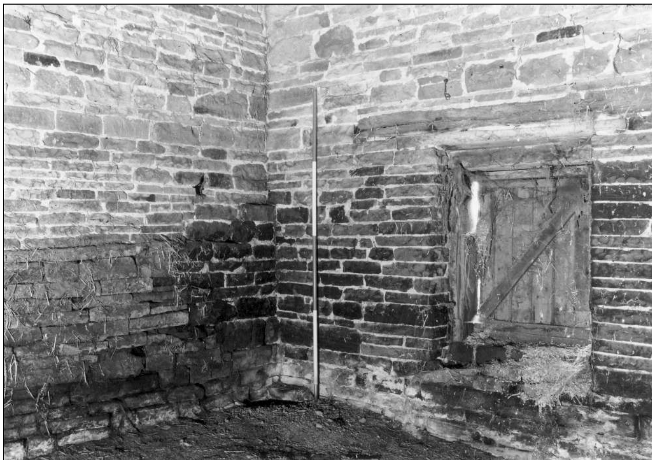
Photo 50: South-east corner inside barn, showing original stonework at left with rebuilt walls above and to right (film 3, frame 16)
