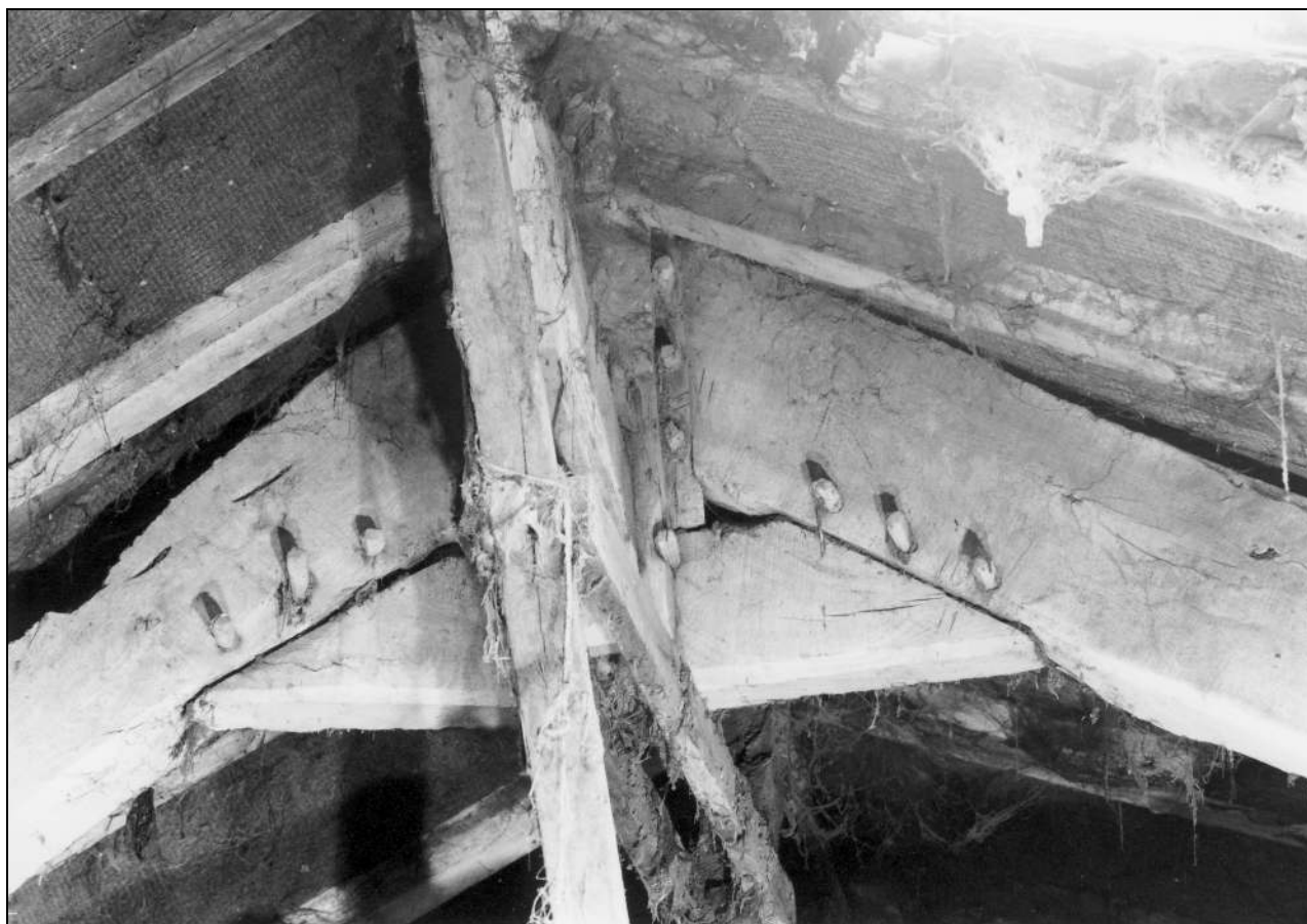
Photo 83: Truss 4: detail of king post and collar, from the south (film 5, frame 12)
