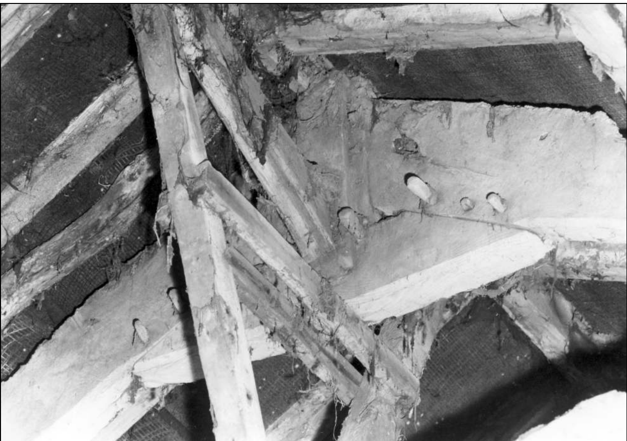
Photo 82: Truss 3: detail of king post and collar, from the north-west (film 4, frame 12)
