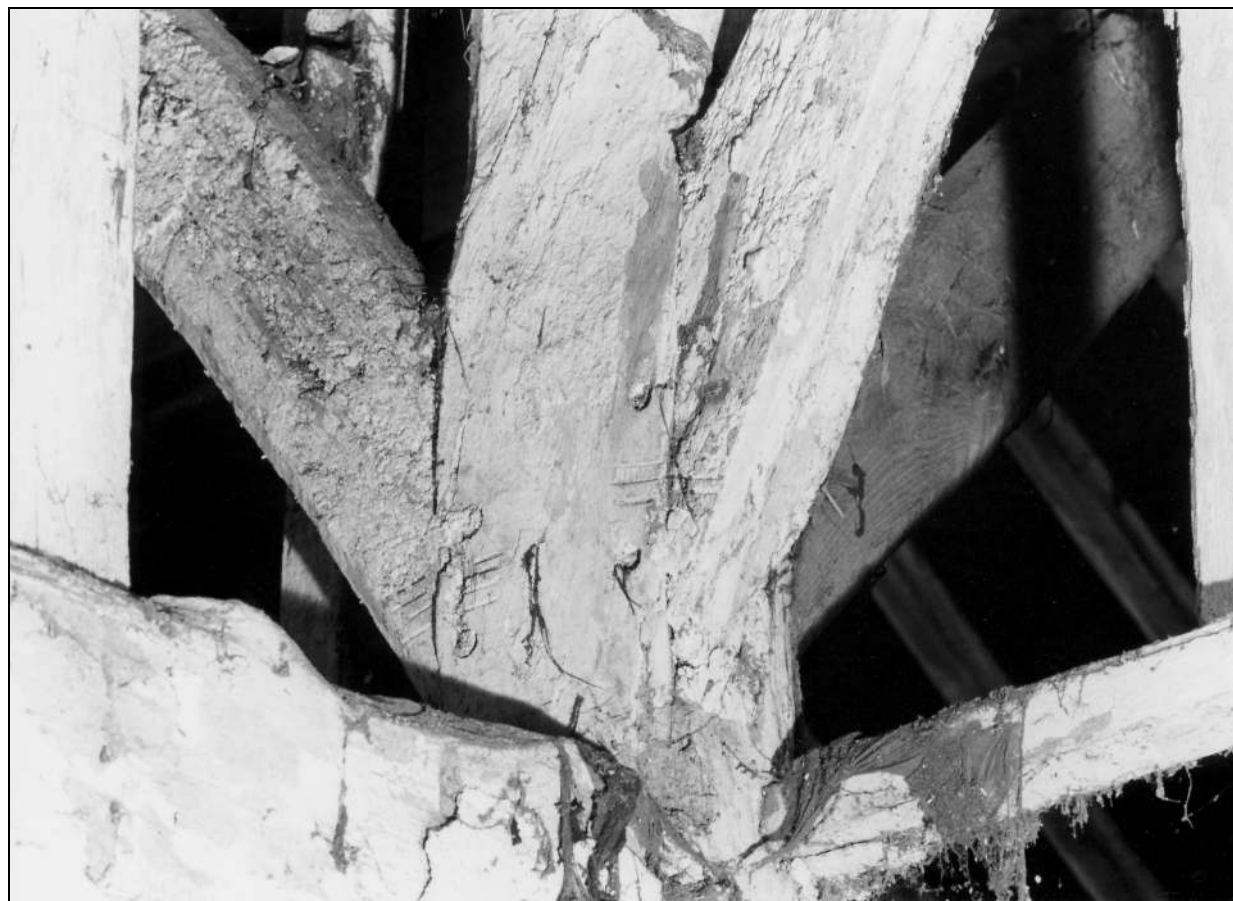
Photo 69: Truss 2: joint numbering "III" and "IIII" on arcade post and braces, from the south-west (film 6, frame 13)
