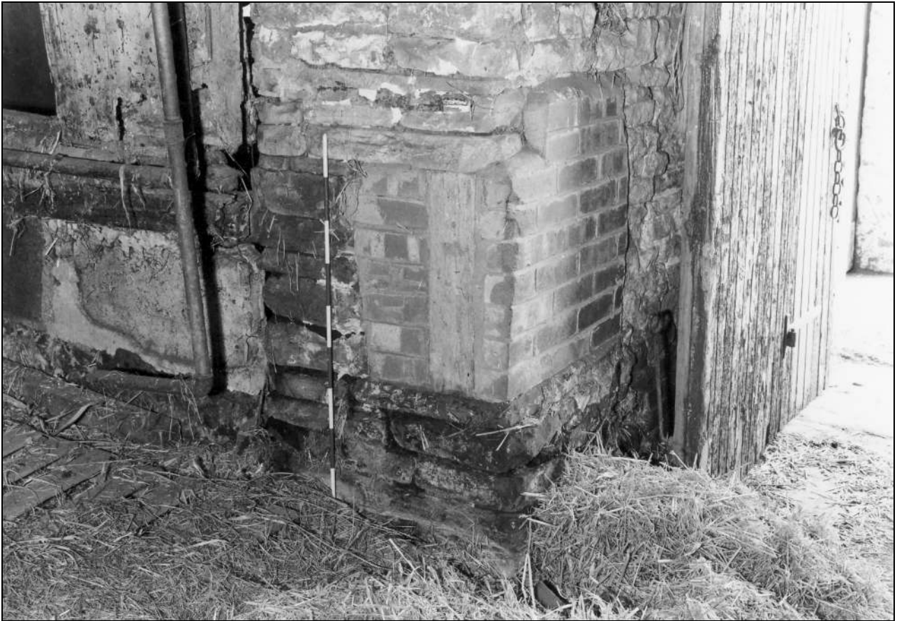
Photo 75: Brickwork repair and softwood timber in south side of west entry (film 4, frame 10)
