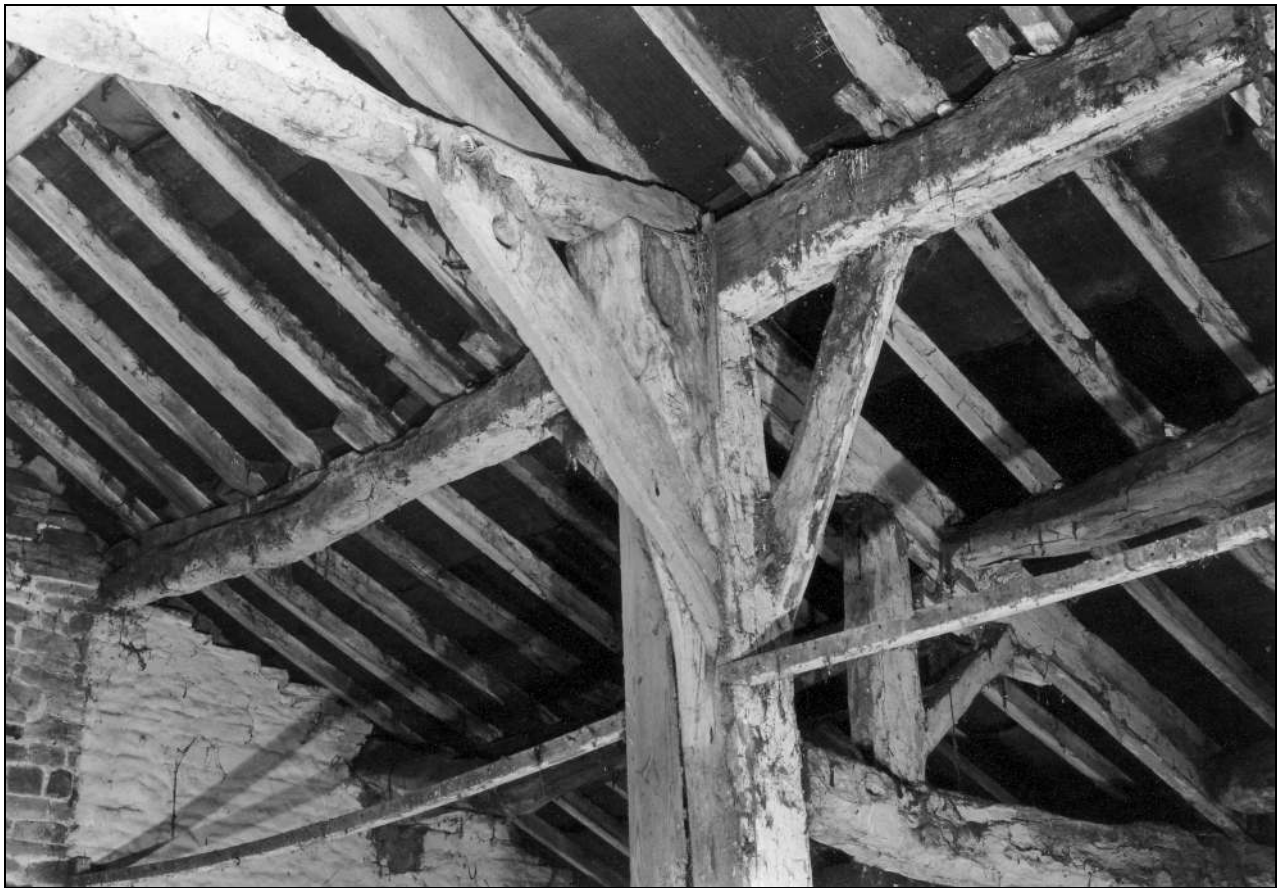
Photo 58: Truss 1: head of arcade post with original arcade plate and braces, with modern arch brace, from the north-east (film 4, frame 3)
