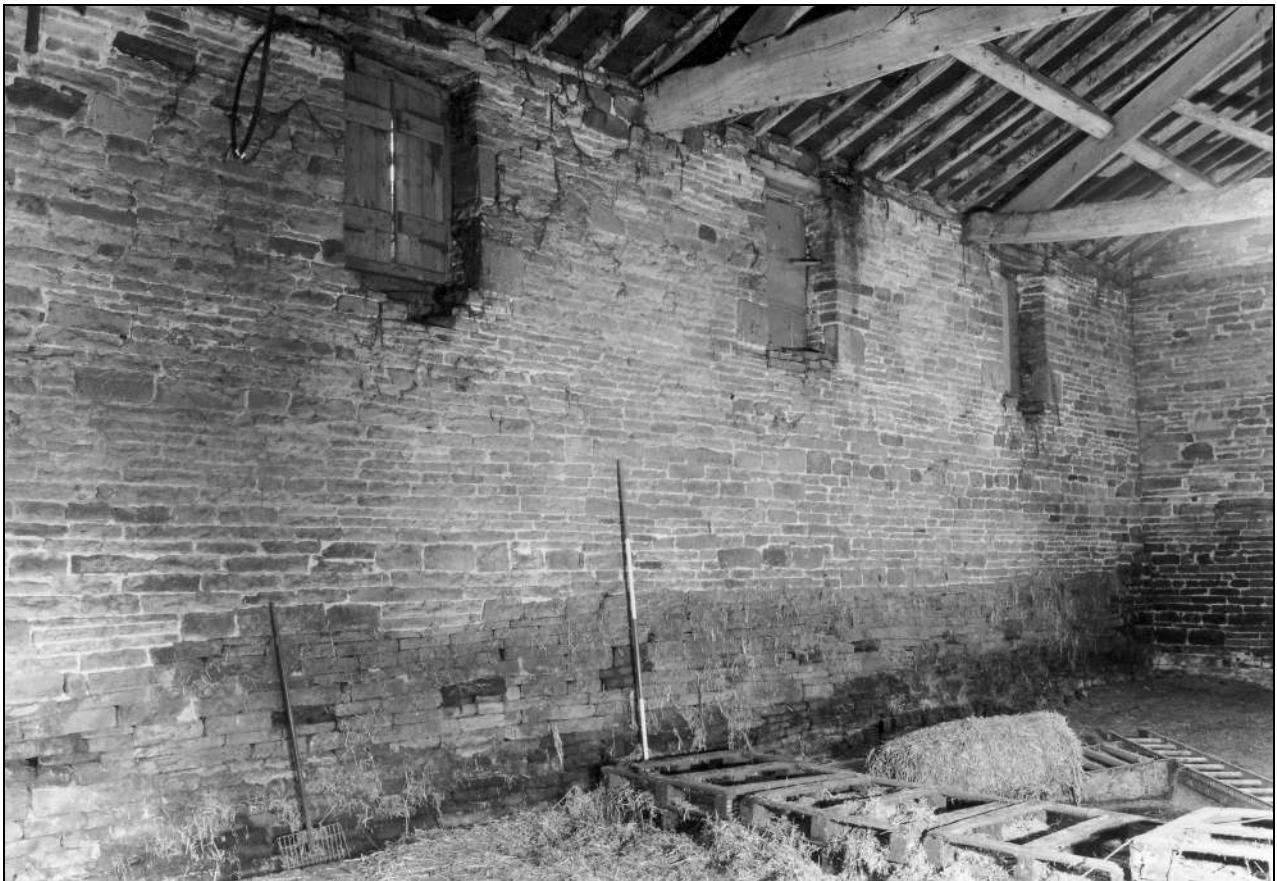
Photo 48: South end of east wall, inside barn, showing original stonework at foot with later openings above (film 3, frame 12)
