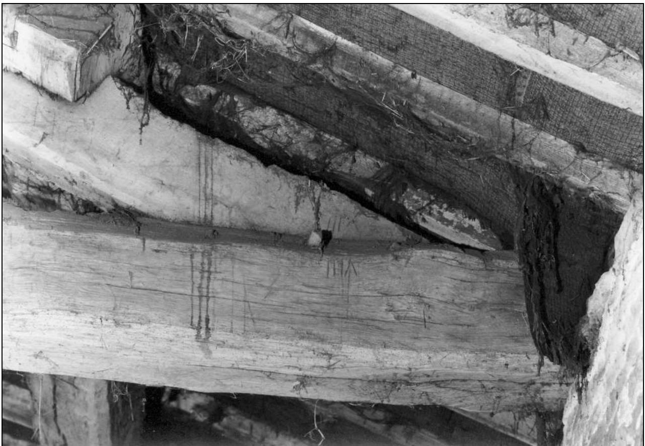
Photo 78: Truss 4: east end of tie beam, from the south, showing joint numbering "IIIV" (film 5, frame 13)
