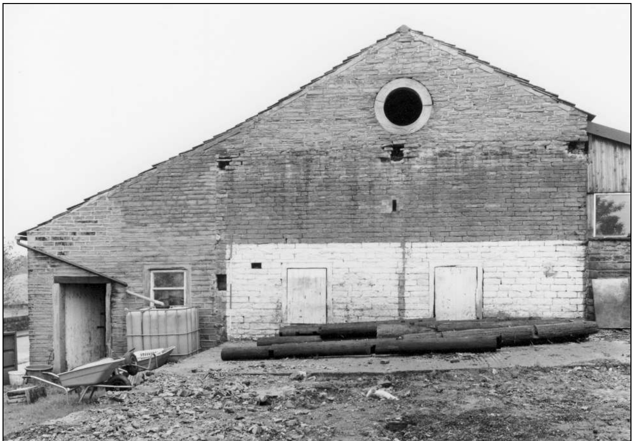
Photo 14: The rebuilt south gable, with nineteenth century openings (film 1, frame 16)
