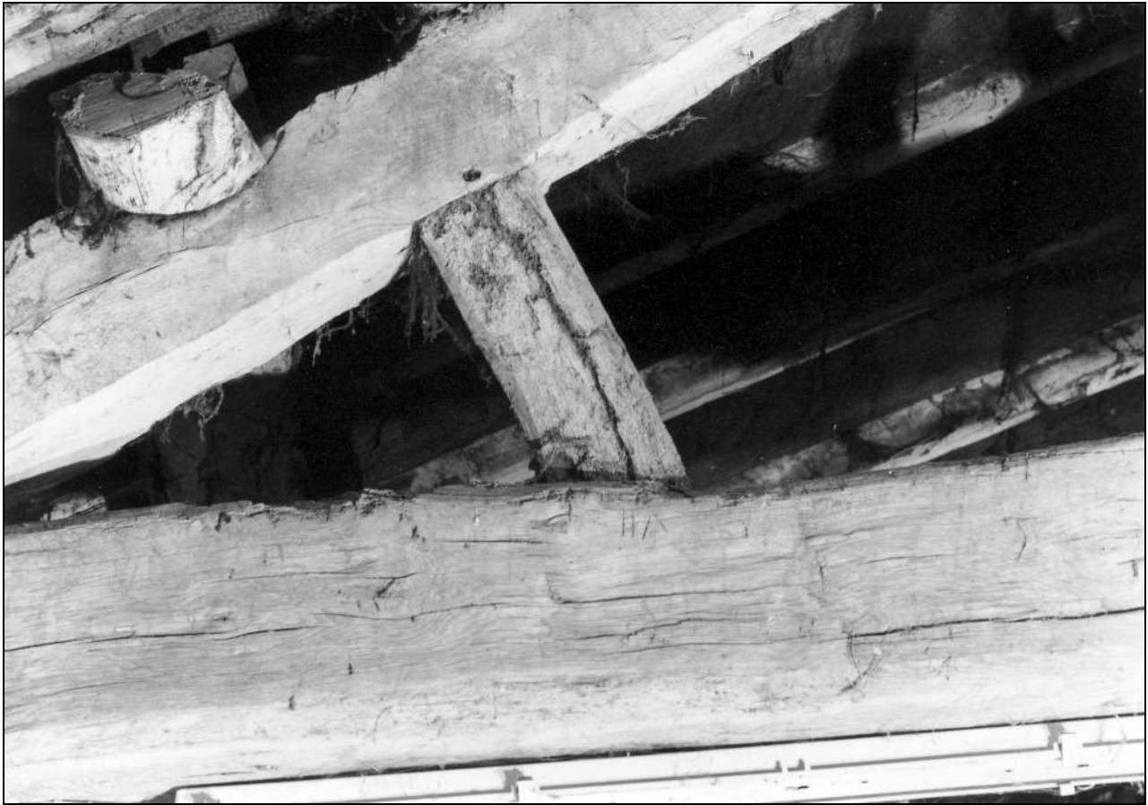
Photo 77: Truss 4: west strut above tie beam, from the south, showing joint numbering "IIIV" (film 5, frame 11)
