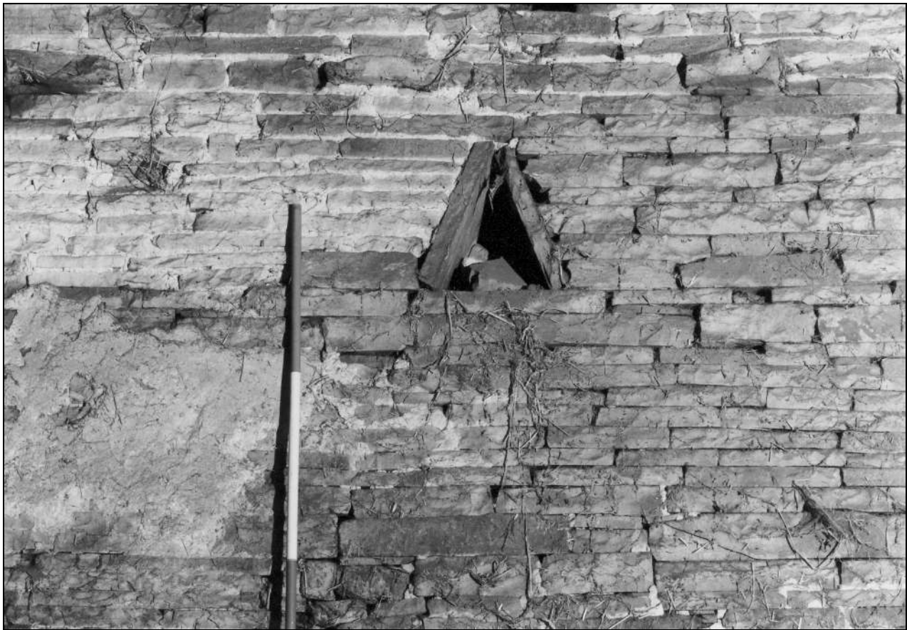
Photo 52: Blocked triangular breather in inside face of east wall (film 5, frame 3)
