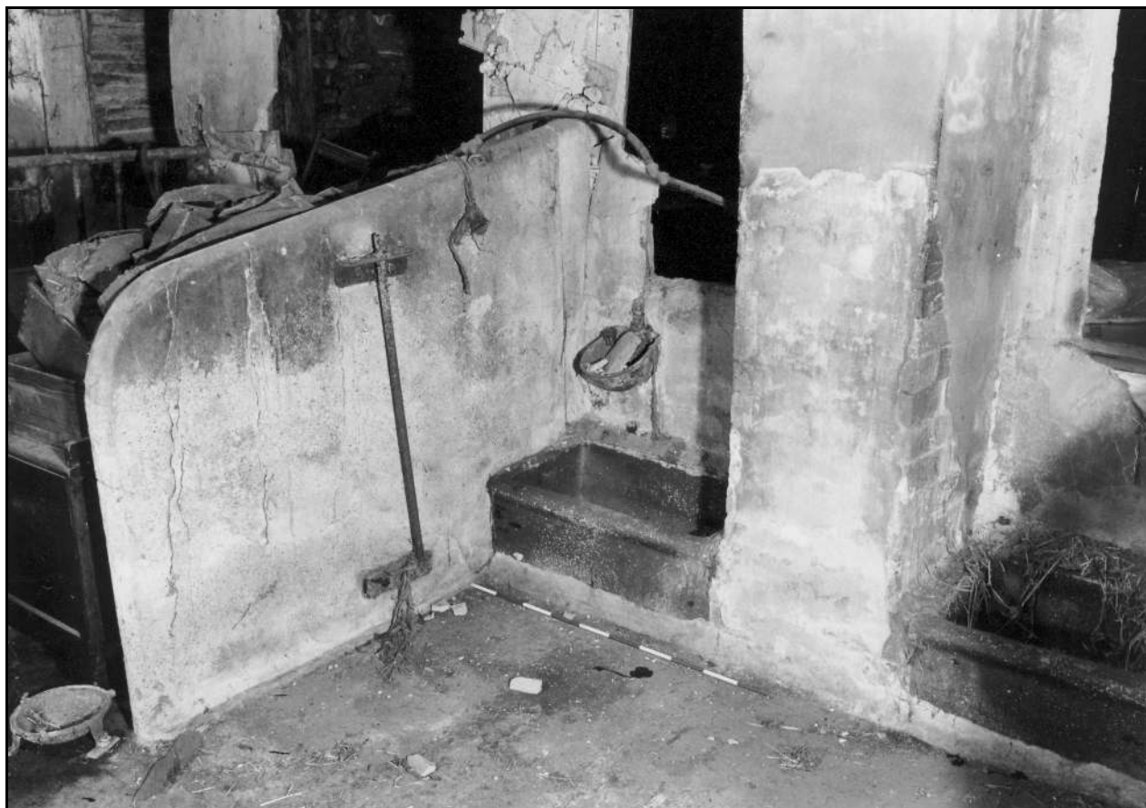
Photo 98: Detail of concrete boskin and ceramic trough, north part of aisle, from the south-west (film 7, frame 3)
