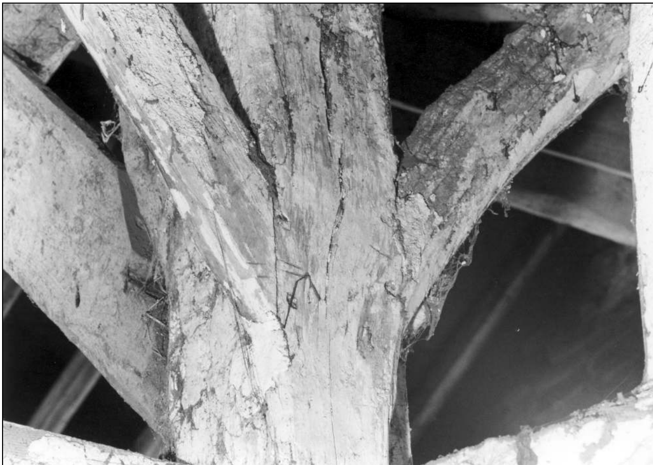
Photo 60: Truss 1: joint numbering "I" and "II" on arcade post and braces, from the north-west (film 6, frame 12)
