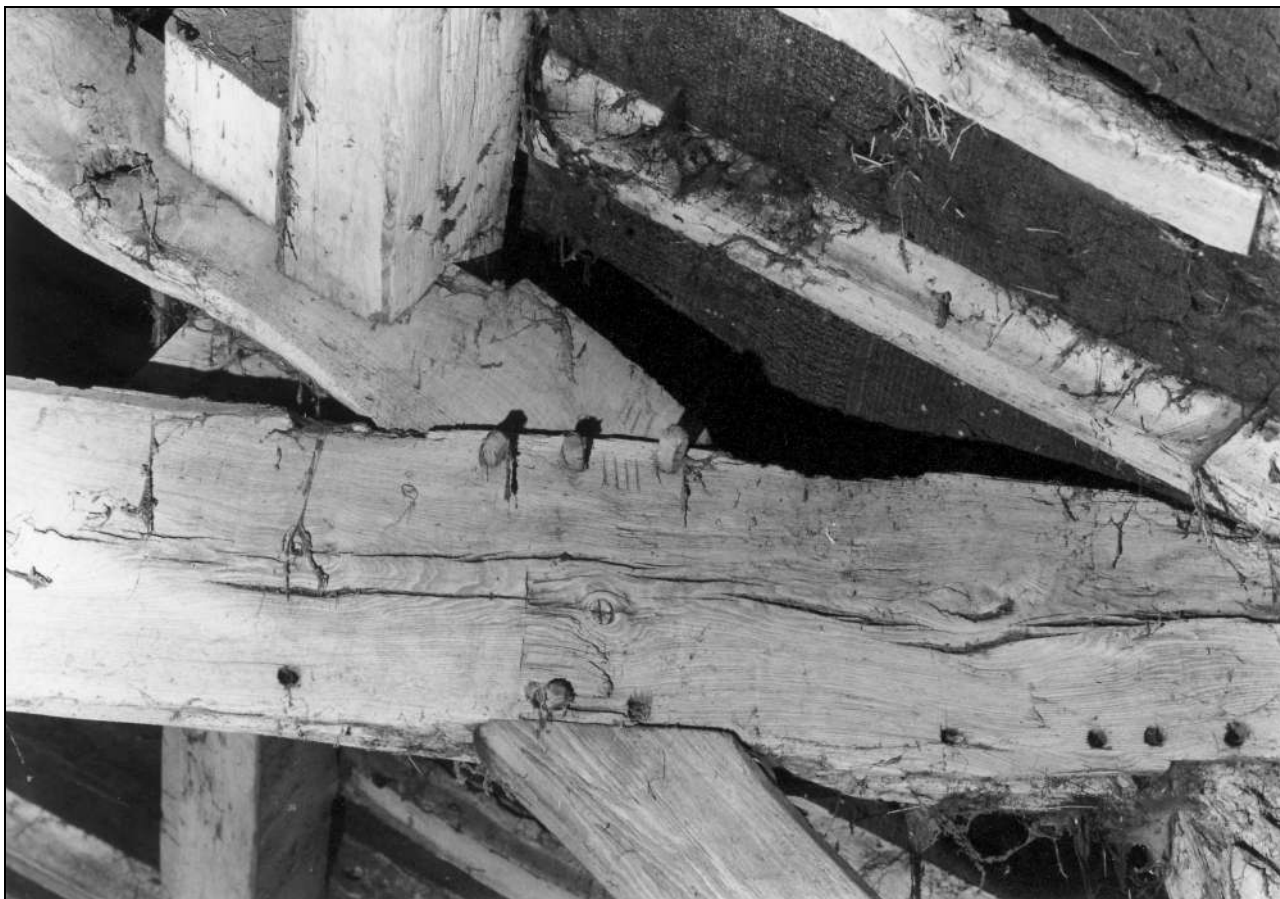
Photo 66: Truss 2: west end of tie beam, from the north, showing joint numbering "IIII" (film 4, frame 14)
