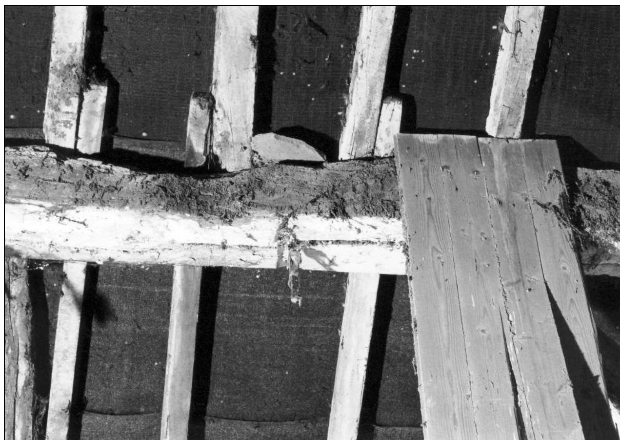
Photo 88: Scarf joint in arcade plate, between trusses 1 and 2, from the east (film 6, frame 4)
