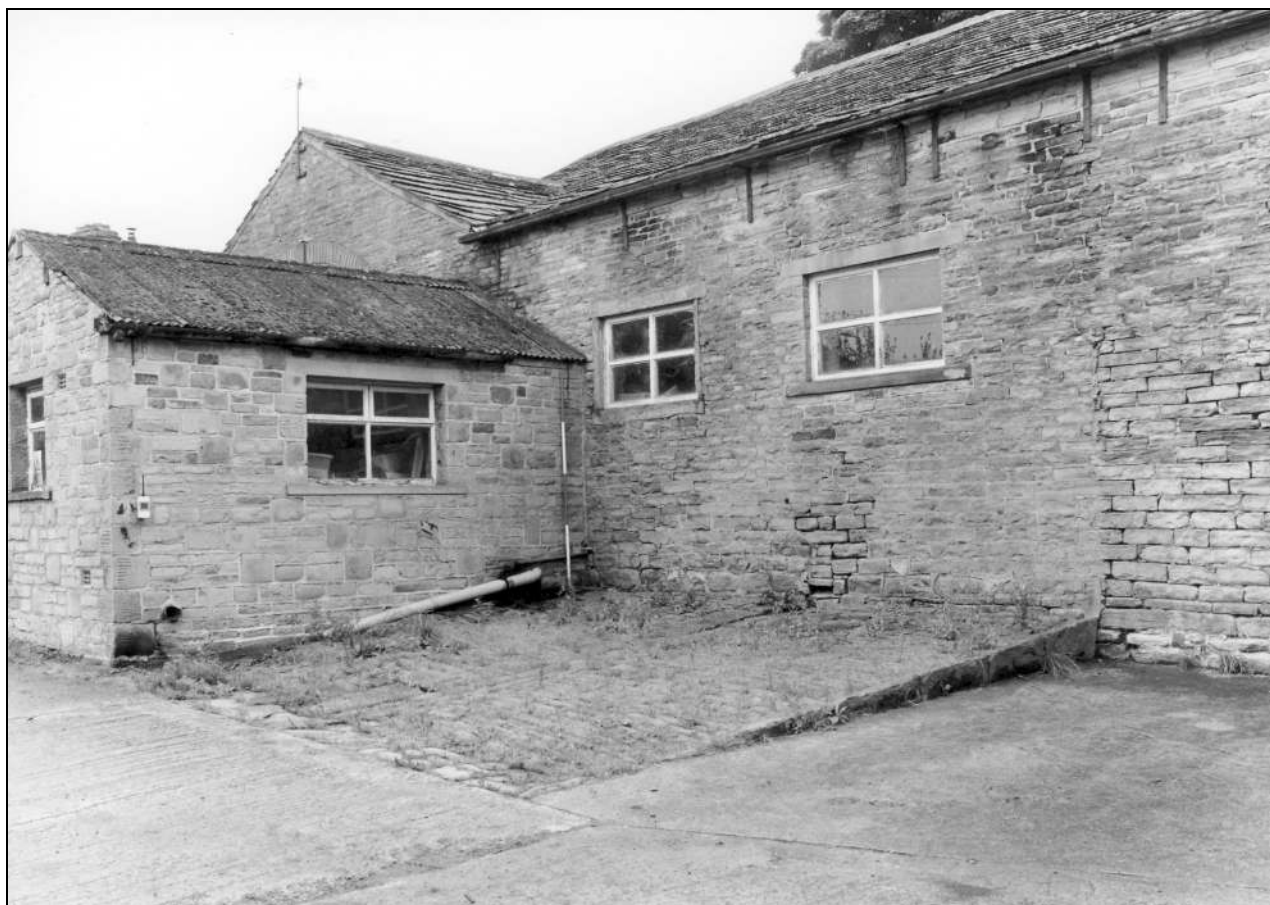
Photo 12: West elevation of barn to south of entrance, with pitched stone surfacing and inserted windows (film 1, frame 15)
