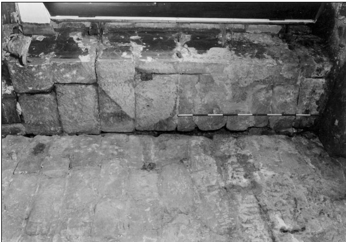
Photo 29: South-east corner of hearth passage, showing location of wall post (film 2, frame 18)
