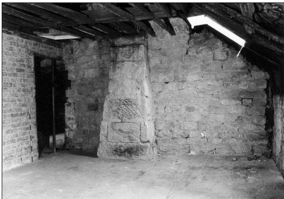
Photo 37: Chamber over housebody, from the south-west, showing eighteenth/early nineteenth century stack for housebody fireplace (film 6, frame 1)
