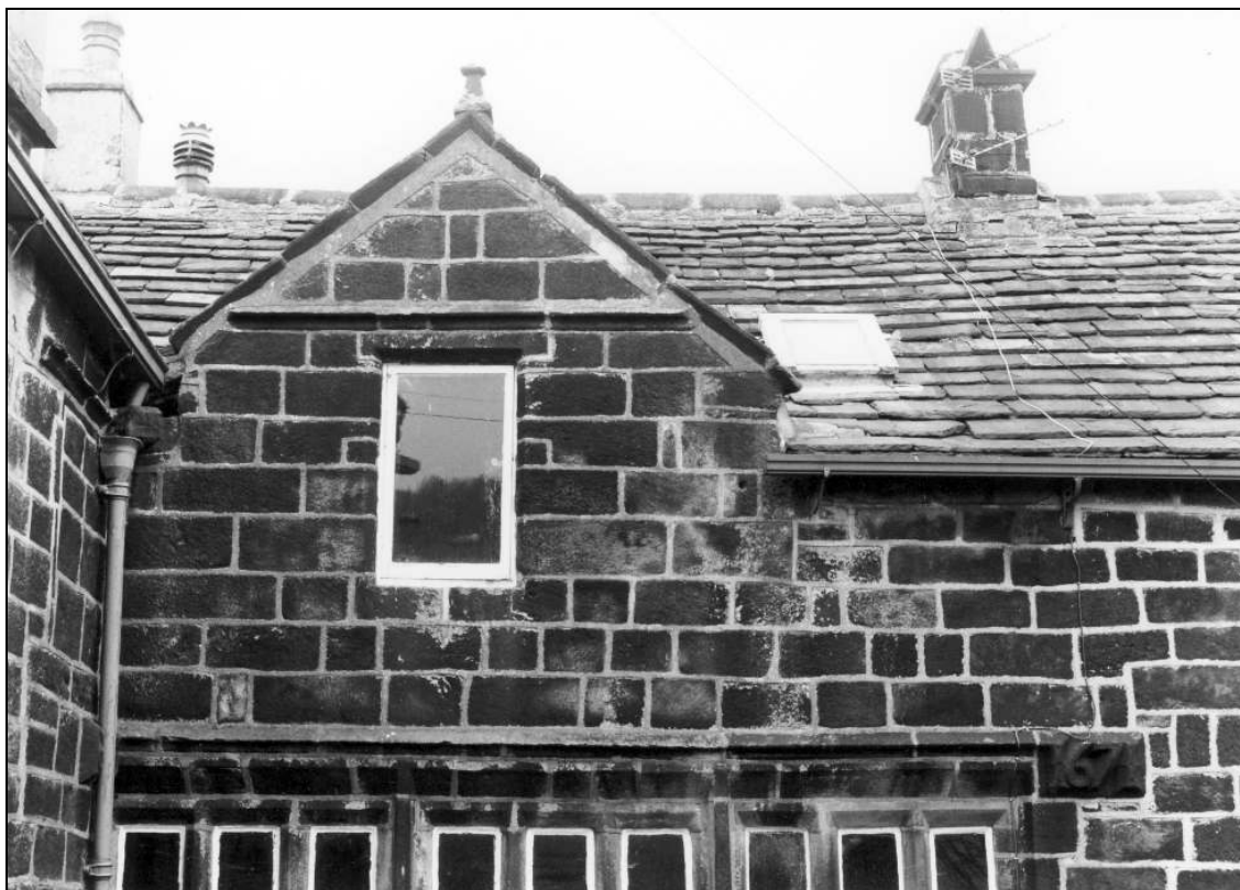
Photo 15: Gablet to chamber over housebody (film 6, frame 13)
