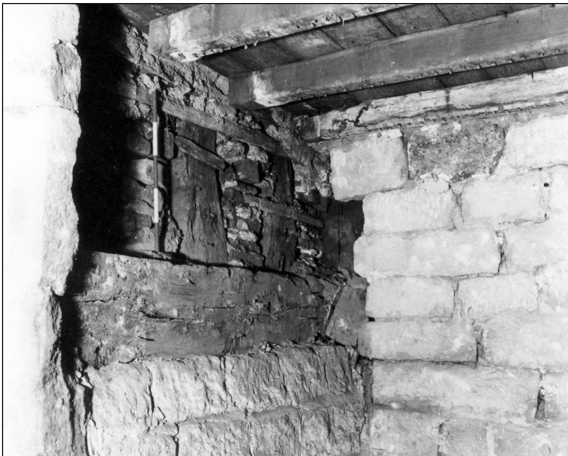
Photo 42: Detail of studs and mid rail in south wall of housebody; wall post just visible within cross wall (film 3, frame 15)
