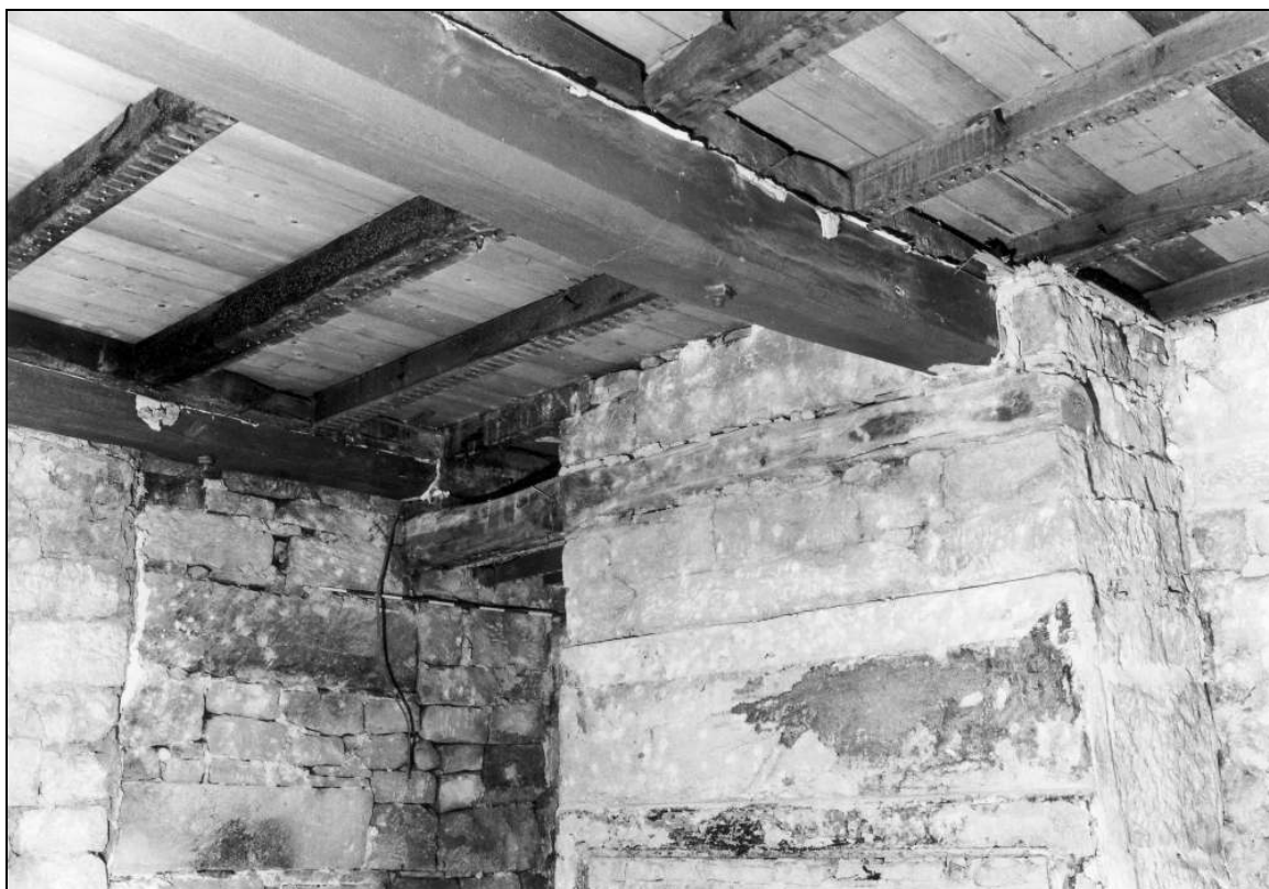
Photo 36: Detail of floor frame with scarf joints in spine beams, over housebody fireplace, from the south-west (film 3, frame 9)
