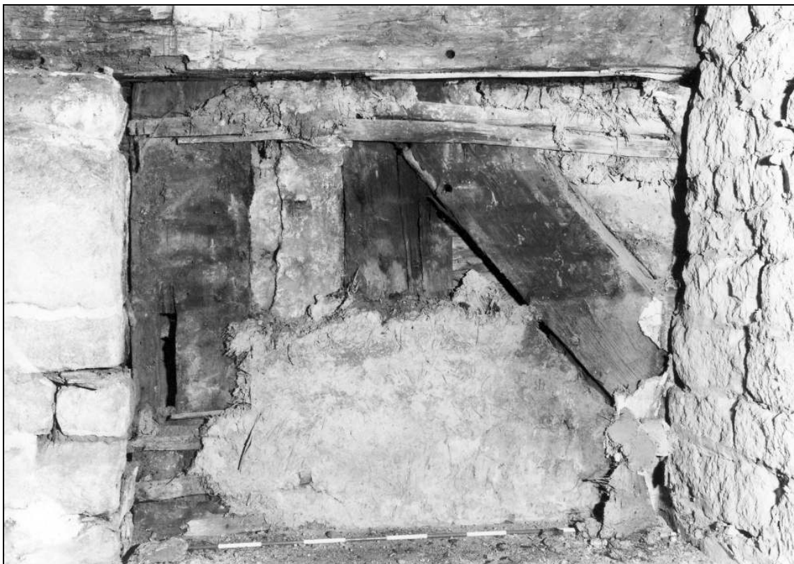
Photo 44: Chamber over housebody: exposed studs and brace, with daub covering below wall plate (film 6, frame 7)
