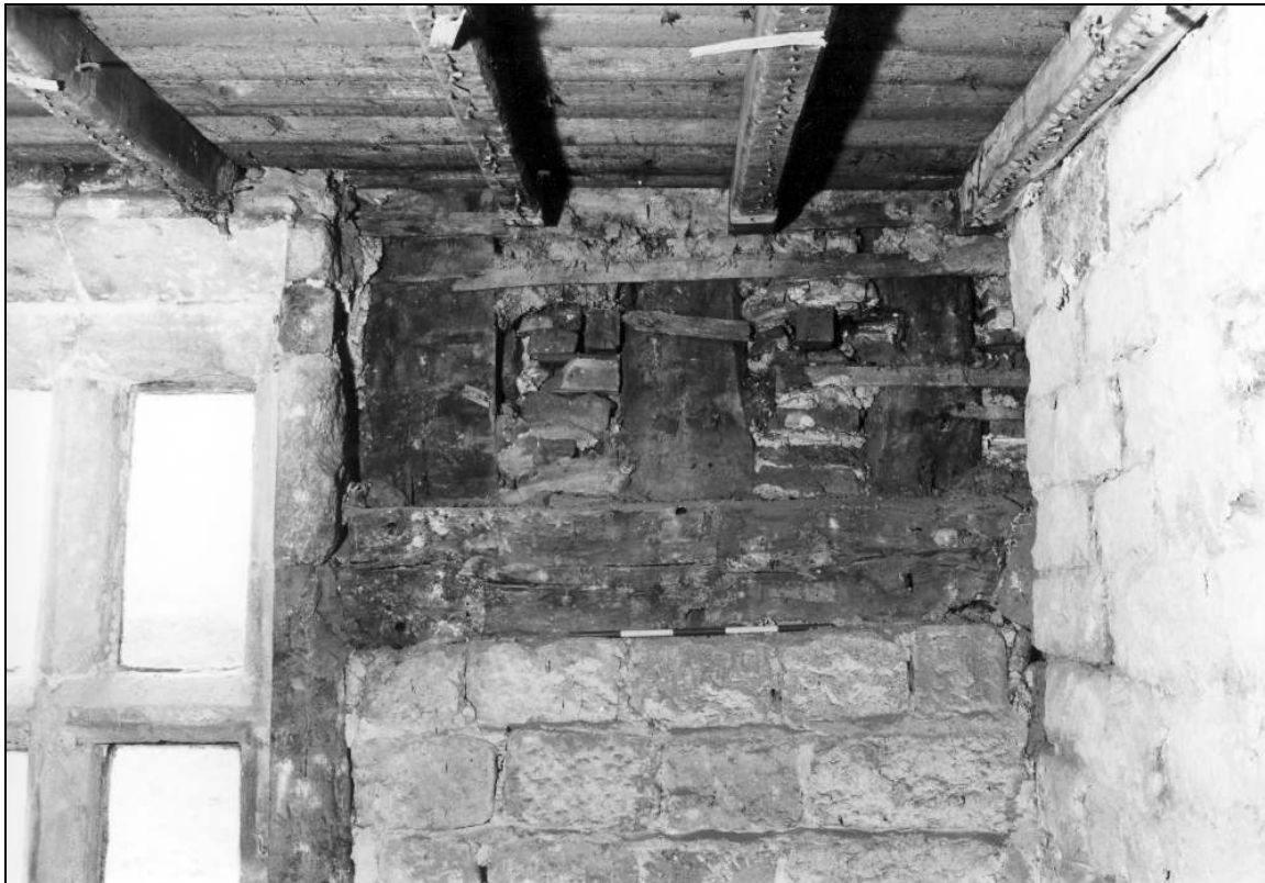
Photo 41: Detail of studs and mid rail in south wall of housebody, (with west wing beyond) (film 3, frame 13)
