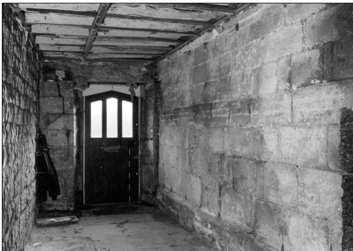
Photo 27: The hearth passage, from the north, showing ashlar reredos to right (film 2, frame 15)
