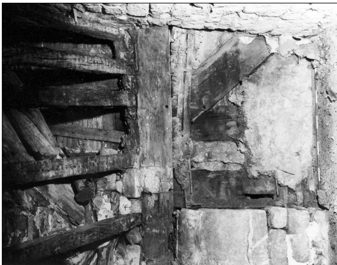
Photo 42: Detail of studs and mid rail in south wall of housebody; wall post just visible within cross wall (film 3, frame 15)
