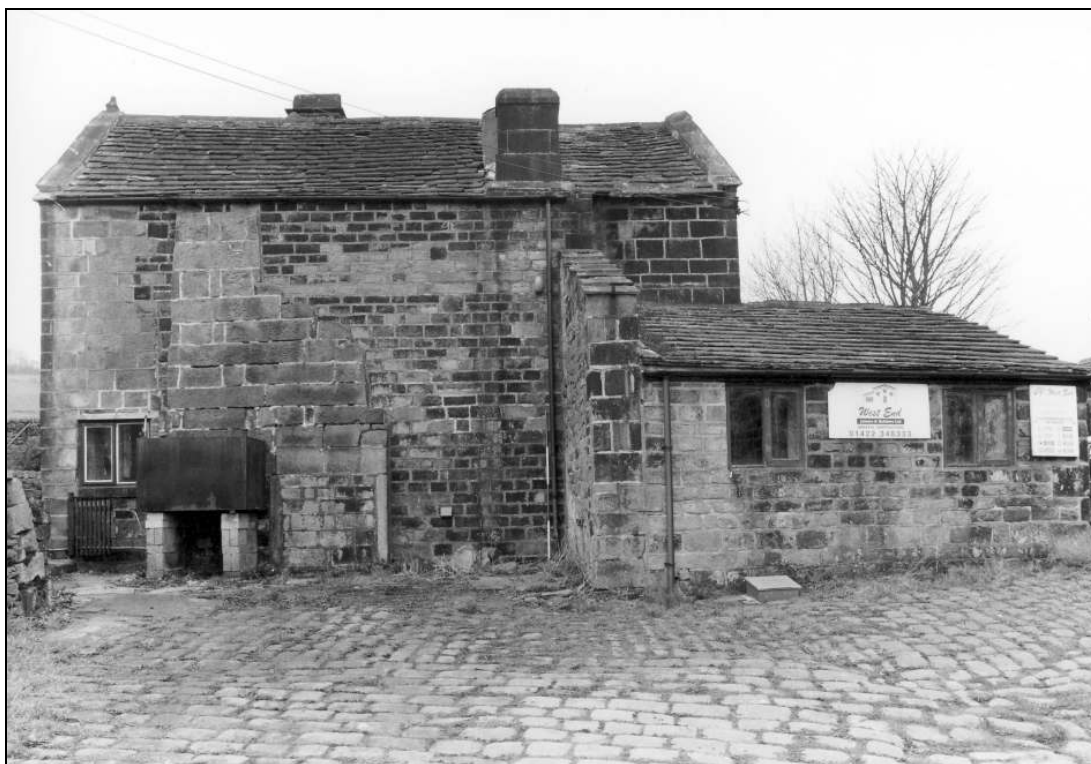
Photo 16: East end of house, showing site of demolished lean-to cottage and dairy at corner (film 1, frame 18)
