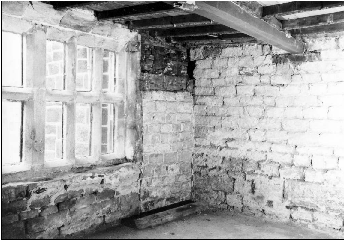
Photo 40: The housebody, from the north-east: note mid rail with studs above, in corner (film 3, frame 11)
