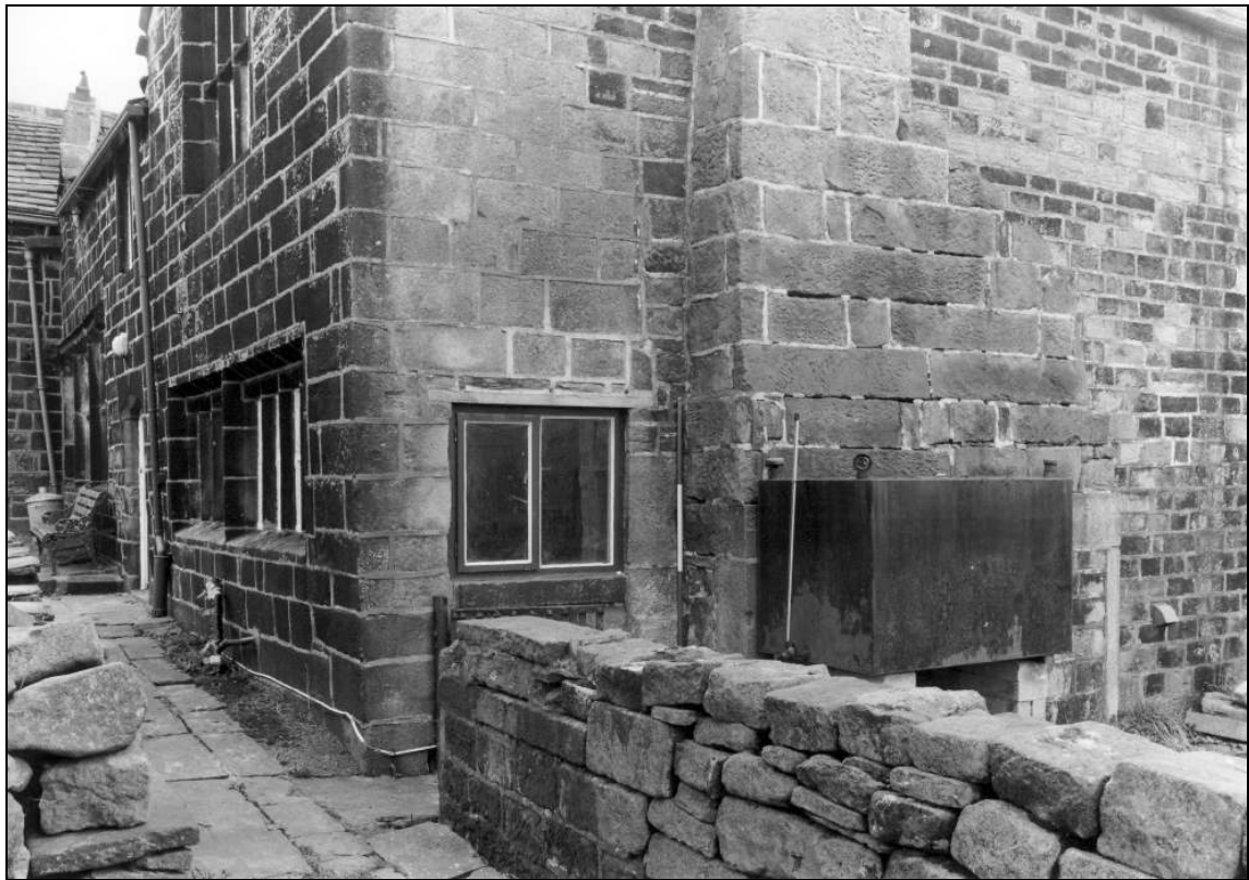
Photo 18: East side of east wing, showing chimney breast of cottage fireplaces (film 2, frame 4)
