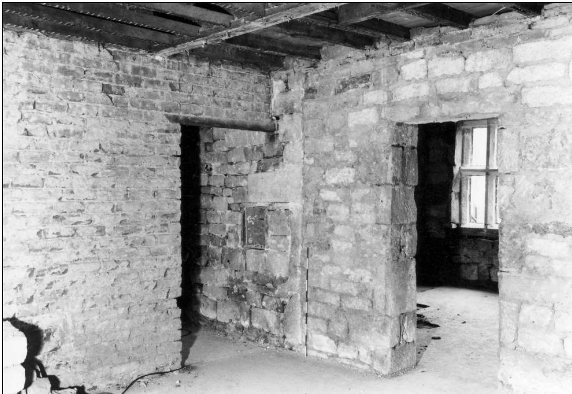
Photo 46: Kitchen, from the north-west, with walls of 1886 to left and right, the latter butting earlier heck (film 3, frame 18)
