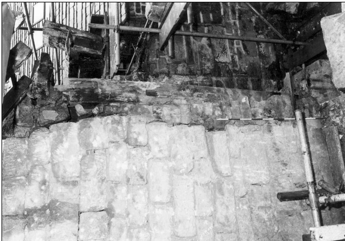
Photo 89: Remains of post at north-east corner of house (first floor), revealed during repairs (film 7, frame 5)
