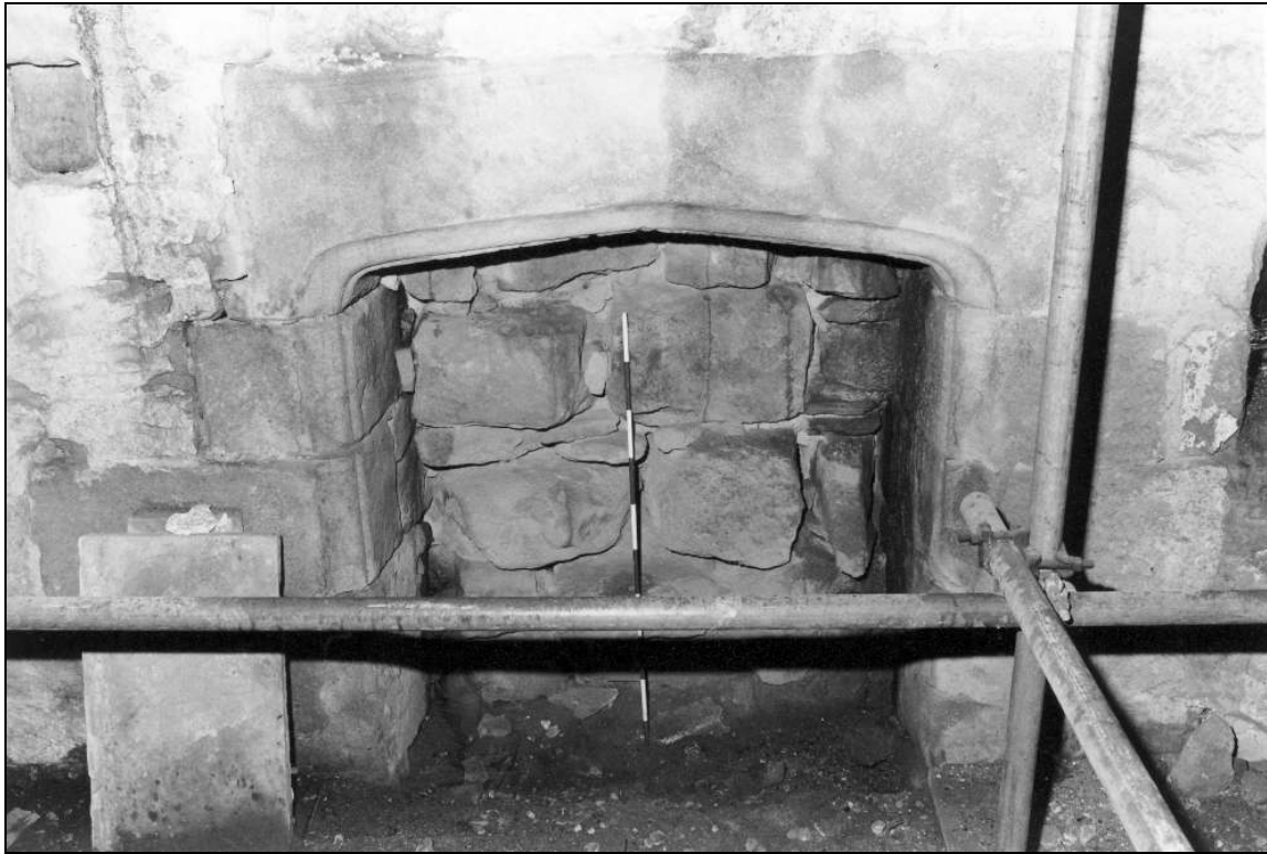
Photo 54: Seventeenth century fireplace in parlour, as revealed during repairs (film 7, frame 4)
