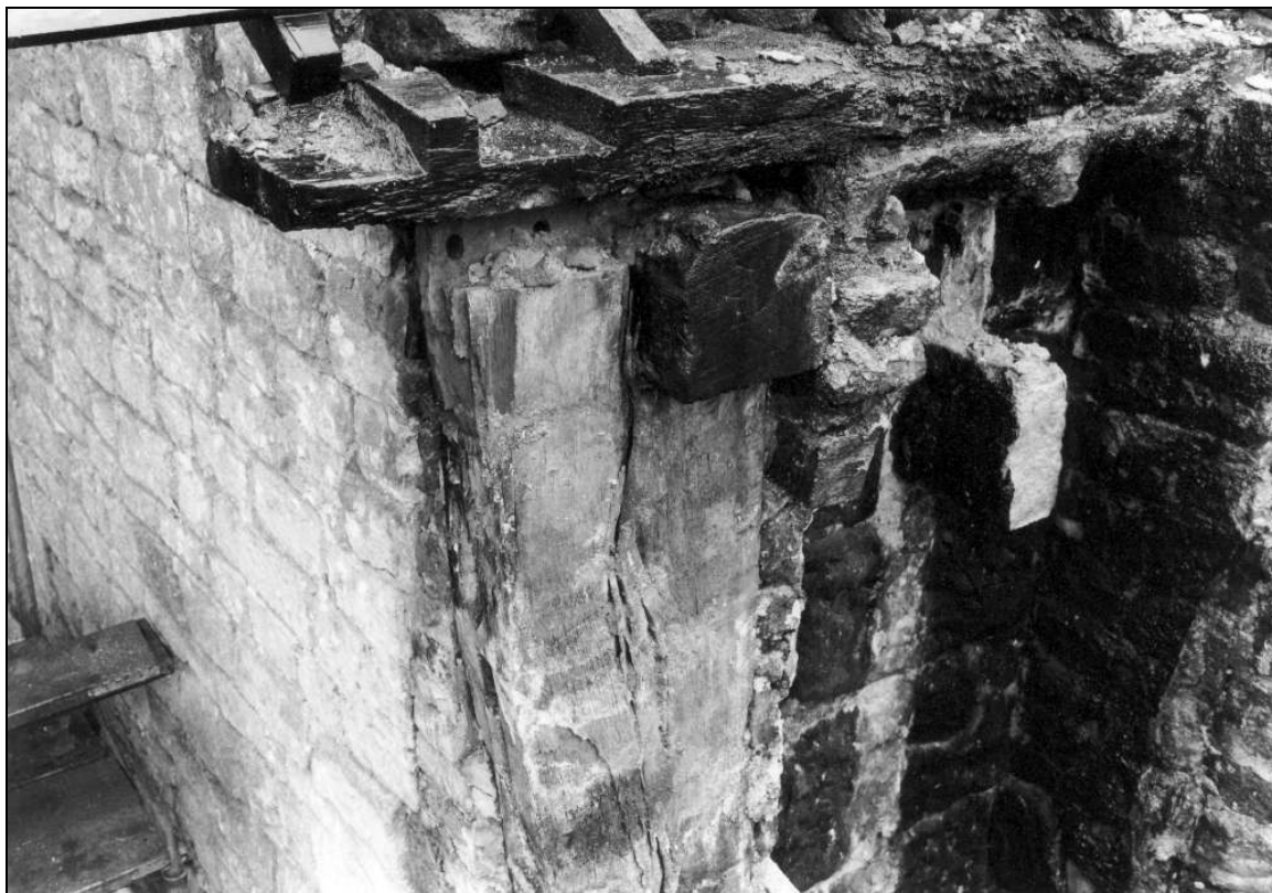
Photo 90: Remains of post at north-east corner of house (first floor), revealed during repairs (film 7, frame 6)
