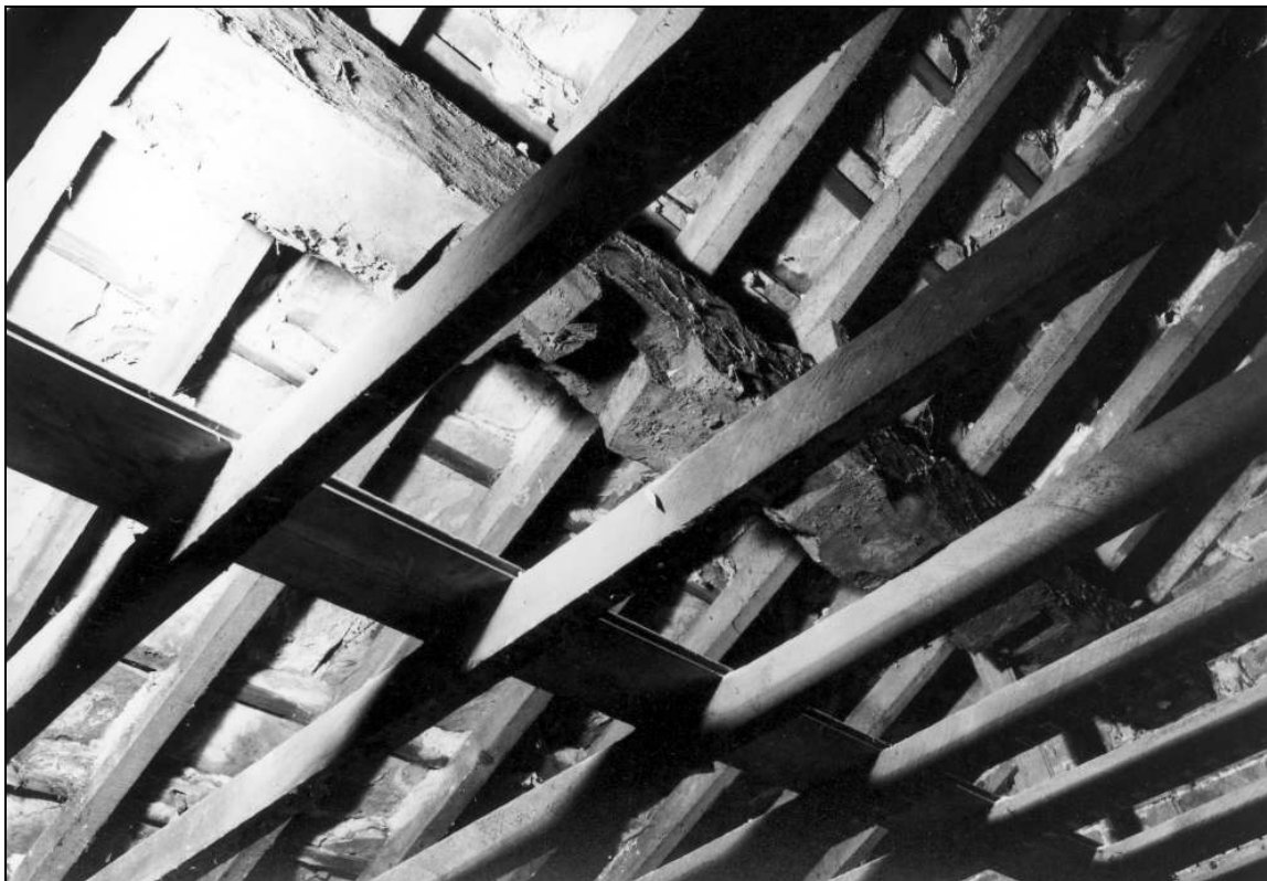
Photo 75: Wall or arcade plate re-used as purlin, over kitchen, from the south-west (film 4, frame 1)
