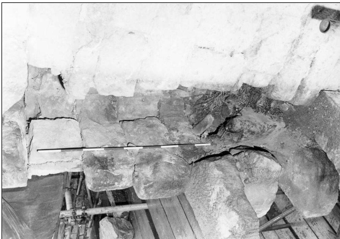
Photo 86: Remains of post at south-east corner of house (first floor), revealed during repairs (film 7, frame 2)
