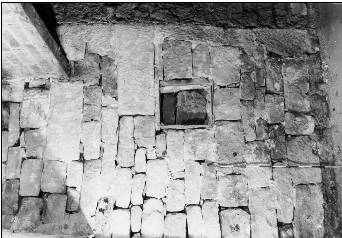
Photo 46: Kitchen, from the north-west, with walls of 1886 to left and right, the latter butting earlier heck (film 3, frame 18)
