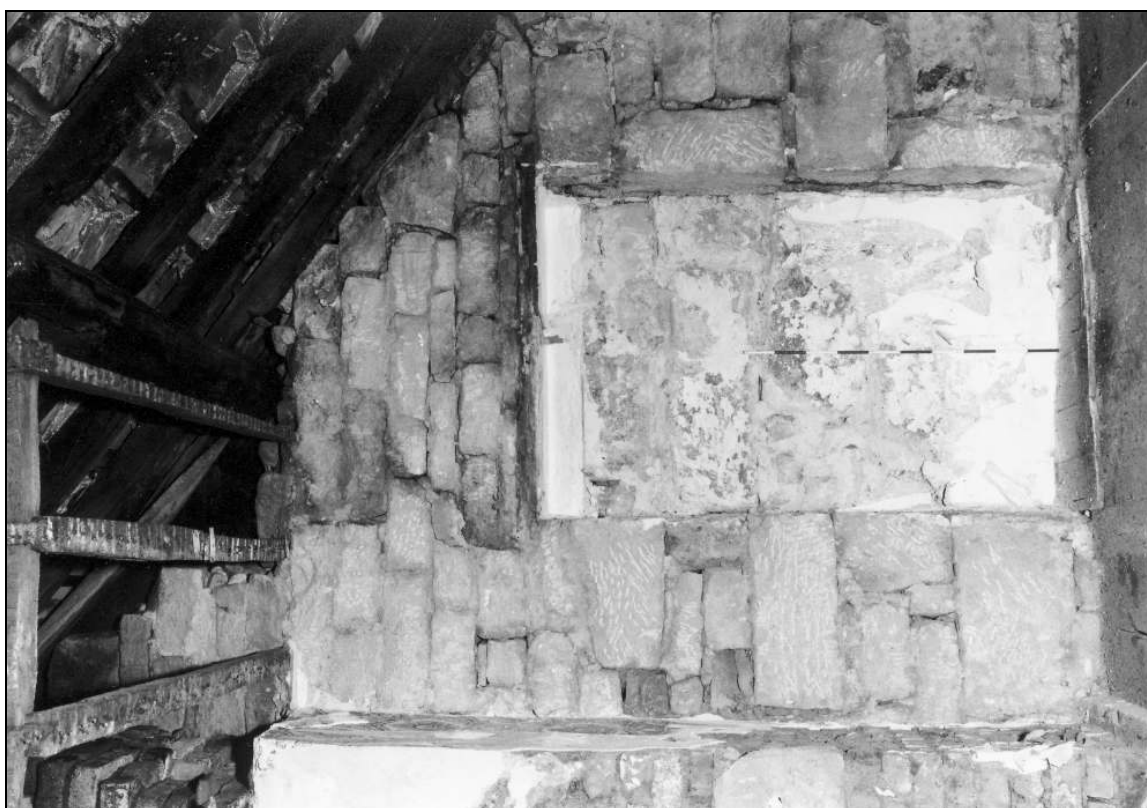
Photo 72: Chamber over housebody: stub of sawn-off tie beam, and scarf joint in wall plate, south wall (film 6, frame 4)
