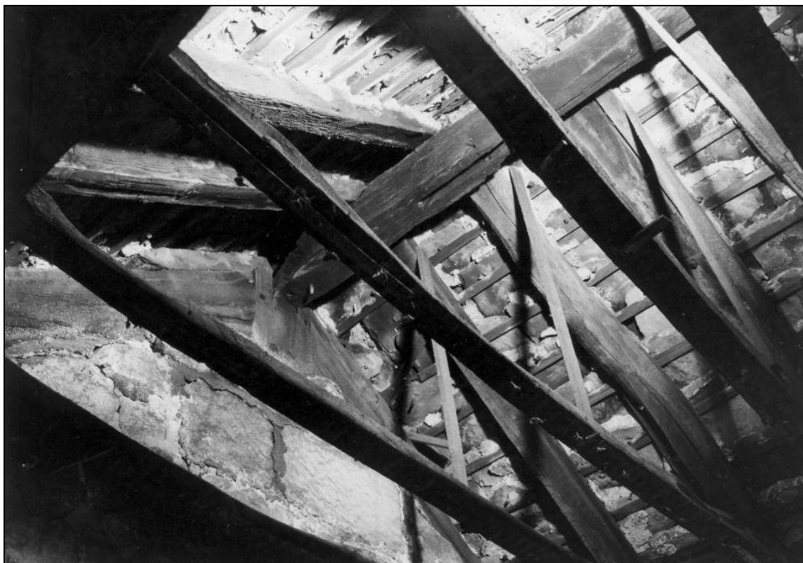
Photo 67: Remains of truss and ridge over hearth passage, from the north-west (film 5, frame 5)
