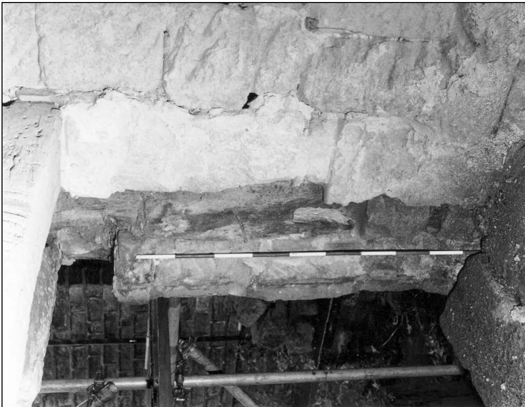
Photo 87: Remains of post at south-east corner of house (ground floor), revealed during repairs (film 7, frame 1)
