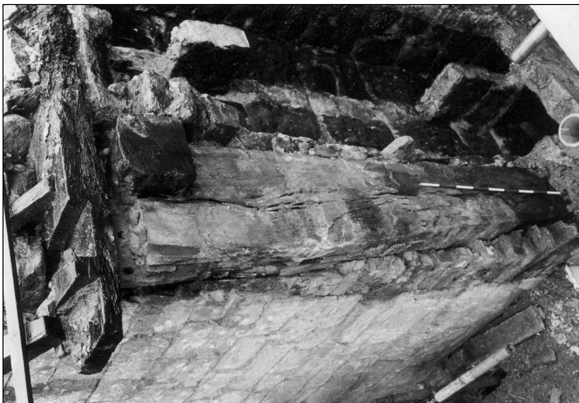
Photo 88: Remains of post at north-east corner of house (first floor), revealed during repairs (film 7, frame 7)
