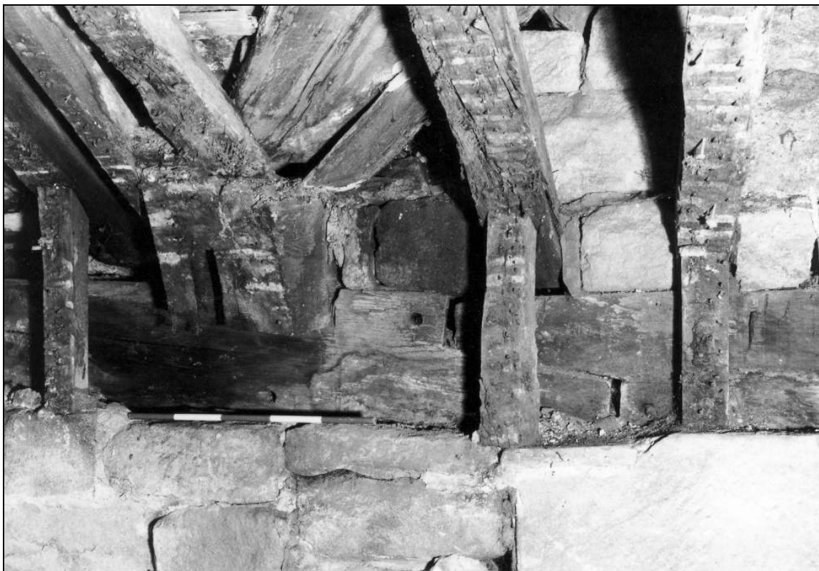
Photo 72: Chamber over housebody: stub of sawn-off tie beam, and scarf joint in wall plate, south wall (film 6, frame 4)
