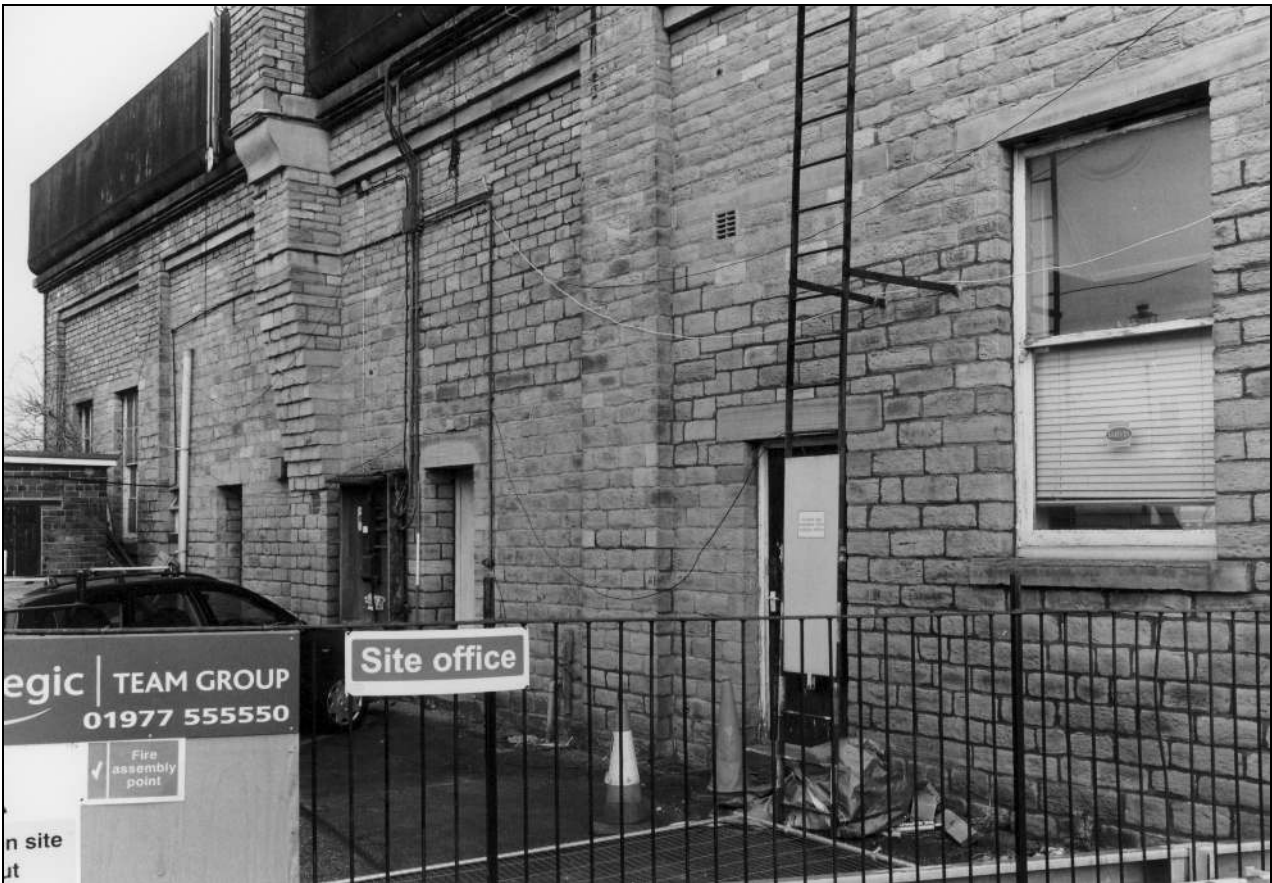
Photo 11: The west elevation; the right hand doorway is inserted (film 1, frame 9)
