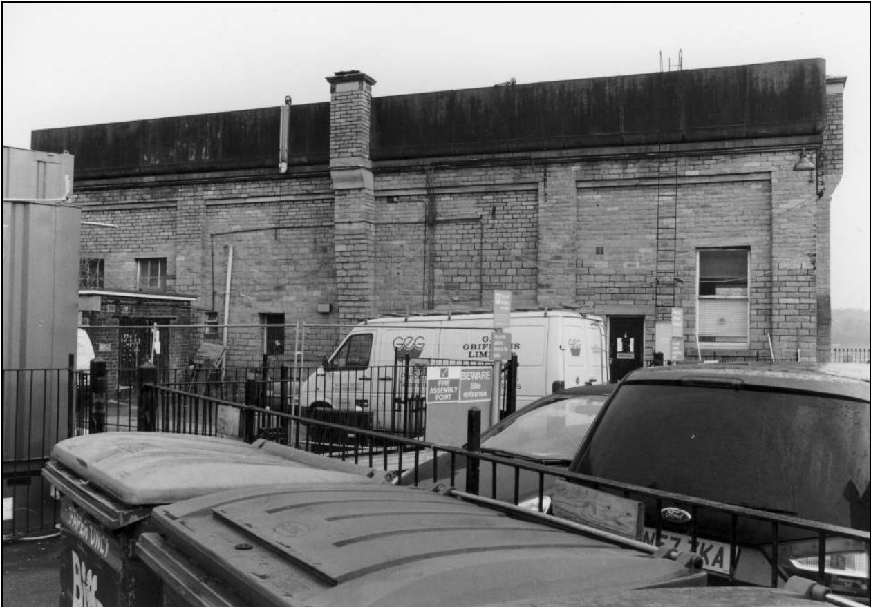
Photo 9: The west elevation (film 1, frame 7)
