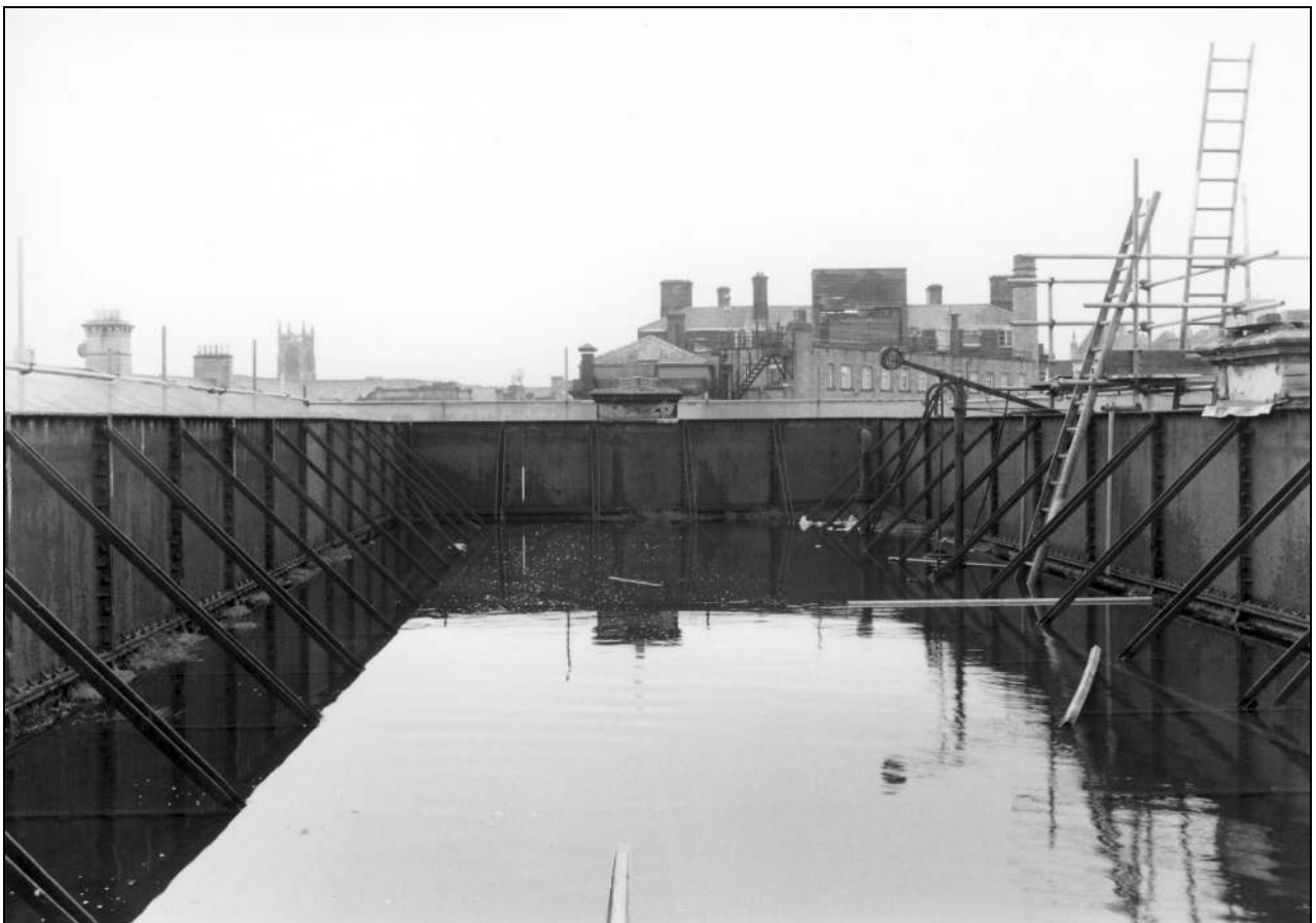
Photo 60: General view of the tank, from the north (film 6, frame 10)
