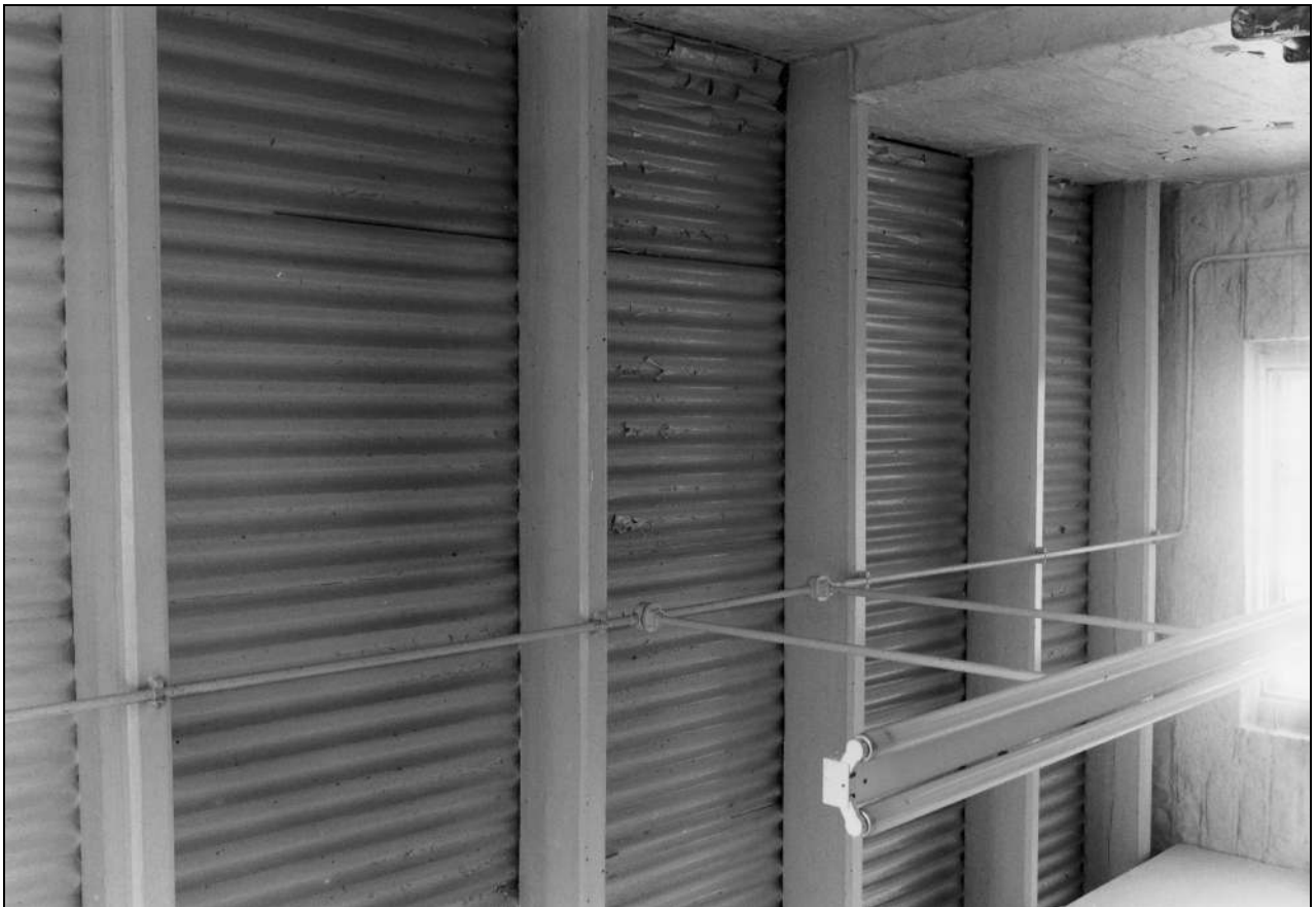
Photo 37: Bay 4: inserted corrugated iron ceiling, from the west (film 3, frame 4)
