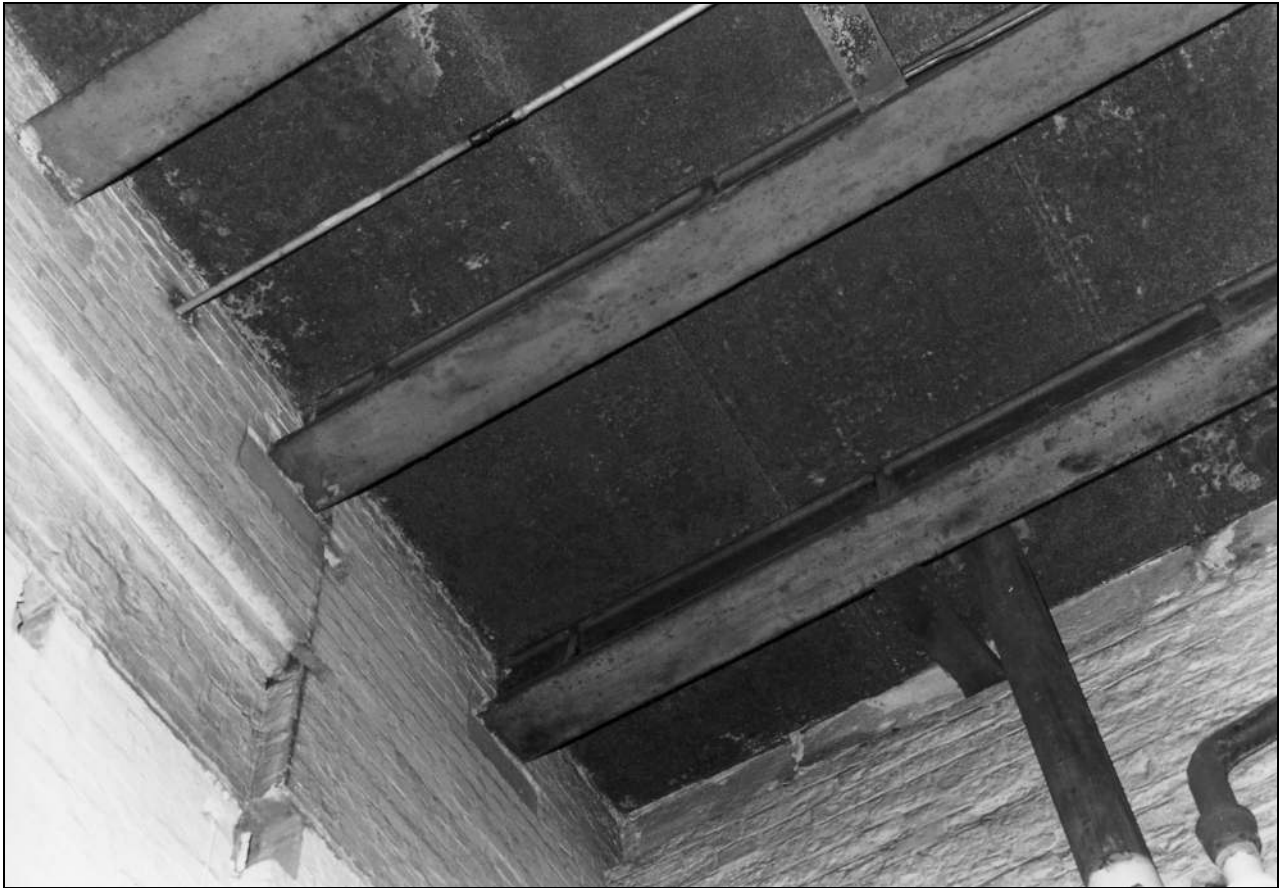
Photo 45: Bay 4: base of tank, south-west corner (film 5, frame 5)
