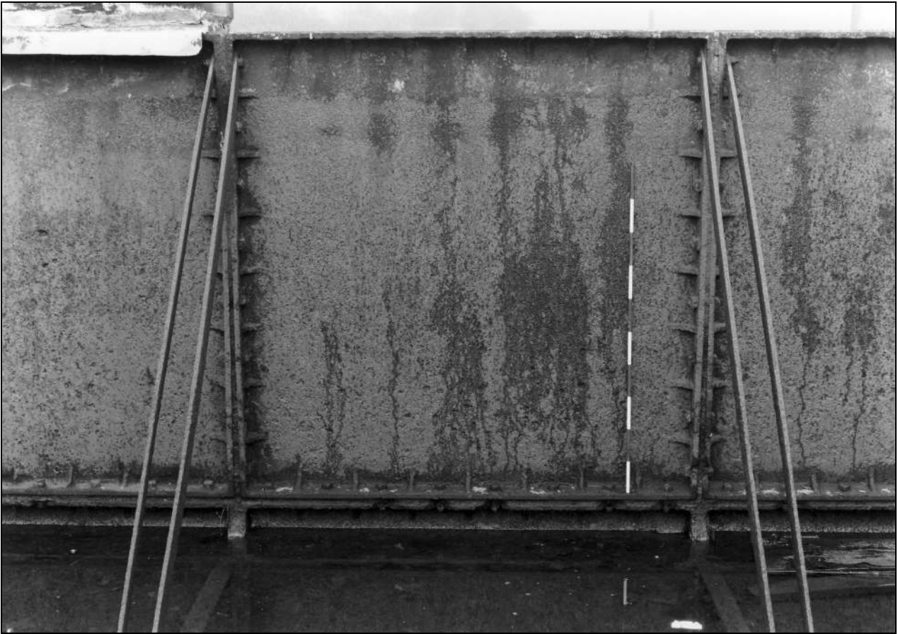
Photo 53: Square cast iron panel forming side of water tank (film 6, frame 13)
