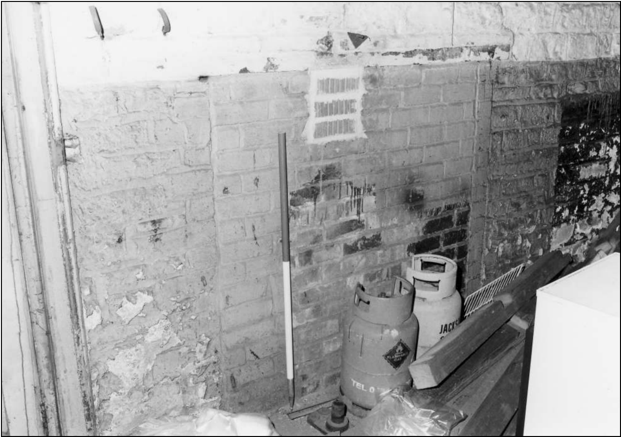
Photo 35: Bay 4: blocked fireplace, north wall (film 3, frame 7)
