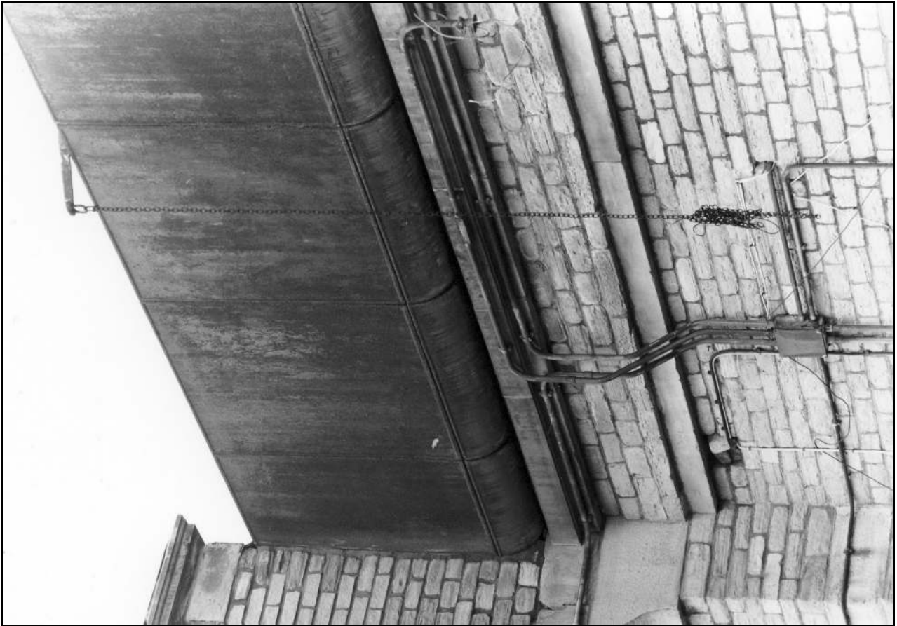
Photo 79: Control lever and chain on outside of tank (film 1, frame 18)
