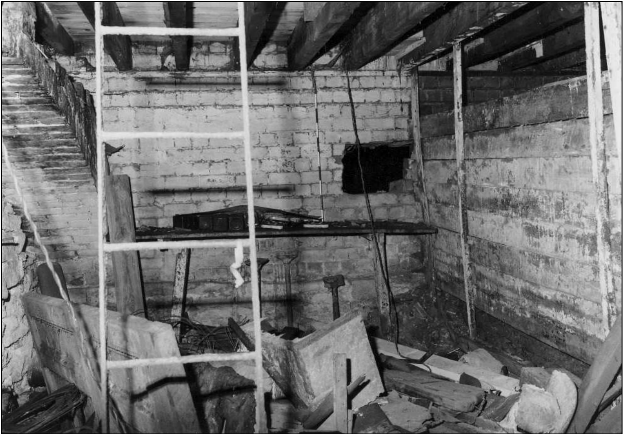
Photo 29: Bay 3: basement, from the north (film 1, frame 4)
