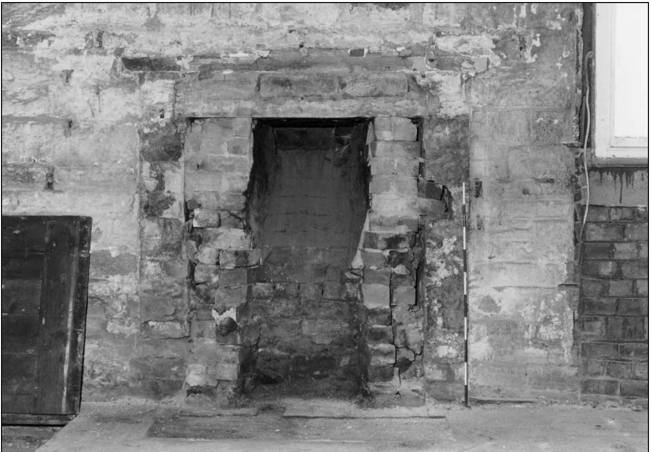
Photo 16: Bay 1: fireplace in south wall (during refurbishment) (film 4, frame 12)
