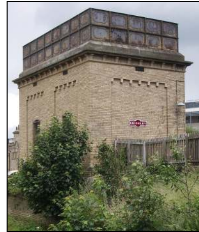
Water tower of c.1883 at Keighley railway station (listed, grade II)
