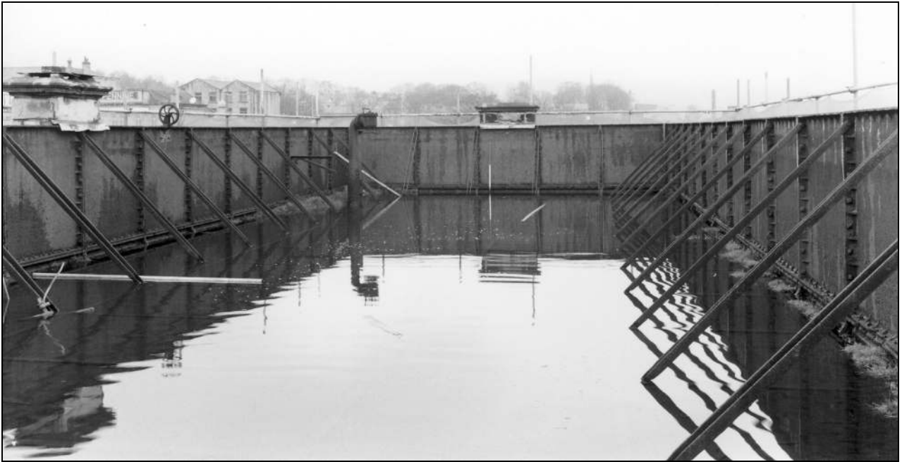
Photo 59: General view of the tank, from the south (film 6, frame 7)
