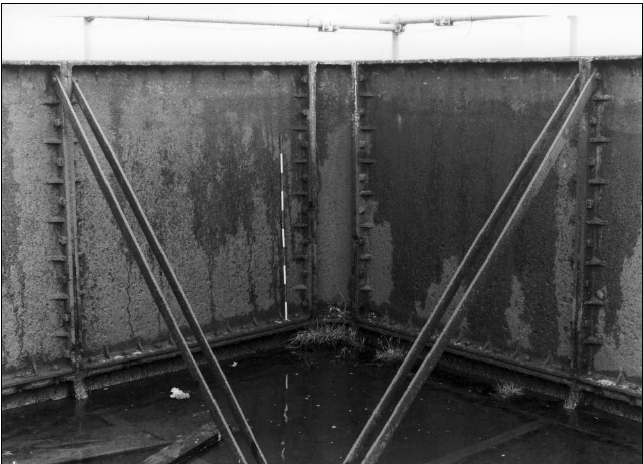
Photo 54: Cast iron panels at south-east corner of water tank (film 6, frame 14)
