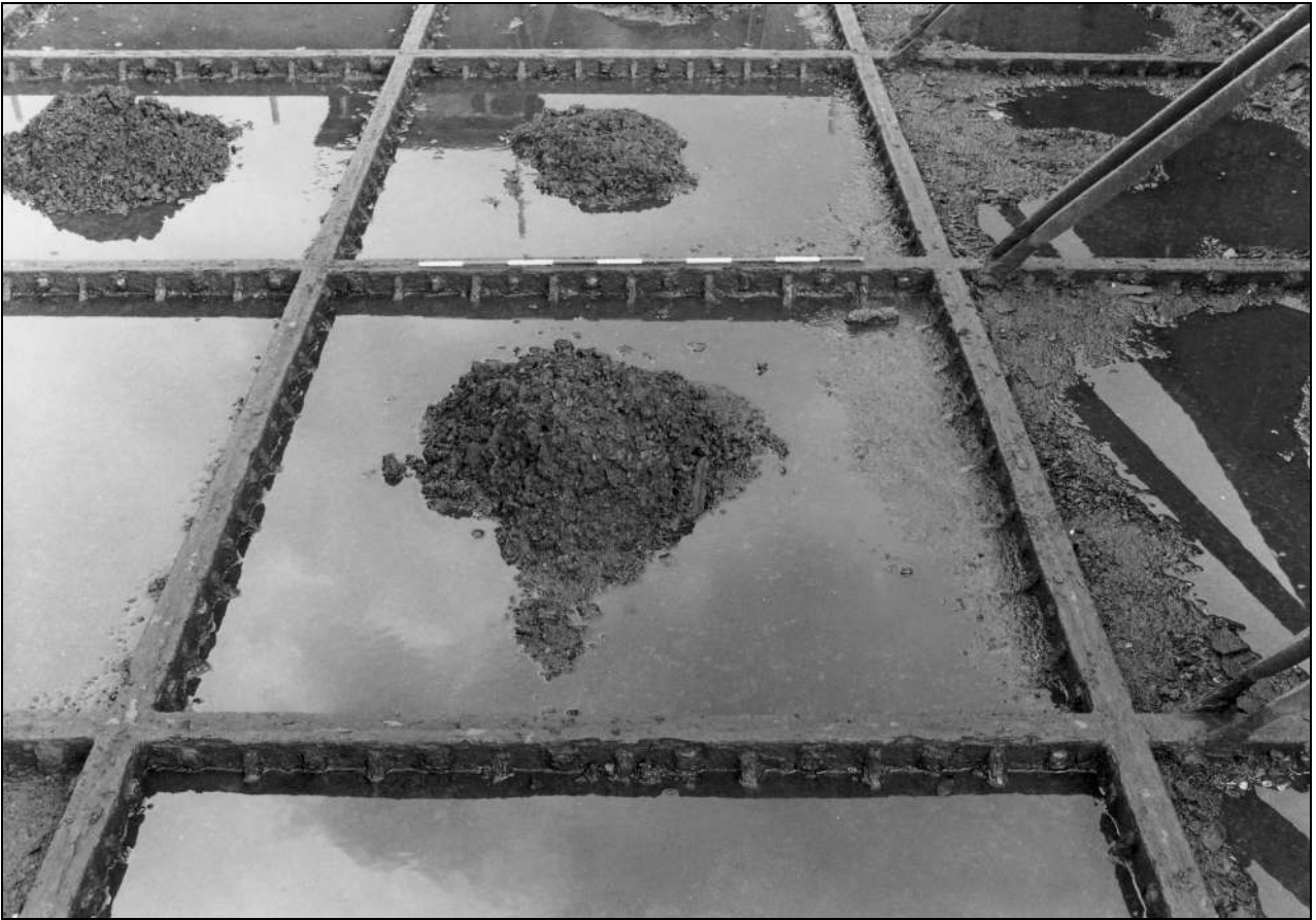
Photo 55: Cast iron panels forming base of water tank (film 8, frame 10)
