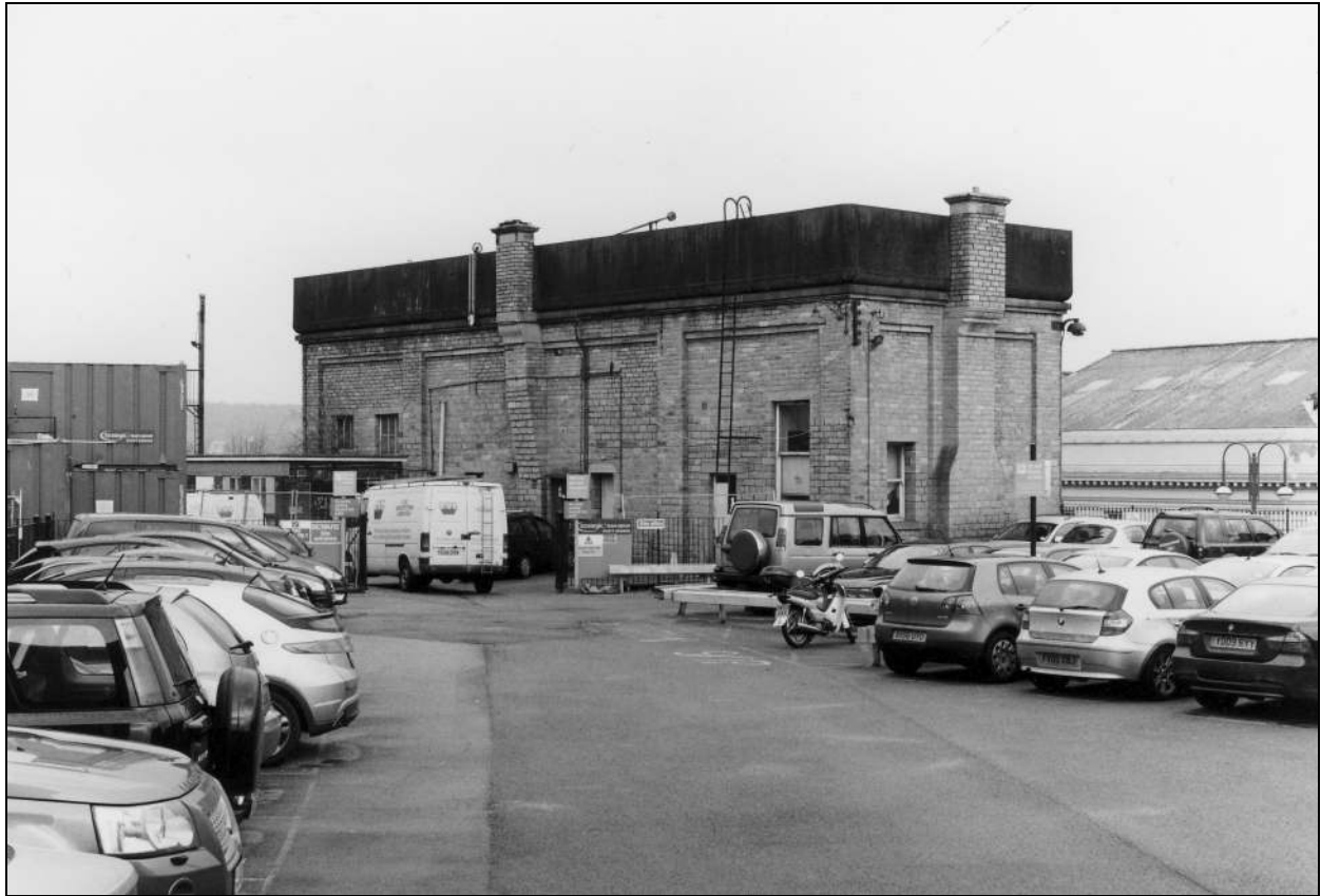
Photo 3: The water tower, viewed from the south-west (film 2, frame 3)
