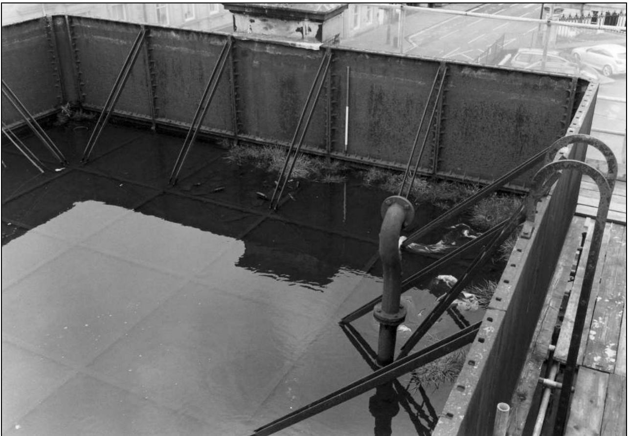
Photo 80: South end of tank, showing original feed pipe (film 7, frame 14)
