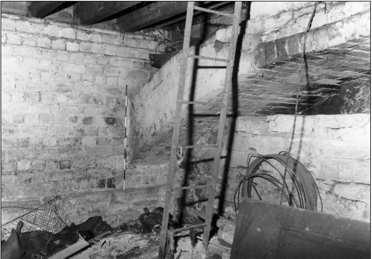
Photo 30: Bay 3: basement, from the south-west (film 1, frame 2)
