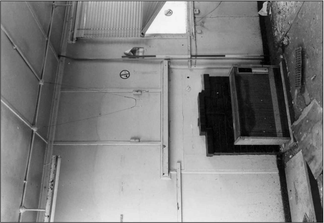
Photo 15: Bay 1: fireplace in south wall (before refurbishment) (film 2, frame 11)
