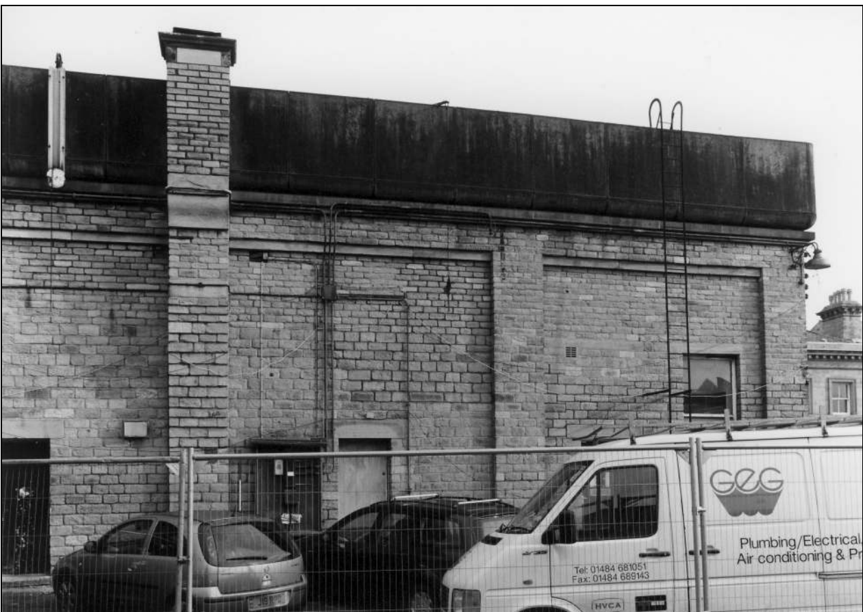
Photo 10: The west elevation (south part) (film 1, frame 10)
