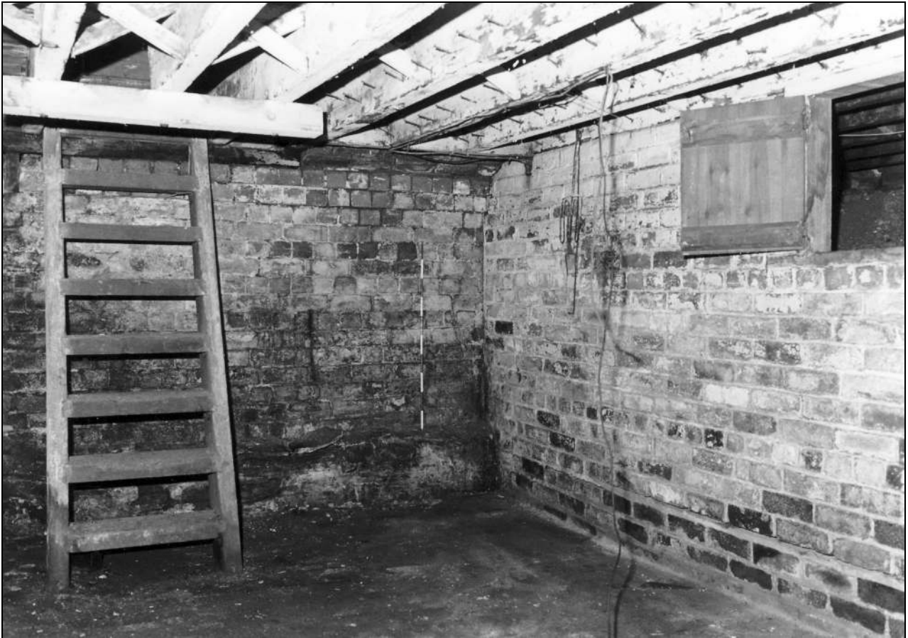
Photo 21: Bay 1: basement, from the north-east (film 4, frame 10)
