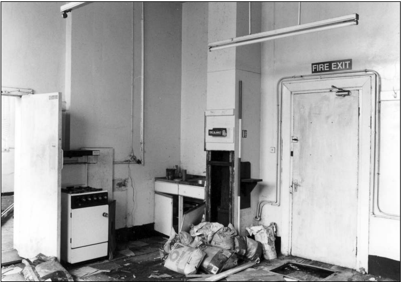
Photo 23: Bay 2: south-west corner, before refurbishment (film 2, frame 15)
