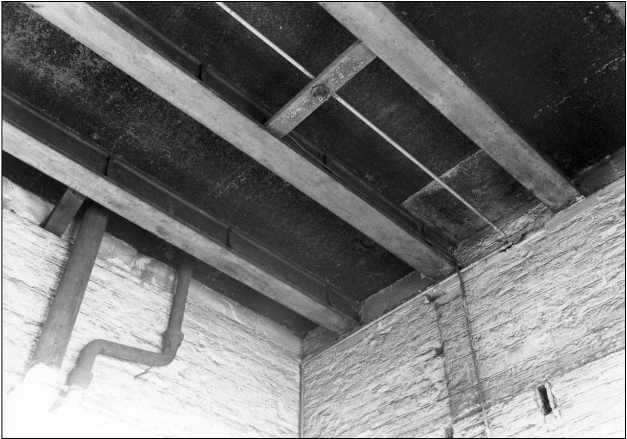
Photo 49: Bay 4: base of tank, north-west corner (film 4, frame 1)
