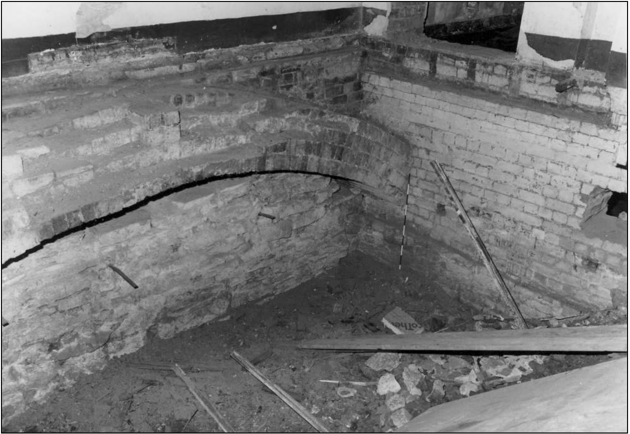
Photo 31: Bay 3: basement, from the north-west (film 5, frame 6)
