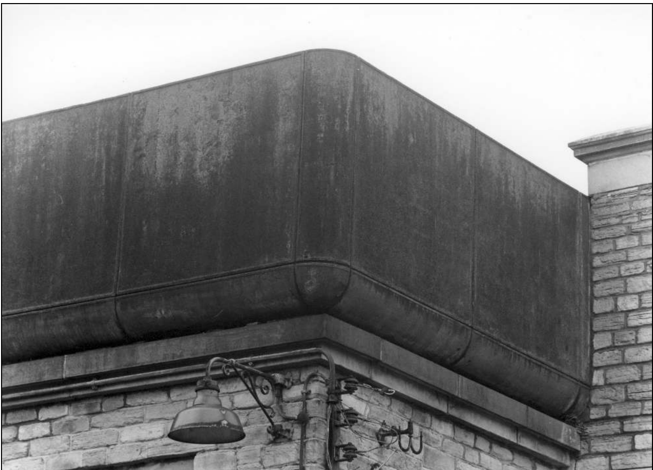
Photo 52: South-west corner of water tank (film 2, frame 1)
