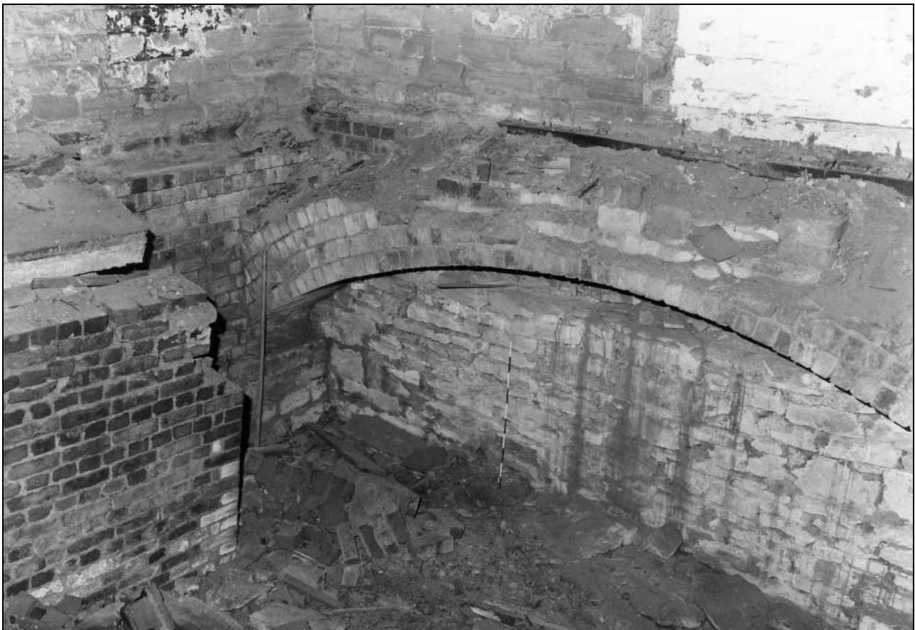
Photo 36: Bay 4: basement, from the south-west (film 5, frame 1)
