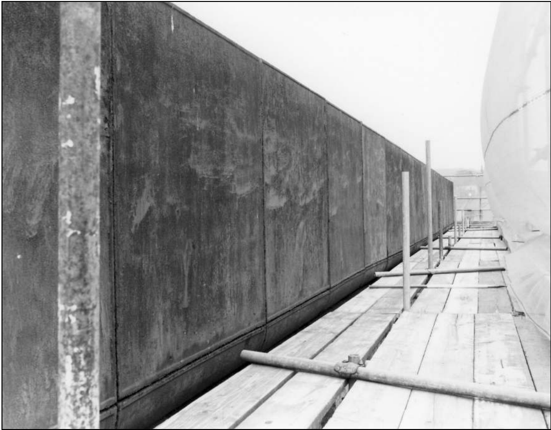
Photo 57: Cast iron panels forming east side of water tank (film 7, frame 18)
