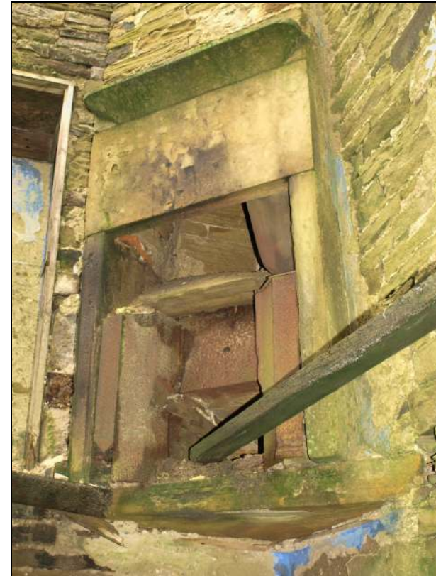
Photo 36: First floor in cottage, showing fireplace in front room
