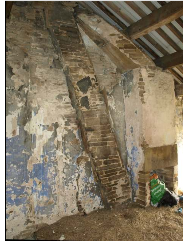
Photo 23: Hayloft over housebody, with inserted fireplace and flues
