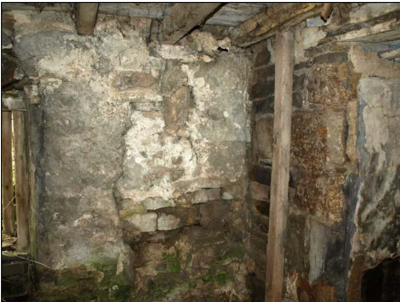
Photo 25: Blocked window in rear of housebody, sighted by cross wall
