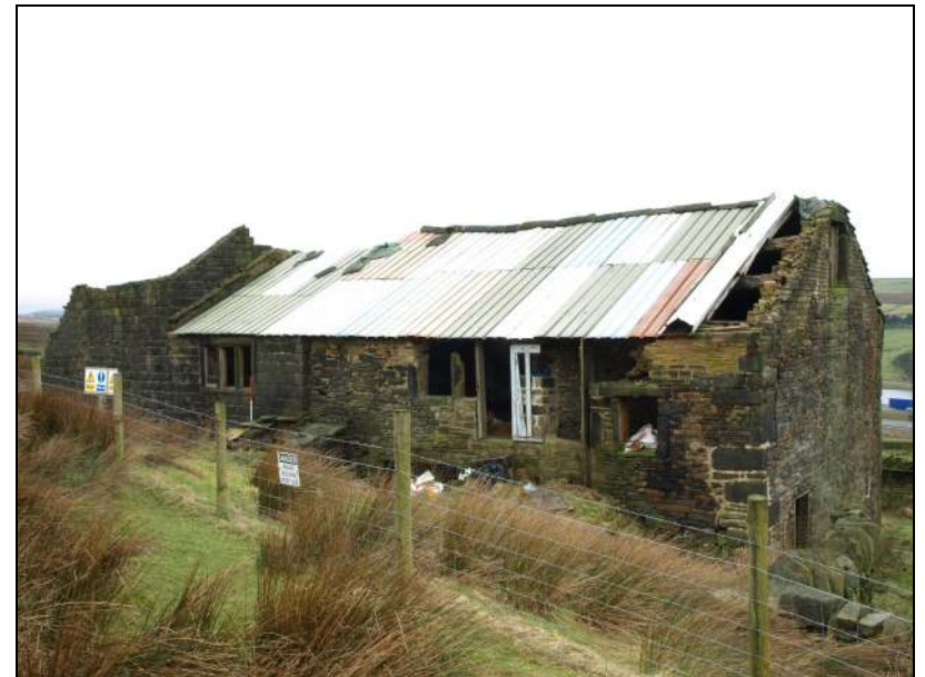
Photo 12: View of the main building range, from the east
