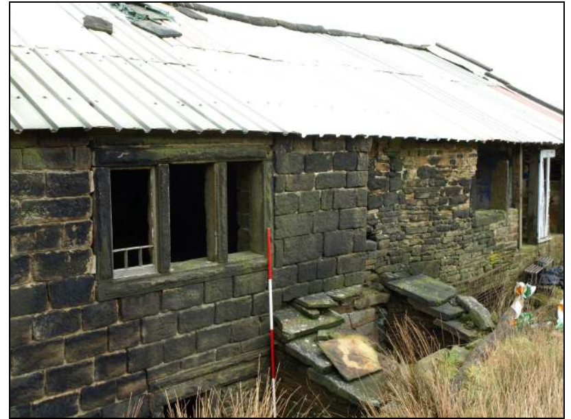
Photo 32: Detail of rear elevation of cottage
