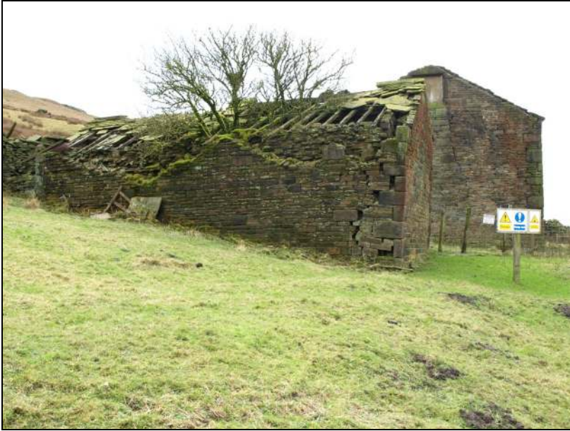
Photo 49: Detached outbuildings, from the north-east
