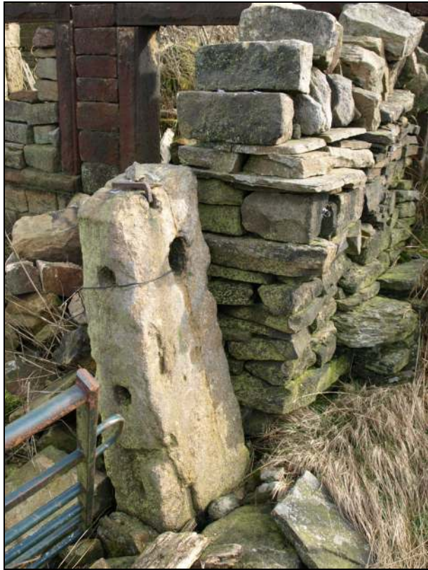
Photo 46: Early gate stoop near west corner of barn
