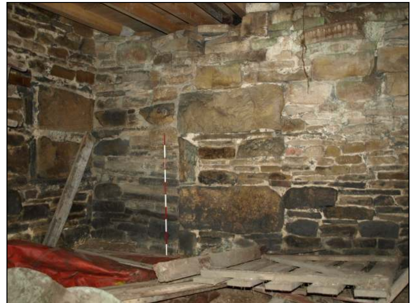
Photo 16: Ground floor store in north-east end of farmhouse
