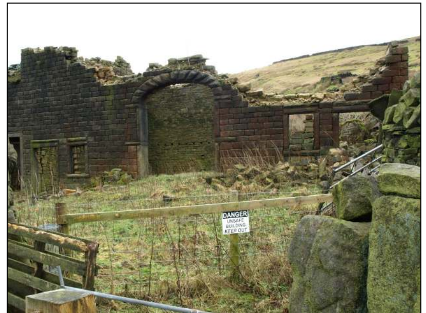
Photo 39: Barn: front elevation
