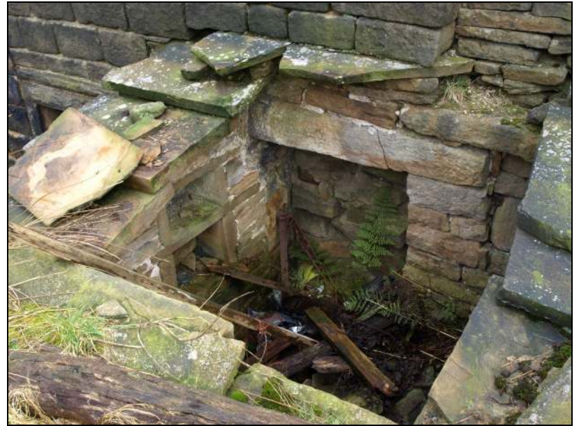
Photo 26: Lean-to pantry to rear of farmhouse, from the north
