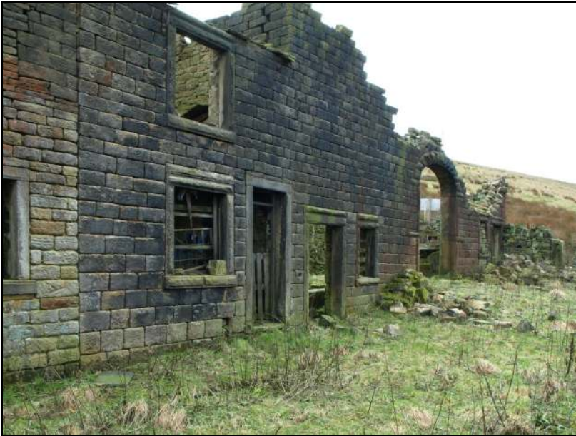
Photo 30: Front elevation of cottage and barn
