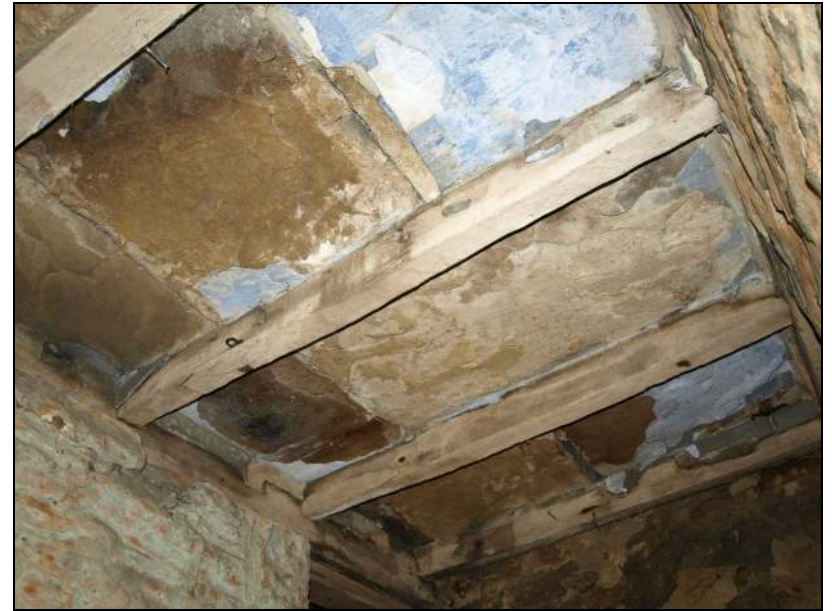
Photo 15: Underside of flagstone first floor, north-east end of farmhouse
