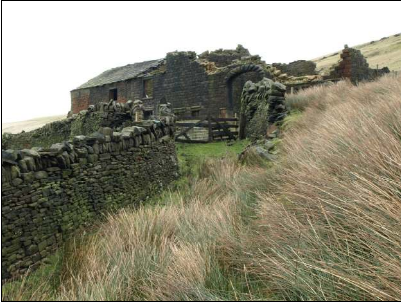
Photo 5: Barn and farmhouse etc, from the west, up the trackway
