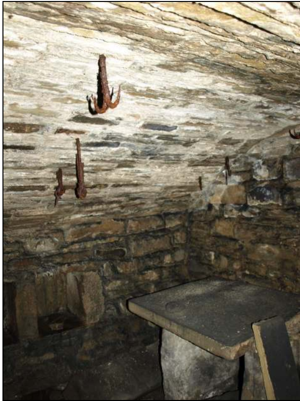
Photo 37: Cellar, below cottage, from the south
