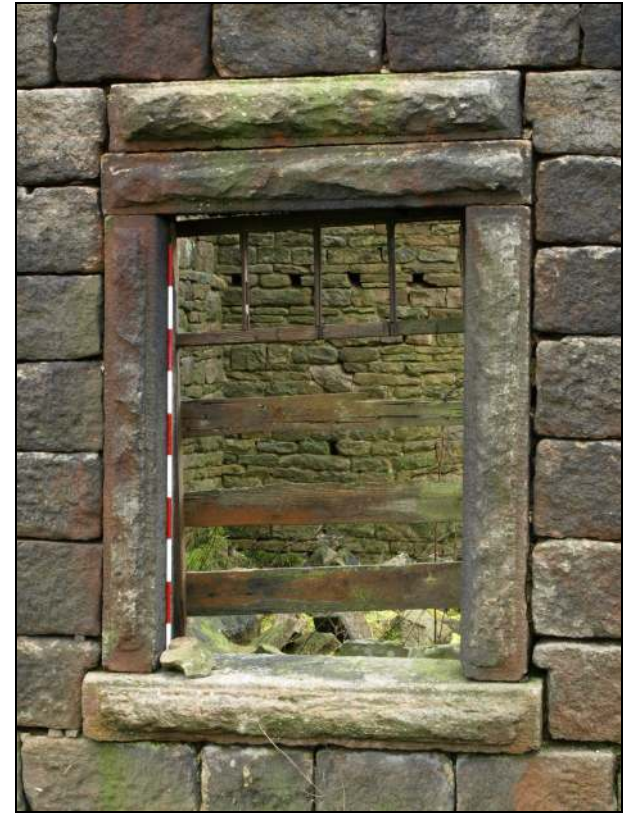
Photo 41: Detail of window in front of barn
