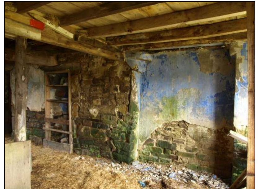
Photo 20: Housebody in farmhouse, from the north
