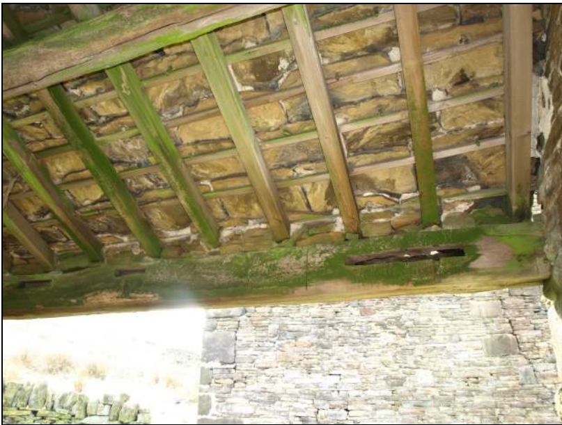
Photo 50: Re-used oak lintel to open shed
