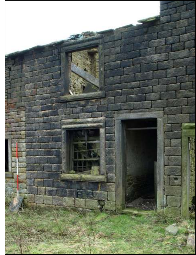
Photo 29: Front elevation of cottage
