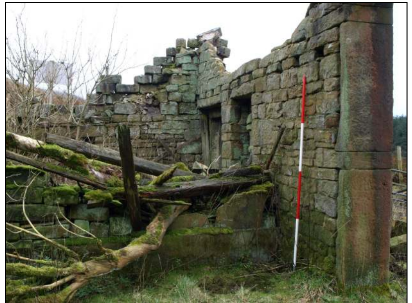
Photo 45: Remains of south-east end of barn, from the north-west
