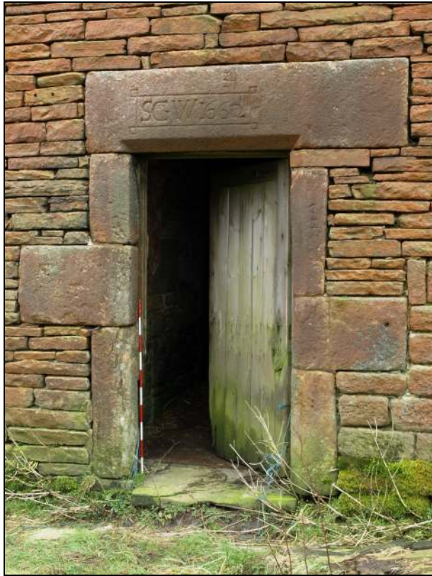
Photo 8: Doorway to hearth passage of farmhouse
