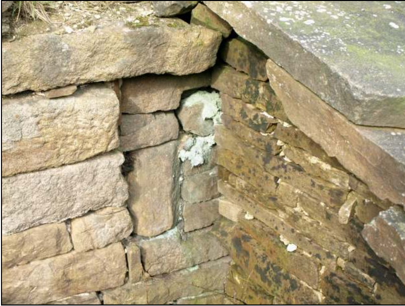
Photo 28: Blocked window in rear of farmhouse, slighted by lean-to pantry
