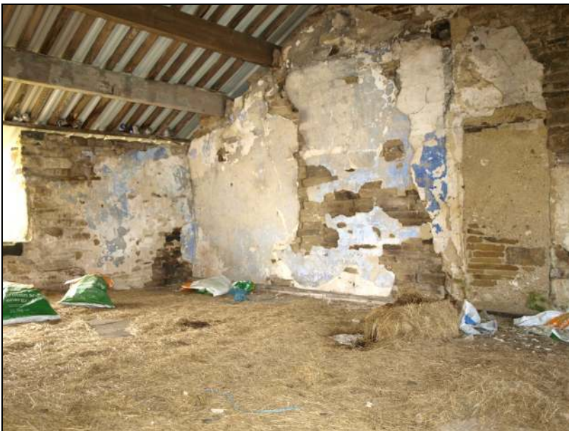
Photo 22: Hayloft over housebody, from the north
