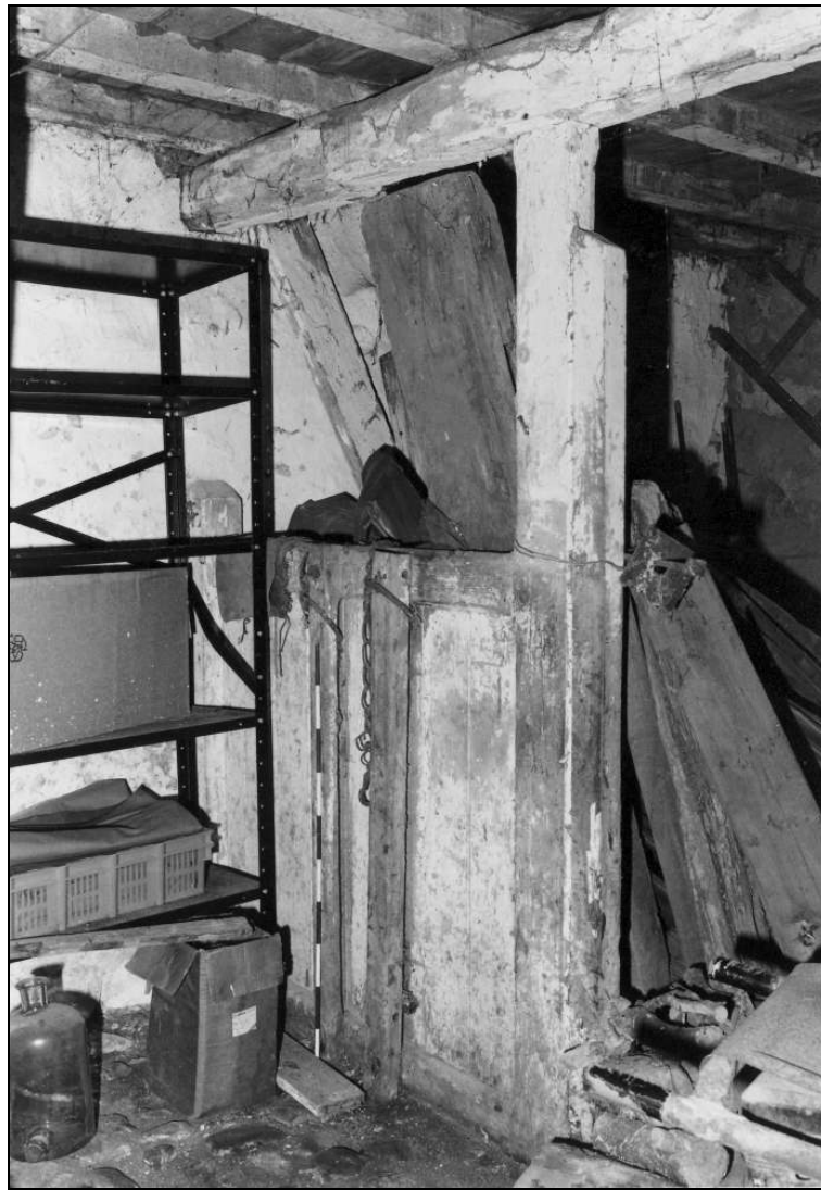
Photo 18: Ground floor: detail of boskin between cow stalls, from the west
