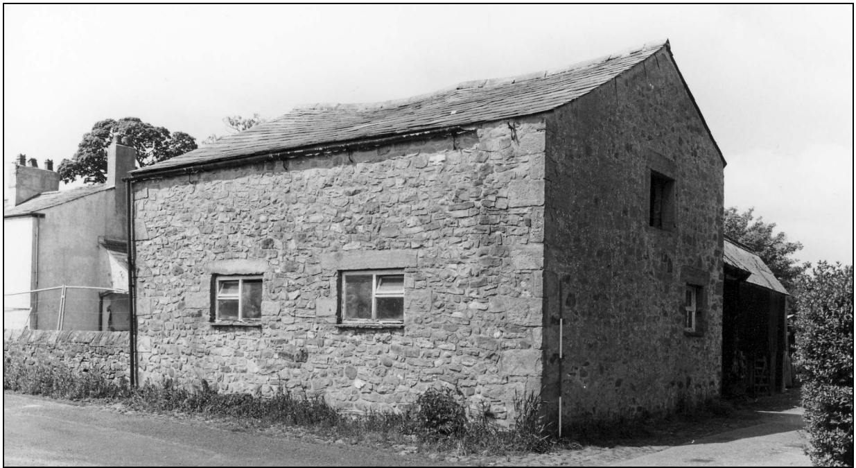
Photo 7: The barn, from the east
