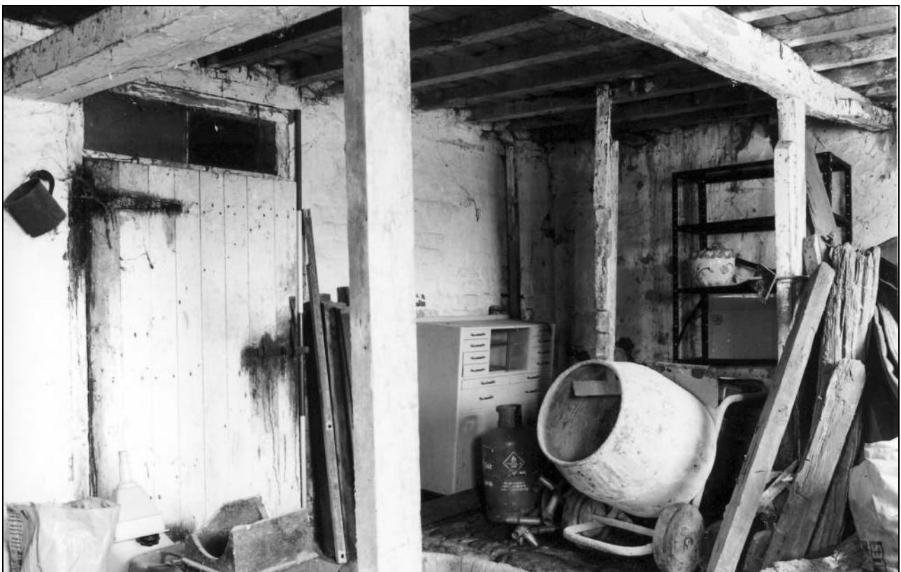
Photo 20: Ground floor: doorway to store with brick walls in north corner
