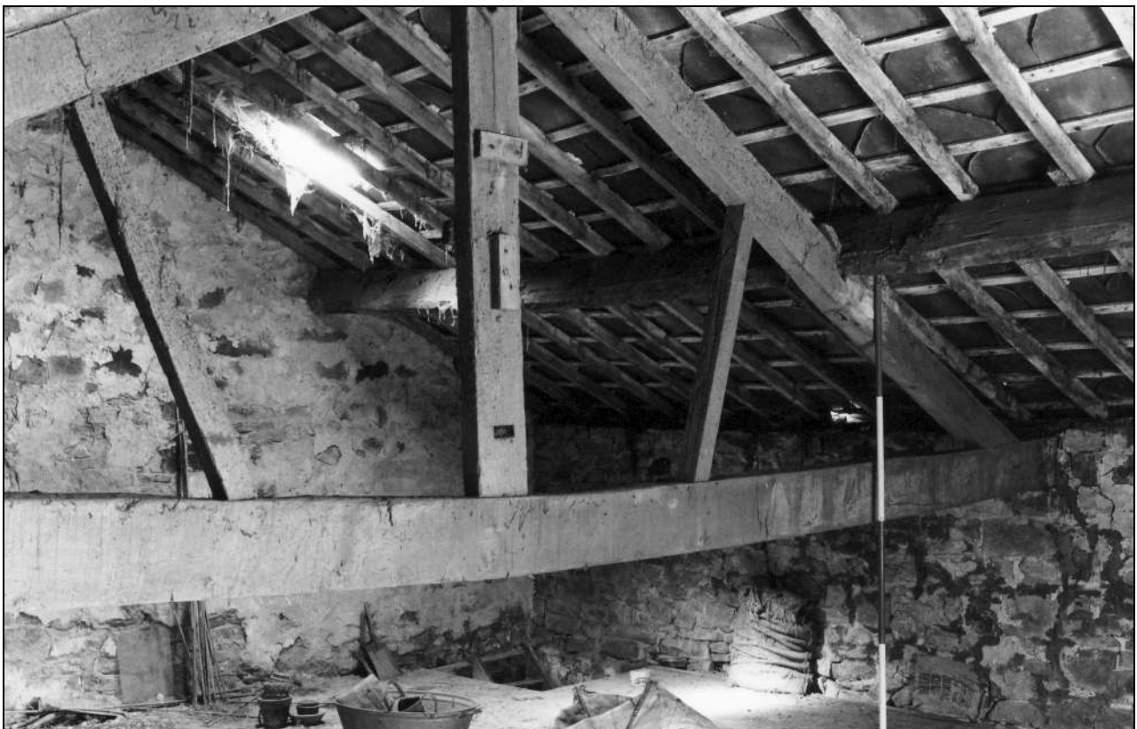
Photo 24: First floor: roof truss, from the east
