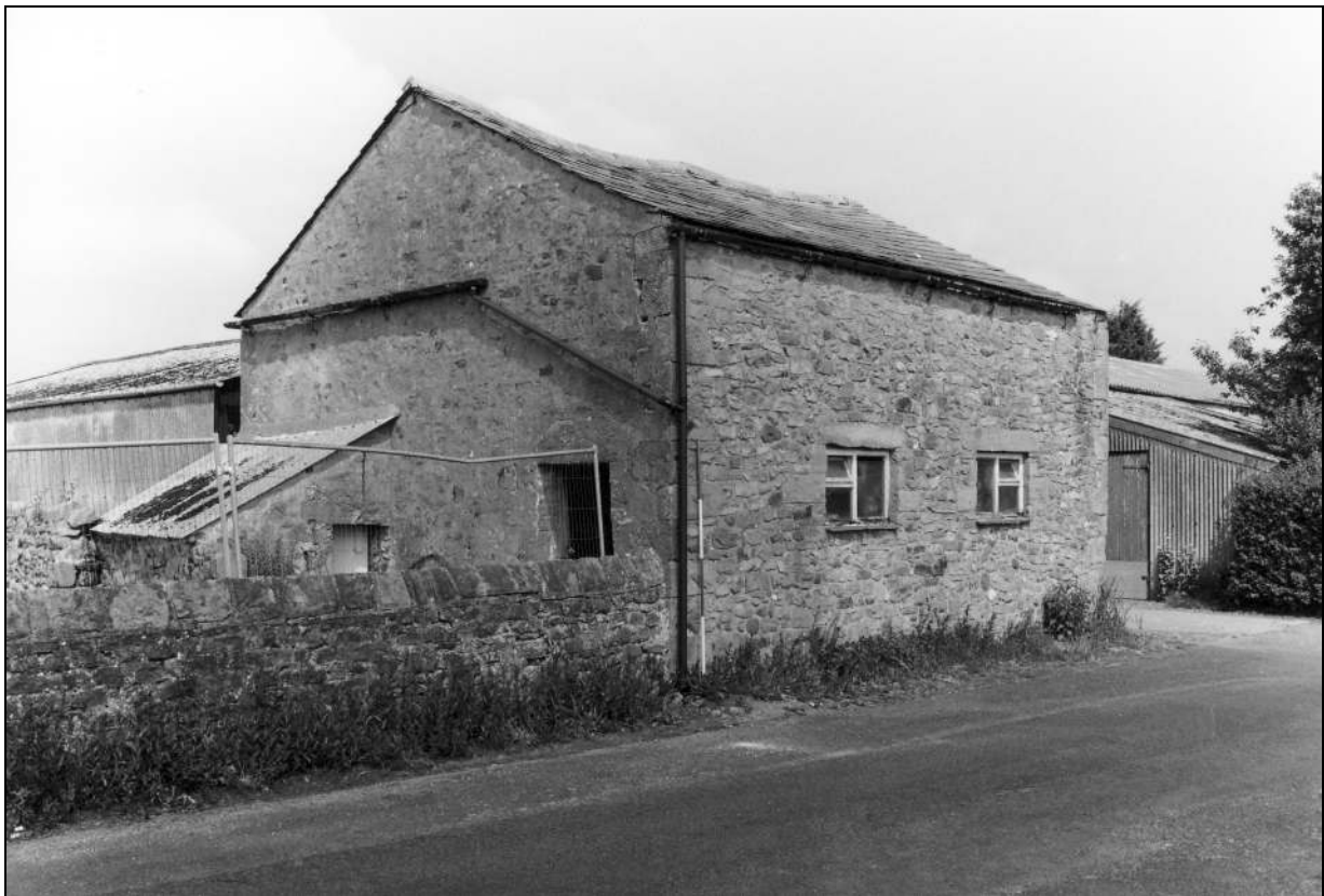
Photo 4: The barn, from the south
