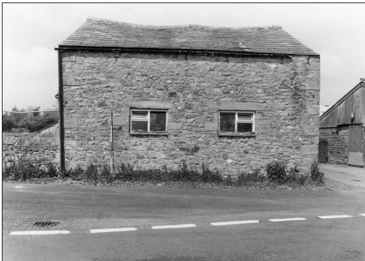
Photo 5: The barn: rebuilt south-east elevation
