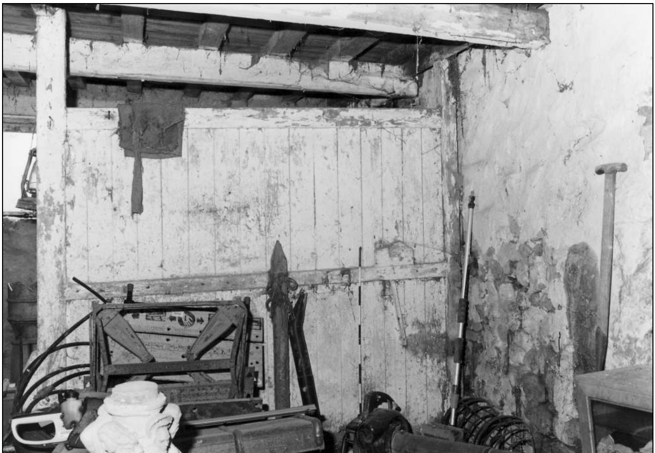
Photo 13: Ground floor: re-sited divider between horse/pony stalls, from the north-west
