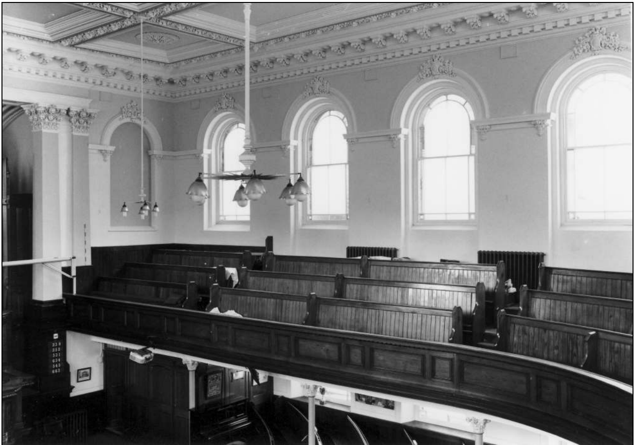
Photo 51: The gallery, from the north-east (film 2, frame 13)
