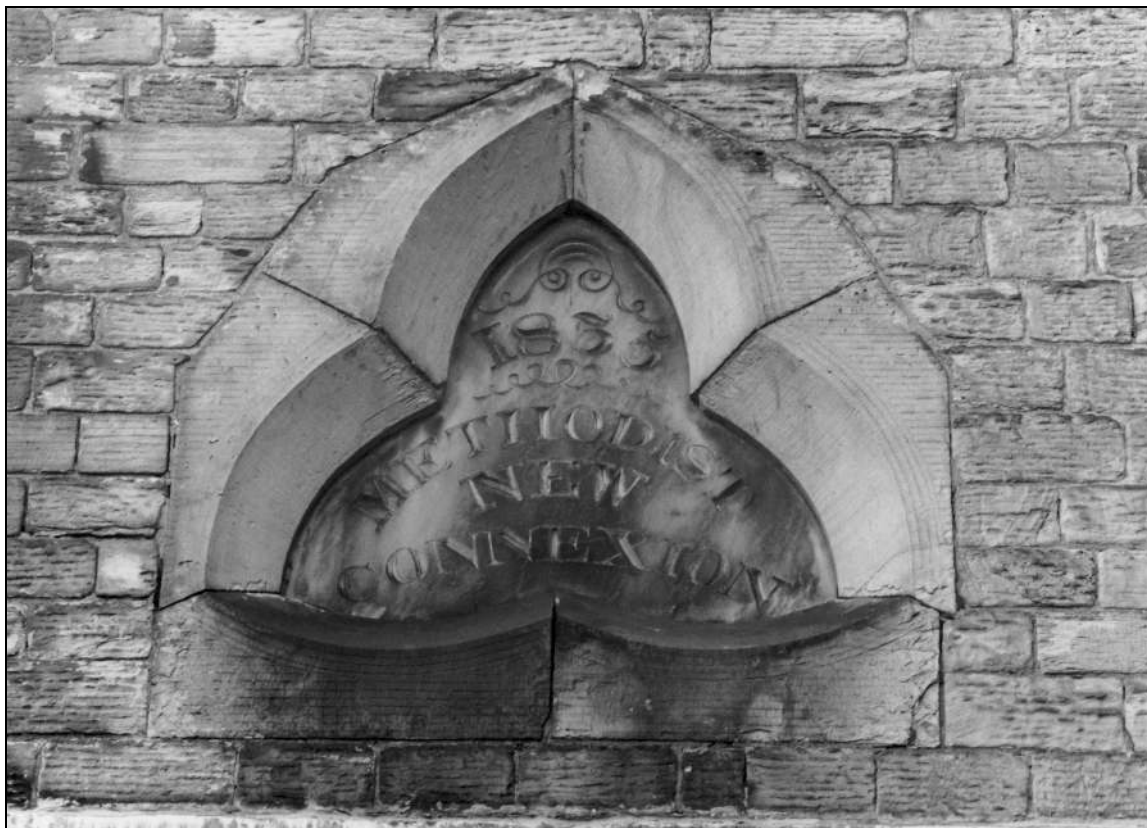
Photo 21: Detail of blind window re-used from the 1835 church, inscribed with date and name (film 10, frame 10)
