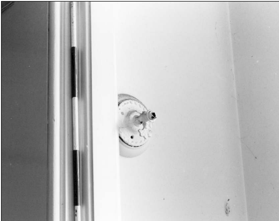
Photo 71: Gas light fixture at top of stairs to basement (film 6, frame 15)
