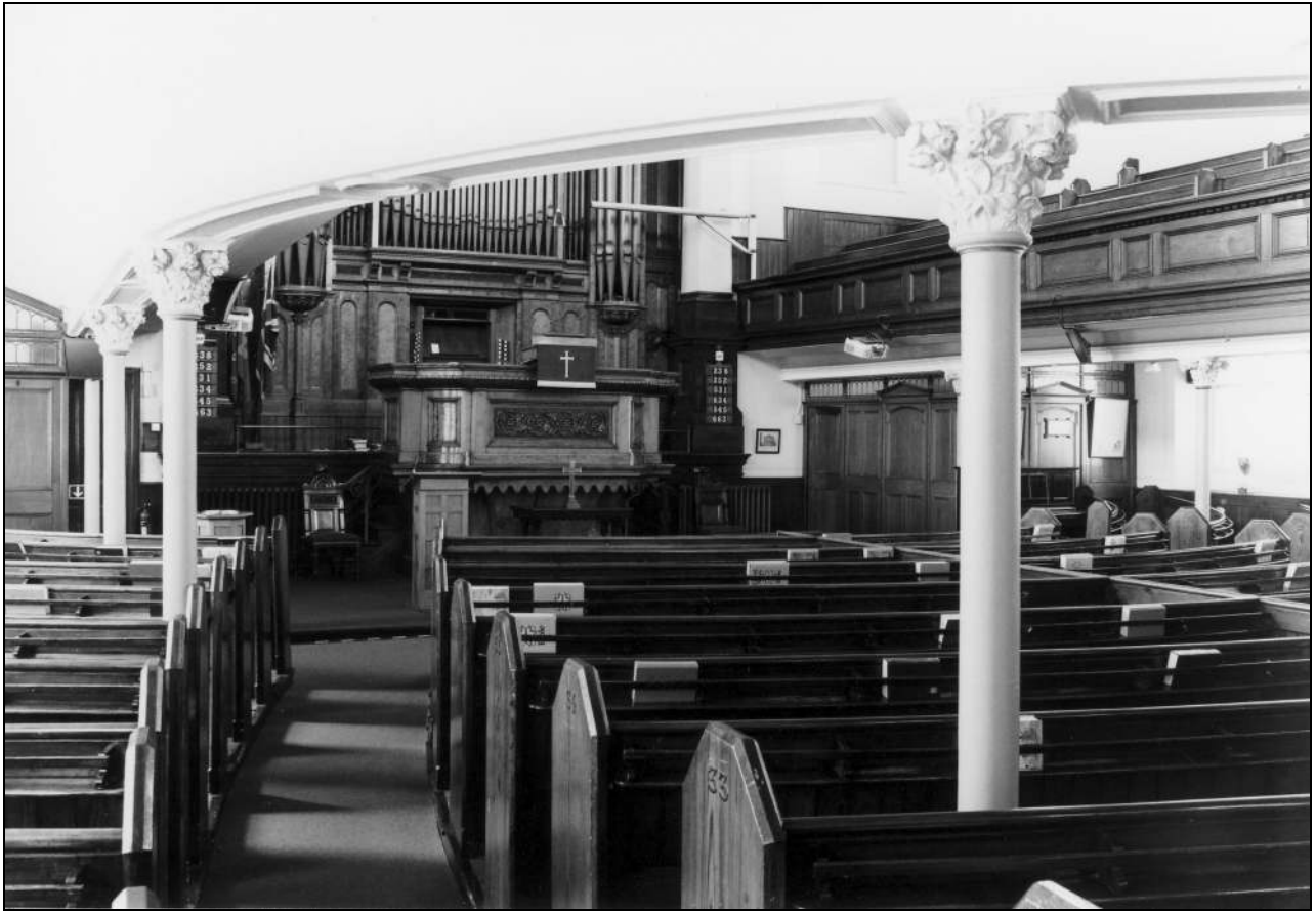
Photo 30: The ground floor of the church, from the north-east (film 2, frame 3)
