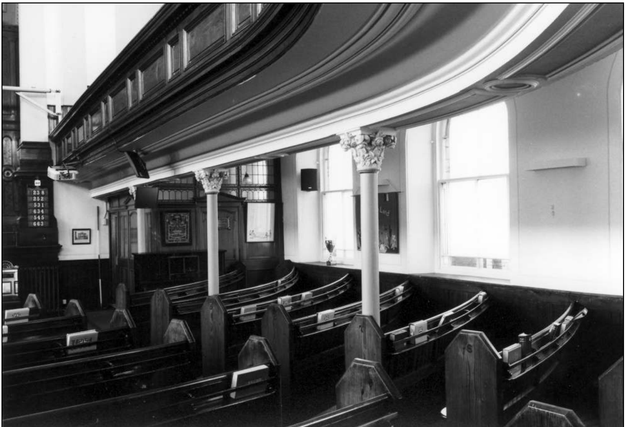
Photo 47: Columns to west side of gallery, from the north (film 2, frame 6)
