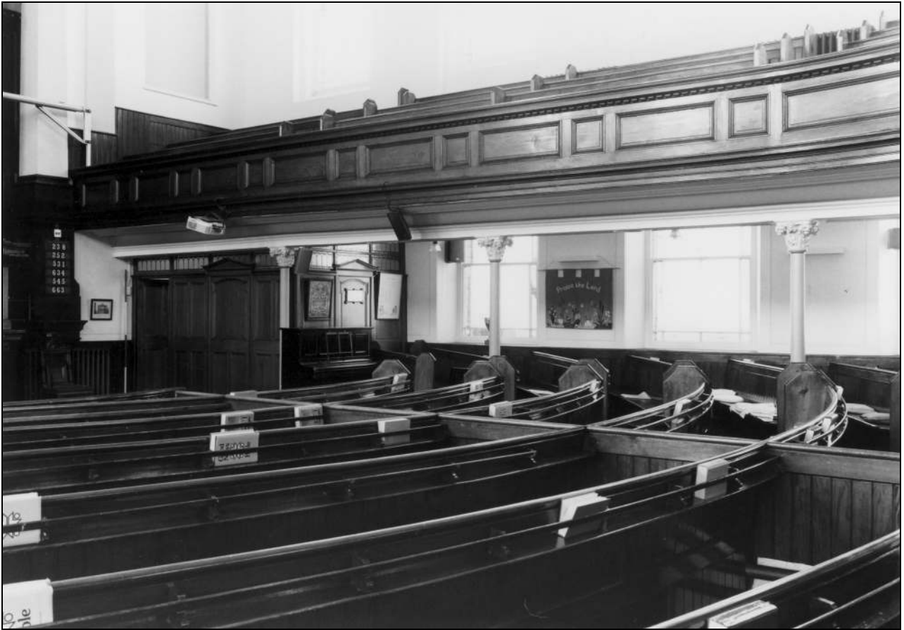
Photo 28: The ground floor of the church, from the north-east (film 2, frame 4)
