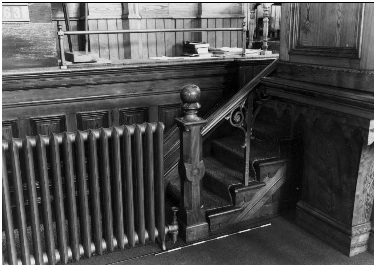
Photo 66: Stairs and balustrade to rostrum (film 5, frame 18)
