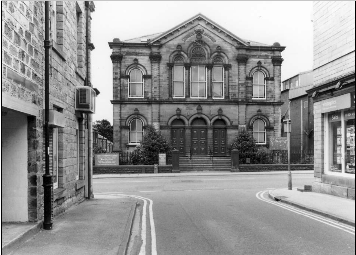
Photo 2: The church, from the north across Huddersfield Road (film 9, frame 7)
