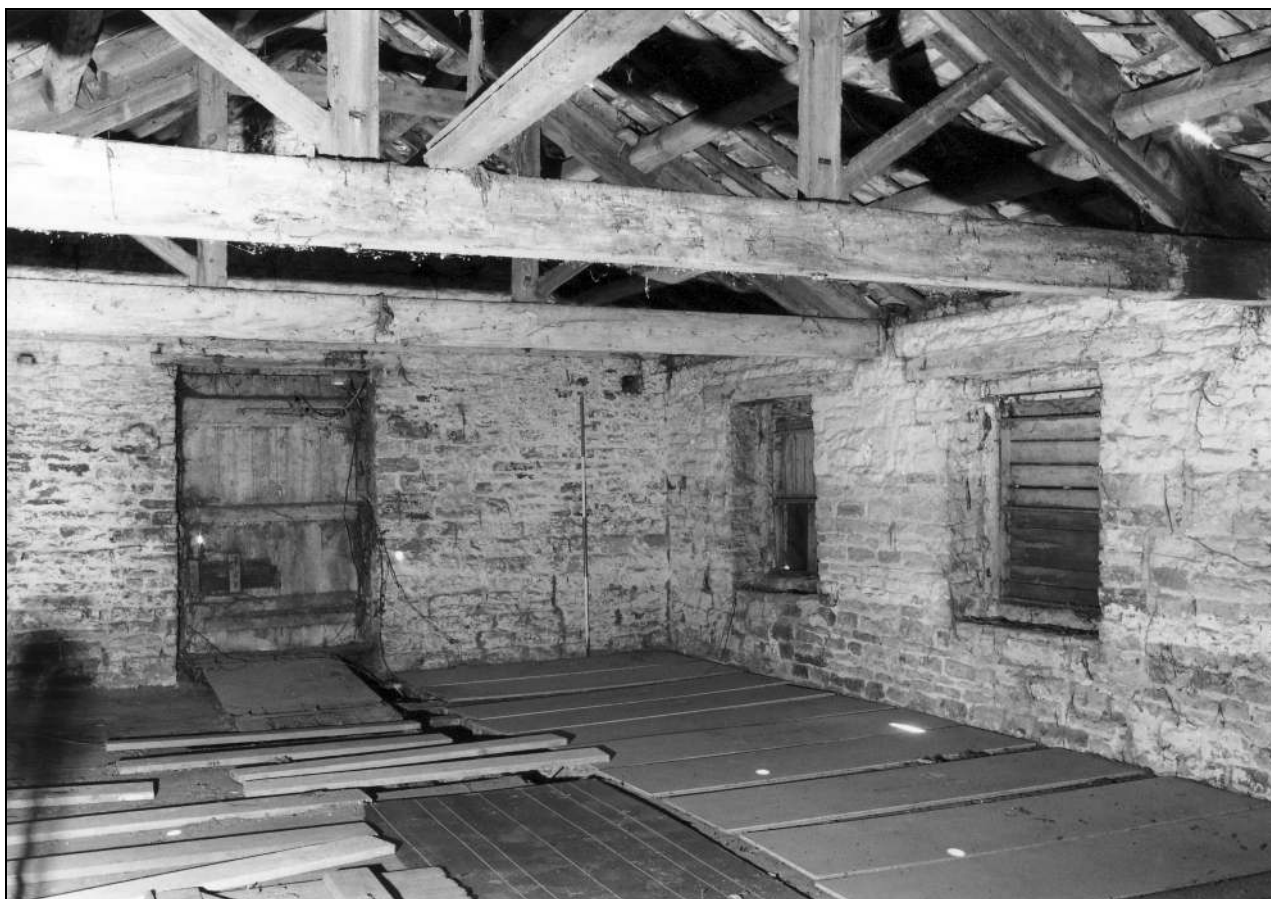
Photo 28: Building 1a: first floor, from the south-west (film 4, frame 10)
