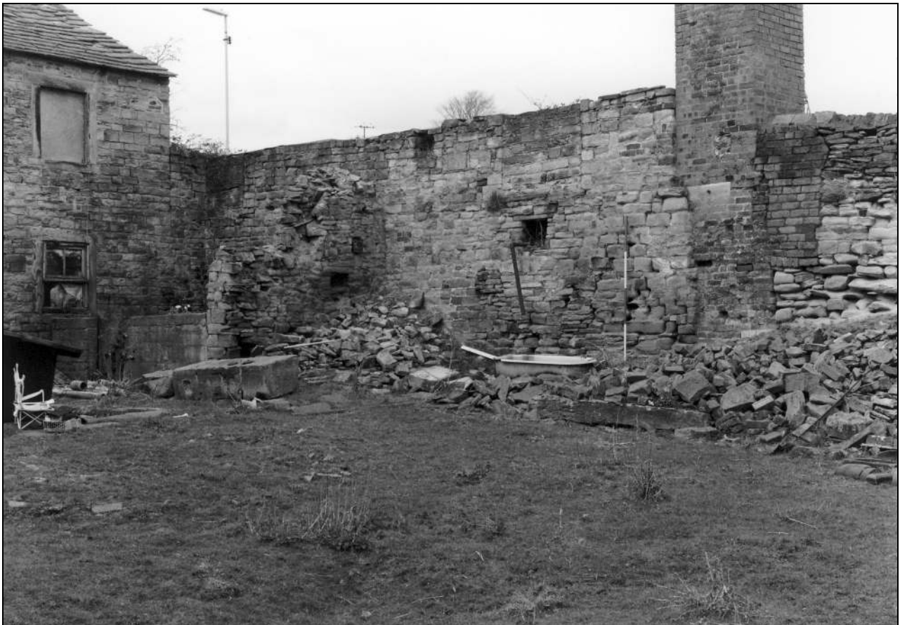
Photo 55: Remains of buildings at foot of chimney, from the south-east (film 2, frame 1)
