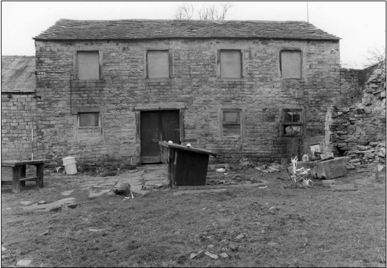
Photo 7: Building 1a: east elevation (film 1, frame 15)
