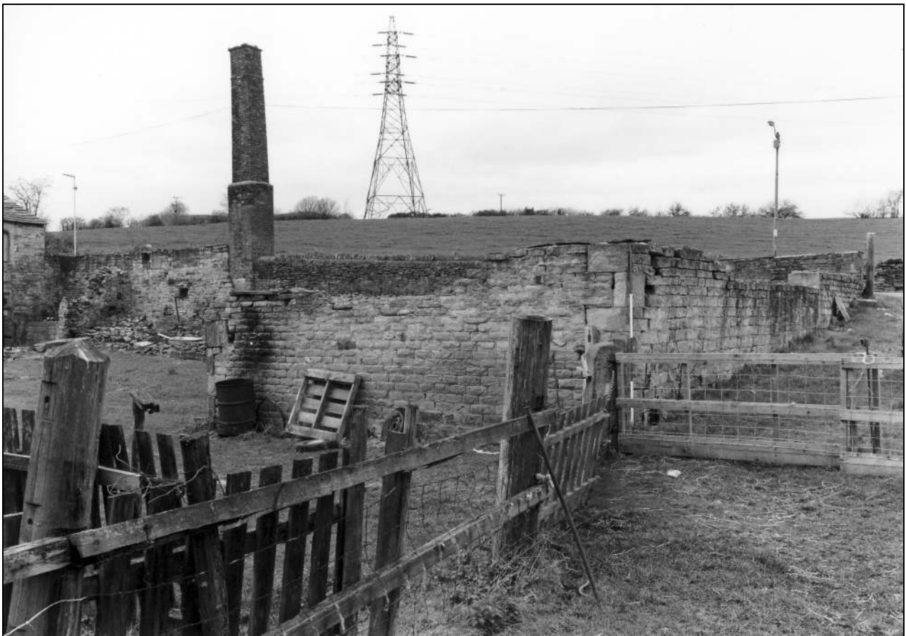
Photo 47: Building 2, from the south-east (film 2, frame 16)
