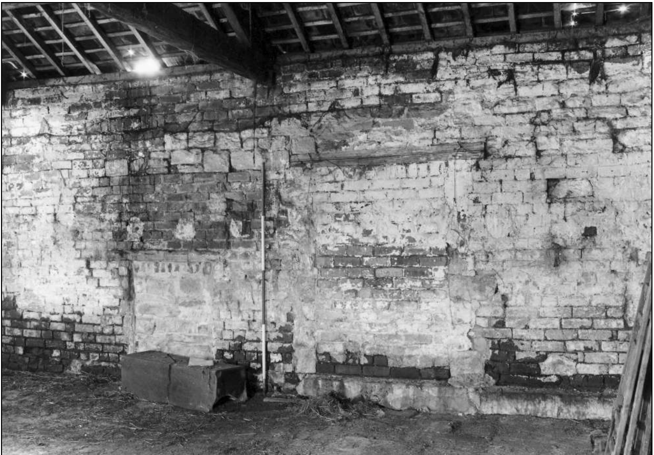
Photo 42: Building 1b: interior, from the north-east (film 4, frame 1)
