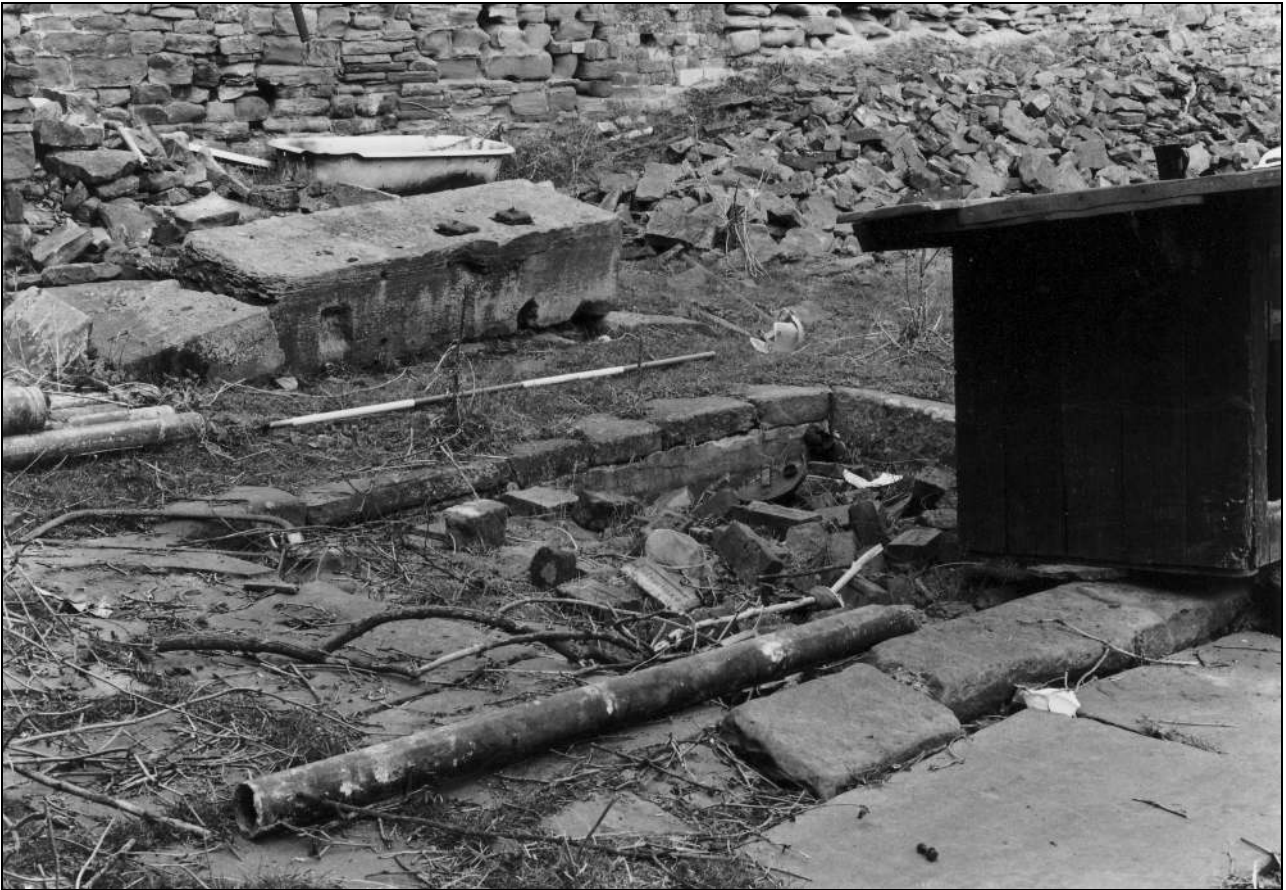
Photo 58: Infilled tanpit and possible engine bed block, from the south-west (film 2, frame 10)
