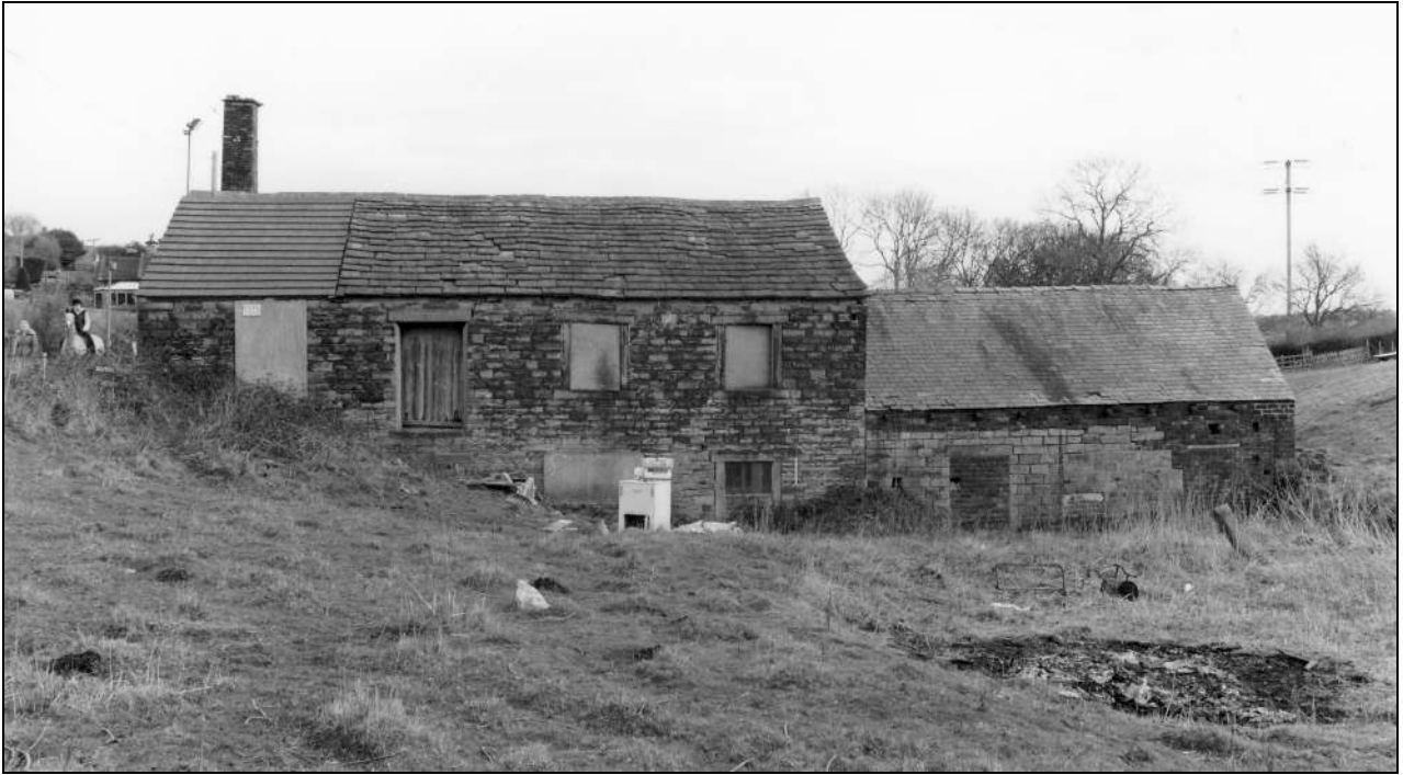
Photo 9: Building 1: west elevation (film 1, frame 1)
