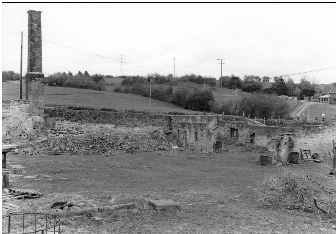
Photo 3: General view of the site (chimney and building 2), from the south-west (film 1, frame 12)
