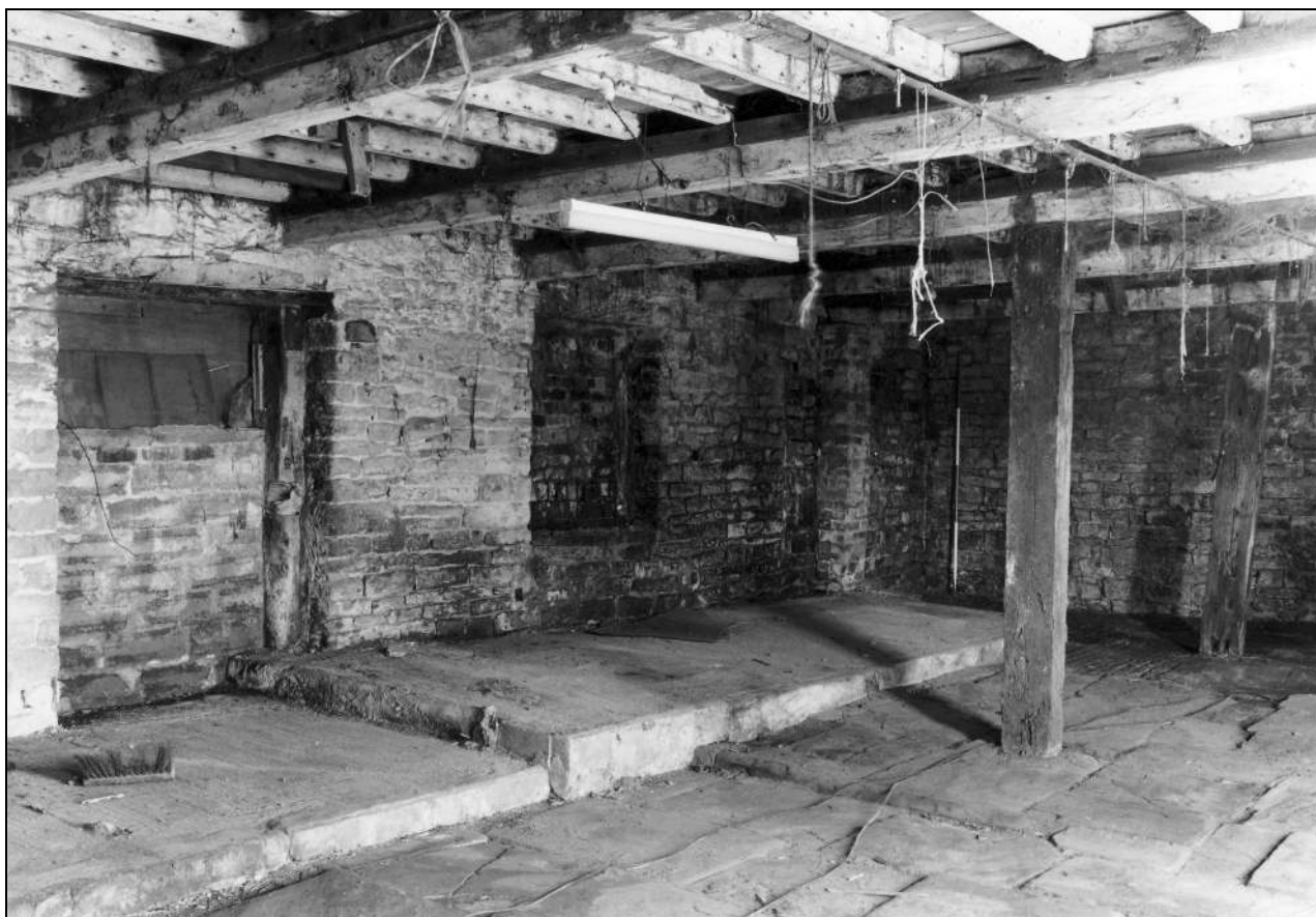
Photo 22: Building 1a: ground floor, from the south-east (film 3, frame 8)
