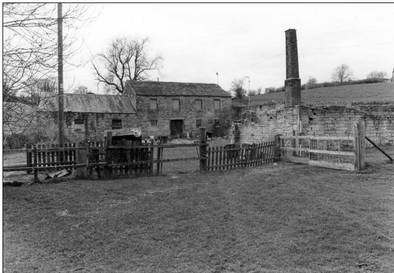
Photo 5: General view of the site, from the south-east (film 2, frame 17)
