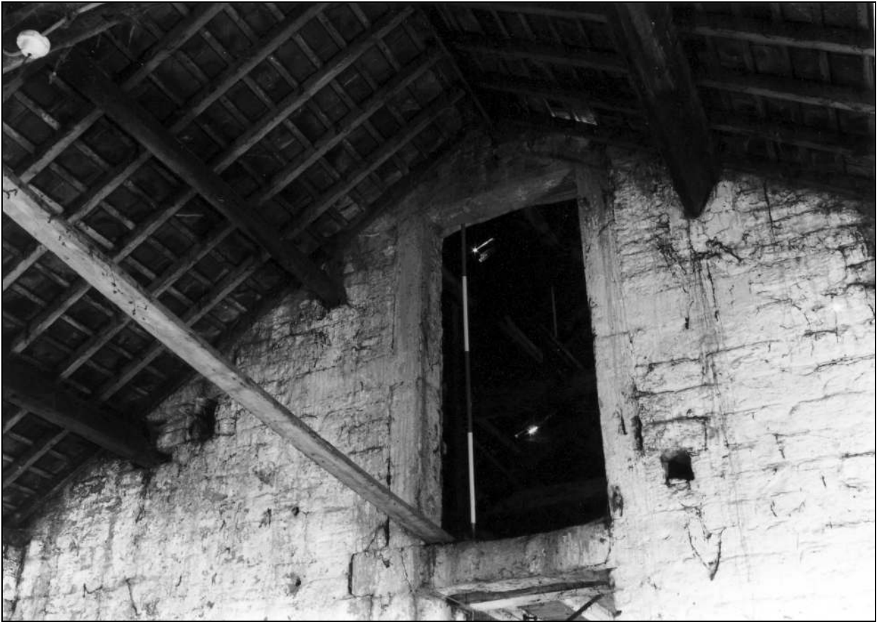
Photo 17: Building 1a: detail of taking-in doorway, south gable (film 3, frame 18)
