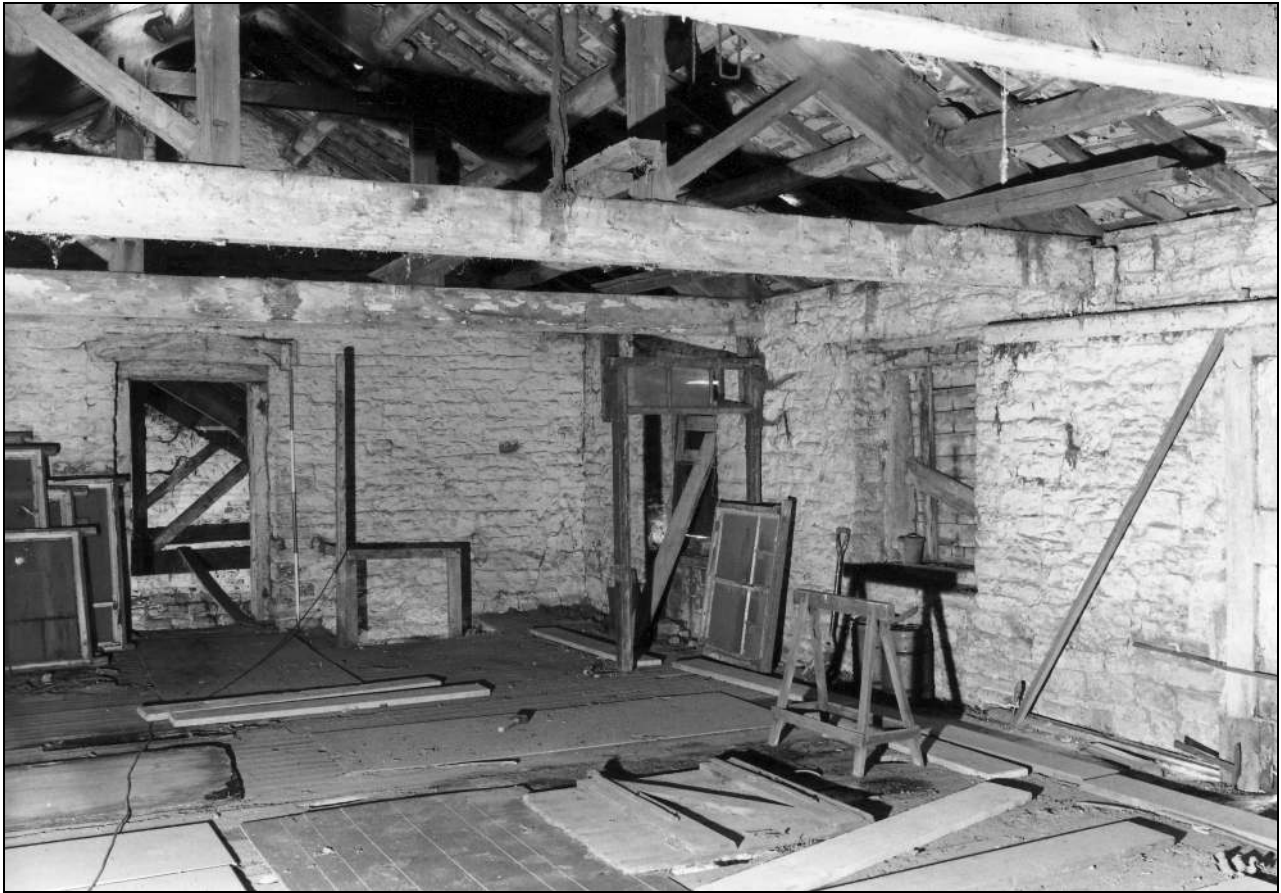
Photo 26: Building 1a: first floor, from the north-east (film 4, frame 12)
