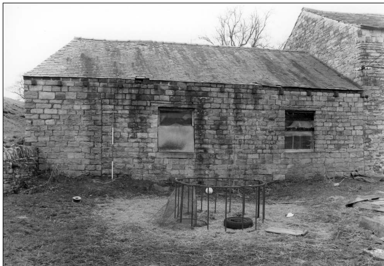
Photo 31: Building 1b: east elevation (film 1, frame 13)
