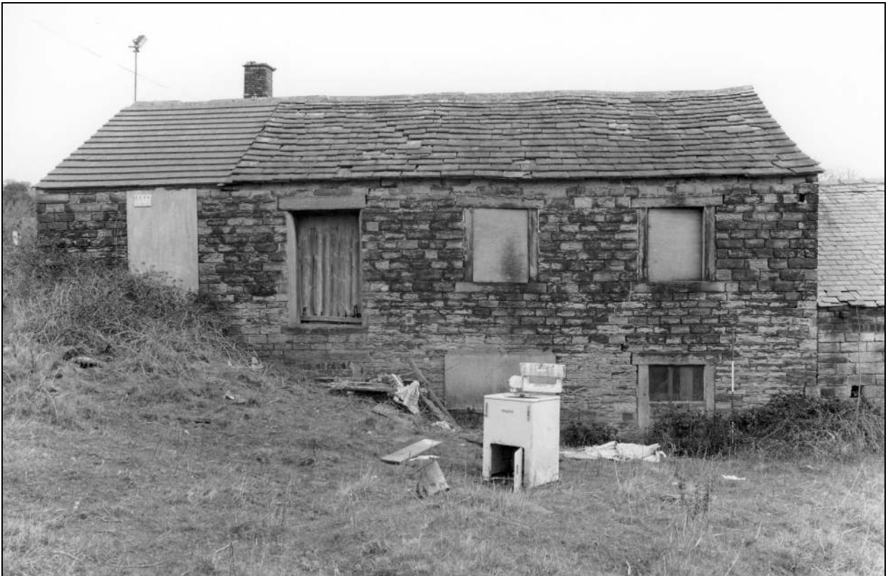
Photo 10: Building 1a: west elevation (film 1, frame 2)
