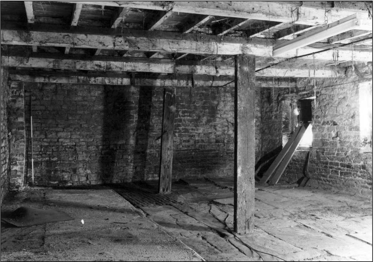
Photo 20: Building 1a: ground floor, from the south-west (film 3, frame 9)
