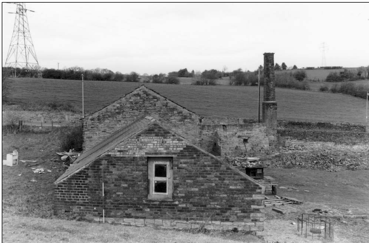
Photo 33: Building 1: general view, from the south (film 1, frame 6)
