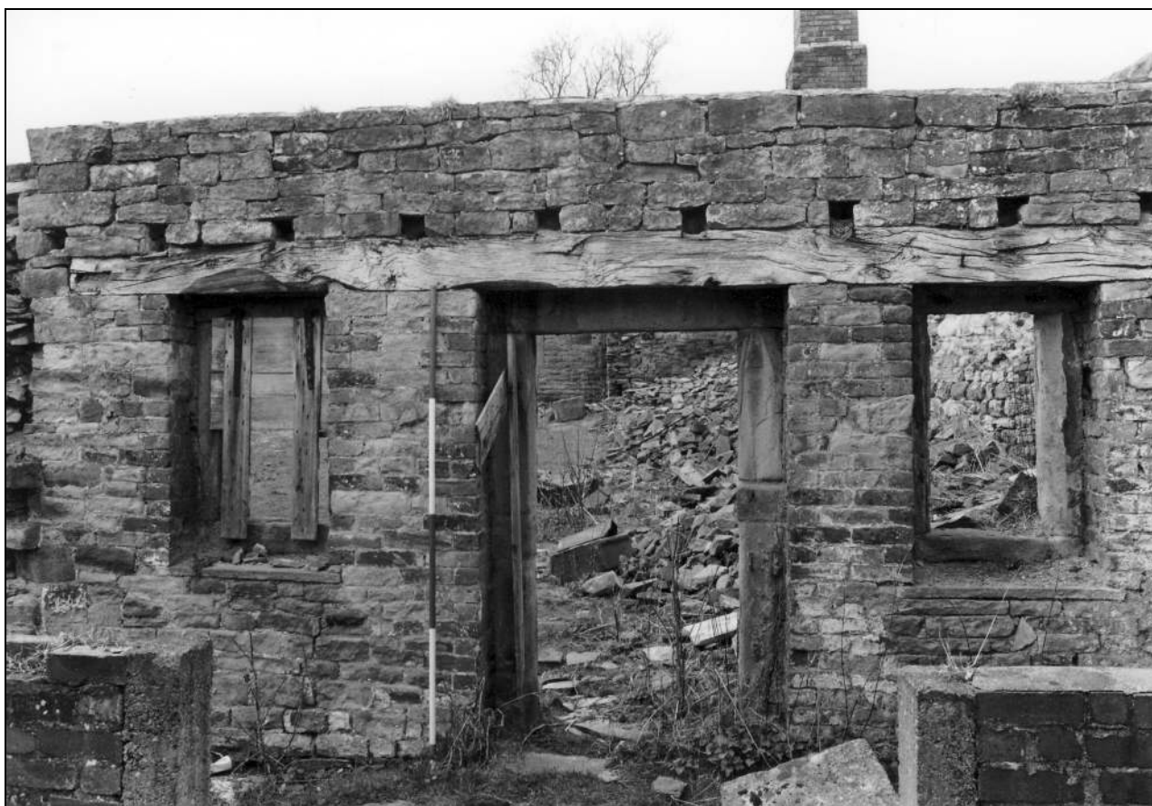
Photo 49: Interior of building 2a, from the east (film 2, frame 14)
