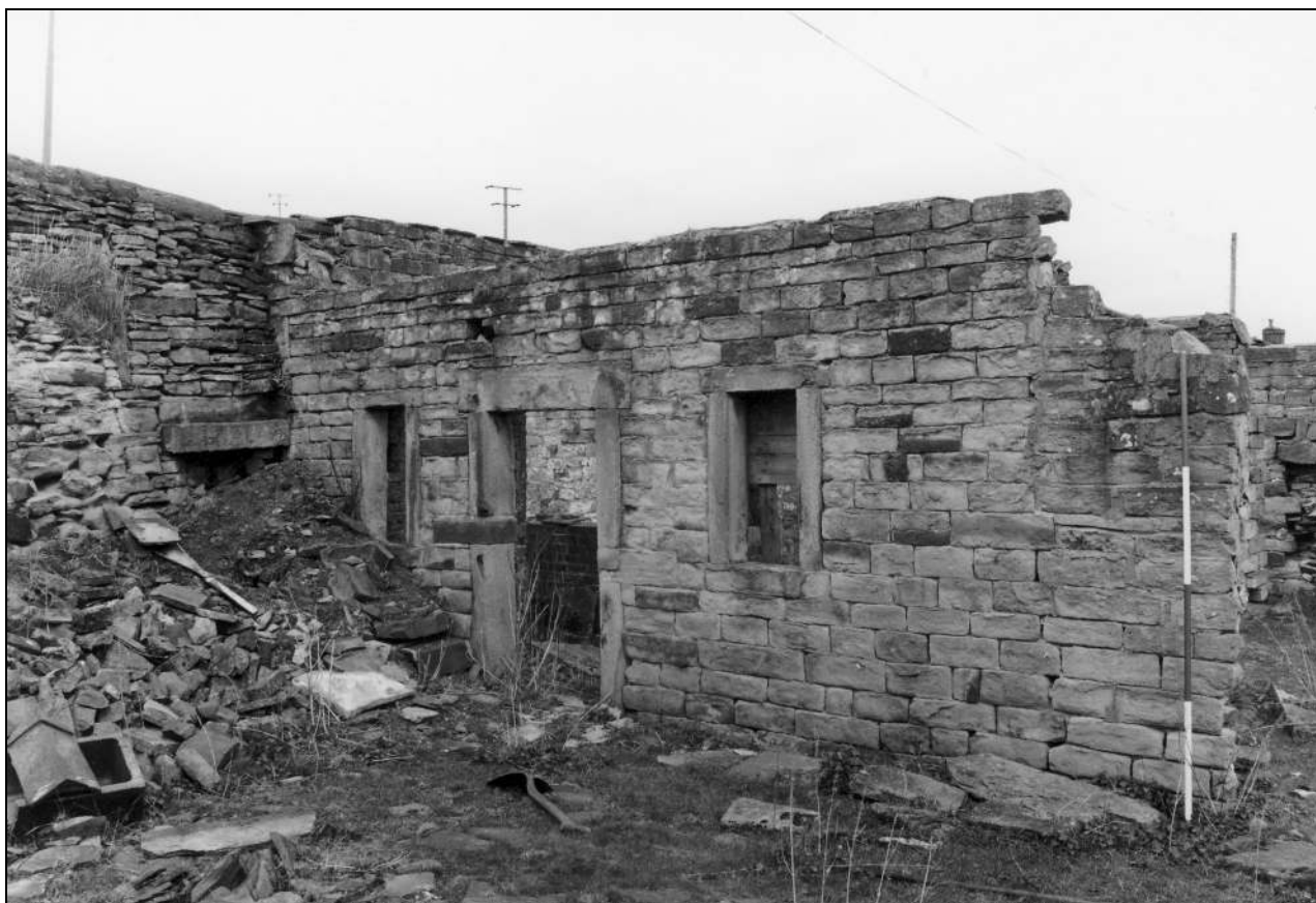
Photo 48: Building 2a: west elevation (film 2, frame 8)
