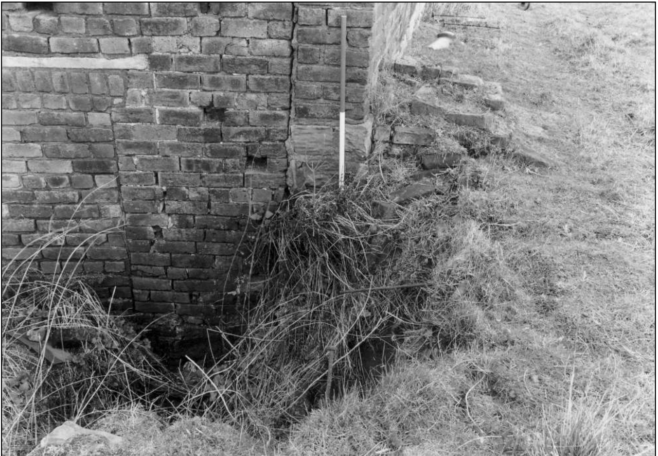
Photo 36: Building 1b: detail of south-west corner (film 1, frame 7)
