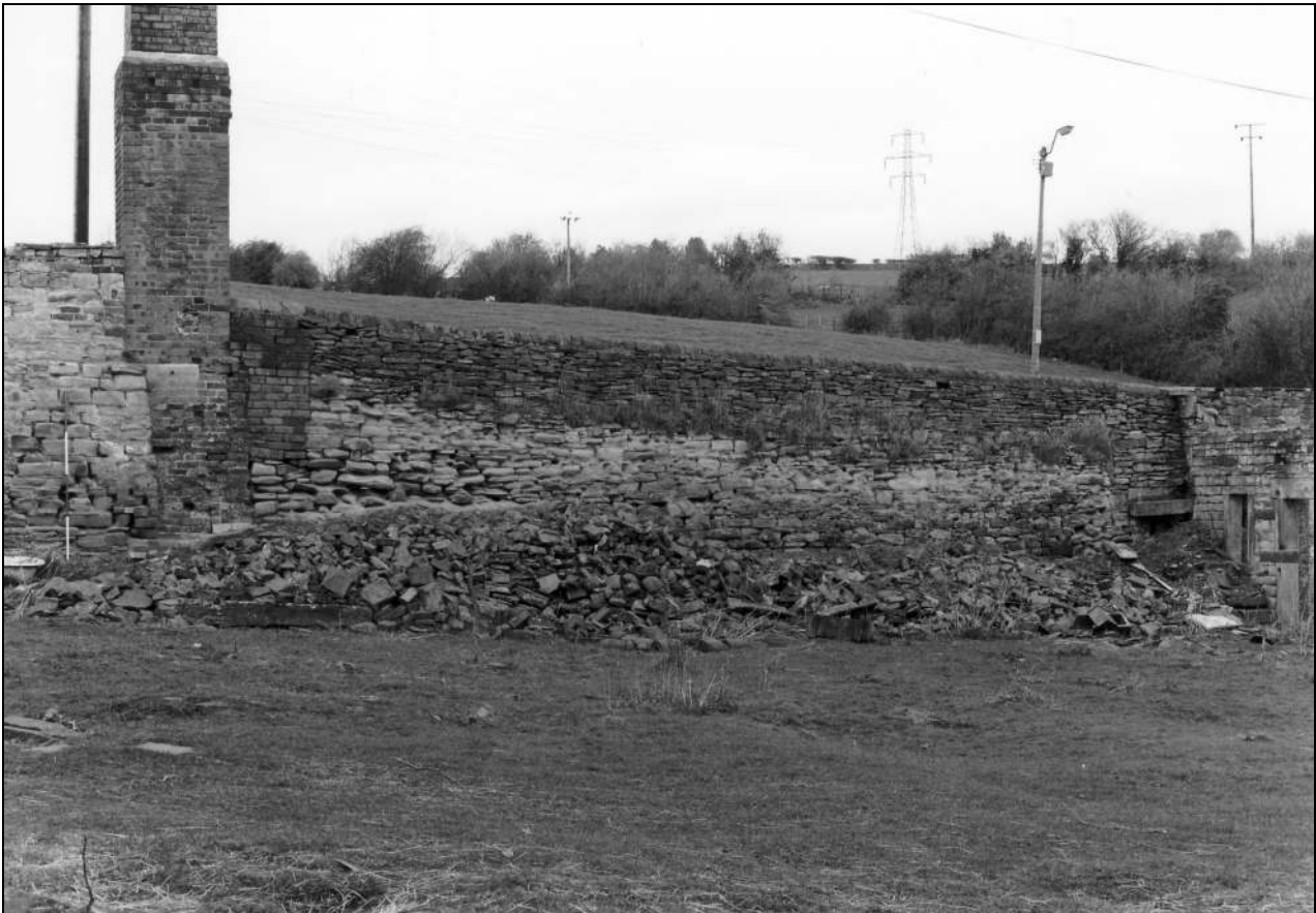
Photo 59: Retaining wall to east of chimney, from the south (film 2, frame 3)
