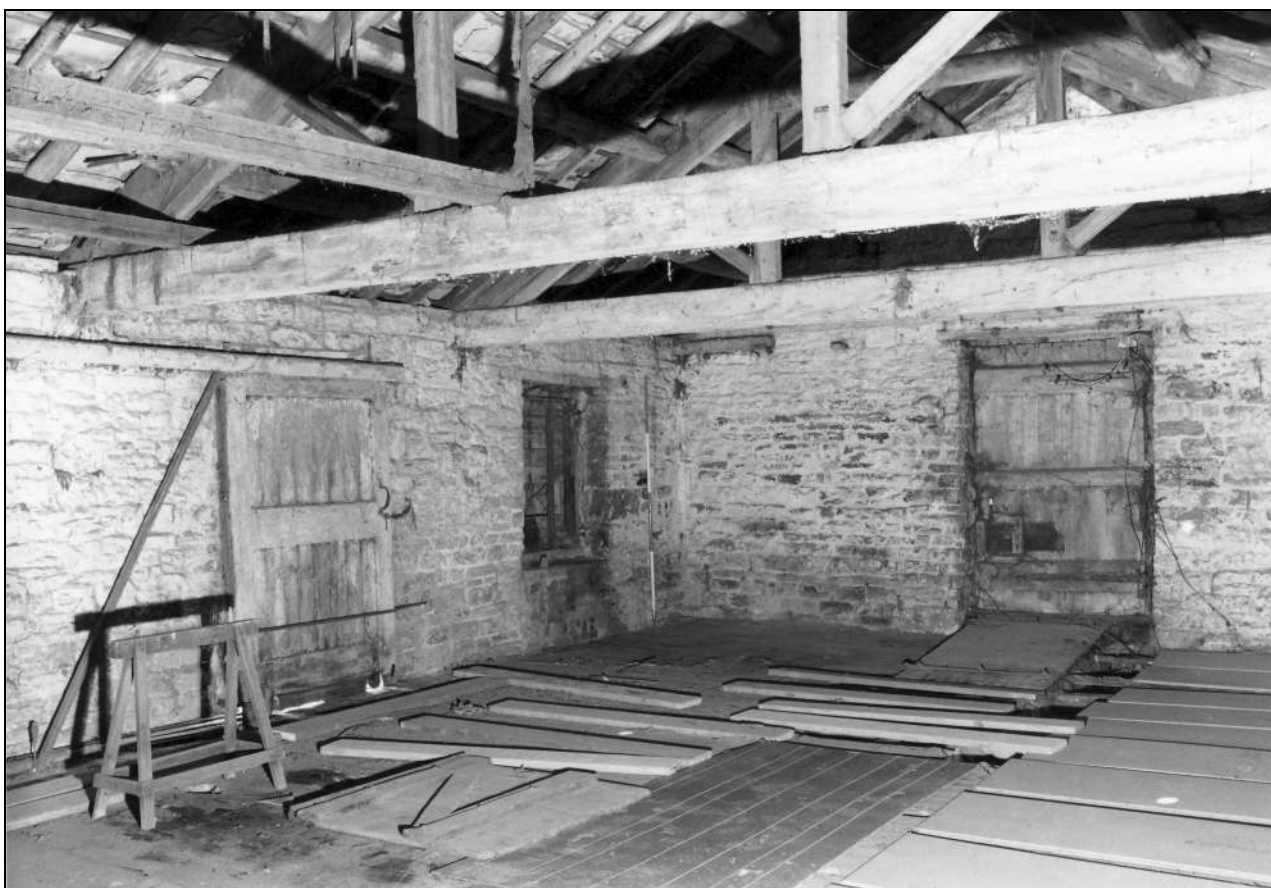
Photo 29: Building 1a: first floor, from the south-east (film 4, frame 11)
