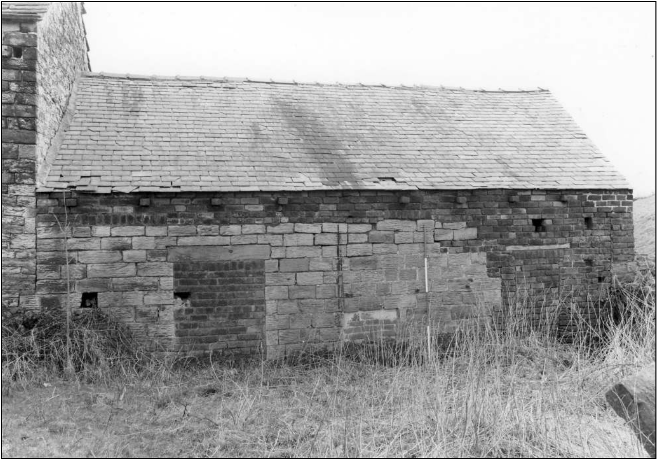
Photo 35: Building 1b: west elevation (film 1, frame 4)
