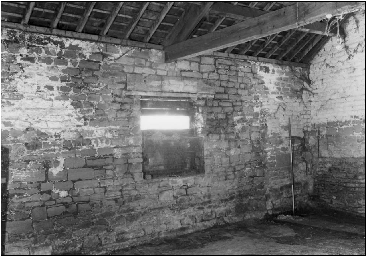
Photo 39: Building 1b: interior, from the north-west (film 4, frame 5)
