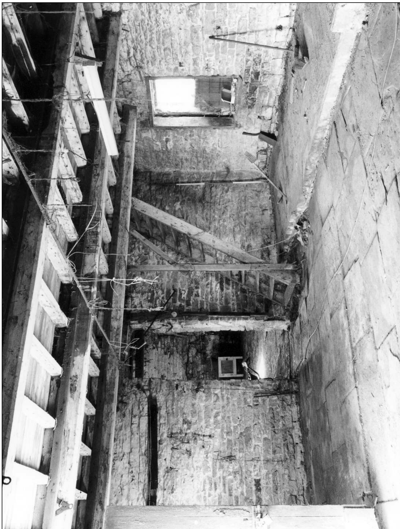
Photo 19: Building 1a: ground floor, from the north-east (film 3, frame 15)
