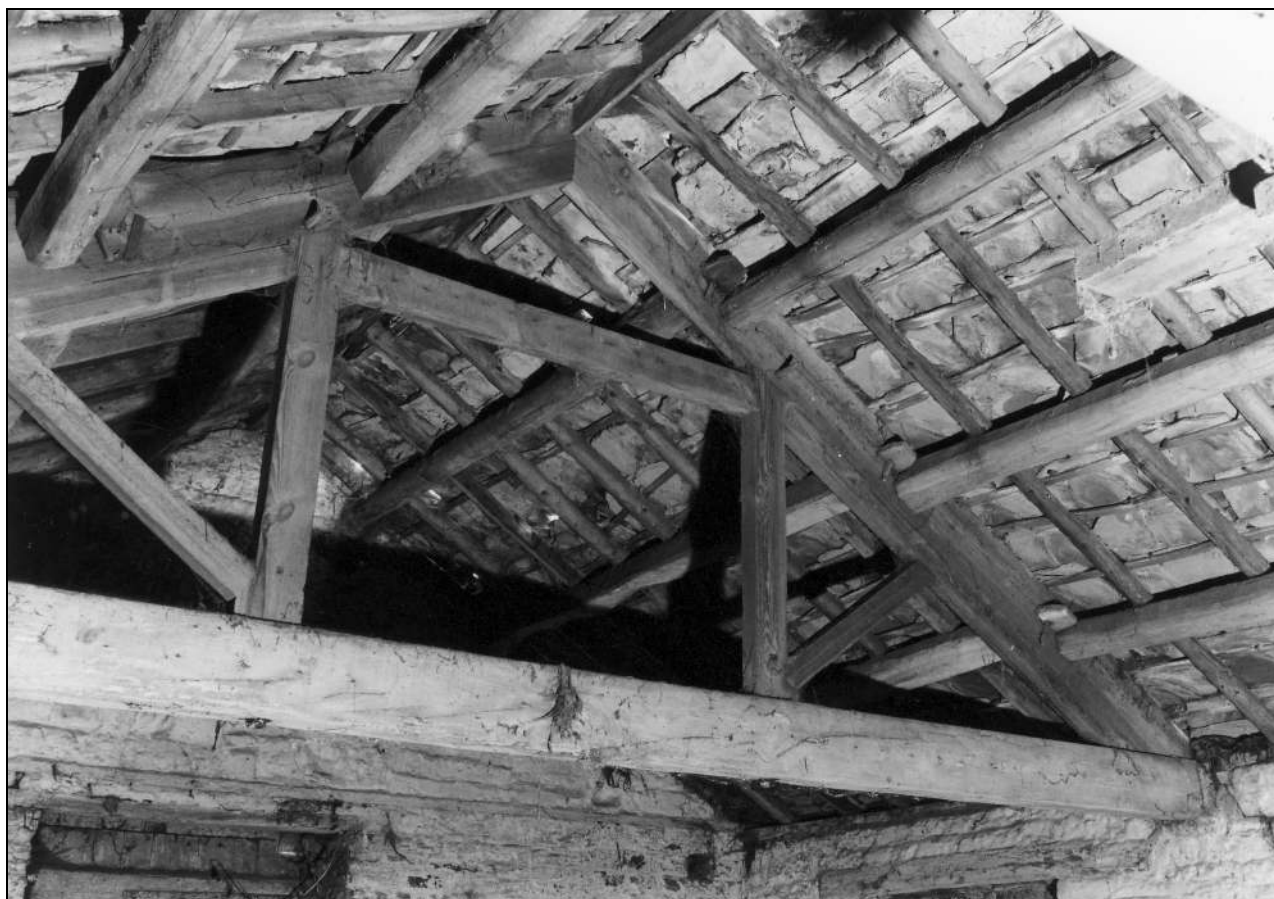
Photo 30: Building 1a: roof truss, from the south-west (film 4, frame 14)
