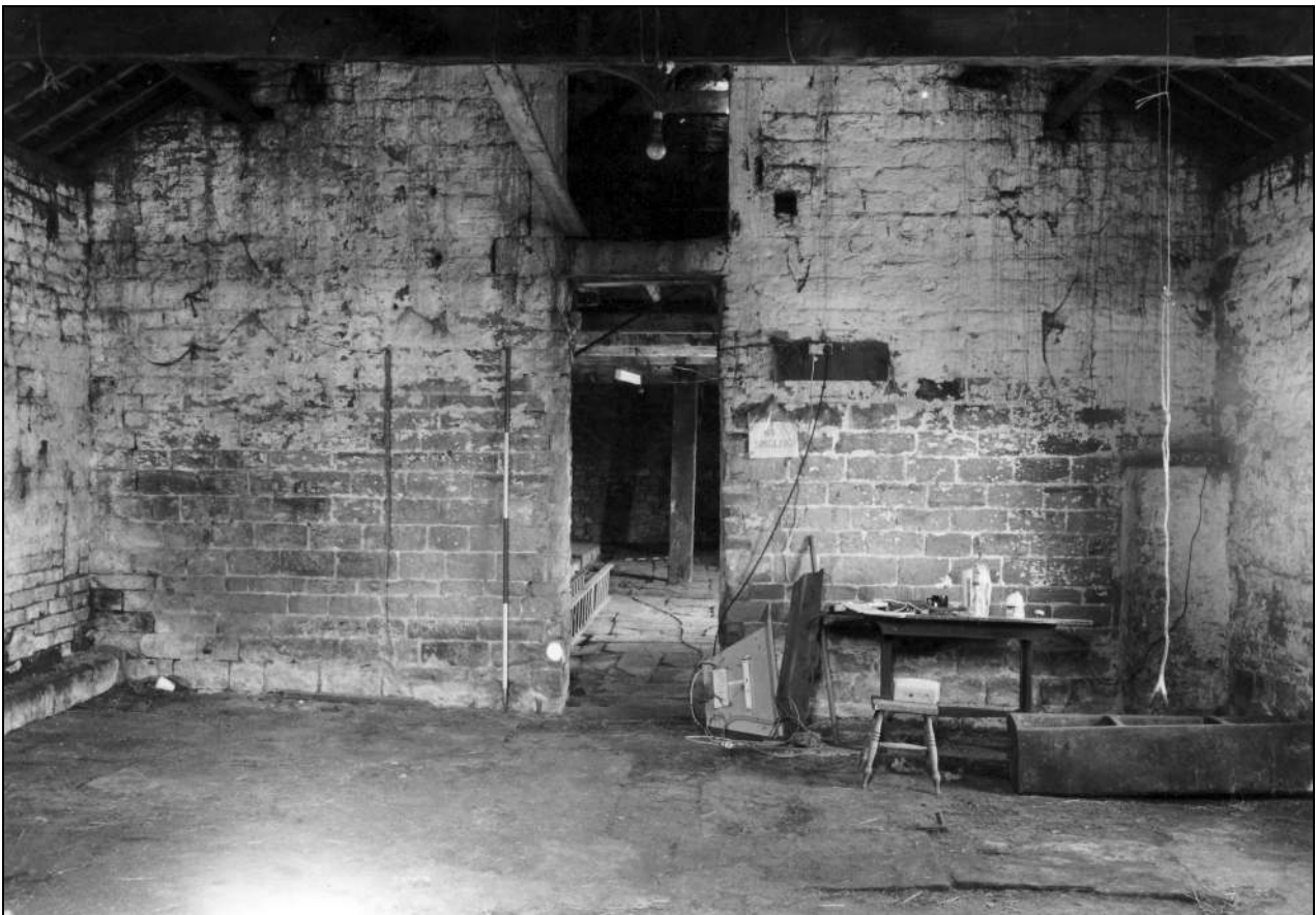
Photo 18: Building 1a: south gable, now within single storey part (film 3, frame 17)
