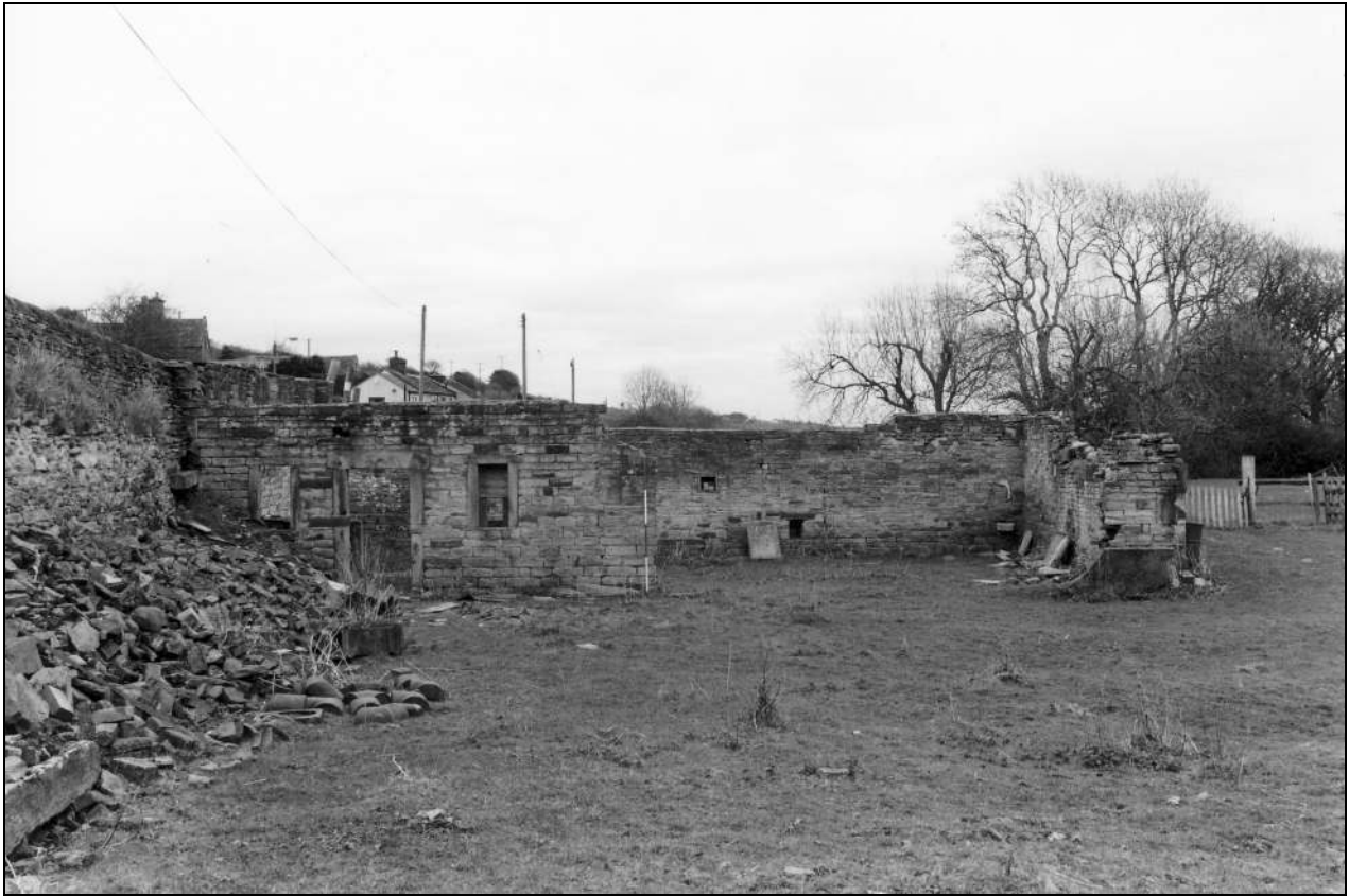
Photo 46: Building 2: west elevation (film 2, frame 6)
