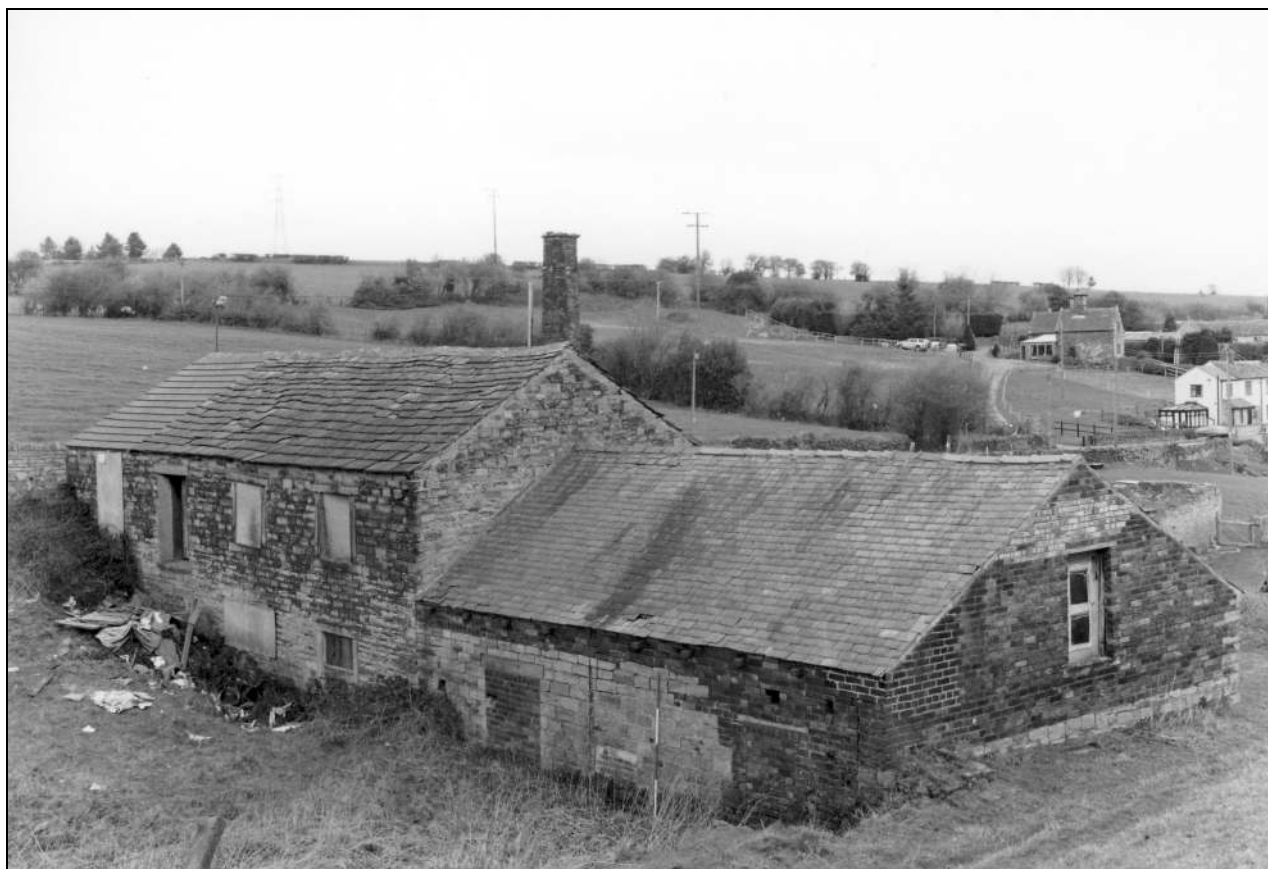
Photo 34: Building 1: general view, from the south-west (film 1, frame 5)
