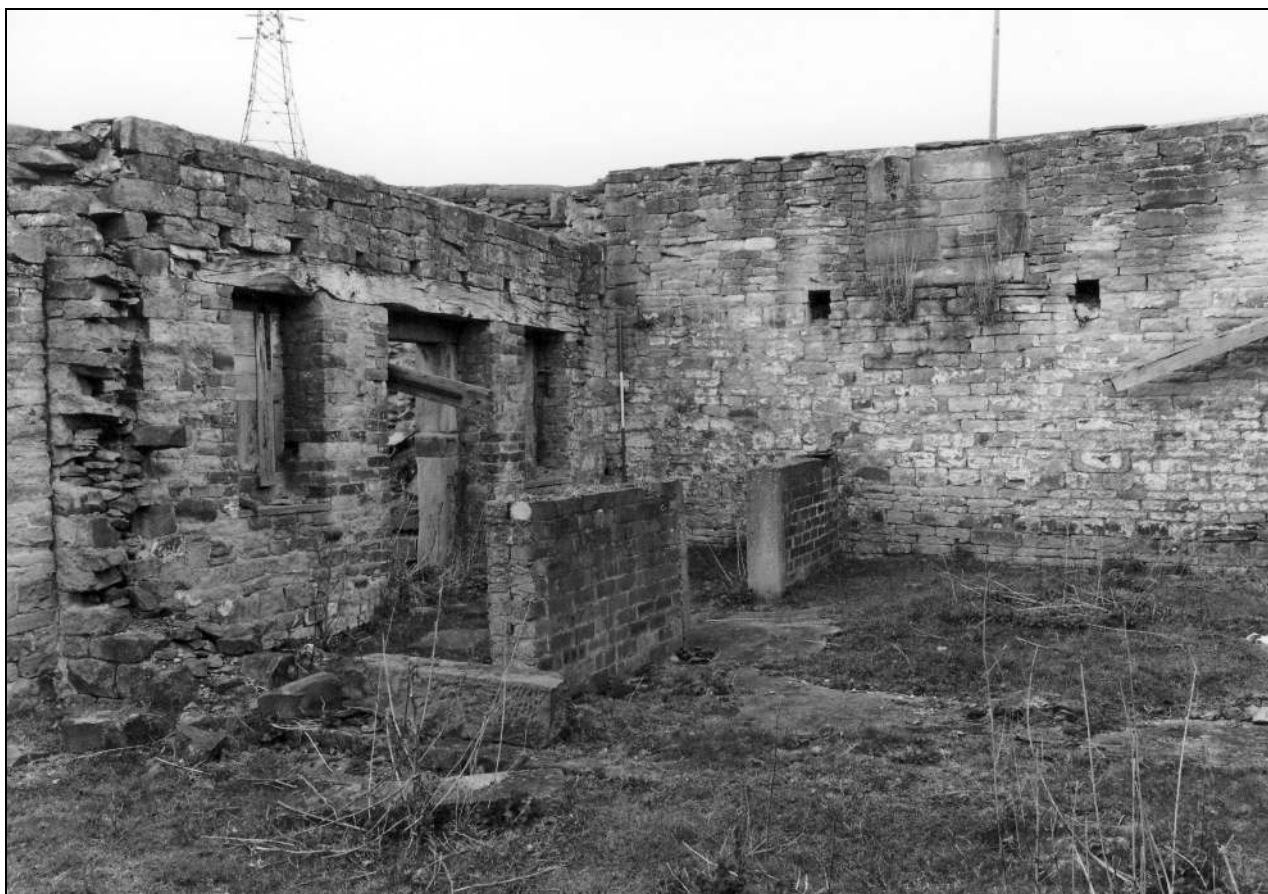
Photo 50: Interior of building 2a, from the south-east (film 2, frame 11)
