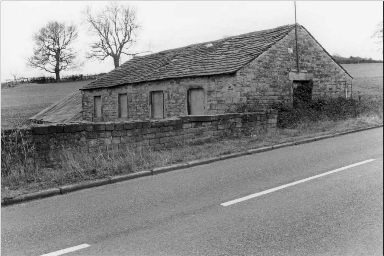
Photo 13: Building 1a, from the north-east (film 3, frame 4)
