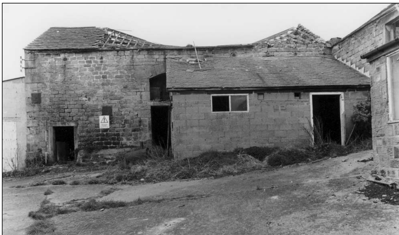
Photo 2: Barn: east elevation (film 1, frame 14)
