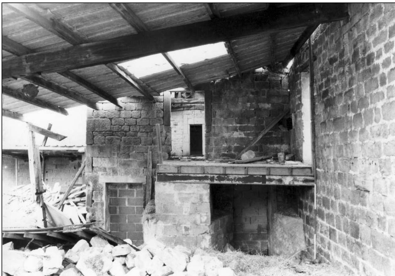
Photo 18: North range: west gable (film 2, frame 6)
