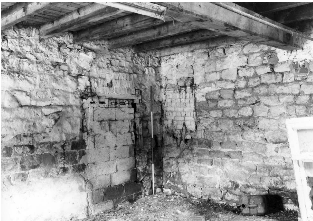
Photo 11: Barn: shippon in south end, from the north-east (film 2, frame 16)
