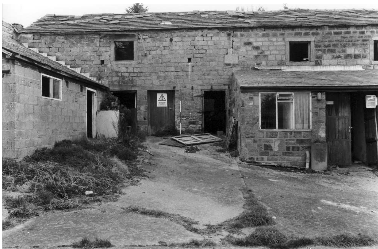
Photo 15: North range: south elevation (west part) (film 1, frame 16)
