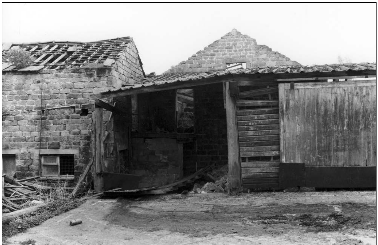
Photo 5: Barn: north gable, and west end of north range (film 2, frame 9)
