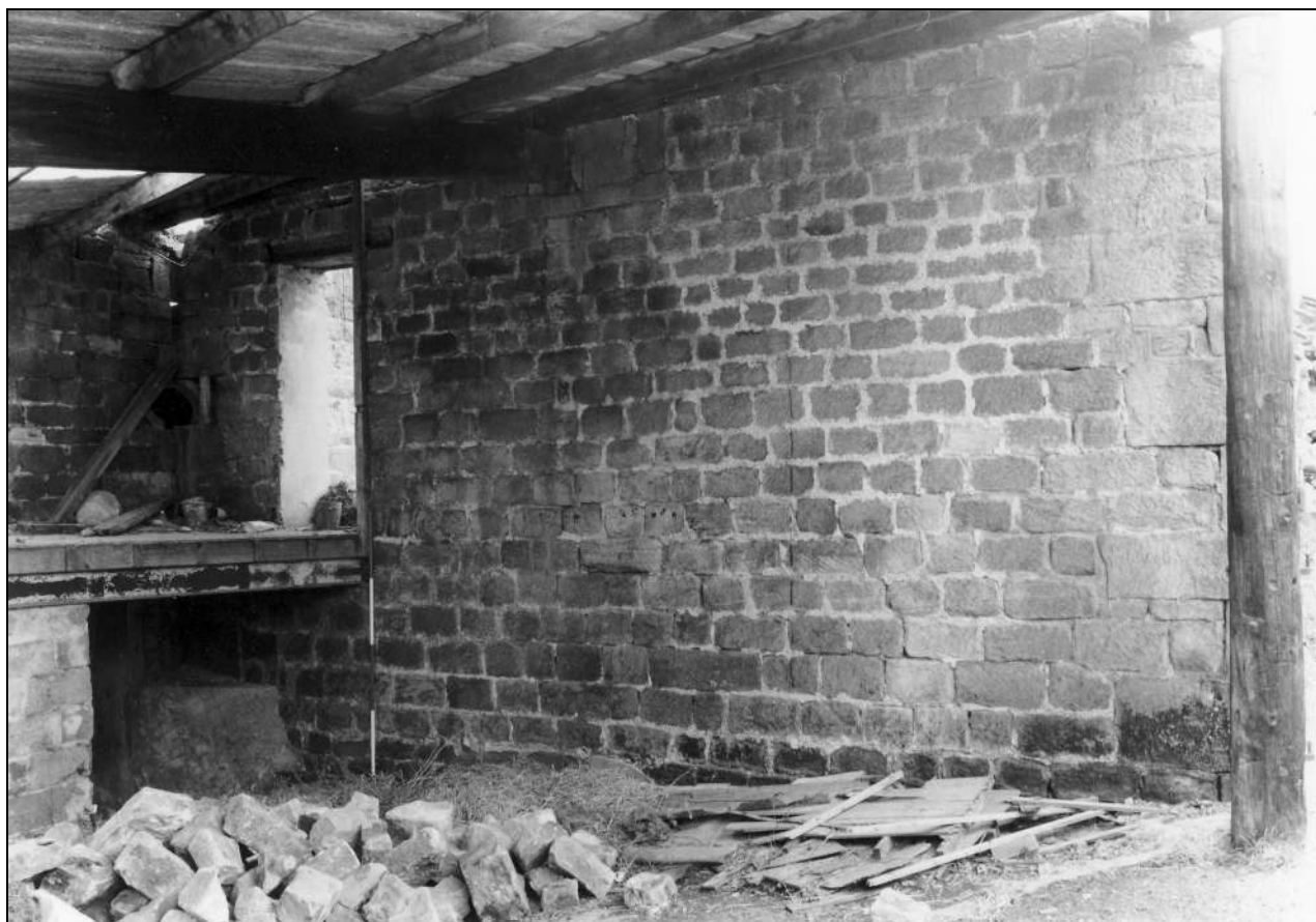
Photo 6: Barn: north gable (film 2, frame 8)
