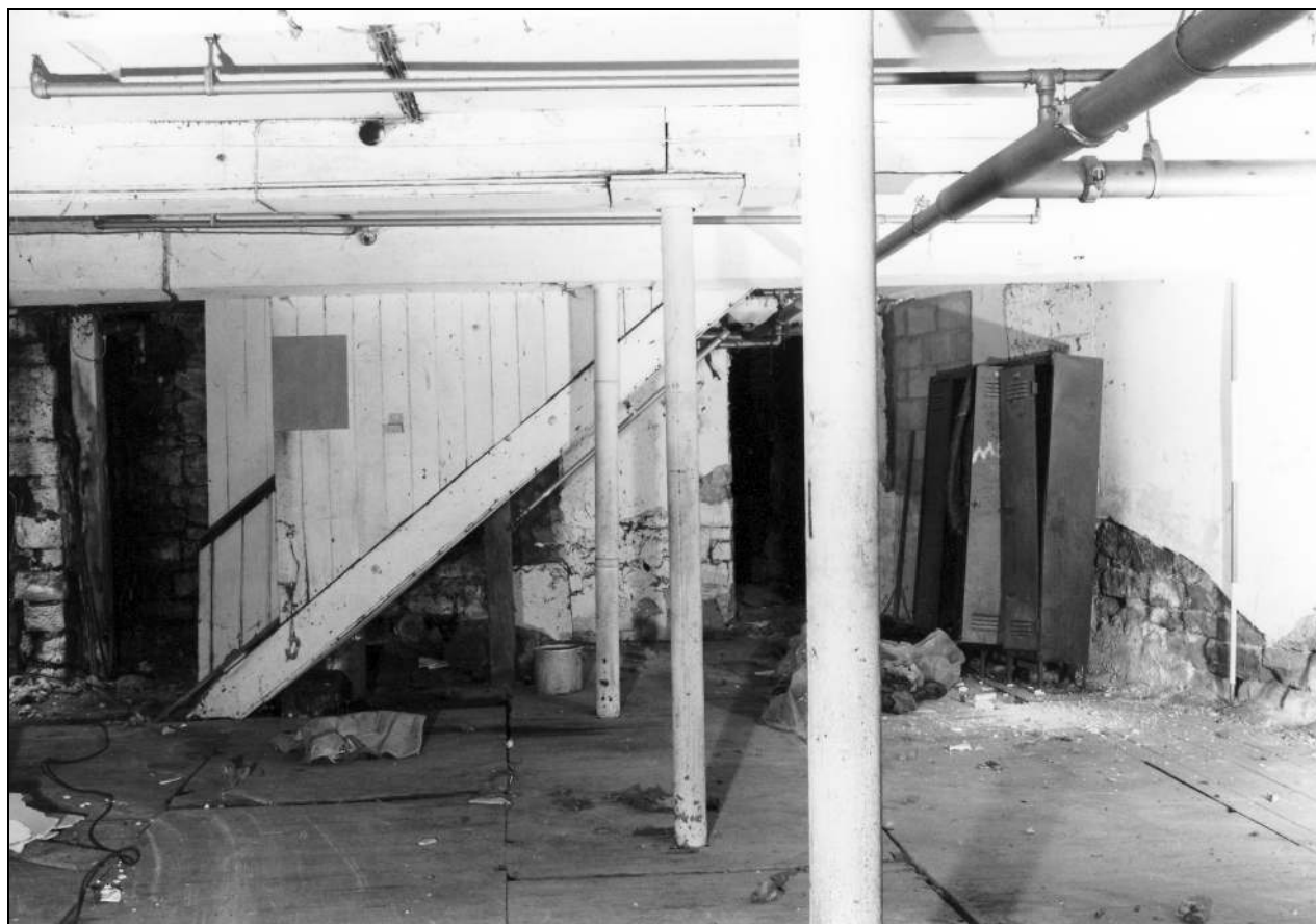
Photo 22: Ground floor of spinning mill, from the east (film 6, frame 17)
