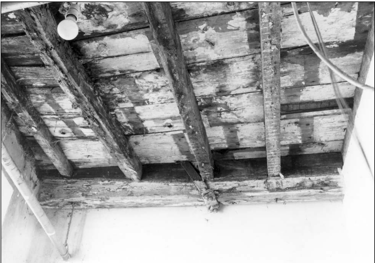
Photo 44: Second floor of spinning mill, from the south-west, showing underside of third floor and tie beam with strap (film 4, frame 5)
