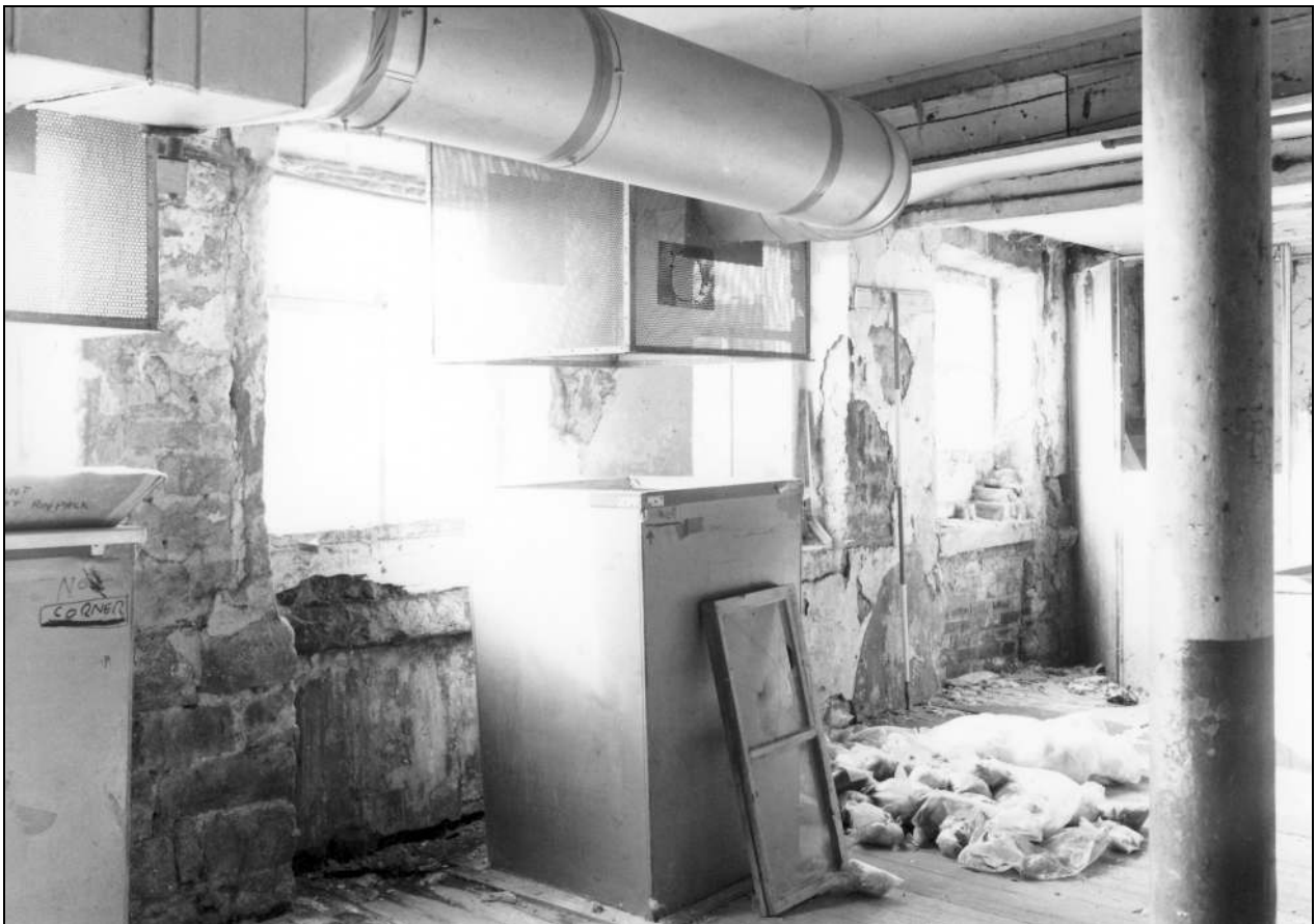
Photo 38: First floor of spinning mill, from the north-east (film 4, frame 2)
