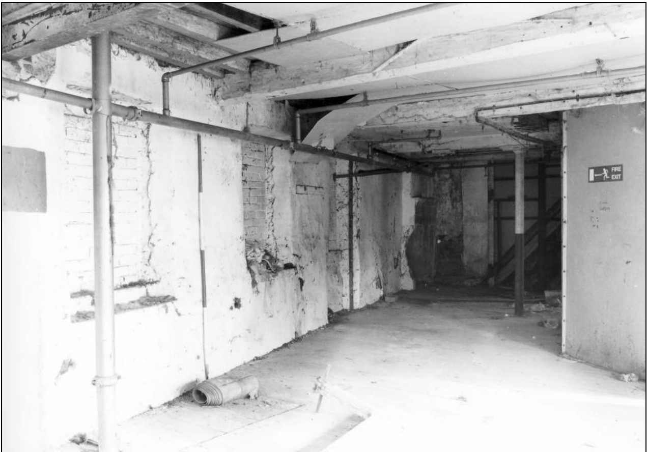
Photo 40: First floor of spinning mill, from the south-west (film 7, frame 11)
