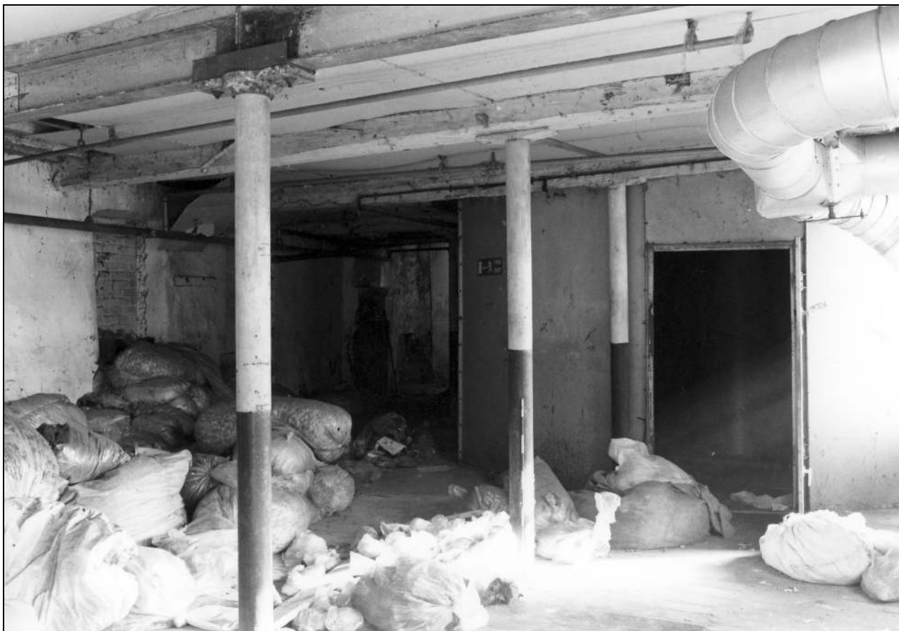
Photo 31: First floor of spinning mill, from the south-west (film 3, frame 15)
