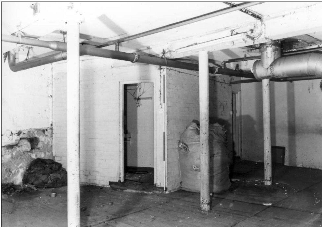
Photo 23: Ground floor of spinning mill, from the south-west (film 6, frame 16)
