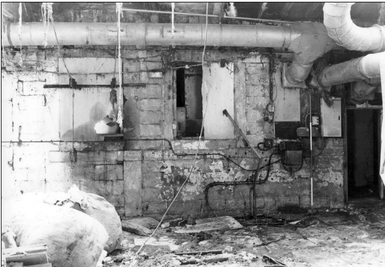
Photo 18: Ground floor openings, south elevation of spinning mill (film 2, frame 9)
