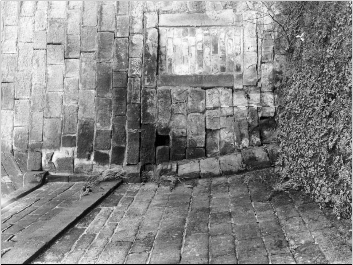
Photo 5: North-east corner of spinning mill, adjoining canal bridge (film 5 frame 9)
