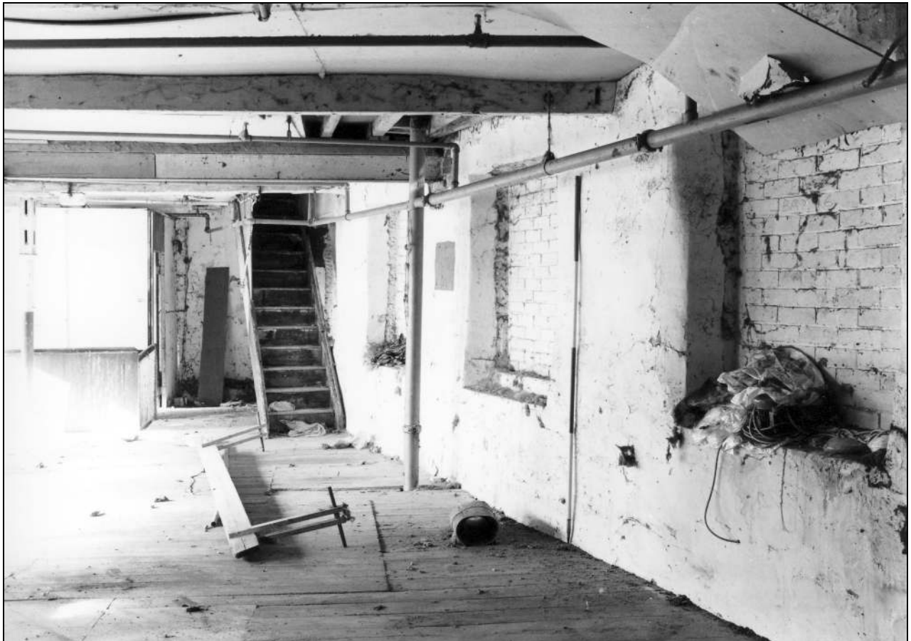
Photo 42: First floor of spinning mill, from the east (film 7, frame 10)
