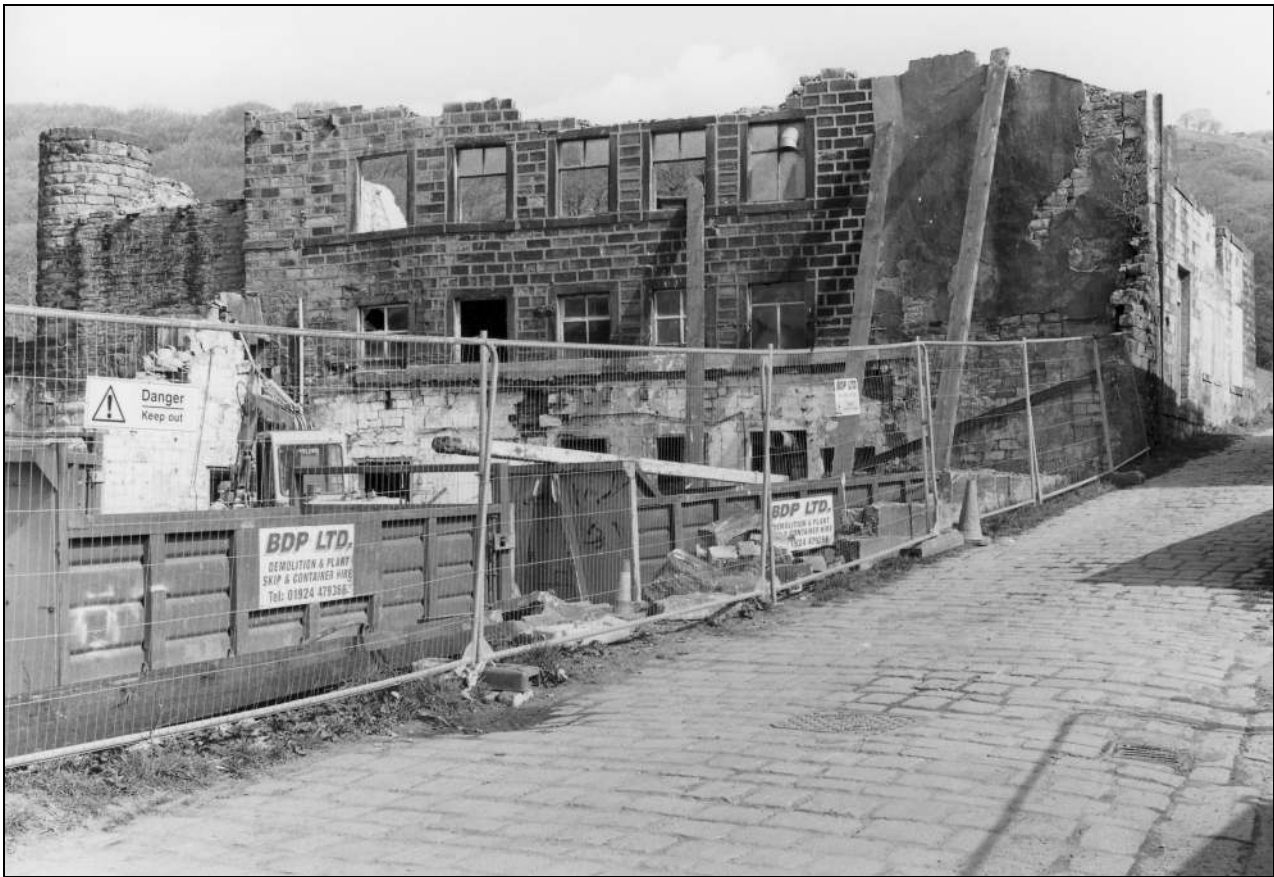
Photo 13: The spinning mill, from the south-east, during demolition (film 10, frame 7)
