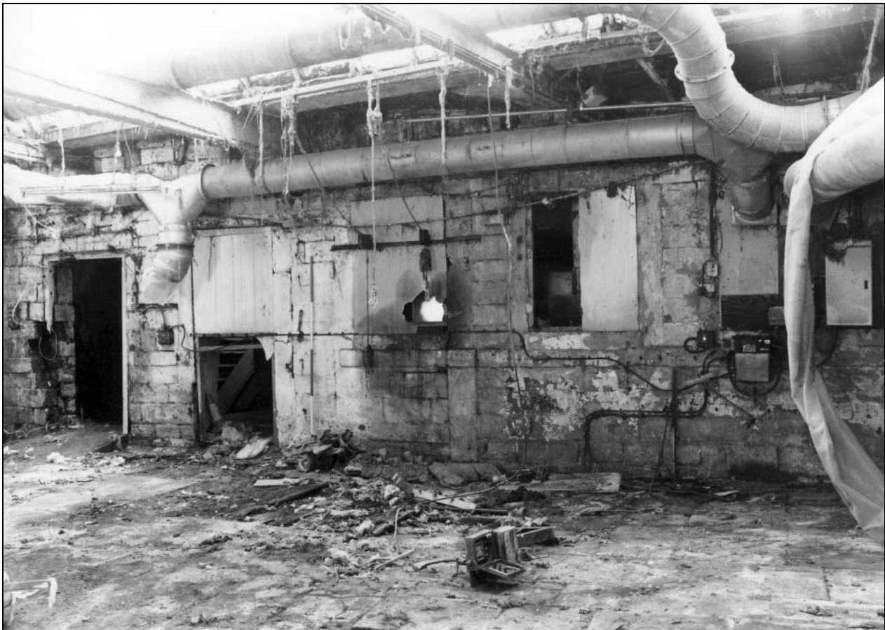
Photo 17: Ground floor openings, south elevation of spinning mill (film 4, frame 9)
