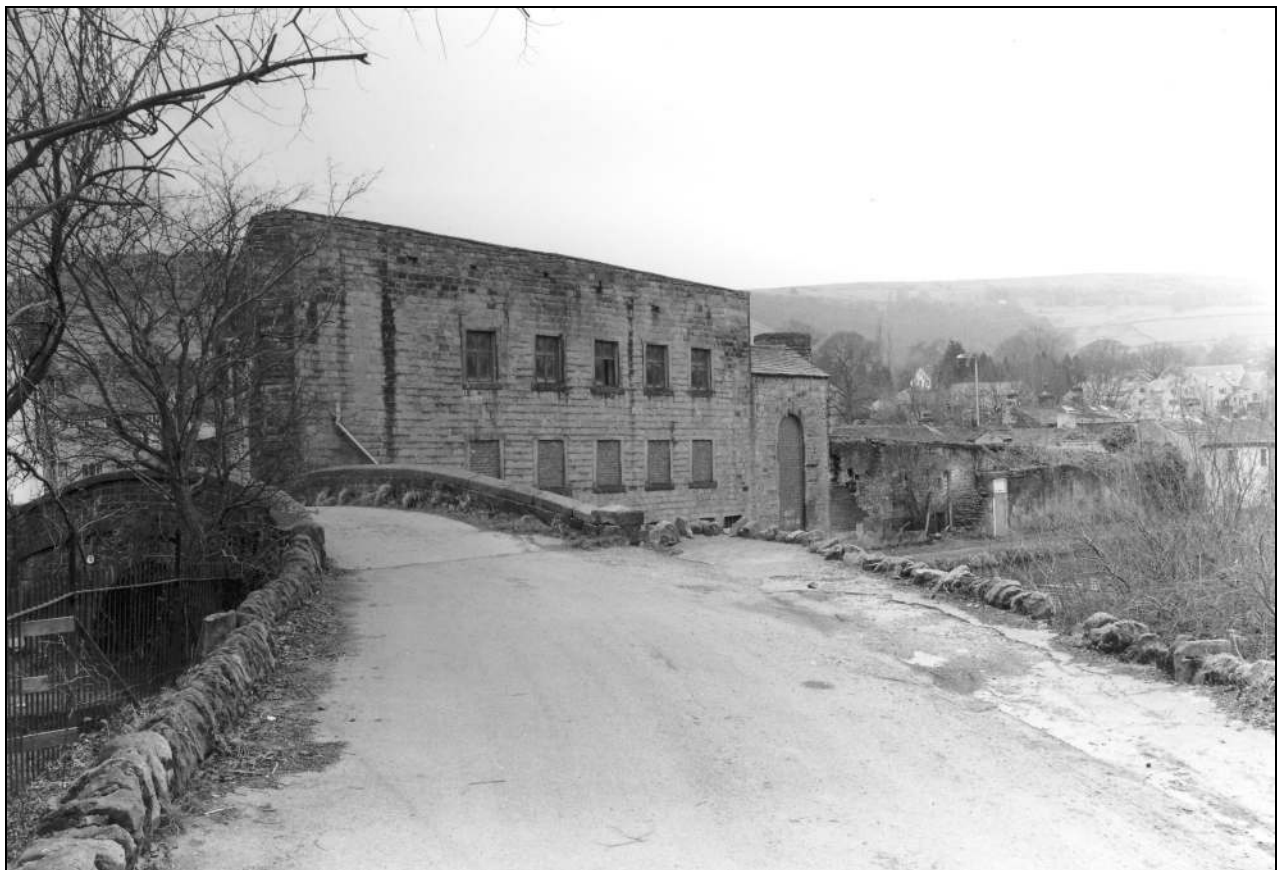
Photo 4: Spinning mill, engine and boiler houses, from the north-east, across Broadbottom Bridge (film 8, frame 6)
