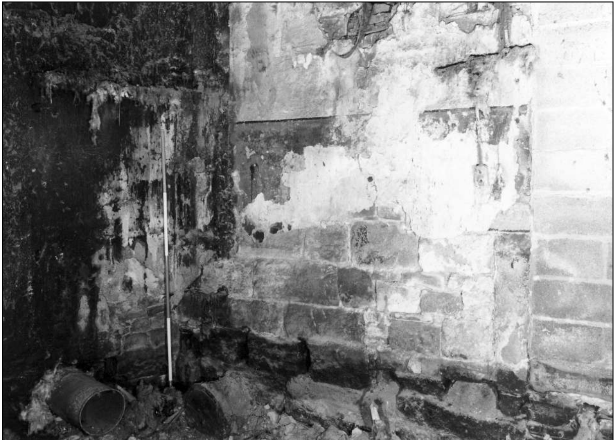
Photo 57: Interior of engine house: south-west corner, showing remains of decoration and grease from flywheel (film 6, frame 3)
