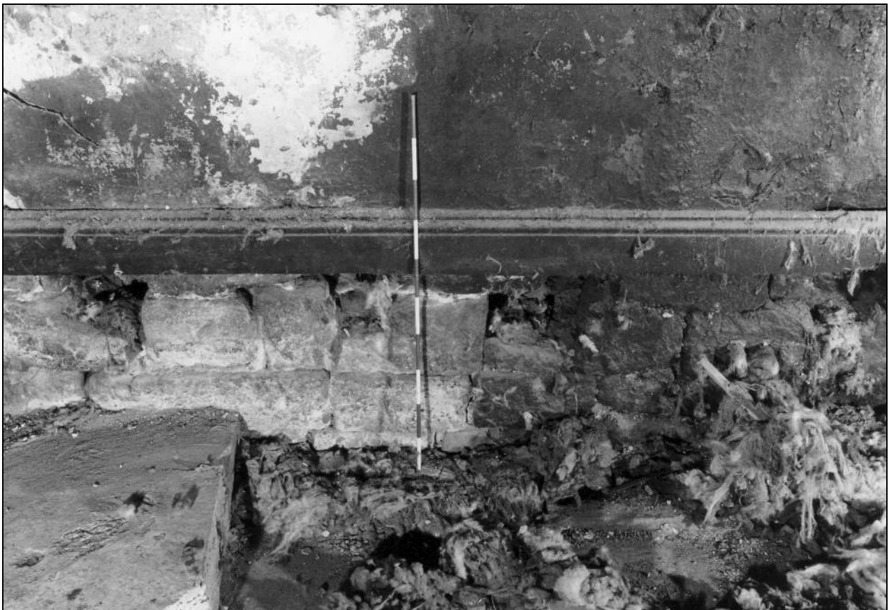
Photo 59: Interior of engine house: remains of skirting, east side (film 5, frame 15)
