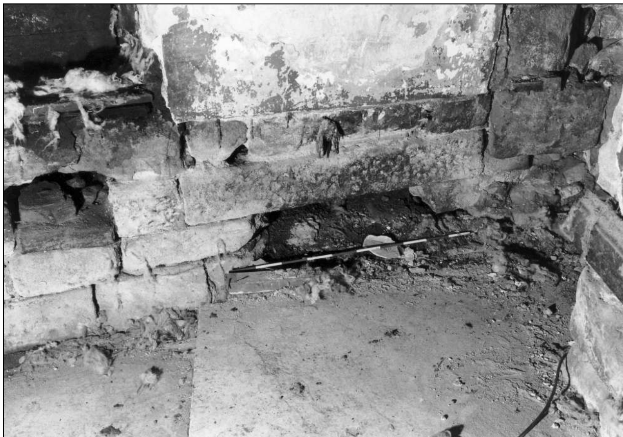
Photo 69: Interior of engine house: ground level opening, north-east corner (film 6, frame 9)
