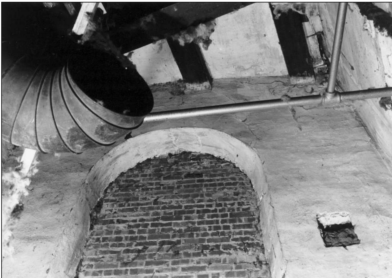
Photo 68: Interior of engine house: top of north window (film 6, frame 10)
