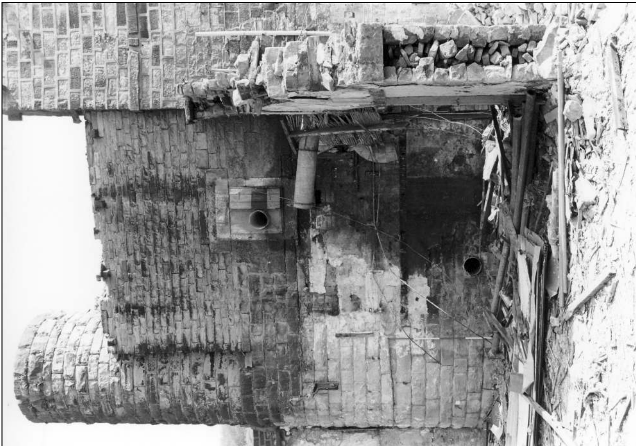
Photo 54: Interior of engine house: south side, showing (later?) bearing to weaving shed and openings for fastening rods (film 5, frame 17)
