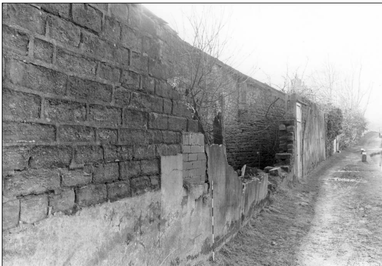
Photo 75: North side of boiler house, from the east (film 5, frame 6)
