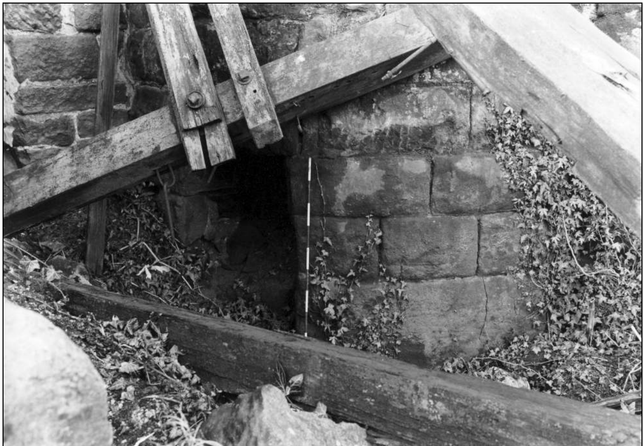
Photo 73: Foot of chimney with flue opening, from the north-west (film 5, frame 4)
