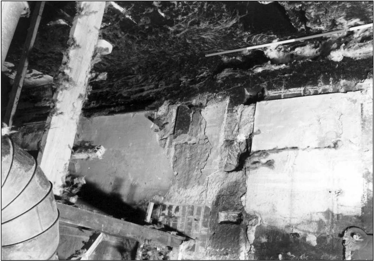
Photo 60: Interior of engine house: south-east corner, upper level, showing gallery and line of former partition enclosing flywheel (film
