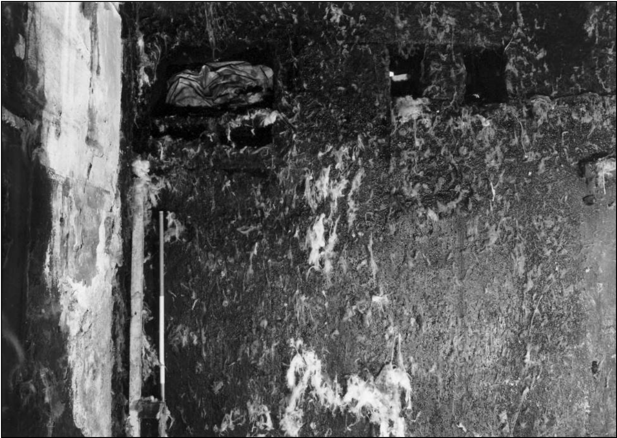
Photo 54: Interior of engine house: south side, showing (later?) bearing to weaving shed and openings for fastening rods (film 5, frame 17)
