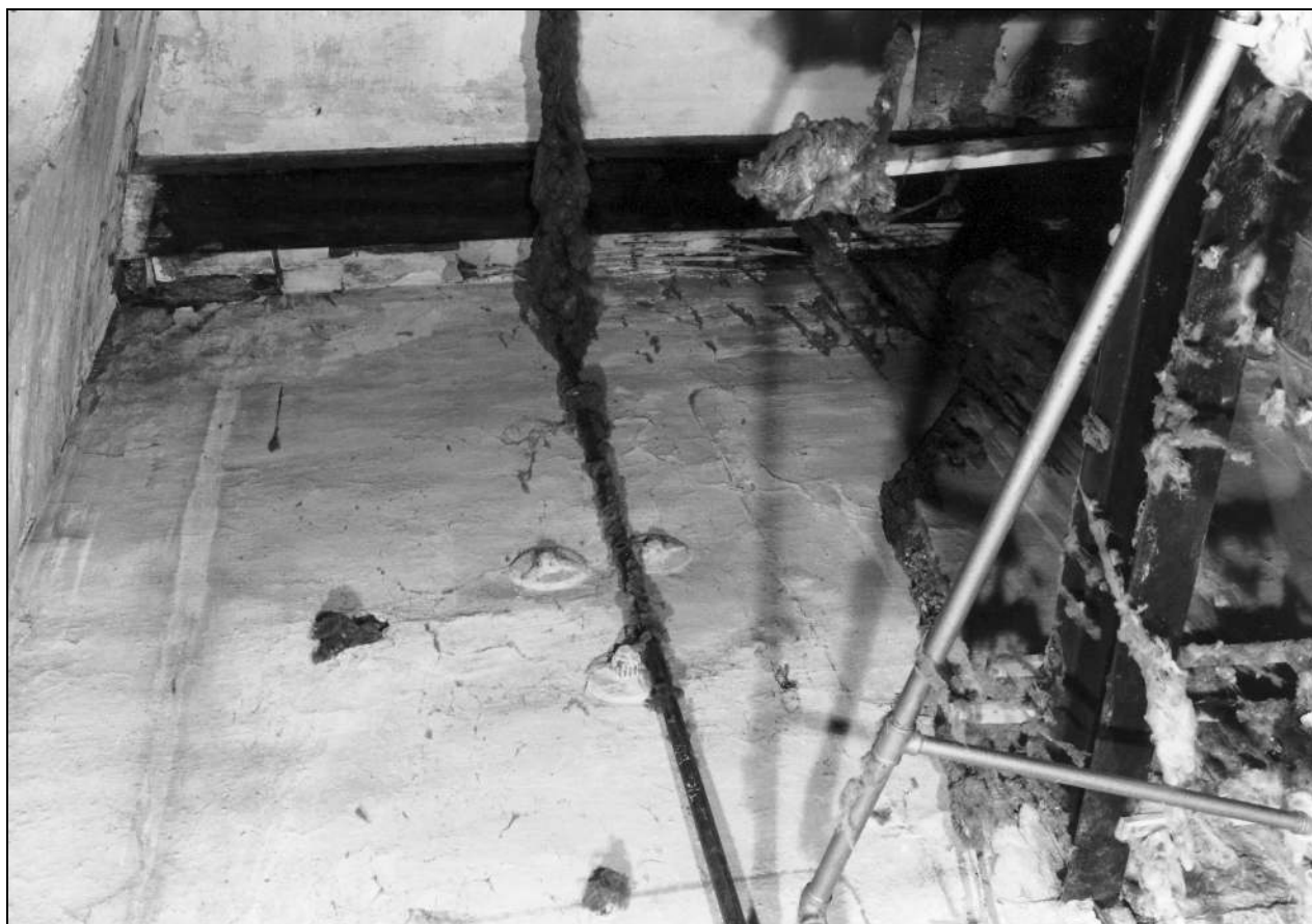
Photo 65: Interior of engine house: upper part of east wall (film 6, frame 11)
