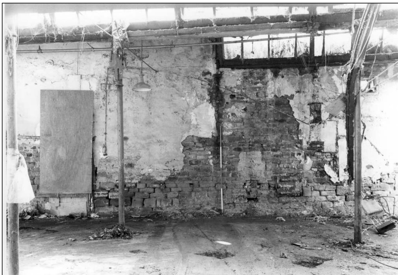
Photo 77: South side of boiler house/north side of weaving shed, from the south (film 1, frame 10)
