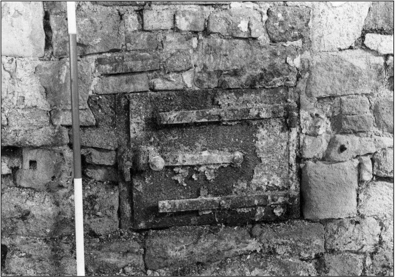
Photo 86: Detail of cast iron door in south side of boiler house, from the south (film 1, frame 15)
