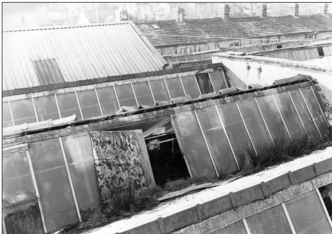
Photo 108: Roof of the covered yard, from the north-east (film 7, frame 13)
