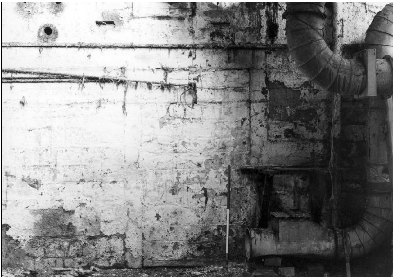
Photo 92: Detail of former doorway in east elevation of weaving shed (film 2, frame 5)
