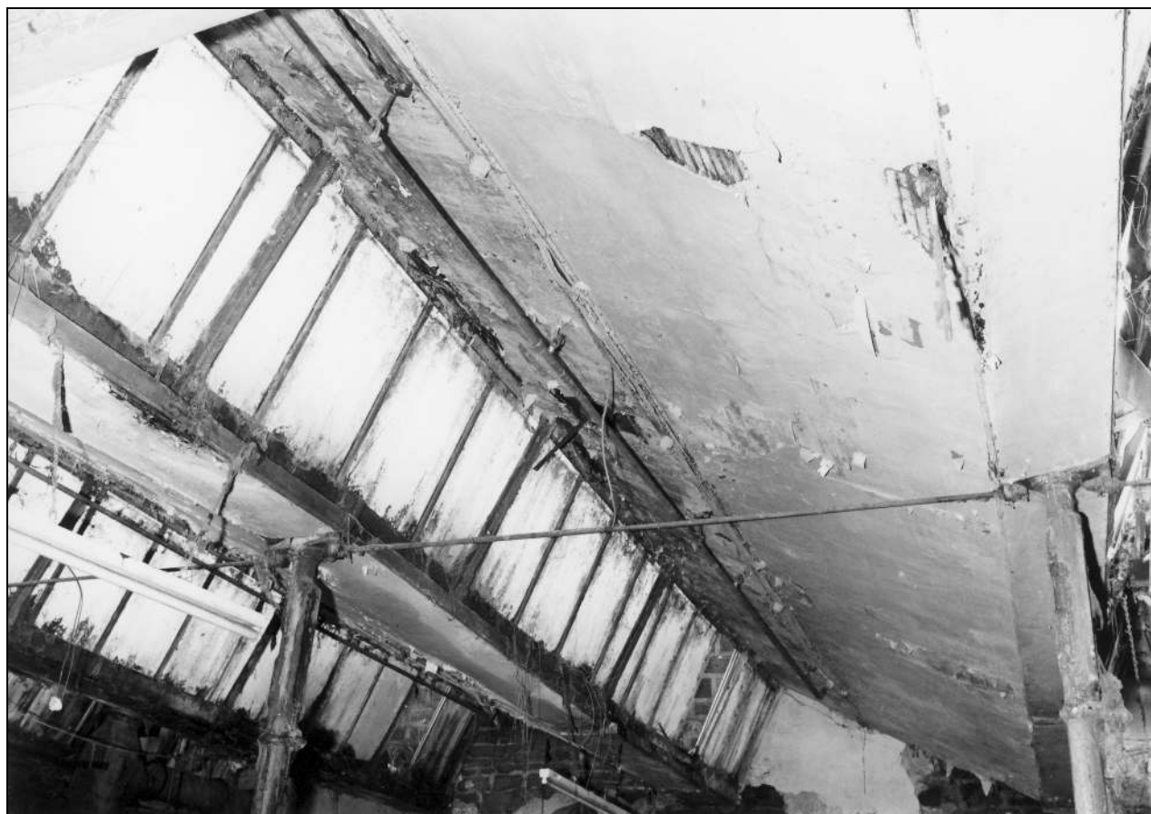
Photo 97: Underside of weaving shed roof, from the west (film 1, frame 6)
