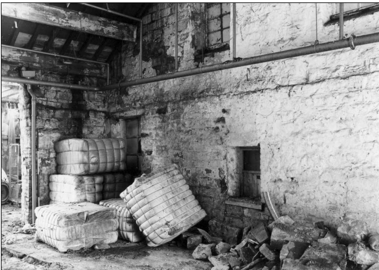
Photo 119: Interior of warehouse, from the south-west (film 2, frame 13)
