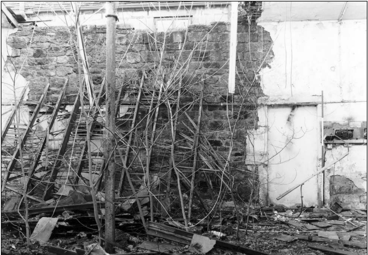
Photo 103: Doorway in south side of weaving shed (film 1, frame 4)
