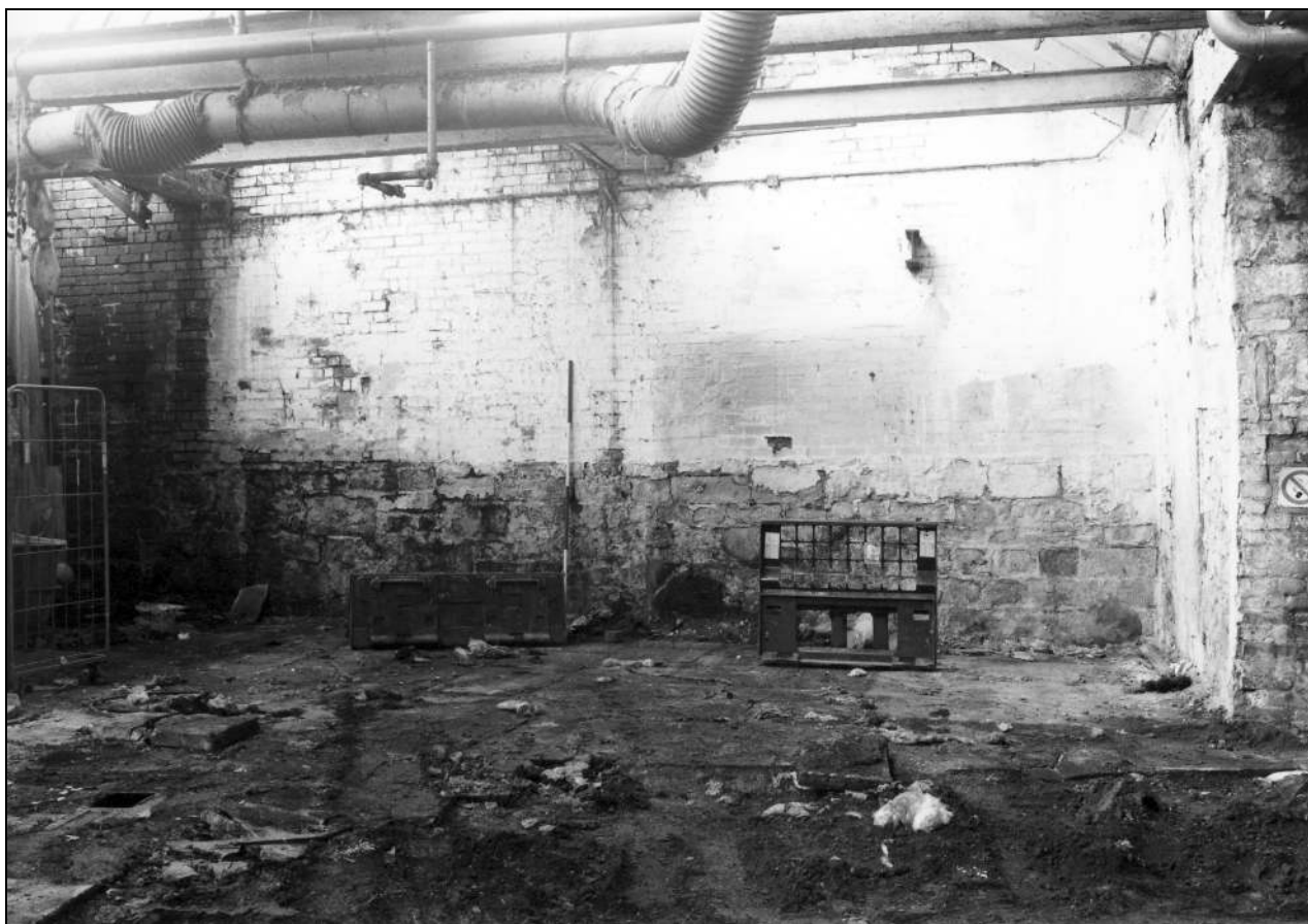
Photo 109: The covered yard: interior view, from the west (film 3, frame 10)
