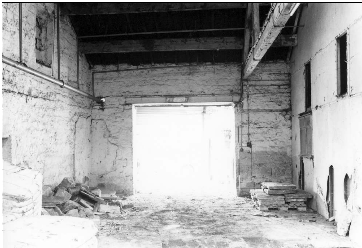
Photo 121: Interior of warehouse, from the north (film 2, frame 17)
