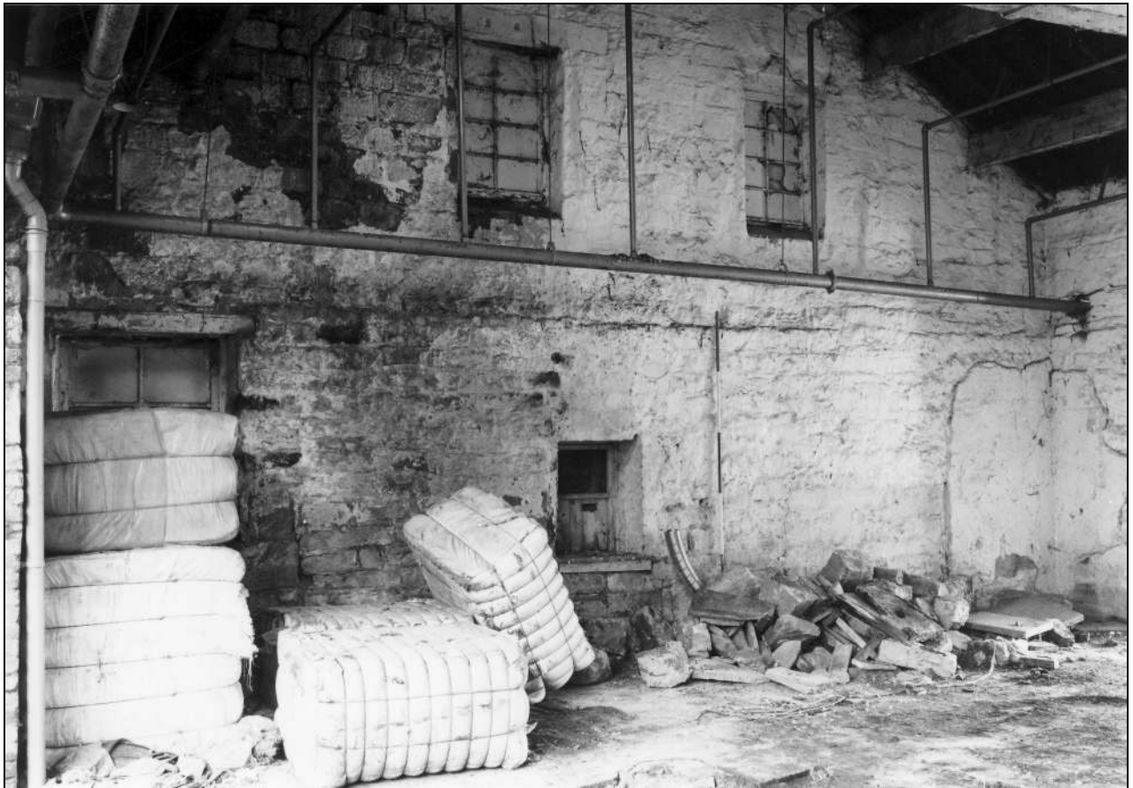
Photo 118: Interior of warehouse, from the north-west (film 2, frame 12)
