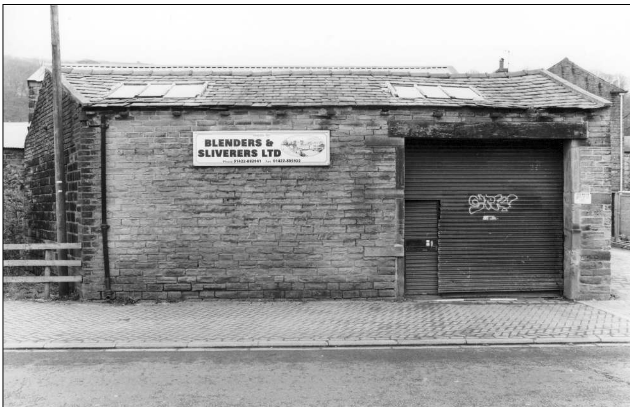
Photo 125: Store fronting Burnley Road, from the south (film 7, frame 16)
