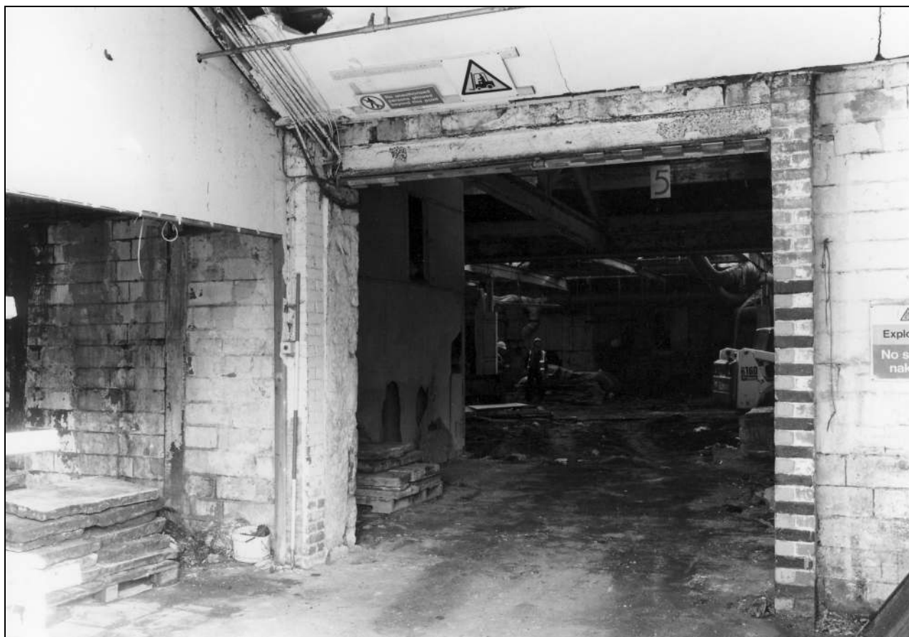
Photo 116: Present south entrance into warehouse, from the south (film 3, frame 5)
