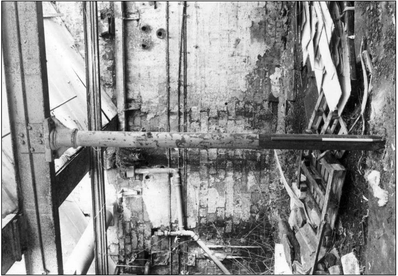
Photo 111: Typical column in covered yard, from the east (film 7, frame 9)
