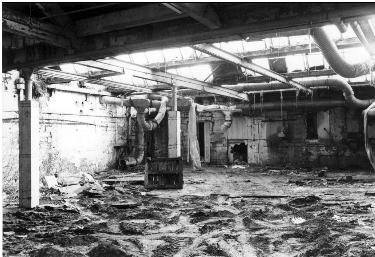
Photo 110: The covered yard: interior view, from the south-east (film 1, frame 18)
