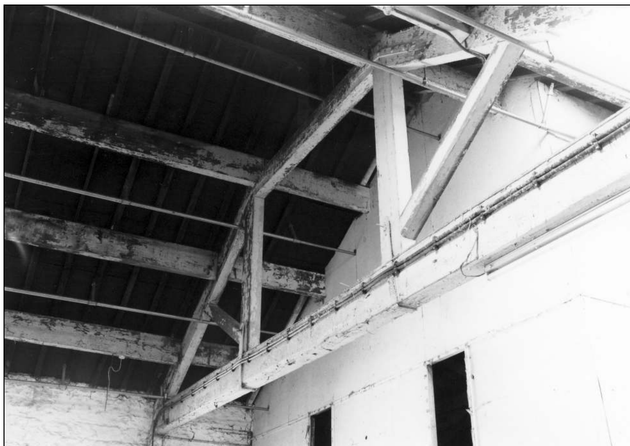
Photo 122: Roof truss in warehouse, from the north-east (film 2, frame 16)
