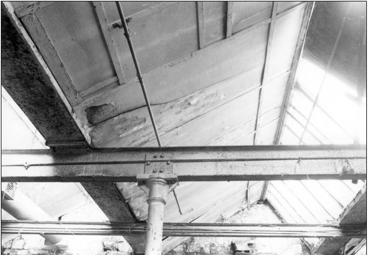
Photo 112: Underside of roof in covered yard, from the east (film 2, frame 6)
