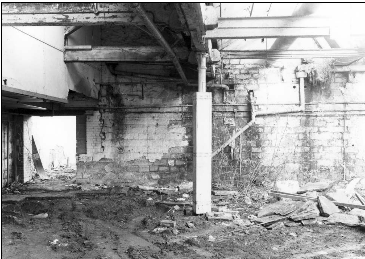
Photo 90: East elevation of weaving shed (south part) (film 2, frame 1)
