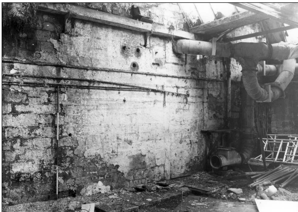
Photo 91: East elevation of weaving shed (central part) (film 2, frame 3)
