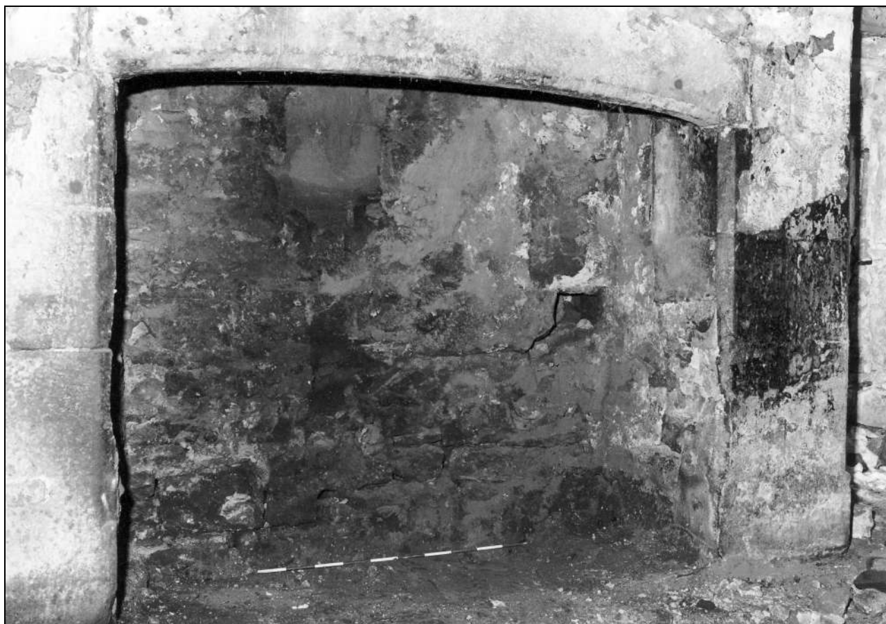
Photo 47: Fireplace in housebody, following removal of range (film 7, frame 11)
