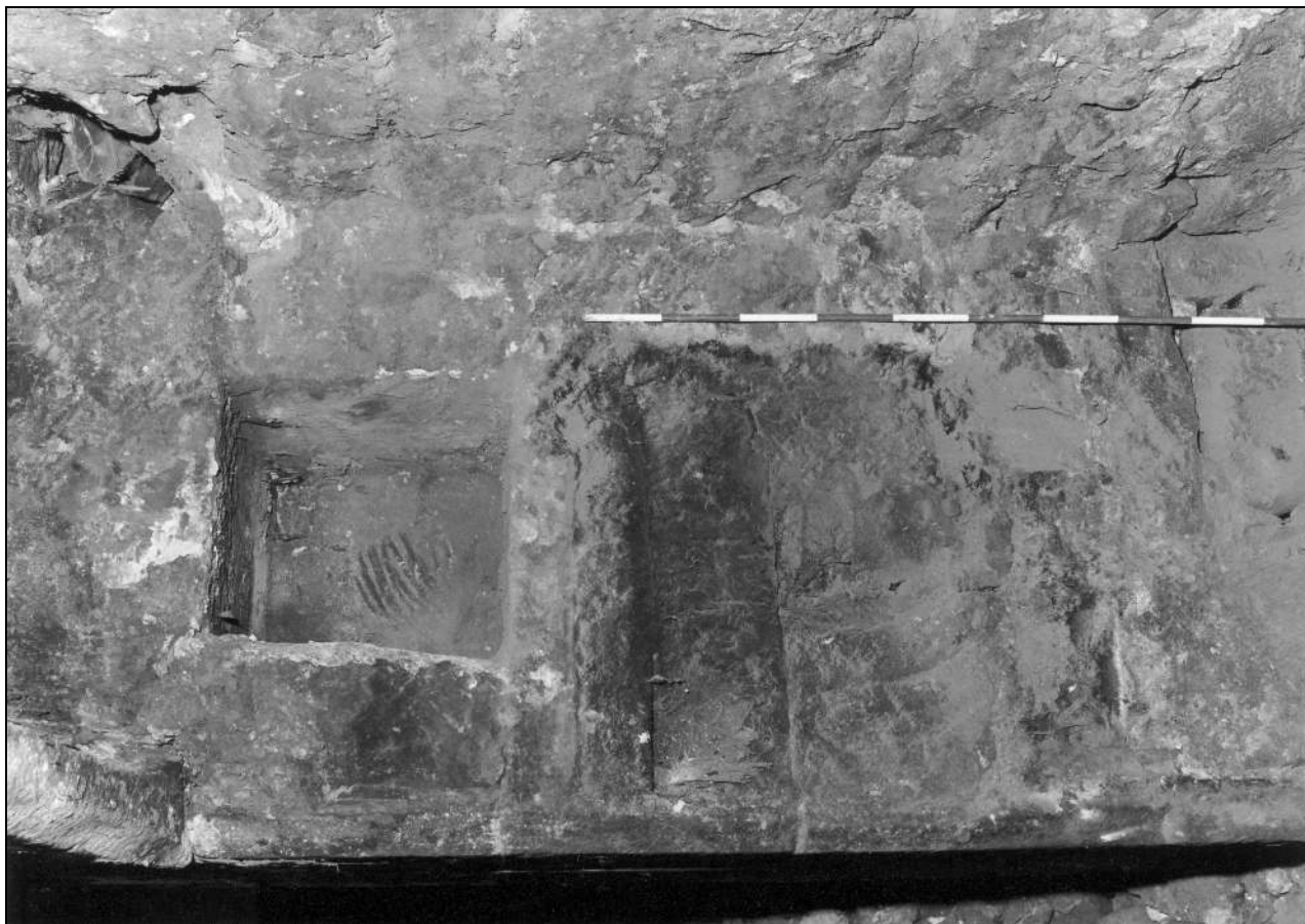
Photo 49: Fireplace in housebody, following removal of range: detail of recess in south side (film 7, frame 15)
