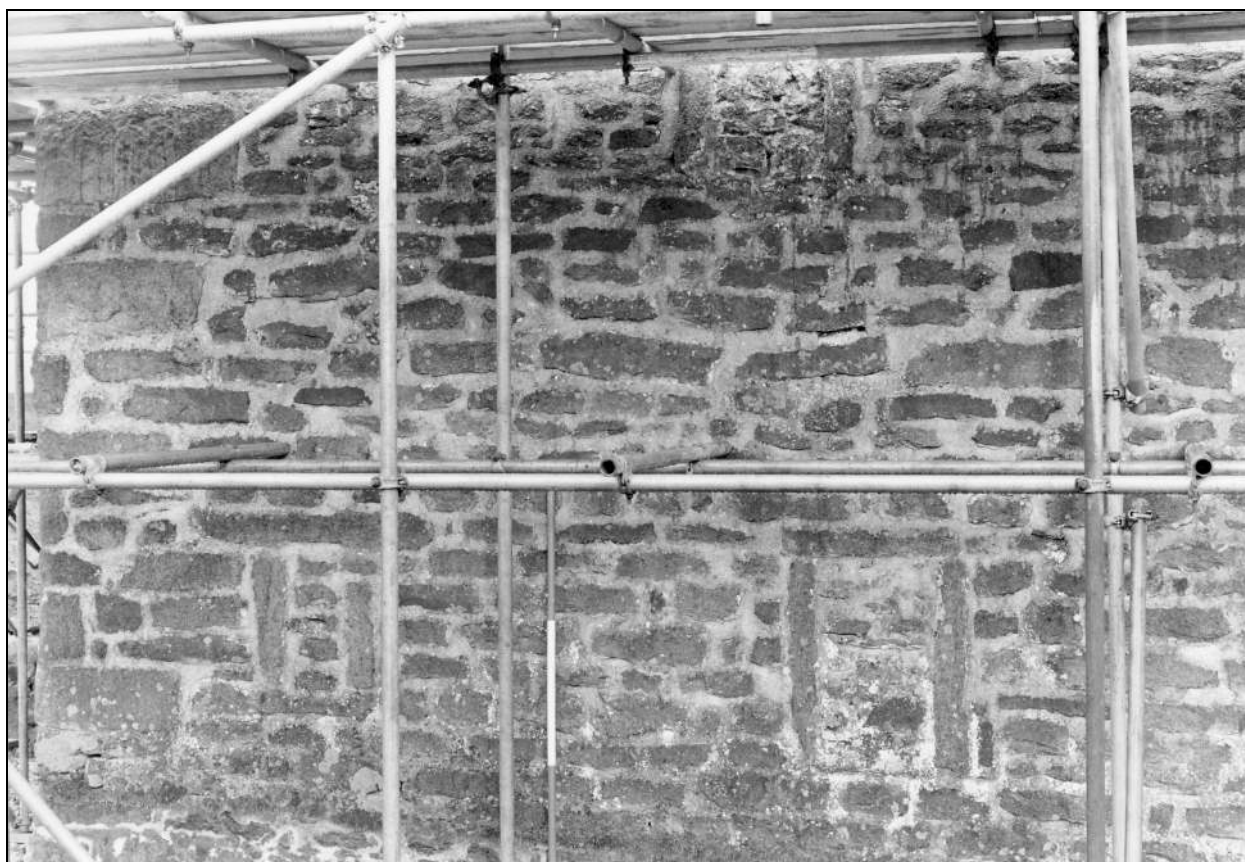
Photo 11: Blocked windows in lower part of west gable to house (film 7, frame 4)
