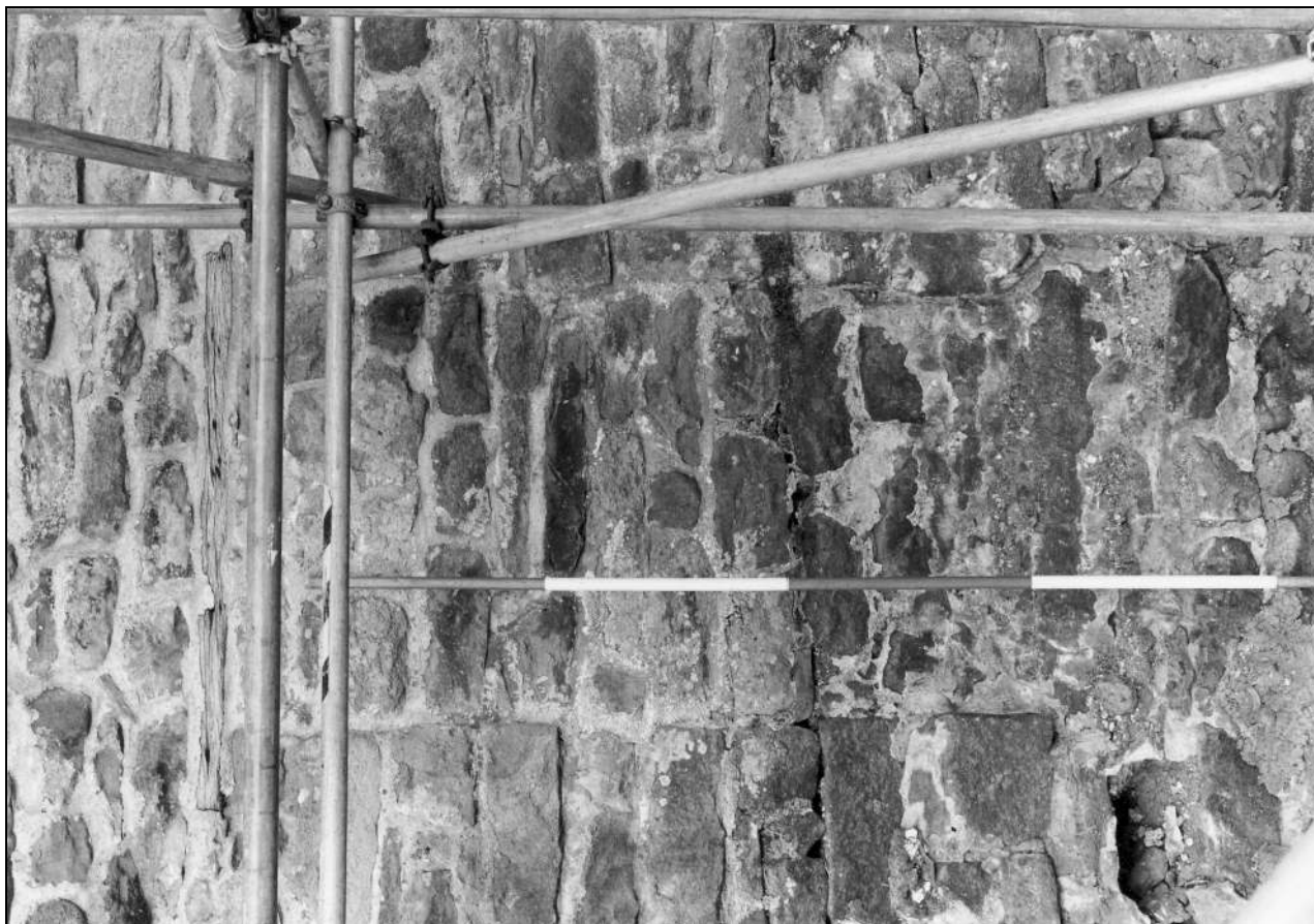
Photo 27: Blocked doorway in north wall of barn (film 7, frame 2)
