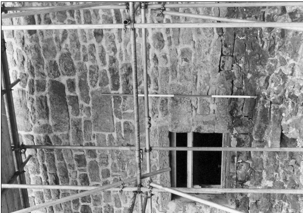
Photo 31: Straight joint in north wall of barn (film 7, frame 1)
