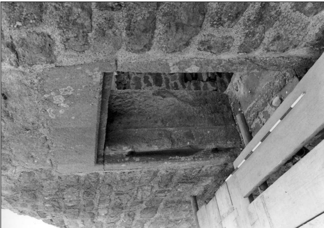
Photo 30: Detail of forking hole with rebate for shutter, east gable of barn (film 5, frame 1)
