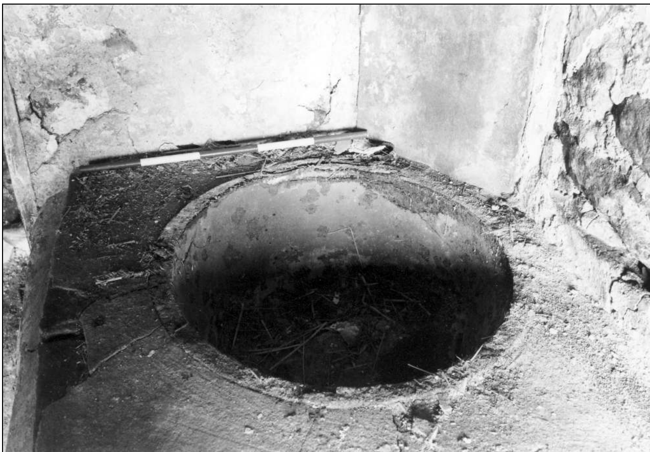
Photo 58: Detail of set pot in former parlour (film 3, frame 17)
