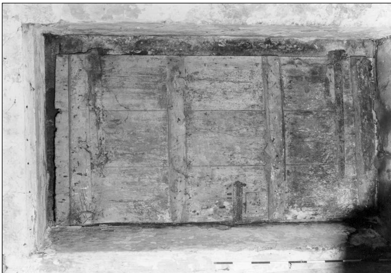
Photo 55: Detail of chamfer and stop to beam over housebody (film 1, frame 16)
