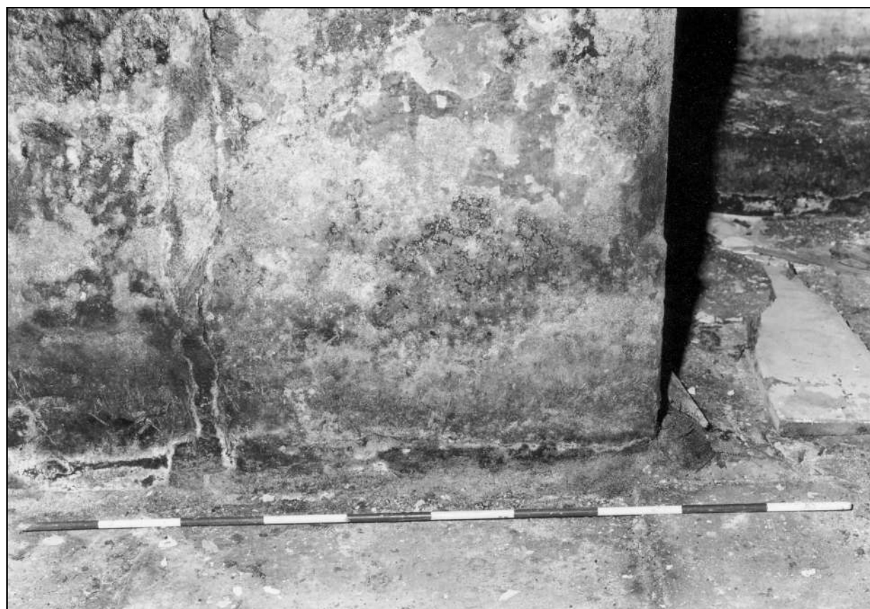
Photo 41: Detail of chamfer to fireplace jamb in housebody (film 4, frame 13)
