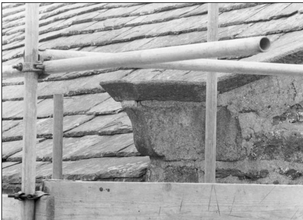
Photo 10: Detail of kneeler at north-west corner of house, while scaffolded (film 5, frame 13)
