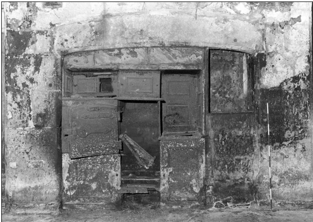
Photo 42: Detail of housebody fireplace and range (film 1, frame 13)
