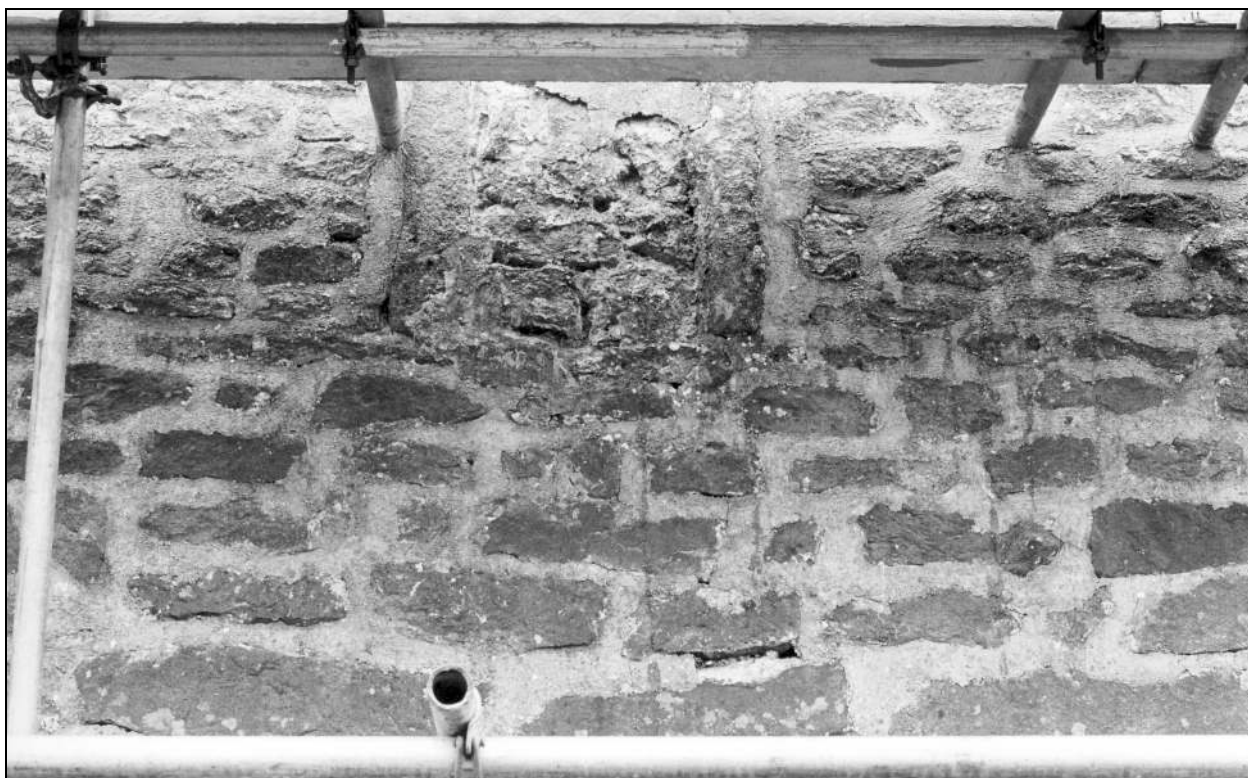
Photo 12: Blocked window in upper part of west gable to house (film 7, frame 5)
