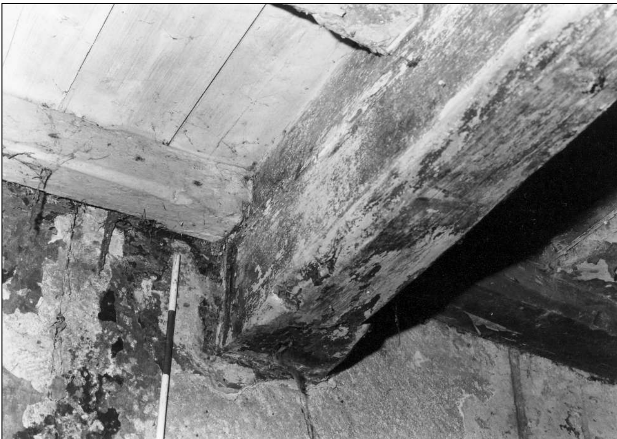
Photo 55: Detail of chamfer and stop to beam over housebody (film 1, frame 16)
