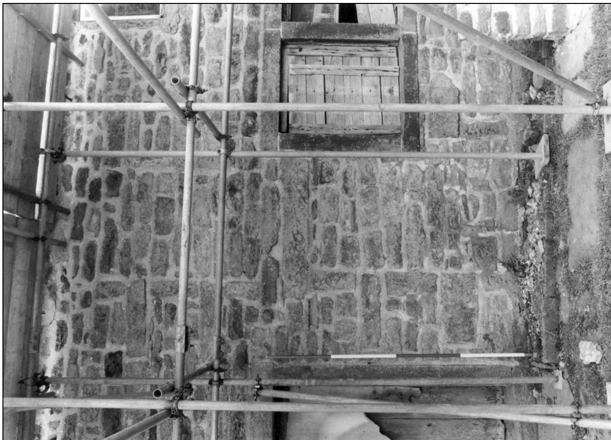
Photo 6: Detail of blocked ground and first floor doorways, front elevation of house, while scaffolded (film 5, frame 6)
