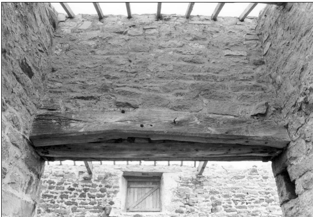
Photo 88: Lintel for barn doors within entry, from the south, while scaffolded (film 6, frame 5)
