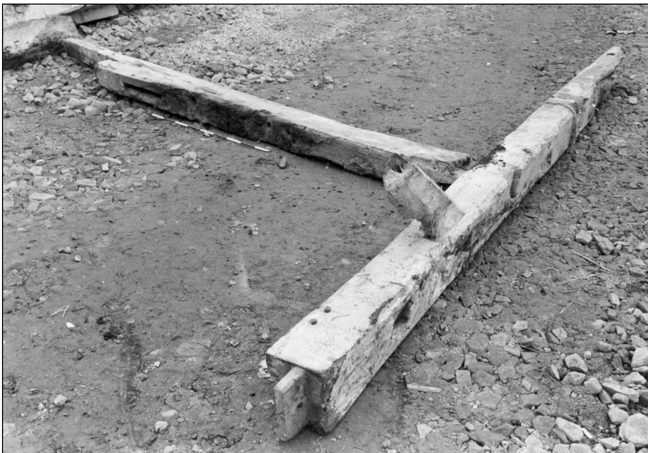
Photo 96: Remains of arcade post and tie, removed from barn (film 6, frame 18)
