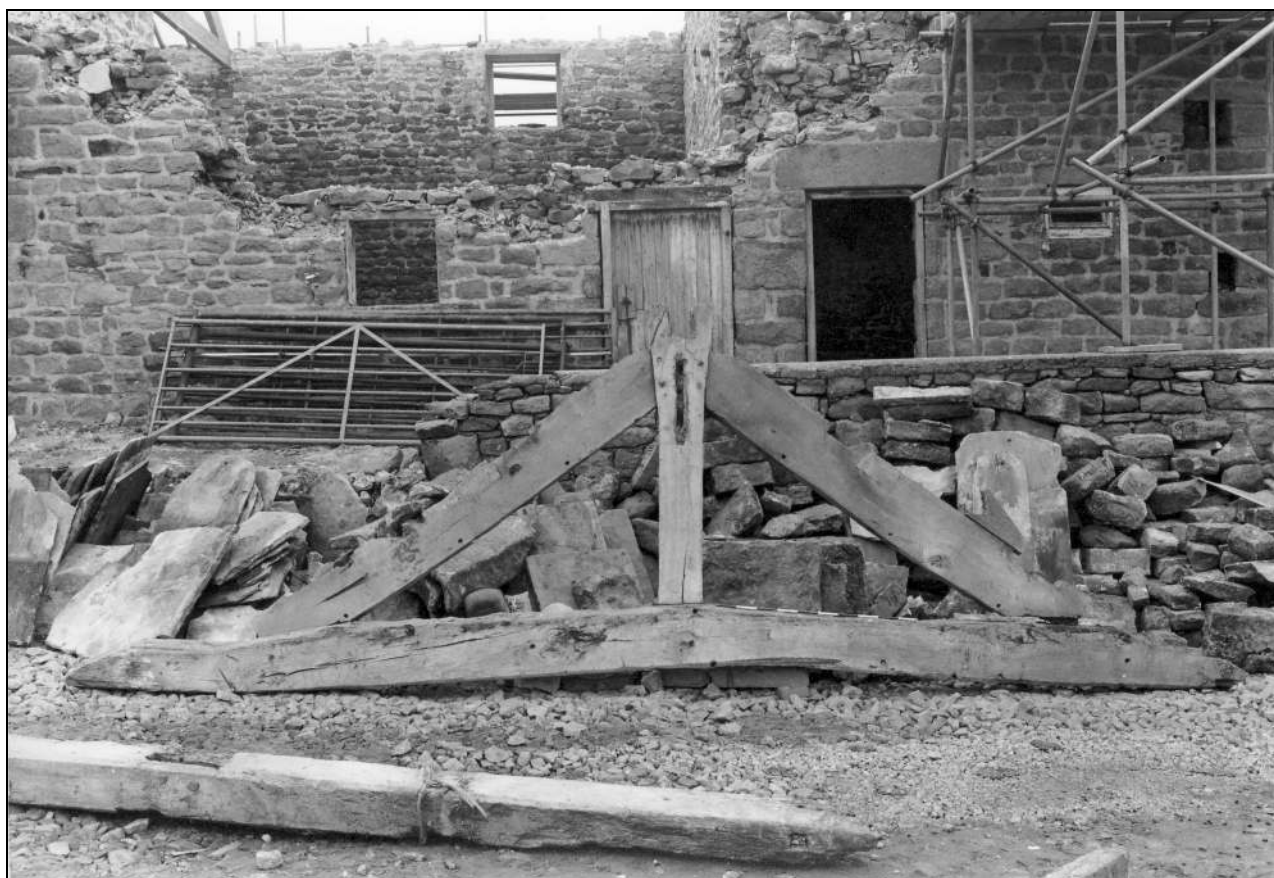
Photo 102: Roof truss removed from barn (film 6, frame 15)
