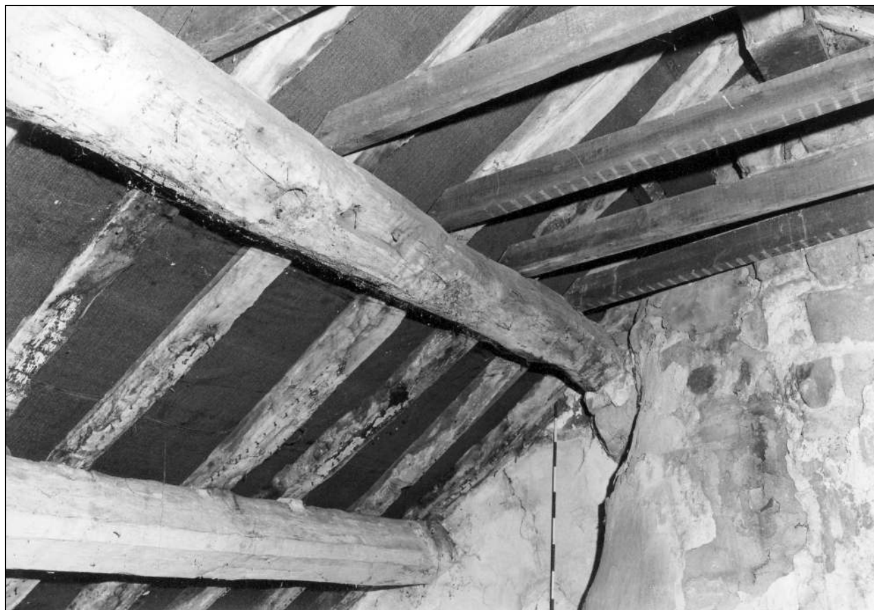
Photo 84: Timber re-used as purlin over east chamber, from the east (film 3, frame 1)
