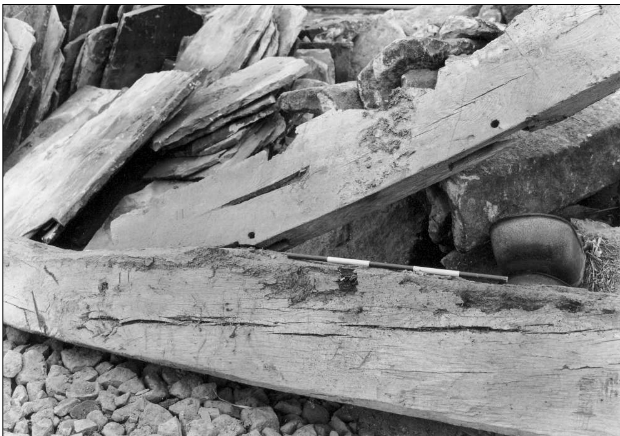
Photo 103: Detail of roof truss removed from barn (film 6, frame 16)
