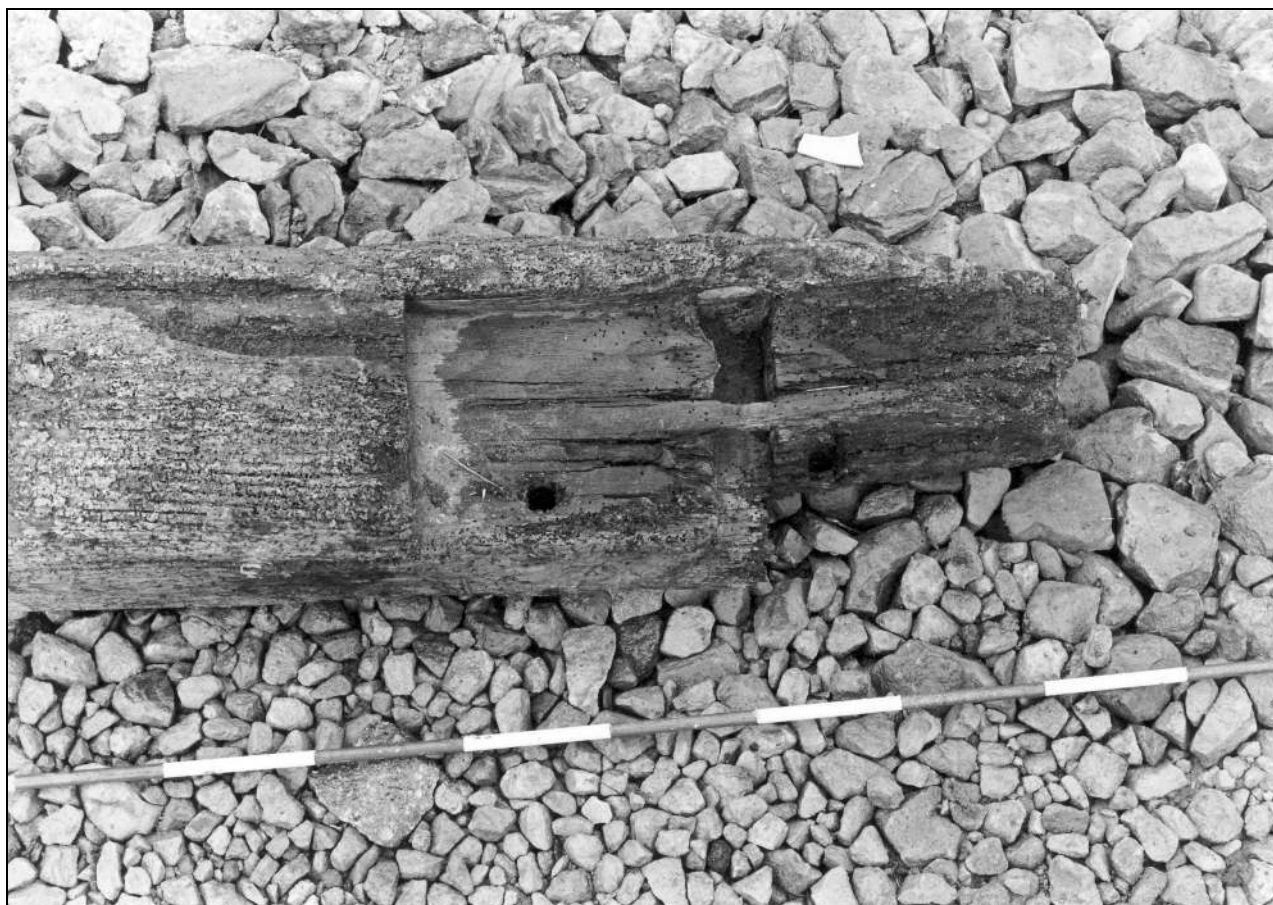
Photo 99: Detail of foot of arcade post, removed from barn (film 7, frame 7)
