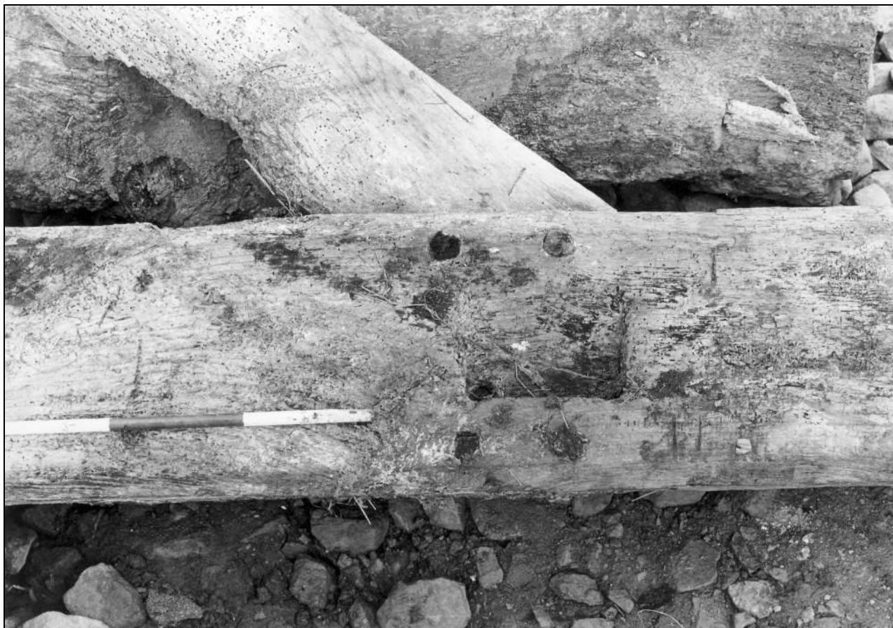
Photo 101: Detail of joint of arcade post and brace, removed from barn (film 7, frame 9)
