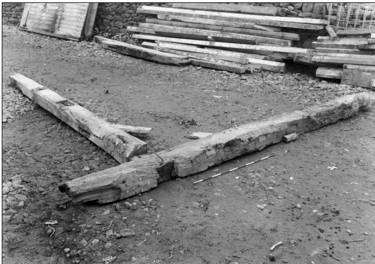
Photo 97: Remains of arcade post and tie, removed from barn (film 6, frame 17)
