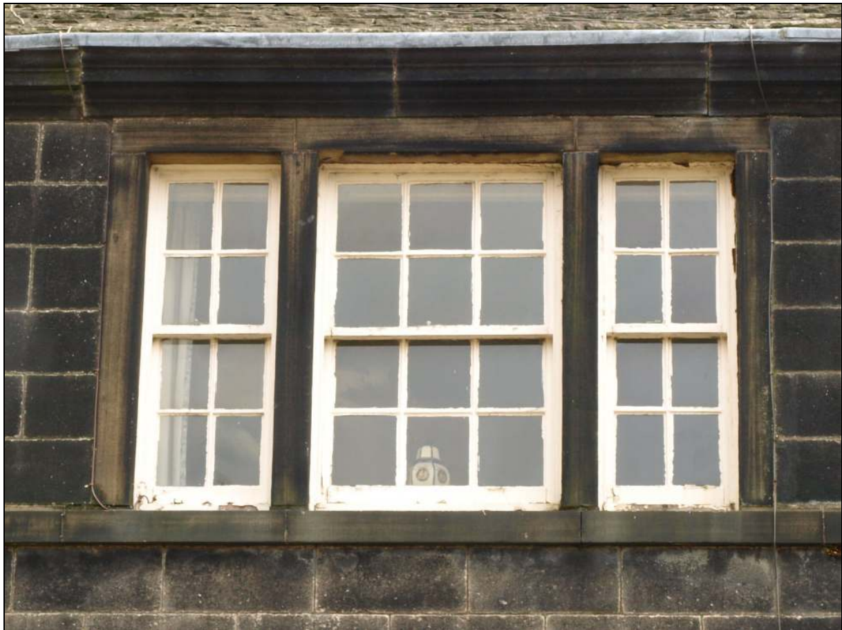
Photo 9: Detail of window with original sashes in front elevation (first floor, north window)
