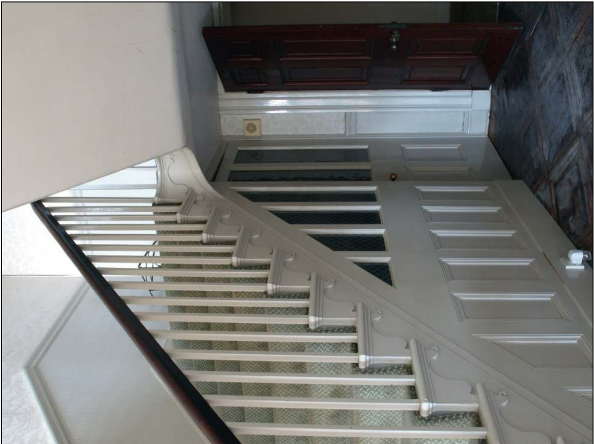
Photo 20: Detail of stair string, with later partition beneath
