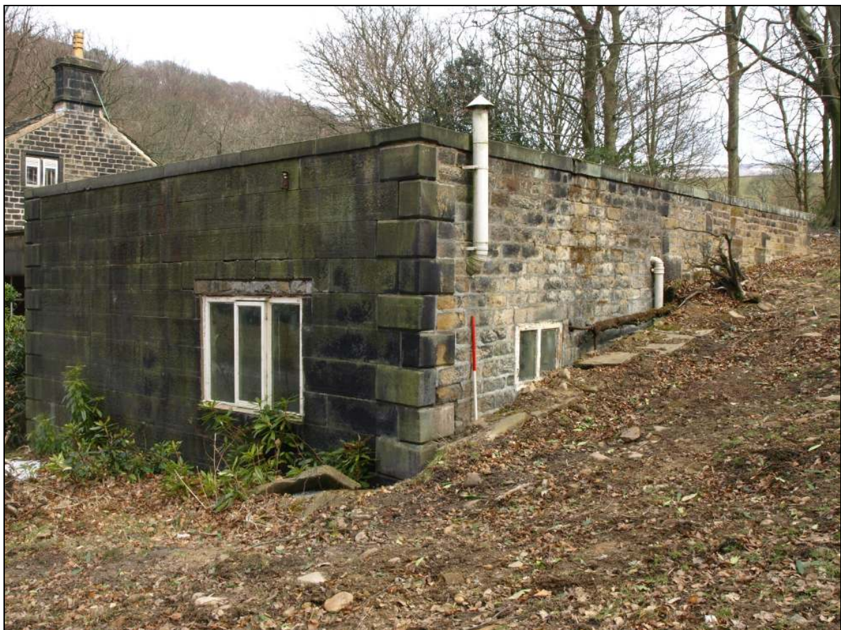
Photo 52: The south end of the service wing, from the south-west
