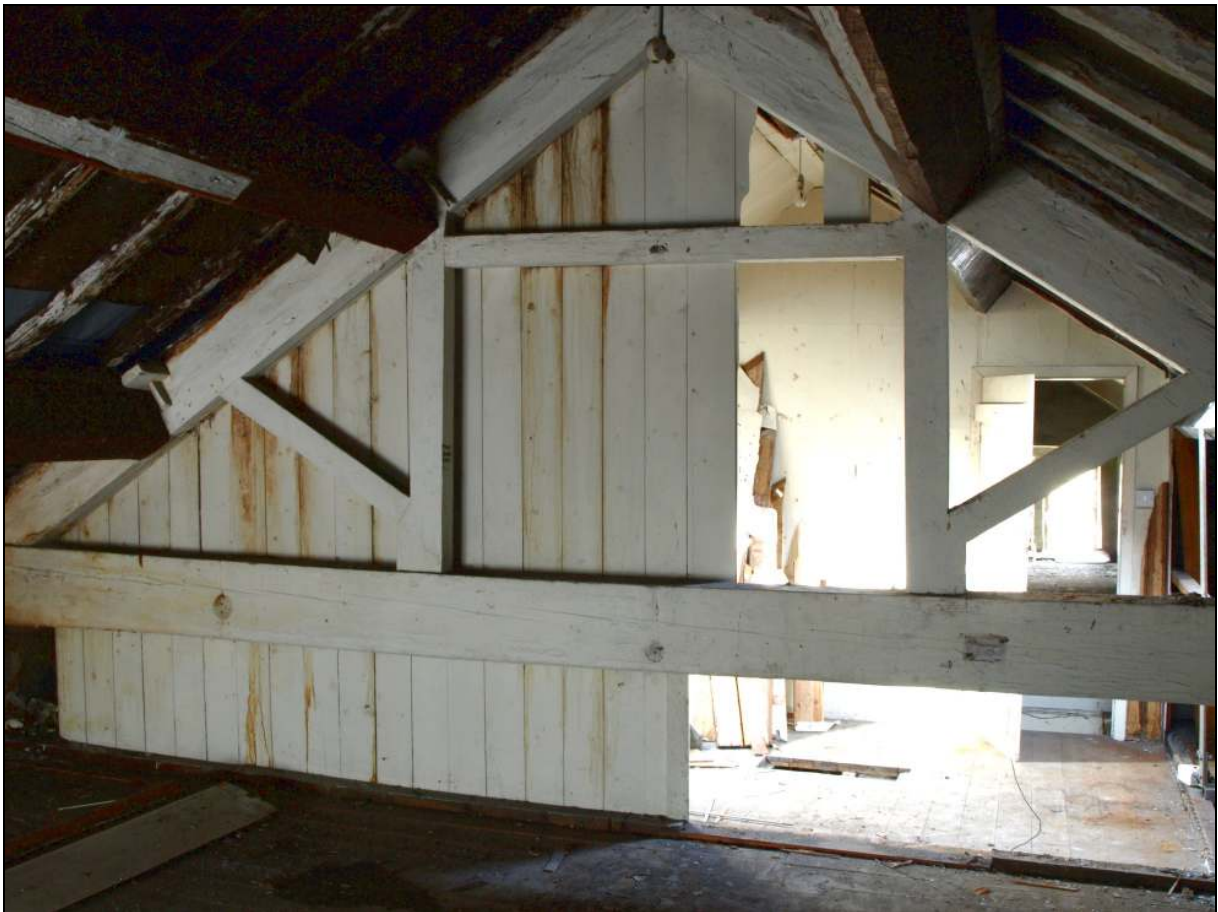
Photo 41: The south roof truss in rear range
