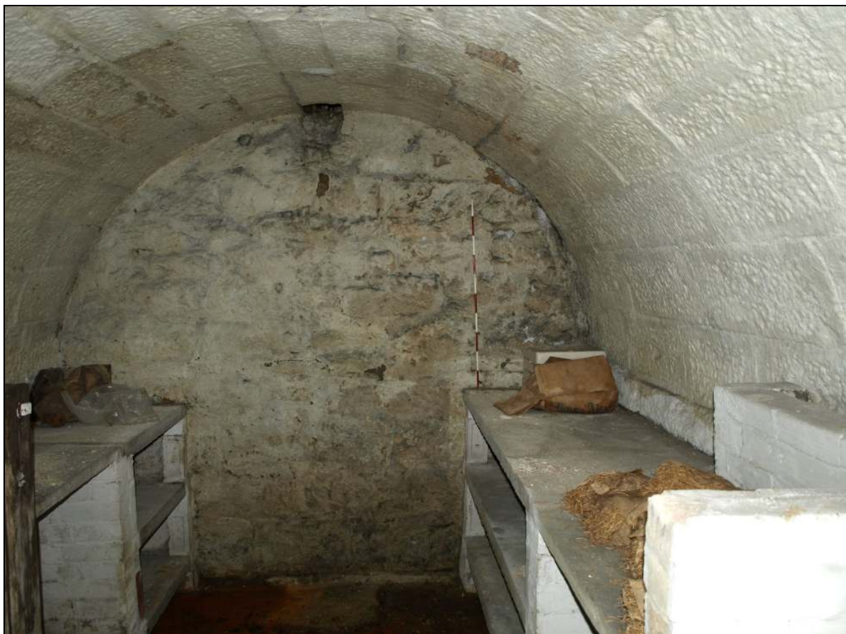
Photo 55: The vaulted room in the south part of the service wing
