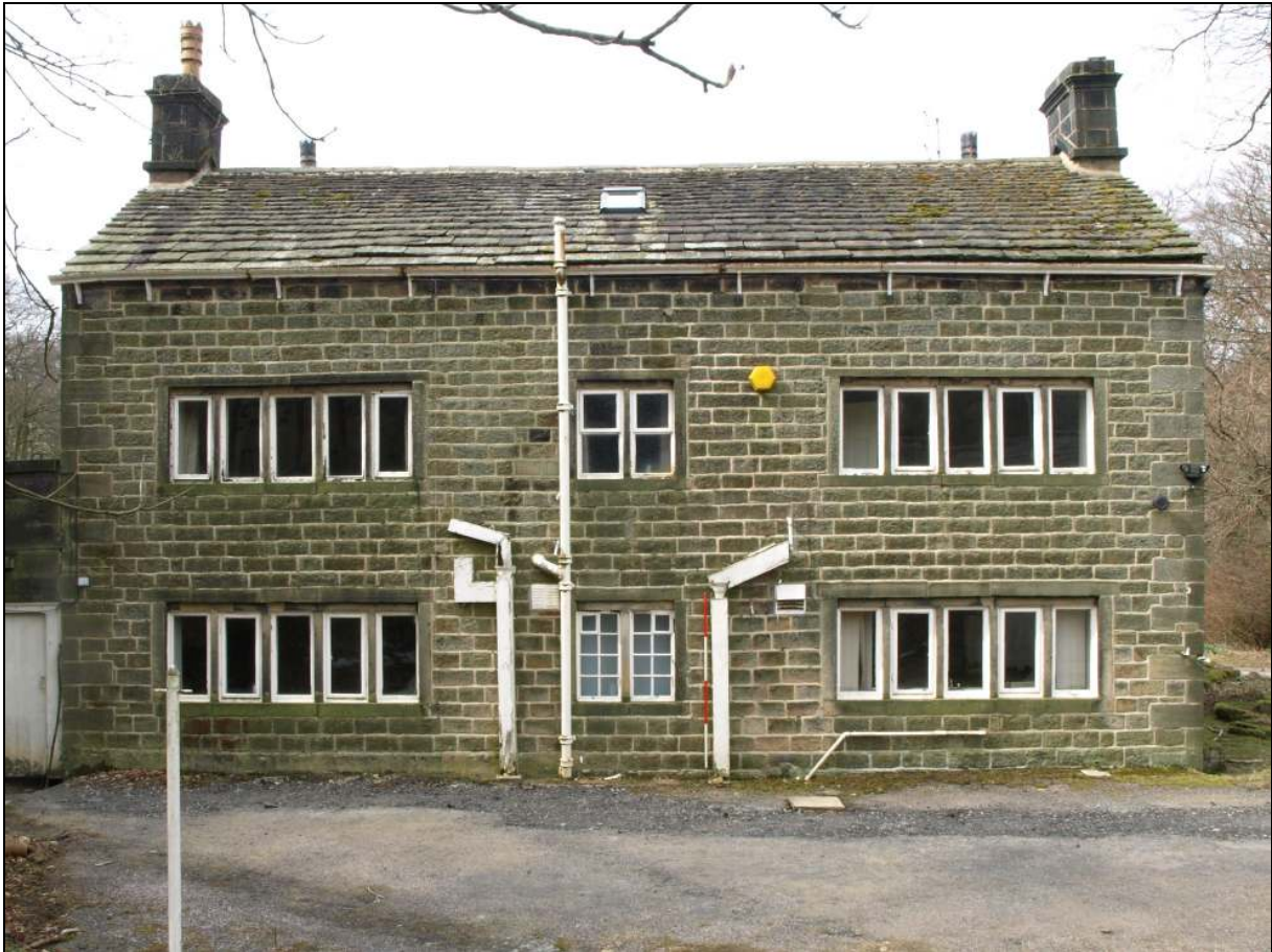
Photo 6: The rear elevation
