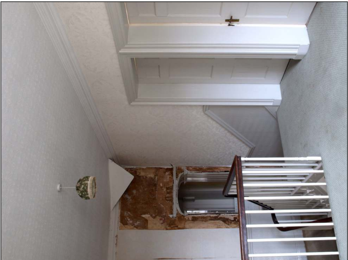
Photo 32: Landing on first floor, front range, from the north-west
