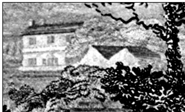
Figure 7: Print from mid nineteenth century, showing the house from the south-west, beyond the mill. This seems to show the original roof over the service wing. Reproduced by courtesy of Saddleworth Museum Archives.
