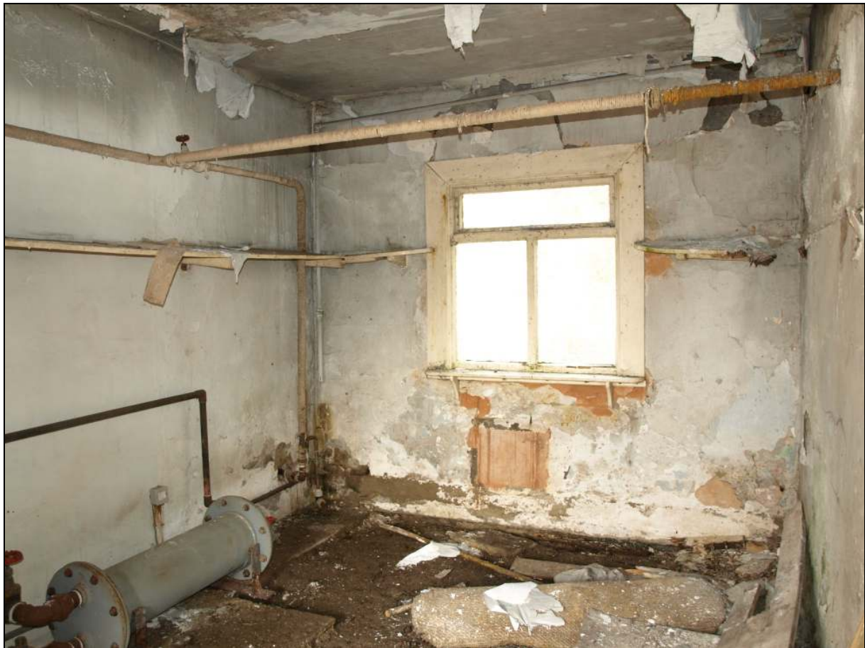
Photo 51: One of the four store rooms in the north arm of the service wing
