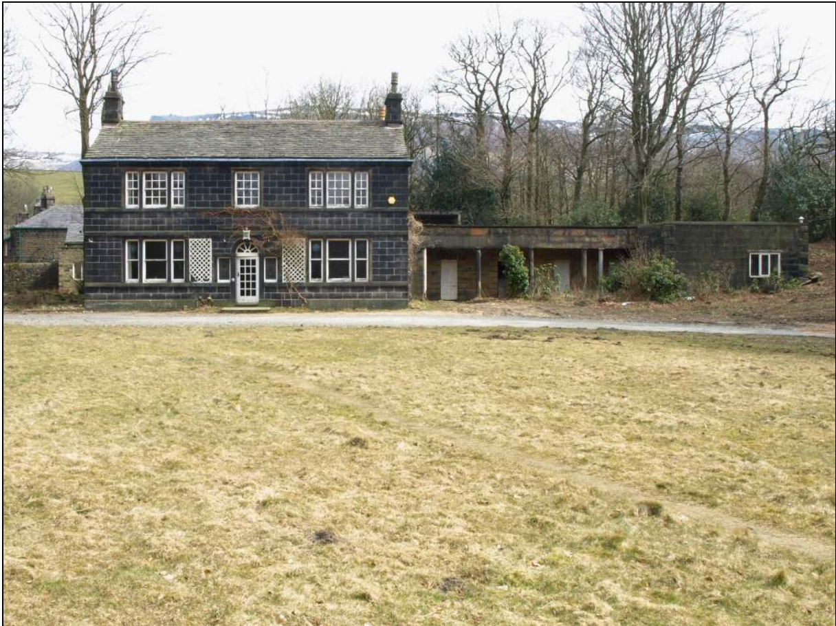
Photo 1: General view of the house and service wing, from the west
