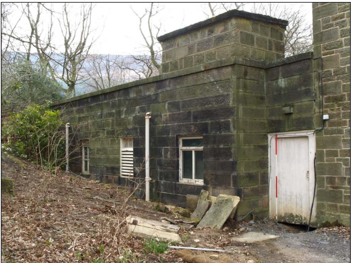
Photo 49: East side of the service wing, from the north-east
