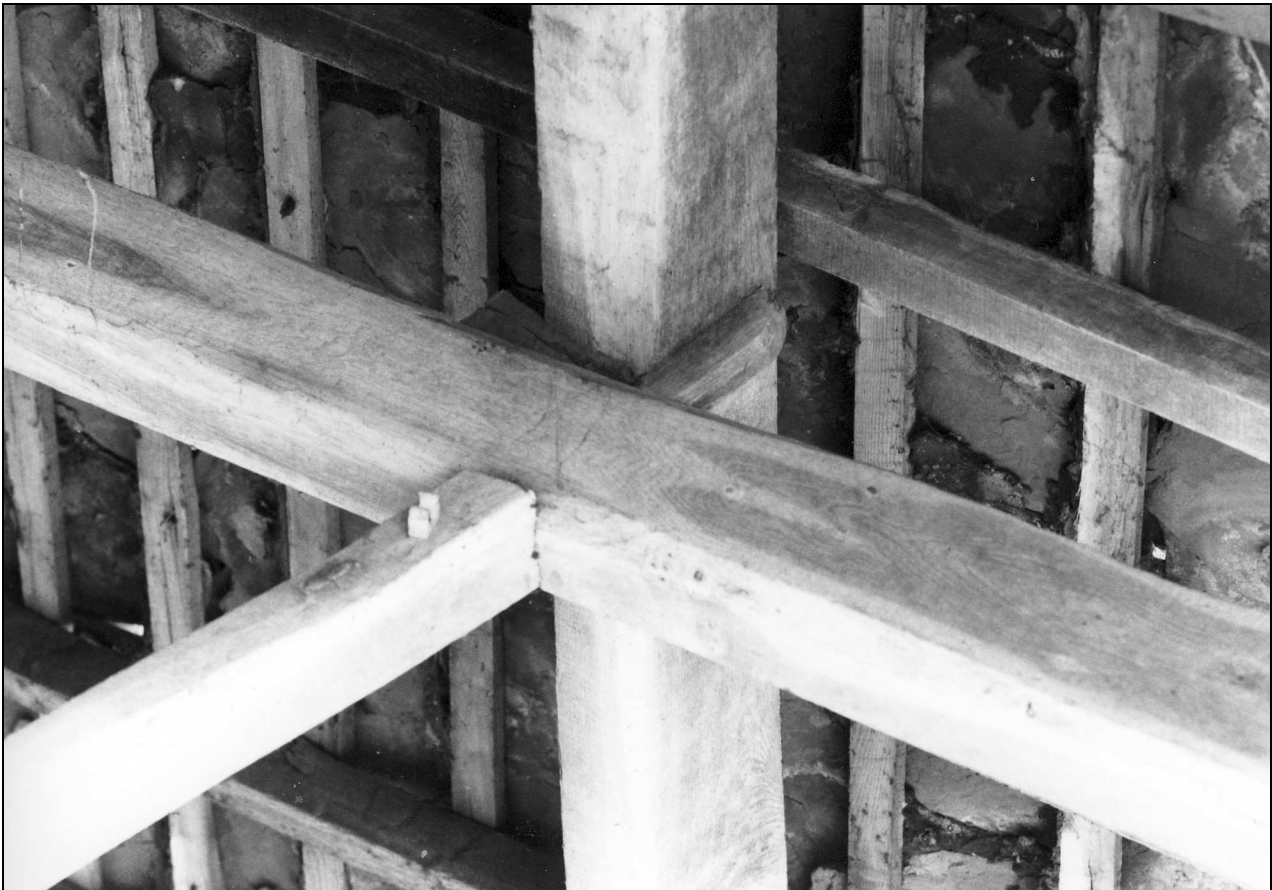
Photo 24: Detail of parge peg holding purlin in place, from the west
