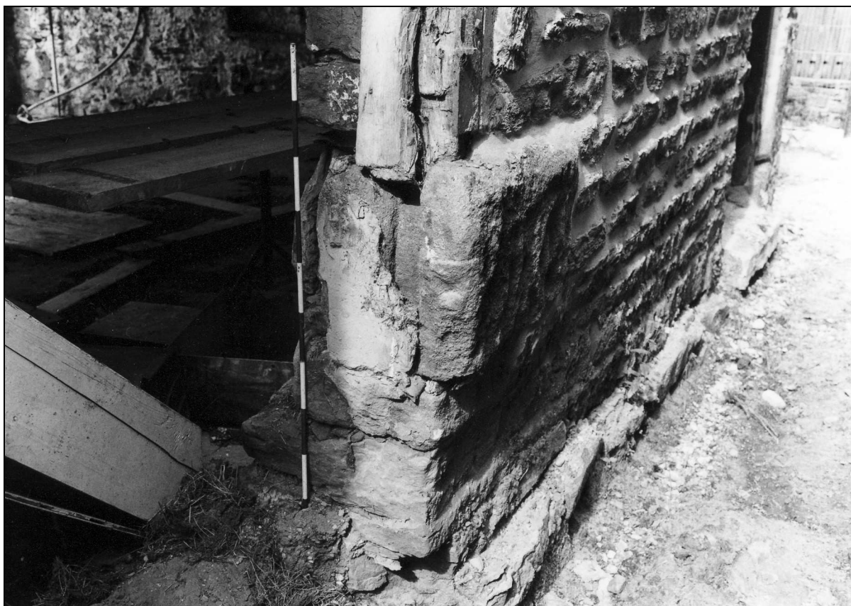
Photo 5: Detail of slot in jamb of cart entrance, for vertical board (or "lift")
