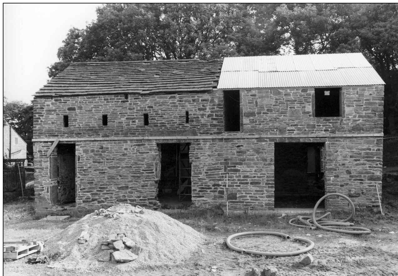
Photo 12: The south-west elevation
