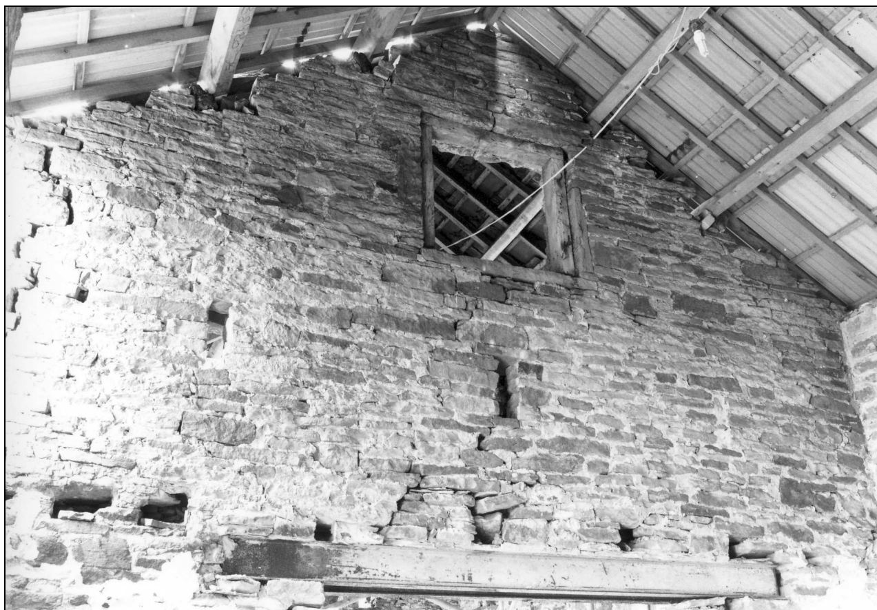
Photo 11: South-east gable of original barn, showing forking hole, now facing into later addition
