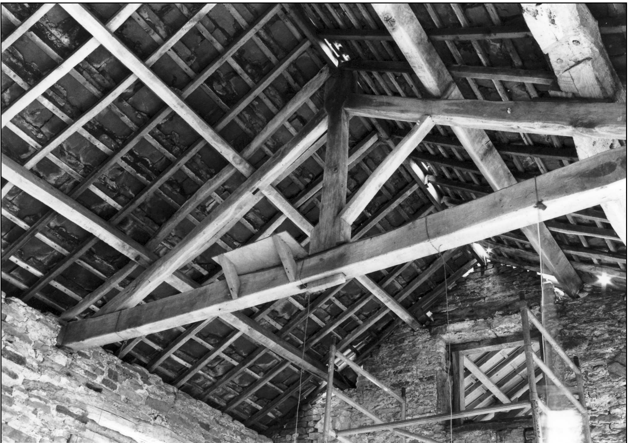
Photo 23: Roof truss over barn, from the west
