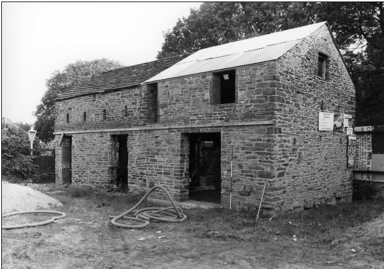
Photo 26: The barn, from the south
