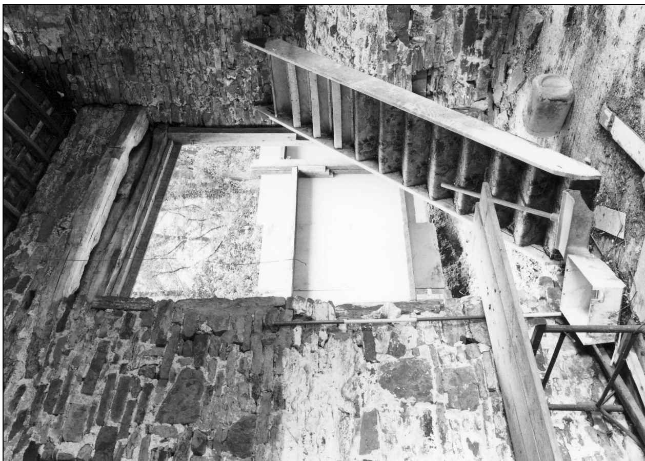
Photo 5: Detail of slot in jamb of cart entrance, for vertical board (or "lift")
