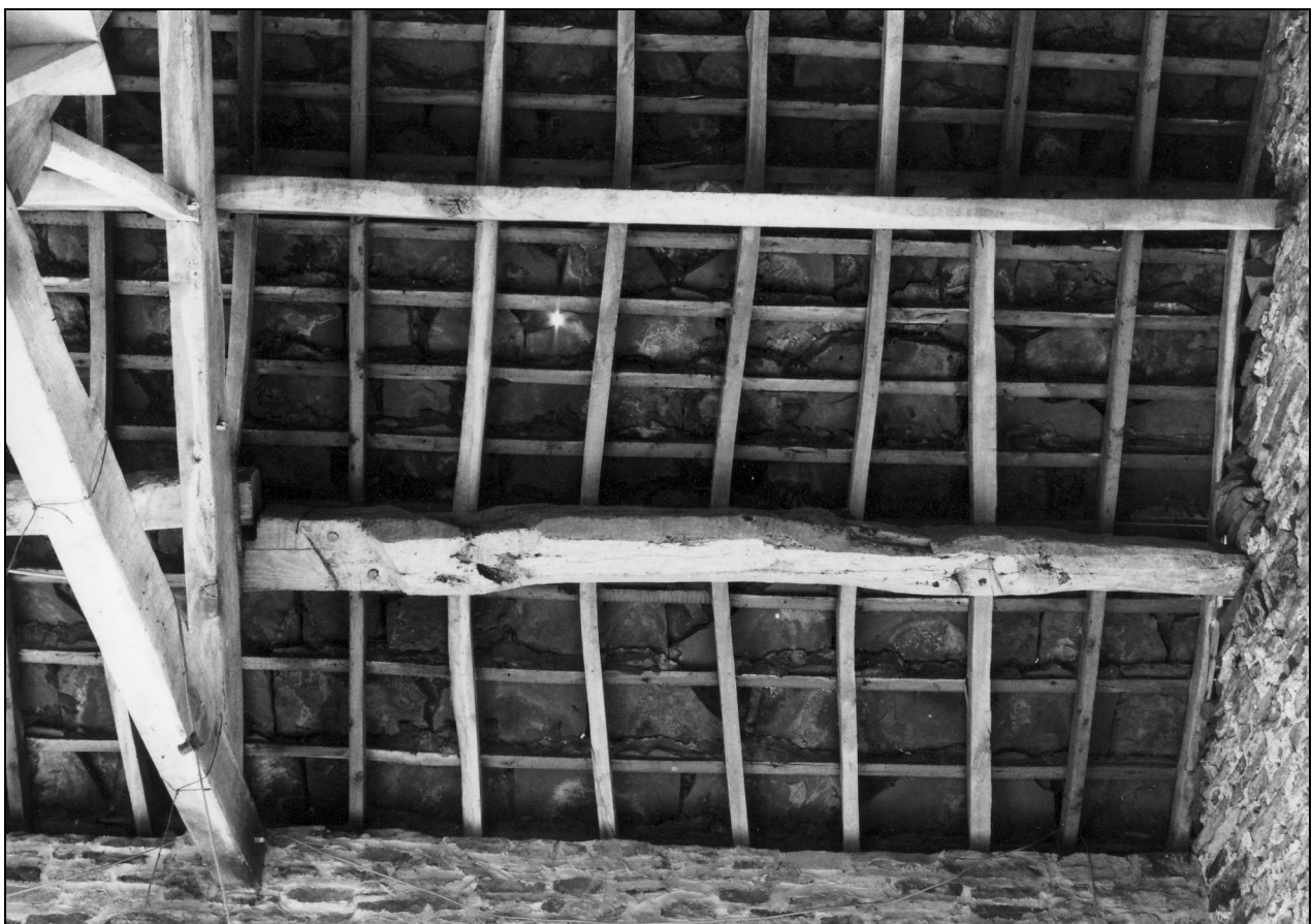
Photo 25: Former cruck blade re-used as purlin, south-west roof pitch
