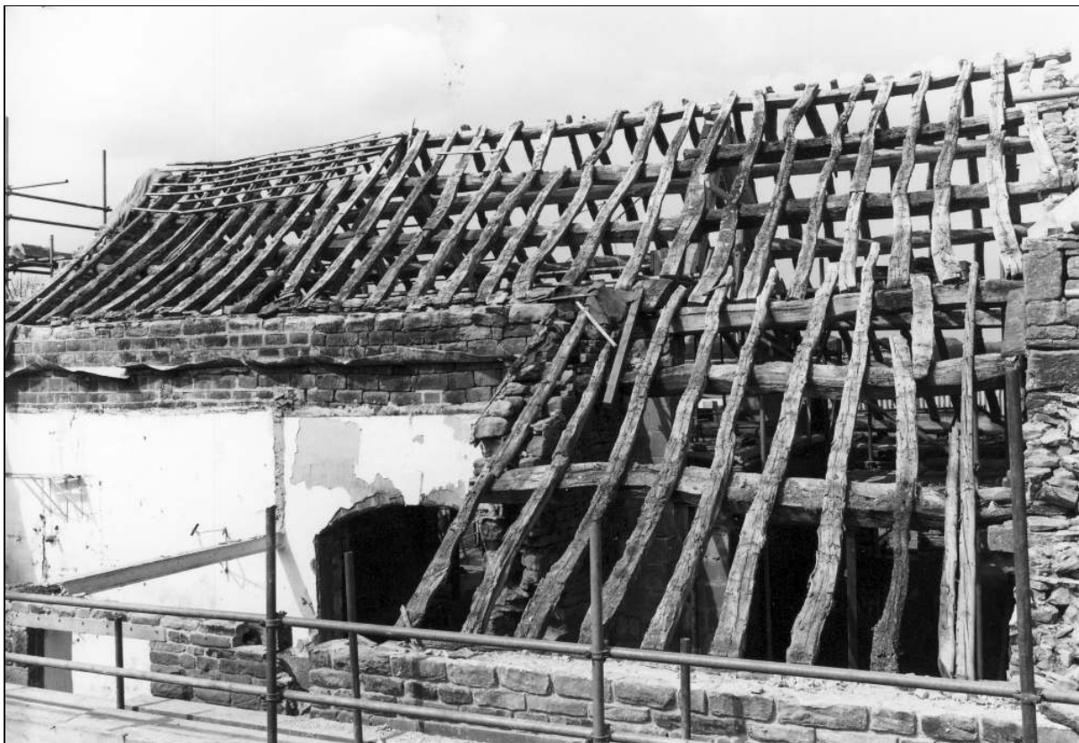
Photo 76: Barn roof, during conversion works, from the south-east (film 6, frame 7)
