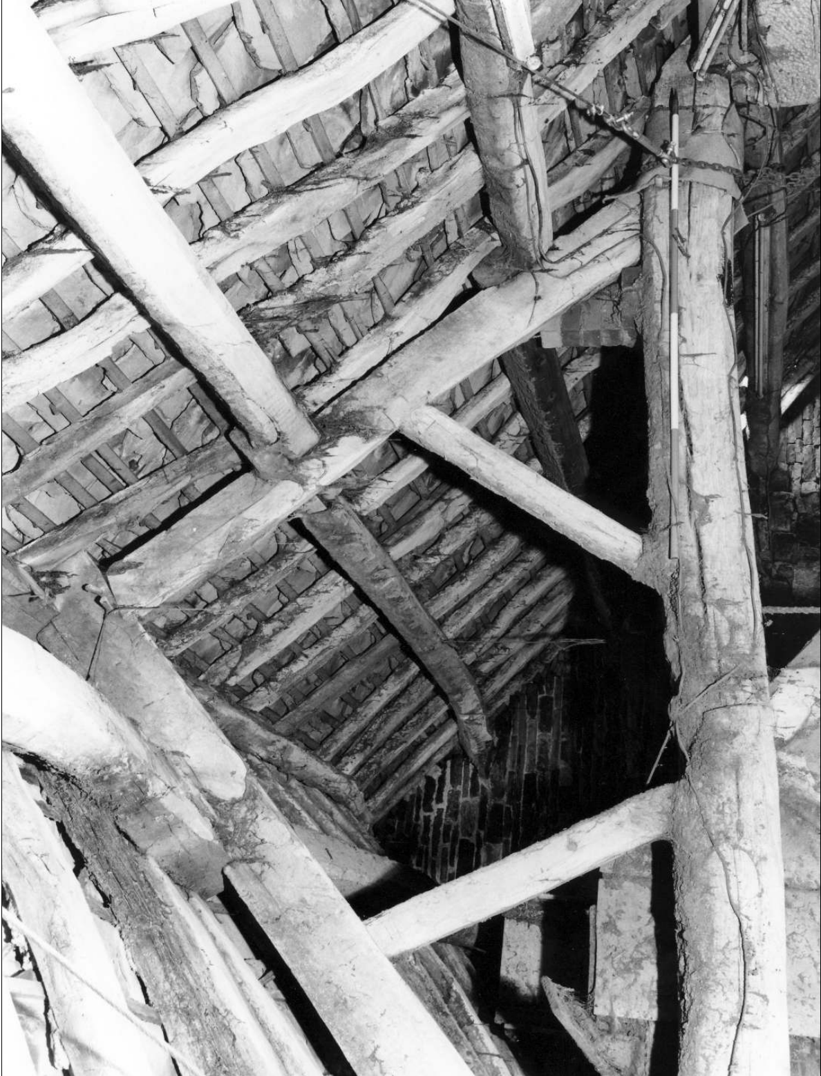
Photo 83: Barn interior: south-west roof truss, from the east (film 5, frame 13)
