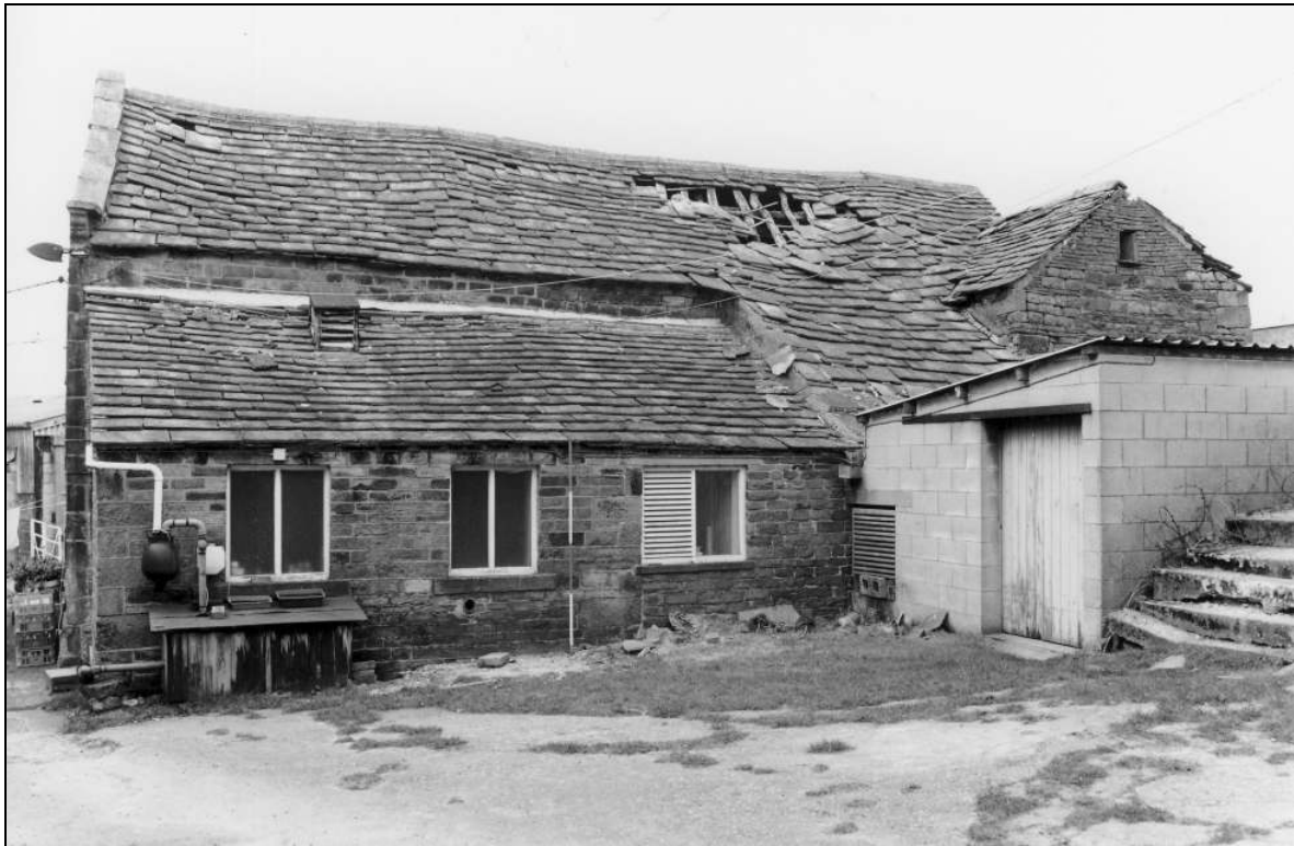
Photo 4: General view of the barn, from the south (film 1, frame 1)
