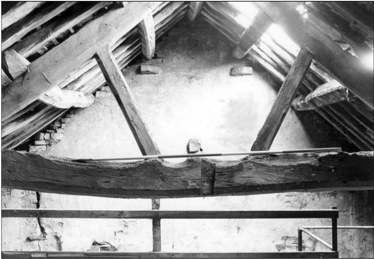
Photo 79: Barn interior: north-east roof truss, from the south-west (film 5, frame 6)
