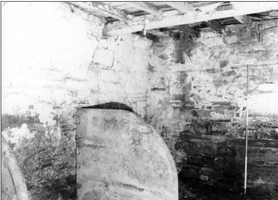
Photo 21: Early wing: interior, from the east (film 3, frame 10)
