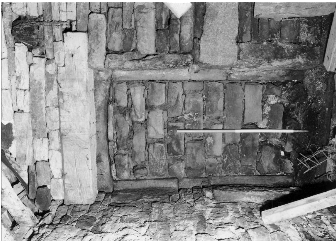
Photo 71: Barn interior: stone base for boskin, east outshut (film 5, frame 3)
