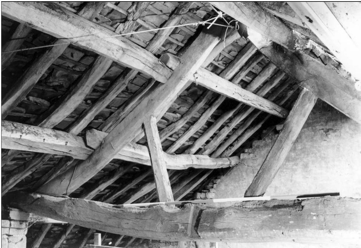
Photo 78: Barn interior: north-east roof truss, from the south (film 5, frame 7)
