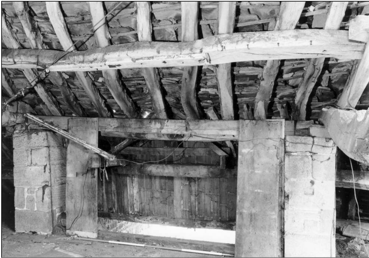
Photo 77: Barn interior: view towards north-west entry, at roof level (film 5, frame 12)
