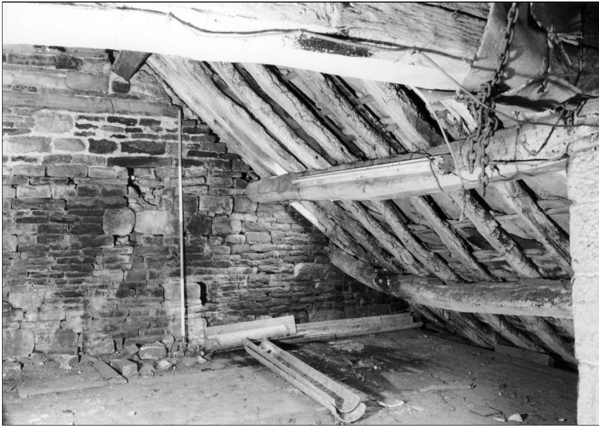
Photo 88: Barn interior: roof over west shippon, from the east (film 5, frame 18)
