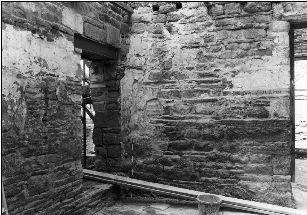
Photo 26: Stable: interior, from the east, during building works (film 6, frame 15)
