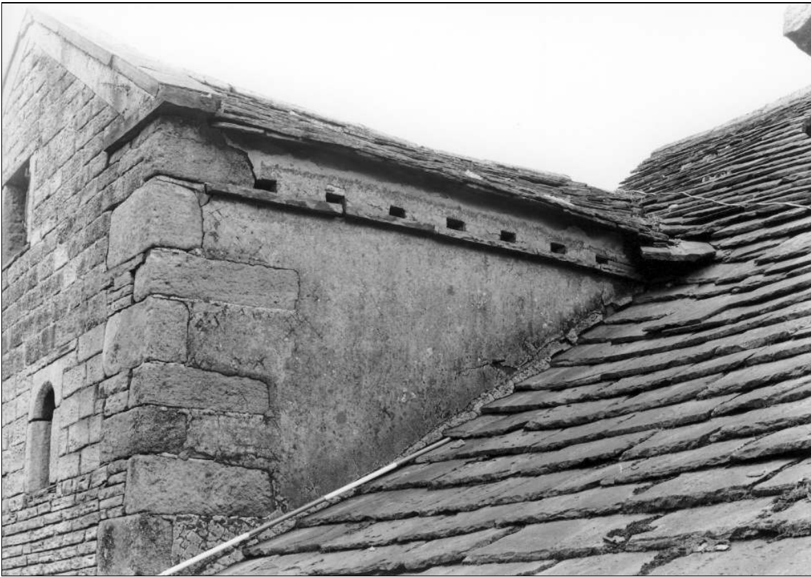
Photo 41: South-west side of the stable: detail of eaves (film 2, frame 3)
