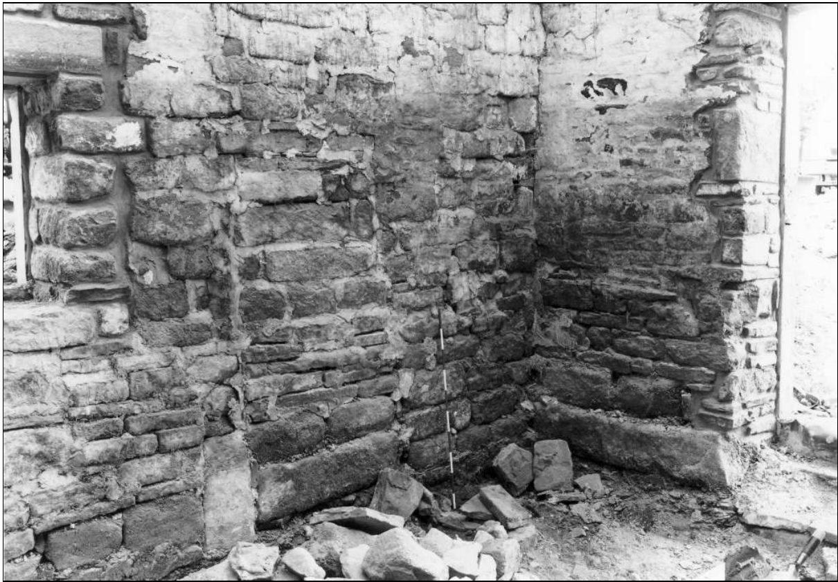
Photo 25: Stable: interior, from the west, during building works (film 6, frame 16)
