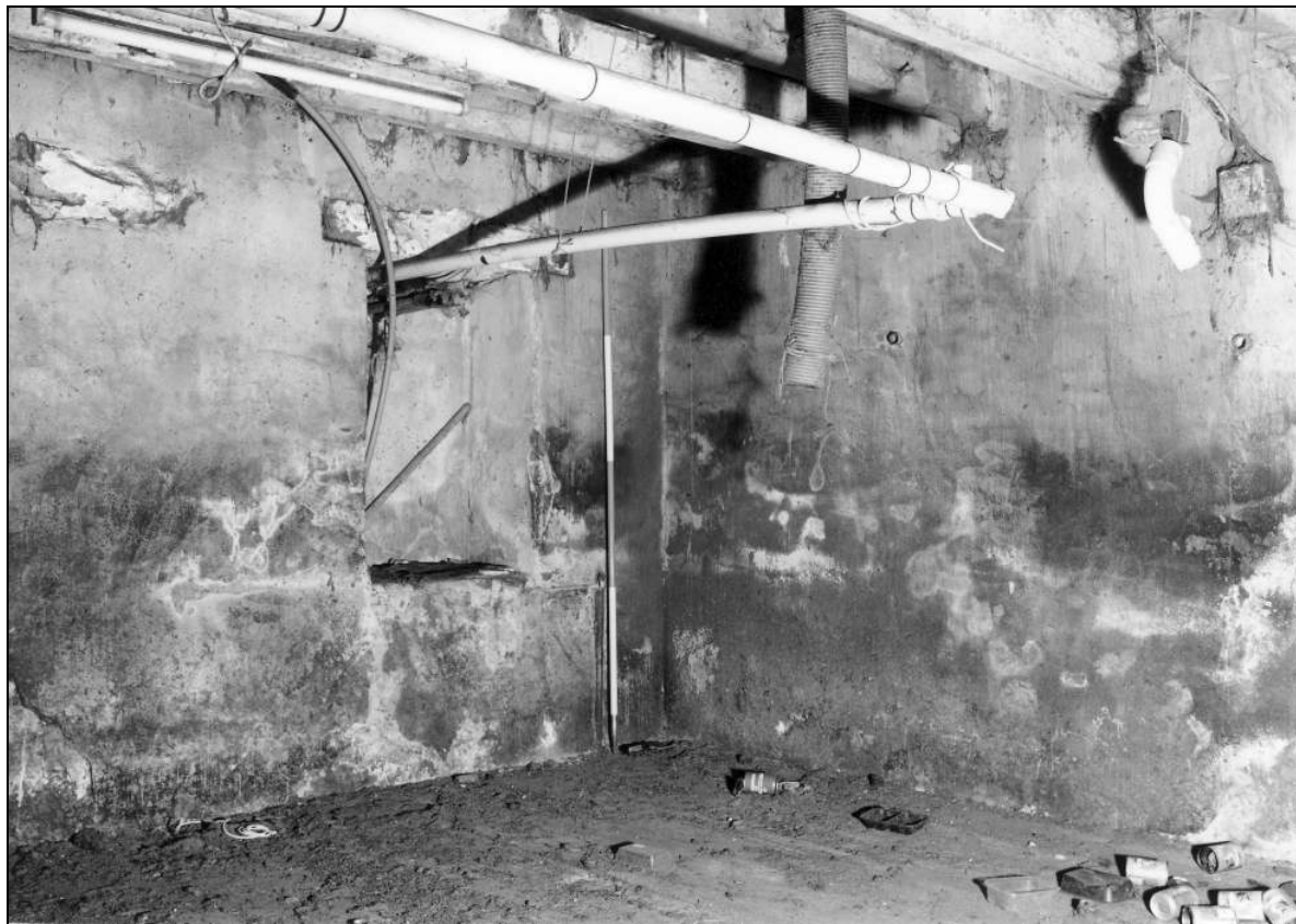
Photo 74: Barn interior: south corner (film 4, frame 13)
