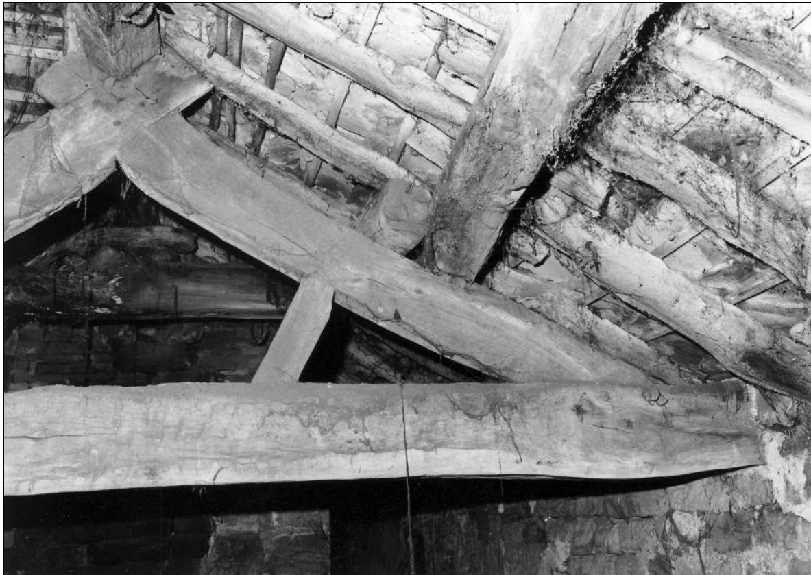
Photo 28: Early wing: detail of roof truss, from the south-east (film 3, frame 17)
