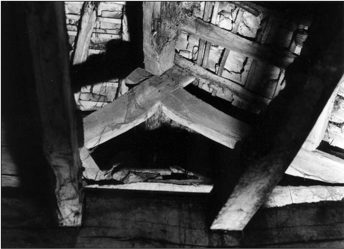
Photo 29: Early wing: detail of roof truss, from the south-east (film 3, frame 14)
