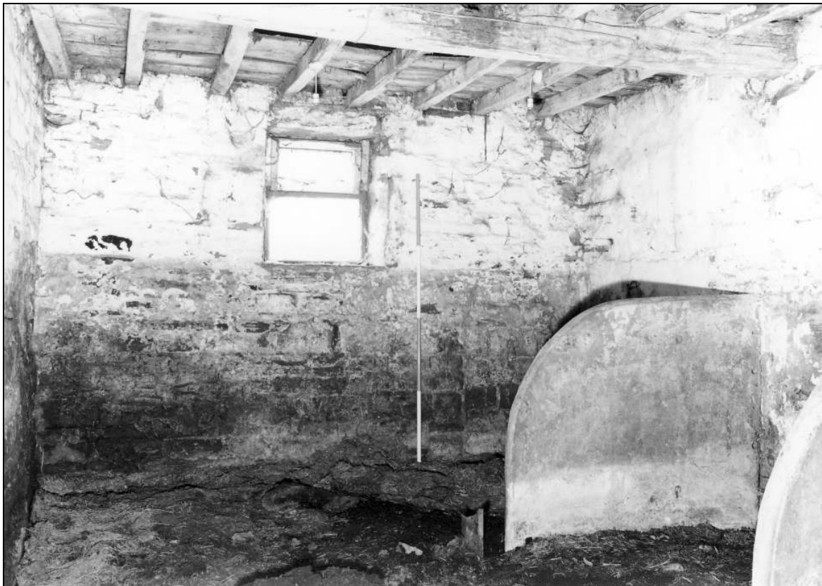
Photo 20: Early wing: interior, from the north (film 3, frame 8)
