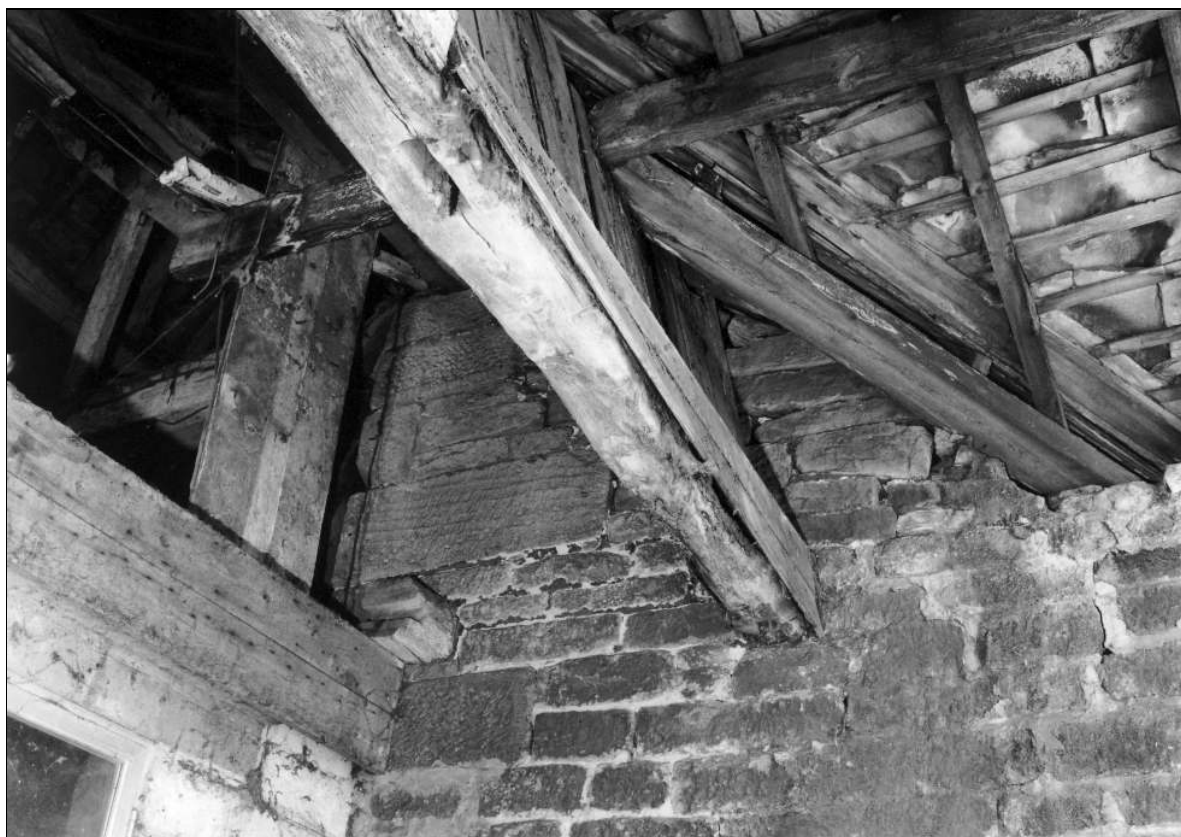
Photo 52: Interior of north-west entry, showing original door lintel (film 3, frame 5)
