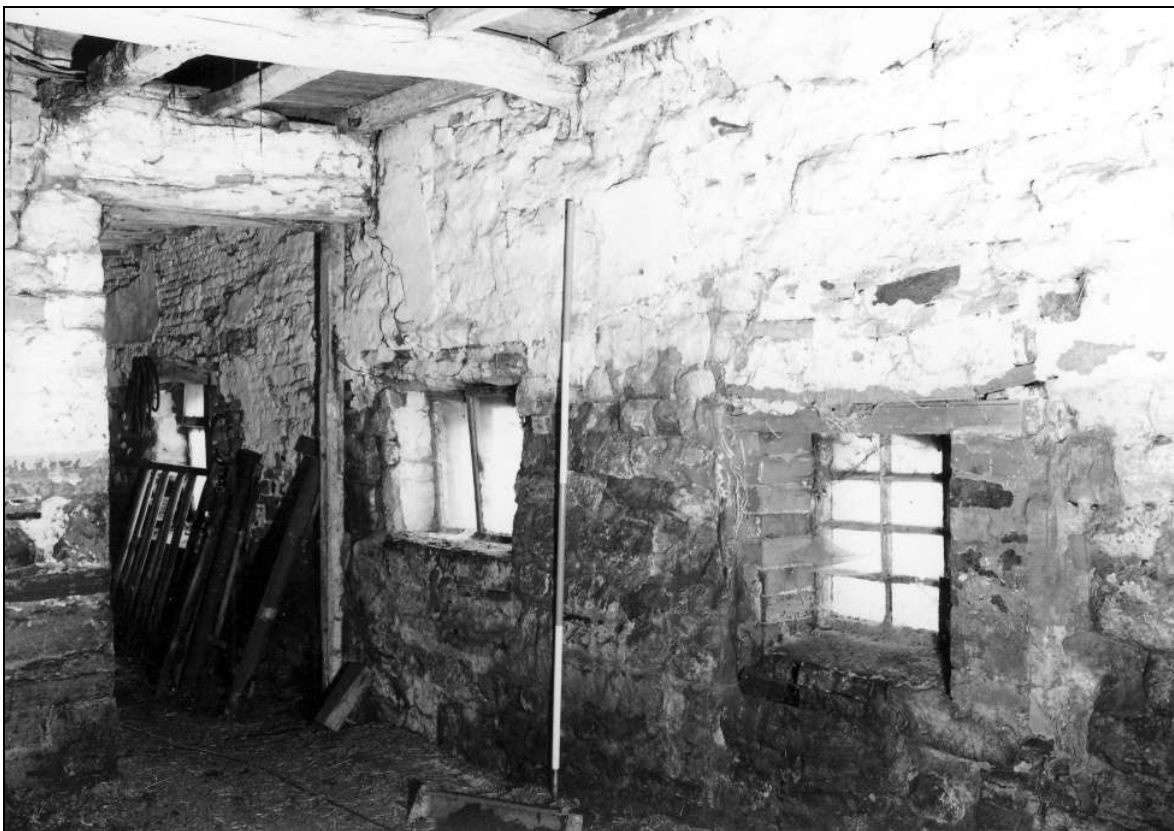
Photo 22: Early wing: interior, from the south (film 3, frame 11)
