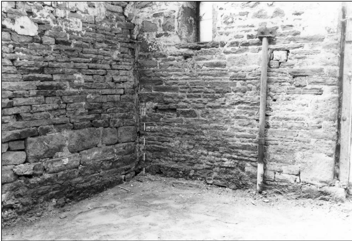
Photo 43: Stable: interior, from the east, during building works (film 6, frame 12)
