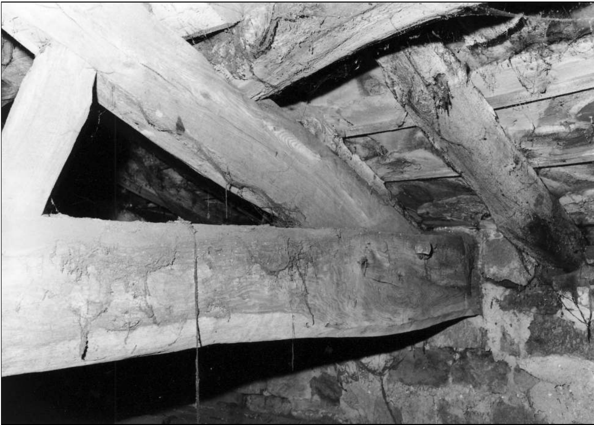
Photo 31: Early wing: detail of roof truss, from the south (film 4, frame 7)
