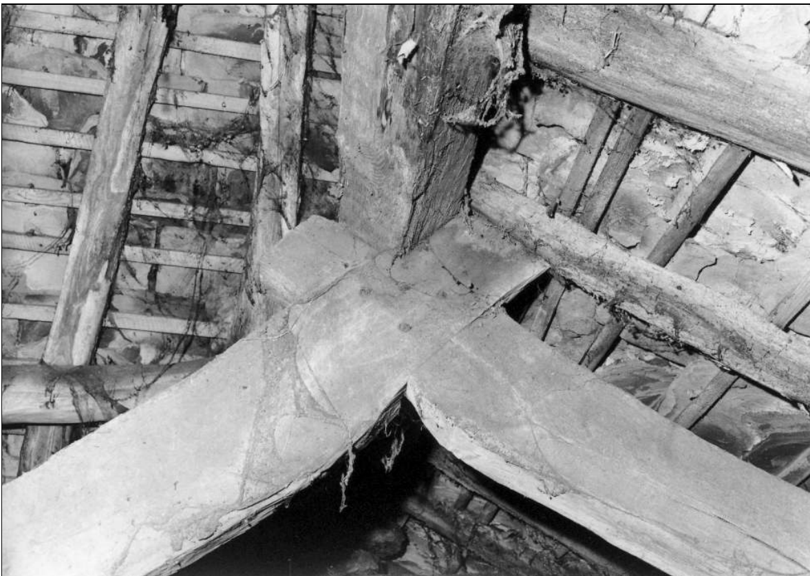
Photo 30: Early wing: detail of roof truss, from the south-east (film 4, frame 6)
