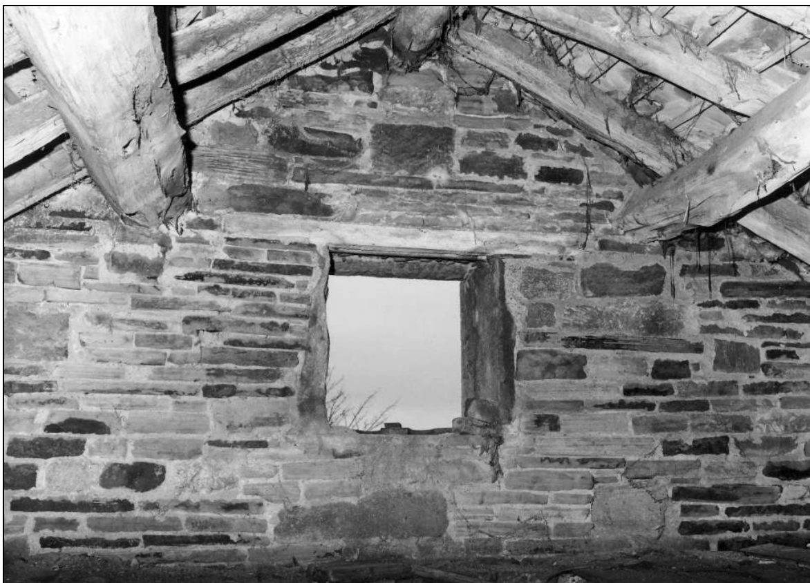
Photo 45: Stable: interior at loft level, from the south-east (film 4, frame 5)
