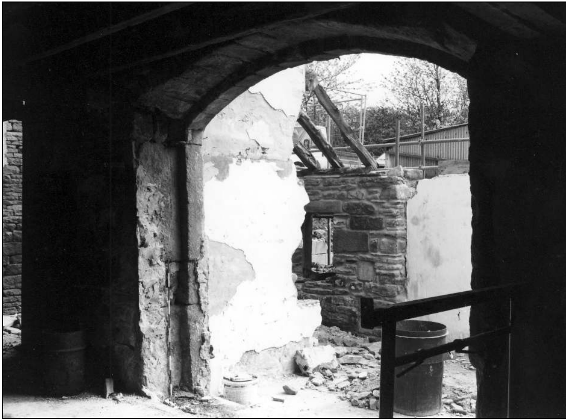
Photo 63: Arched doorway in south-east elevation of barn, after unblocking (film 6, frame 11)
