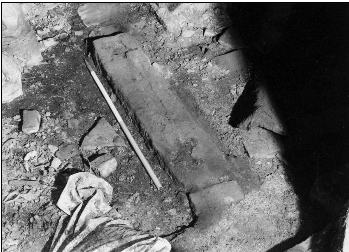
Photo 71: Barn interior: stone base for boskin, east outshut (film 5, frame 3)
