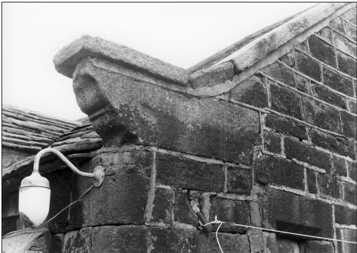
Photo 56: Detail of kneeler, at west corner of barn (film 2, frame 10)
