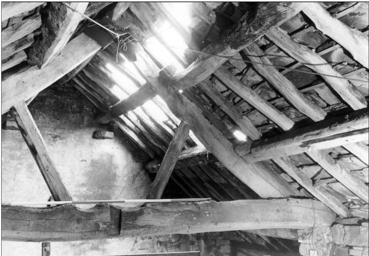
Photo 80: Barn interior: north-east roof truss, from the west (film 5, frame 9)
