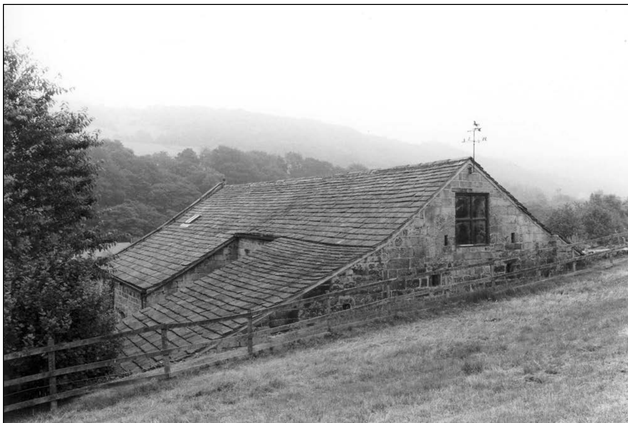
Photo 27: General view of the barn, from the north-west (film 2, frame 4)
