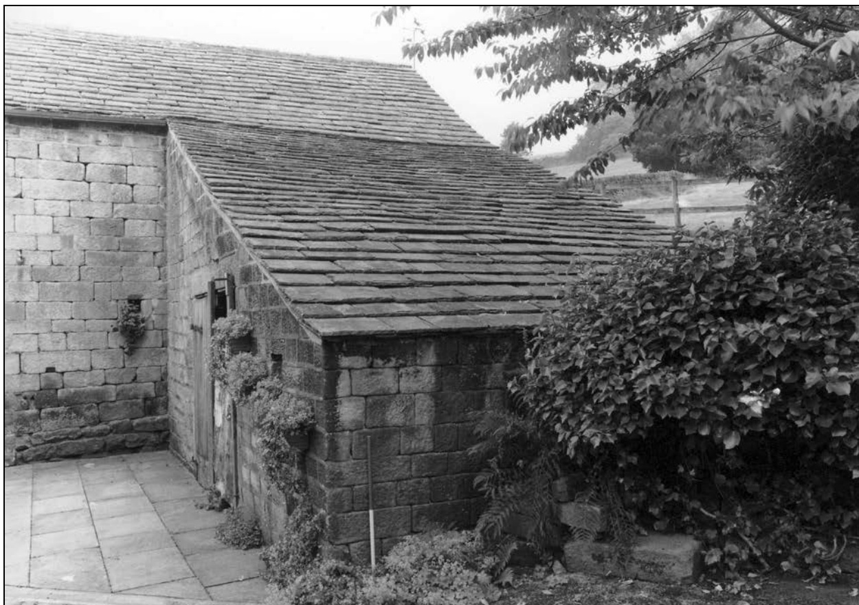
Photo 26: Nineteenth century addition at north-west corner of the barn, from the north (film 3, frame 1)
