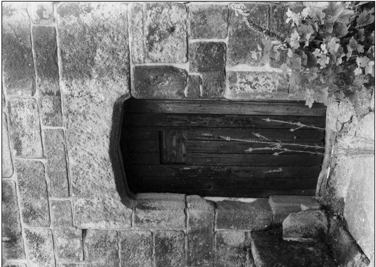
Photo 5: Detail of original doorway in south elevation (film 1, frame 12)
