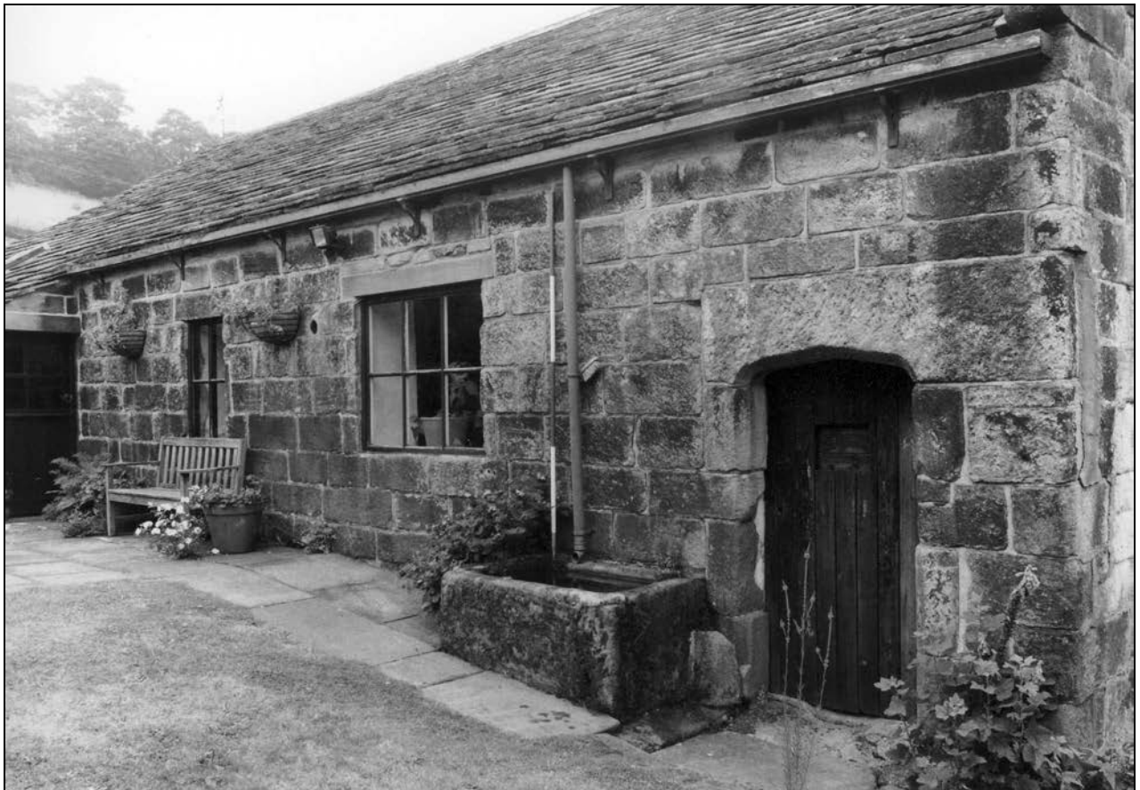
Photo 4: The south elevation (east end), with original doorway at right and later windows to left (film 1, frame 11)
