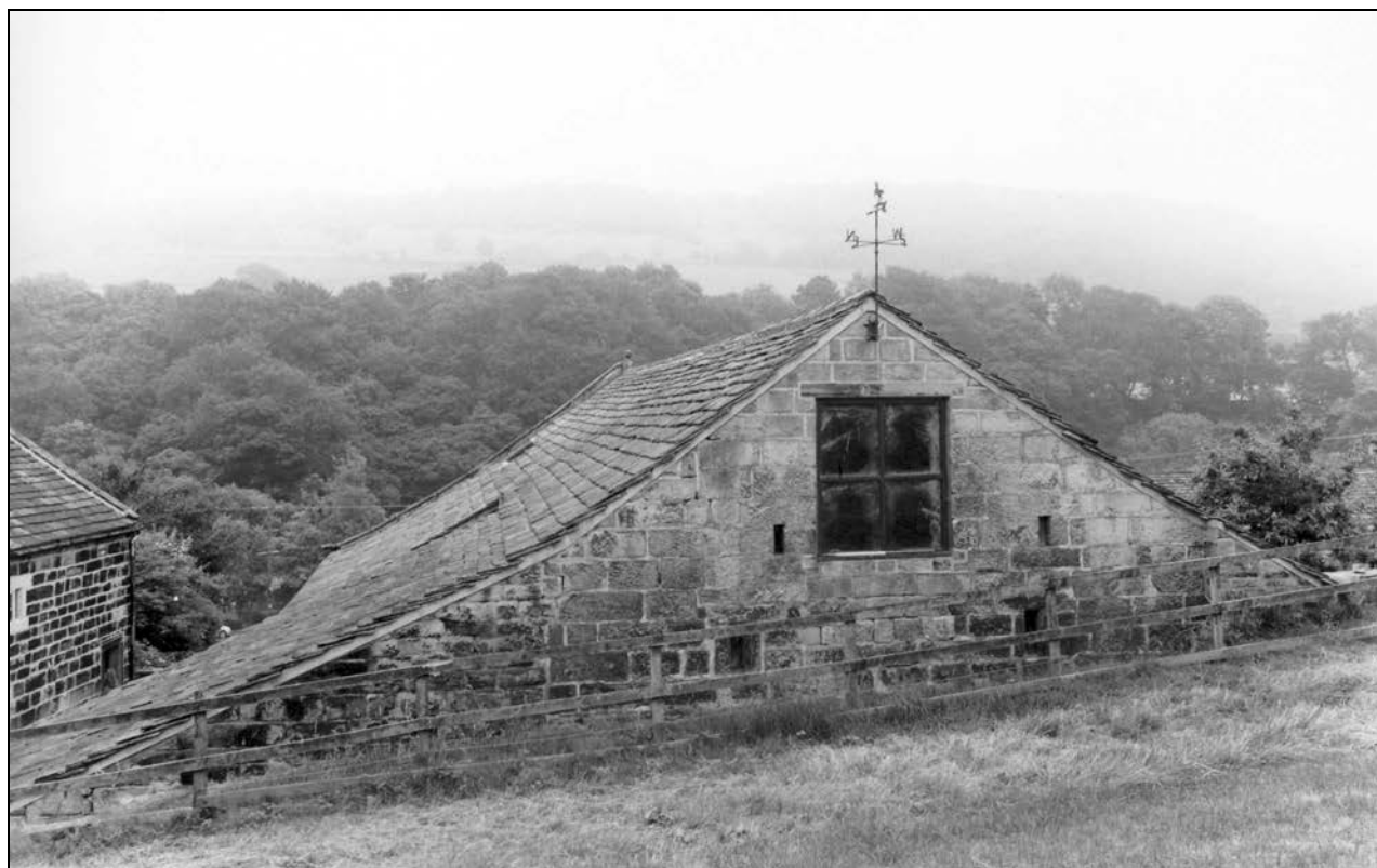
Photo 28: General view of the barn, from the west (film 2, frame 1)
