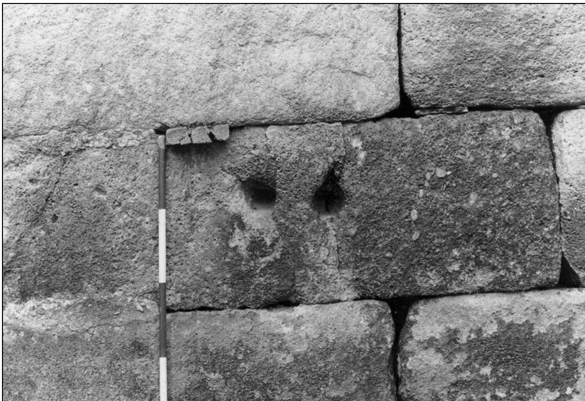
Photo 21: Possible wuzzing holes to right of north entrance to threshing bay (film 3, frame 2)
