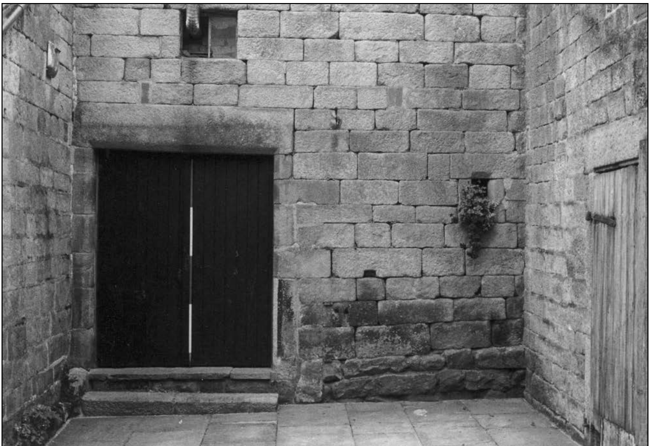
Photo 20: The north entrance to the threshing bay (film 2, frame 17)
