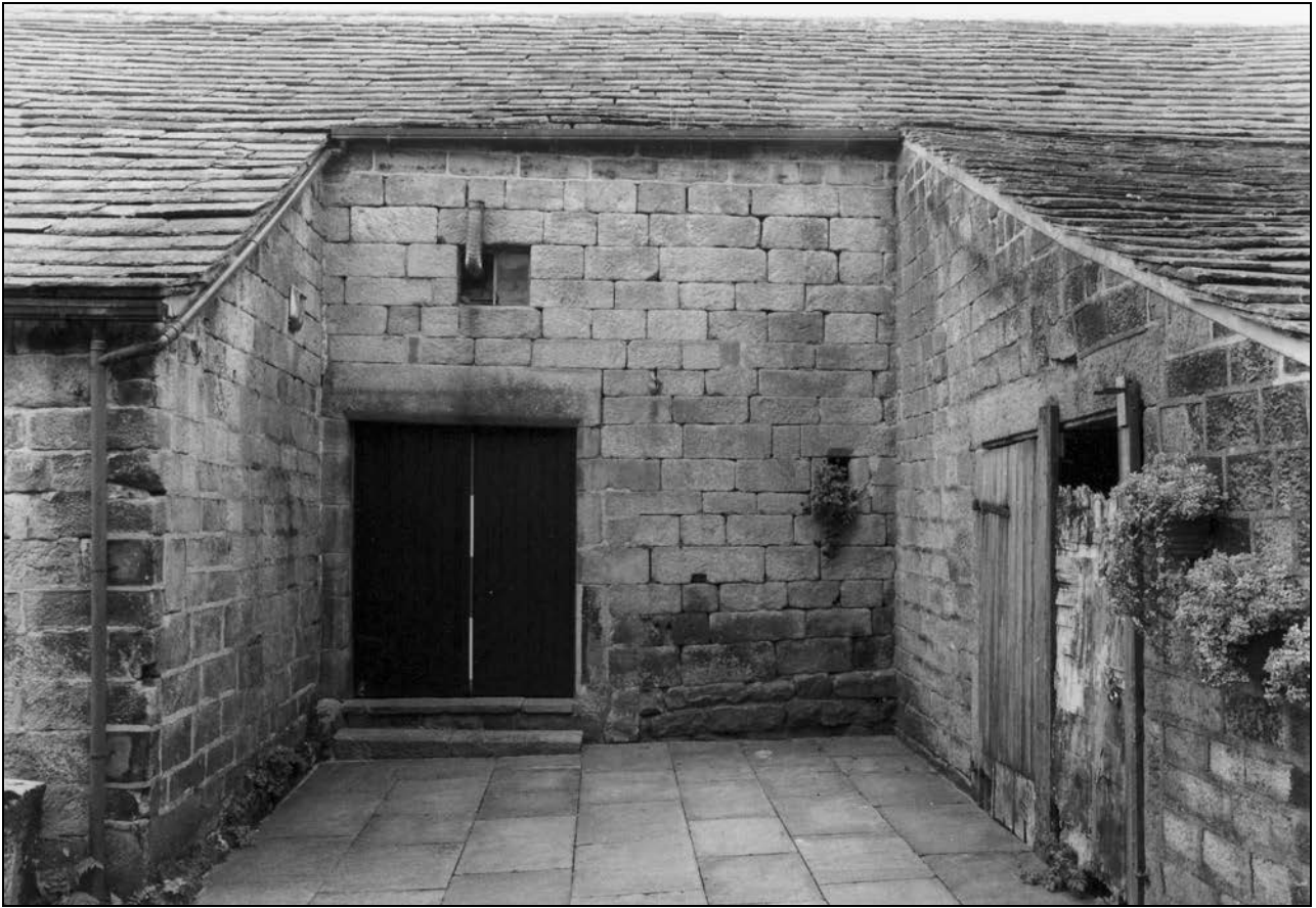
Photo 19: The north entrance to the threshing bay, between original projection (left) and nineteenth century addition (right) (film 2, frame 17)
