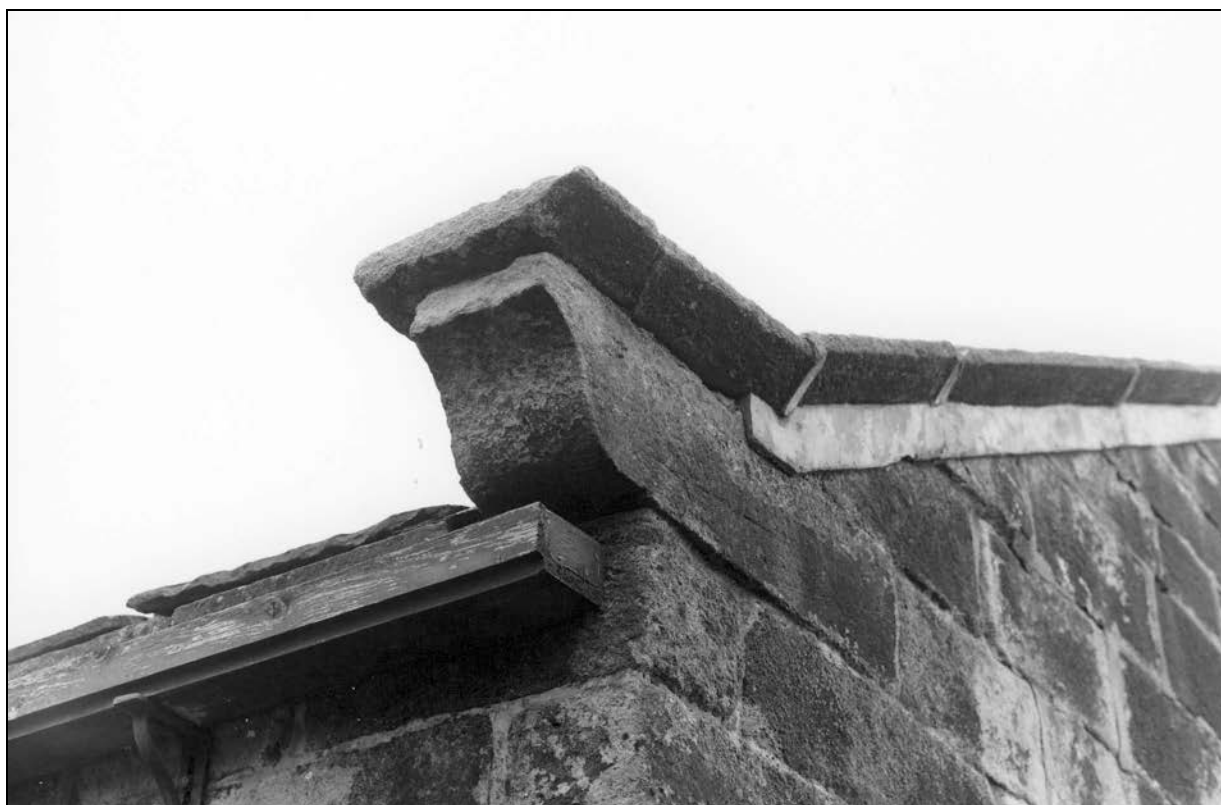
Photo 15: Detail of kneeler and coping, east gable (film 3, frame 5)
