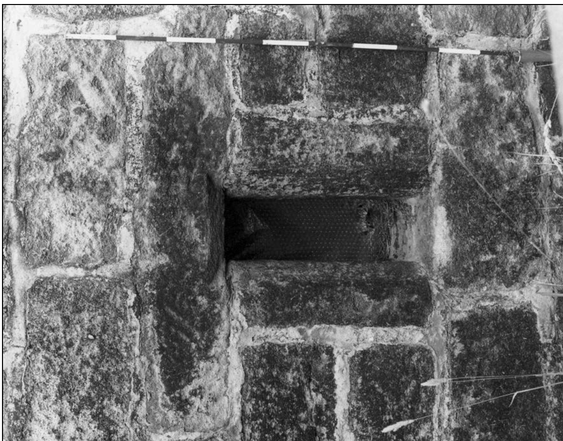
Photo 14: Detail of typical chamfered, arched breather, in west gable (film 2, frame 6)
