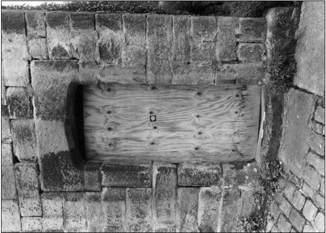
Photo 10: Detail of original (possibly heightened) doorway in east gable (film 2, frame 9)
