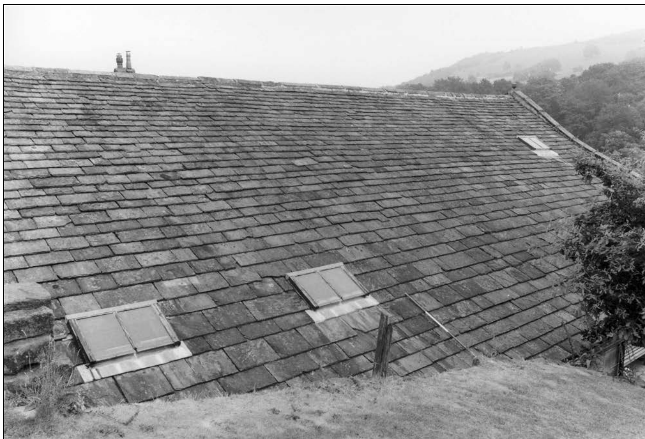
Photo 31: The barn's southern roof pitch, from the south-west (film 1, frame 8)
