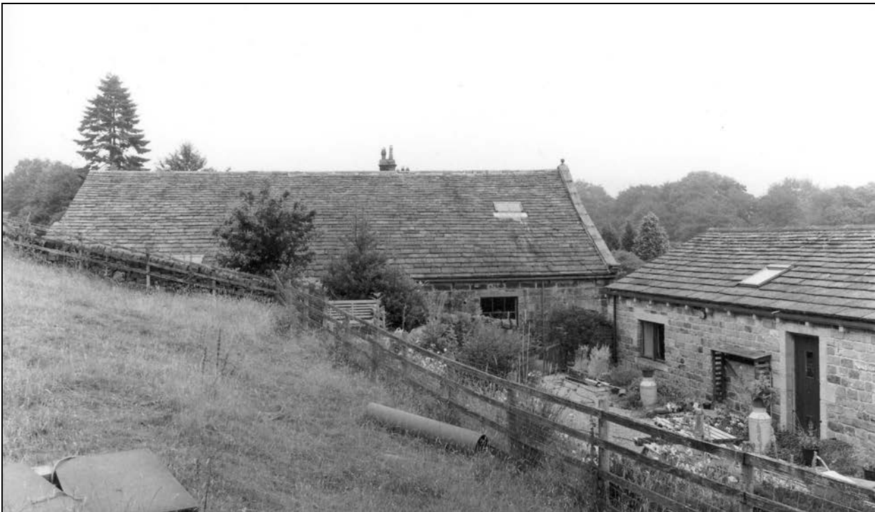
Photo 2: View of the barn, from the south (film 1, frame 7)
