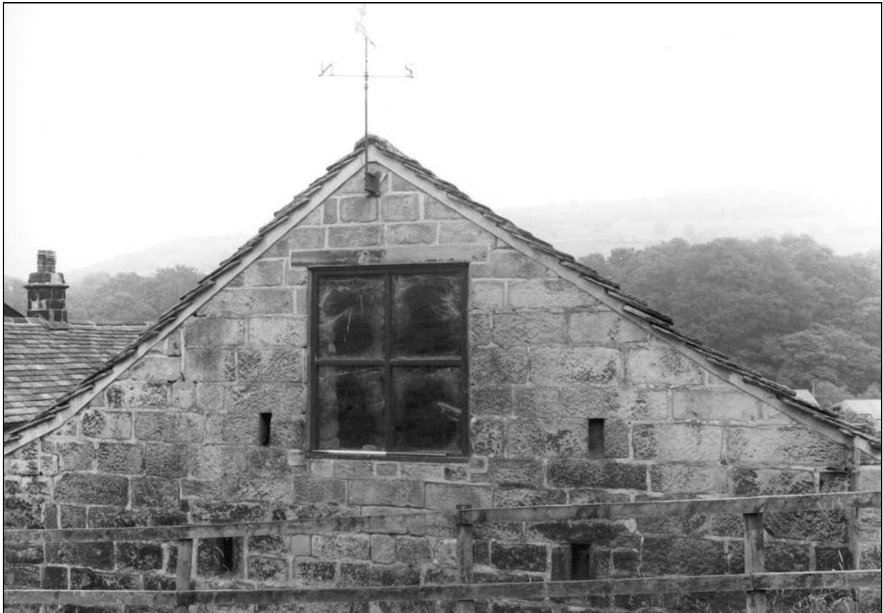
Photo 30: Upper part of barn's west gable (film 2, frame 2)
