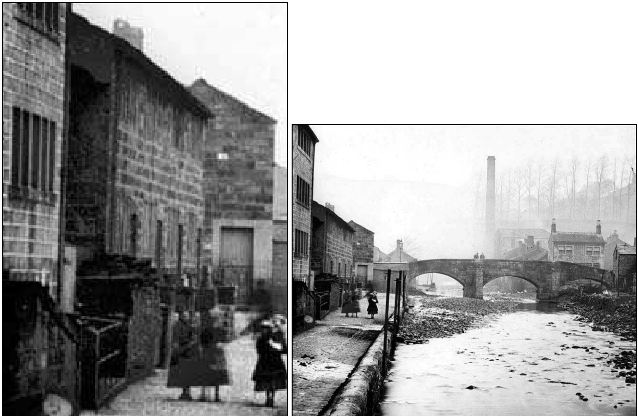
Figure 6: Photograph of Old Gate and the Hebden Water from the south-west, before c.1905 The row of four cottages stands detached and elevated above the then lower street level © PHDA – Hebden Bridge Local History Society; ref no HLS05065
