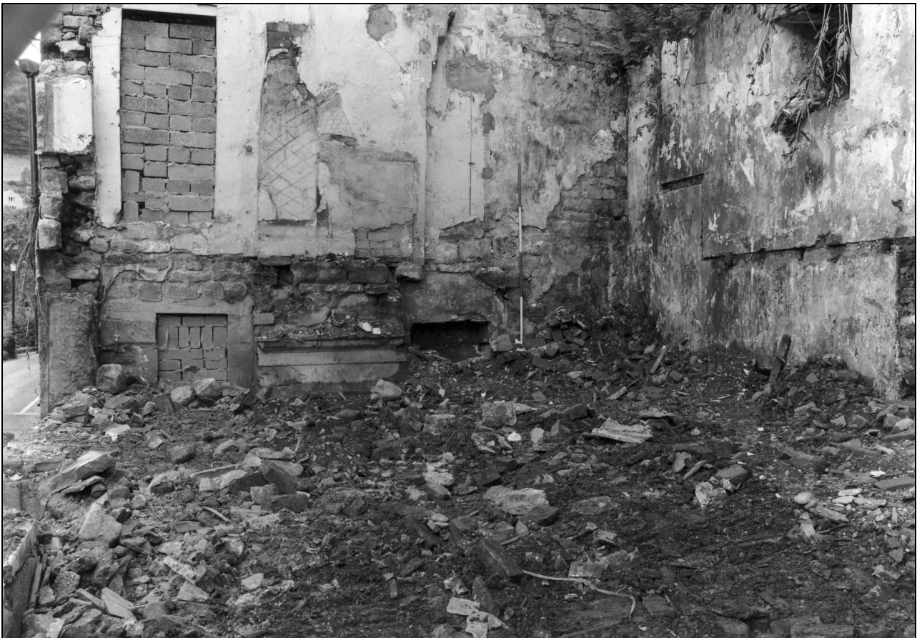
Photo 25: Cottage 1: interior, during demolition (film 5, film 5)
