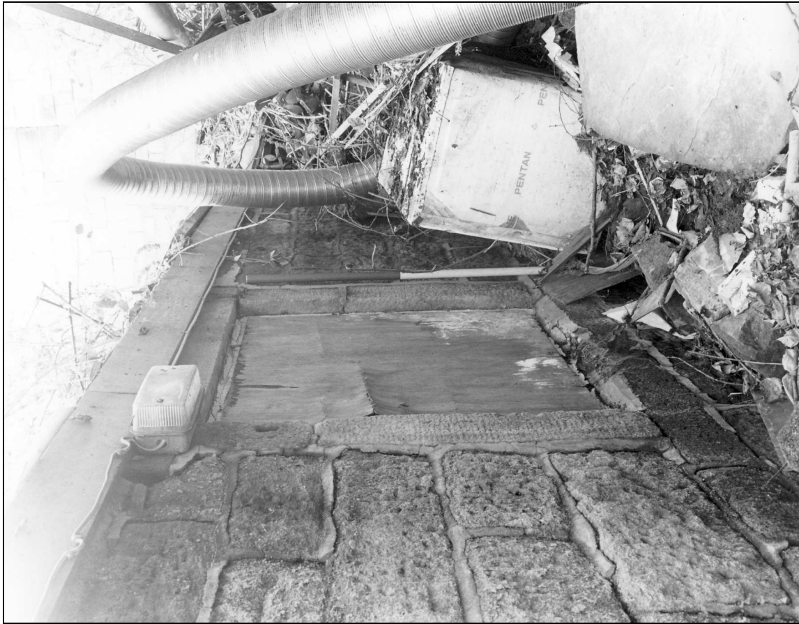
Photo 18: Cottage 2: rear, first floor window (film 3, film 10)
