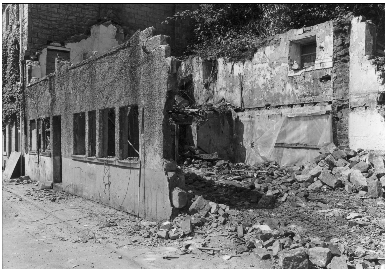
Photo 5: Cottages 1 and 2 during demolition (film 5, film 1)
