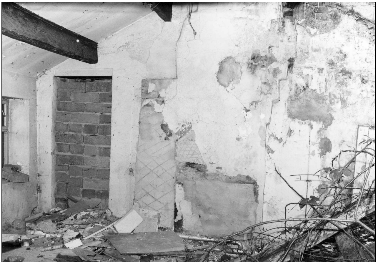
Photo 44: Cottage 1: south-west gable at first floor, with blocked fireplace (film 1, film 11)
