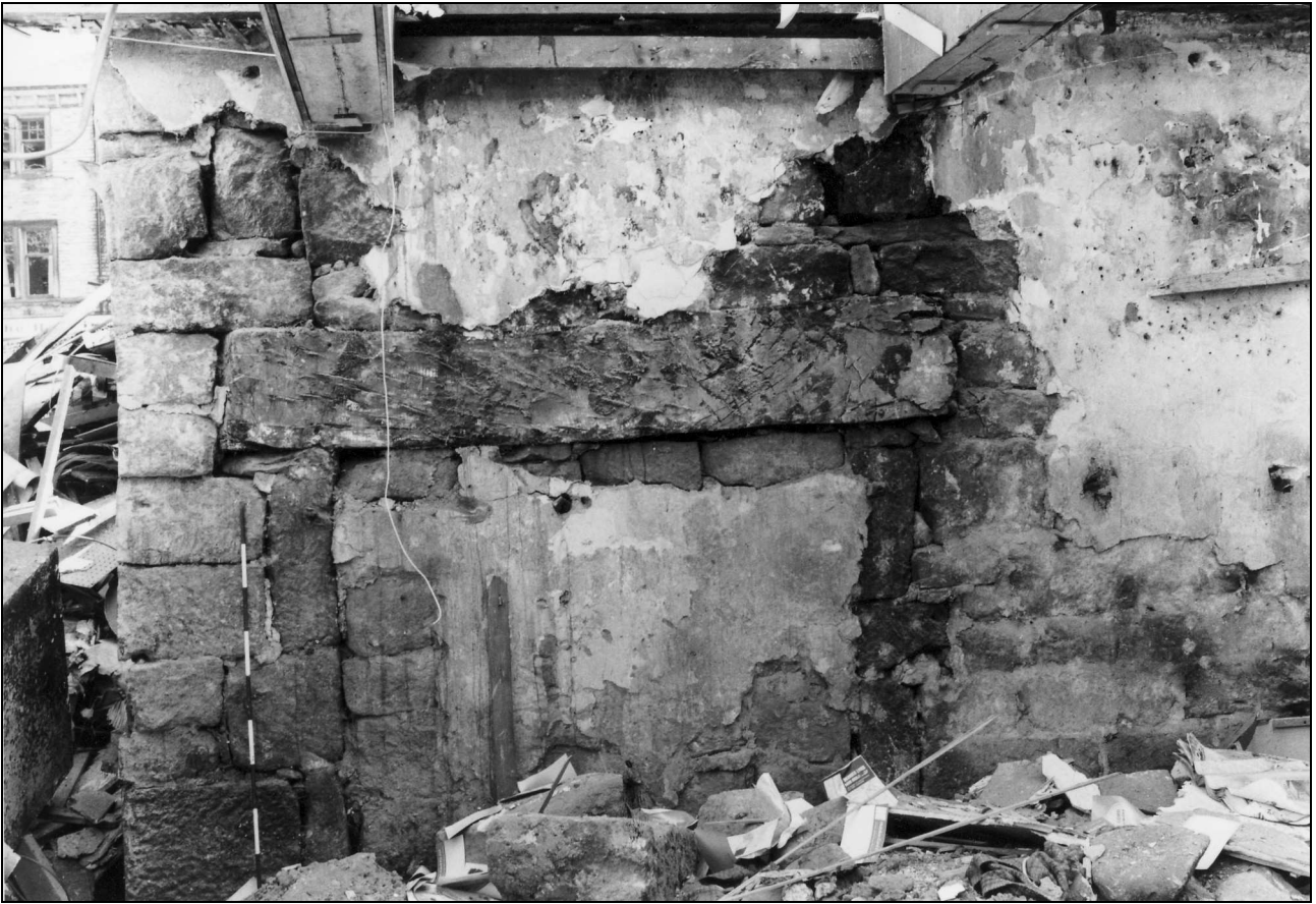
Photo 47: Cottage 4: inserted fireplace in north-east gable, ground floor (film 4, film 1)
