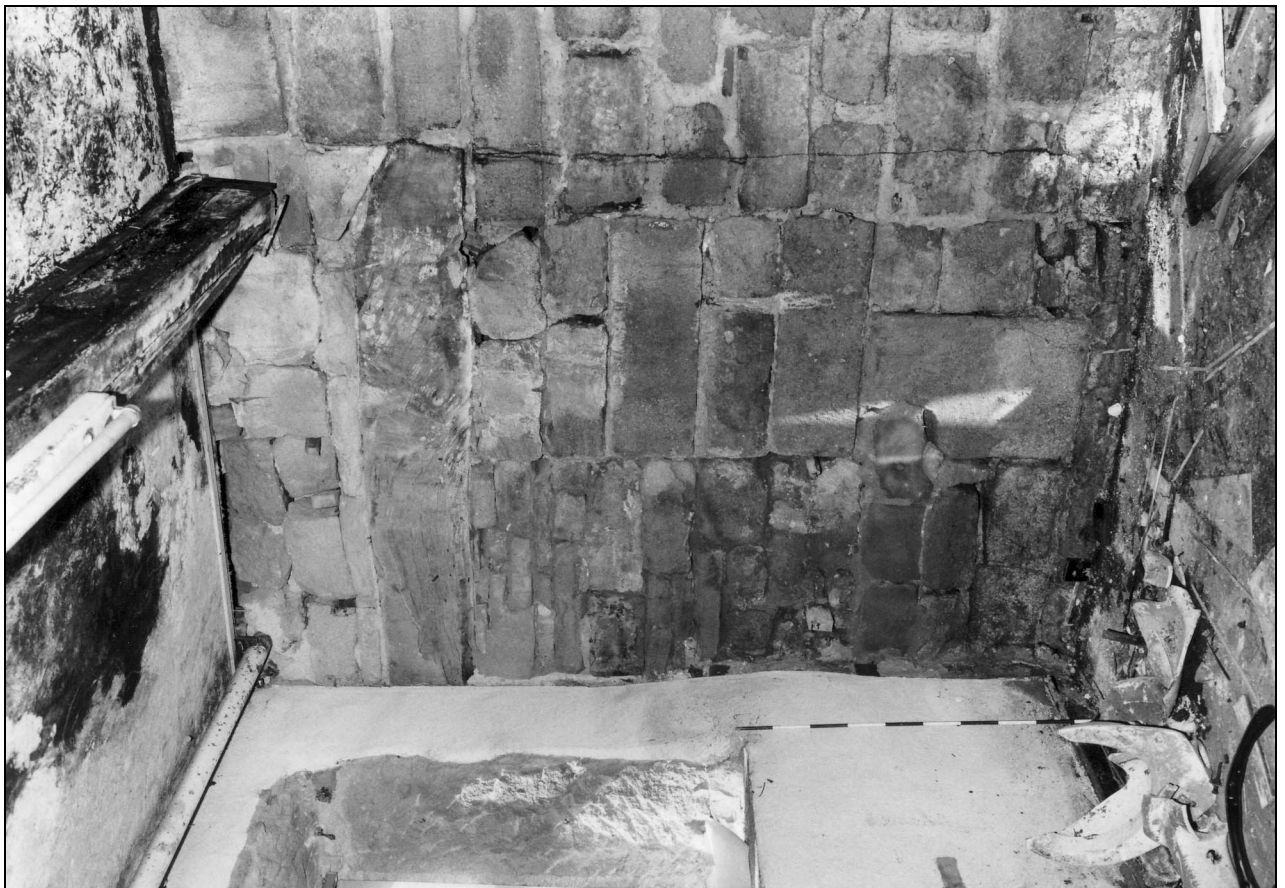
Photo 31: Cottage 1: south-west gable on ground floor, showing remains of oak timber, cut by modern doorway (film 6, film 5)
