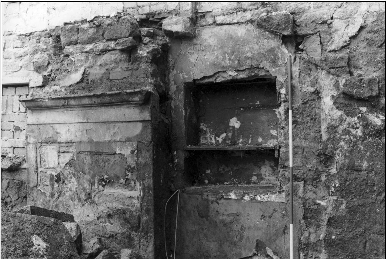
Photo 34 : Cottage 1: cupboard in south-west gable, beneath former stairs (film 5, film 11)
