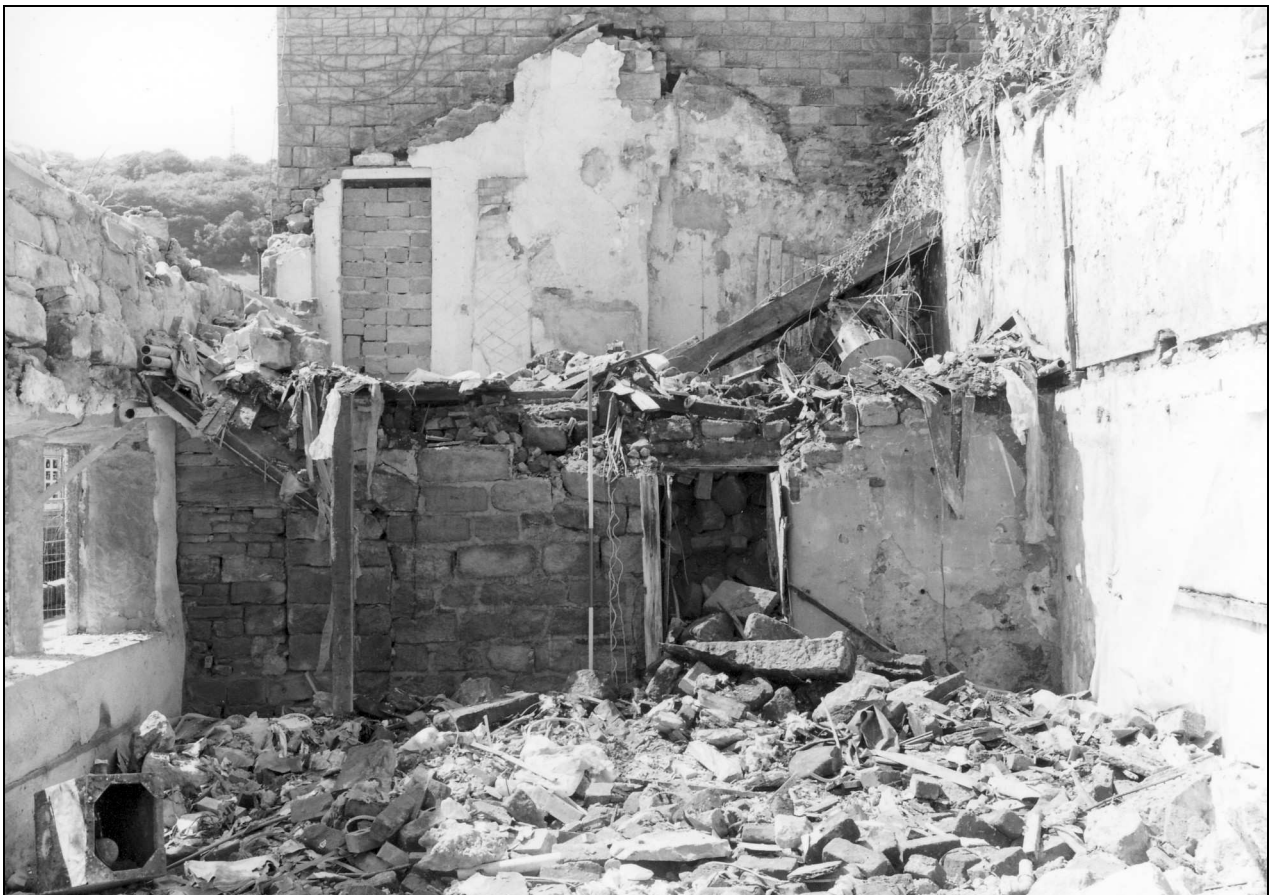
Photo 54: Cottage 2, during demolition (film 5, film 2)
