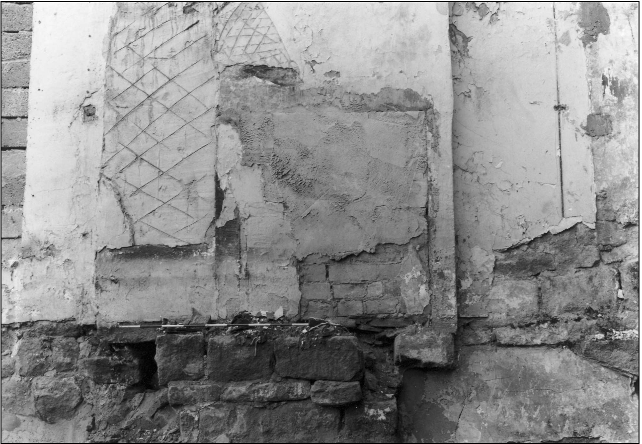
Photo 45: Cottage 1: detail of first floor fireplace (film 6, film 10)
