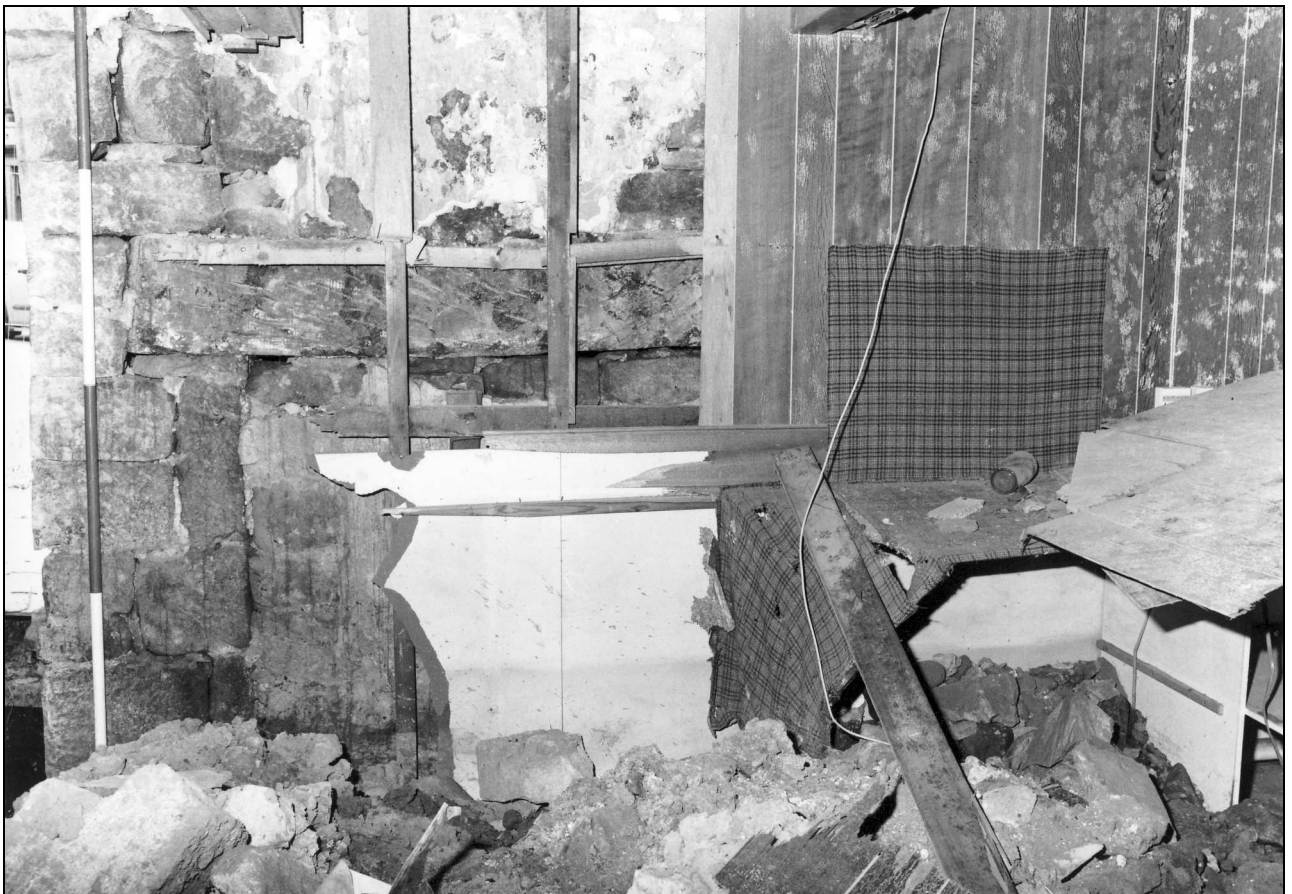
Photo 46: Cottage 4: inserted fireplace in north-east gable, ground floor (film 1, film 10)
