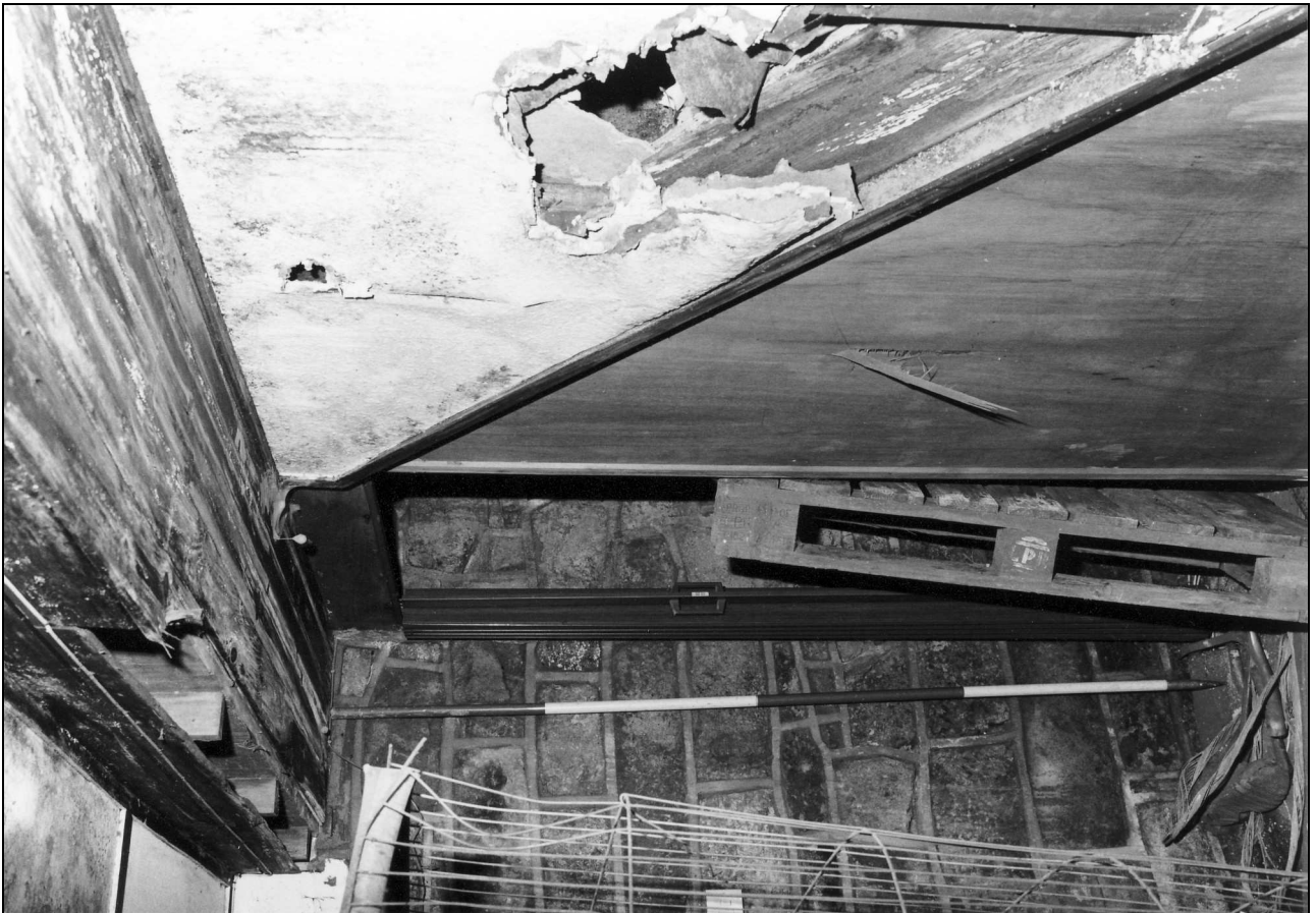
Photo 49: Cottage 3: modern stairs against rear wall (film 1, film 6)
