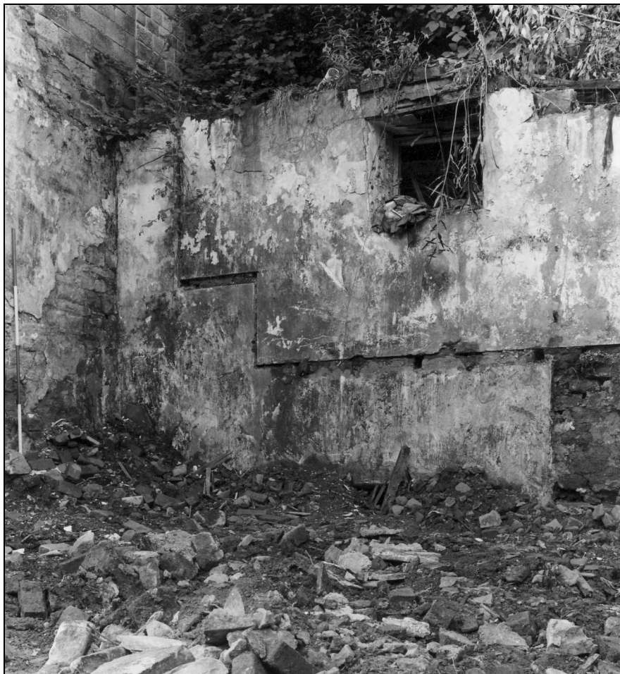
Photo 40: Cottage 1: interior, during demolition (film 5, film 7)
