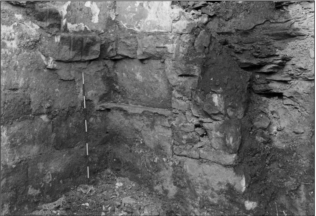
Photo 37: Cottage 1: recess or former shelf base beneath stairs (film 6, film 11)
