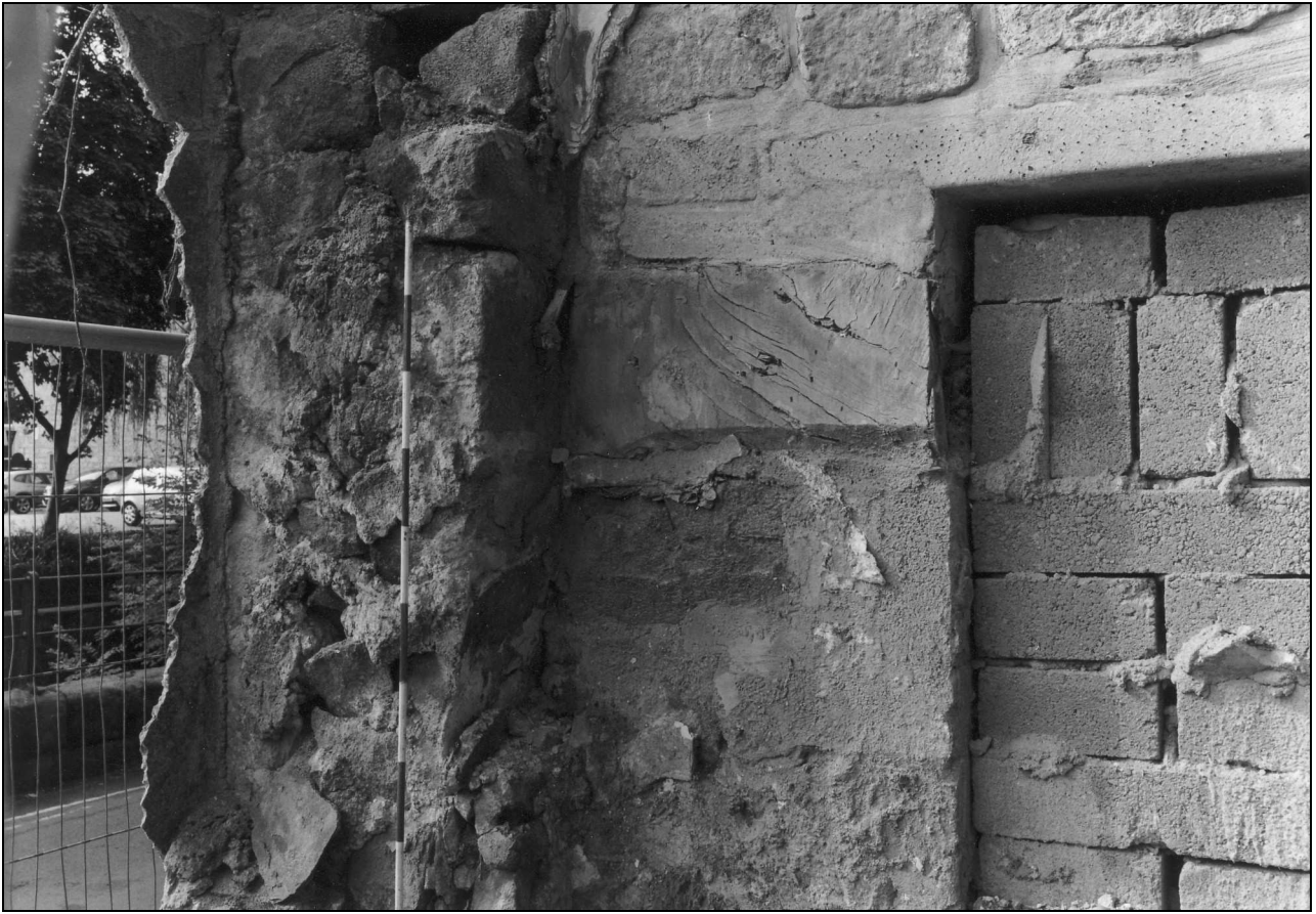
Photo 31: Cottage 1: south-west gable on ground floor, showing remains of oak timber, cut by modern doorway (film 6, film 5)
