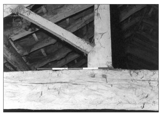
Photo 44: Detail of truss (type 1), with carpenter's marks "V", over milking parlour, from the south (film 1, frame 12)
