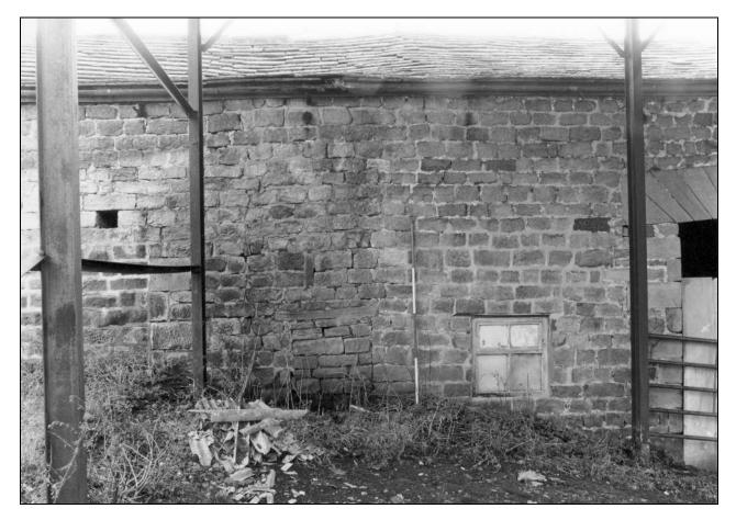
Photo 14: West side of barn range beneath Dutch barn, showing altered openings (film 4, frame 1)
