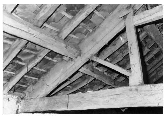
Photo 42: Detail of truss (type 1), over milking parlour, from the south-east (film 1, frame 14)
