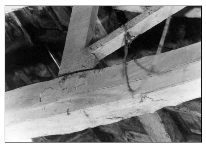
Photo 43: Detail of truss (type 1), with carpenter's marks "III", over barn, from the north-east (film 2, frame 17)
