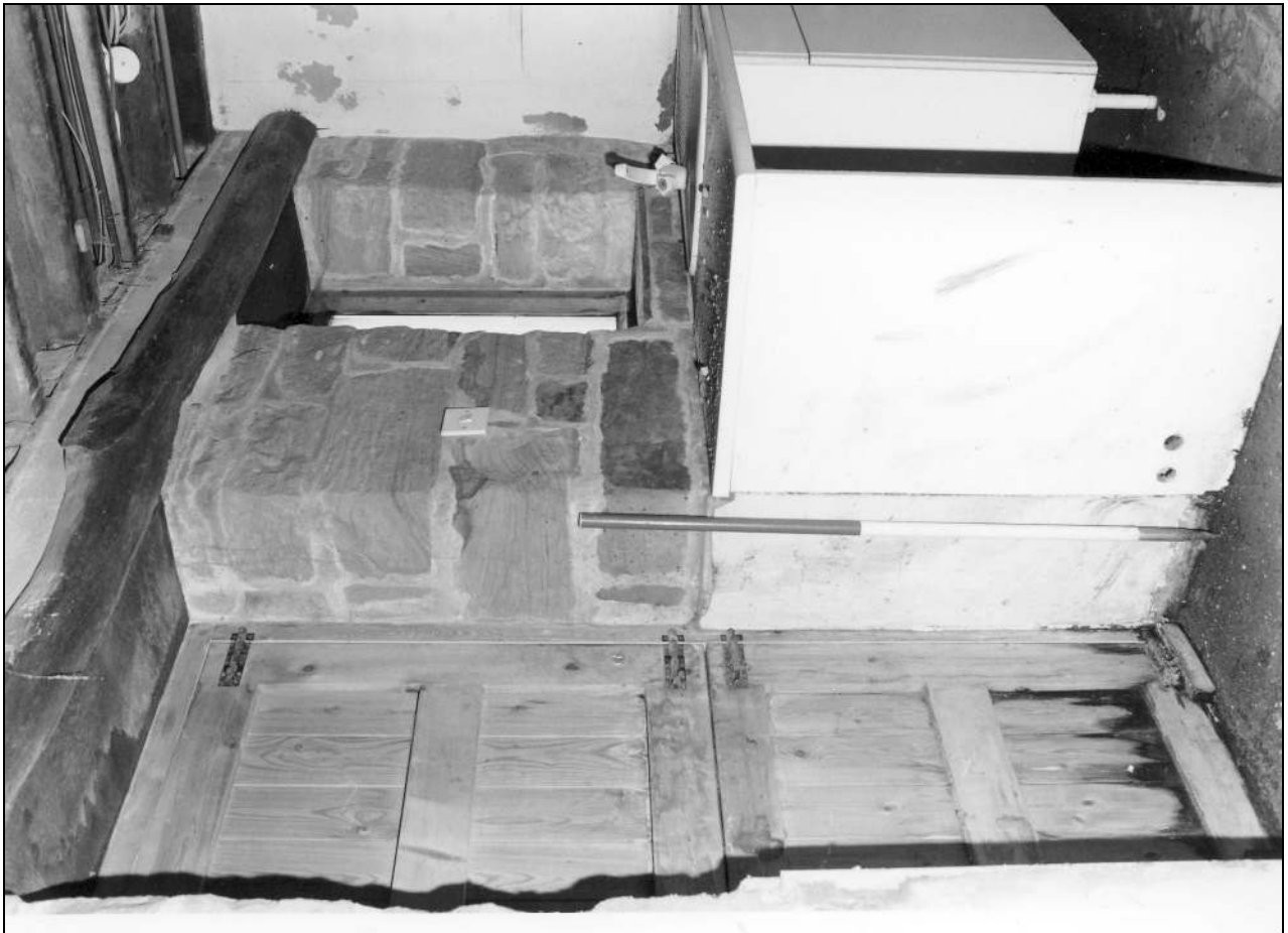
Photo 41: Rear wall of kitchen, from the south-west (film 2, frame 5)
