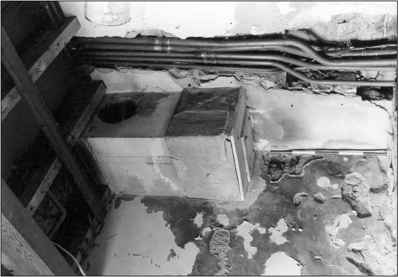
Photo 42: Detail of corbelled chimney in kitchen, from the north-west (film 2, frame 6)
