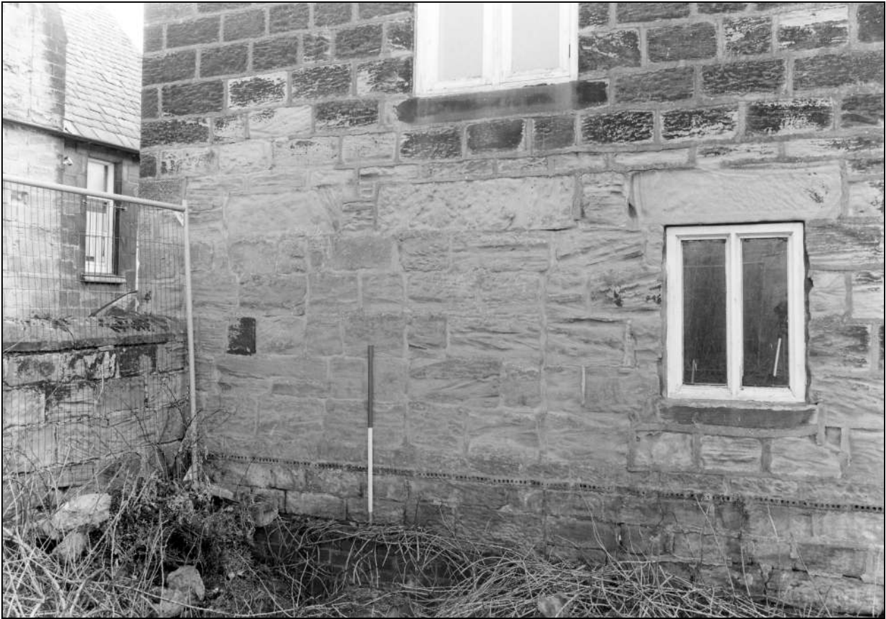
Photo 18: Rear of outshut, showing blocked window and doorway (film 3, frame 3)
