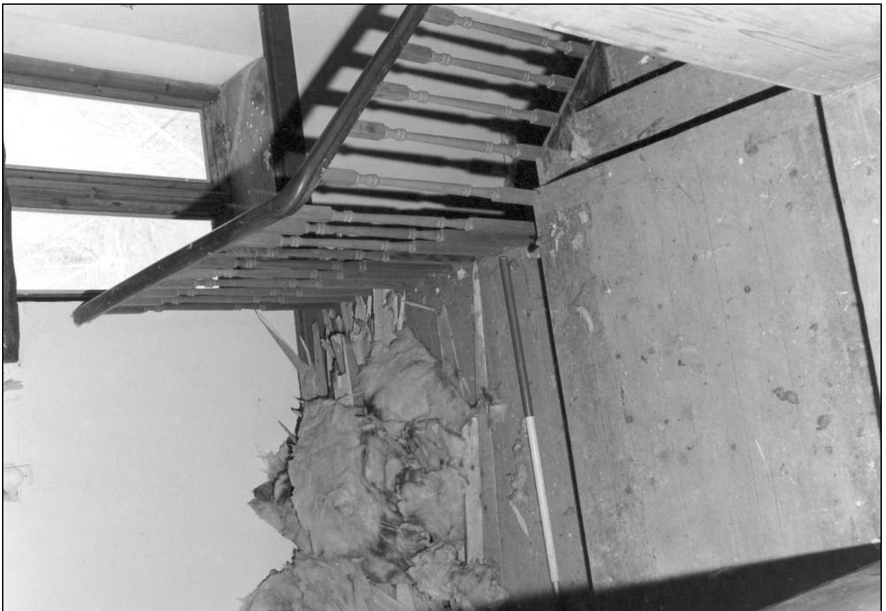
Photo 45: View down onto first floor landing, from the south (film 4, frame 6)
