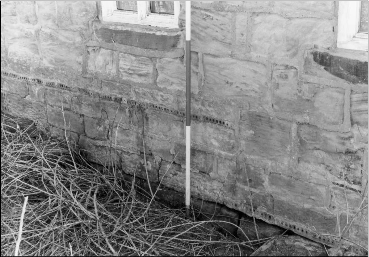
Photo 20: Rear of outshut, showing step down in damp-course (film 5, frame 7)
