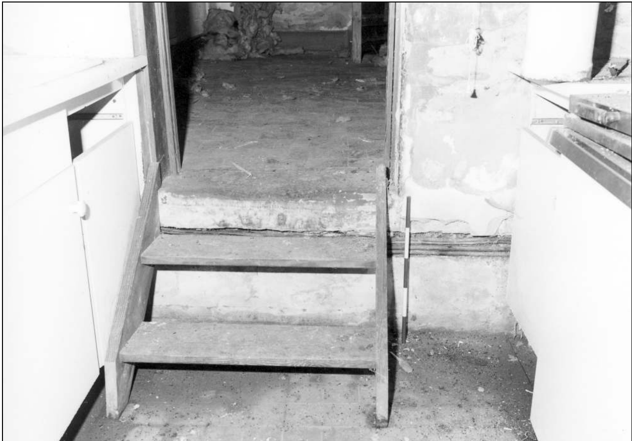
Photo 40: Detail of steps down into kitchen, from the west (film 2, frame 4)
