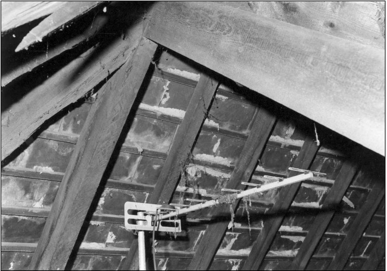
Photo 61: Roof space over bedroom 3, from the north-west (film 5, frame 6)
