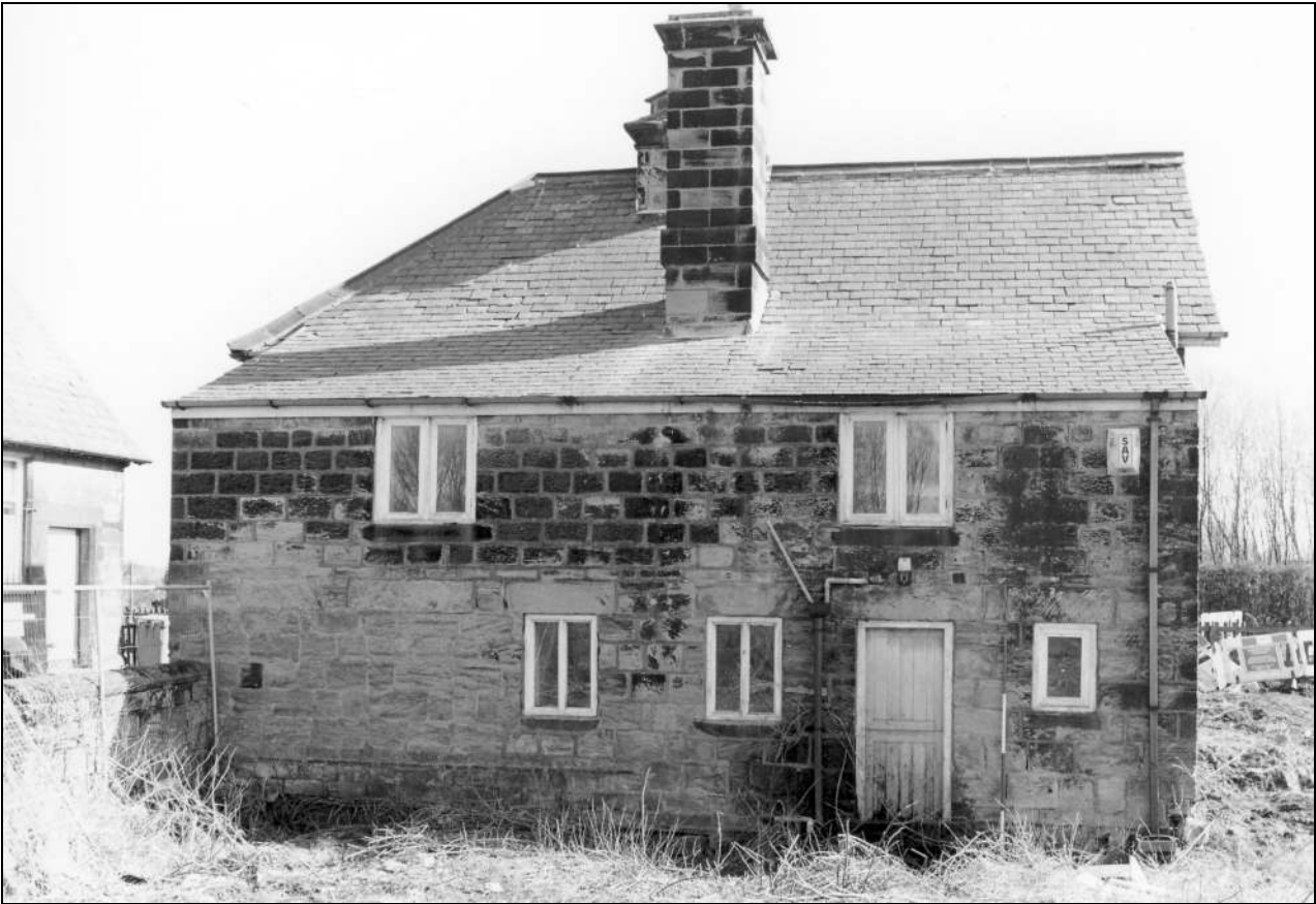
Photo 4: Rear elevation, from the north (film 5, frame 10)
