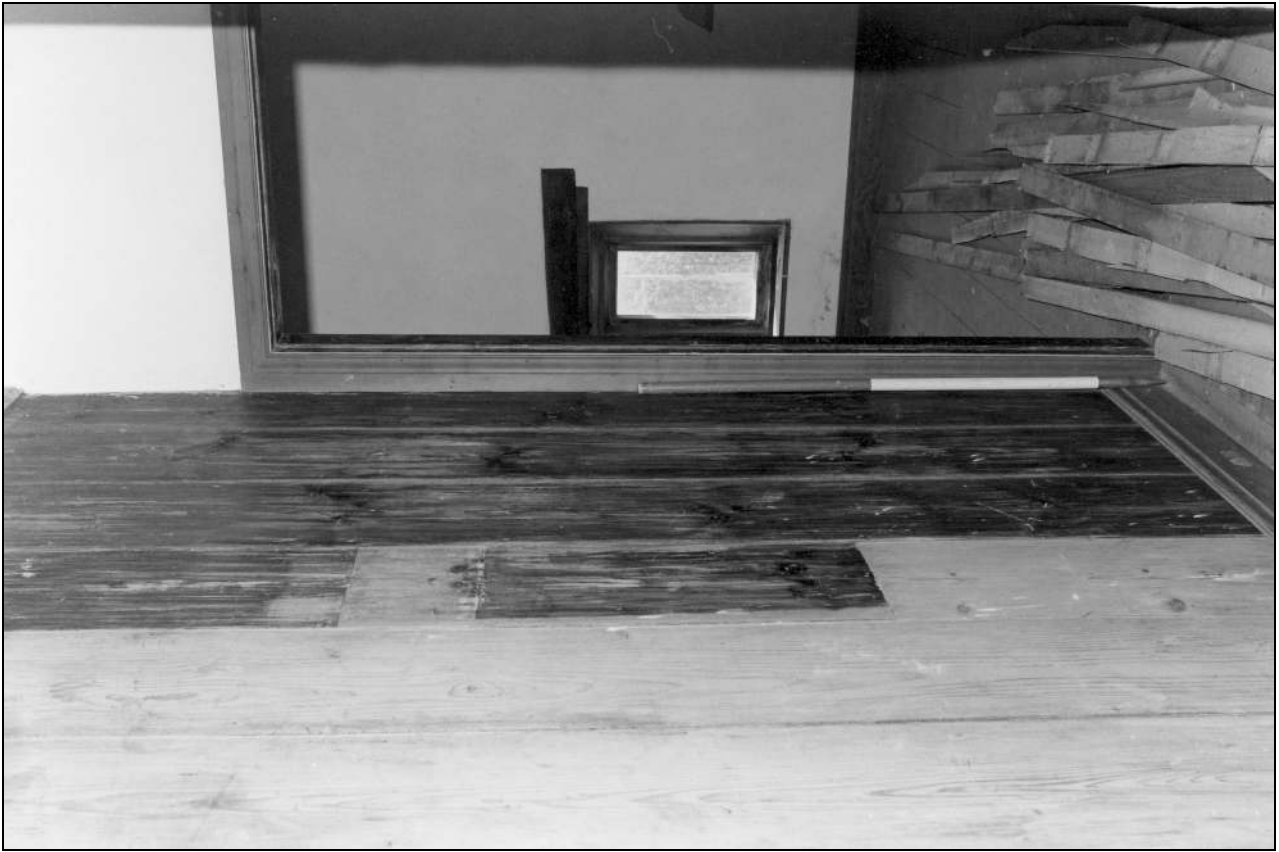
Photo 56: Historic partition and doorway to bedroom 2 from the south-east (film 4, frame 15)
