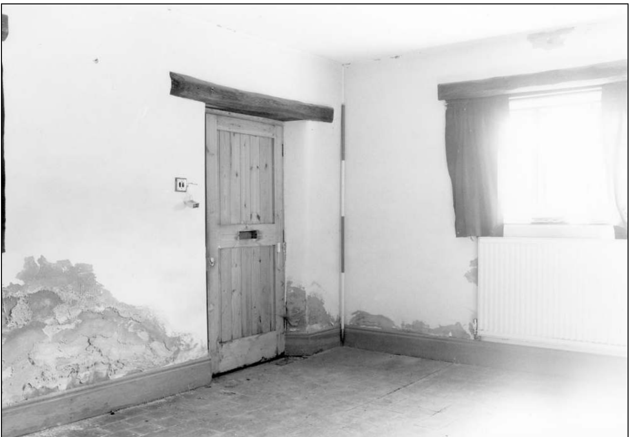
Photo 30: Living room 2, from the north-west (film 1, frame 4)
