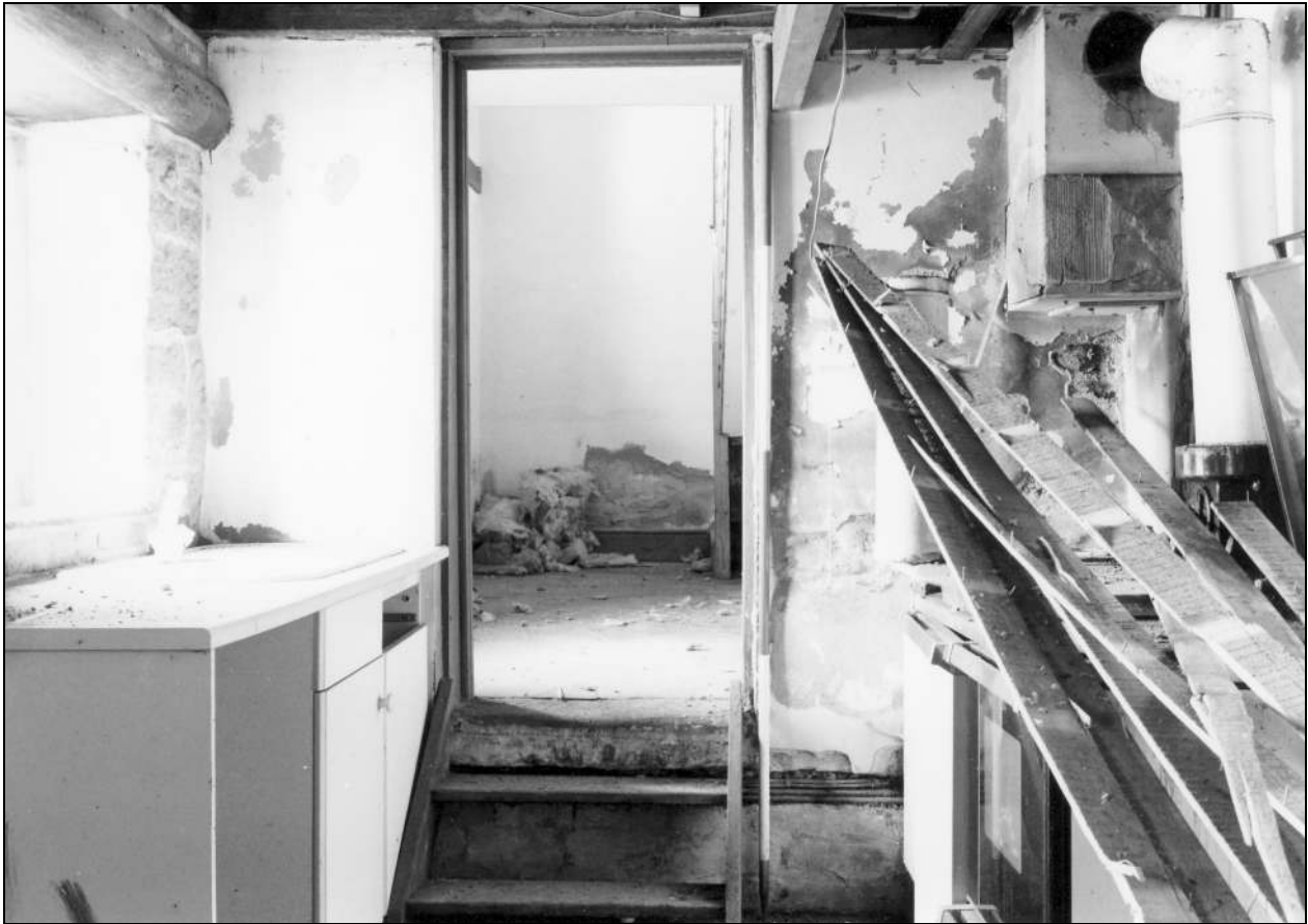
Photo 39: Kitchen, from the west (film 2, frame 3)
