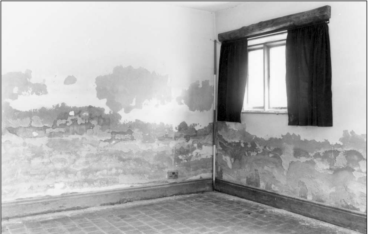
Photo 31: Living room 2, from the south-west (film 1, frame 2)
