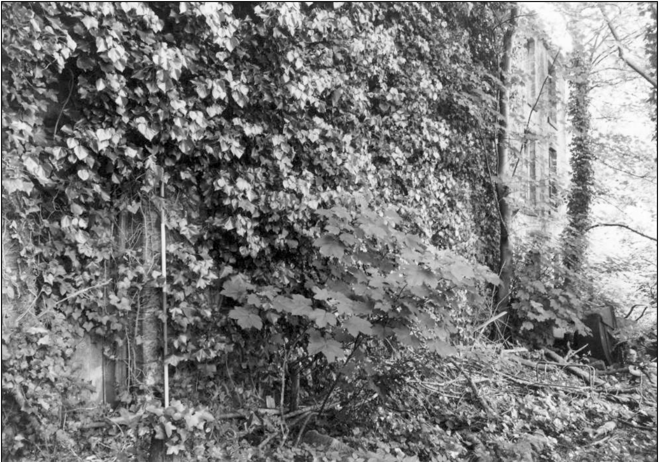
Photo 33: East side of boiler house (overgrown), from the south-east (film 3, frame 10)
