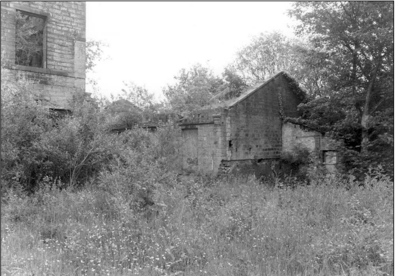
Photo 31: Boiler house, from the south-west (film 3, frame 7)
