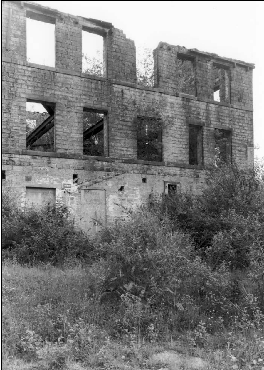
Photo 12: Spinning mill: east end of south elevation (film 3, frame 5)
