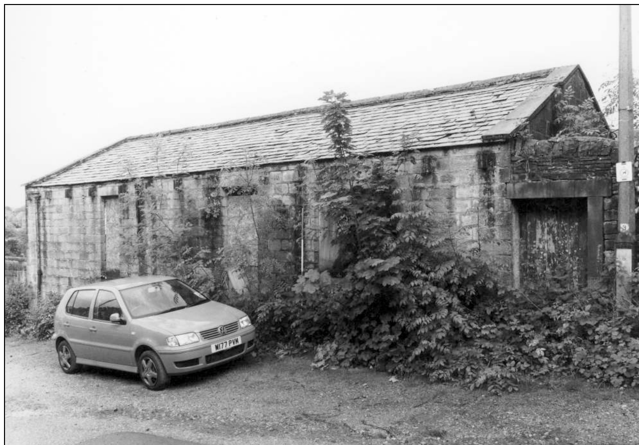
Photo 48: Offices, from the south-west (film 4, frame 11)
