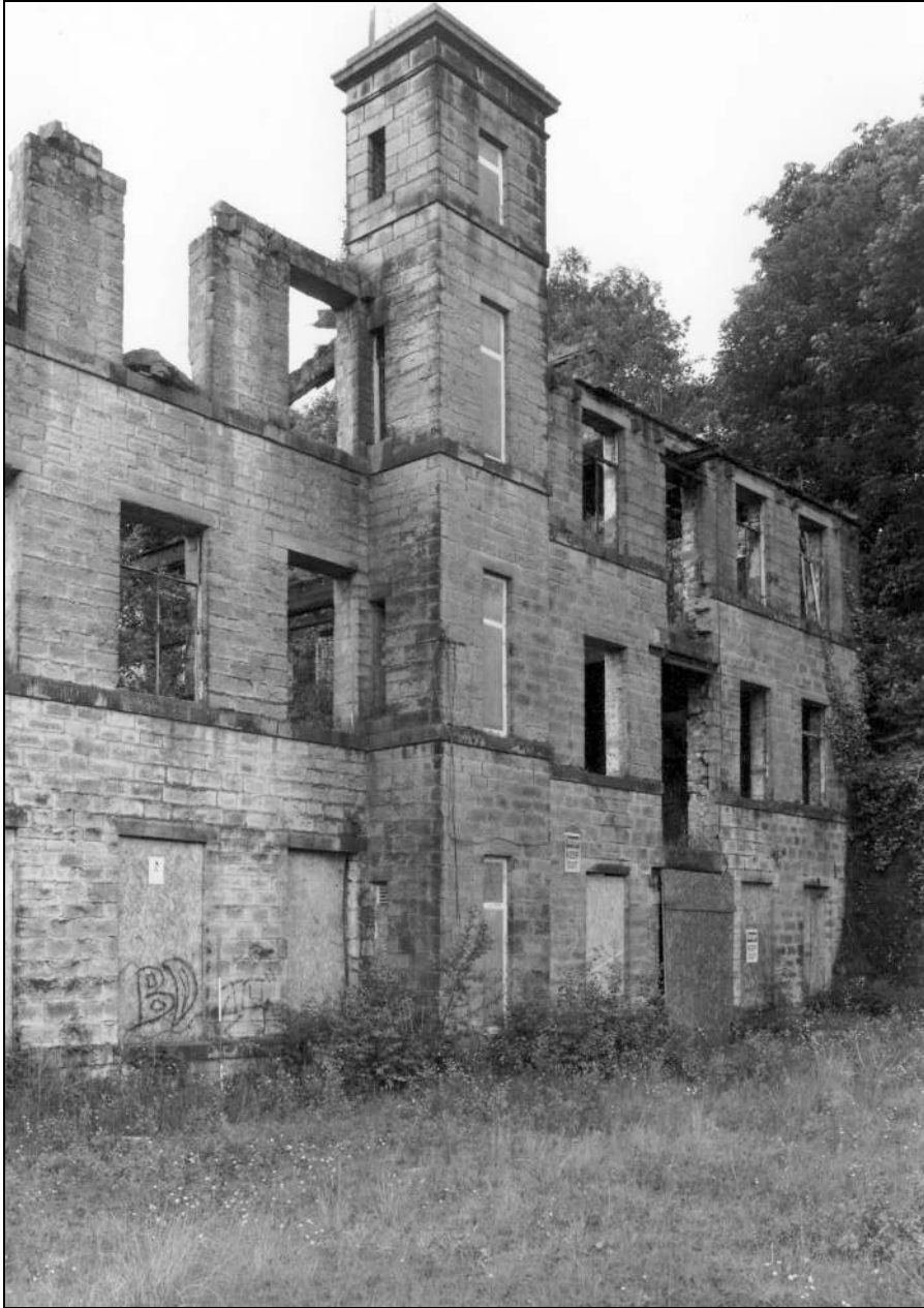
Photo 4: Spinning mill: detail of lavatory tower, from the north-east (film 1, frame 5)
