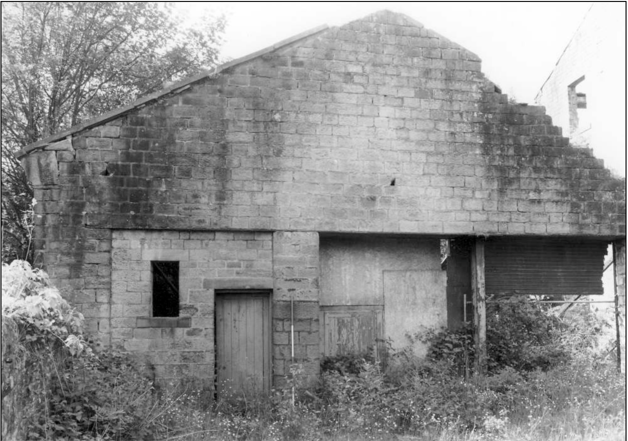
Photo 29: North gable of boiler house (film 2, frame 1)
