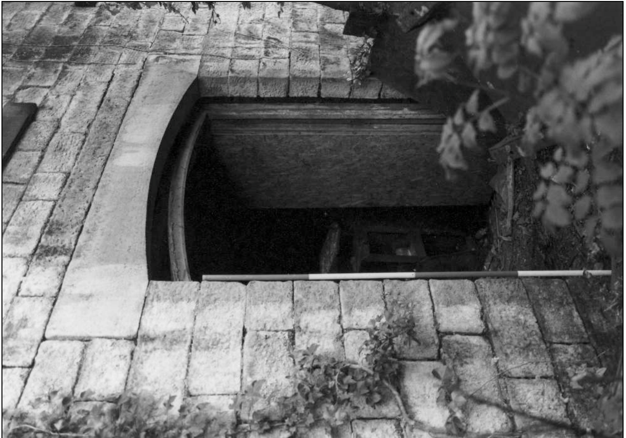
Photo 35: Ground floor doorway in east side of boiler house (film 3, frame 15)
