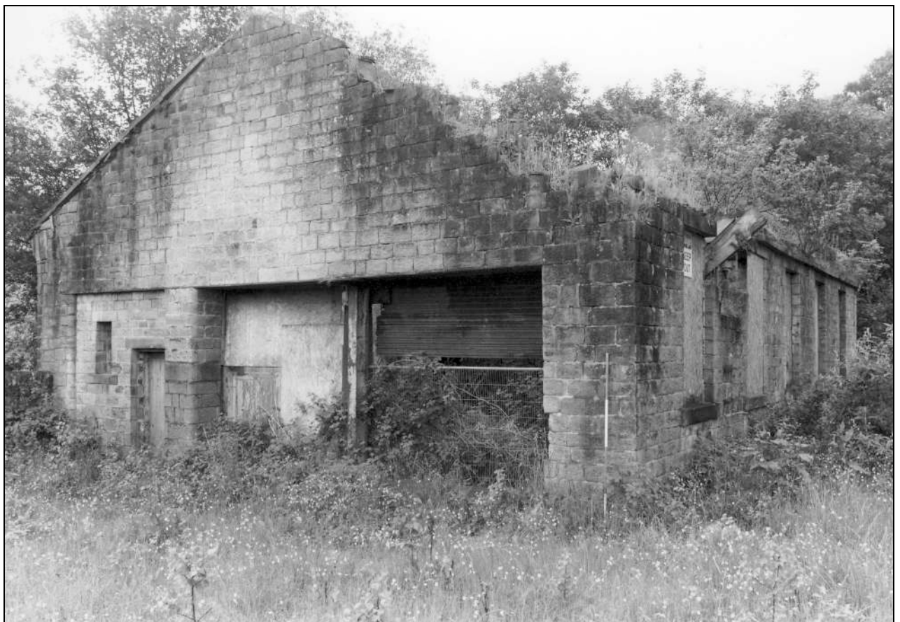
Photo 30: Boiler house, from the north-west (film 4, frame 6)
