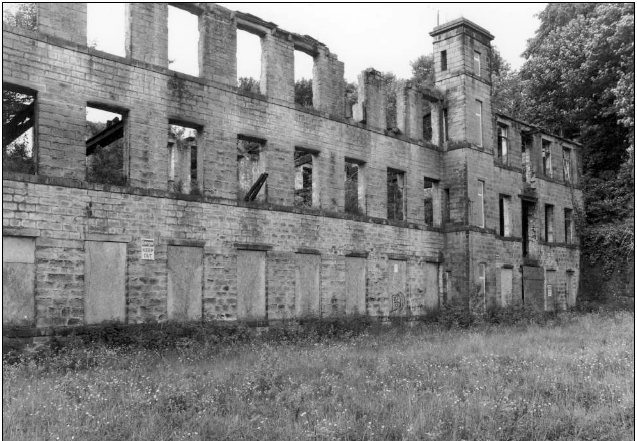
Photo 2: The spinning mill, from the north-east (film 1, frame 4)
