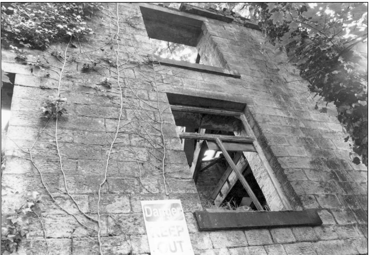
Photo 34: Upper windows in east side of boiler house (film 3, frame 16)
