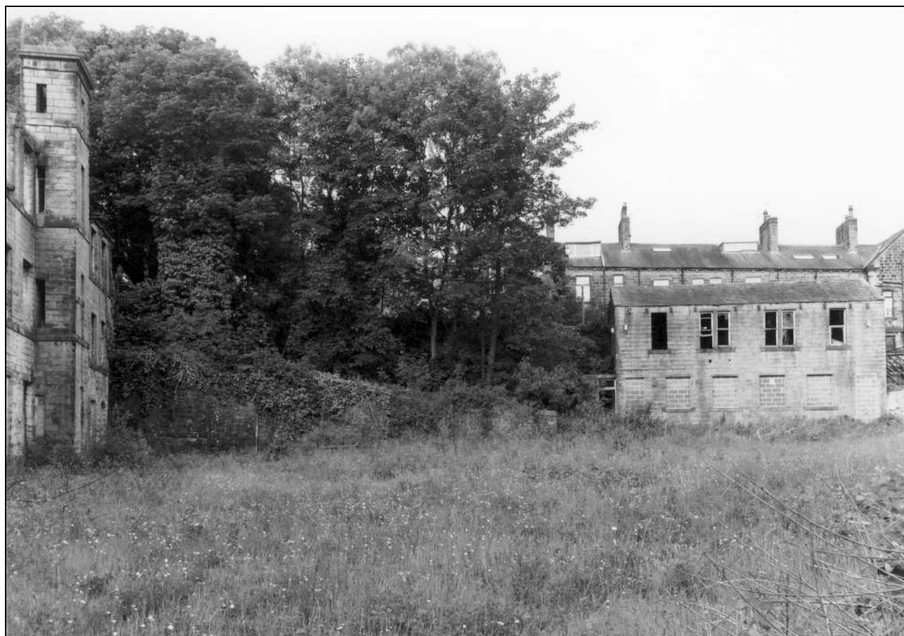
Photo 44: Offices at north-west corner of site, from the east (film 1, frame 10)
