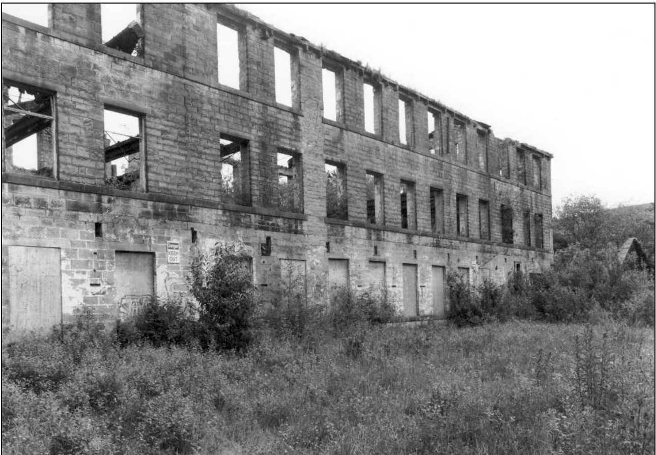
Photo 9: Spinning mill: south elevation, from the south-west (film 3, frame 1)
