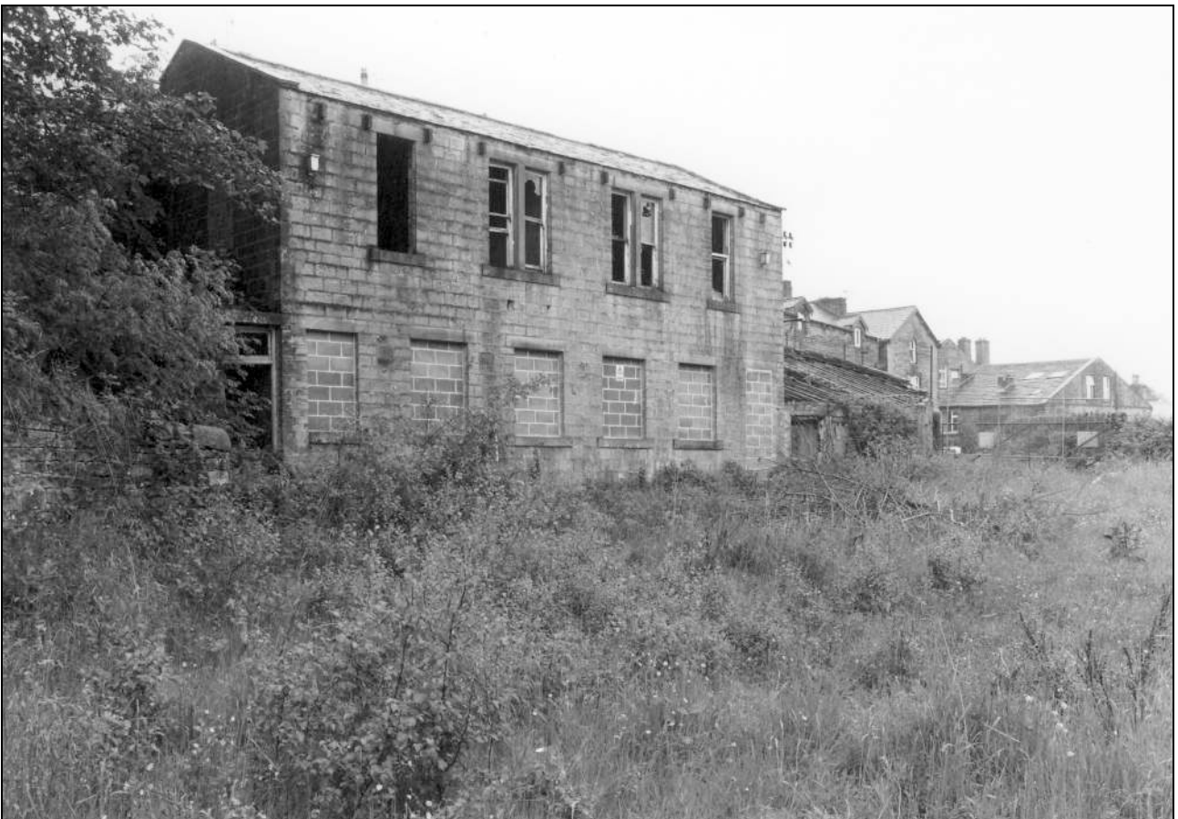
Photo 46: Offices and cart shed, from the south-east (film 4, frame 7)
