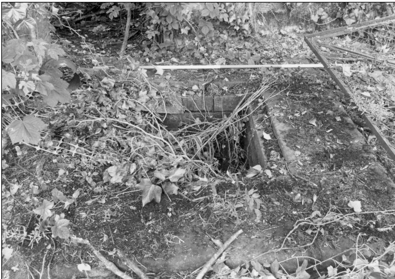
Photo 43: Man-hole over culvert forming outfall from mill pond (film 3, frame 12)
