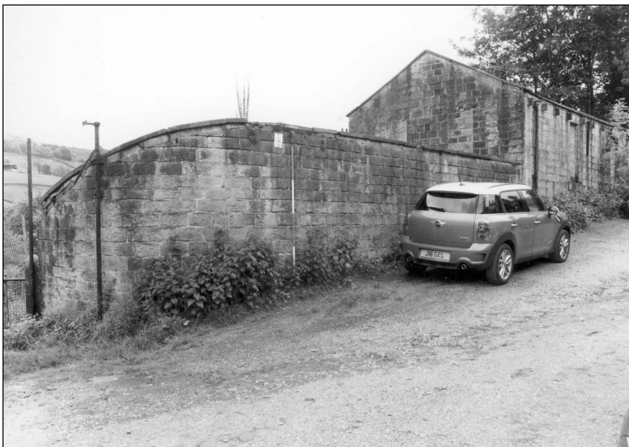
Photo 50: Rear of cart shed, from the north-west (film 4, frame 10)
