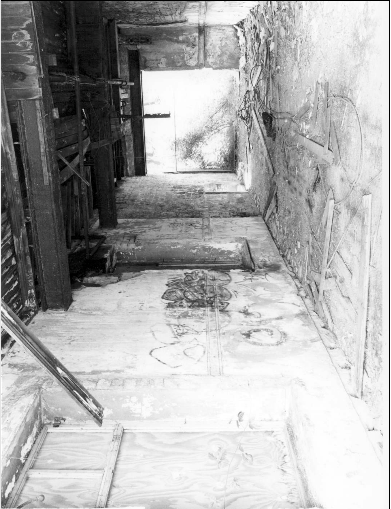
Photo 16: Horizontal engine room, from the north (film 1, frame 16)
