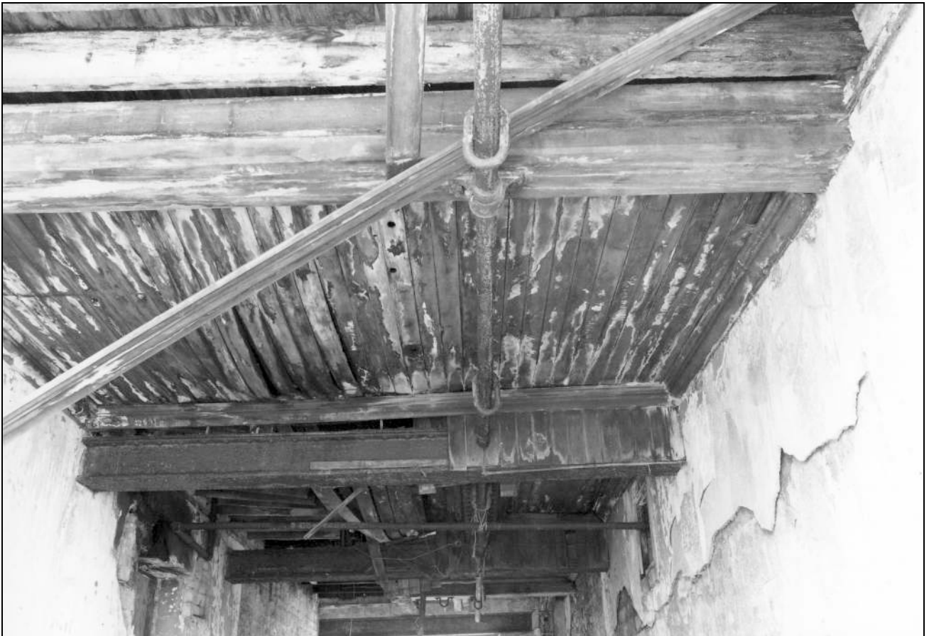
Photo 15: Ceiling over horizontal engine room, from the north (film 1, frame 17)
