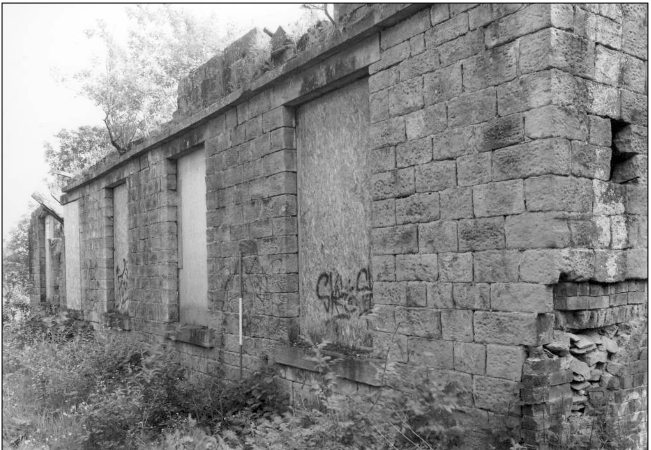
Photo 32: West side of boiler house, from the south-west (film 2, frame 10)
