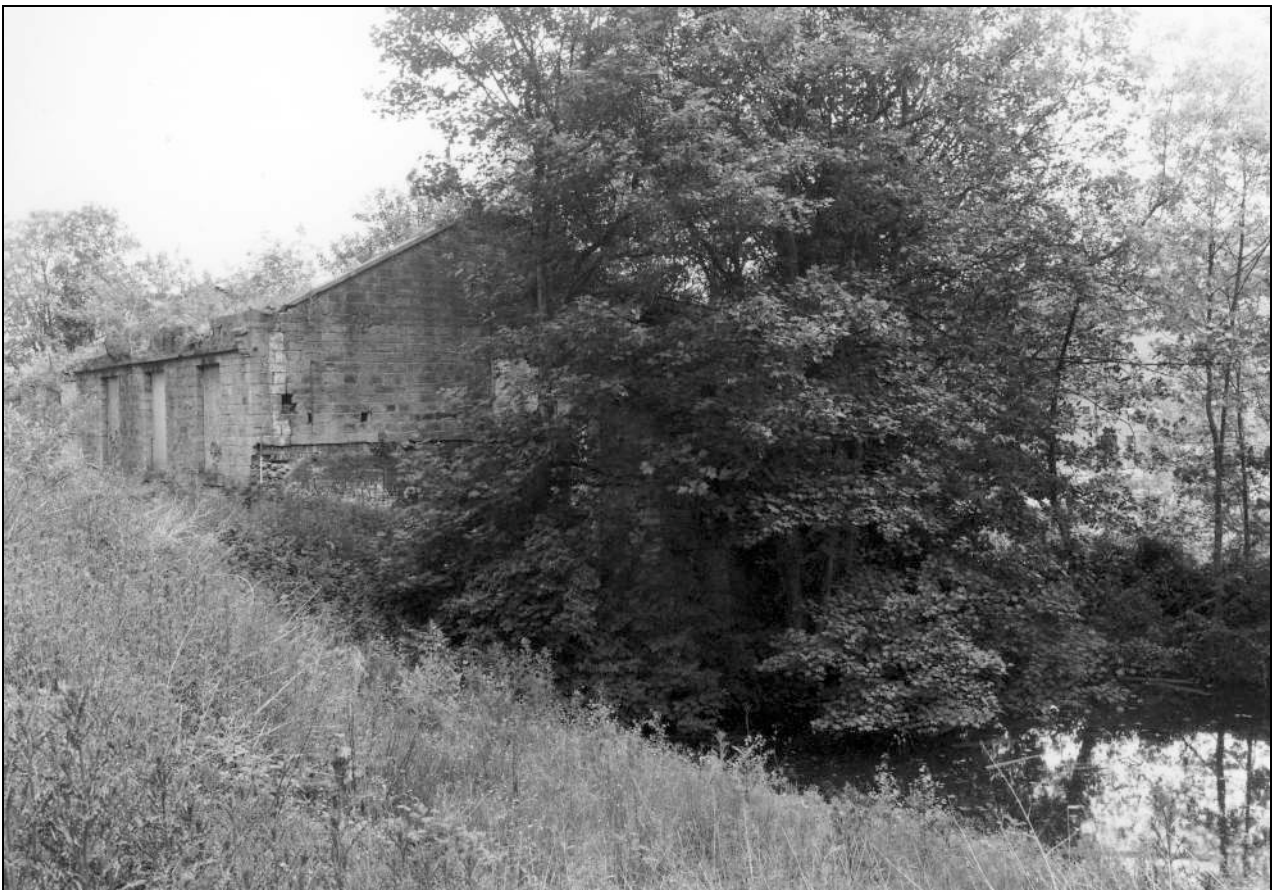
Photo 36: Boiler house and mill pond, from the south-west (film 2, frame 15)
