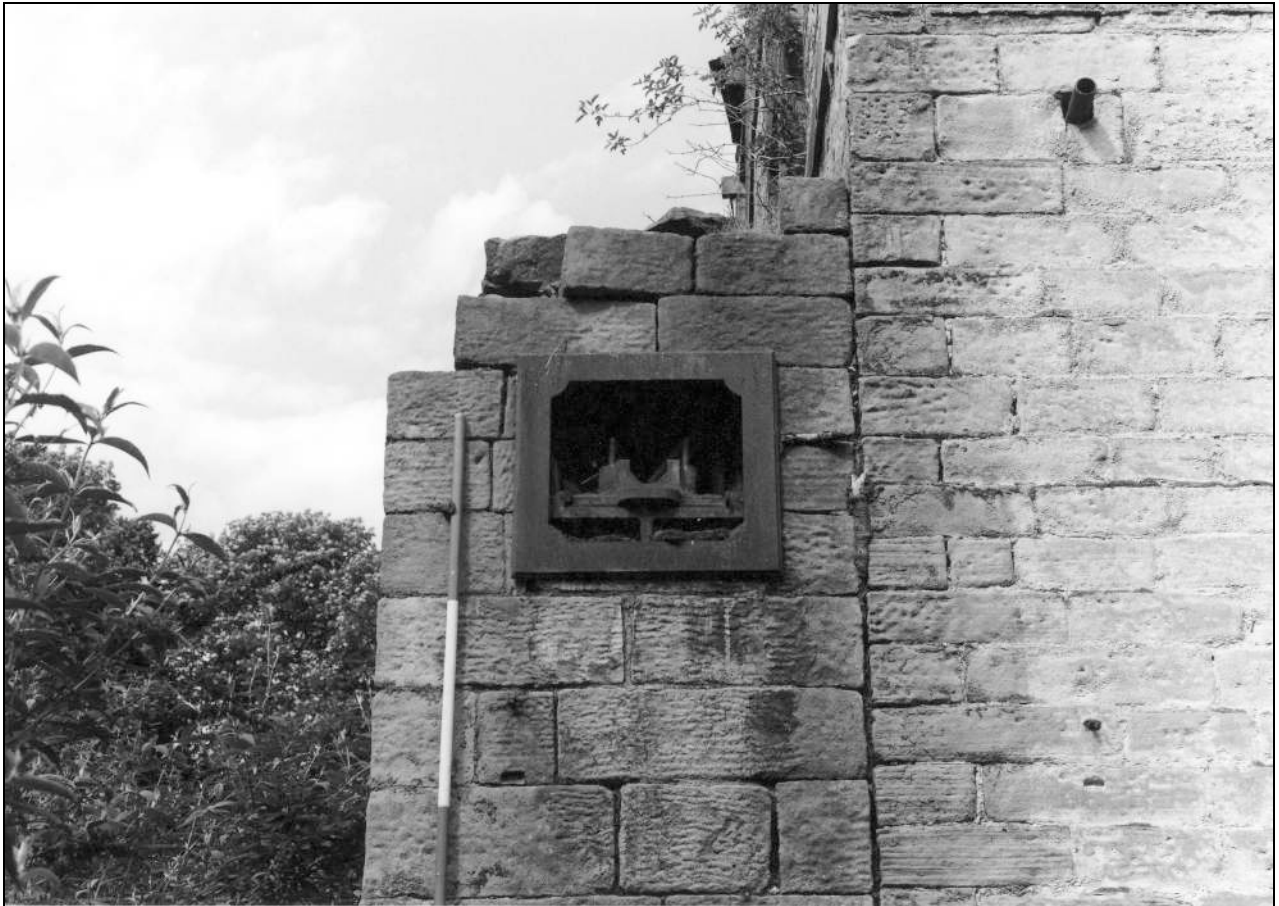
Photo 25: Wall bearing in east side of former weaving shed (film 2, frame 5)
