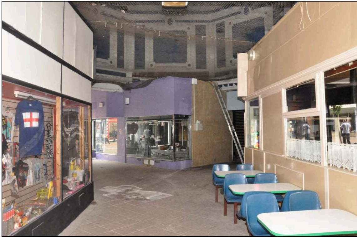
Photo 15: Existing shop fronts within arcade, Leeds Road end
