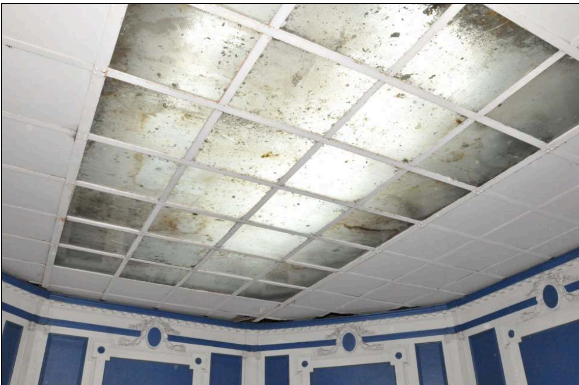
Photo 20: Ceiling light within atrium
