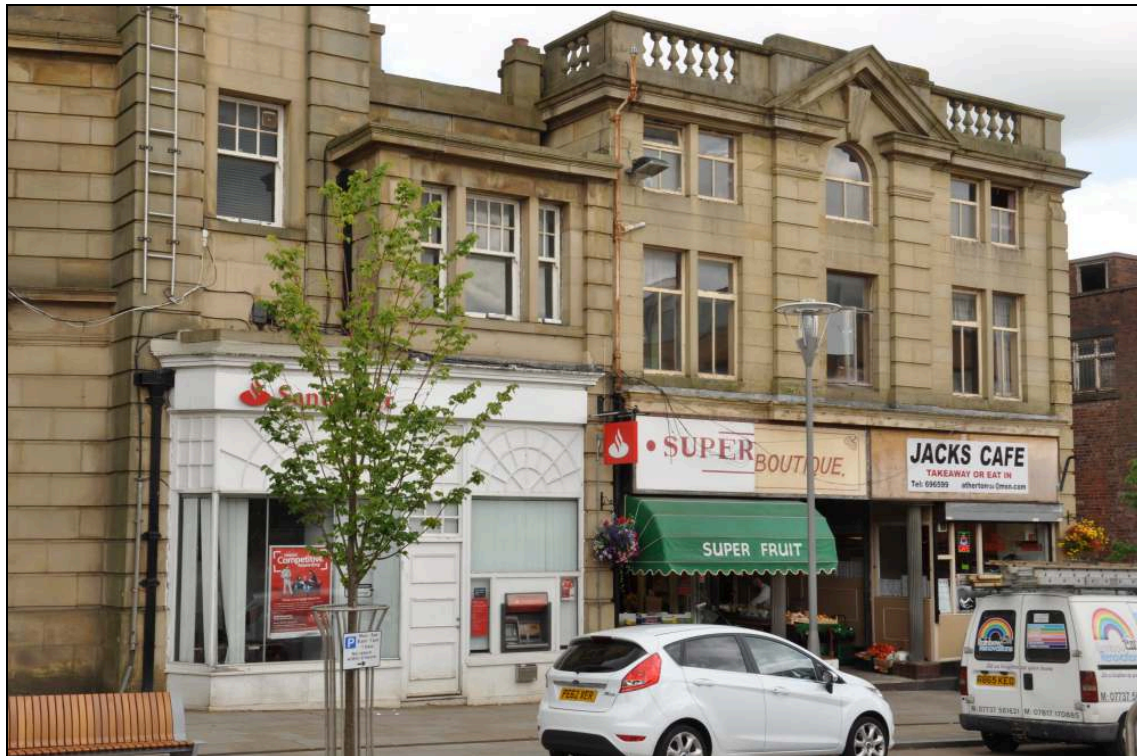
Photo 3: Union Bank building: Leeds Road frontage to arcade
