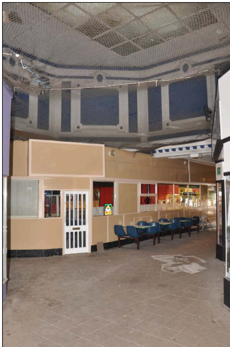
Photo 16: Atrium within arcade, from Scotland Road end
