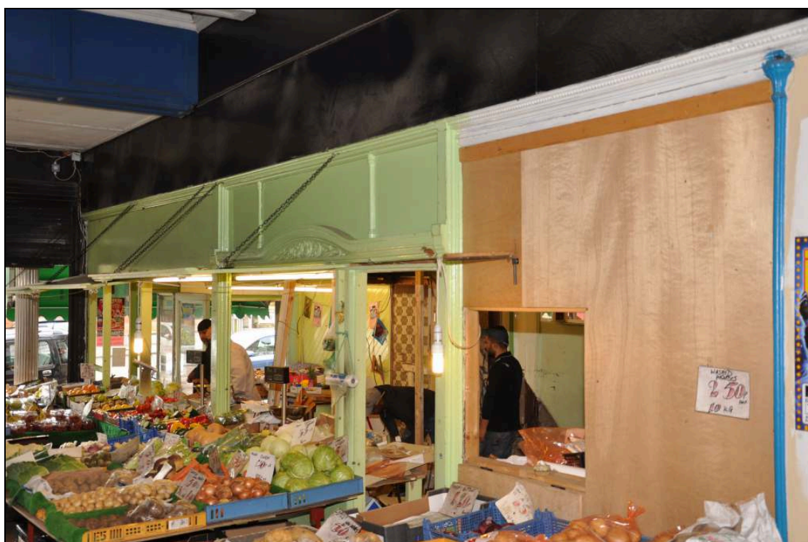
Photo 10: Existing shop fronts within arcade, Leeds Road end
