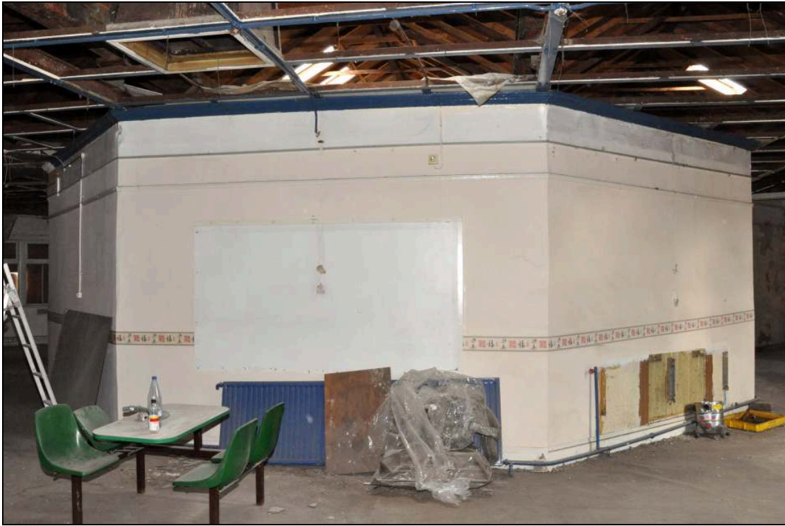
Photo 29: Outer face of atrium, at upper floor level
