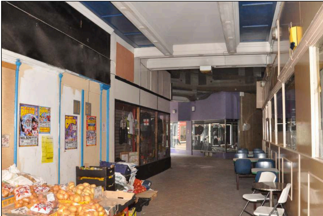
Photo 13: Existing shop fronts within arcade, Leeds Road end
