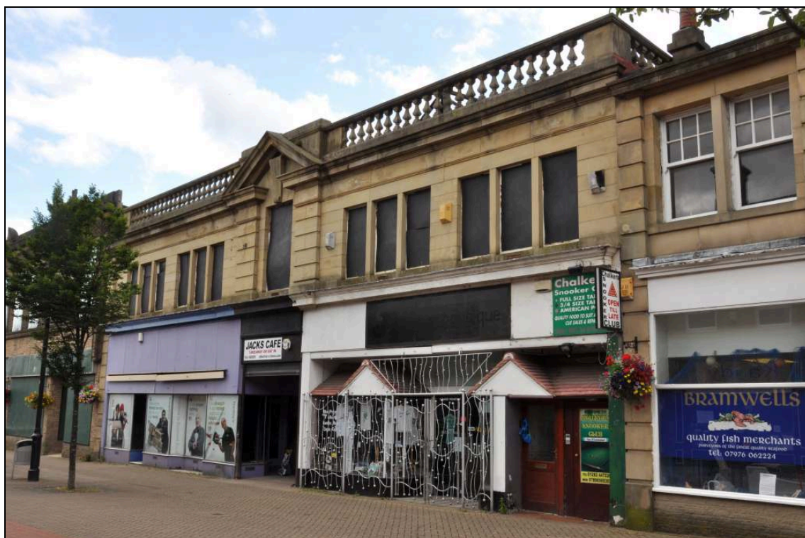
Photo 6: Union Bank building: Scotland Road frontage to arcade
