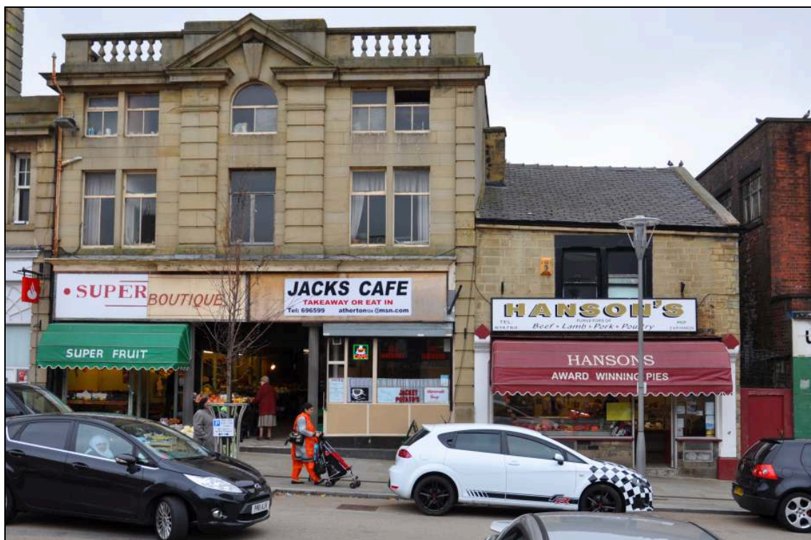
Photo 4: Union Bank building: Leeds Road frontage to arcade, and 11 Leeds Road
