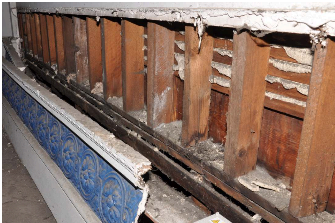
Photo 28: Detail of panelling and studwork within upper part of atrium
