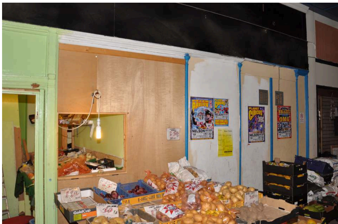
Photo 12: Existing shop fronts within arcade, Leeds Road end
