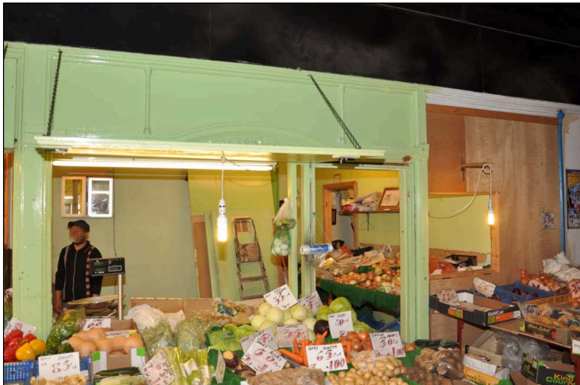
Photo 11: Existing shop fronts within arcade, Leeds Road end
