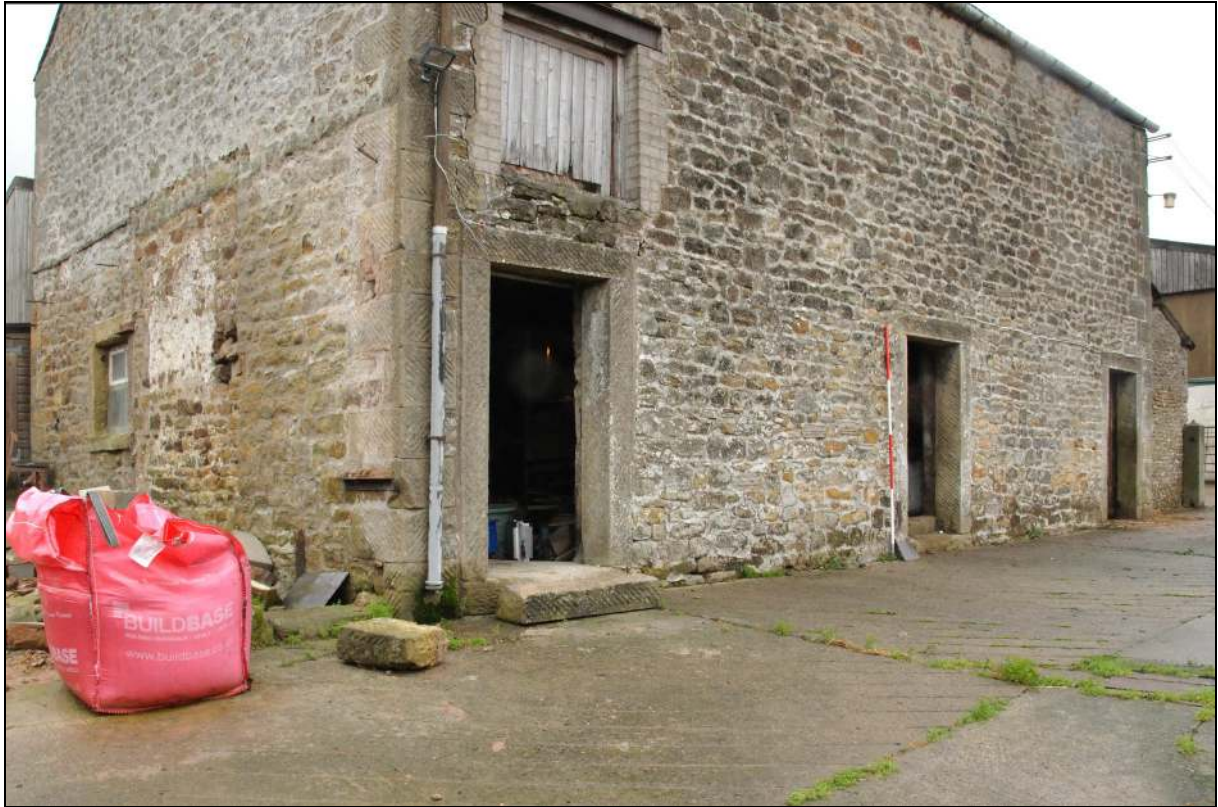
Photo 5: West elevation, from the north-west
