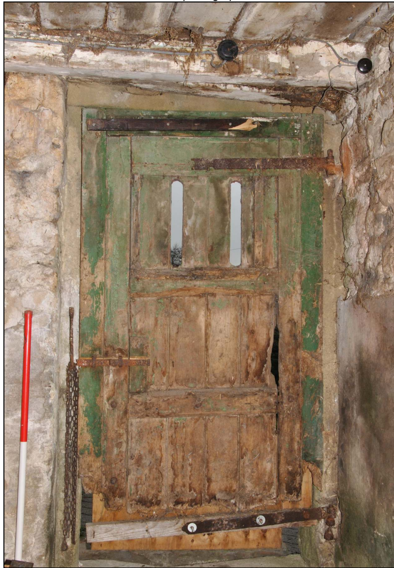
Photo 19: Rear of door to north shippon, from the west
