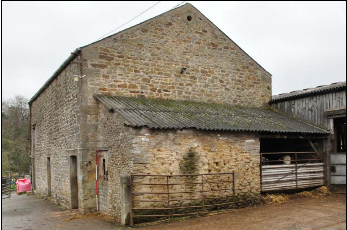
Photo 12: South gable with later lean-to
