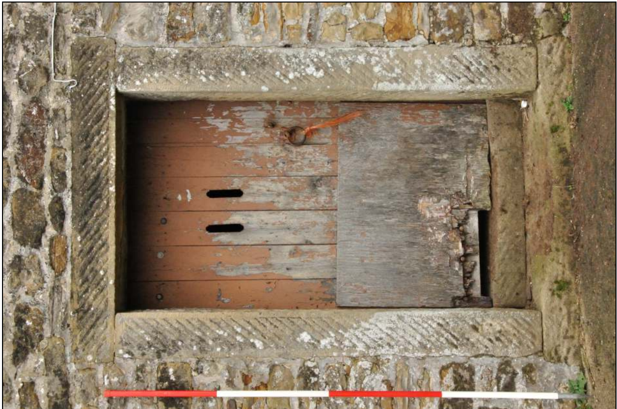
Photo 9: Detail of central doorway, west side of barn
