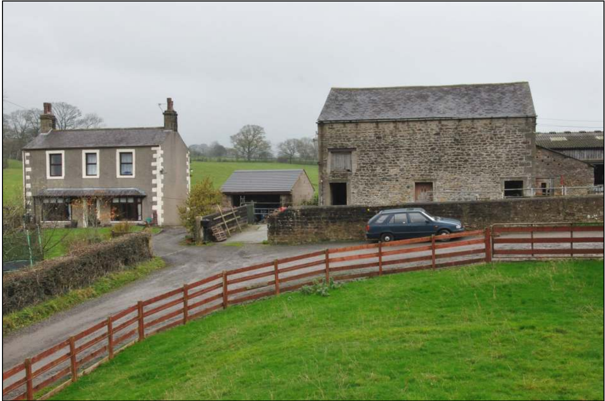
Photo 1: General view of the farmhouse and barn, from the west
