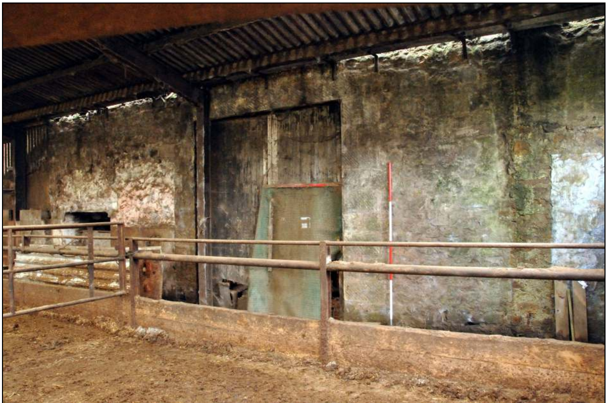
Photo 3: East elevation of the barn, within modern shed
