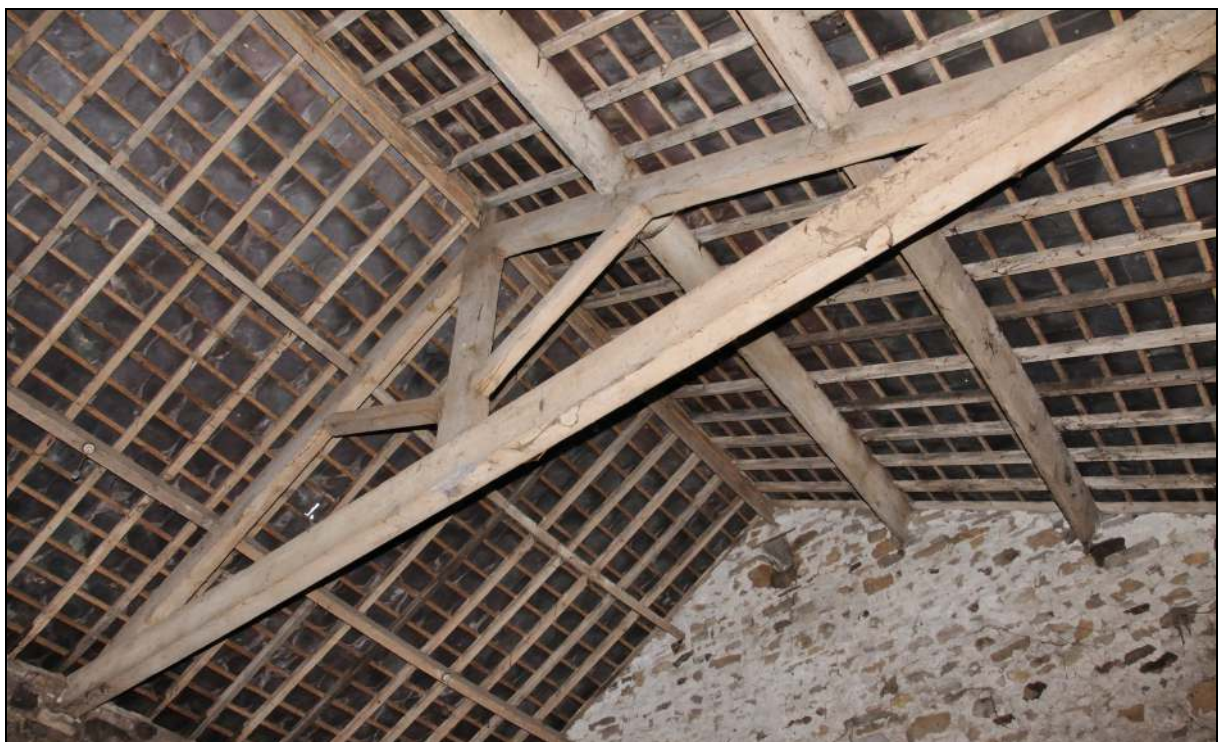
Photo 20: North roof truss, from the south-east
