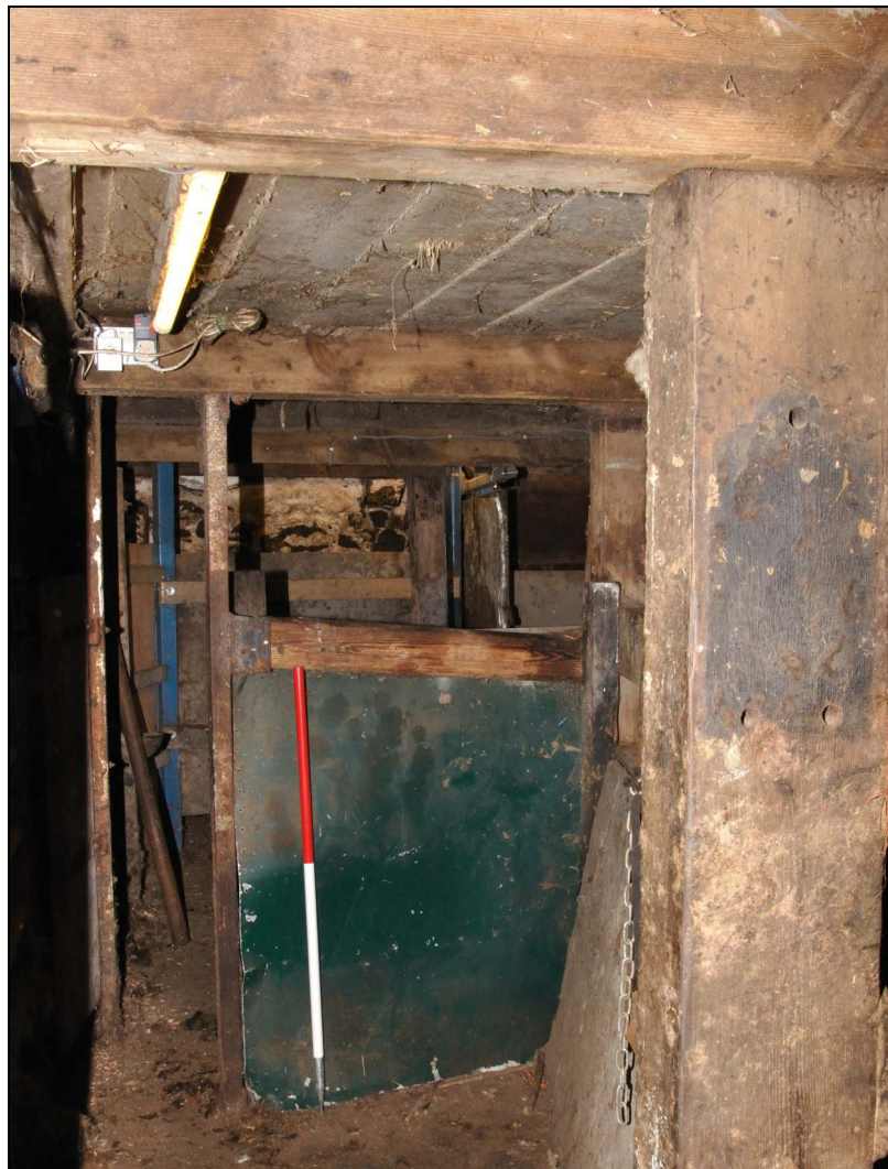
Photo 17: Remains of timber boskins in south shippon, from the west
