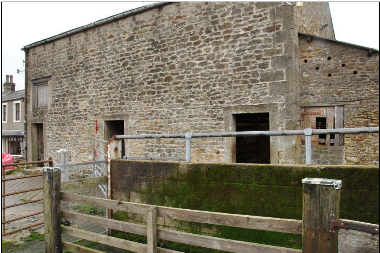
Photo 7: West elevation, from the south-west
