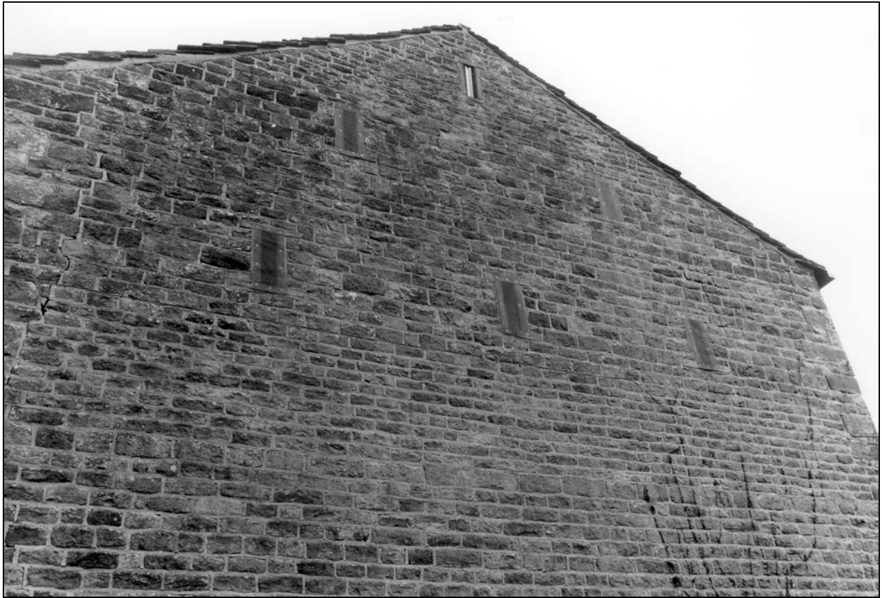
Photo 18: Detail of high level breathers in west gable (film 1, frame 11)
