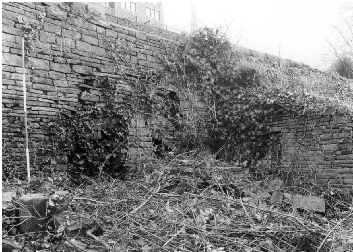
Photo 15: Remains of arch in retaining walls and adjoining buildings, to north of barn (film 2, frame 4)
