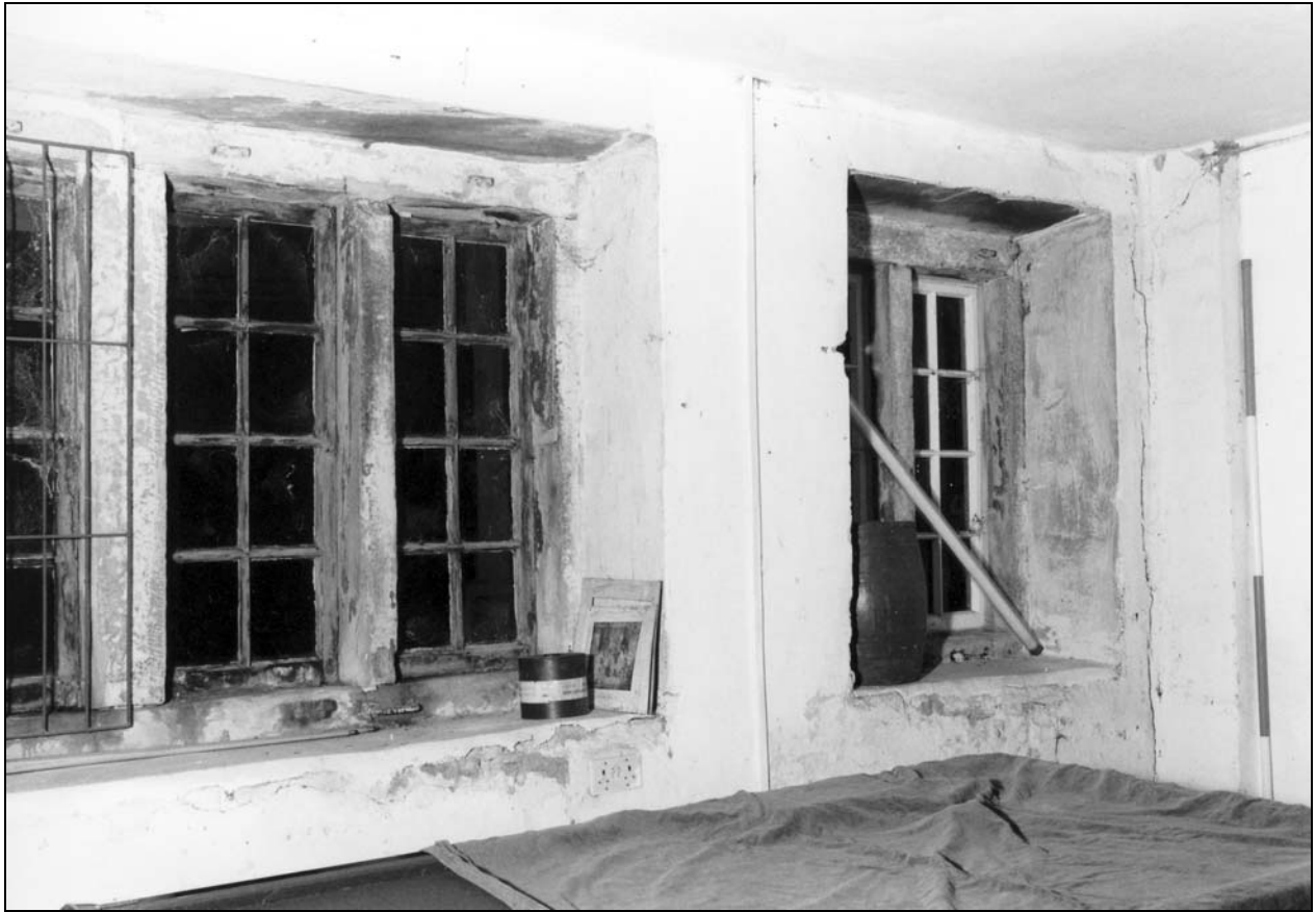
Photo 55: Internal view of first floor windows in workshop, south side (film 4, frame 2)
