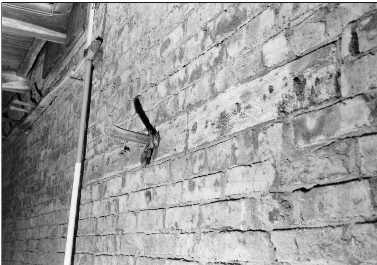
Photo 38: Detail of original timber for harness pegs in east side of central bay (later pegs to top left) (film 3, frame 11)
