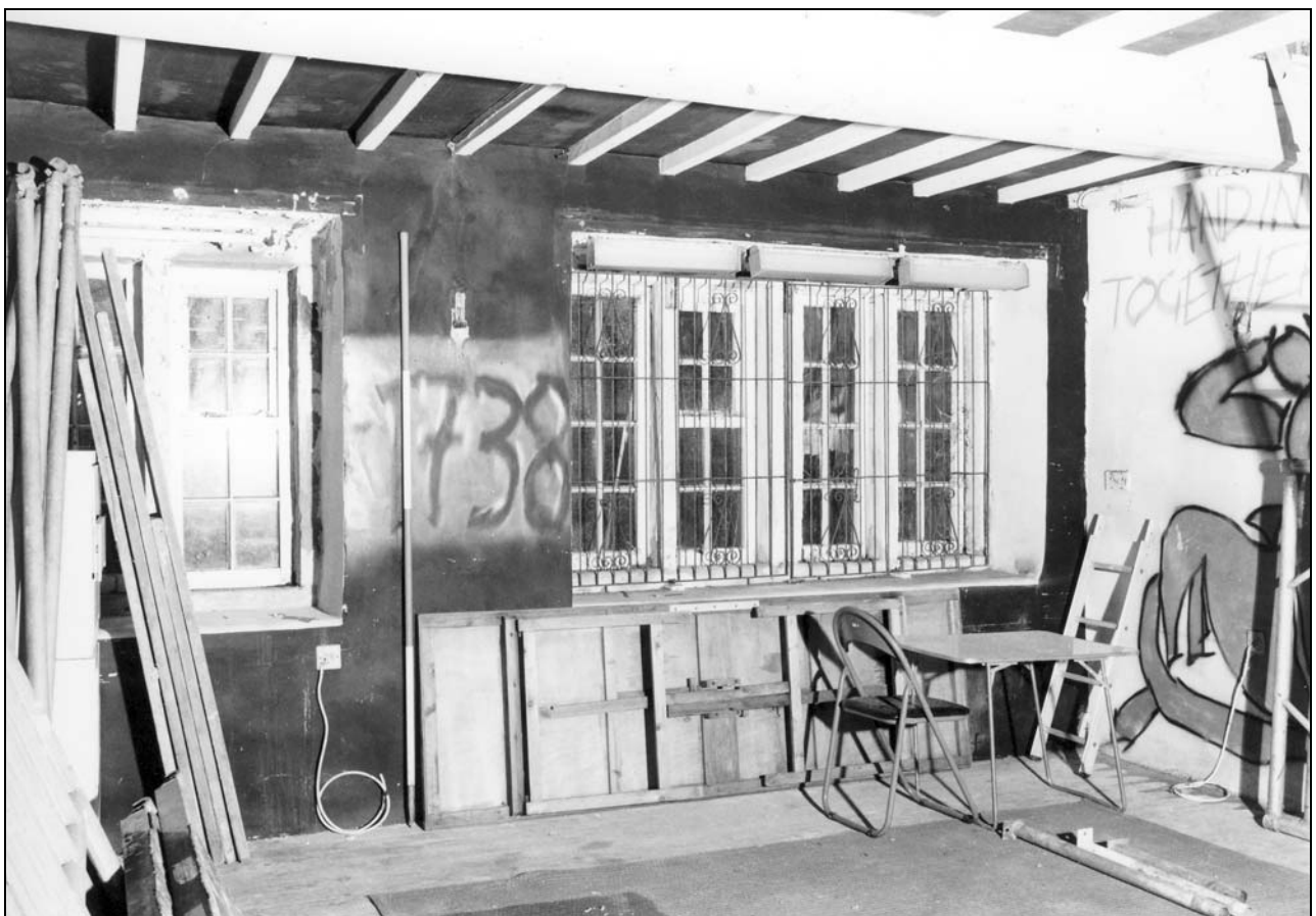
Photo 56: First floor of workshop (north part), from the south-west (film 4, frame 7)
