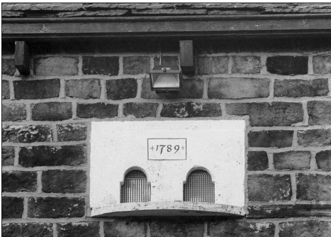
Photo 5: Detail of date-stone and landing ledge to pigeon loft, front elevation (film 1, frame 1)
