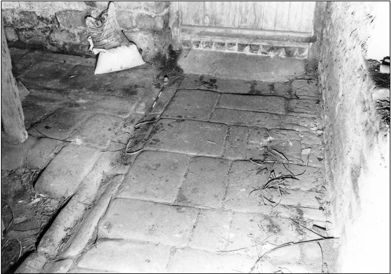
Photo 23: Detail of floor to passage with drain, in stable (film 2, frame 18)
