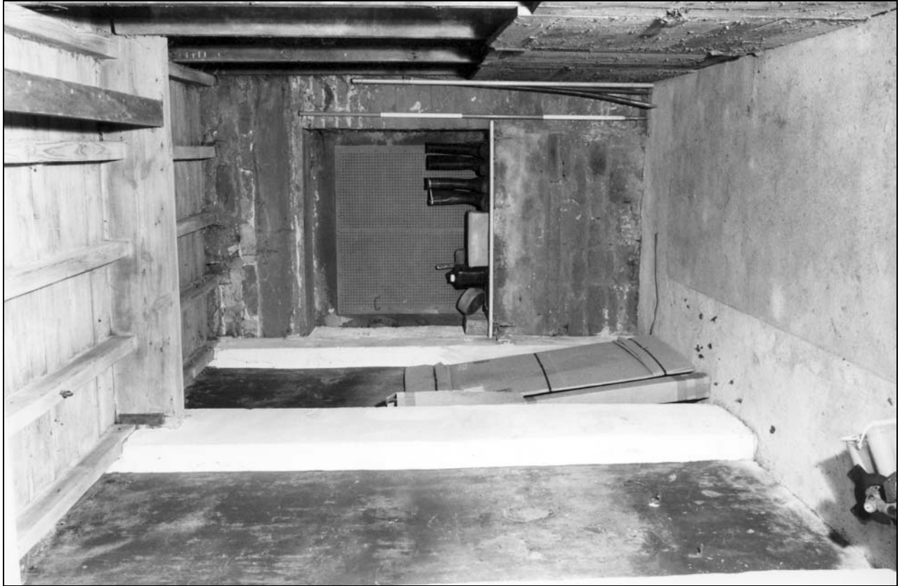
Photo 49: Ground floor of workshop: north-west corner (blocked doorway) (film 5, frame 2)
