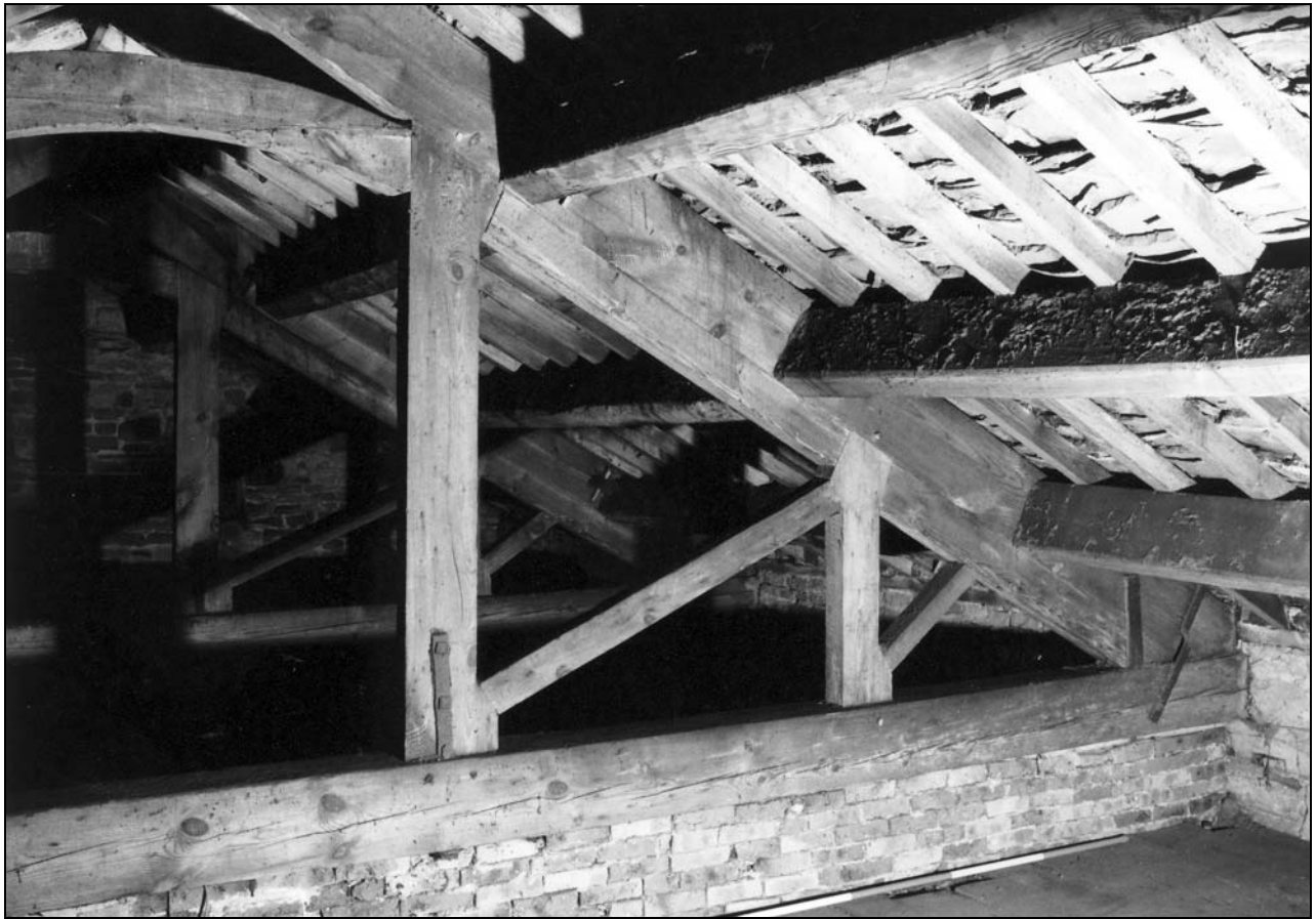
Photo 64: The east roof truss (north part), from the south-east (film 4, frame 16)
