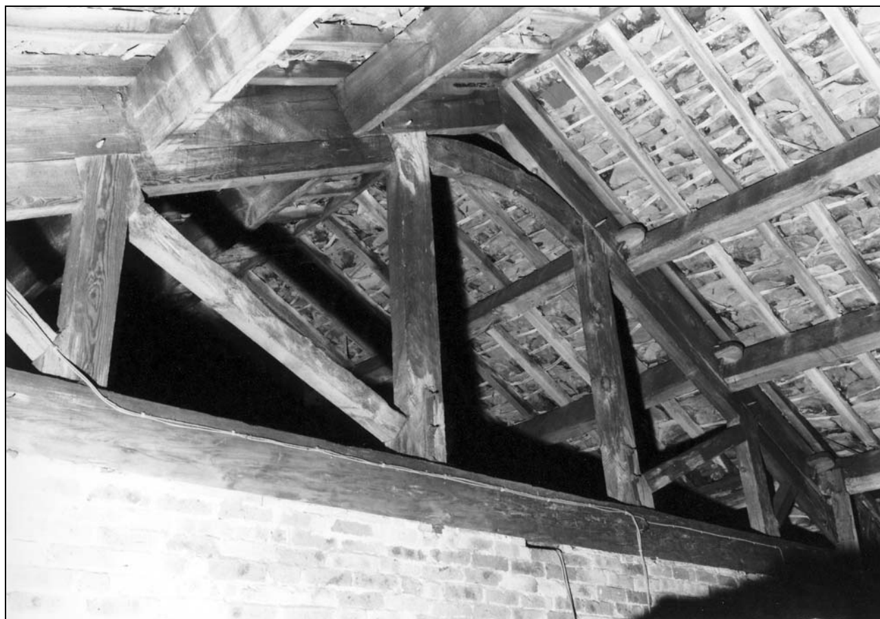
Photo 60: The east roof truss, from the north-west (film 4, frame 1)
