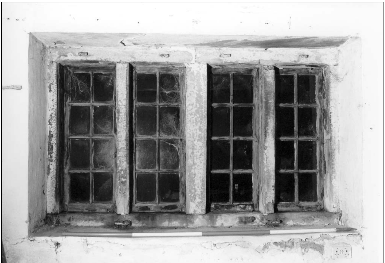
Photo 54: Internal view of first floor window in workshop (south side), showing hinge pintles and barring staples (film 4, frame 4)
