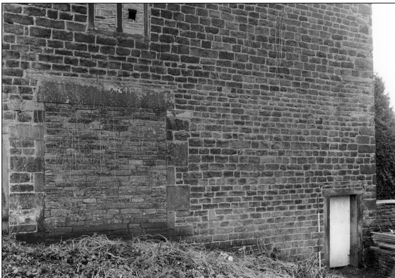
Photo 13: West end of rear (north) elevation (film 2, frame 6)
