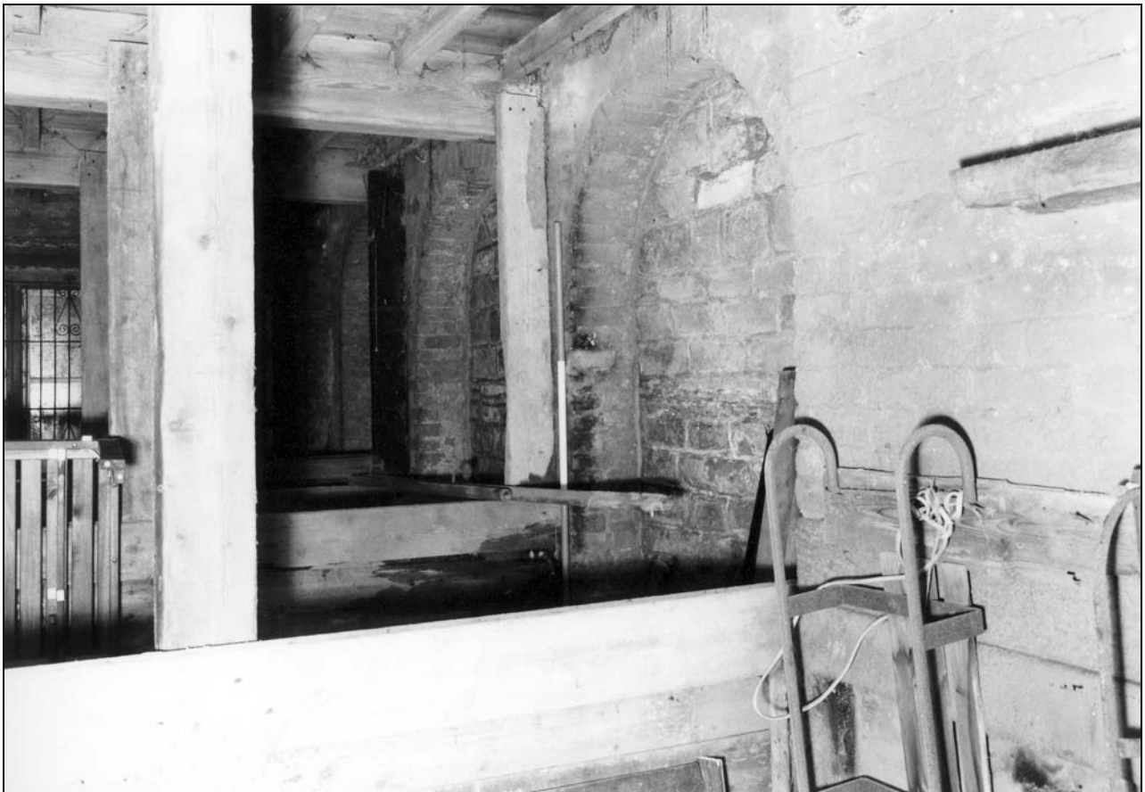
Photo 46: Ground floor of workshop, from the south-west (film 5, frame 5)
