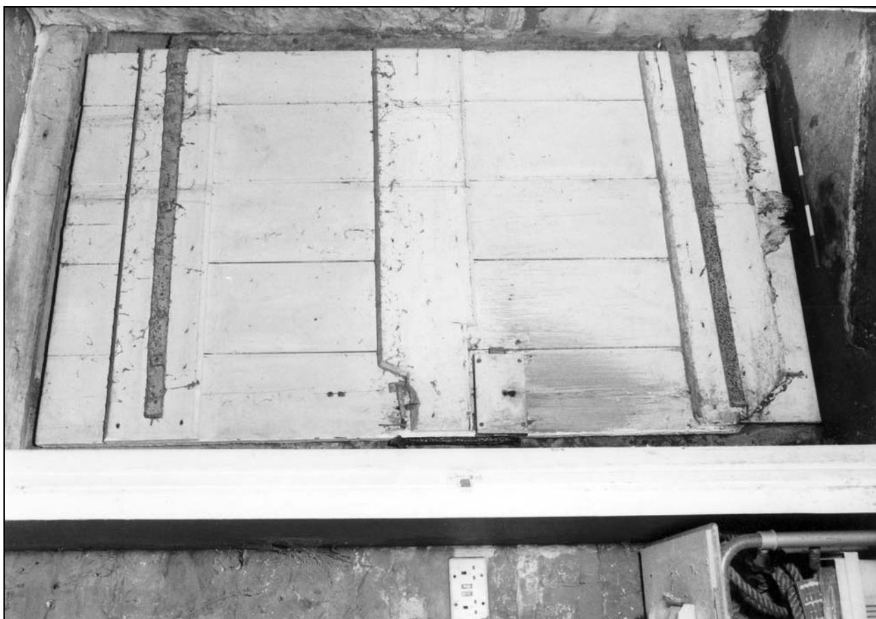
Photo 43: Internal view of north door to workshop (film 4, frame 18)
