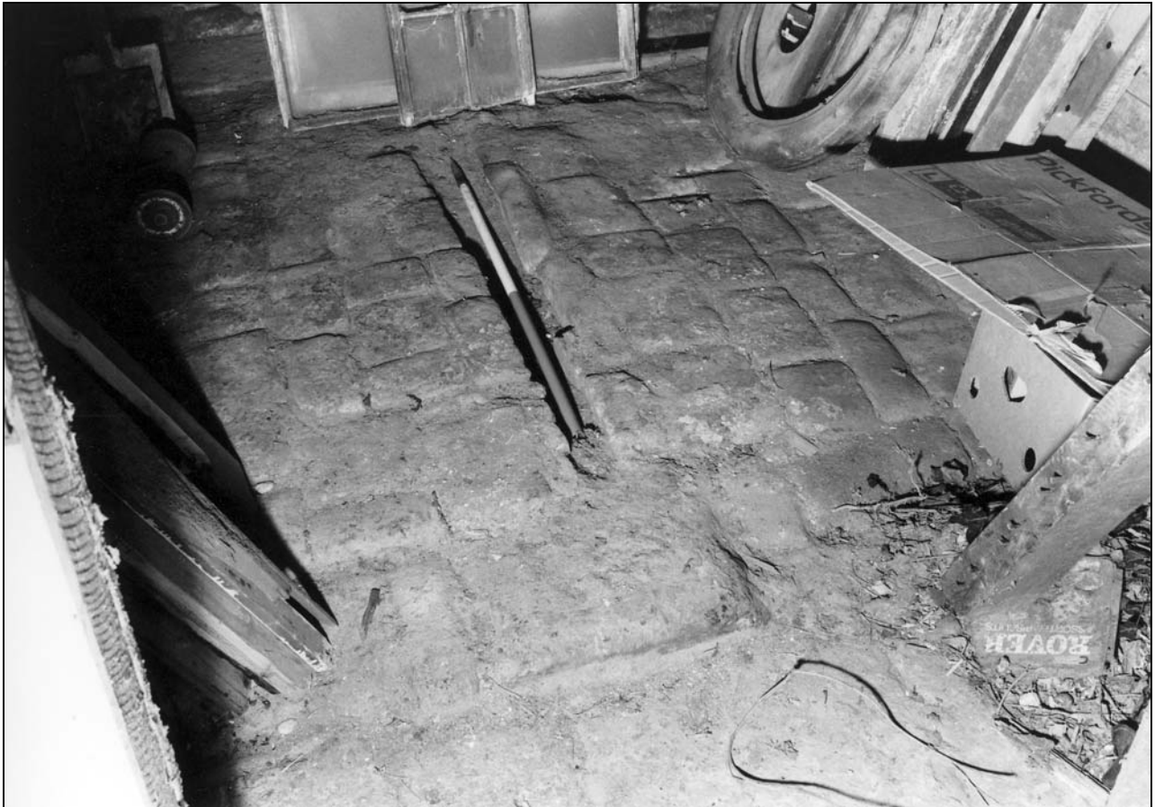
Photo 27: Detail of floor in former shippon, from the west (film 2, frame 13)
