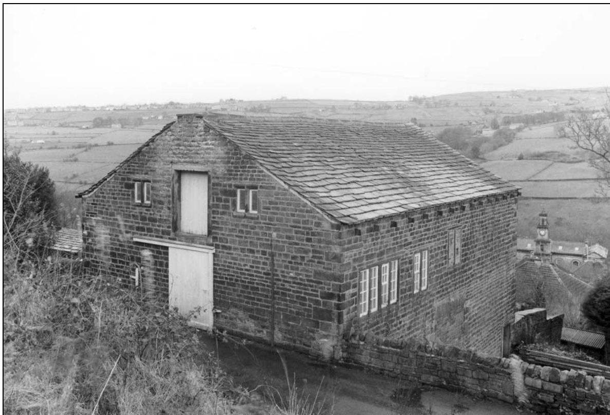
Photo 7: General view, from the north-east (film 2, frame 9)
