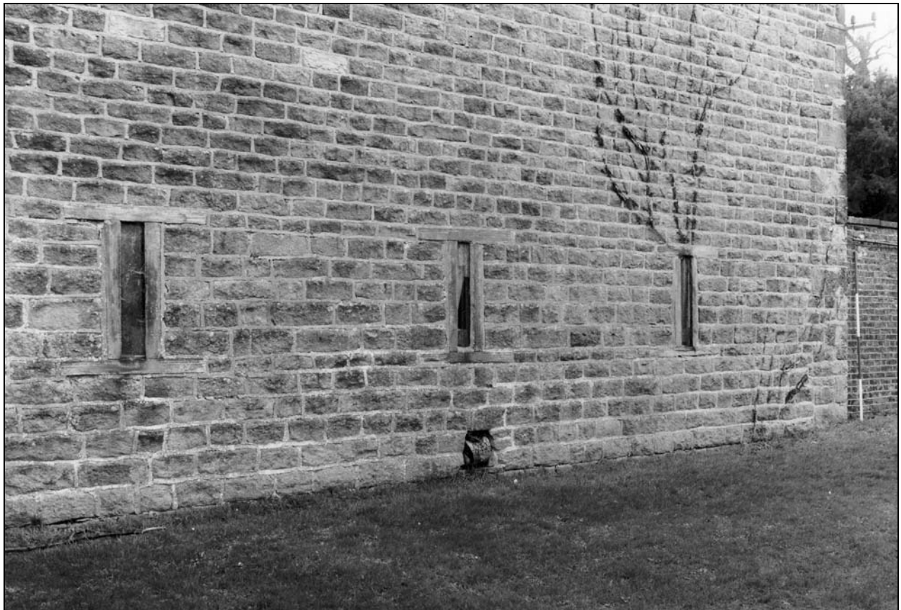
Photo 17: Detail of breathers at foot of west gable (film 1, frame 10)
