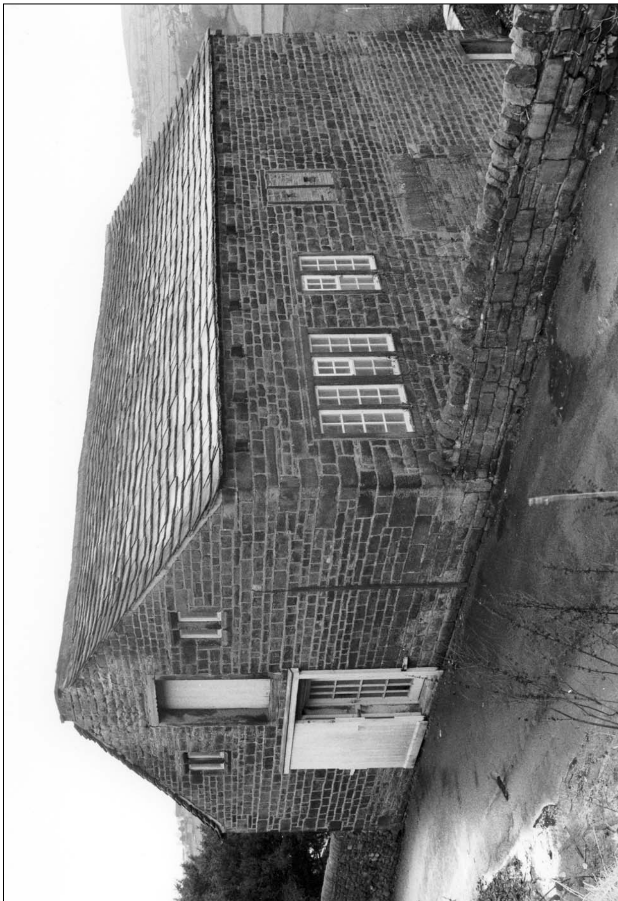
Photo 8: General view, from the north-east (film 1, frame 18)
