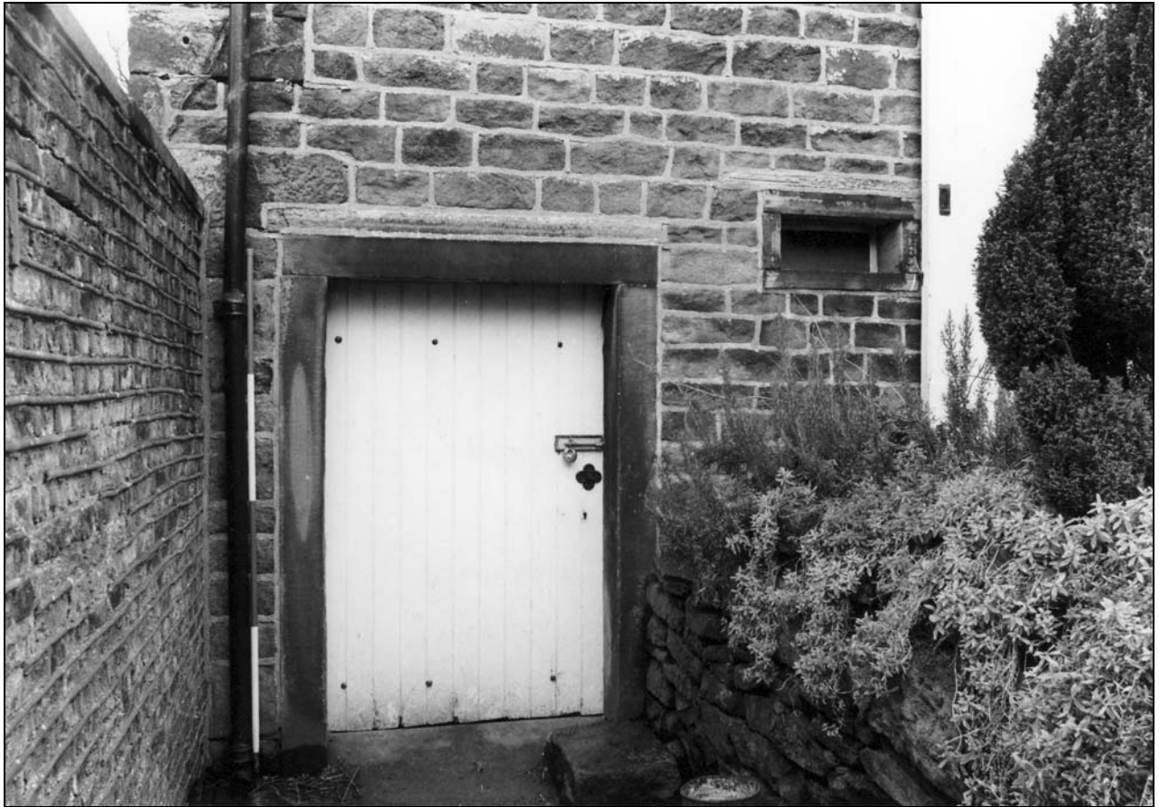
Photo 2: Doorway to stable in west end of front elevation (film 1, frame 8)
