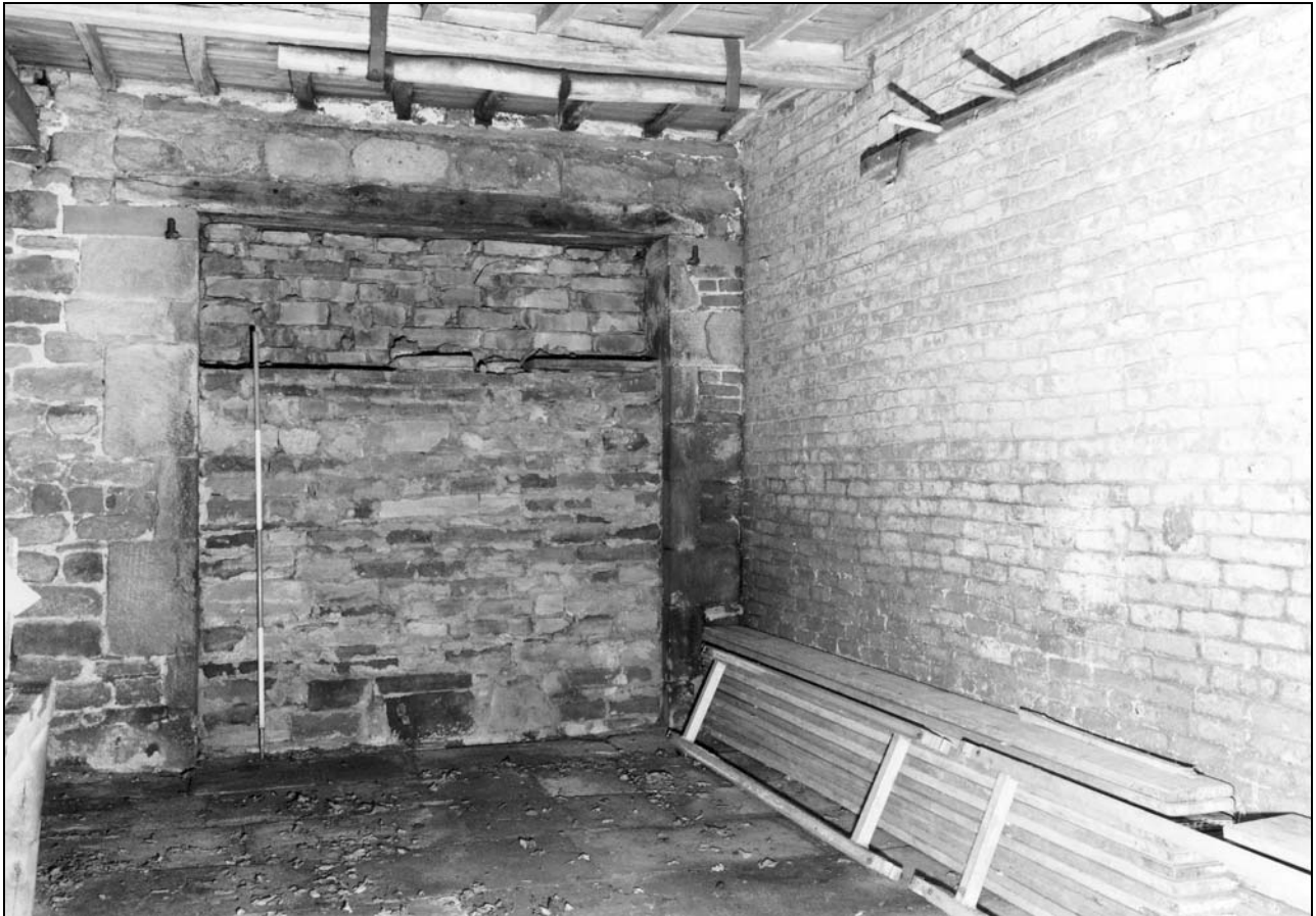
Photo 35: Blocked north doorway to central bay, with later harness pegs to right (film 3, frame 3)
