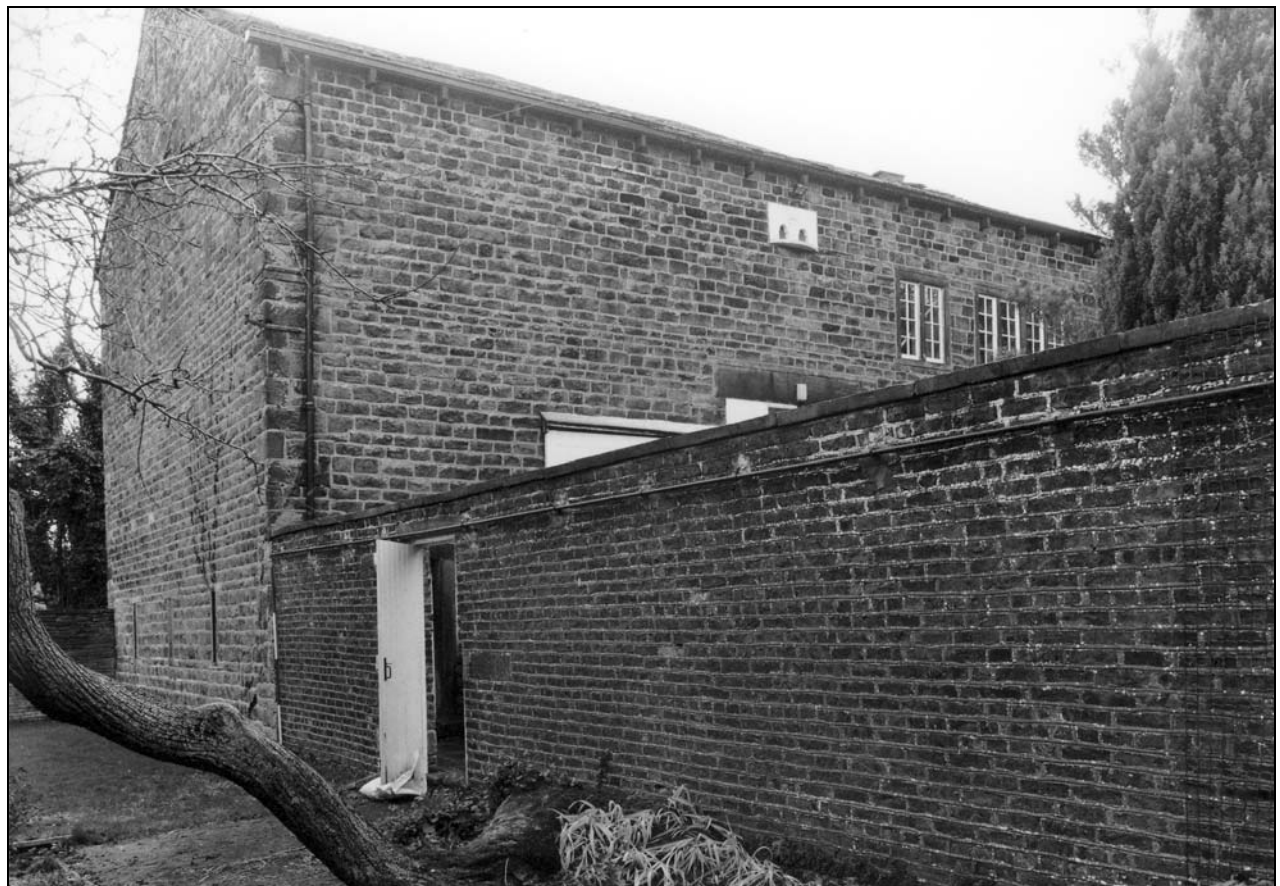
Photo 19: General view from the south-west, showing adjoining garden wall (film 1, frame 9)
