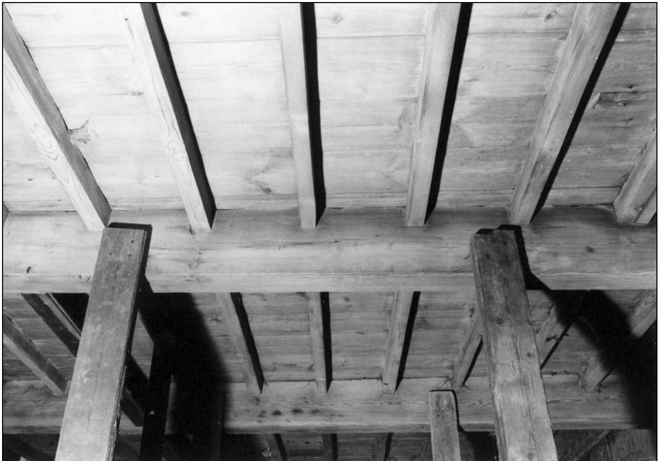
Photo 50: Underside of first floor of workshop, from the south (film 5, frame 9)
