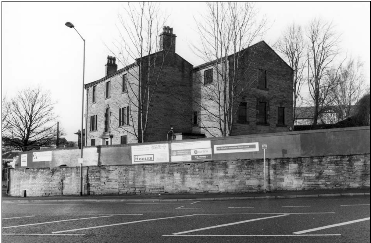
Photo 12: General view, from the south-east (film 4, frame 17)
