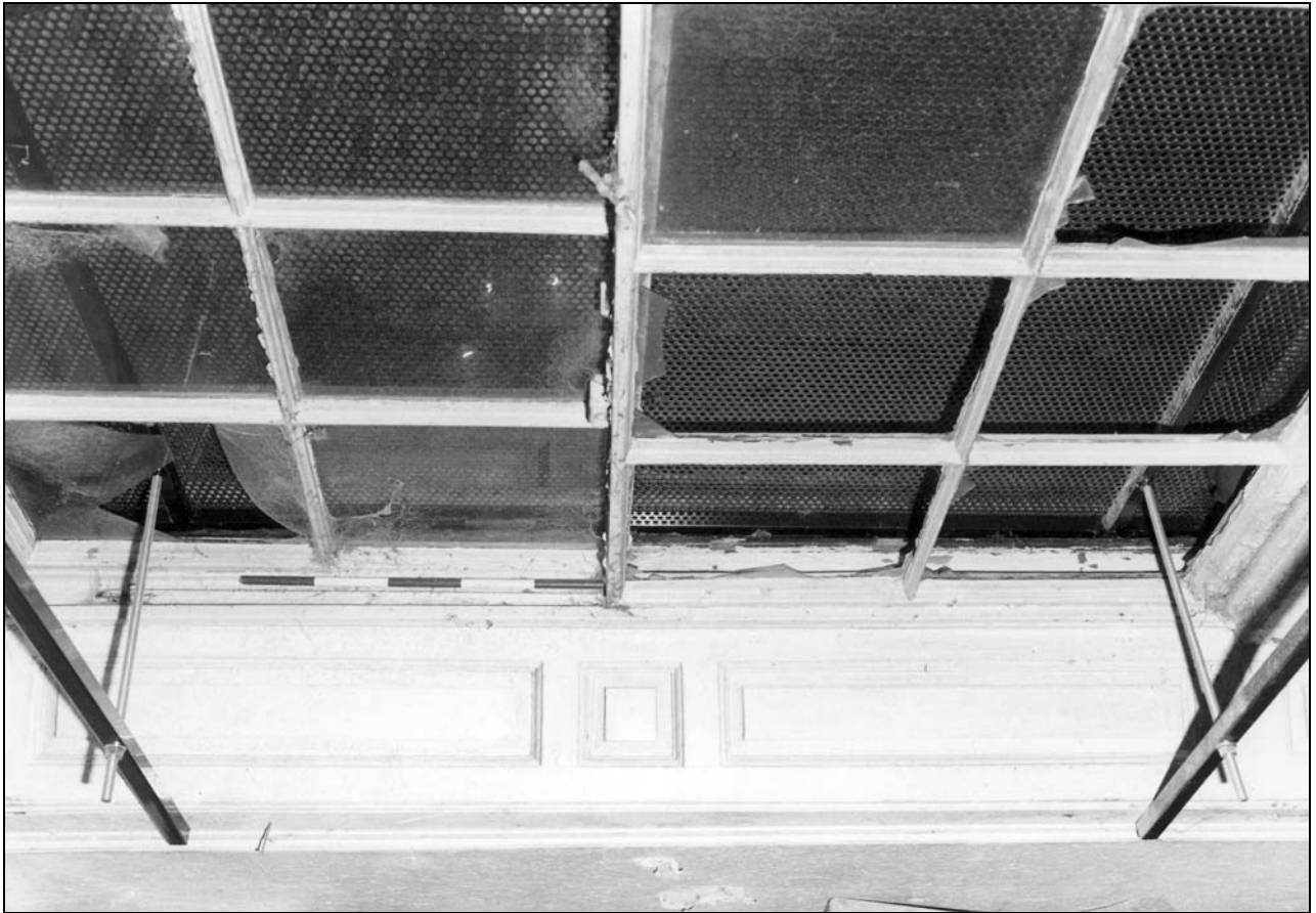
Photo 53: North wing: detail of window in kitchen G05 (film 3, frame 5)
