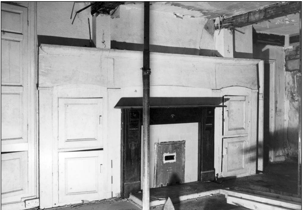
Photo 54: North wing: former cooking range in kitchen G05 (film 3, frame 9)
