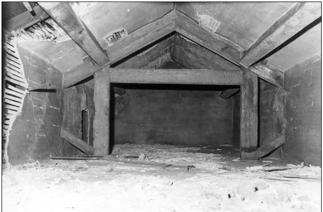
Photo 80: North wing: attic and roof truss, from the east (film 6, frame 13)
