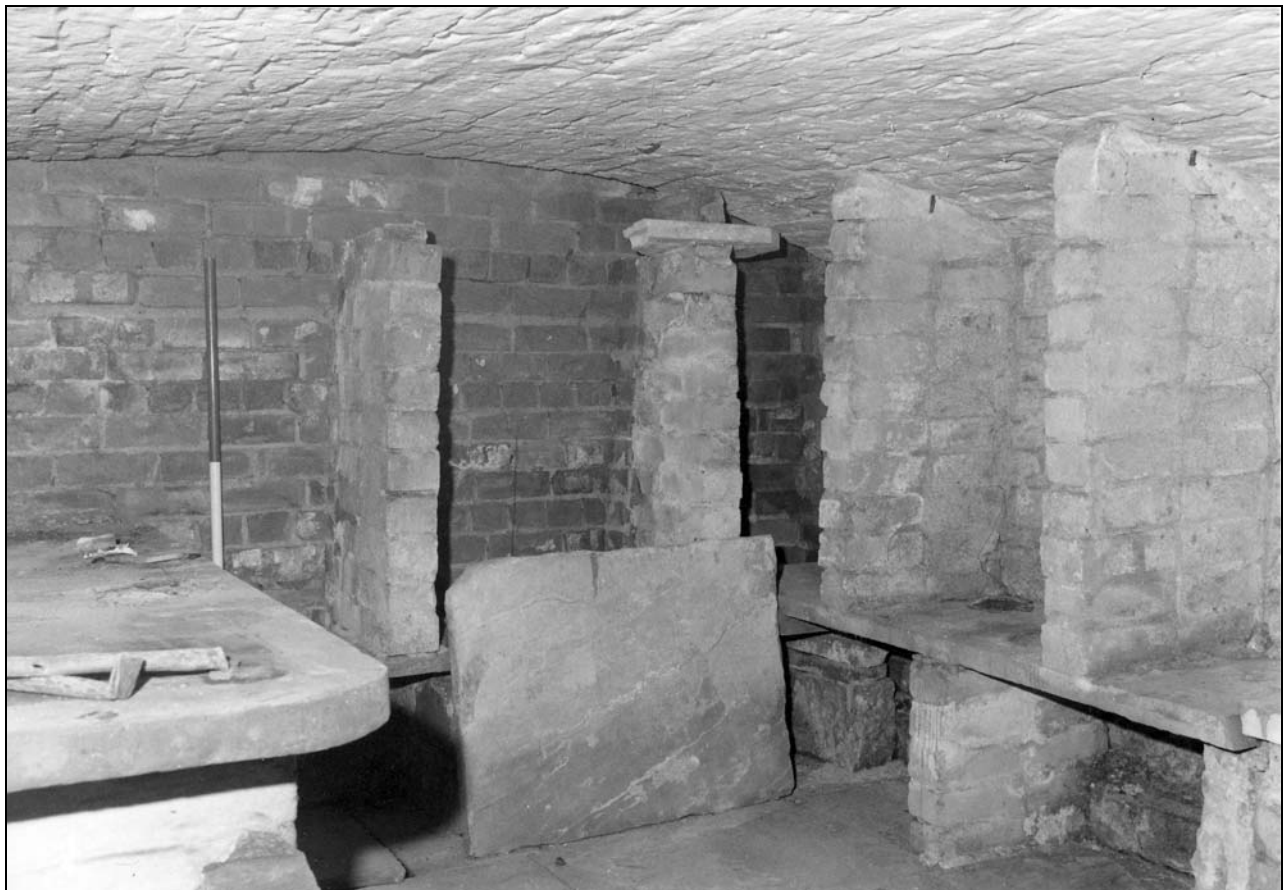
Photo 38: South wing: cellar B02, from the north (film 1, frame 7)
