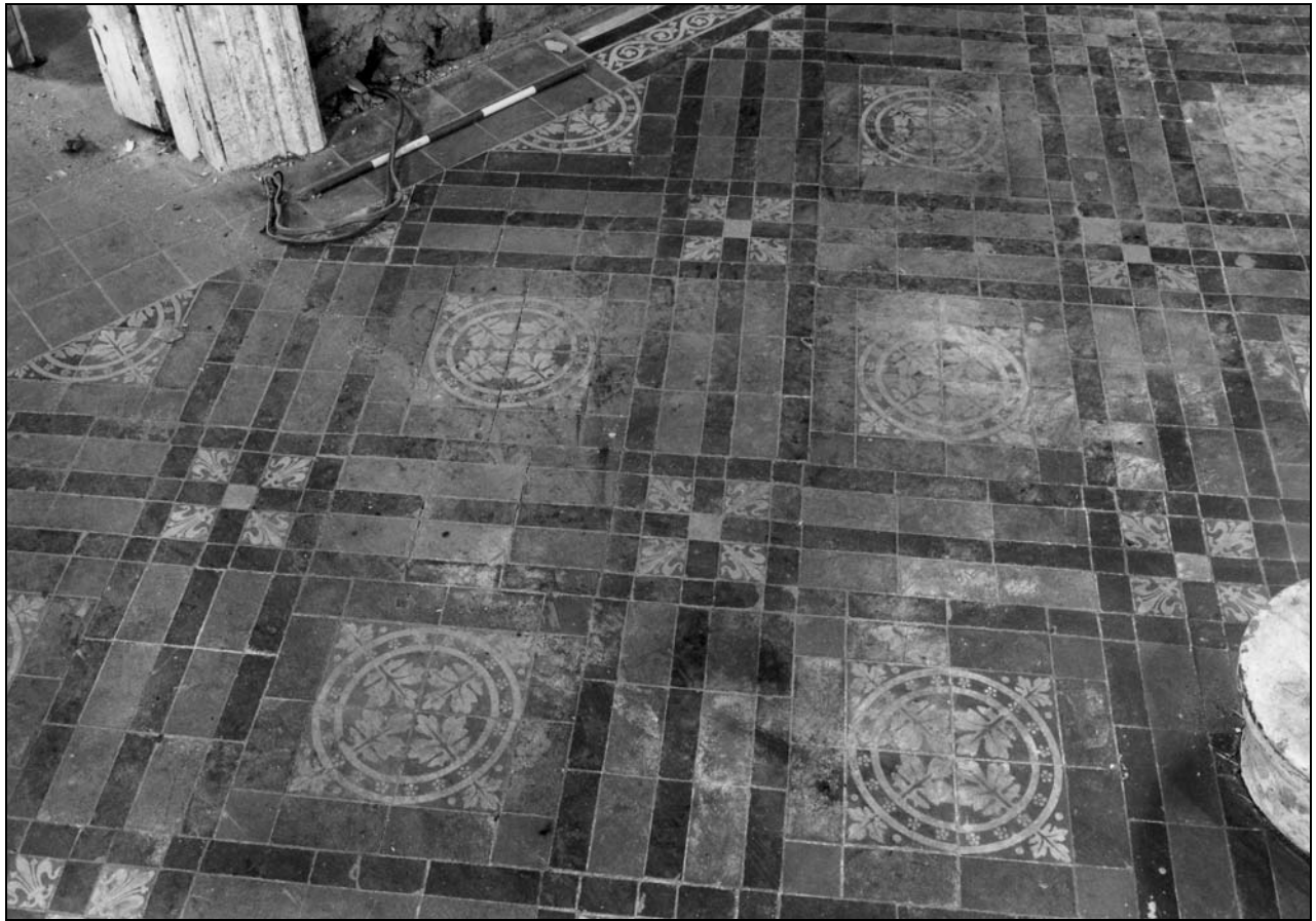
Photo 27: South wing: encaustic tile floor in entrance hall G11 (film 2, frame 11)
