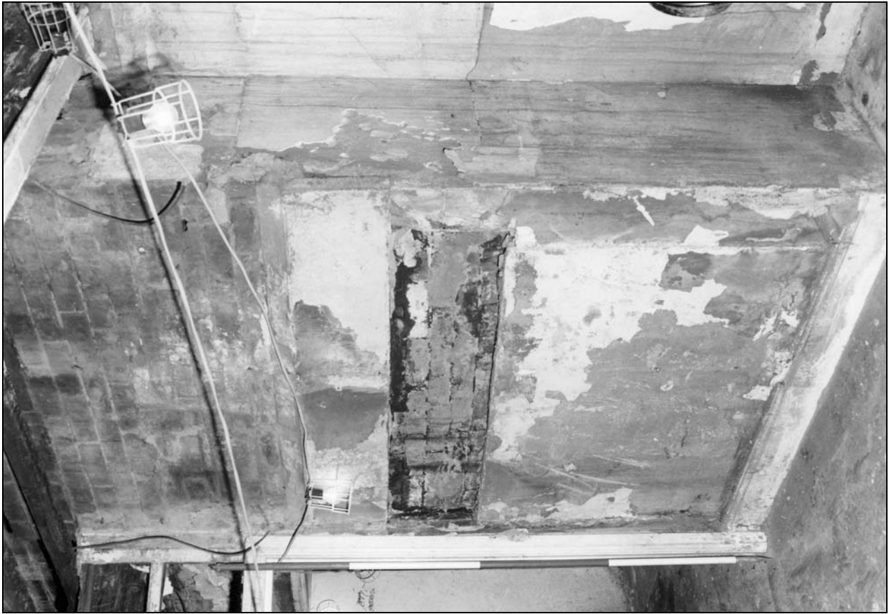
Photo 59: North wing: blocked fireplace in back kitchen G03 (film 3, frame 16)
