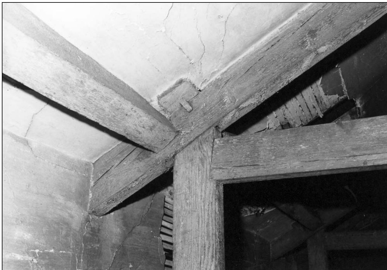
Photo 81: North wing: detail of roof truss, from the east (film 6, frame 15)
