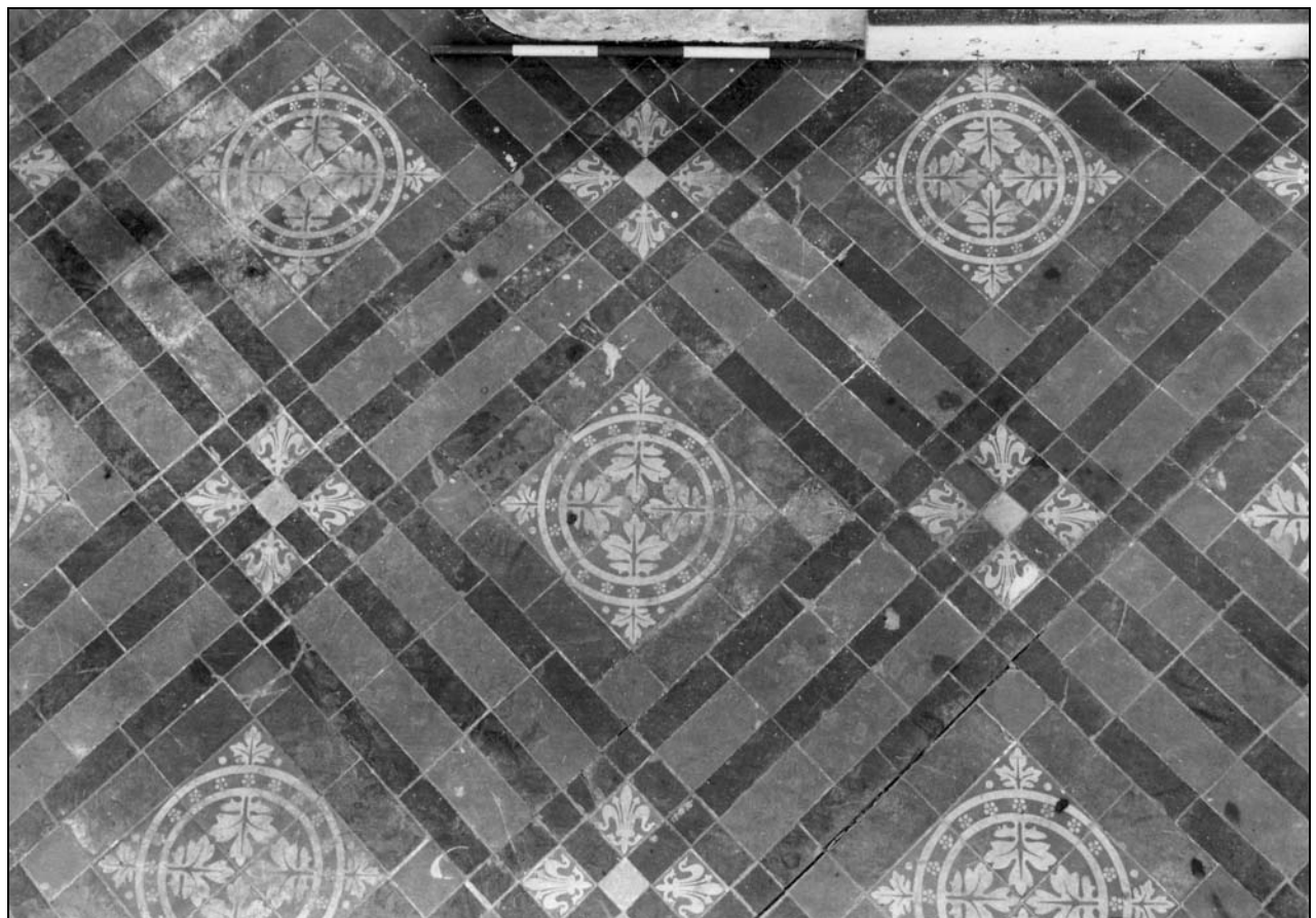
Photo 28: South wing: encaustic tile floor in entrance hall G11 (film 2, frame 12)
