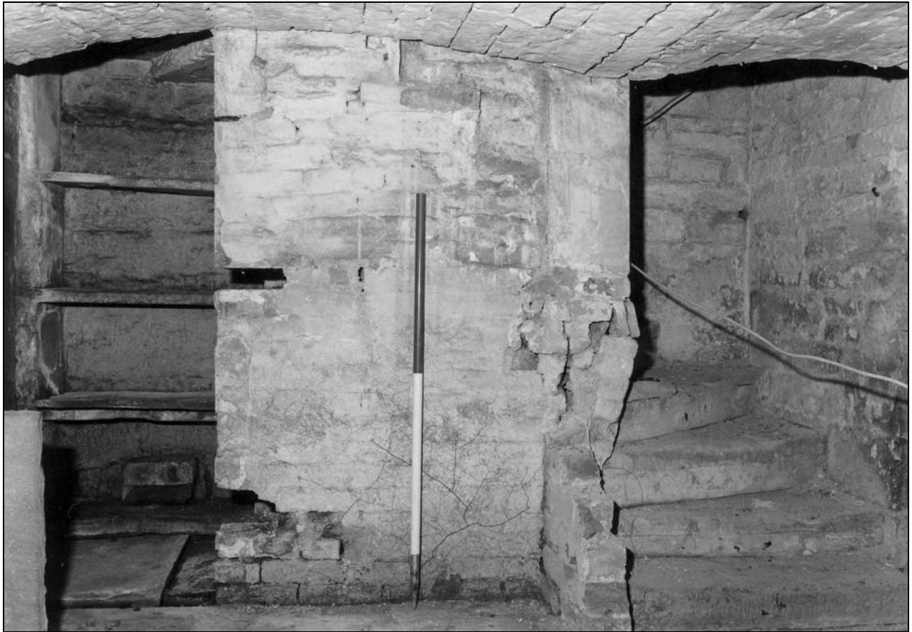
Photo 37: South wing: cellar B02, from the south (film 1, frame 10)
