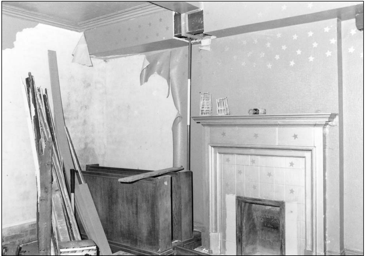
Photo 33: South wing: ground floor room G01, from the north-east (film 2, frame 17)
