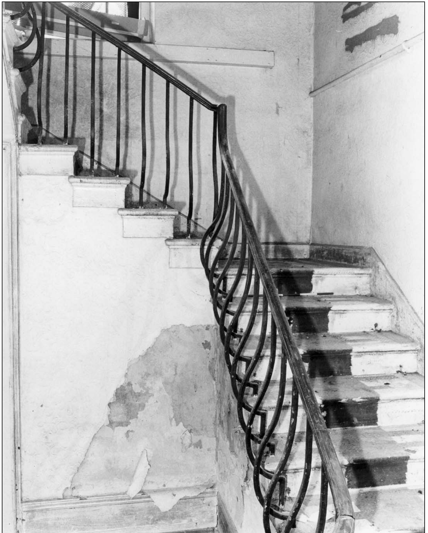
Photo 24: South wing: staircase in entrance hall G11 (film 2, frame 6)
