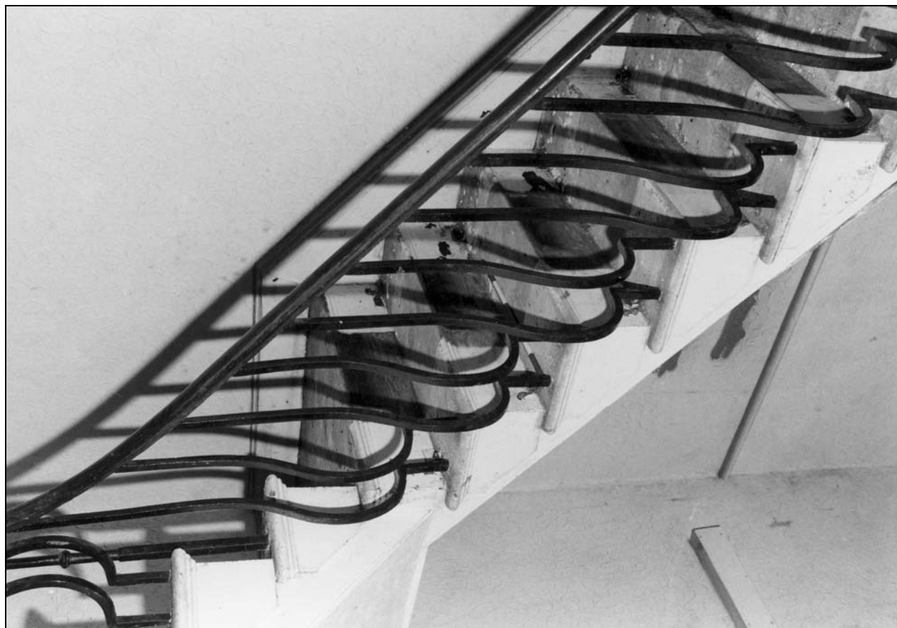
Photo 46: South wing: detail of stairs up to second floor (film 4, frame 6)
