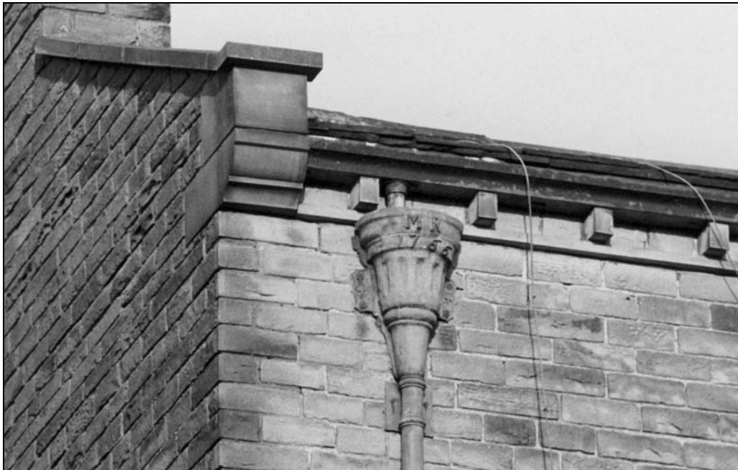
Photo 7: Detail of rainwater hopper bearing initials MR and date 1766 (film 5, frame 2)
