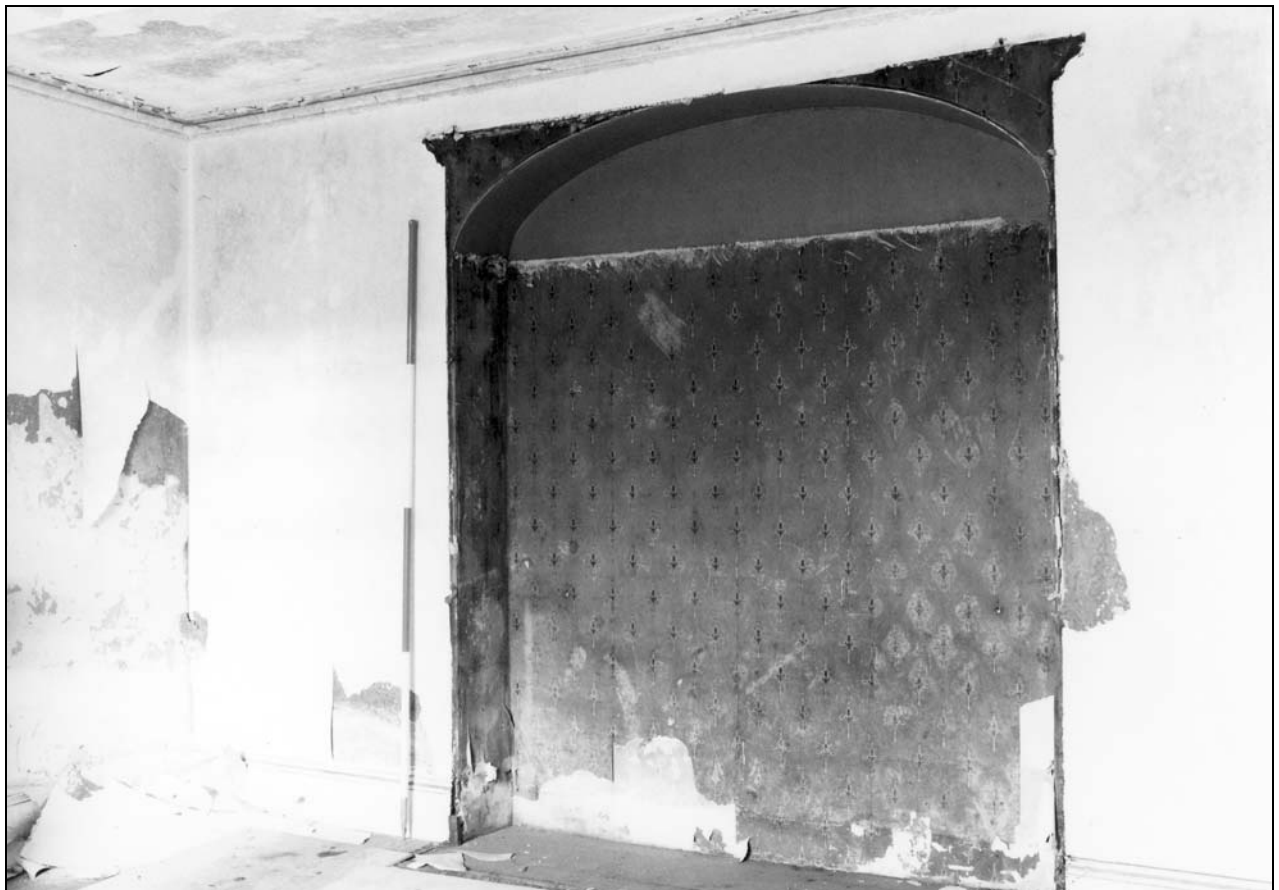
Photo 30: South wing: ground floor room G02, from the south-east (film 2, frame 15)
