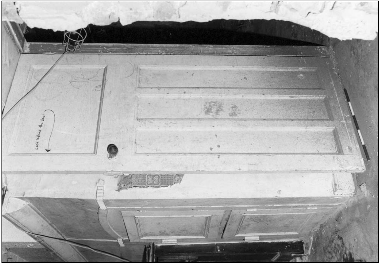
Photo 58: North wing: door of c. 1930 in kitchen G05 (film 3, frame 13)
