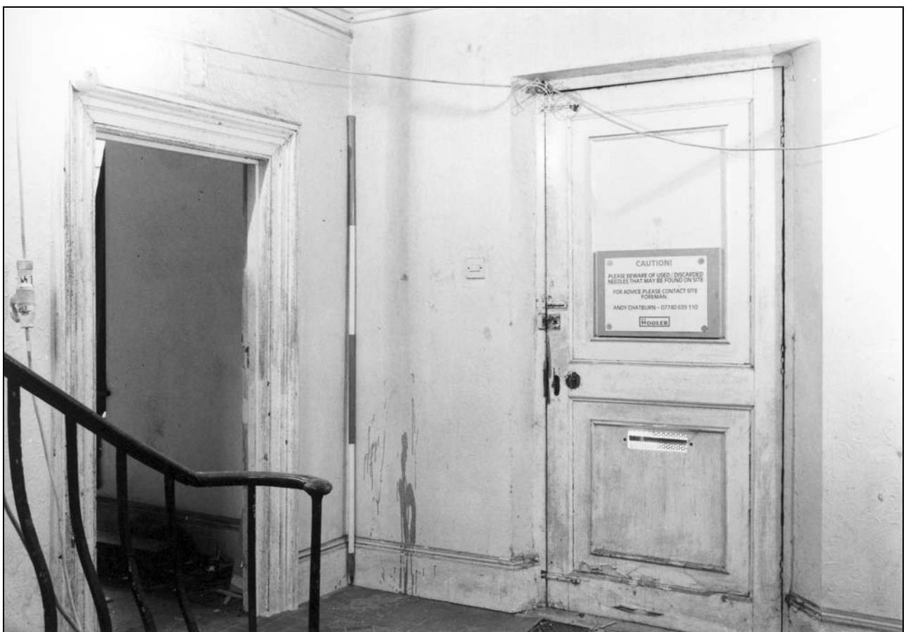
Photo 21: South wing: the entrance hall G11, from the north-west (film 2, frame 4)
