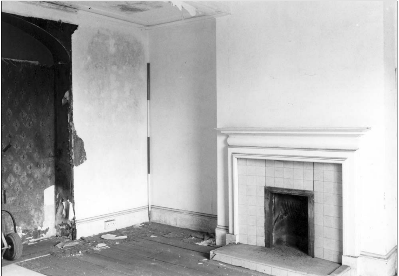
Photo 29: South wing: ground floor room G02, from the south-west (film 2, frame 13)
