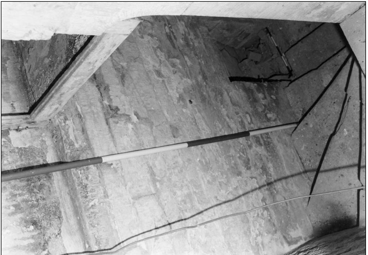
Photo 35: South wing: steps down to cellar B02, from the west (film 1, frame 11)
