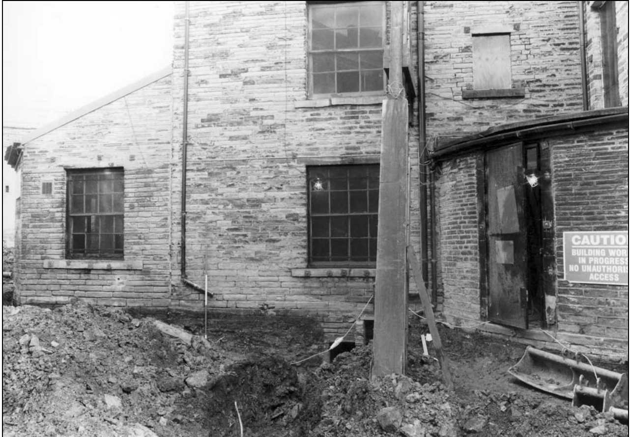
Photo 17: The original west gable of the north wing, with porch at bottom right and later lean-to at left (film 5, frame 10)
