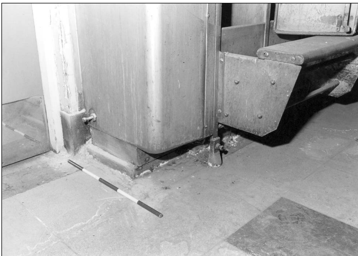
Photo 67: Detail of metal casing at end of row of “dirty lockers”, containing warm air duct from below (film 4, frame 14)
