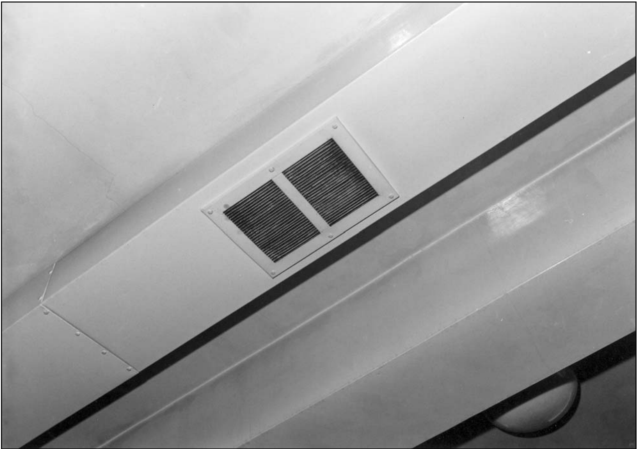
Photo 25: Grill in overhead extraction duct, in “dirty lockers” room (film 4, frame 8)
