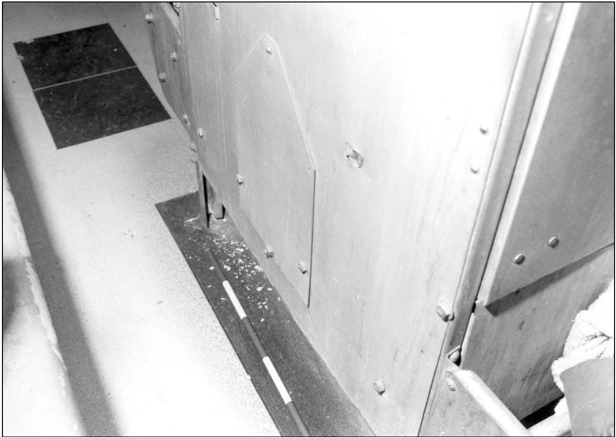
Photo 68: Detail of panel for warm air ducts at end of row of “clean” lockers (film 6, frame 6)
