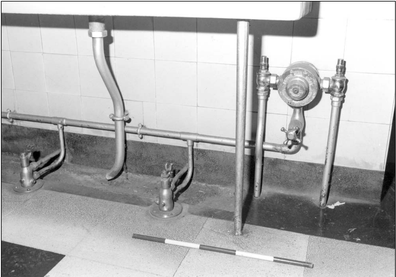
Photo 48: Detail of mixer control and foot-operated taps for wash basin in “washroom” (film 5, frame 9)
