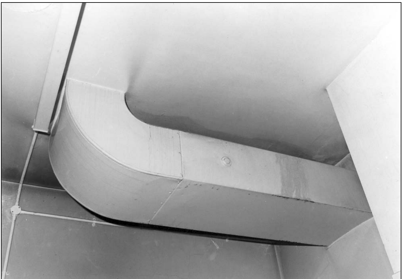
Photo 26: Detail of overhead extraction duct in “works lavs” (film 5, frame 14)
