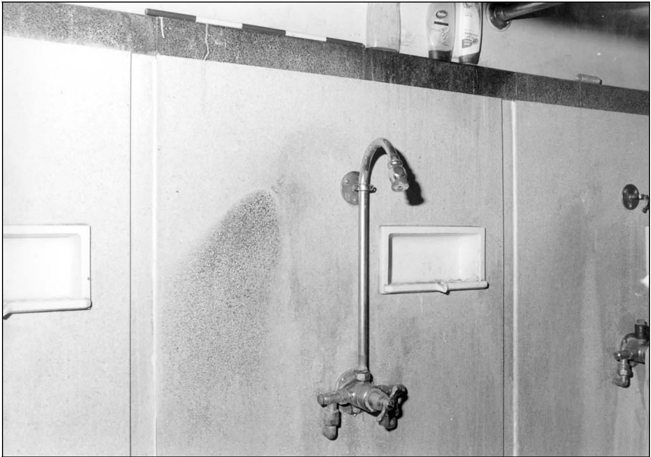
Photo 58: Detail of shower tap and head in open showers (film 6, frame 13)
