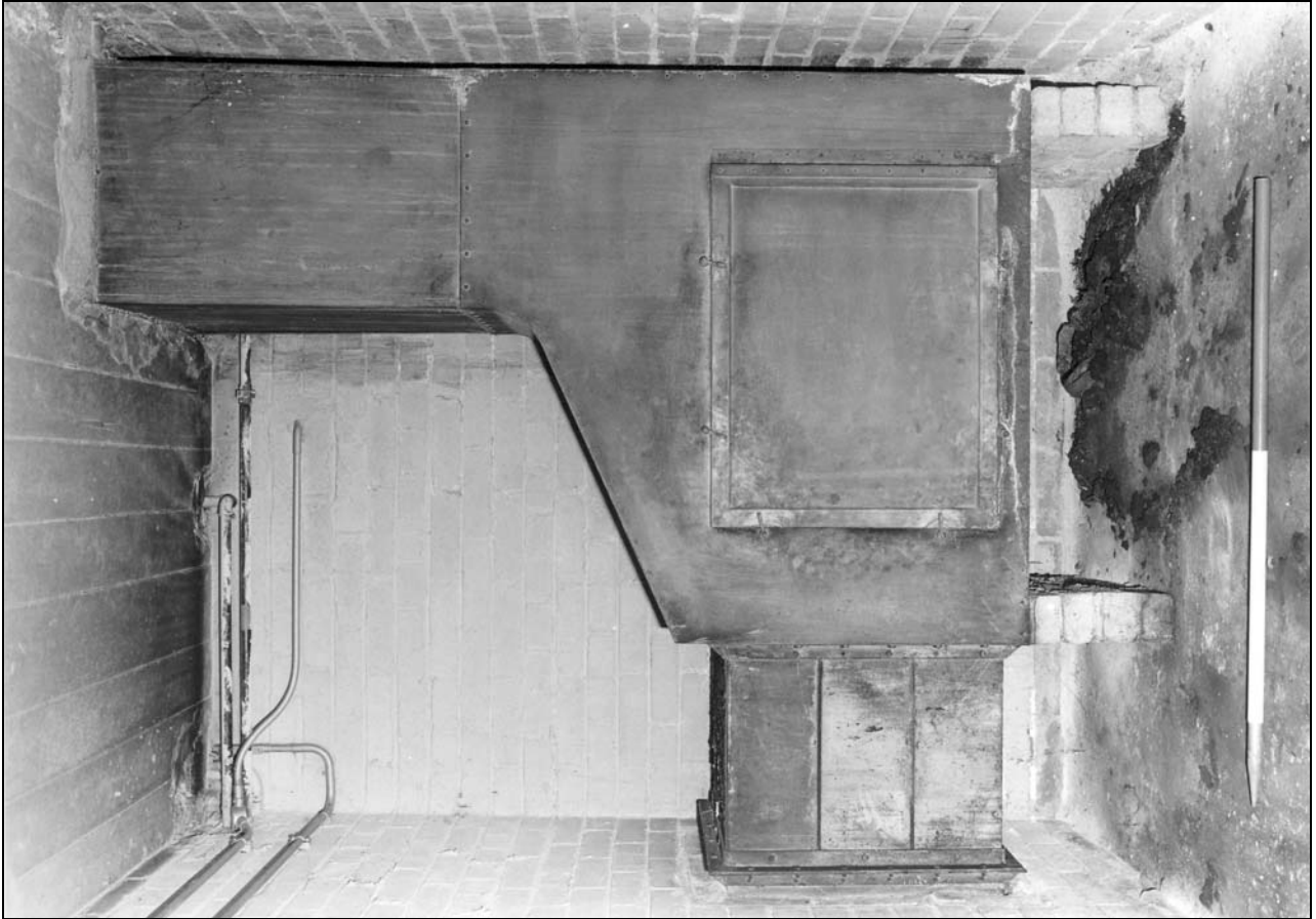
Photo 77: Basement: main air duct at foot of intake (film 1, frame 13)
