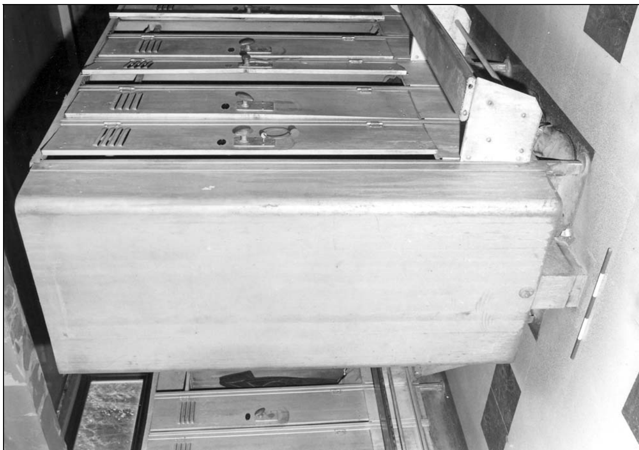
Photo 66: End of row of “clean” lockers”, showing casing and warm air duct at floor level (film 6, frame 4)
