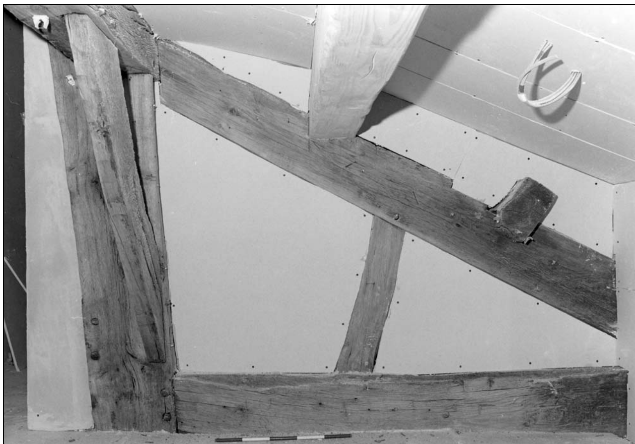
Photo 11: Aisle roof structure, from the north (film 1, frame 5)
