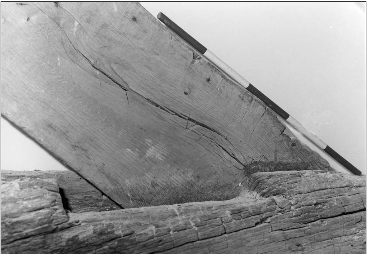
Photo 18: Detail of carpenter's numbering at foot of principal rafter, truss Y (film 1, frame 10)
