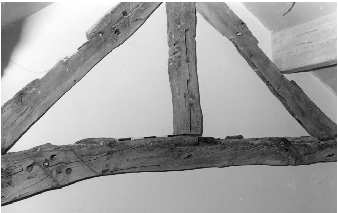
Photo 16: Truss Y, re-sited, from the south (film 1, frame 2)
