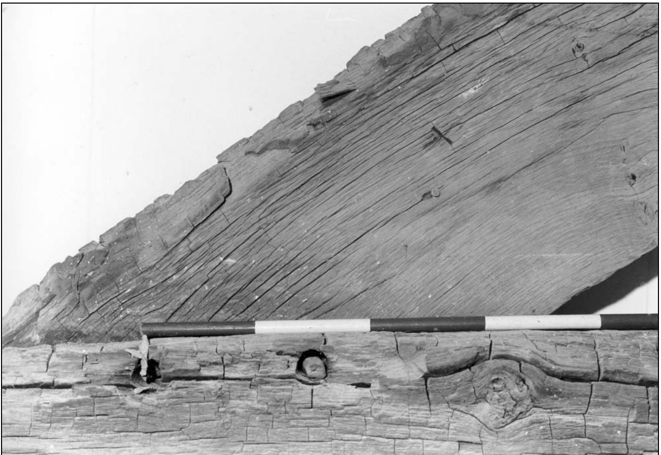
Photo 22: Detail of carpenter's numbering at foot of principal rafter, truss Z (film 1, frame 14)
