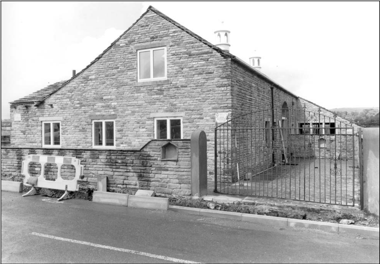
Photo 1: General view, from the south-east (film 2, frame 6)
