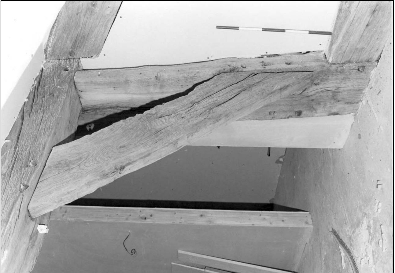
Photo 14: Arcade brace, from the north-west (film 1, frame 6)
