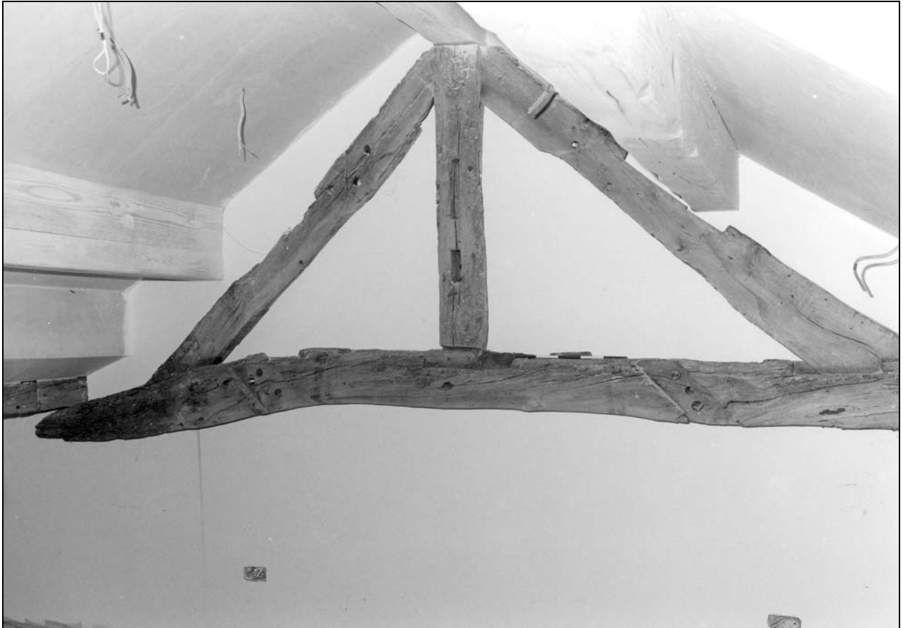
Photo 15: Truss Y, re-sited, from the south (film 1, frame 1)
