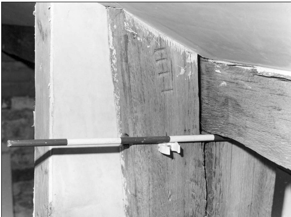
Photo 10: Carpenter's numbering at head of arcade post, from the north (film 1, frame 12)
