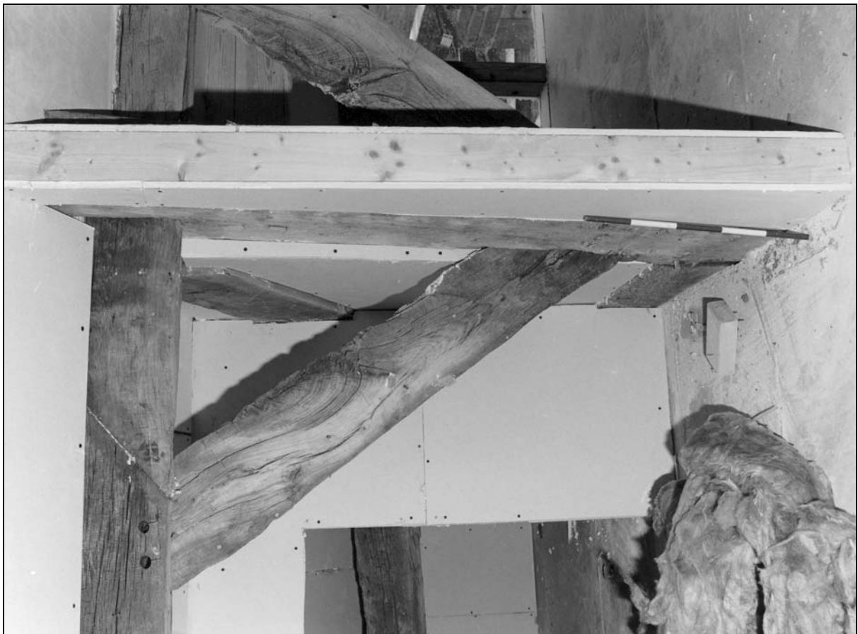
Photo 13: Arcade brace and scarf joint in arcade plate, from the east (film 1, frame 7)
