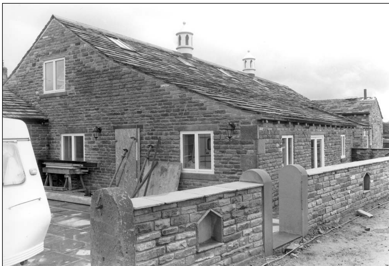
Photo 6: General view, from the north-west (film 2, frame 12)
