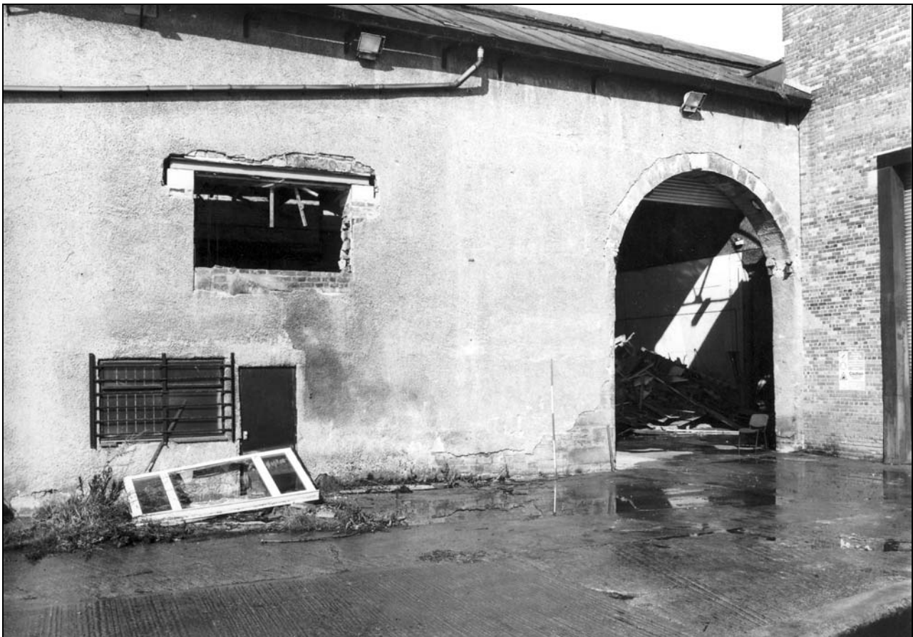
Photo 32: Building 1: external view of east wall, south end (film 1, frame 3)
