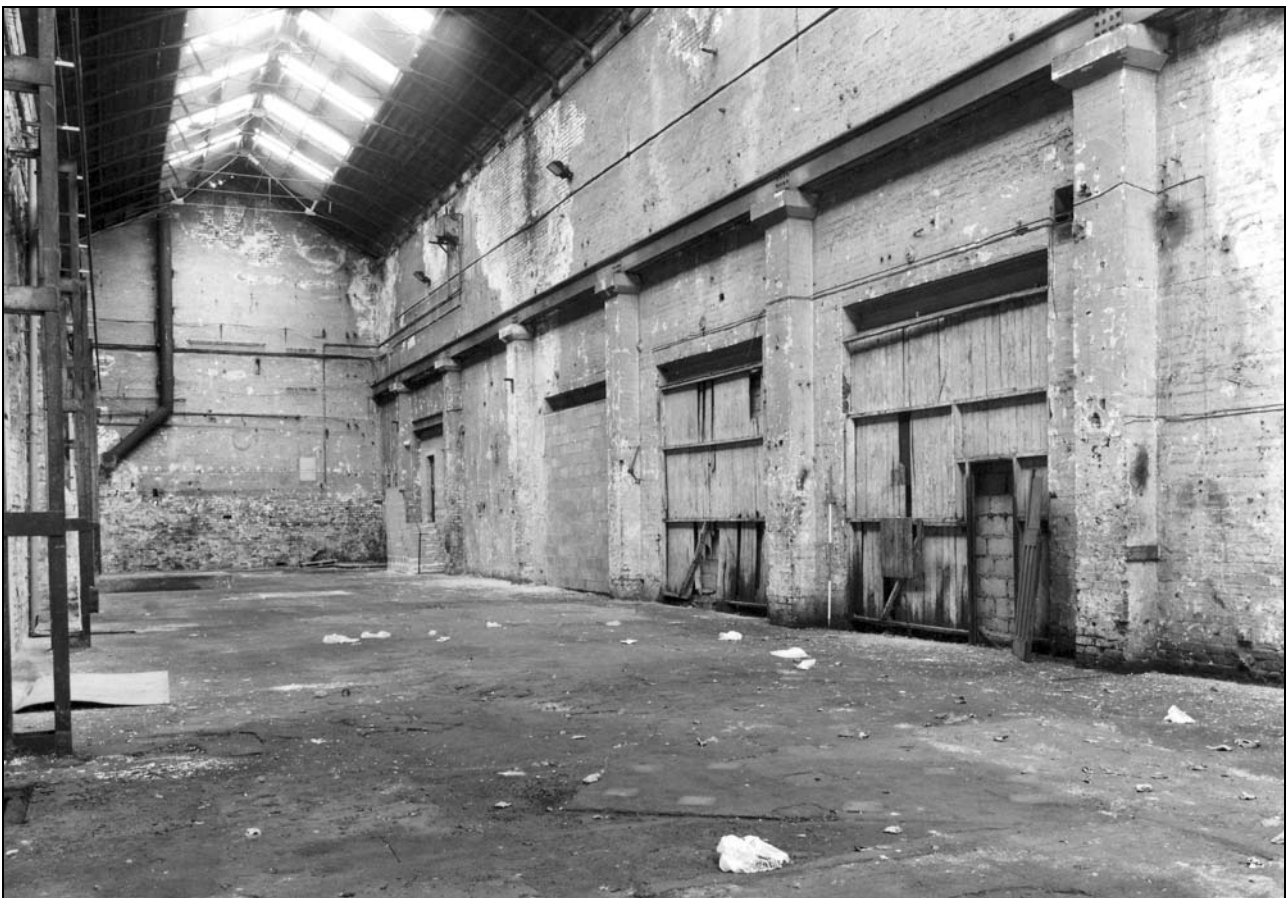
Photo 56: Building 2: interior, from the south-west (film 2, frame 17)
