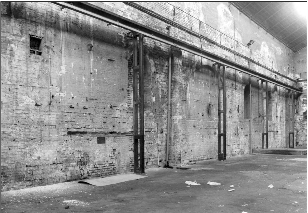
Photo 41: Building 1: external view of east wall, now within Building 2 (film 2, frame 4)
