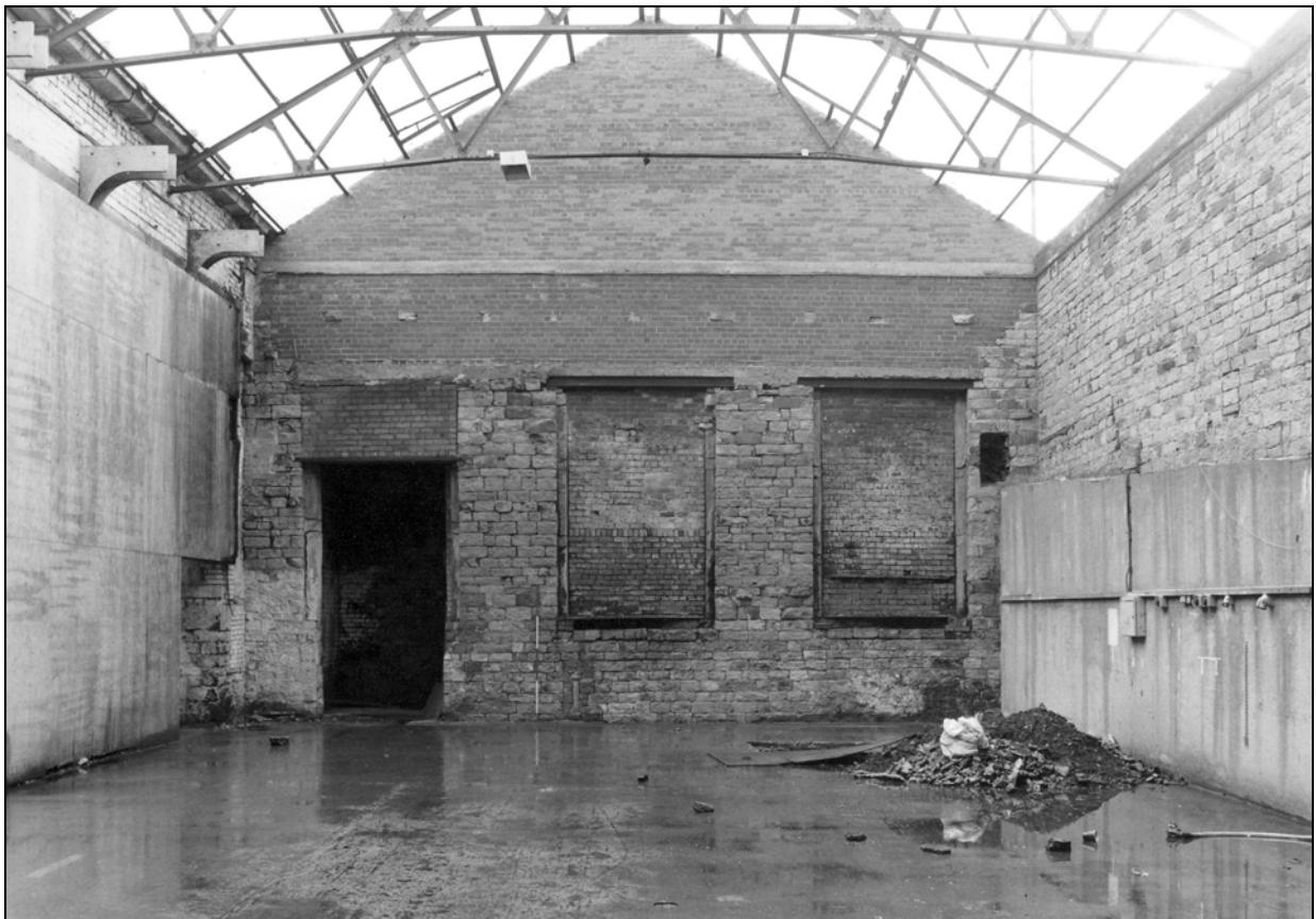
Photo 60: Building 3: internal view of south end (film 5, frame 12)
