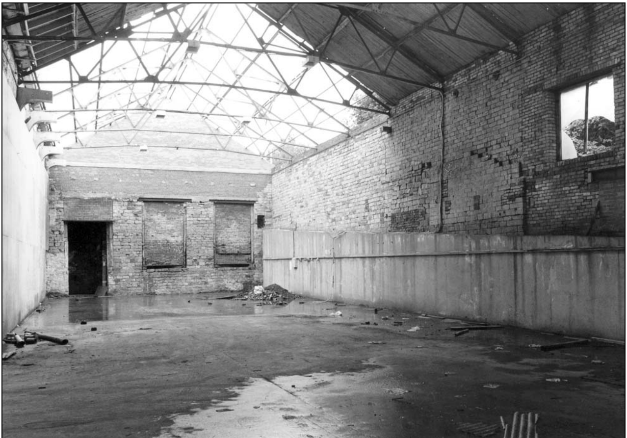
Photo 64: Building 3: interior at south end (film 5, frame 10)
