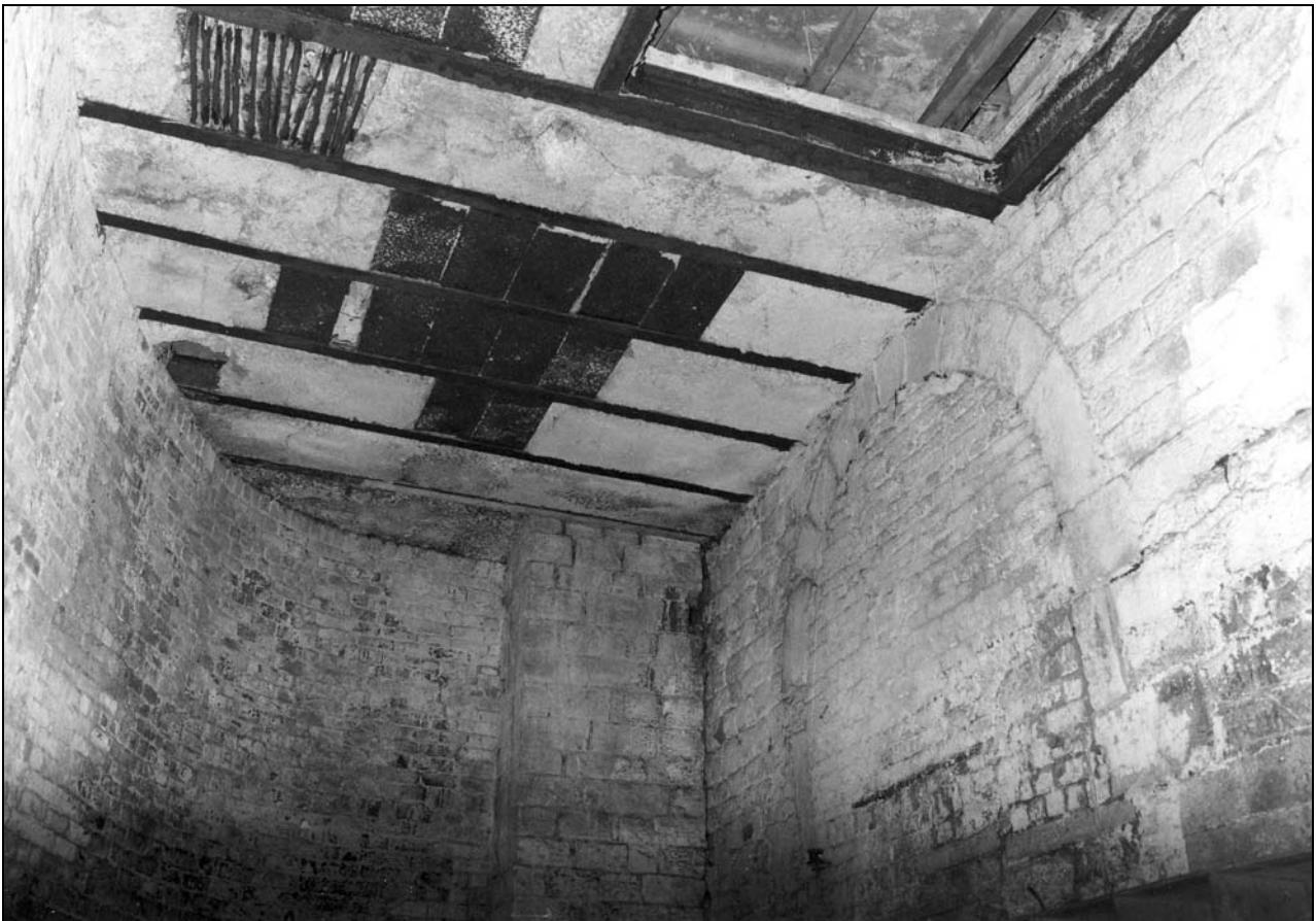
Photo 22: Building 1: external view of south wall, showing arched former window and floor of modern building above (film 3, frame 17)
