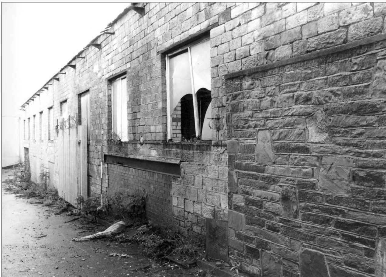
Photo 67: Building 3: external view of west wall, north end (film 1, frame 7)
