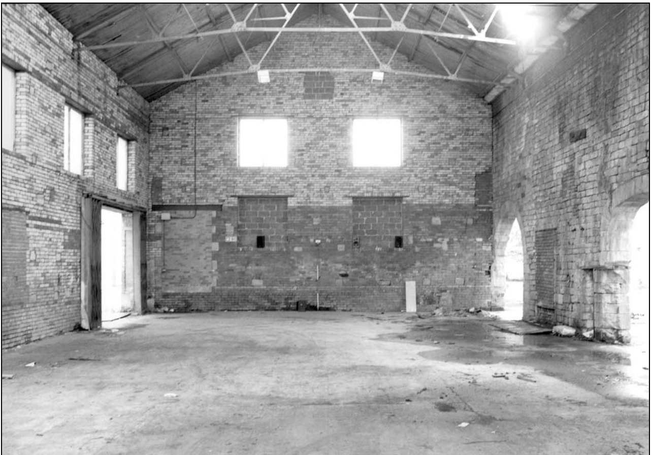
Photo 70: Building 3: interior at north end (film 5, frame 7)
