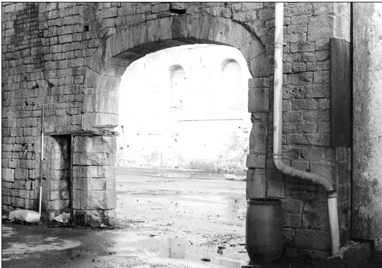
Photo 3: Doorway with basket arch in phase 1 wall, external view (film 5, frame 4)
