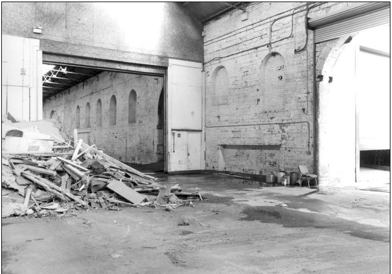
Photo 43: Building 1: internal view of east wall, from the south-west (film 3, frame 10)
