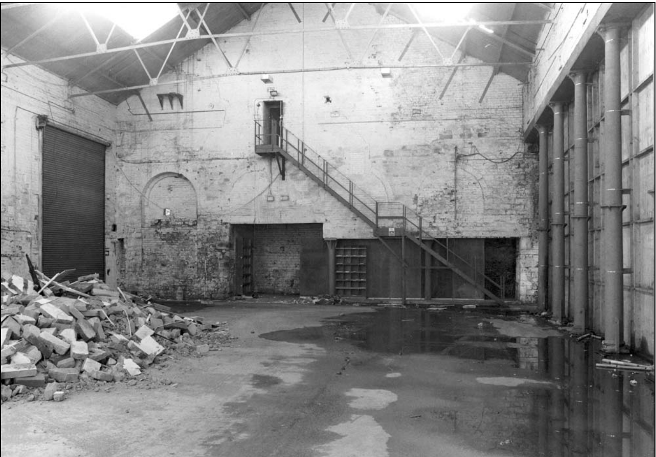
Photo 26: Building 1: interior view of south wall (film 3, frame 2)
