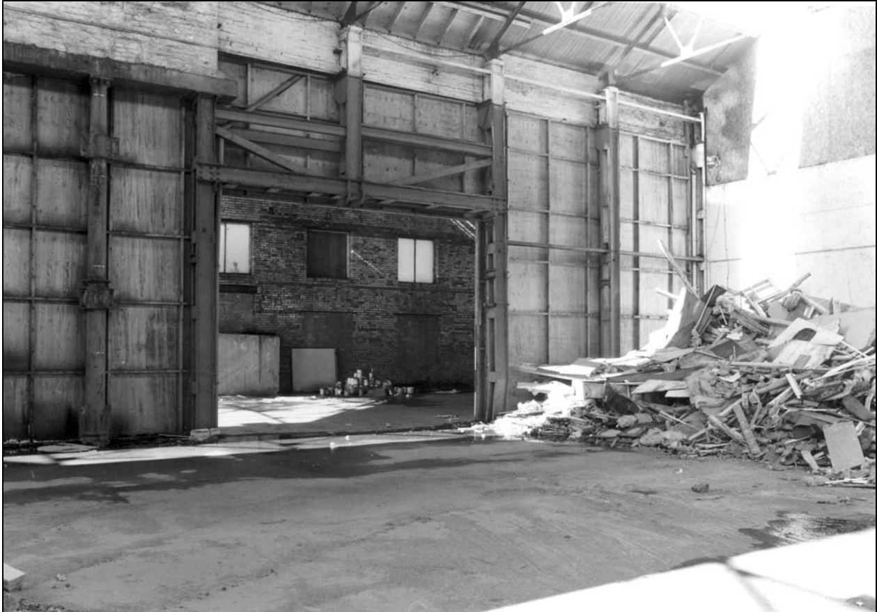
Photo 9: Building 1: internal view of west side, showing former position of blast furnaces (steel stanchions) and columns (film 3, frame 8)
