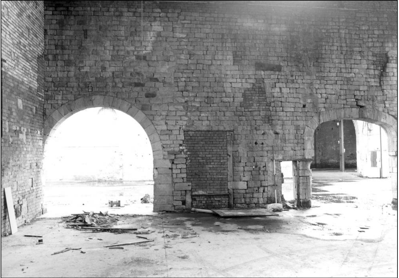
Photo 5: Building 1: external view of phase 1 wall in west side (film 5, frame 6)
