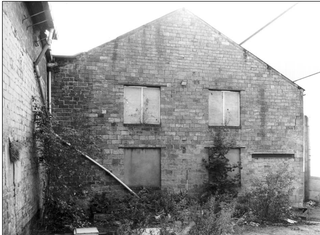
Photo 68: Building 3: external view of north wall (film 1, frame 10)
