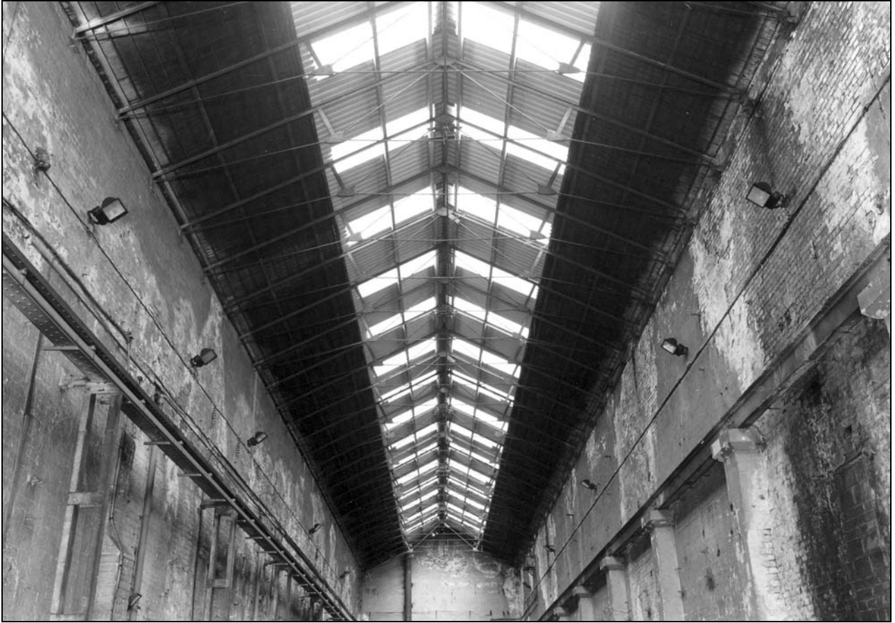
Photo 57: Building 2: view up towards roof, from the south (film 3, frame 1)
