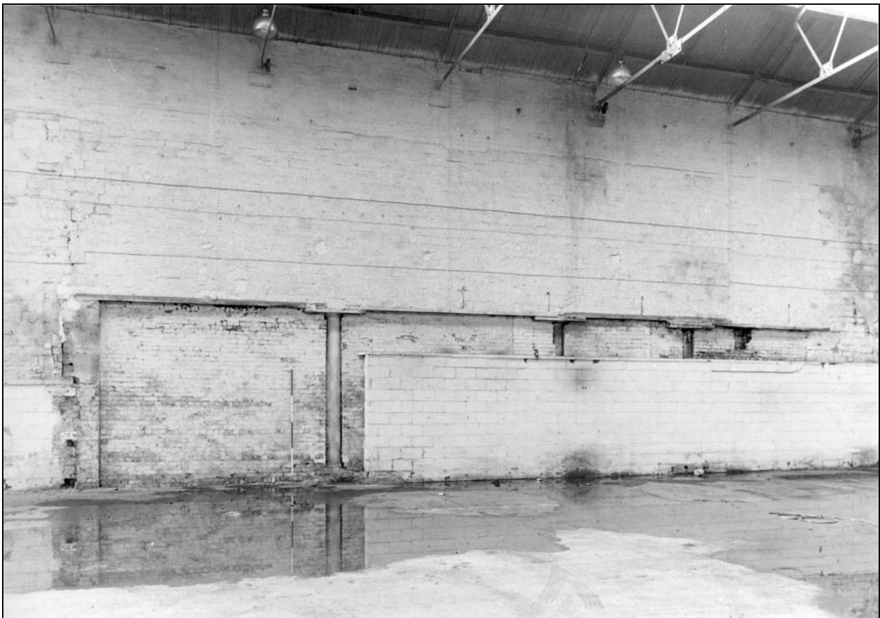
Photo 18: Building 1: internal view of west wall, showing inserted colonnade (film 4, frame 12)
