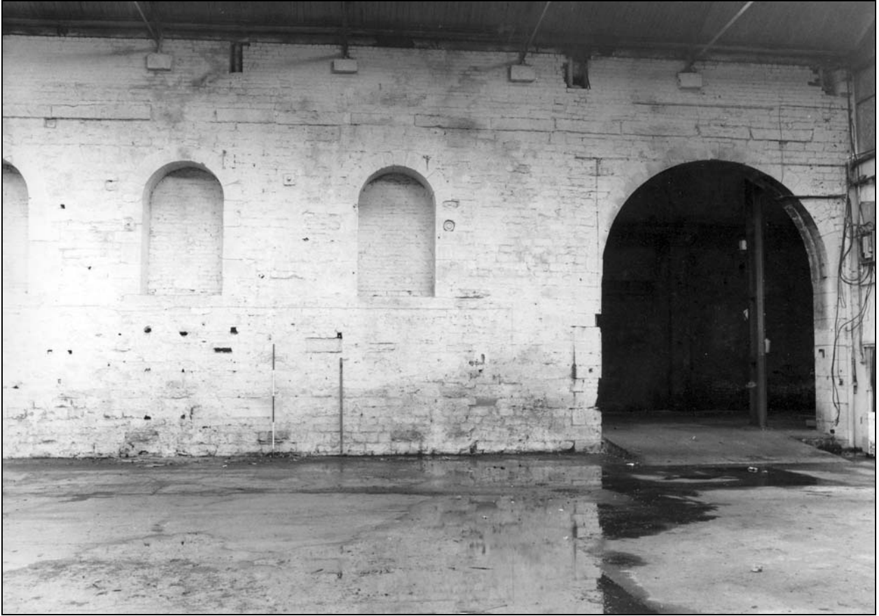
Photo 44: Building 1: internal view of east wall (film 4, frame 6)
