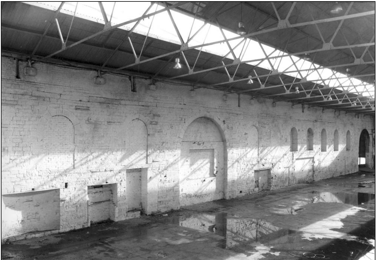
Photo 53: Building 1: internal view of east wall, from the north-west (film 4, frame 15)
