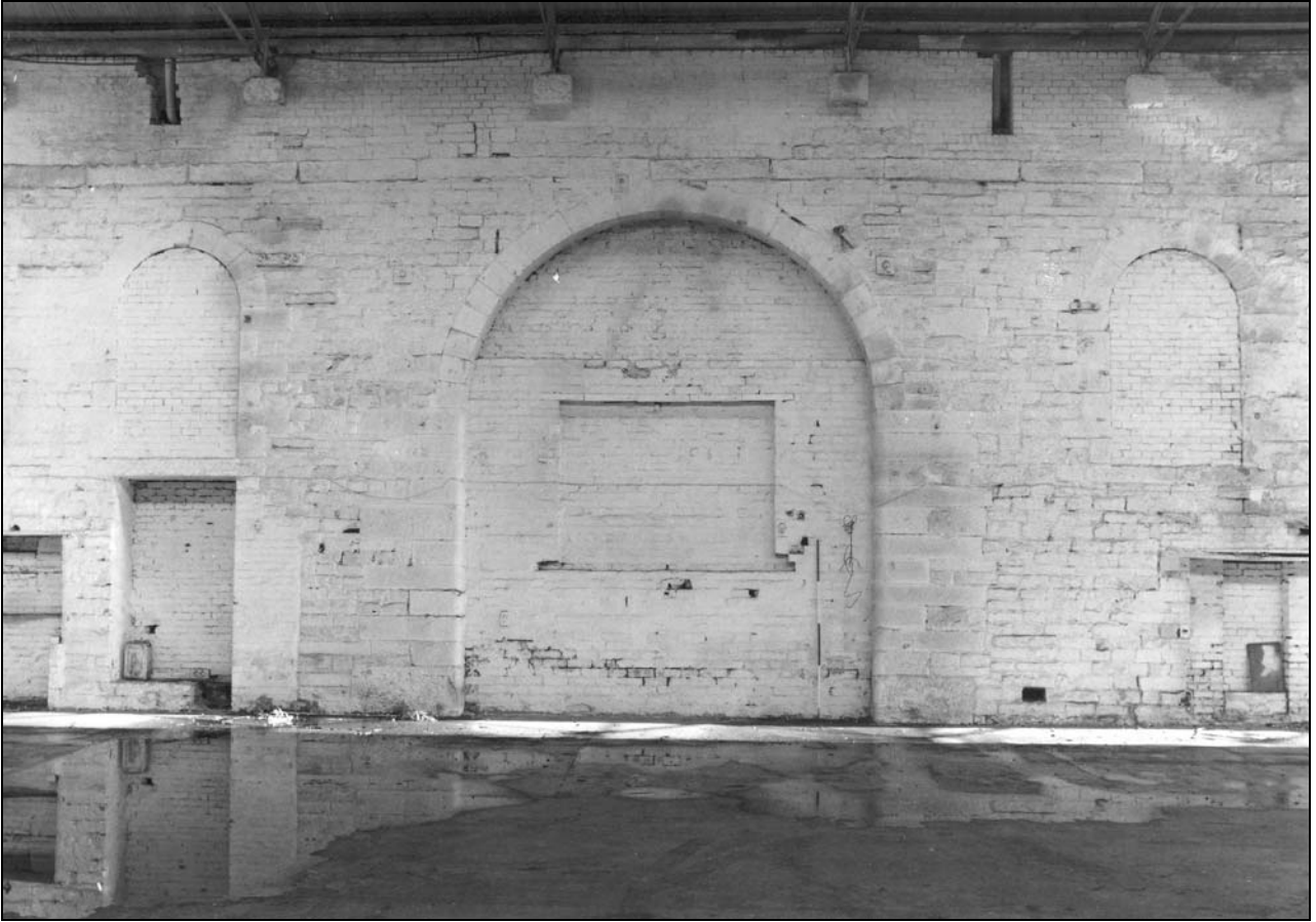
Photo 46: Building 1: internal view of east wall (film 4, frame 2)
