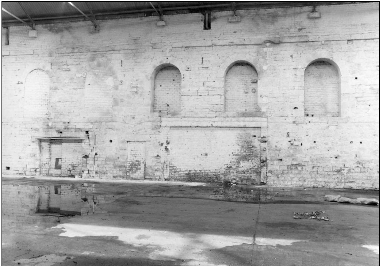
Photo 45: Building 1: internal view of east wall (film 4, frame 5)
