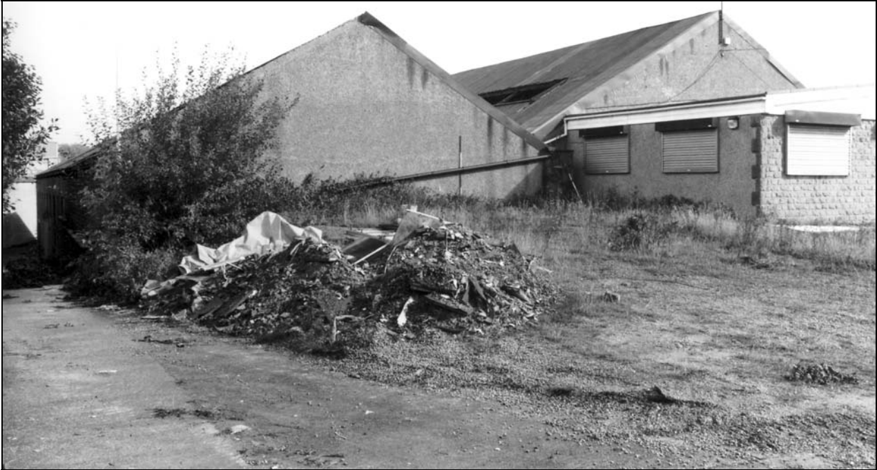
Photo 23: Buildings 1 and 3, from the south-west, with modern annex at right (film 1, frame 5)
