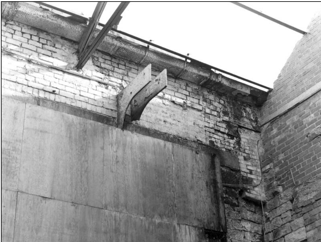
Photo 12: Building 1/3: detail of bracket for roof truss over Building 3 (film 5, frame 14)
