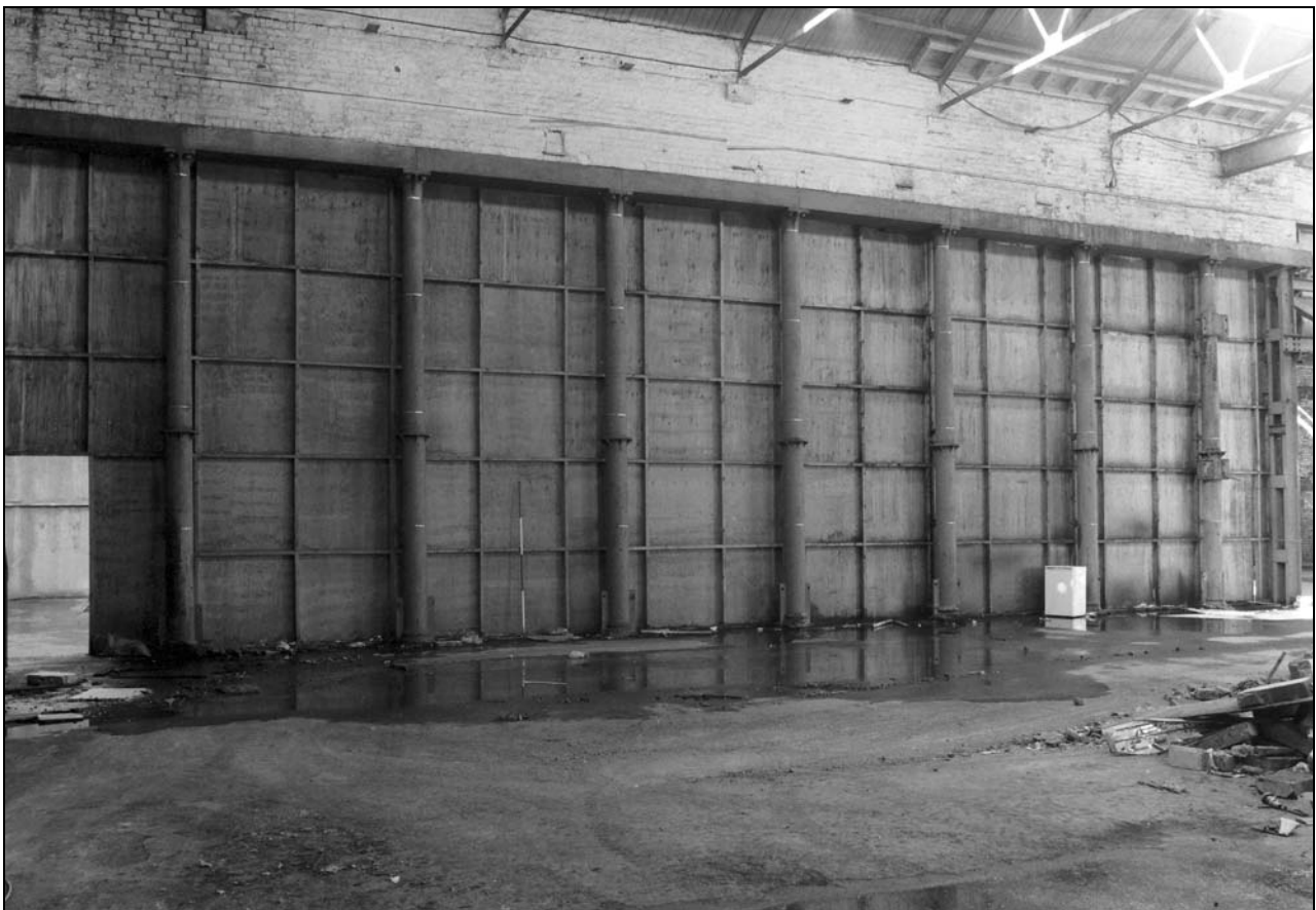
Photo 10: Building 1: internal view of large colonnade, west side (film 3, frame 6)
