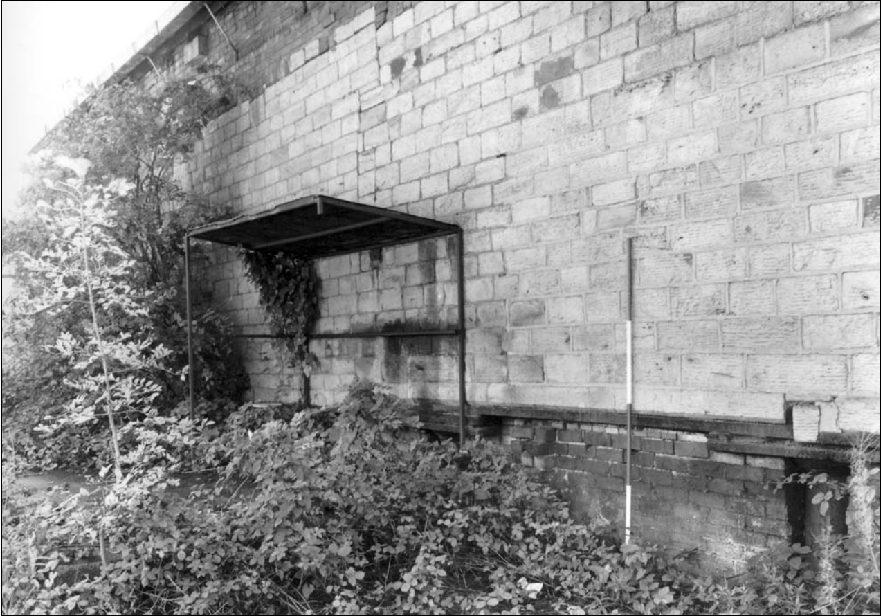
Photo 17: Building 1: external view of west wall, showing inserted colonnade (film 1, frame 15)
