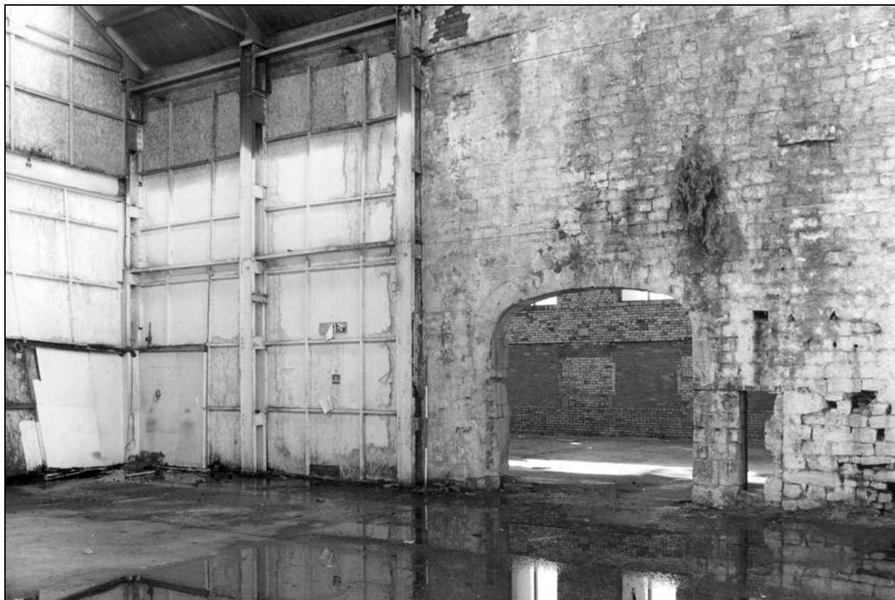
Photo 8: Building 1: internal view of phase 1 wall in west side, with former position of blast furnaces to left (film 4, frame 8)
