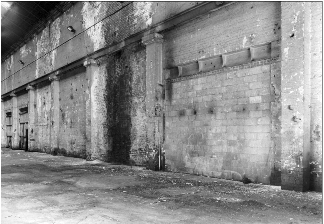
Photo 58: Building 2: internal view of east wall, from the south-west (film 2, frame 18)
