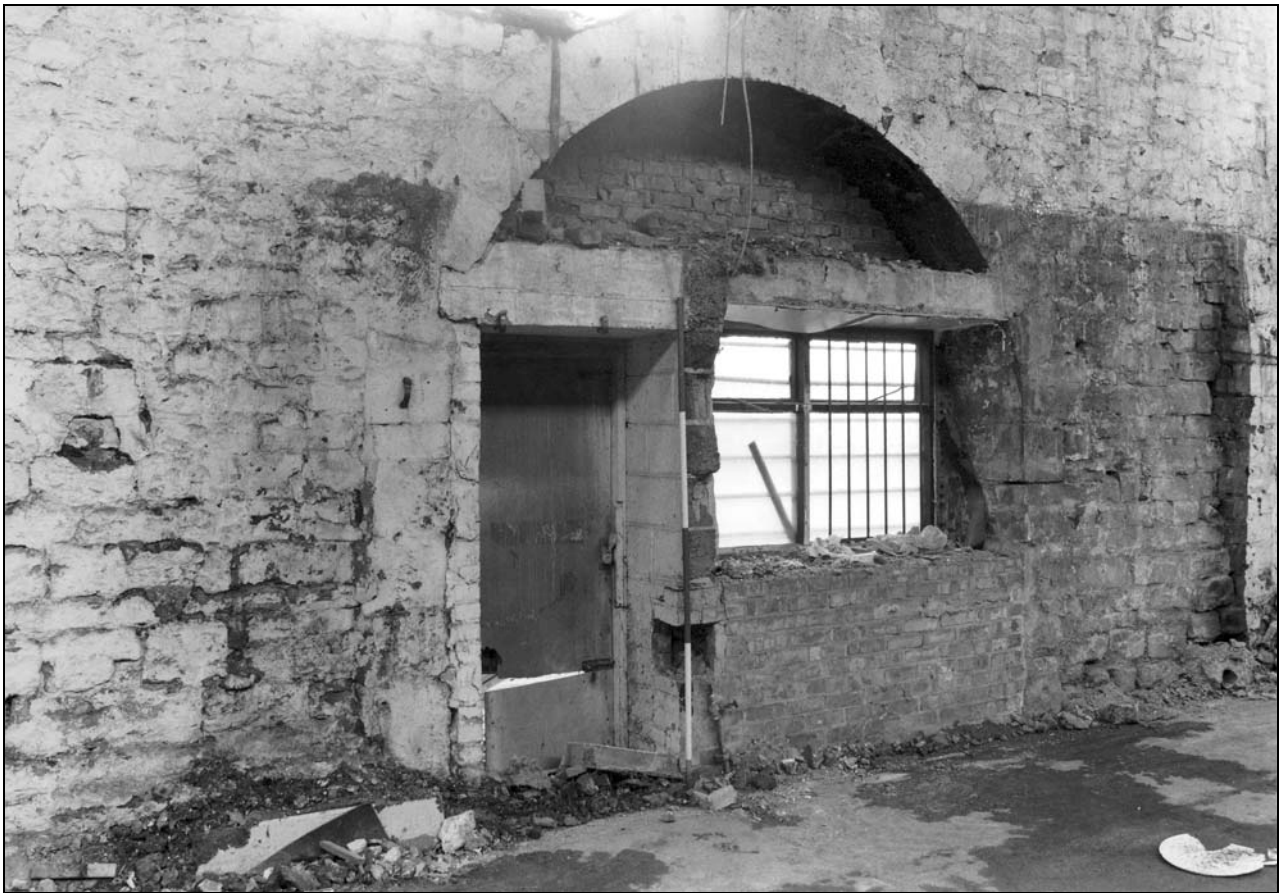
Photo 34: Building 1: interior view of one of two arched former openings in east wall, south end (film 3, frame 12)
