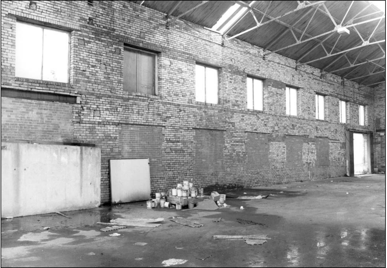
Photo 69: Building 3: internal view of west wall, north end (film 5, frame 8)
