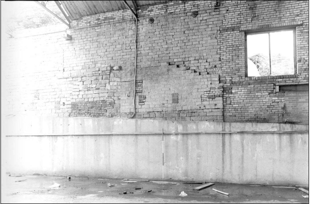
Photo 63: Building 3: internal view of west wall, south end (film 5, frame 11)
