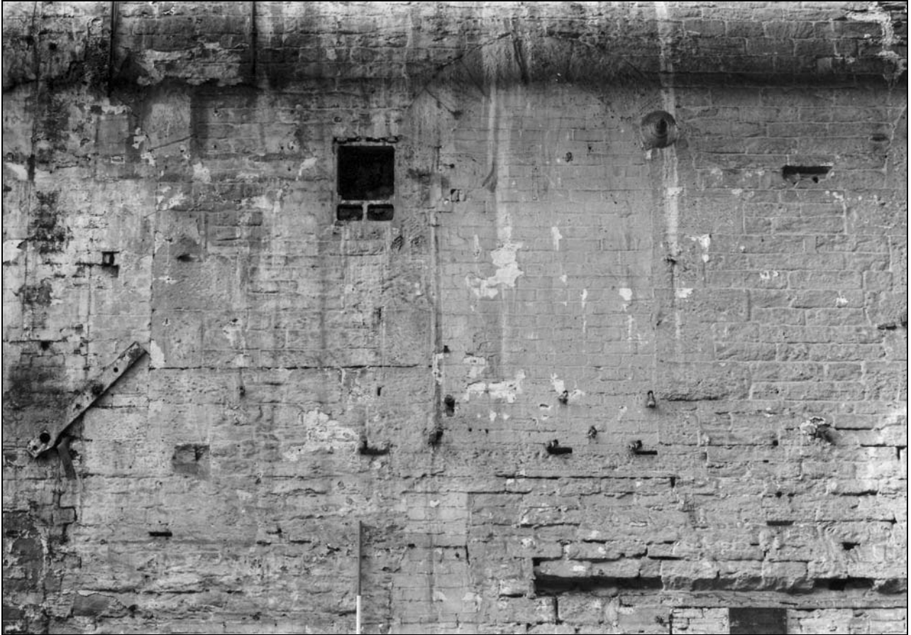
Photo 59: Building 2: wall bearing box in west wall (film 2, frame 14)
