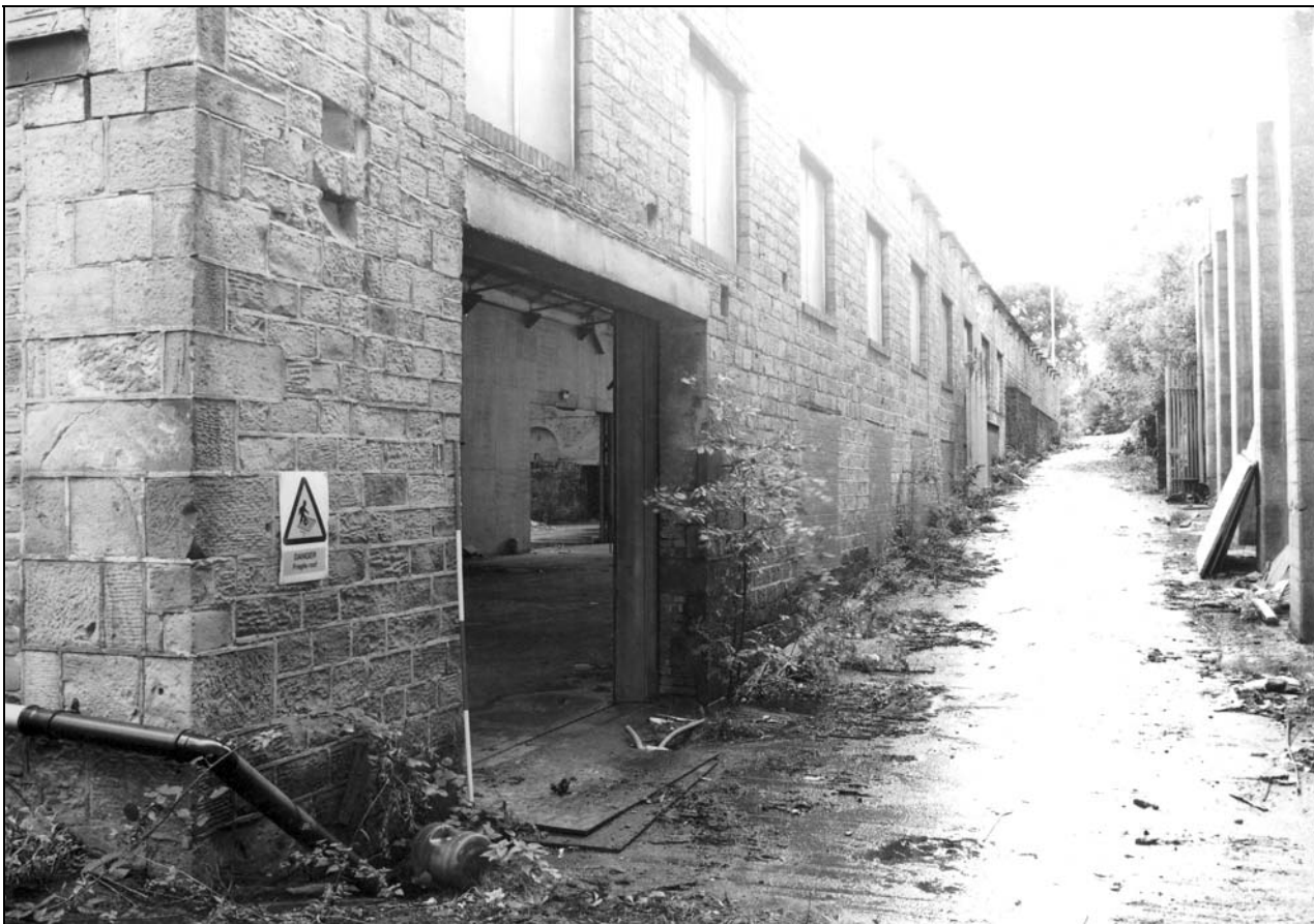
Photo 66: Building 3: external view of west wall, north end (film 1, frame 8)
