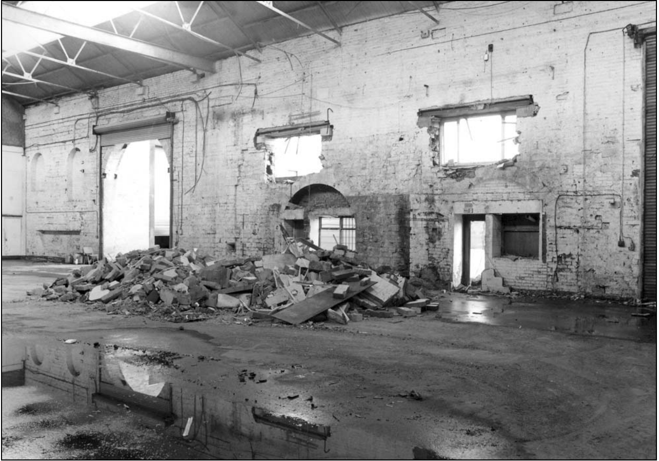
Photo 33: Building 1: internal view of east wall, south end (film 3, frame 11)
