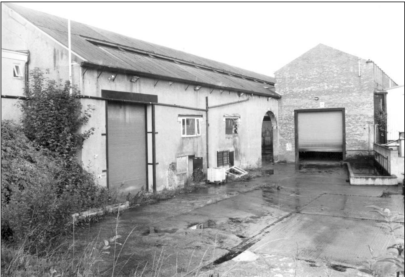
Photo 30: Building 1 (left) and Building 2 (right), from the south-east (film 1, frame 1)
