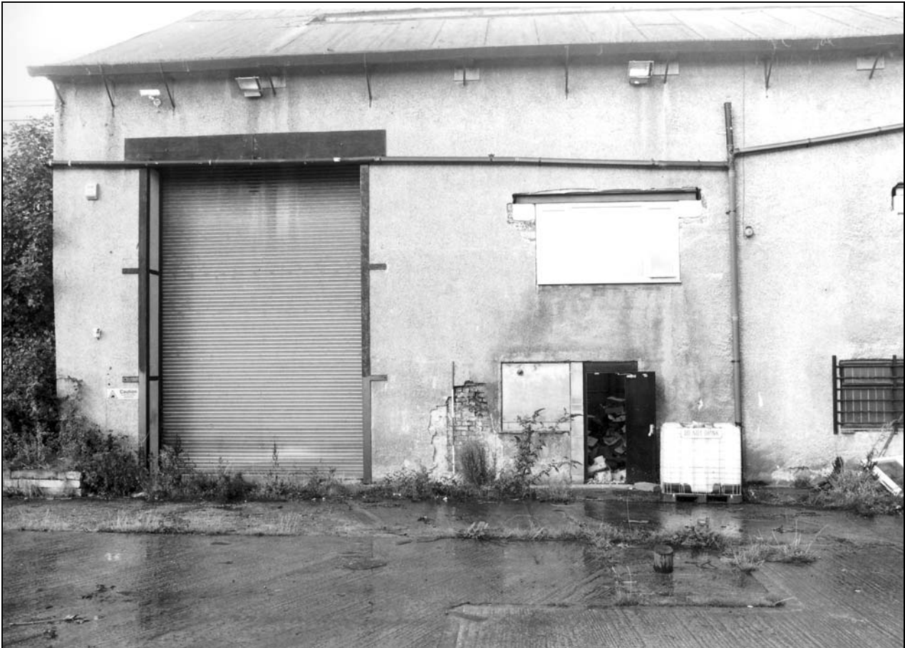
Photo 31: Building 1: external view of east wall, south end (film 1, frame 2)
