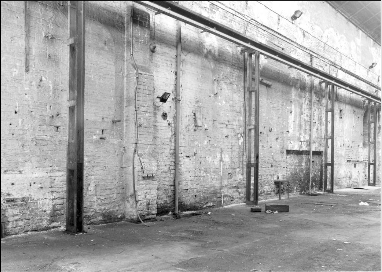
Photo 40: Building 1: external view of east wall, now within Building 2 (film 2, frame 2)
