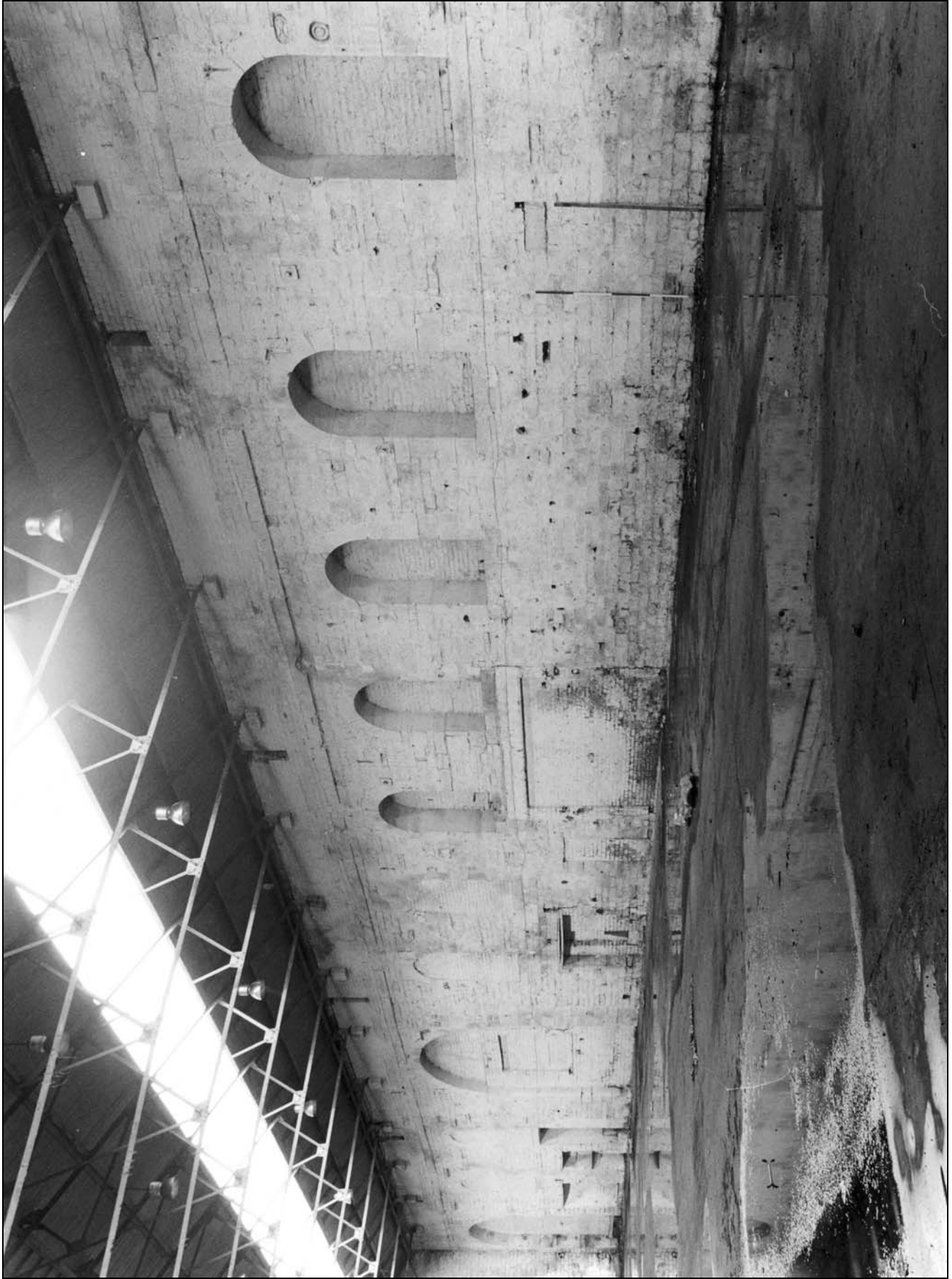
Photo 54: Building 1: internal view of east wall, from the south-west (film 4, frame 7)
