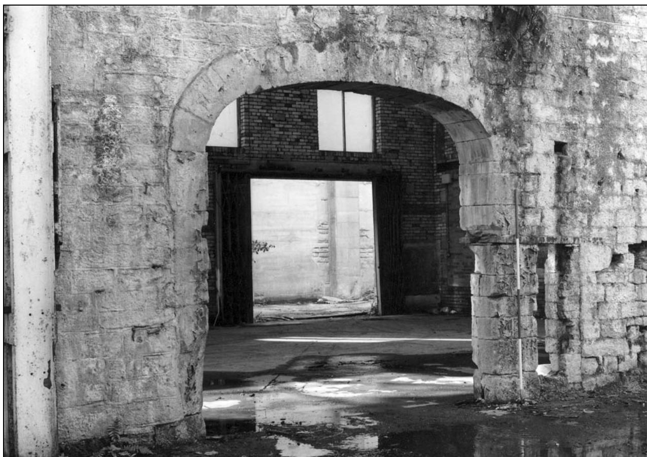
Photo 4: Doorway with basket arch in phase 1 wall, internal view (film 5, frame 2)
