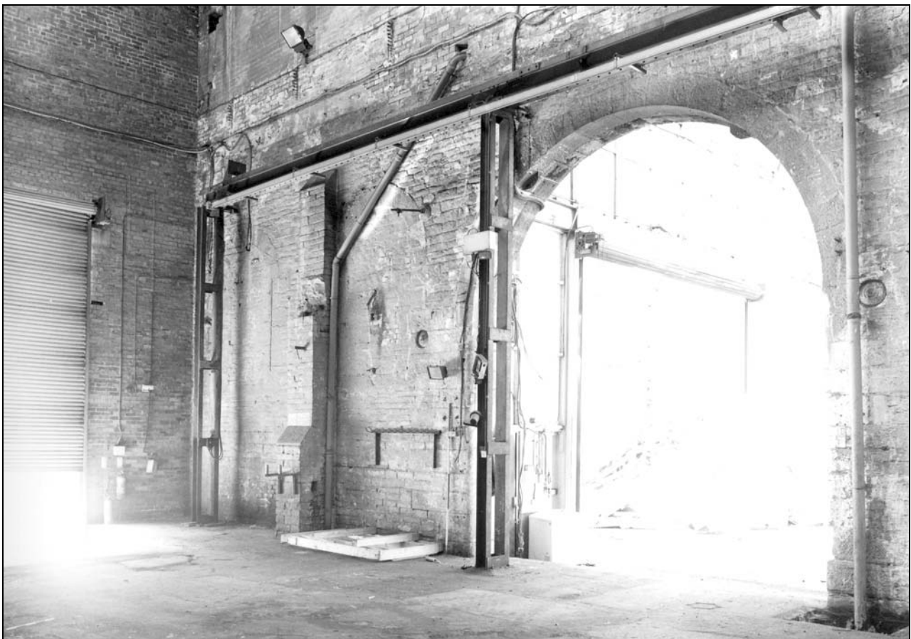
Photo 36: Building 1: external view of east wall, now within Building 2 (film 2, frame 1)
