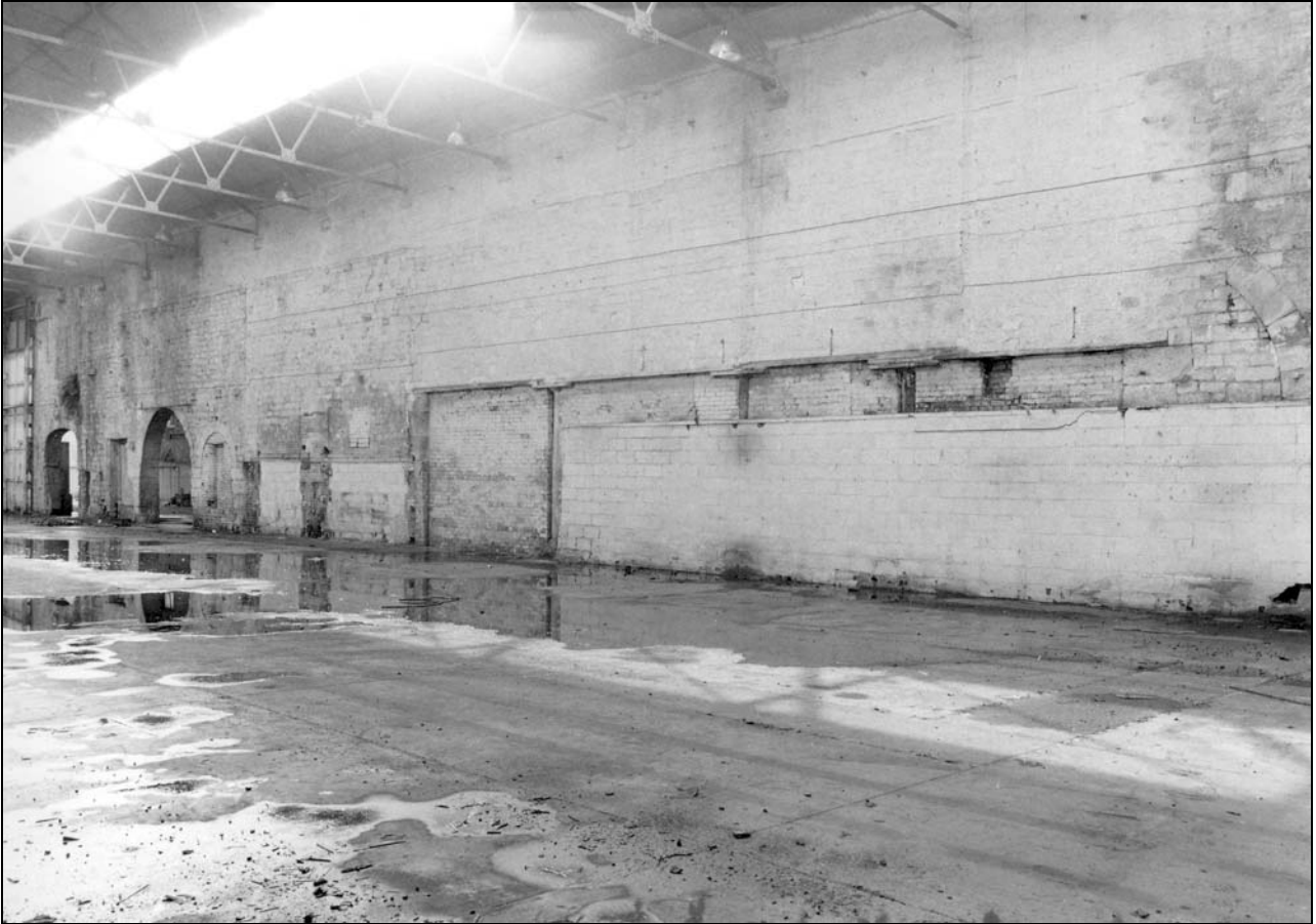
Photo 55: Building 1: internal view of west wall, from the north-east (film 4, frame 17)
