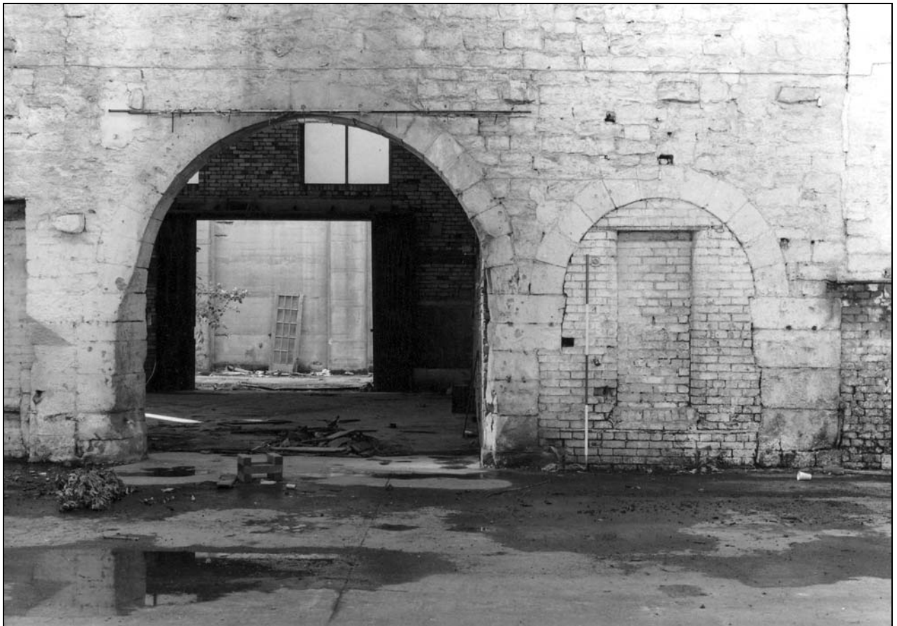
Photo 6: Building 1: internal view of phase 1 wall in west side (film 5, frame 1)
