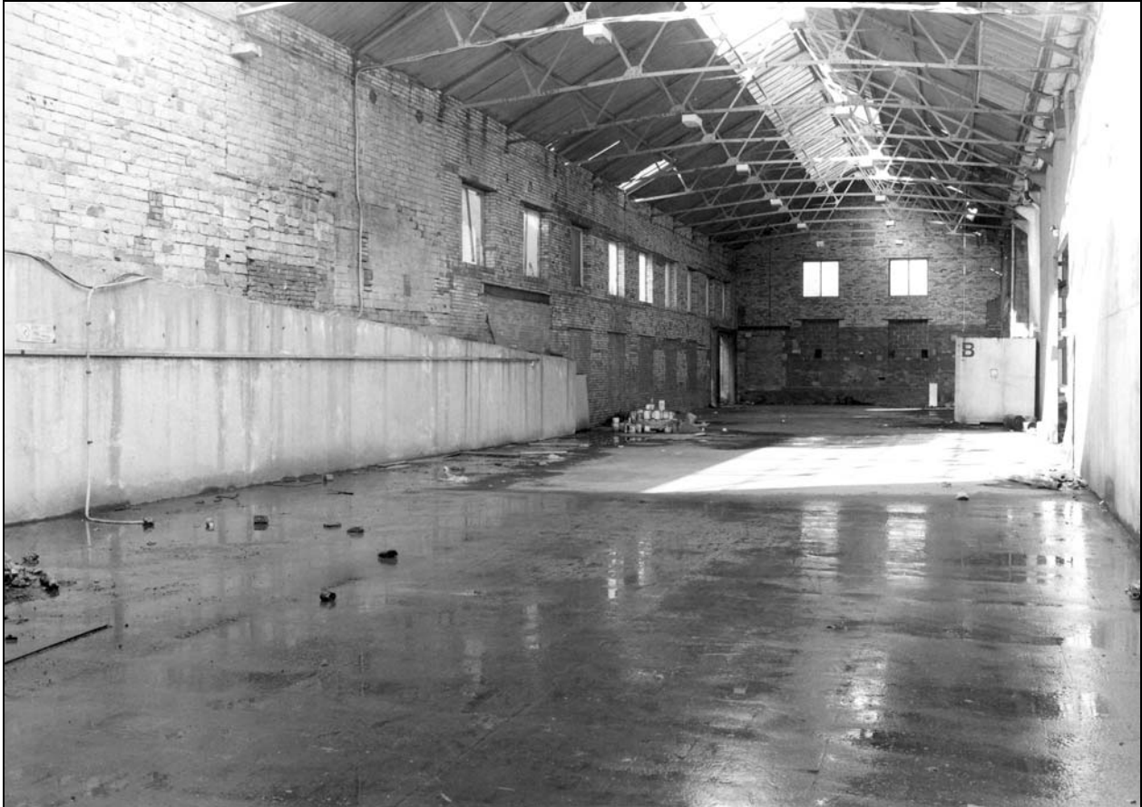
Photo 65: Building 3: interior, from the south-east (film 5, frame 16)
