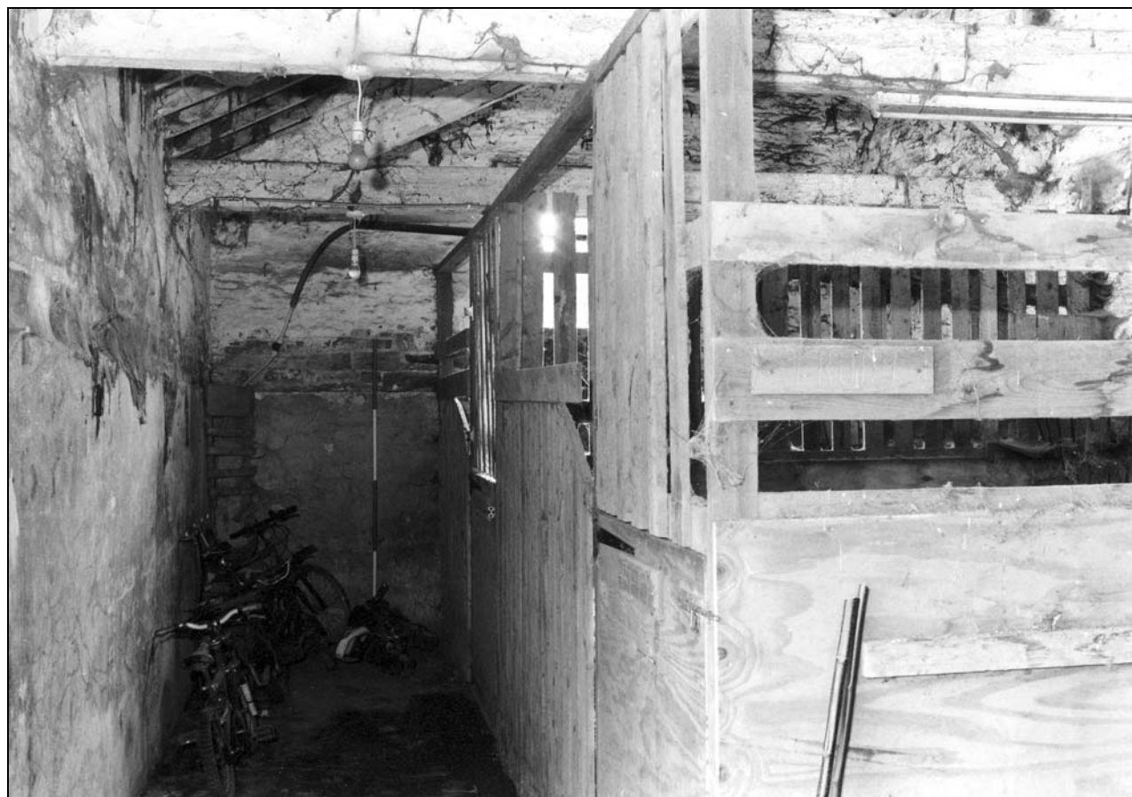
Photo 25: Building 1: east ground floor room, from the north (film 2, frame 2)
