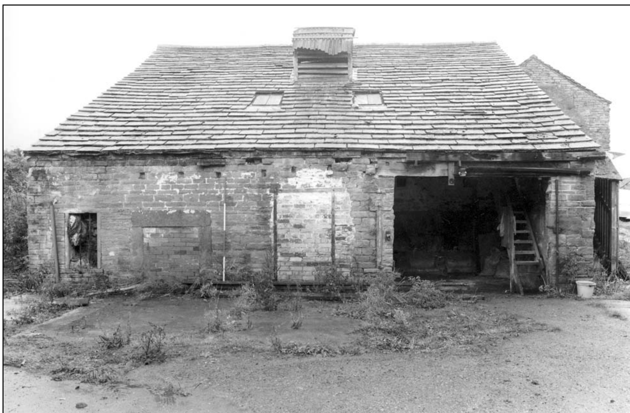
Photo 7: East side of Building 1 (film 1, frame 1)
