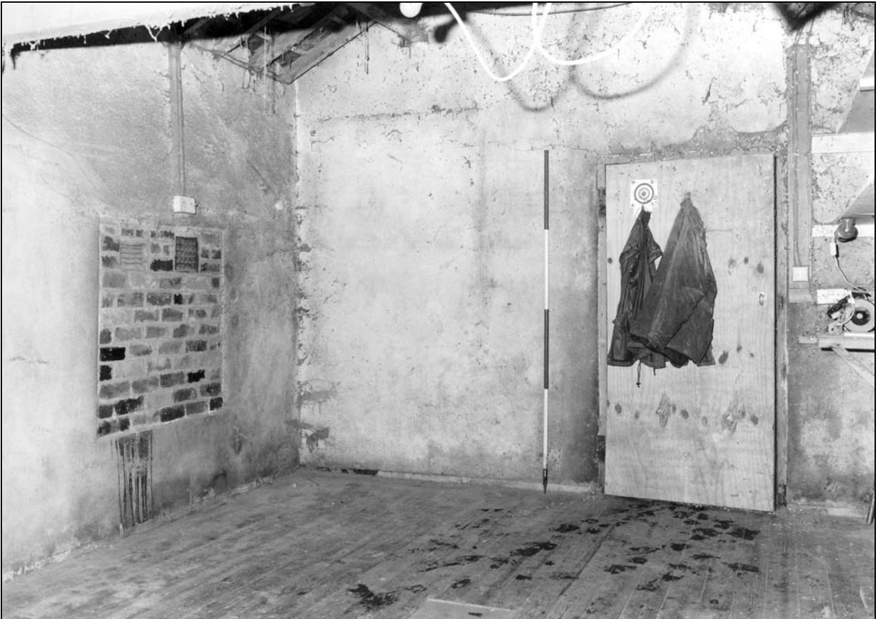
Photo 30: Building 1: upper ground floor room, from the south (film 3, frame 2)
