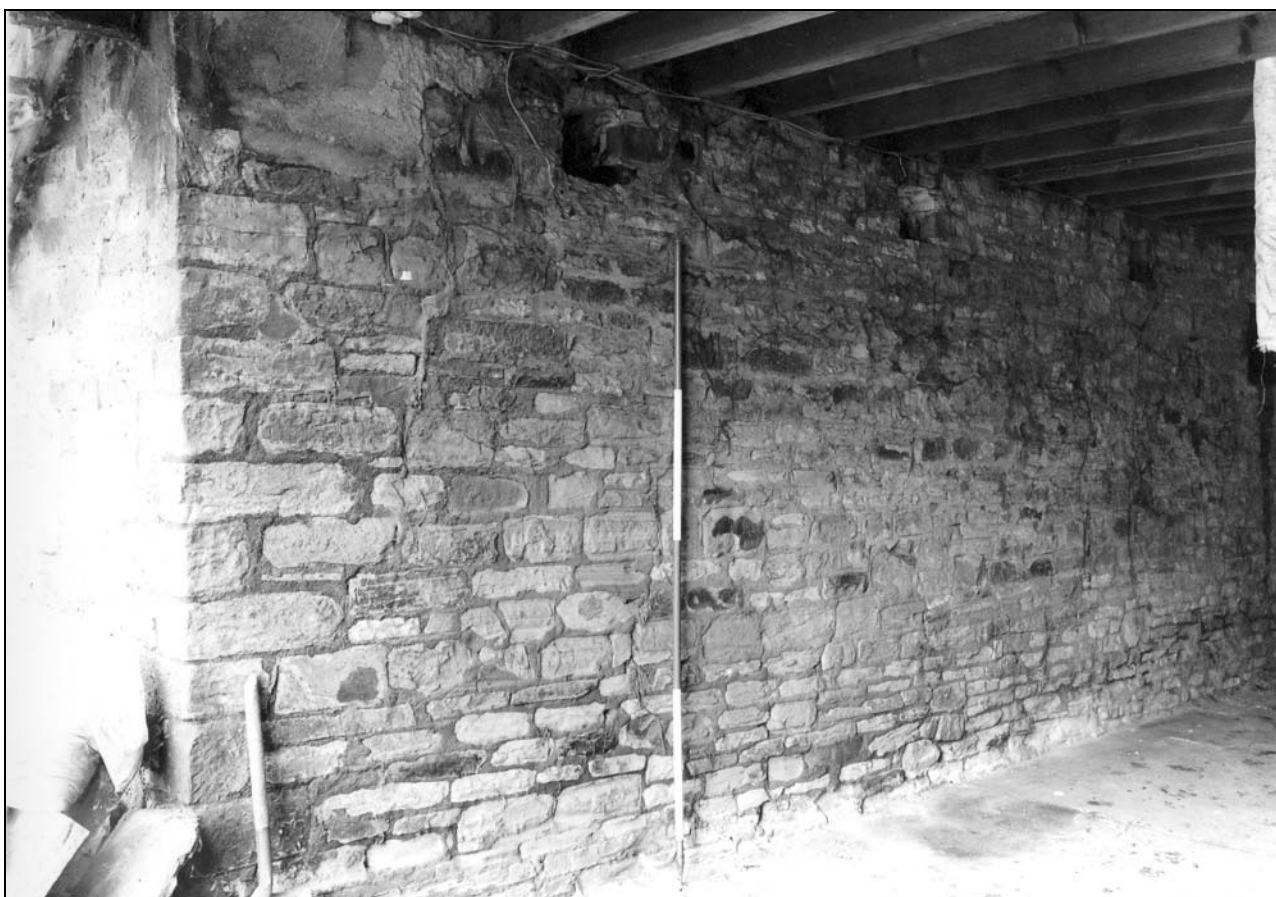
Photo 24: Building 1: east side of west ground floor room (film 2, frame 12)
