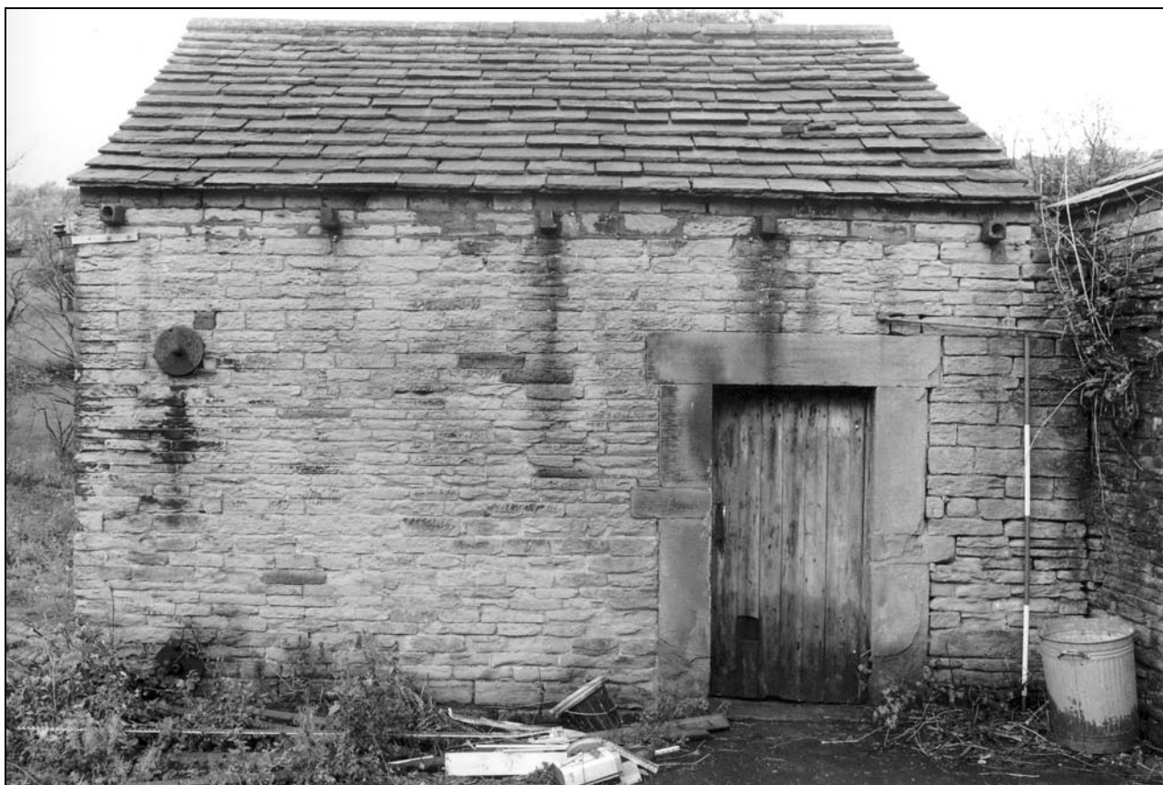
Photo 13: South side of Building 2, at upper ground floor level (film 1, frame 11)
