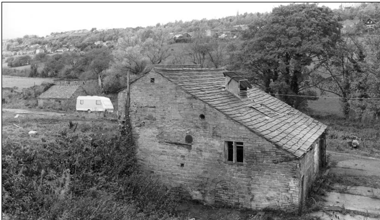
Photo 4: Building 1, from the south-east (film 1, frame 13)
