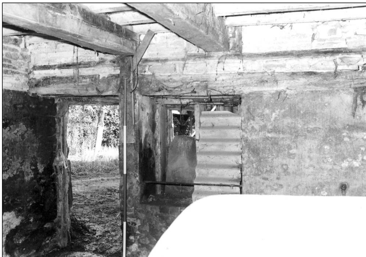
Photo 33: Building 2: ground floor, from the south-west (film 2, frame 16)
