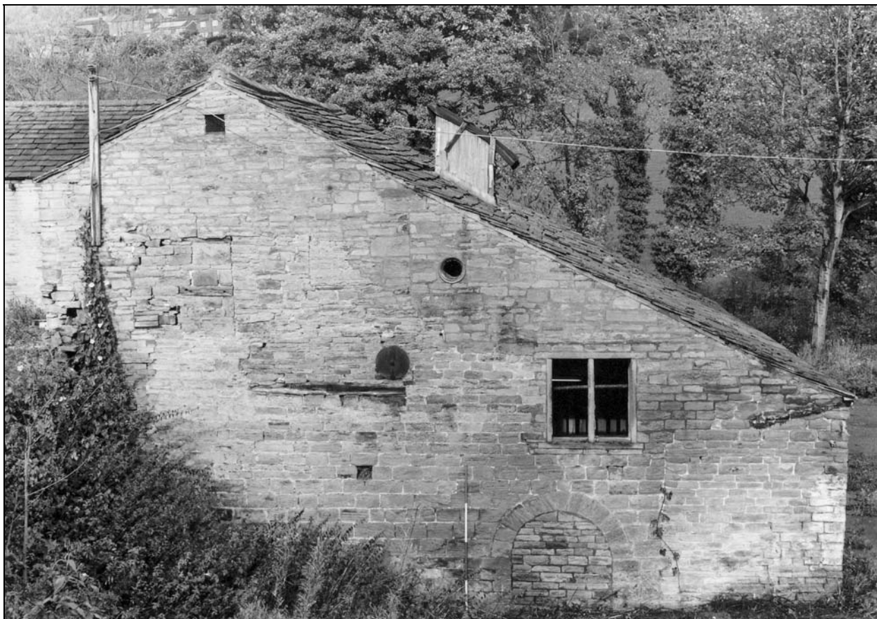
Photo 6: South gable of Building 1, from the south (film 1, frame 14)
