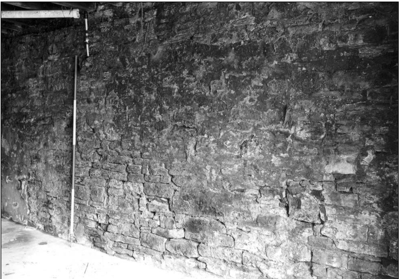
Photo 23: Building 1: west side of west ground floor room (film 2, frame 11)
