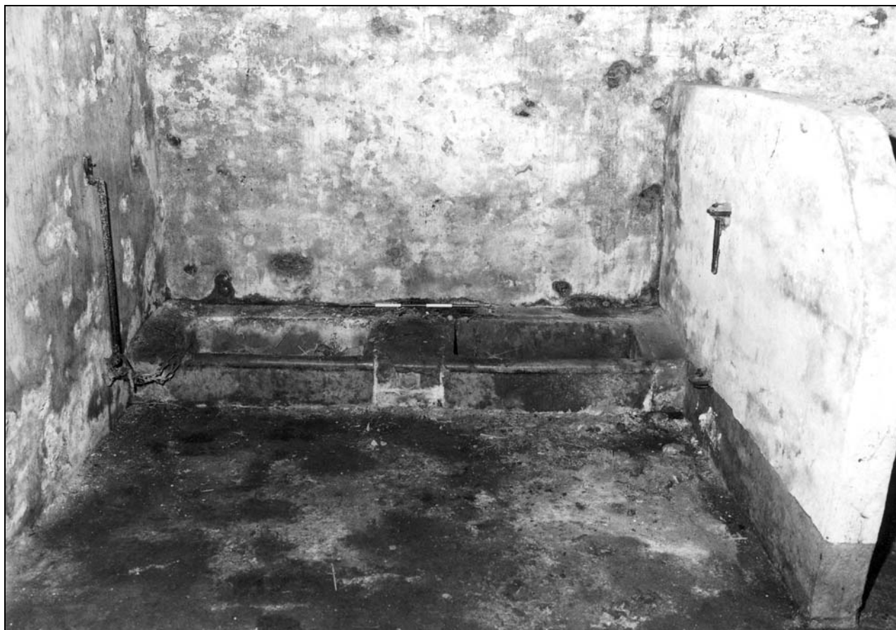
Photo 32: Building 2: cattle stall on ground floor, from the north (film 2, frame 17)
