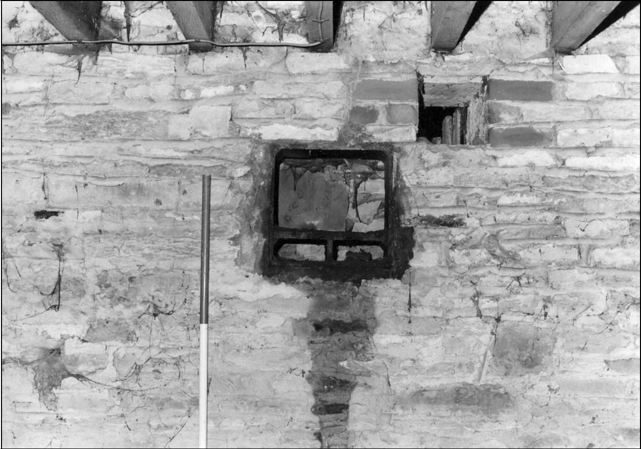
Photo 22: Building 1: detail of bearing box, east side of west ground floor room (film 2, frame 13)
