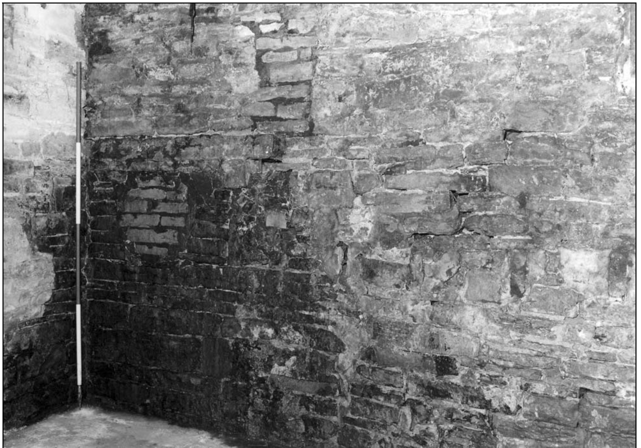
Photo 19: Building 1: south-west corner of west ground floor room (film 2, frame 7)
