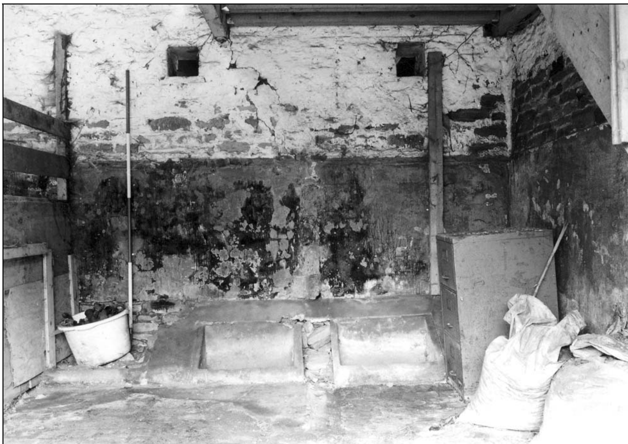
Photo 26: Building 1: cattle troughs in east ground floor room, from the east (film 1, frame 18)
