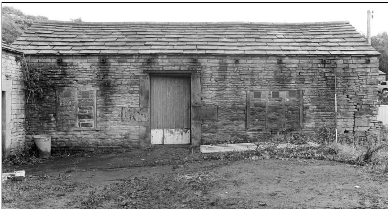
Photo 10: West side of Building 1, at upper ground floor level (film 1, frame 10)
