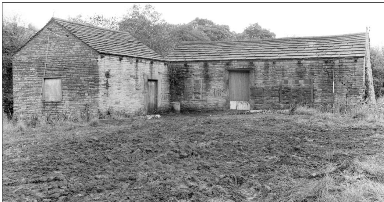
Photo 9: General view of the buildings, from the west, at upper ground floor level (film 1, frame 8)
