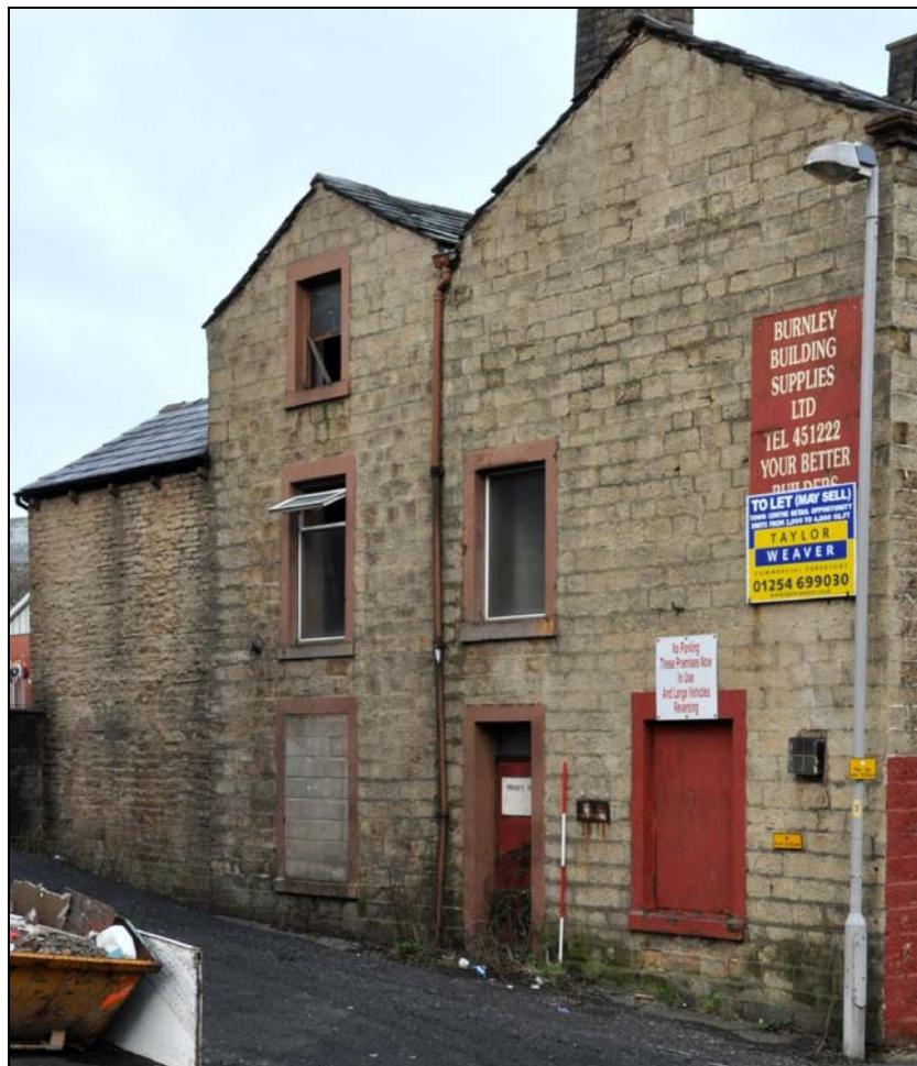
Photo 2: South-east side of Building 1, from the south-east
