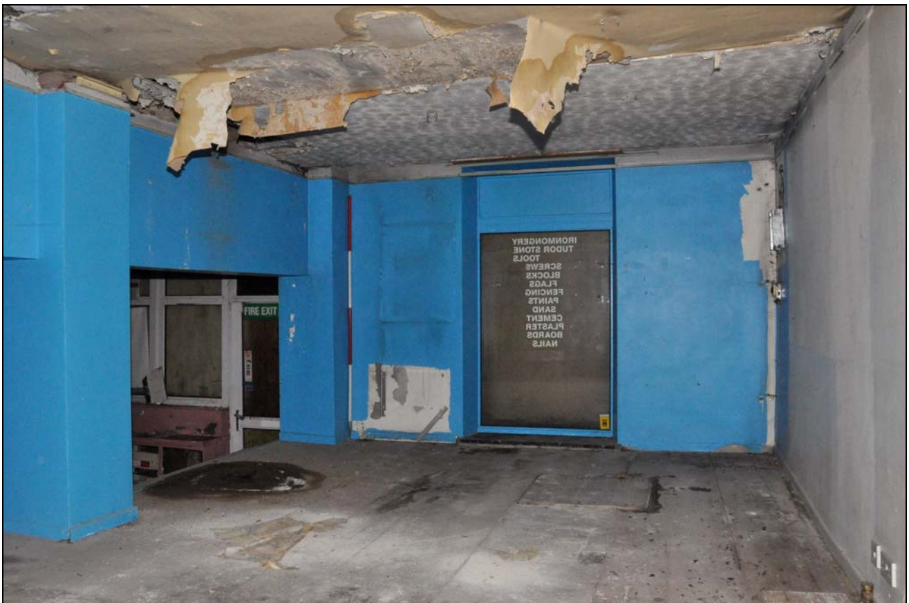
Photo 10: Building 1 – interior on ground floor, phases 1 and 2, from the south-west
