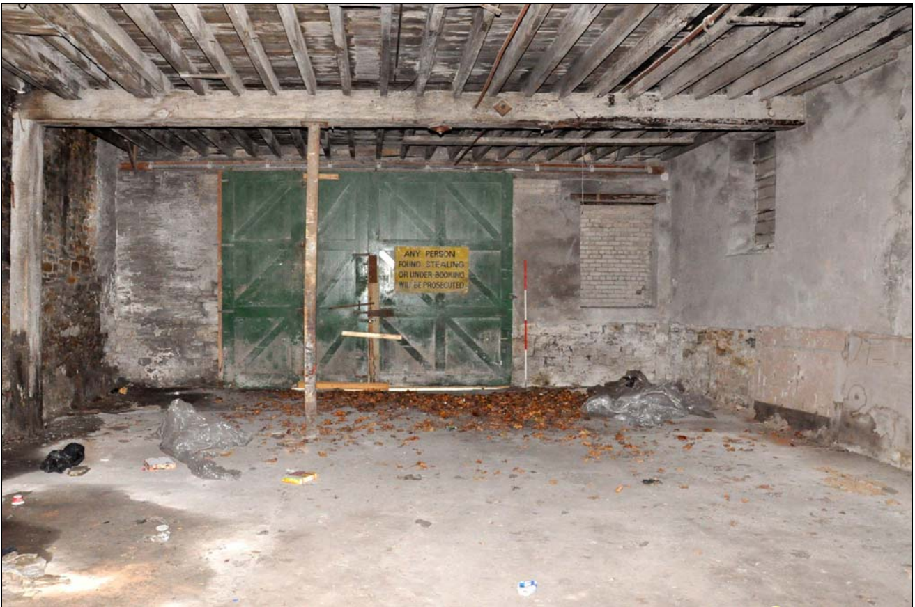
Photo 36: Building 2 – ground floor, from the south-east
