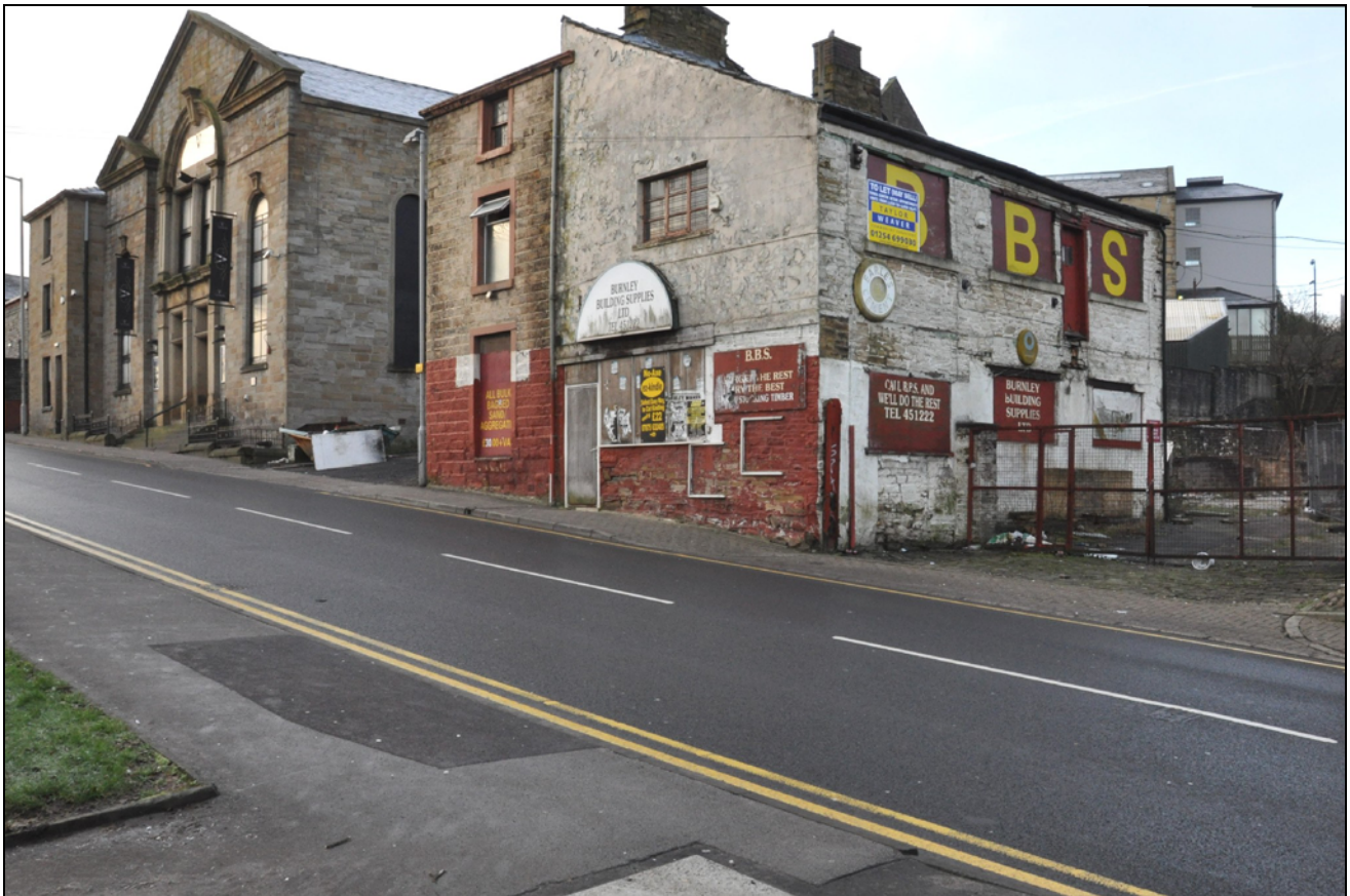
Photo 4: Building 1, from the north, across Hammerton Street, with former Mount Pleasant Chapel beyond
