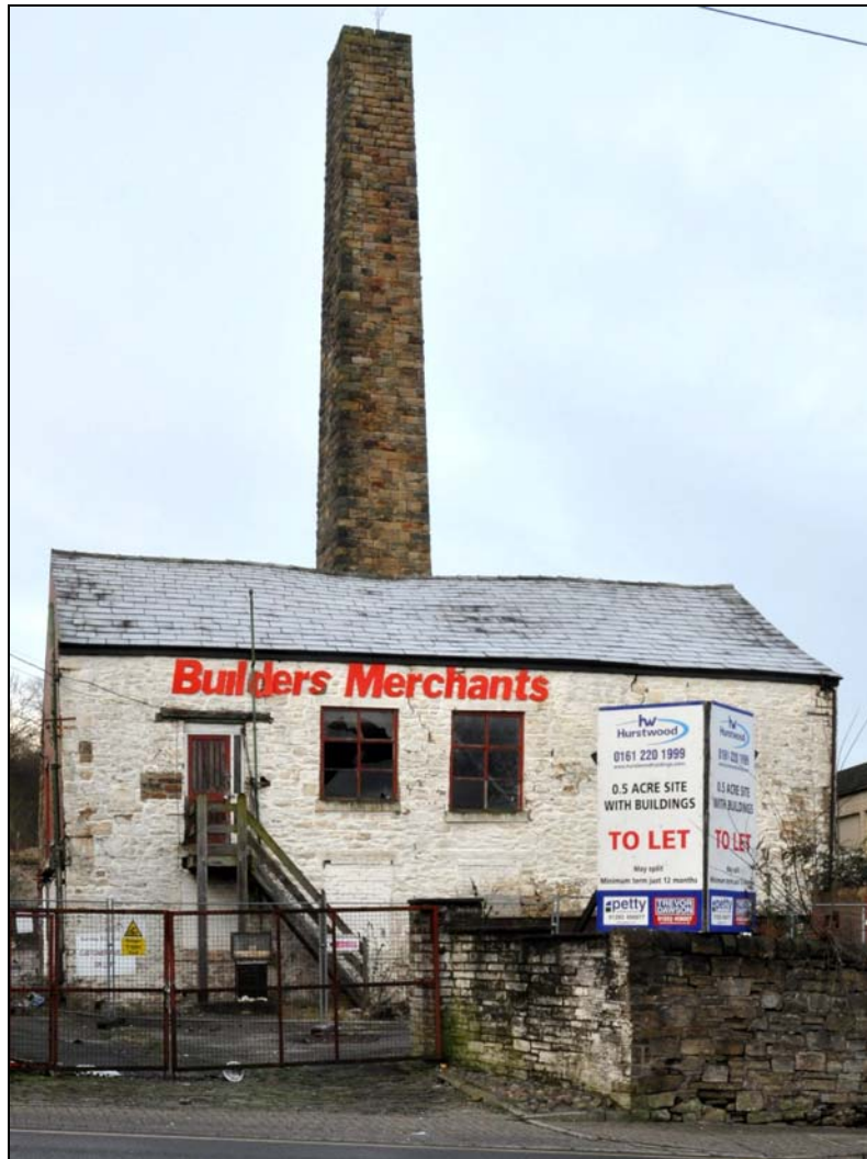
Photo 24: Building 2 – general view from the north-east, across Hammerton Street
