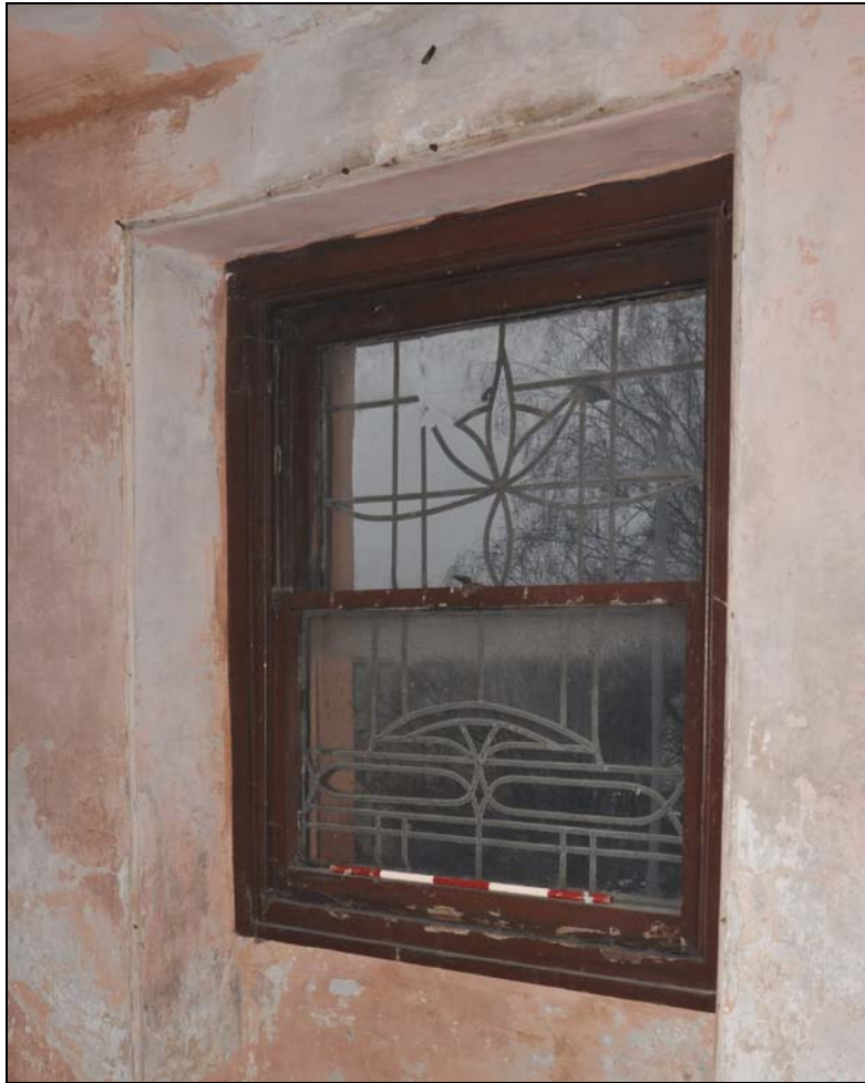
Photo 21: Building 1 – detail of window, second floor, front room (phase 1)
