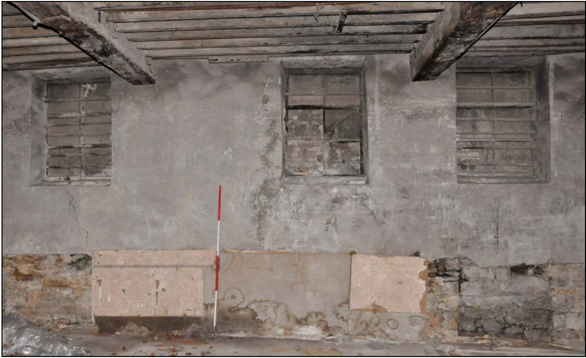
Photo 37: Building 2 – ground floor, from the south-west
