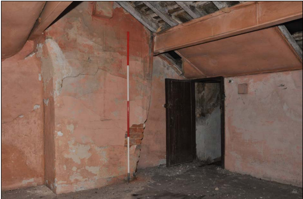
Photo 22: Building 1 – second floor, back room (phase 2), from the south
