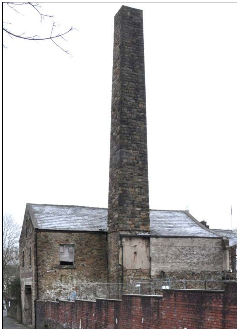
Photo 30: Building 2 – general view from the west, across Mount Pleasant Street
