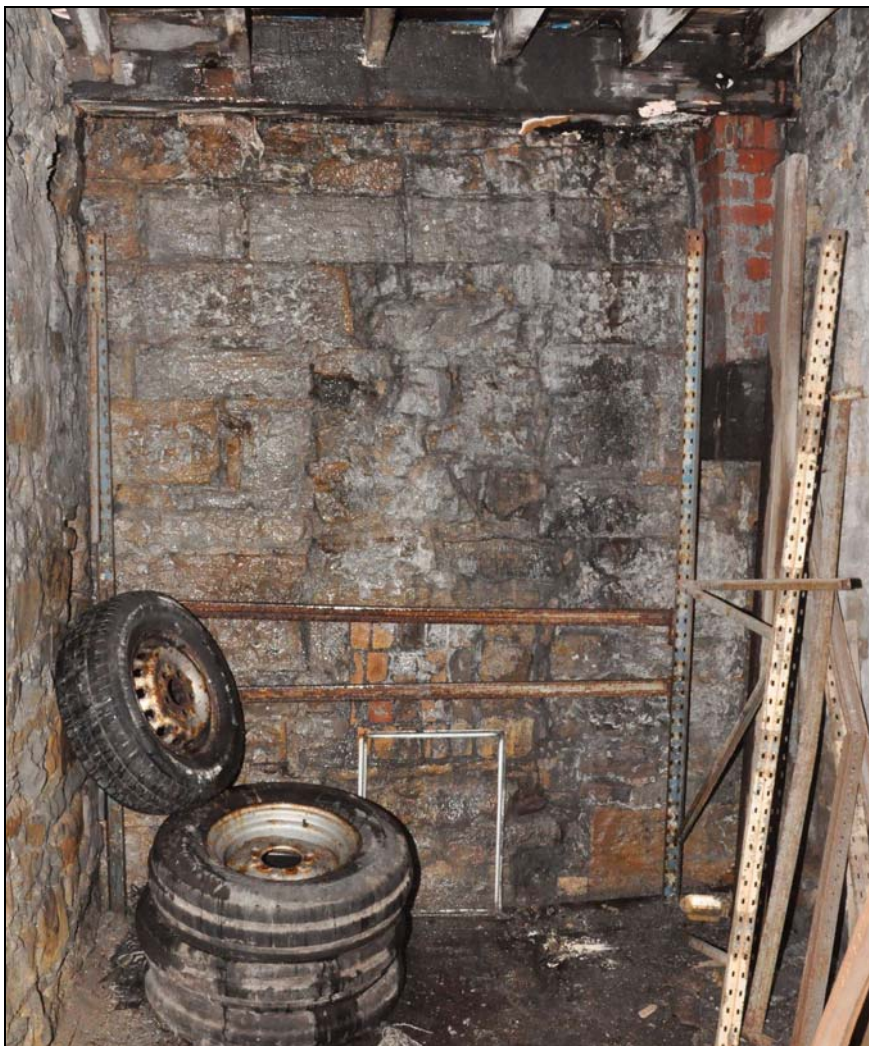
Photo 44: Building 2 – boiler/engine room, from the south-east
