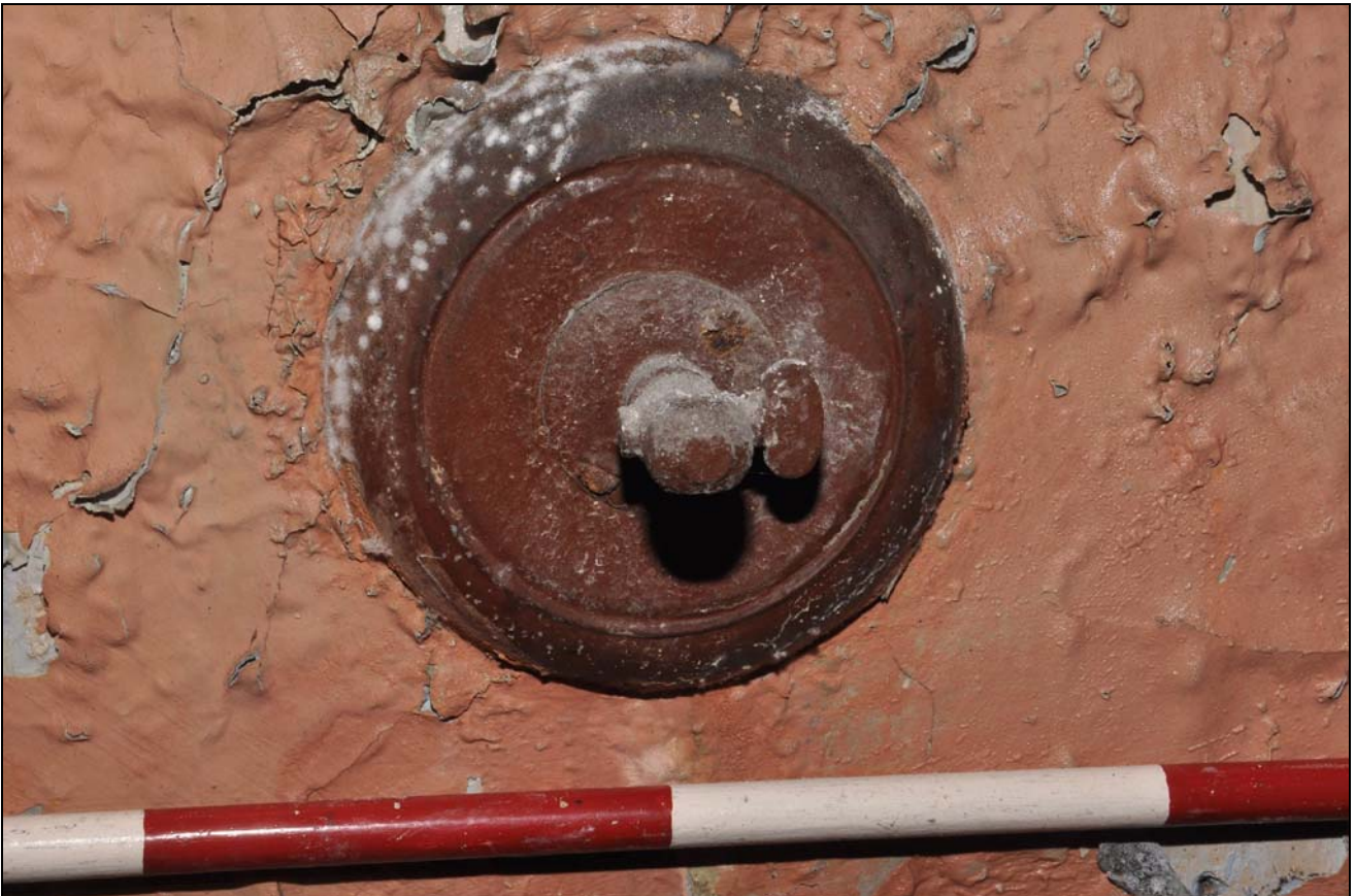
Photo 19: Building 1 – detail of gas light bracket, second floor, front room (phase 1)
