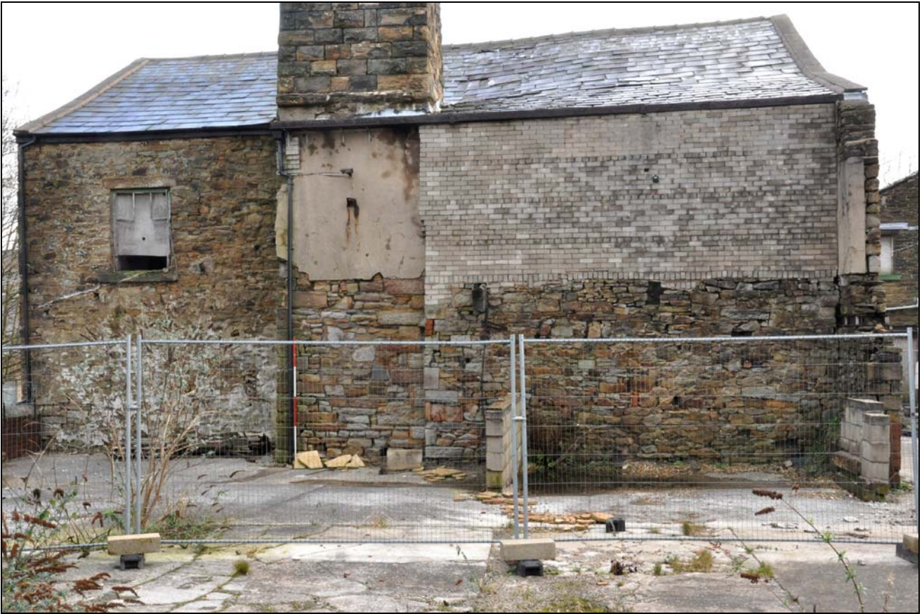
Photo 31: Building 2 – south-west elevation of mill
