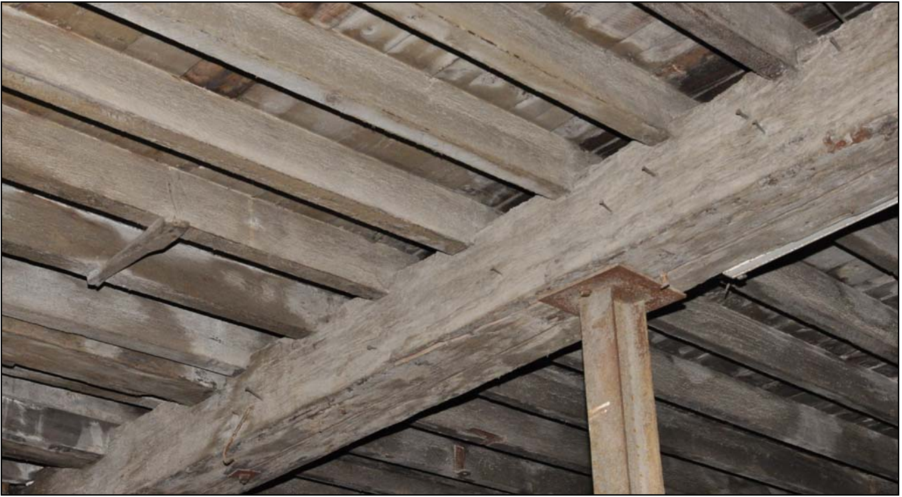
Photo 42: Building 2 – underside of first floor
