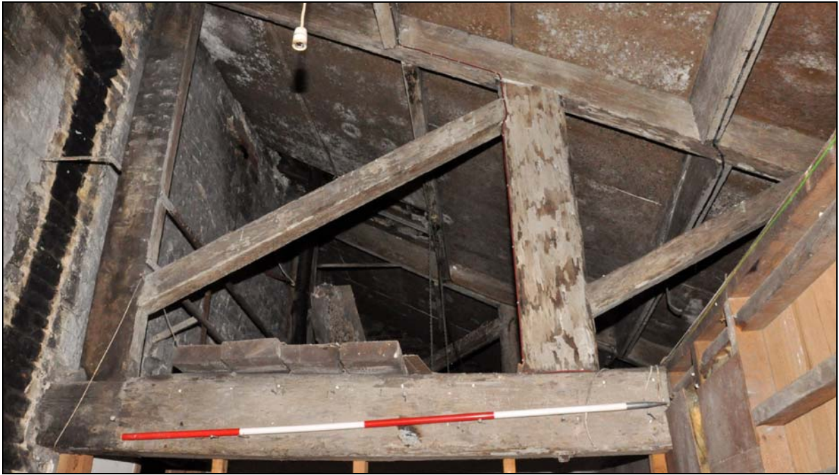
Photo 15: Building 1 – raking truss over first floor of phase 3, from the north-east
