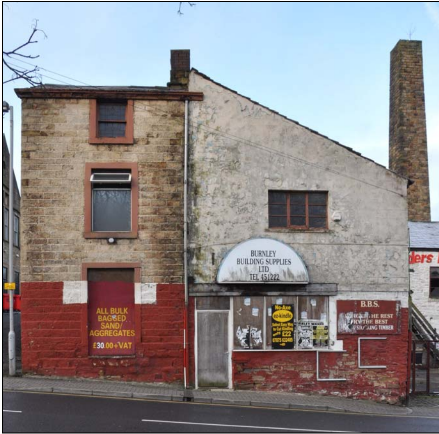
Photo 3: Building 1, from the north-east, across Hammerton Street
