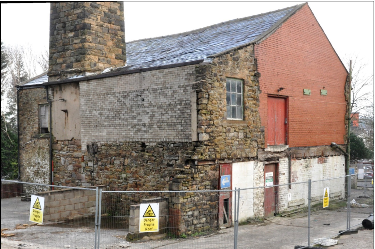
Photo 33: Building 2, from the south
