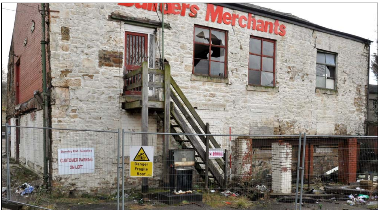
Photo 26: Building 2 – north-east elevation
