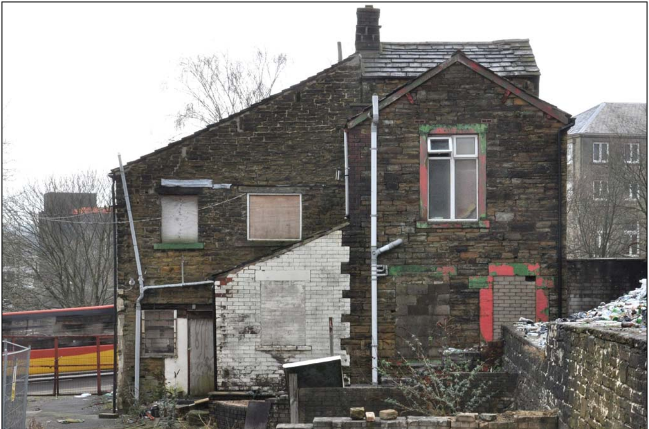
Photo 7: Building 1, from the south-west
