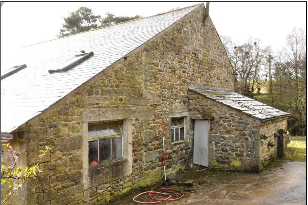
Photo 9: The barn, from the north-east
