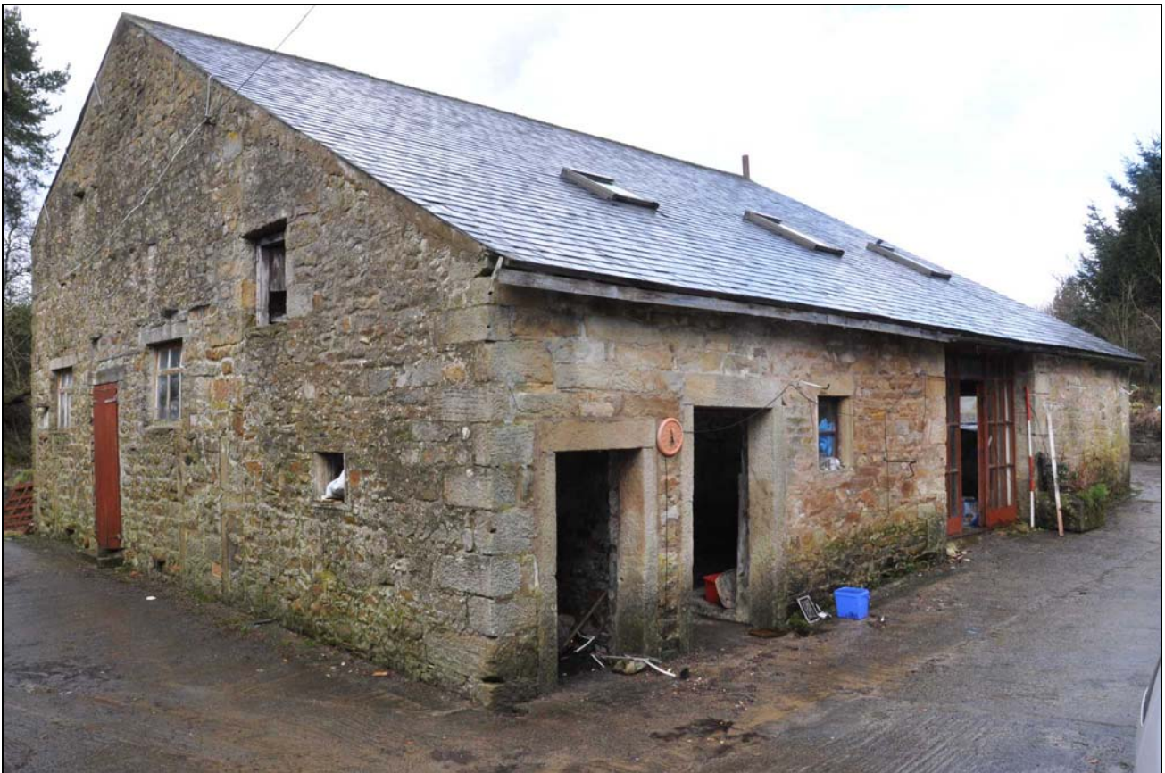
Photo 2: The barn, from the south-east
