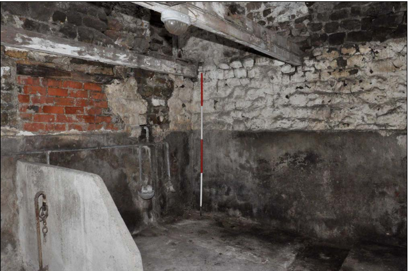
Photo 28: Former stable in outshut, from the south-east
