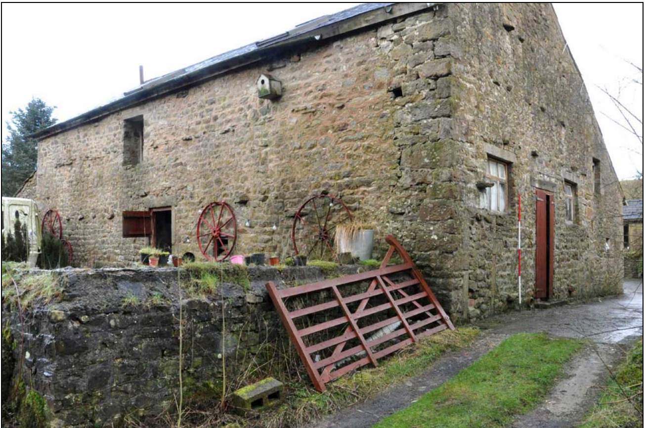
Photo 4: The barn, from the south-west
