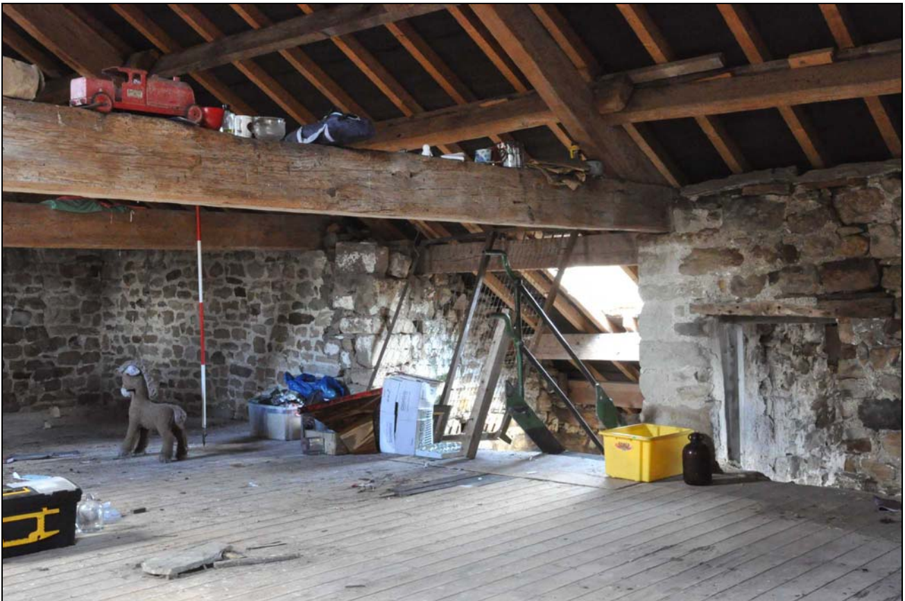
Photo 19: Interior of barn, first floor, north-east corner, towards porch
