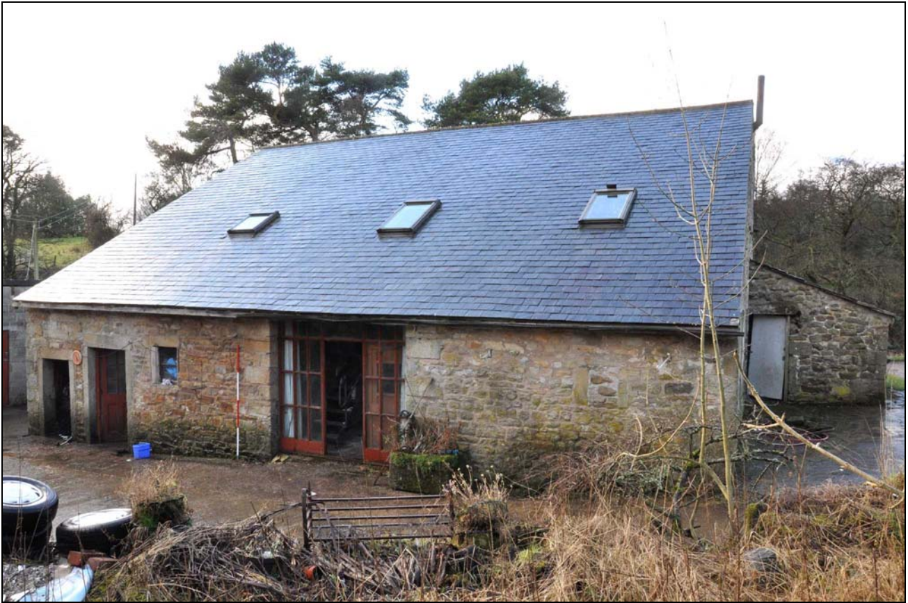
Photo 1: The barn, from the north-east
