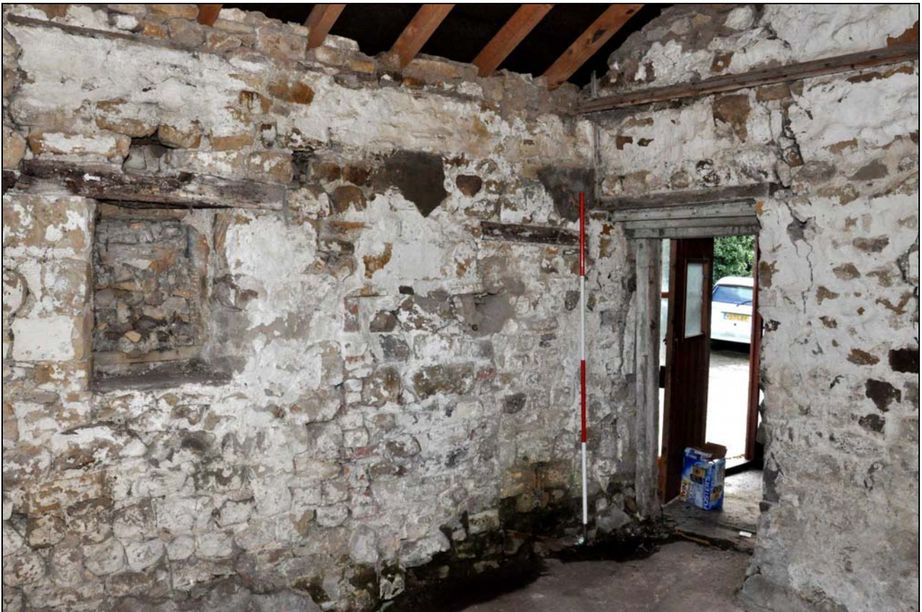
Photo 31: Interior of north-east outshut, from the north-west
