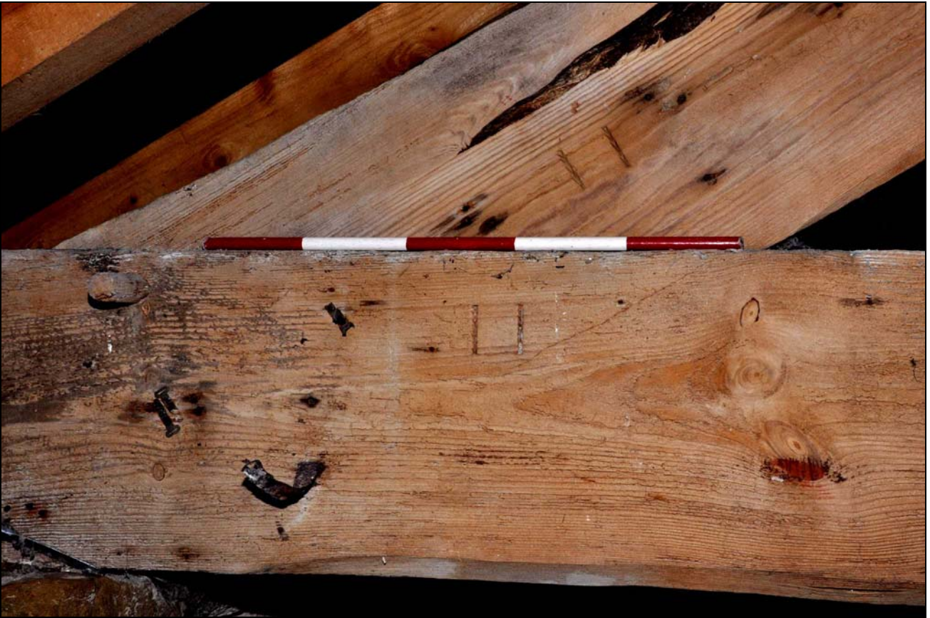
Photo 24: Detail of numbering at east end of middle roof truss, north side of tie beam
