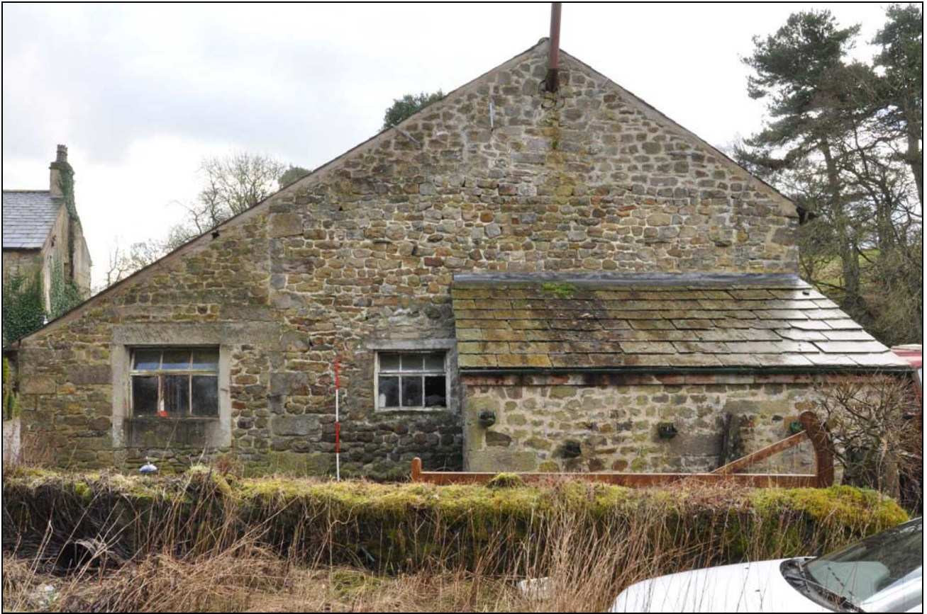
Photo 3: The barn, from the north
