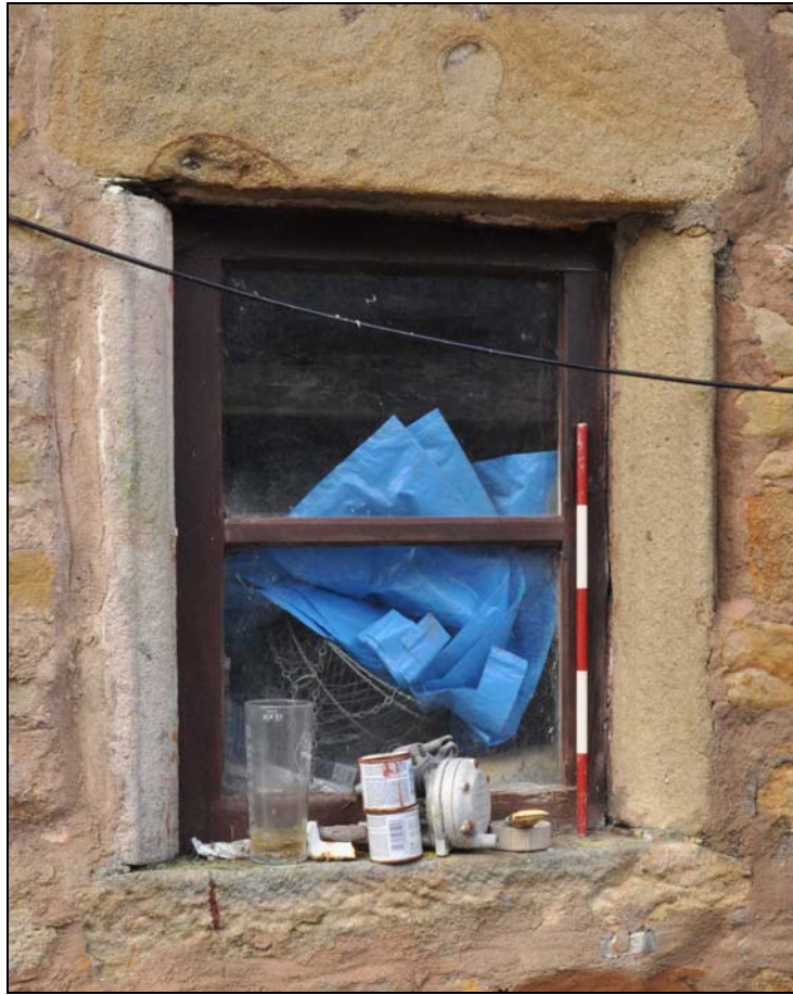
Photo 10: Detail of window with re-used mullions, in east elevation of stable
