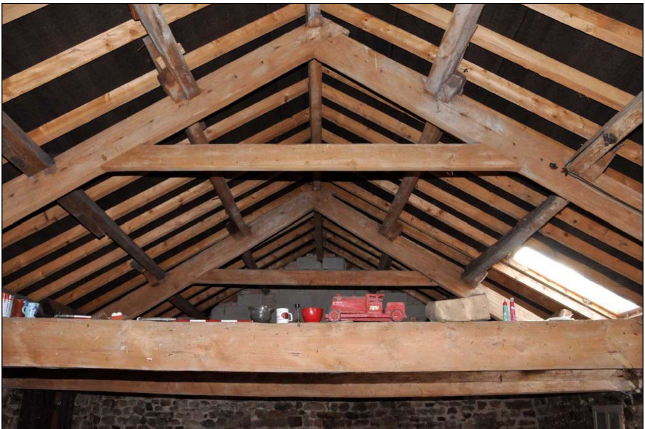
Photo 21: Middle roof truss in barn, from the north
