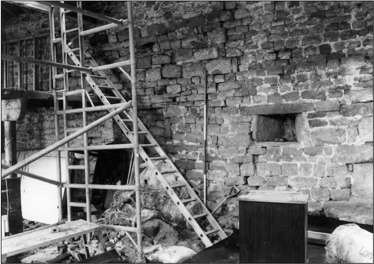
Photo 6: Interior of the barn, from the south-east (film 1, frame 13)
