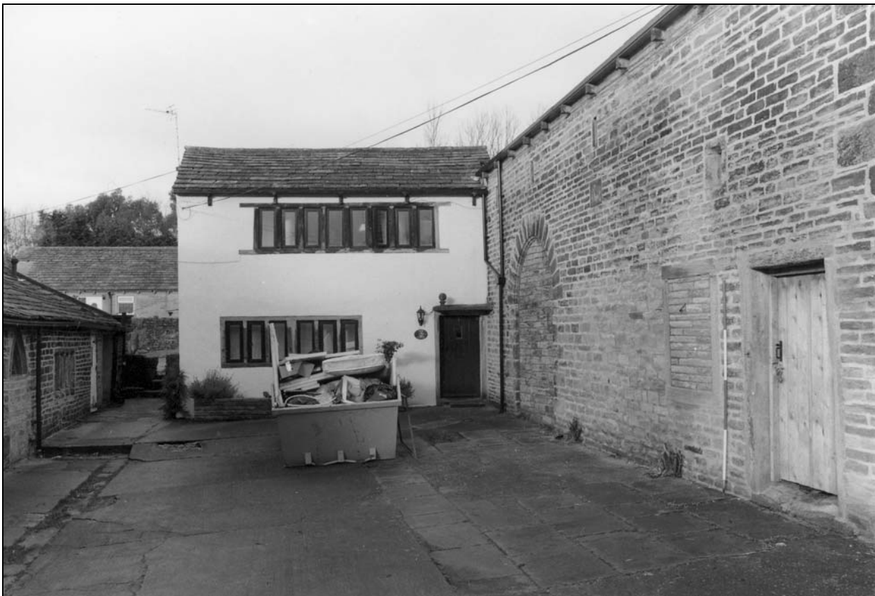
Photo 5: Building 1 (barn) and adjoining cottage, from the east (film 1, frame 8)
