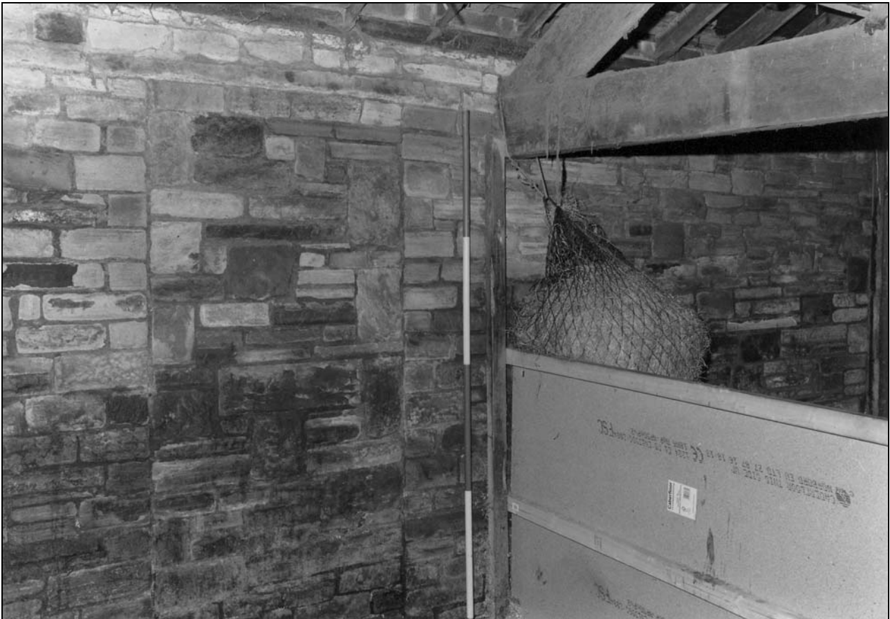
Photo 28: Building 2: blocked doorway in west wall, from the south-east (film 3, frame 10)
