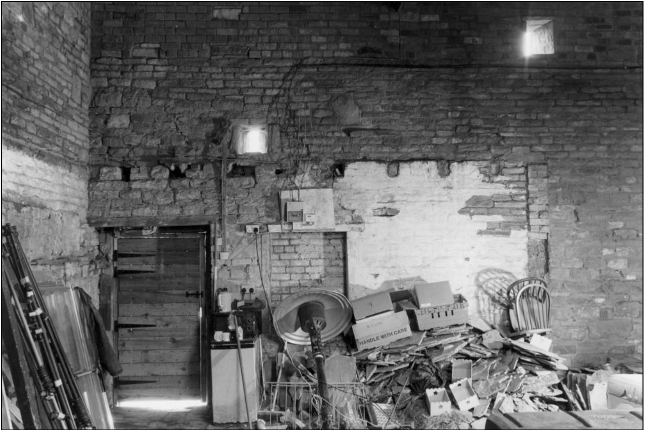
Photo 20: Building 1 (barn): interior, from the north-east corner, showing outline of former mistal in south wall (film 3, frame 14)
