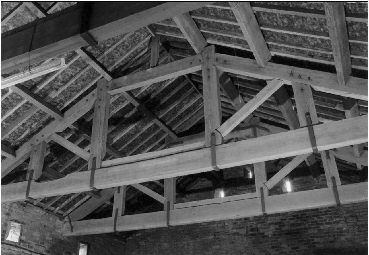
Photo 23: Building 1 (barn): roof trusses, from the north-east (film 1, frame 2)
