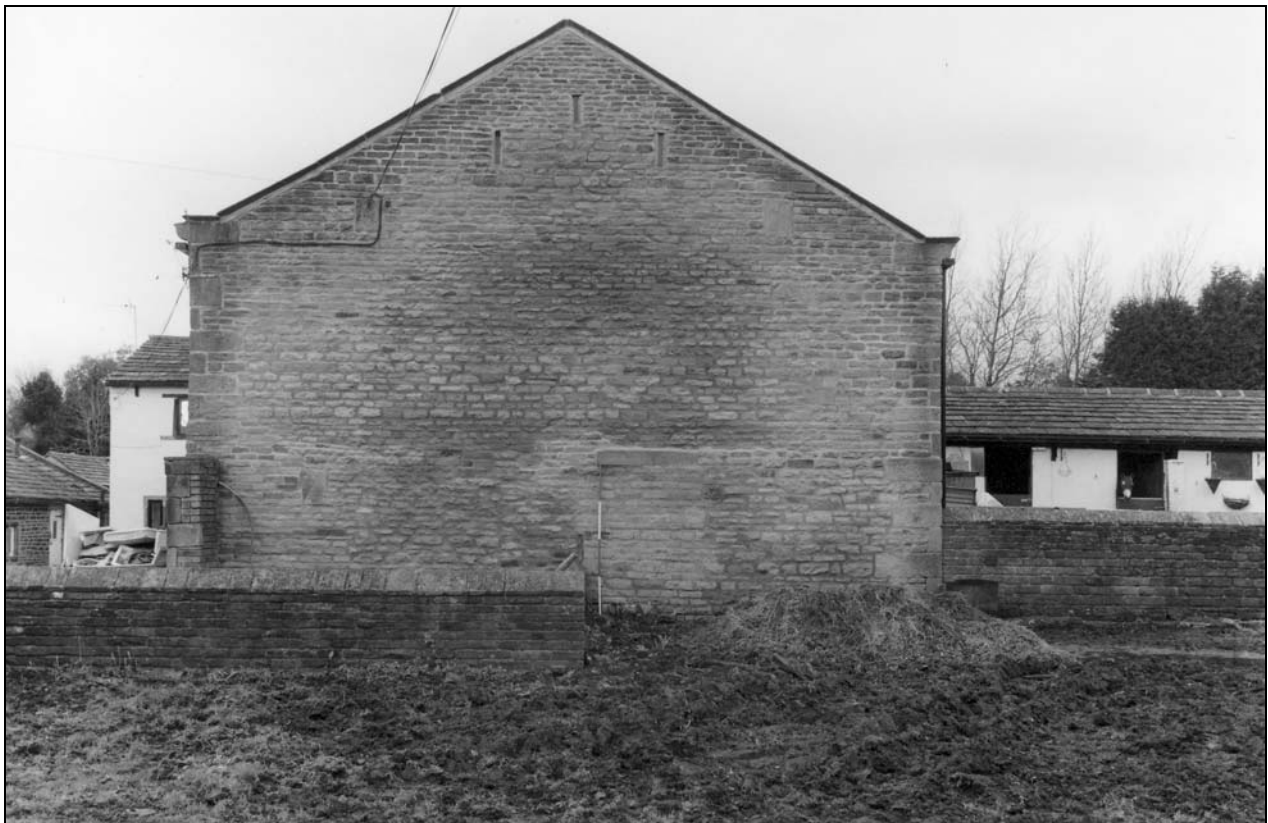
Photo 10: Building 1 (barn): east gable (film 1, frame 12)
