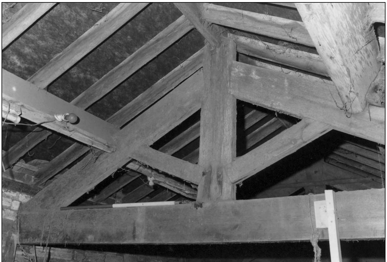
Photo 29: Building 2: roof truss, from the south-east (film 3, frame 11)
