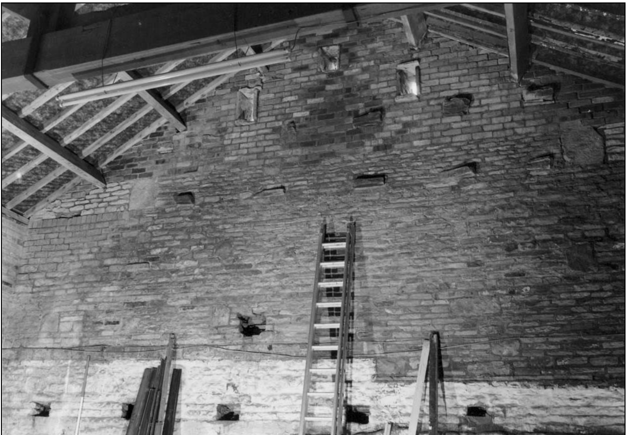
Photo 19: Building 1 (barn): interior view of east gable (film 1, frame 5)
