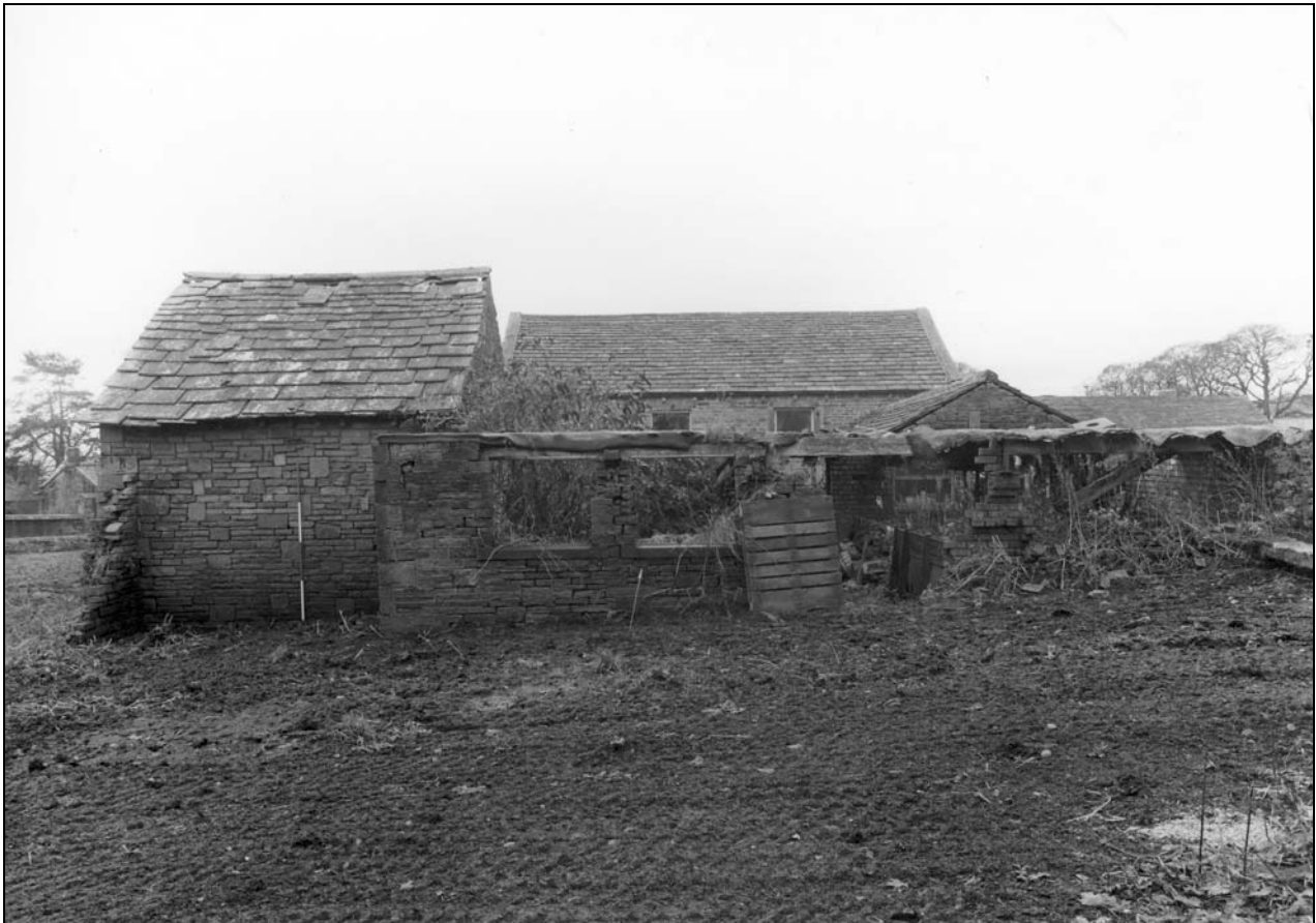
Photo 31: Buildings 3 & 4, from the north (film 2, frame 5)
