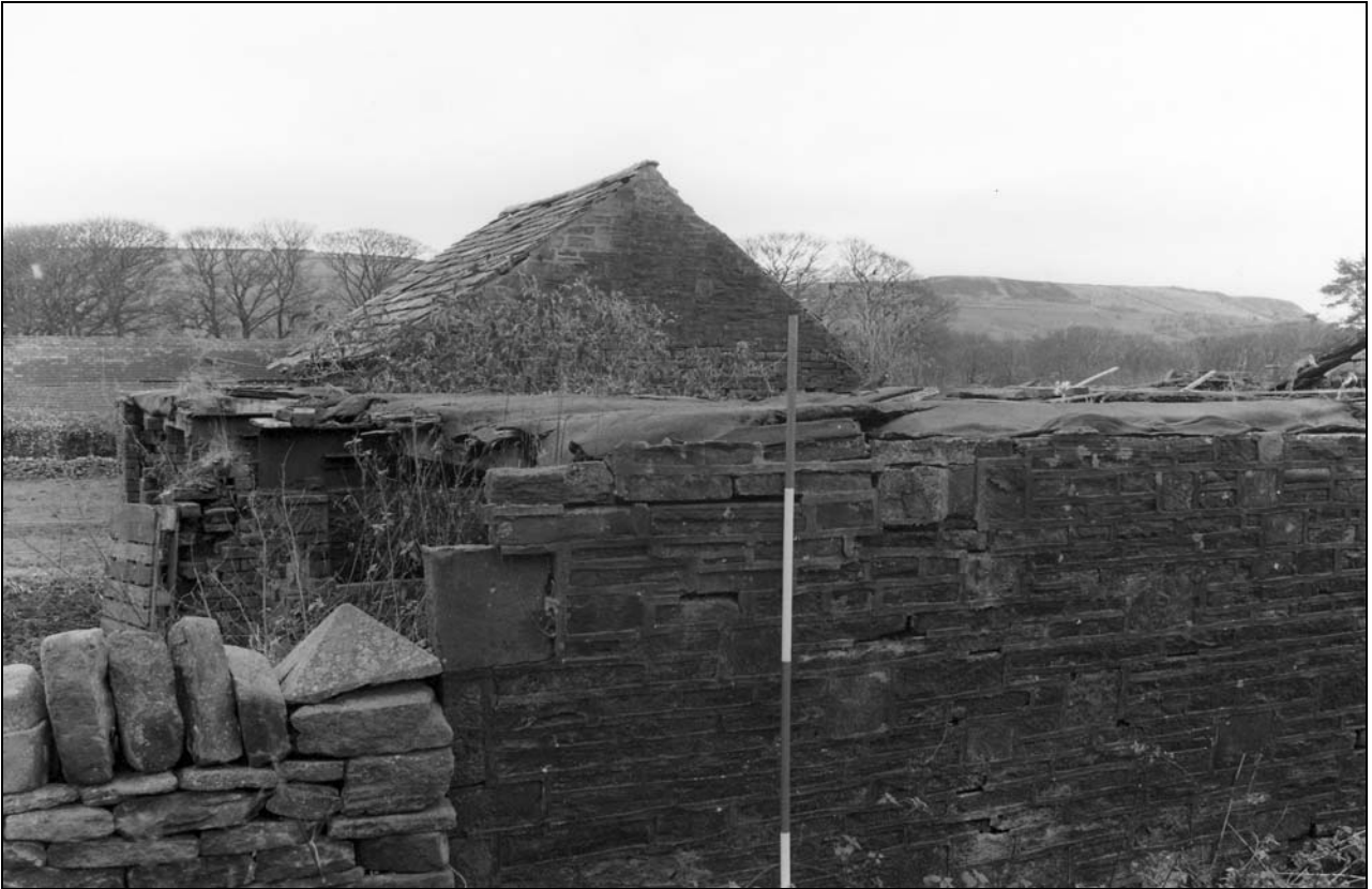
Photo 32: Buildings 3 & 4, from the north-west (film 2, frame 7)
