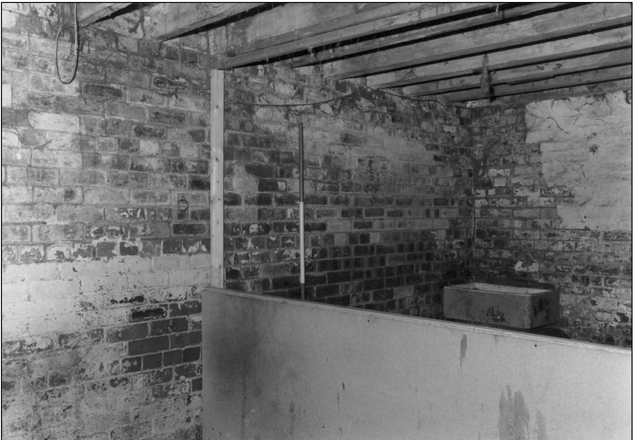
Photo 43: Building 4: interior, from the north-west (film 3, frame 7)
