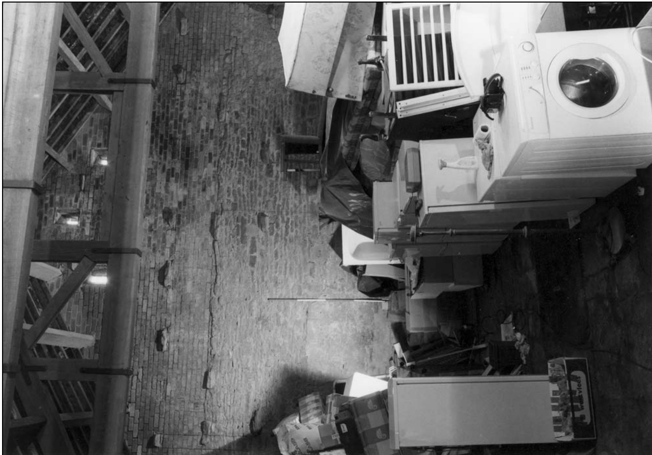
Photo 24: Building 1 (barn): interior, from the east (film 3, frame 16)
