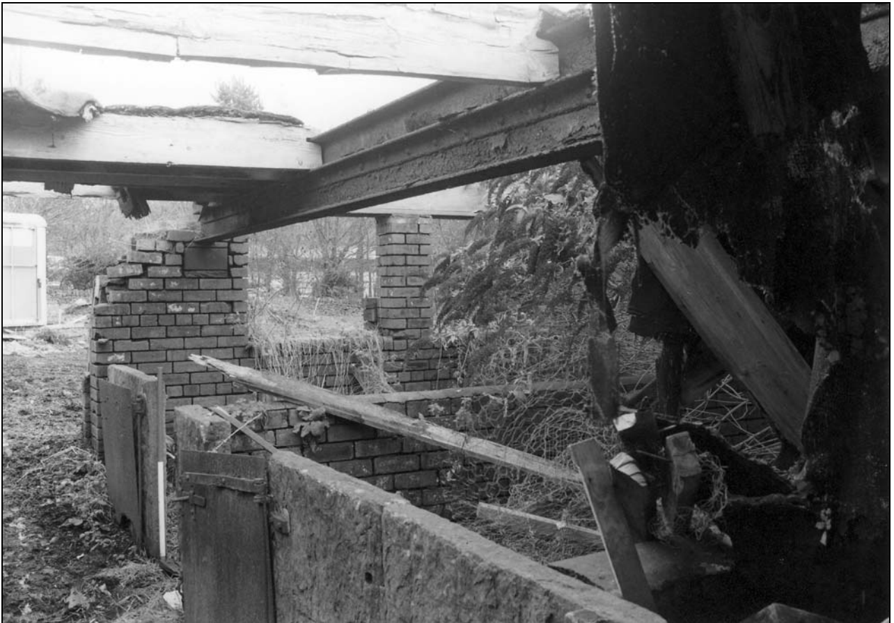
Photo 37: Building 3: interior, from the south-west (film 3, frame 4)
