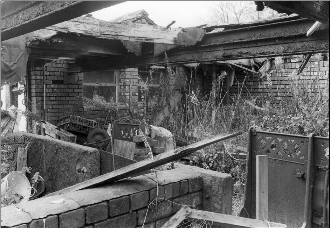
Photo 38: Building 3: interior, from the north-east (film 2, frame 18)
