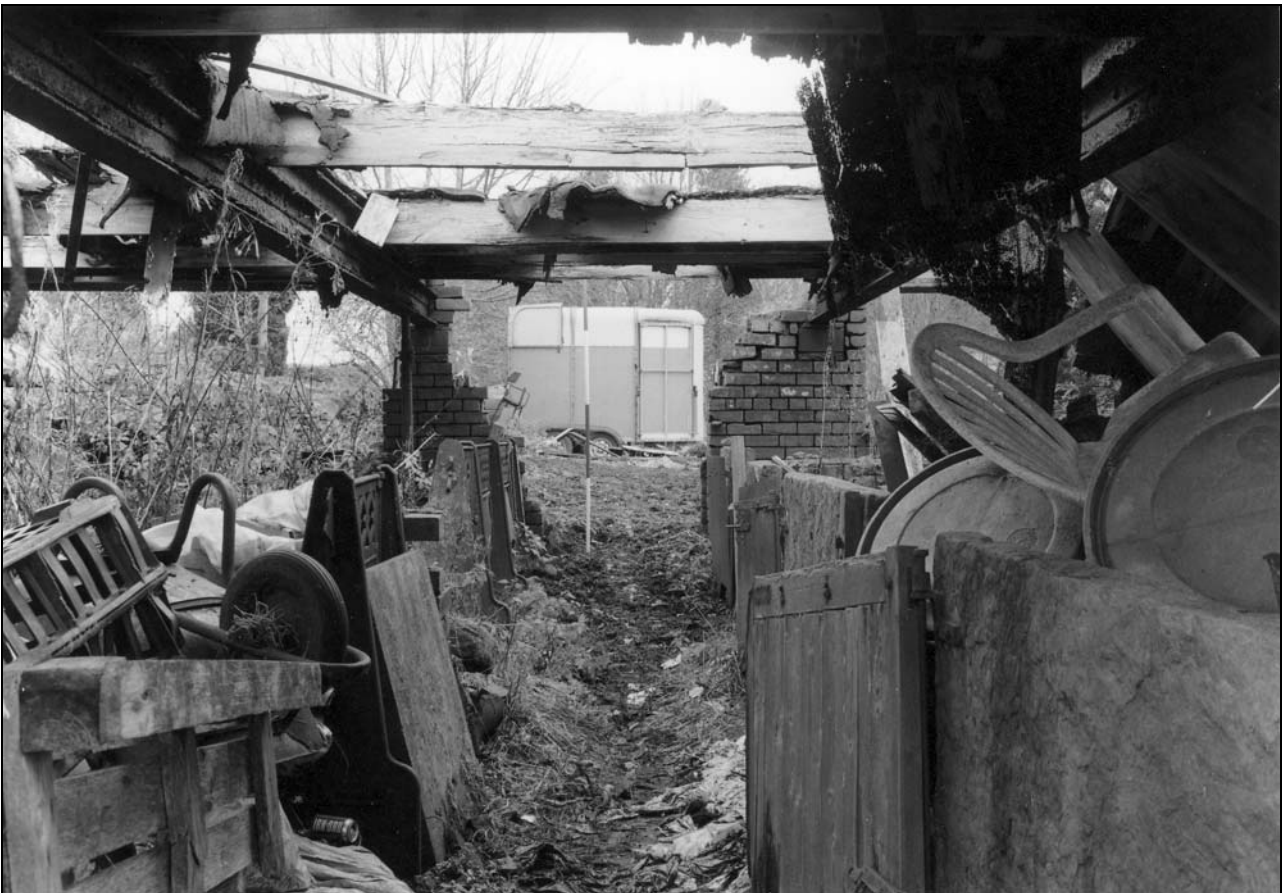
Photo 33: Building 3: feeding passage, from the south (film 2, frame 15)
