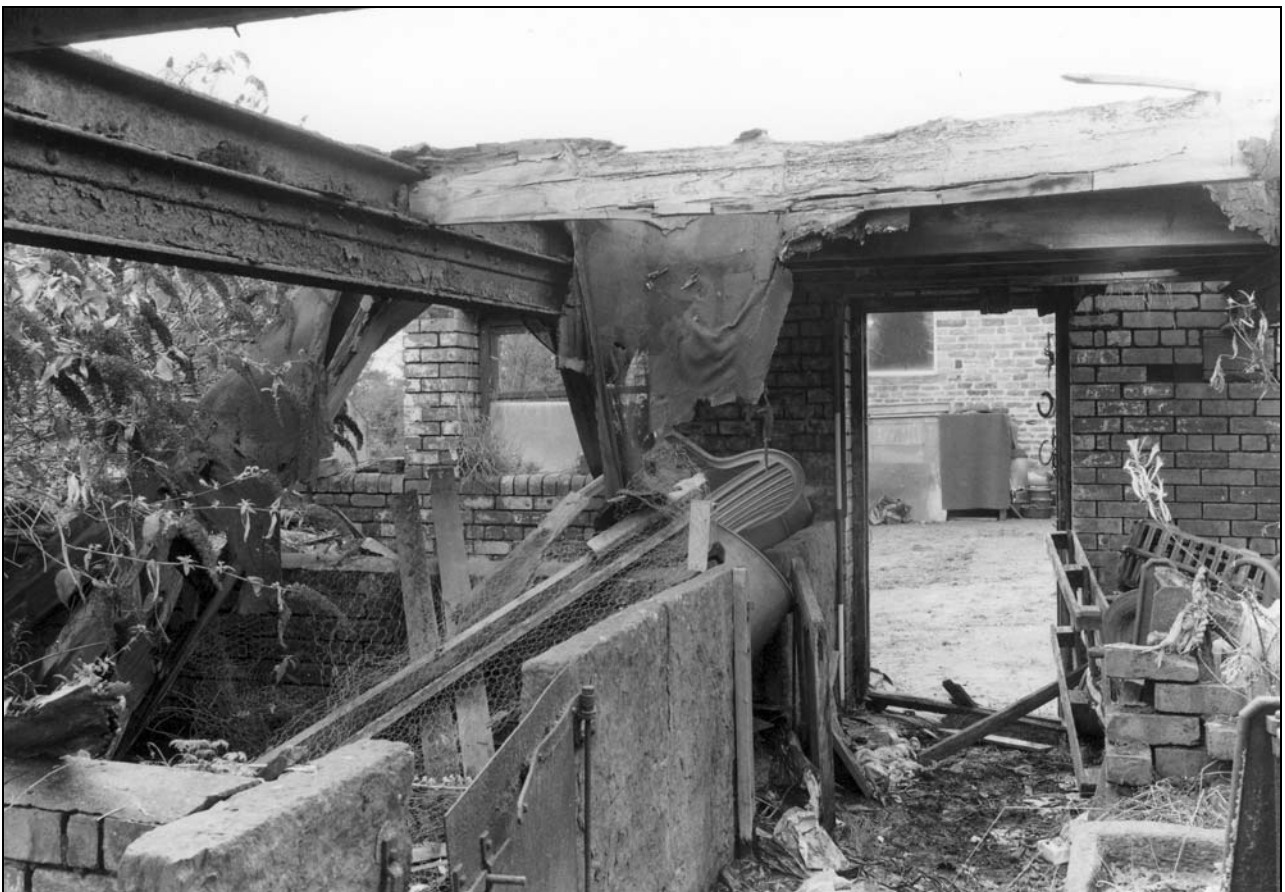
Photo 35: Building 3: interior, from the north-west (film 3, frame 6)
