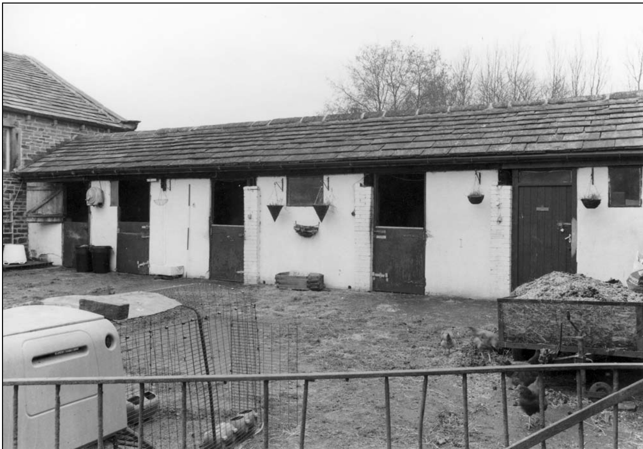
Photo 25: Building 2, from the north-east (film 1, frame 18)
