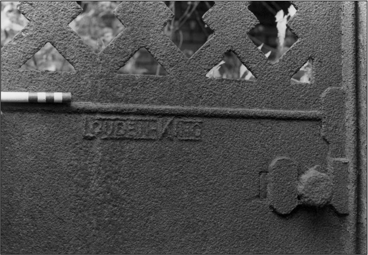
Photo 40: Building 3: detail of foundry mark "Ouden King" (?) on cast iron pig pen gate (film 3, frame 5)
