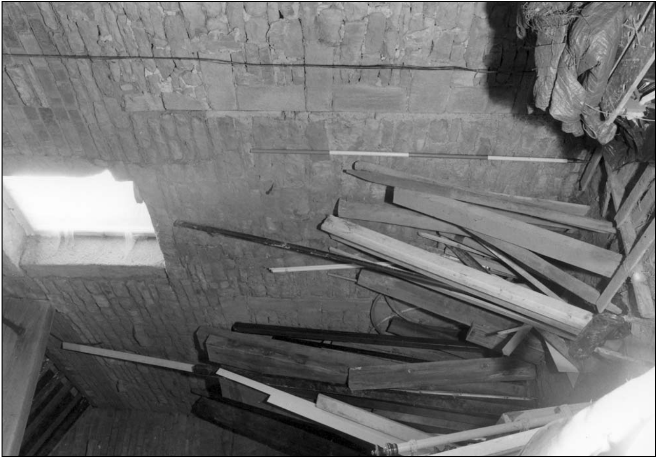
Photo 18: Building 1 (barn): interior view of blocked cart entrance, north wall (film 1, frame 1)
