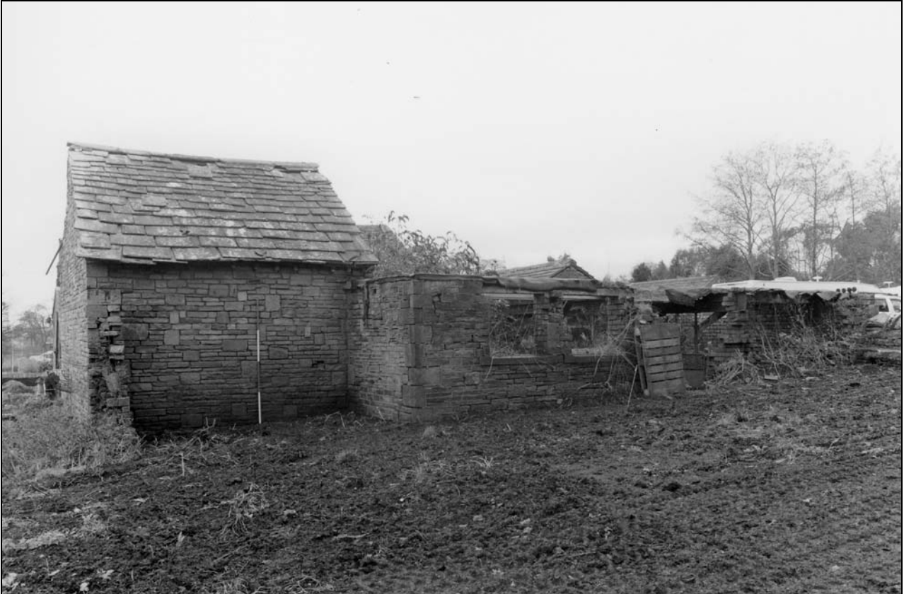
Photo 42: Buildings 3 & 4, from the north-east (film 2, frame 4)
