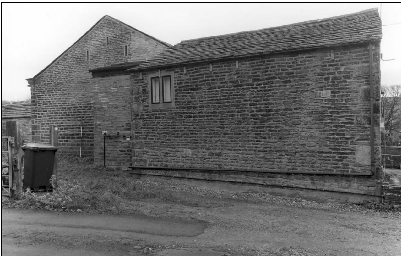
Photo 14: Building 1 (barn) and adjoining cottage, from the south-west (film 2, frame 11)
