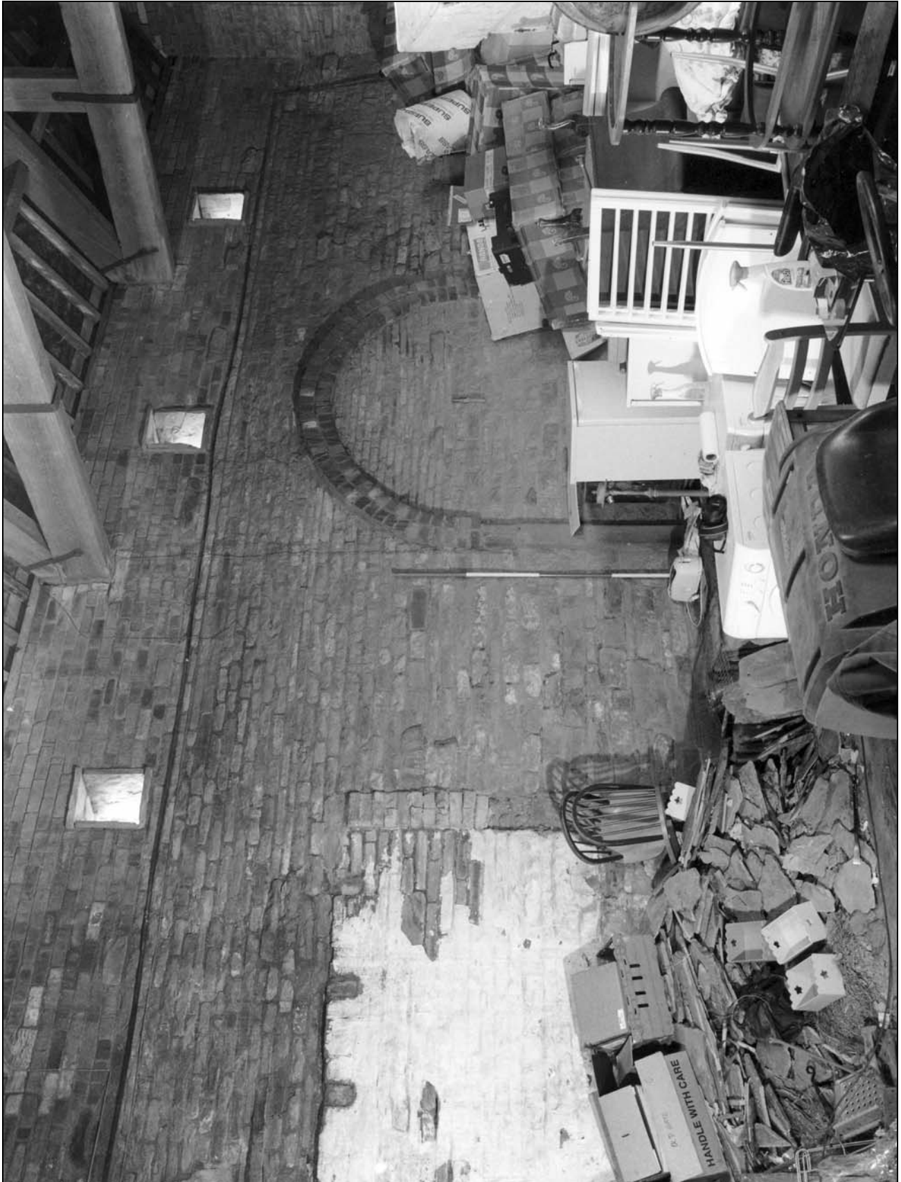
Photo 17: Building 1 (barn): interior, from the north-east corner, showing blocked cart entrance in south wall (film 3, frame 13)
