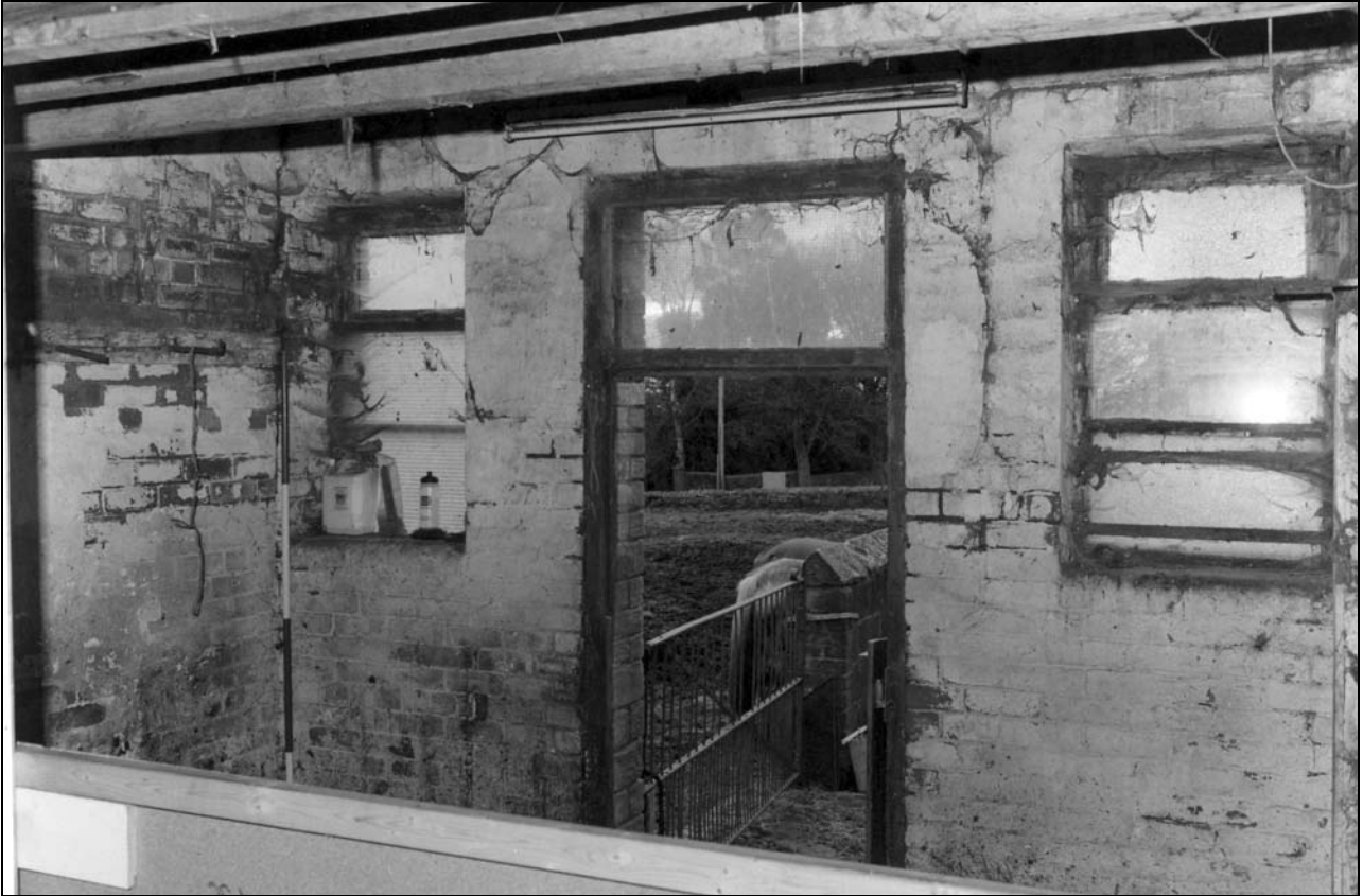
Photo 44: Building 4: interior, from the south-west (film 3, frame 8)
