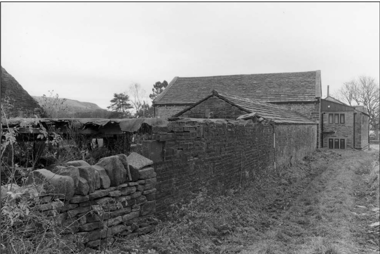
Photo 27: Buildings 1, 2 and 3 from the north-west (film 2, frame 6)
