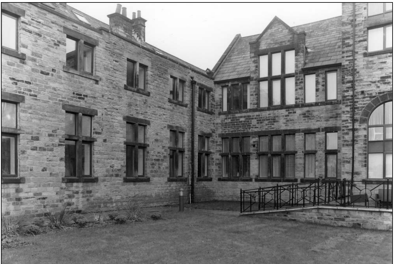
Photo 27: General view of the rear of the school, from the north-east (film 3, frame 8)
