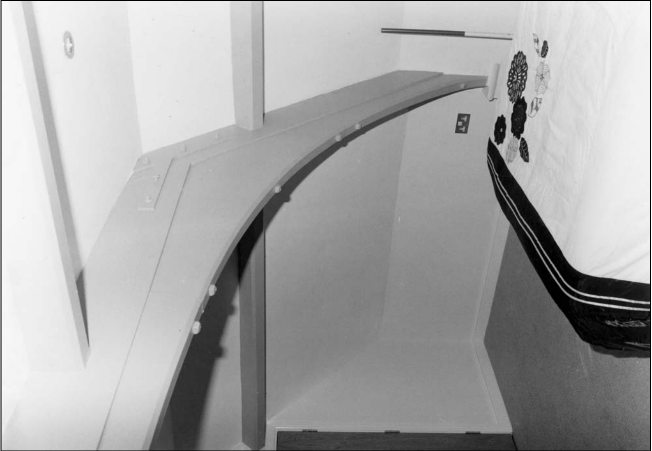
Photo 45: Part of exposed roof truss over south wing (film 4, frame 5)
