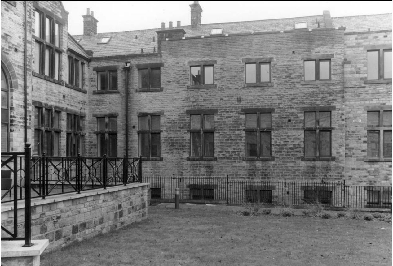
Photo 35: General view of the north wing, from the south (recently extended at right) (film 3, frame 4)
