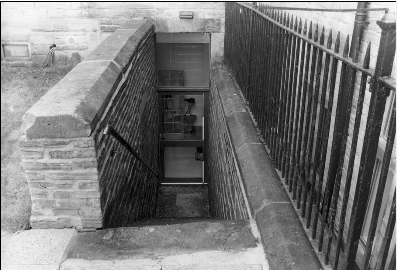
Photo 37: Steps down to basement at north end of school, from the east (film 3, frame 5)
