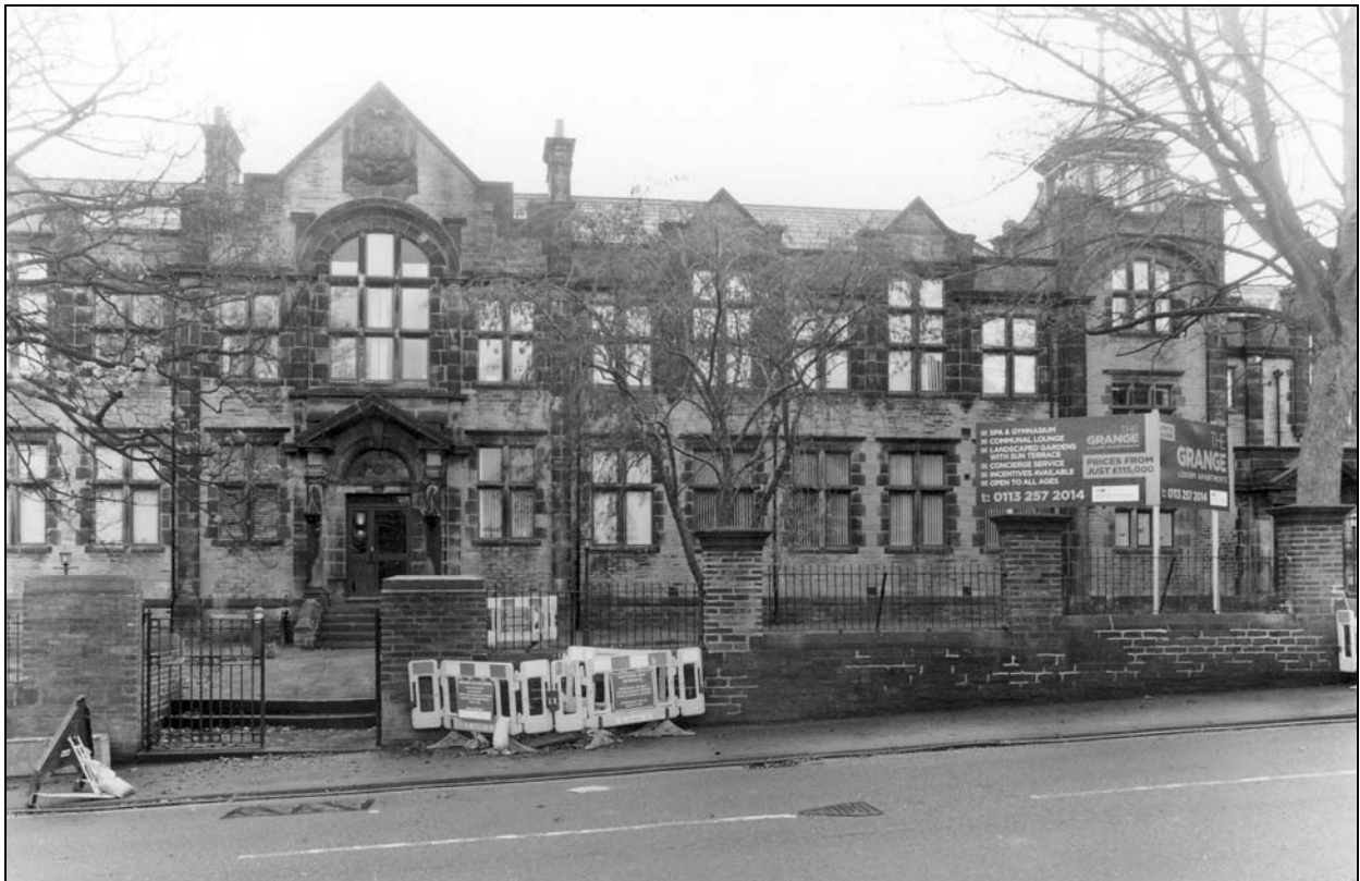
Photo 4: General view of the school, from the west (film 1, frame 7)
