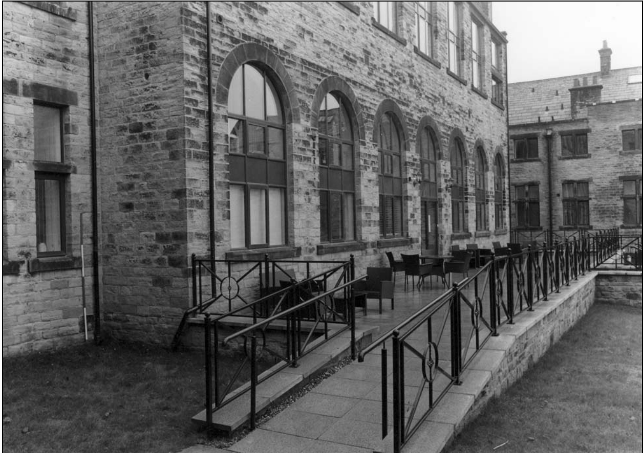
Photo 22: Rear of main block, from the south-east (film 3, frame 7)
