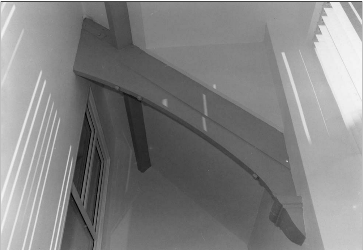
Photo 44: Part of exposed roof truss over south wing (film 4, frame 6)
