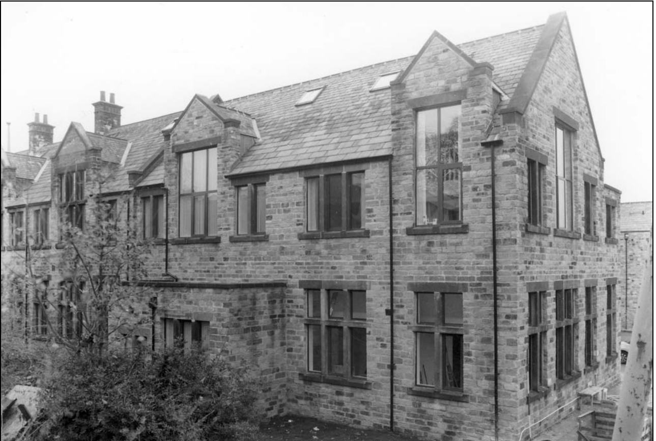
Photo 28: The south wing, from the south-east (modern extension in foreground) (film 3, frame 15)
