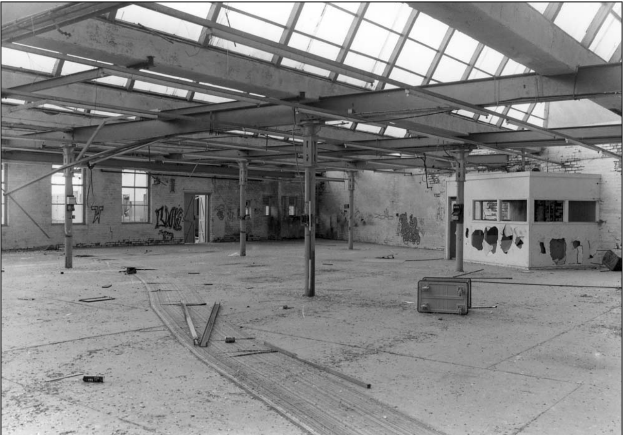
Photo 28: Interior of phase three weaving shed, from the south-west (film 2, frame 10)
