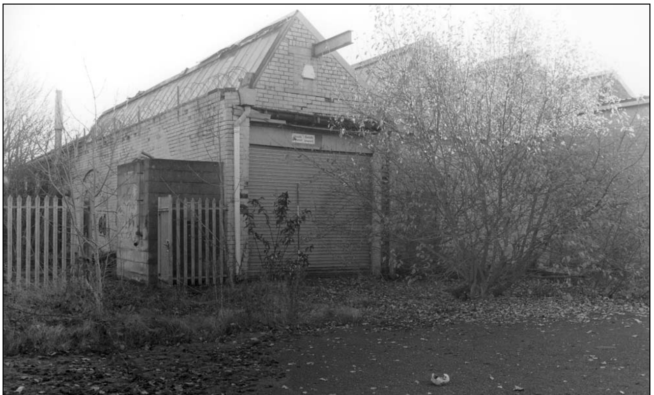
Photo 29: Phase four weaving shed, from the north-west (film 2, frame 15)
