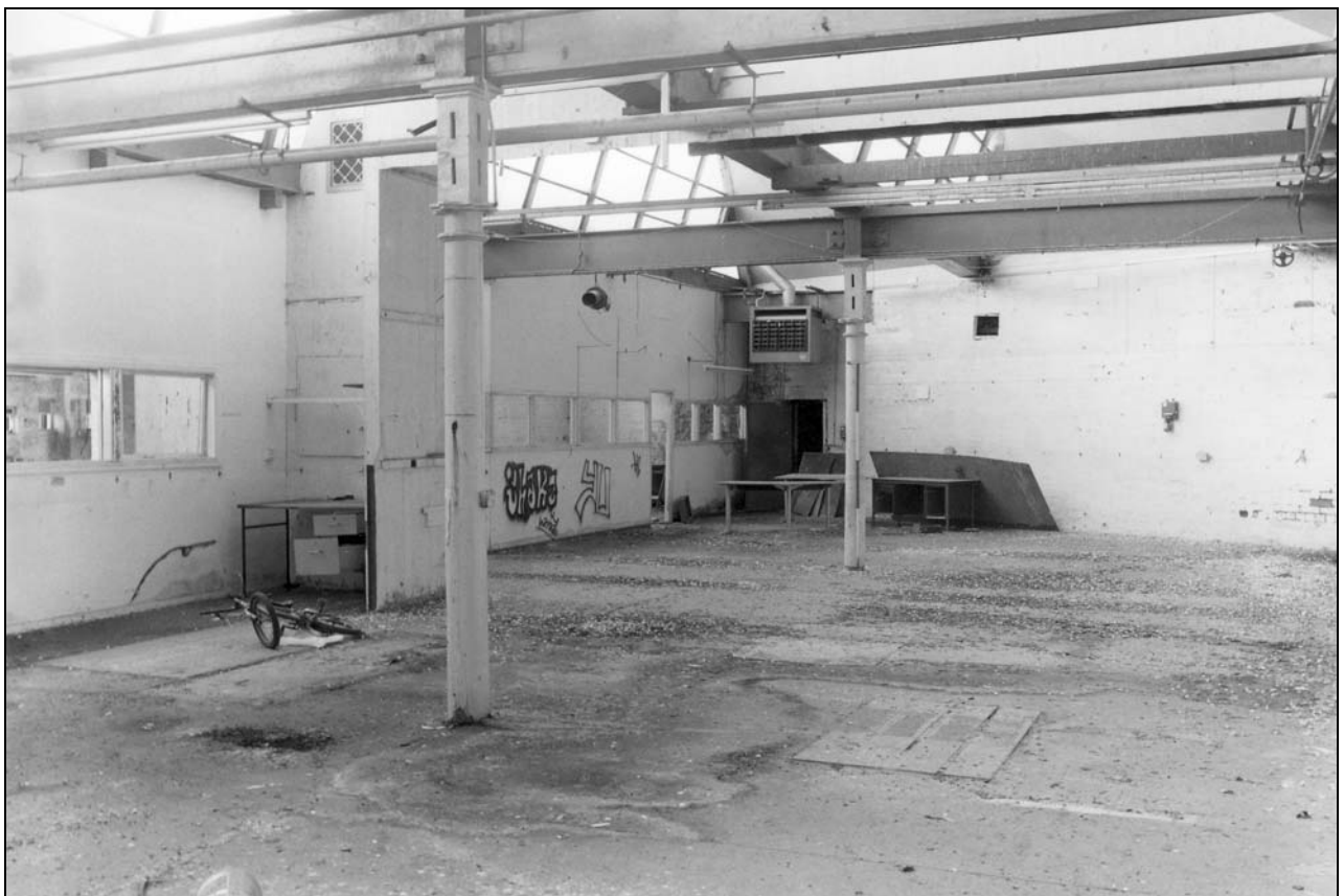
Photo 27: Interior of phase two weaving shed, from the west (film 2, frame 8)
