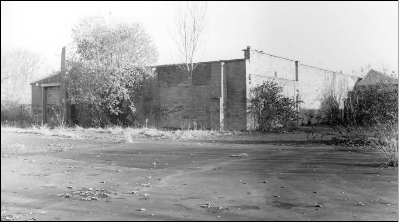
Photo 22: Late nineteenth century weaving shed, from the south-west (film 2, frame 13)
