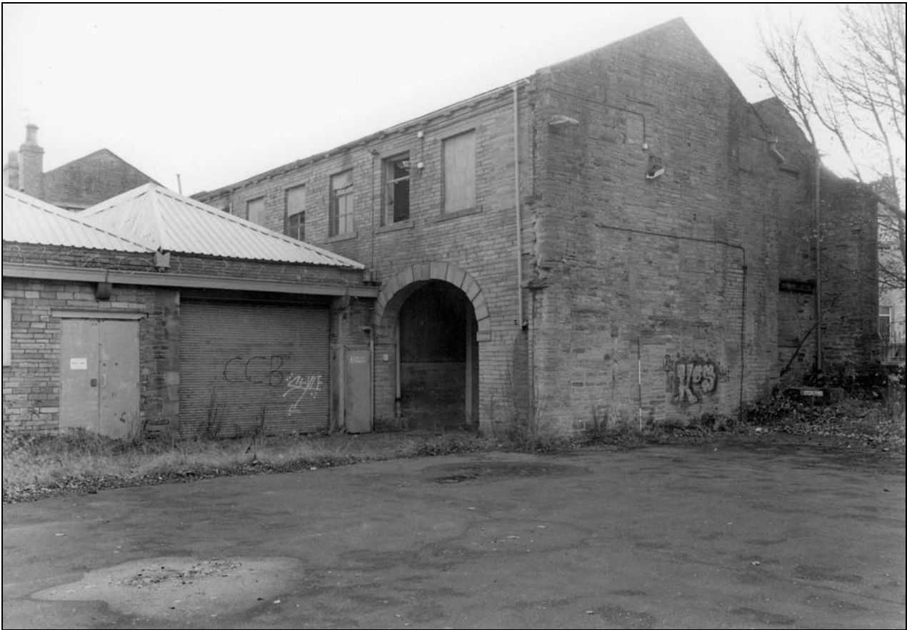
Photo 15: General view of two storey block, from the north-west (film 1, frame 17)
