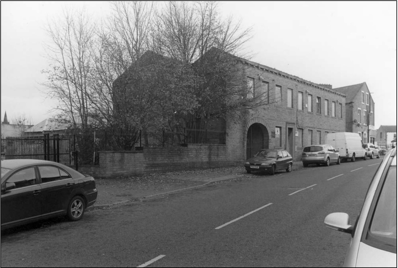
Photo 8: General view of the site, from the south-west (film 1, frame 13)
