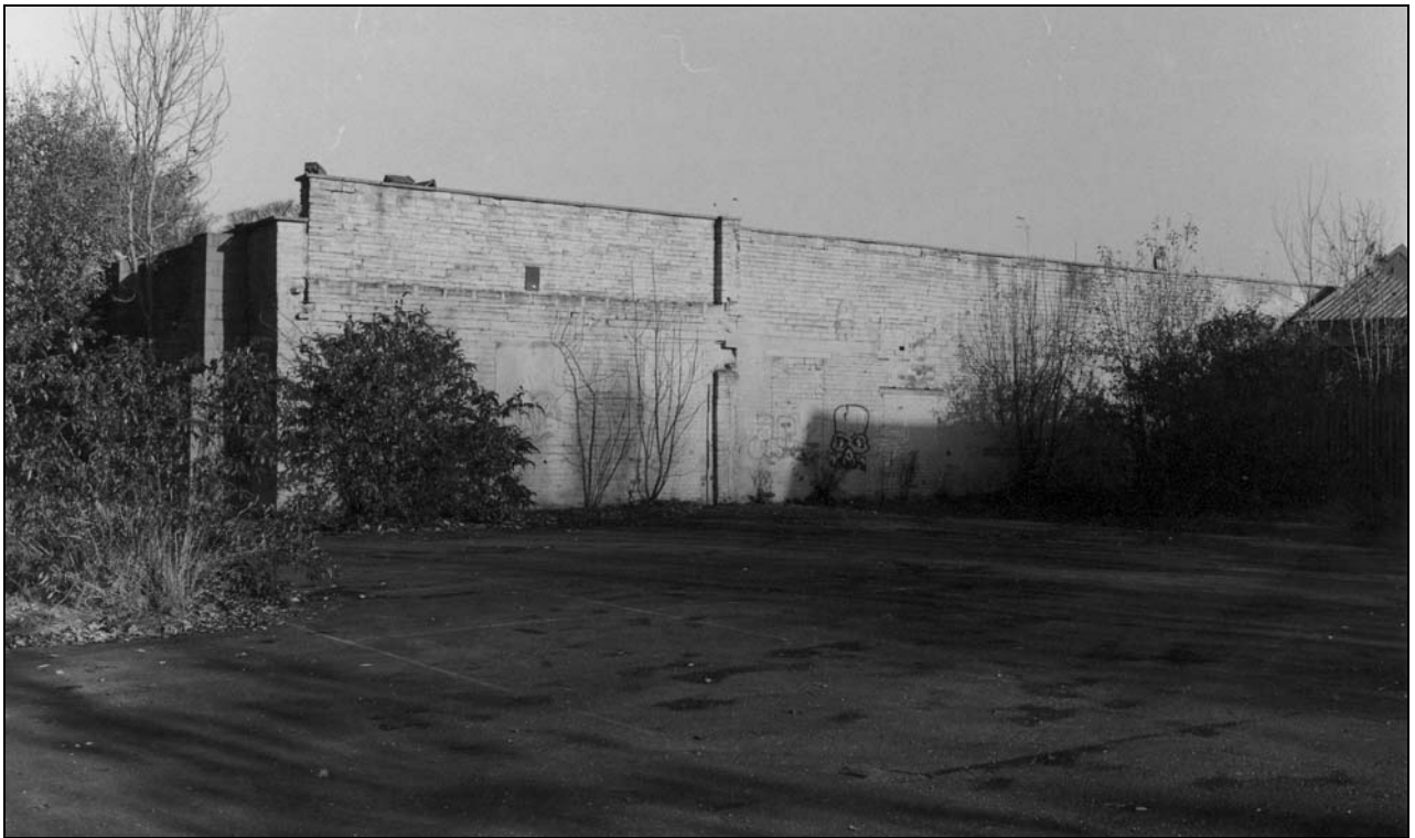
Photo 21: Late nineteenth century weaving shed, from the south-west (film 2, frame 17)
