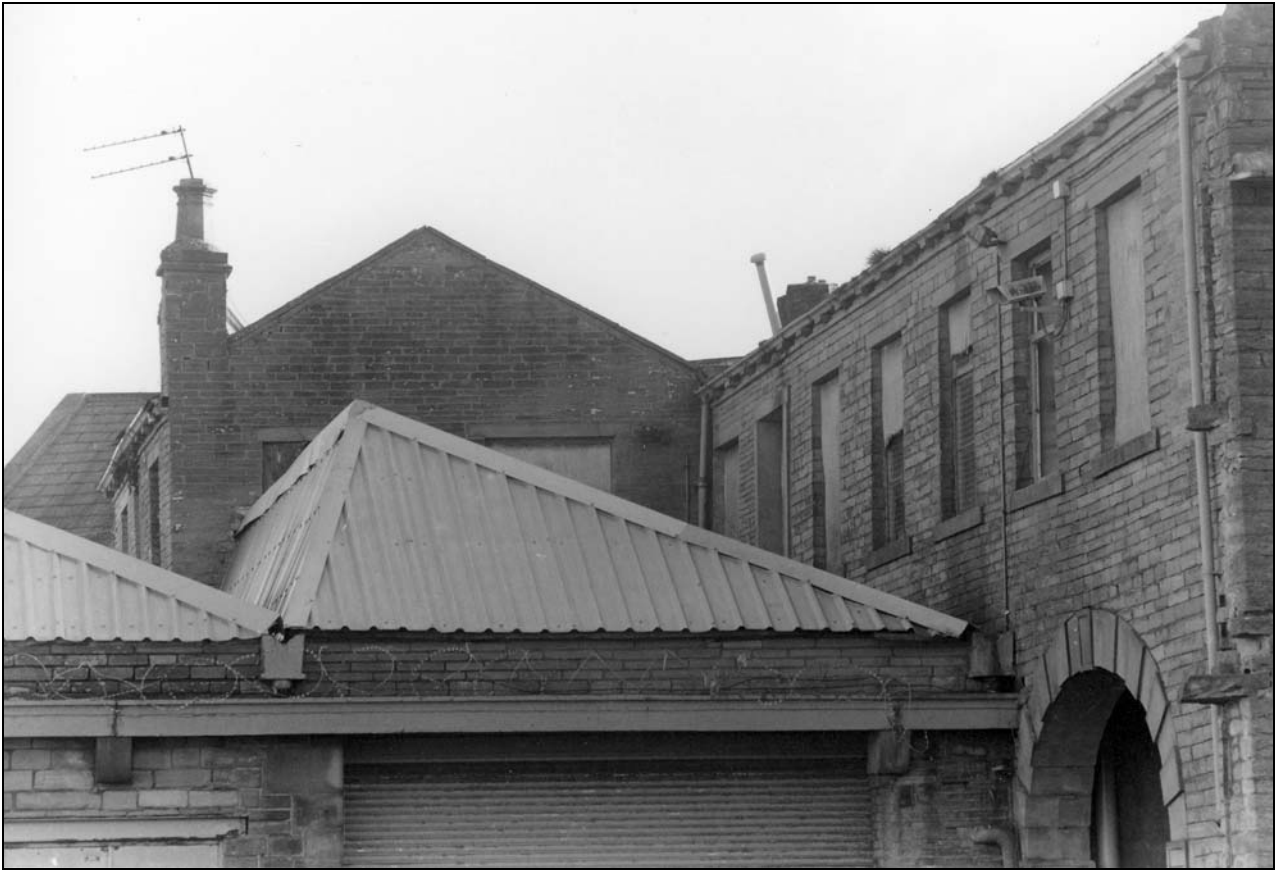
Photo 17: Rear elevation of two storey block, from the north-west (film 2, frame 18)
