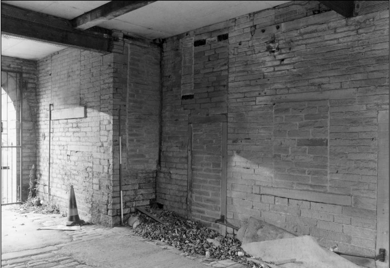
Photo 18: Covered passage through two storey block, from the north-east (film 2, frame 1)
