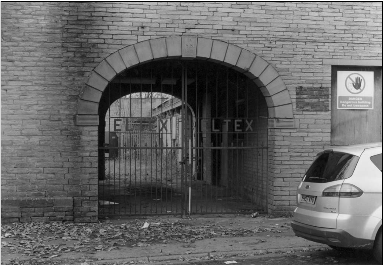
Photo 5: Arched entrance to covered passage through two storey block, from the south (film 1, frame 8)
